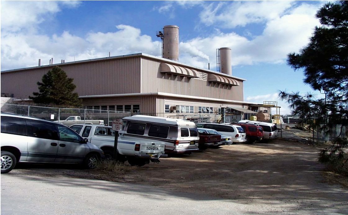
Figure 2-1. Main Steam Plant at LANL TA-3.
