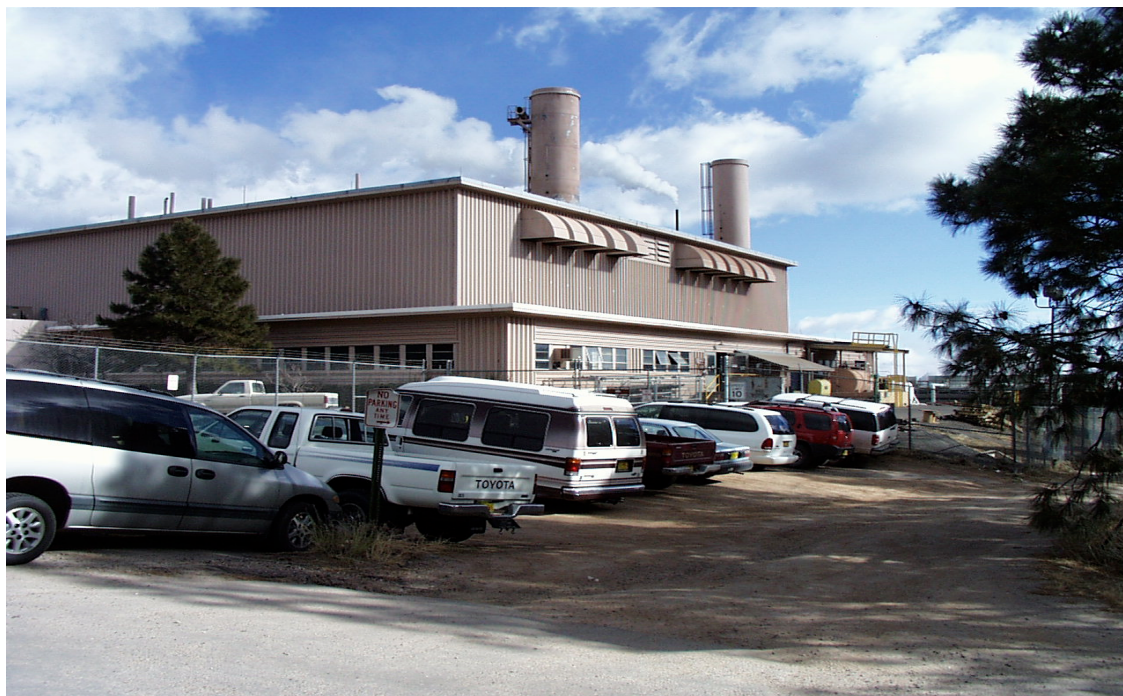
Figure 2-1. Main steam plant at LANL TA-3.
