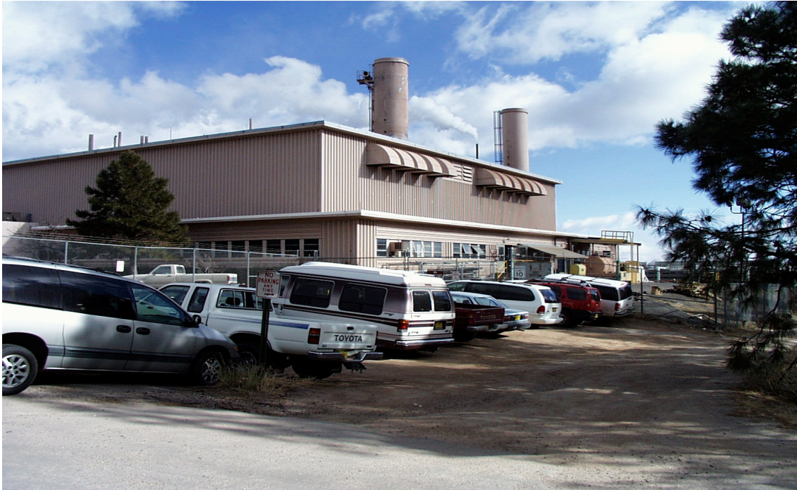
Figure 2-1. Main steam plant at LANL TA-3.
