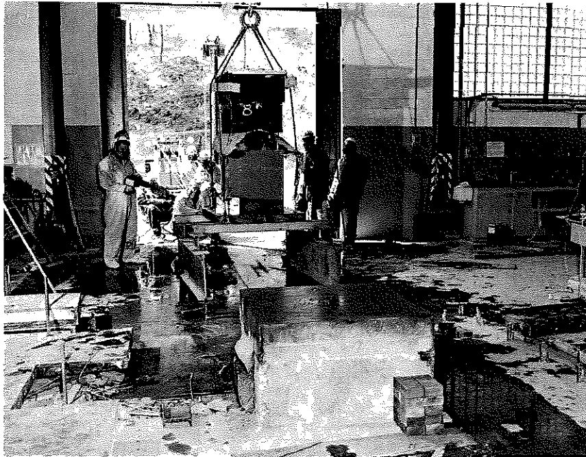
Figure 26. Removal of Reactor, circa 1953
