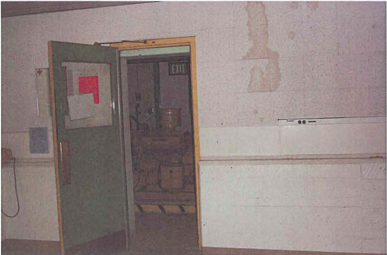
TA-2-1, Rooms 116 & 116A
