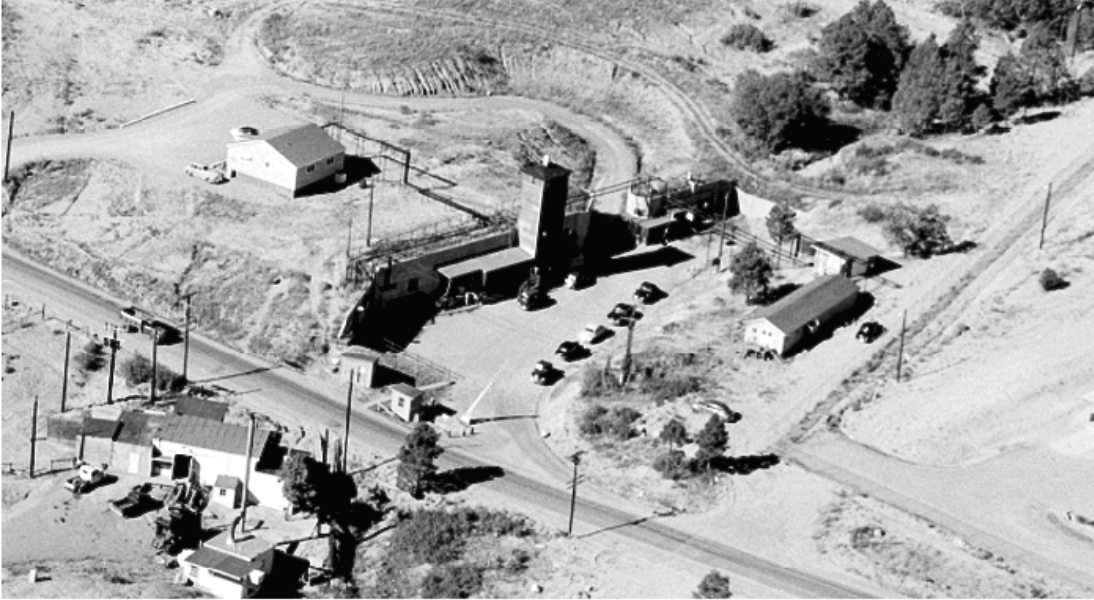
Figure 15.5. Anchor Ranch Proving Ground.
