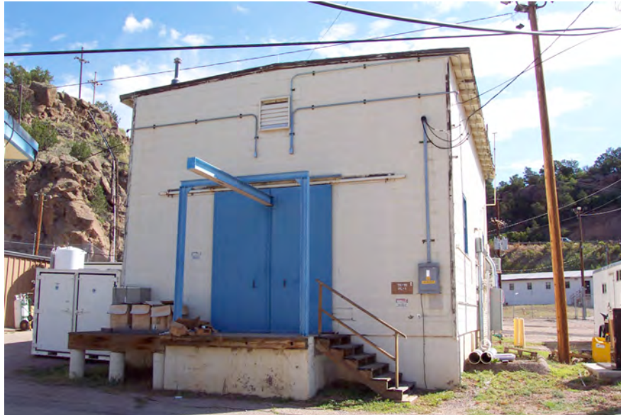
Figure 15.9. Building 18-1, site of a fatal criticality accident.
