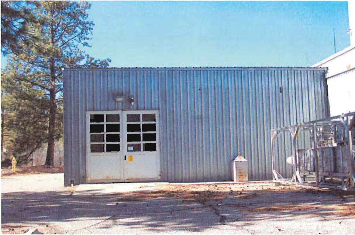
TA-3-16, East elevation, photo 7
