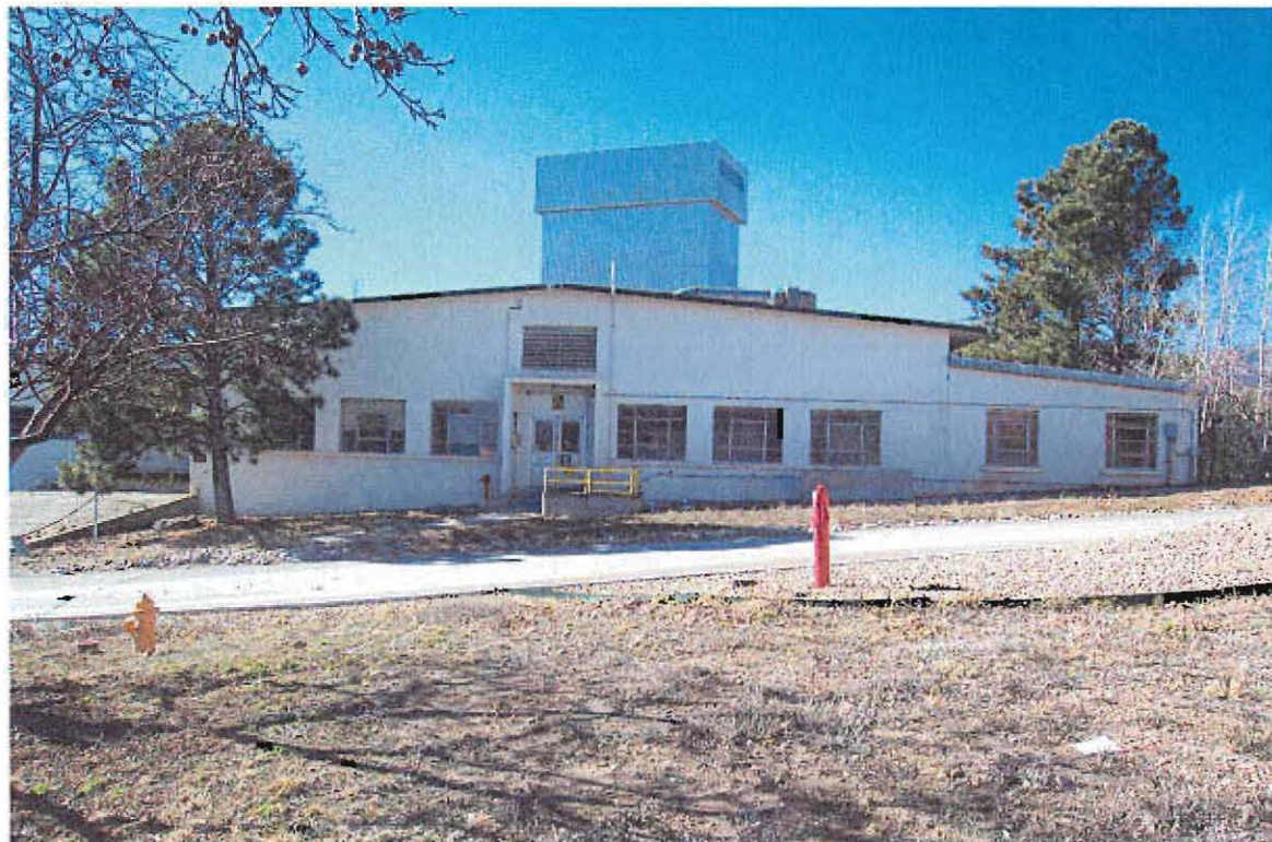
Figure 2. TA-3-16, Front Entrance (office portion)
