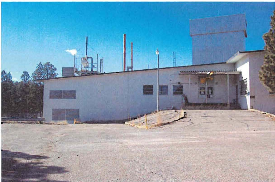
TA-3-16, East elevation, south half, photo 2
