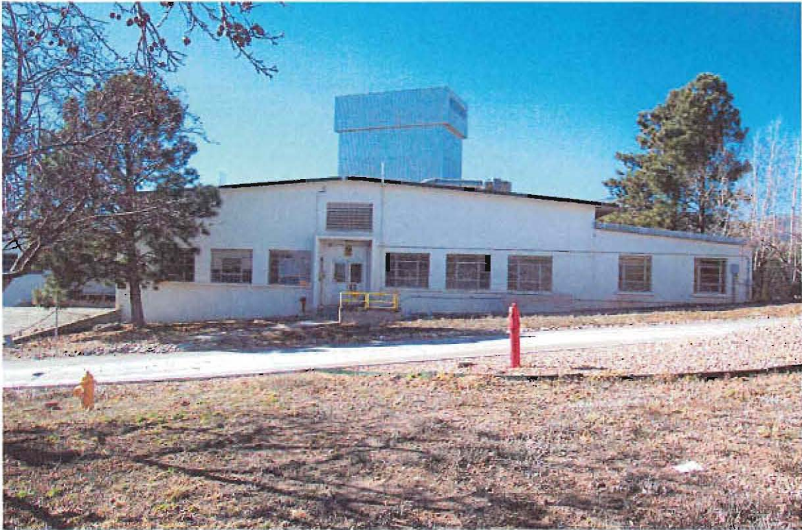
TA-3-16, East elevation, north half, photo 1
