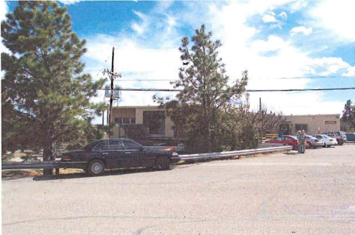
TA-8-21, North side
