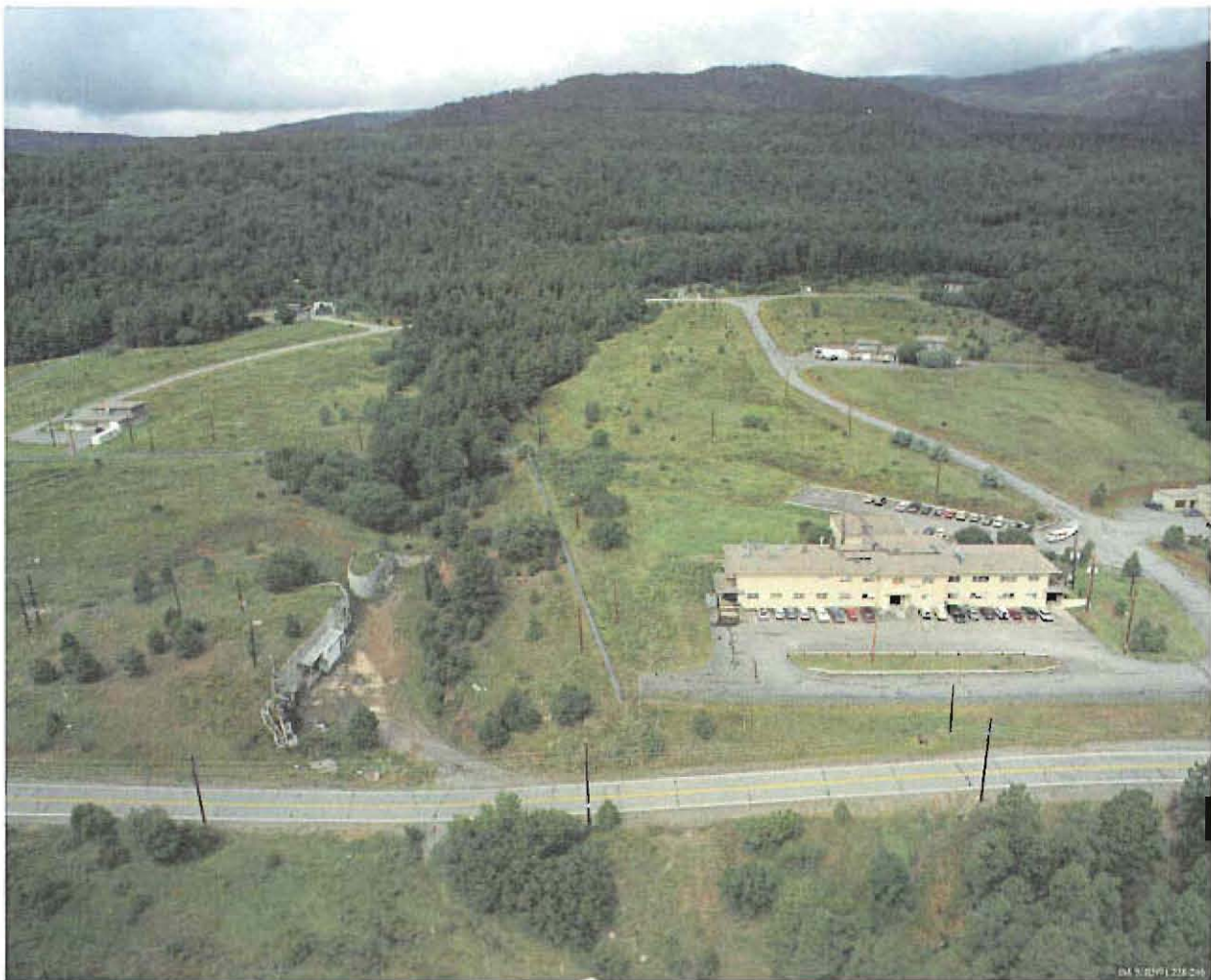
Figure 1. 1991 Aerial of TA-8
