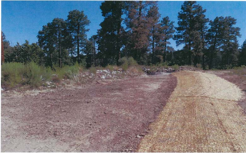
E00105020013 Sediment traps and basins—sediment basin
