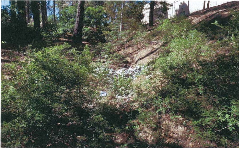
E00106010023 Check dam—rock check dam
