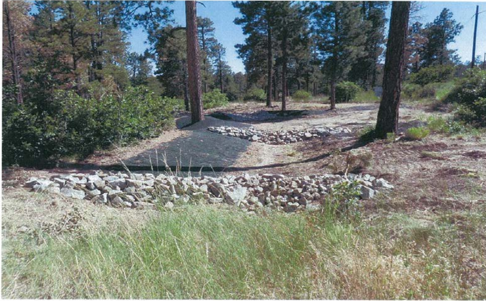
E00103010014 Berms—earthen berm
