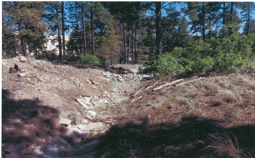
E00106010021 Check dam—rock check dam
