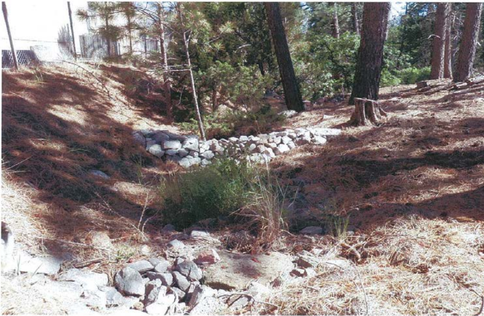
E00106010025 Check dam—rock check dam
