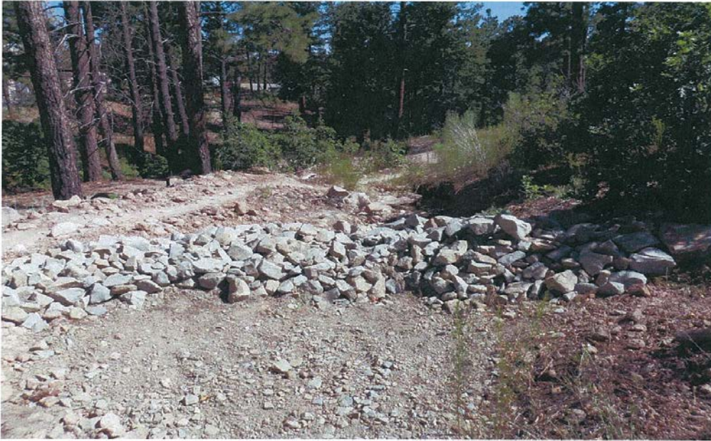
E00106010022 Check dam—rock check dam
