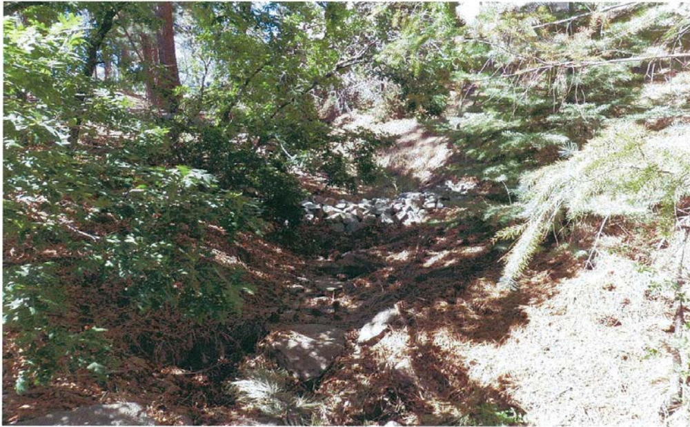
E00106010024 Check dam—rock check dam
