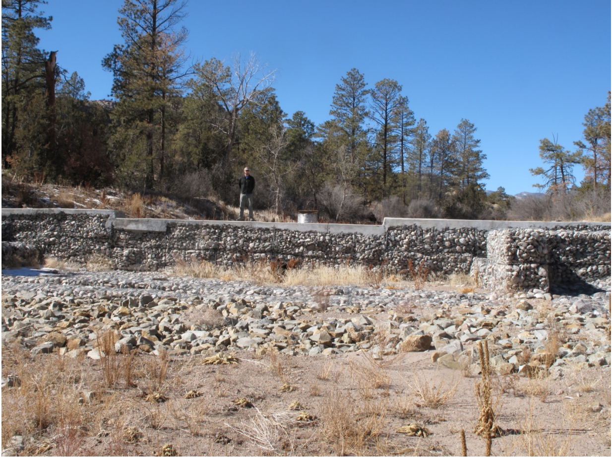
Photo A1-10 February 2013 photograph of the Pueblo Canyon CGS, looking upstream
