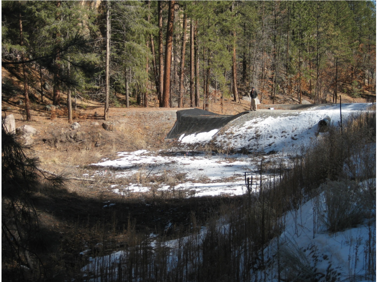
Photo A1-11 February 2013 photograph of the upper sediment retention basin at LA-SMA2, looking downstream
