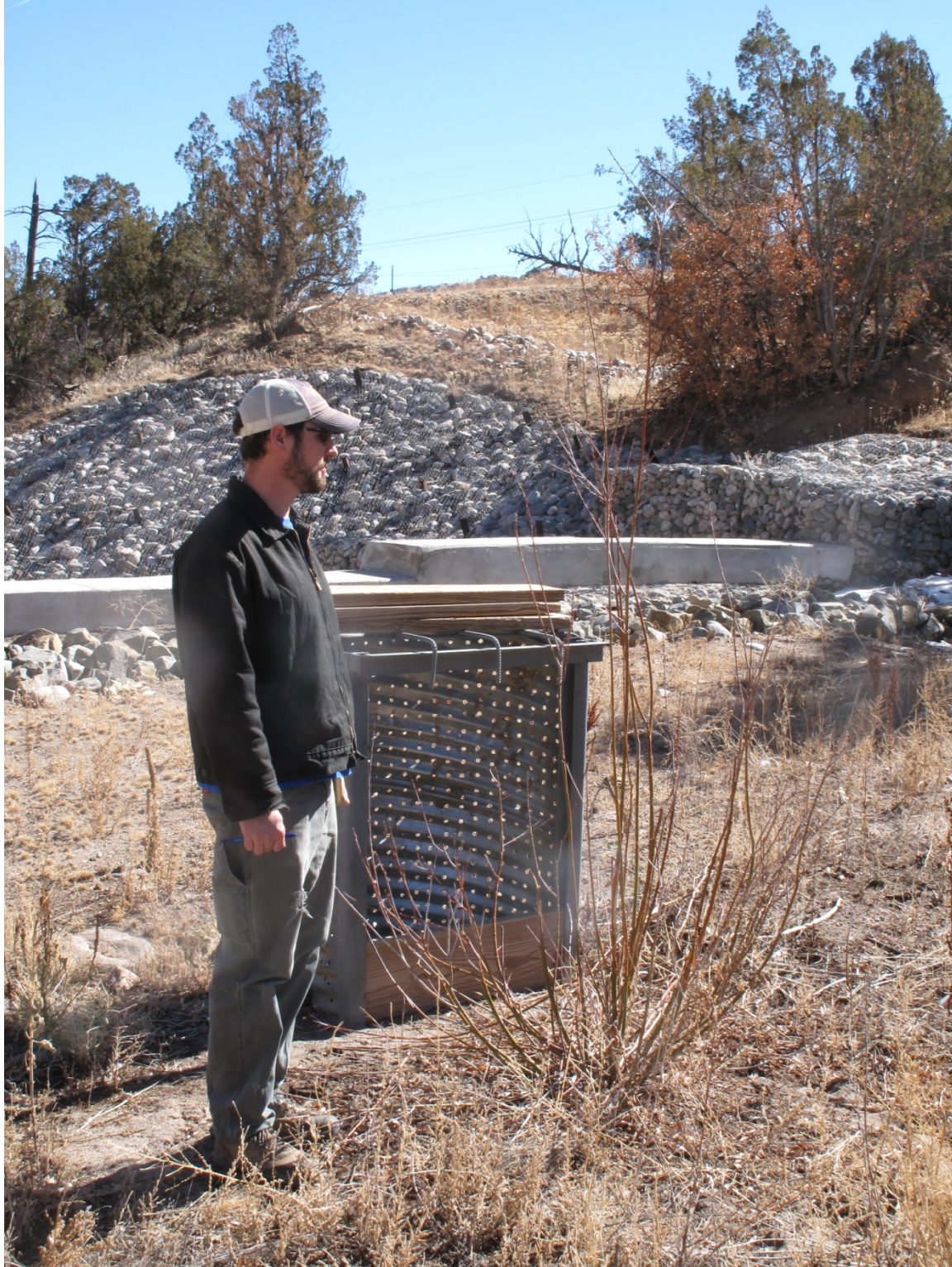
Photo A1-23 February 2013 photograph of the largest observed willow in the Pueblo Canyon GCS willow-planting area, near the GCS inlet
