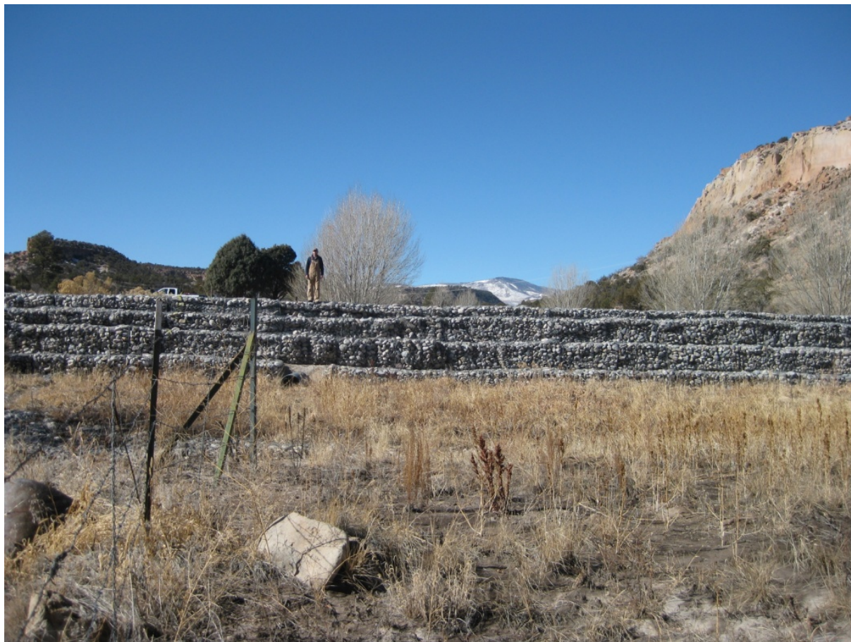
Photo A1-17 February 2013 photograph of the Los Alamos Canyon low-head weir looking upstream
