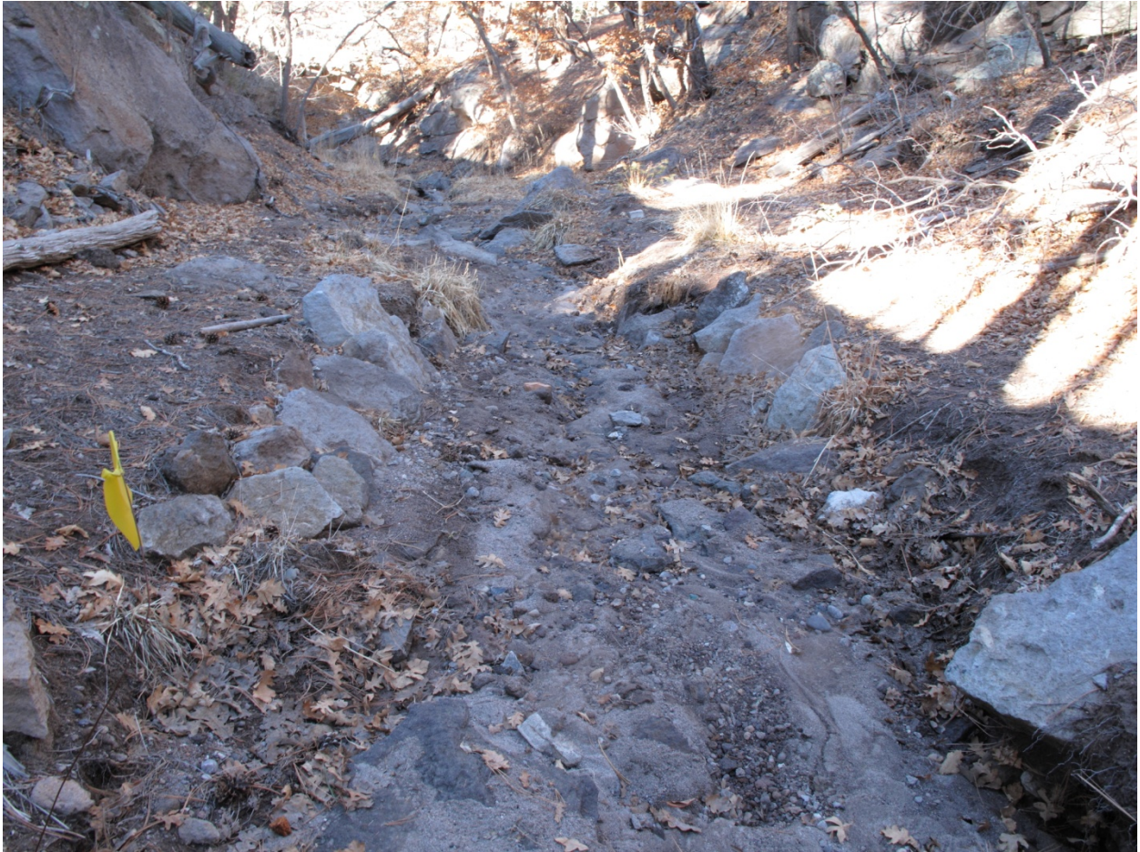
Photo A1-24 February 2013 photograph of rock armoring along stream banks in the south fork of Acid Canyon looking upstream
