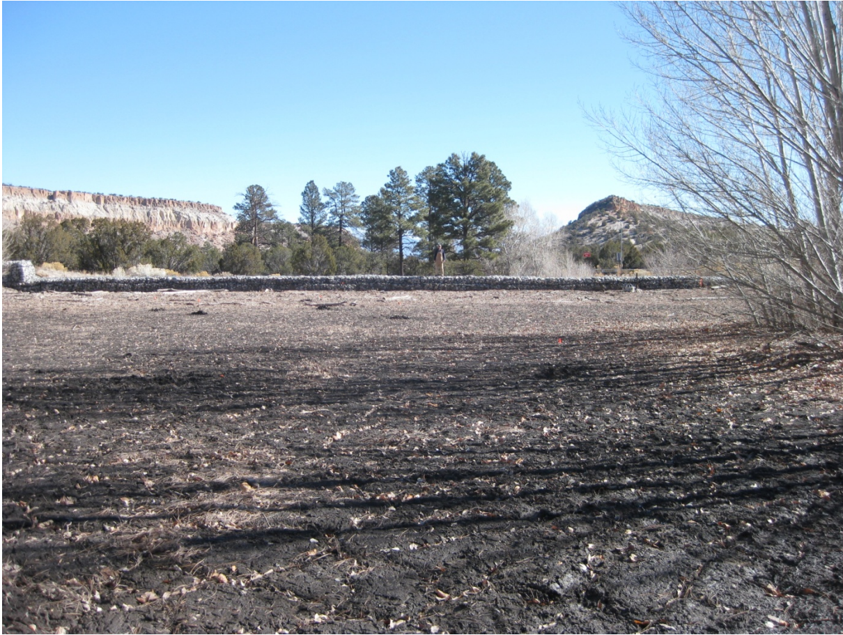
Photo A1-18 February 2013 photograph of sediment accumulation in the lower basin at the Los Alamos Canyon low-head weir
