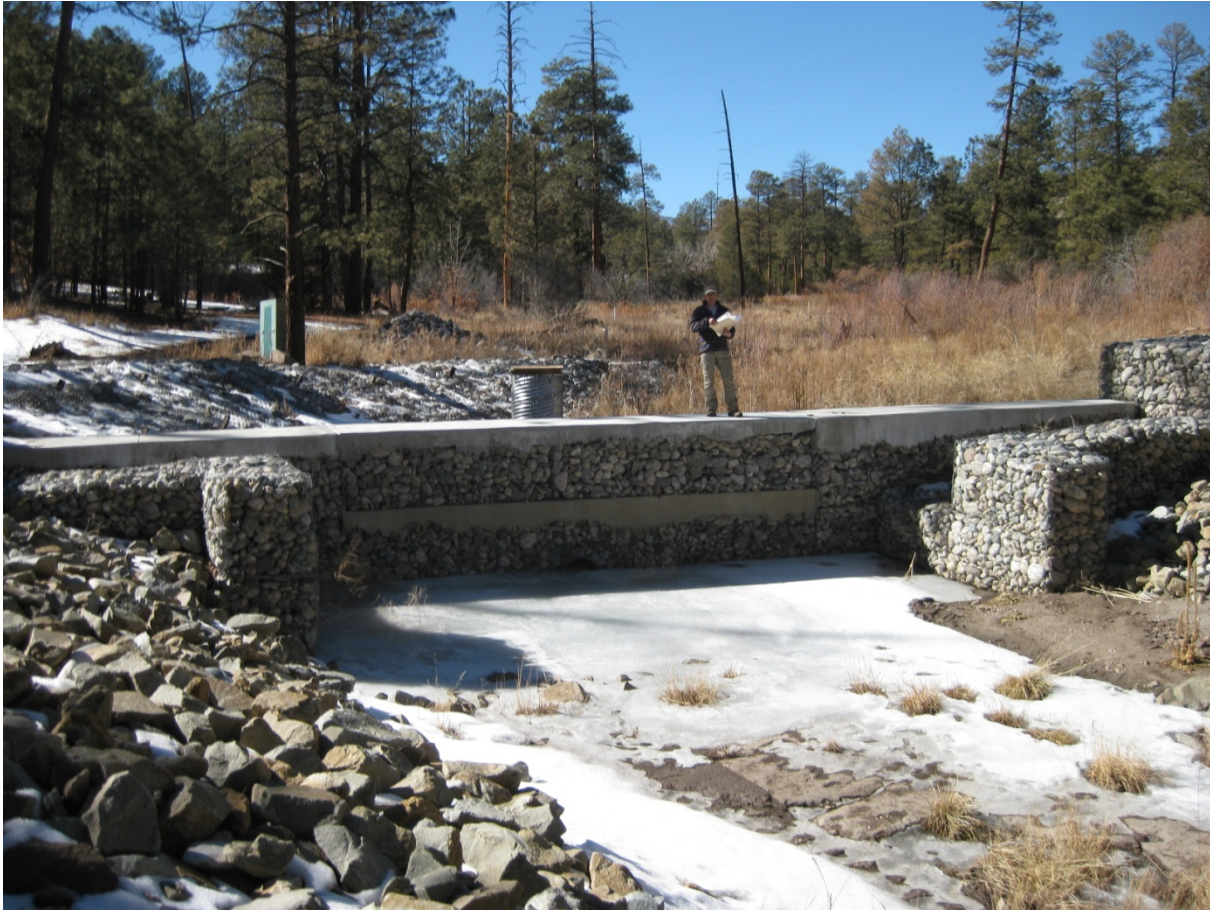
Photo A1-13 February 2013 photograph of the DP Canyon GCS, looking upstream
