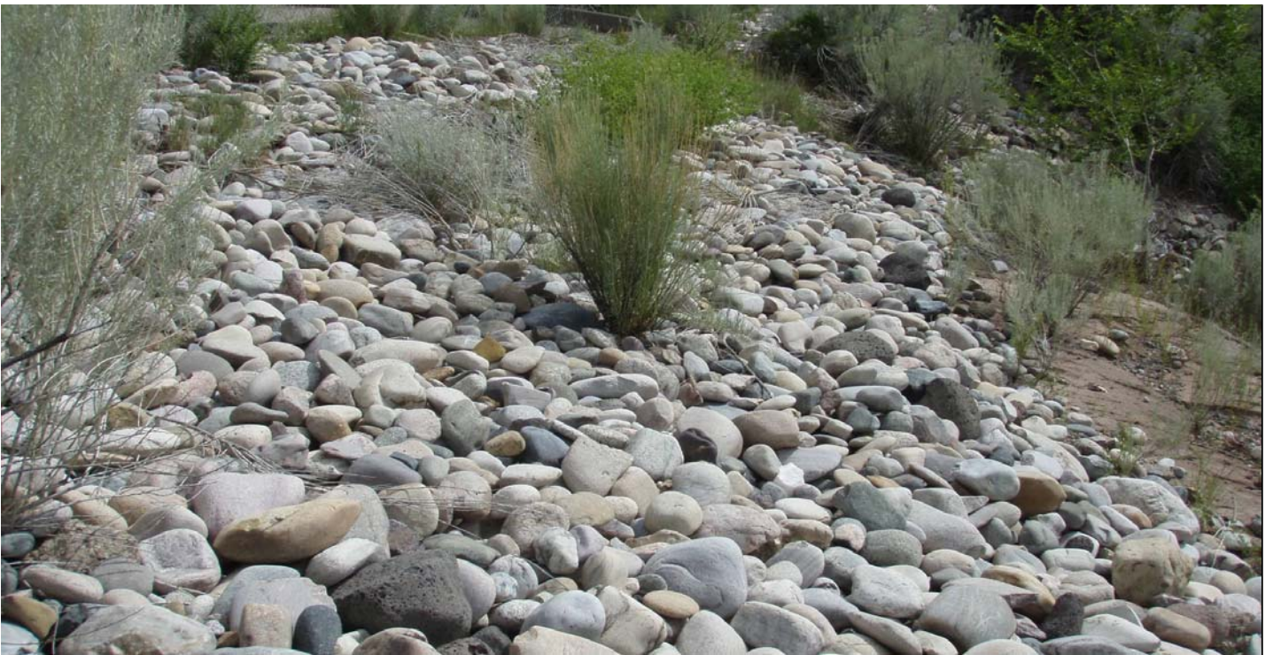
Photo 7600-5.JPG (taken 08/03/10) S00304060010 : Channel/Swale - Rip Rap.
