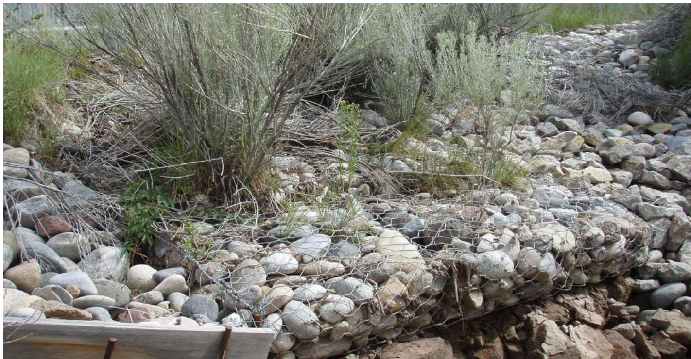
Photo 7600-6.JPG (taken 08/03/10) S00307020006 : Gabions - Gabion Blanket.
