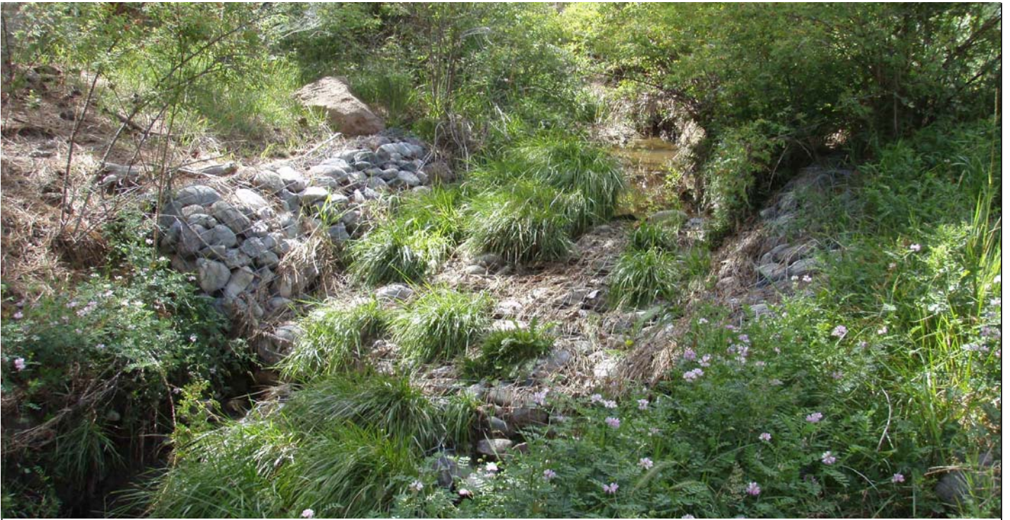
Photo 7599-5.JPG (taken 08/03/10) S00107020003 : Gabions - Gabion Blanket.
