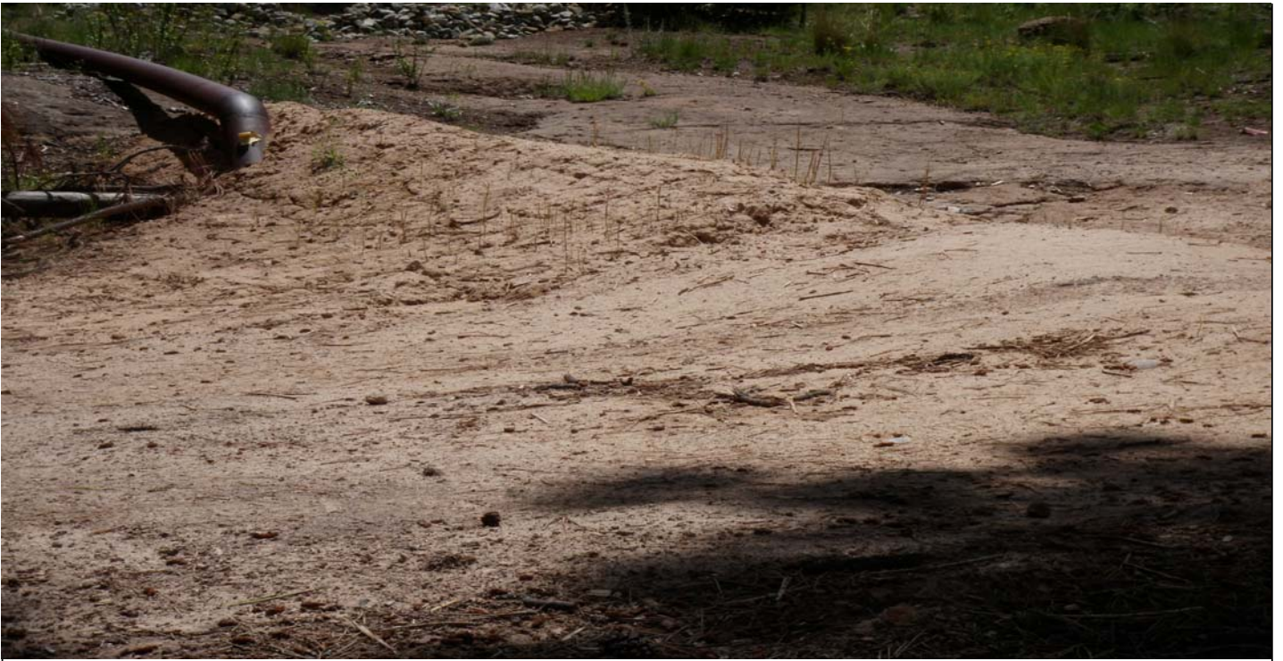
Photo 7465-5.JPG (taken 08/06/10) M01003010004 : Berms - Earthen Berm.
