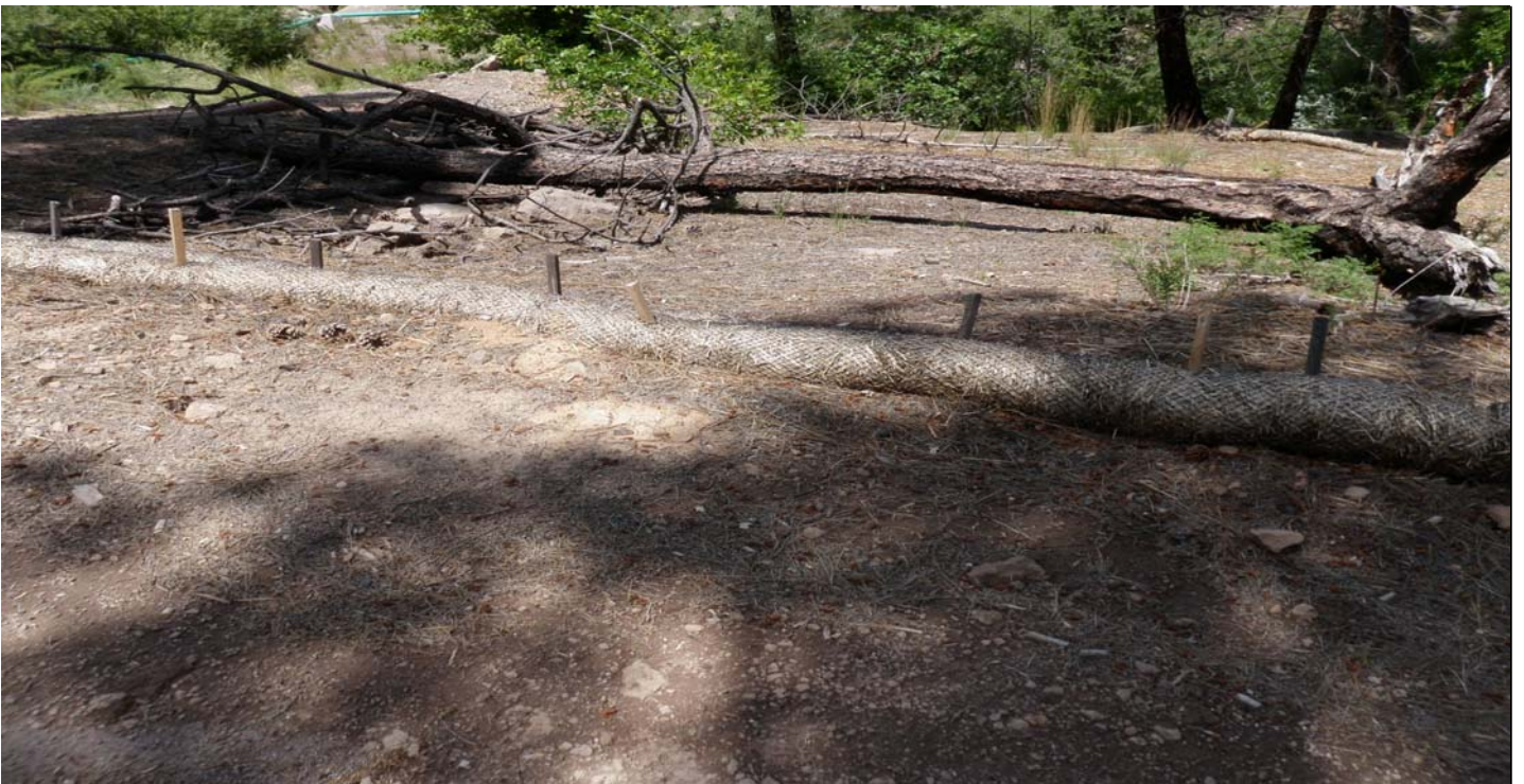
Photo 7465-3.JPG (taken 08/06/10) M01003060007 : Berms - Straw Wattles.
