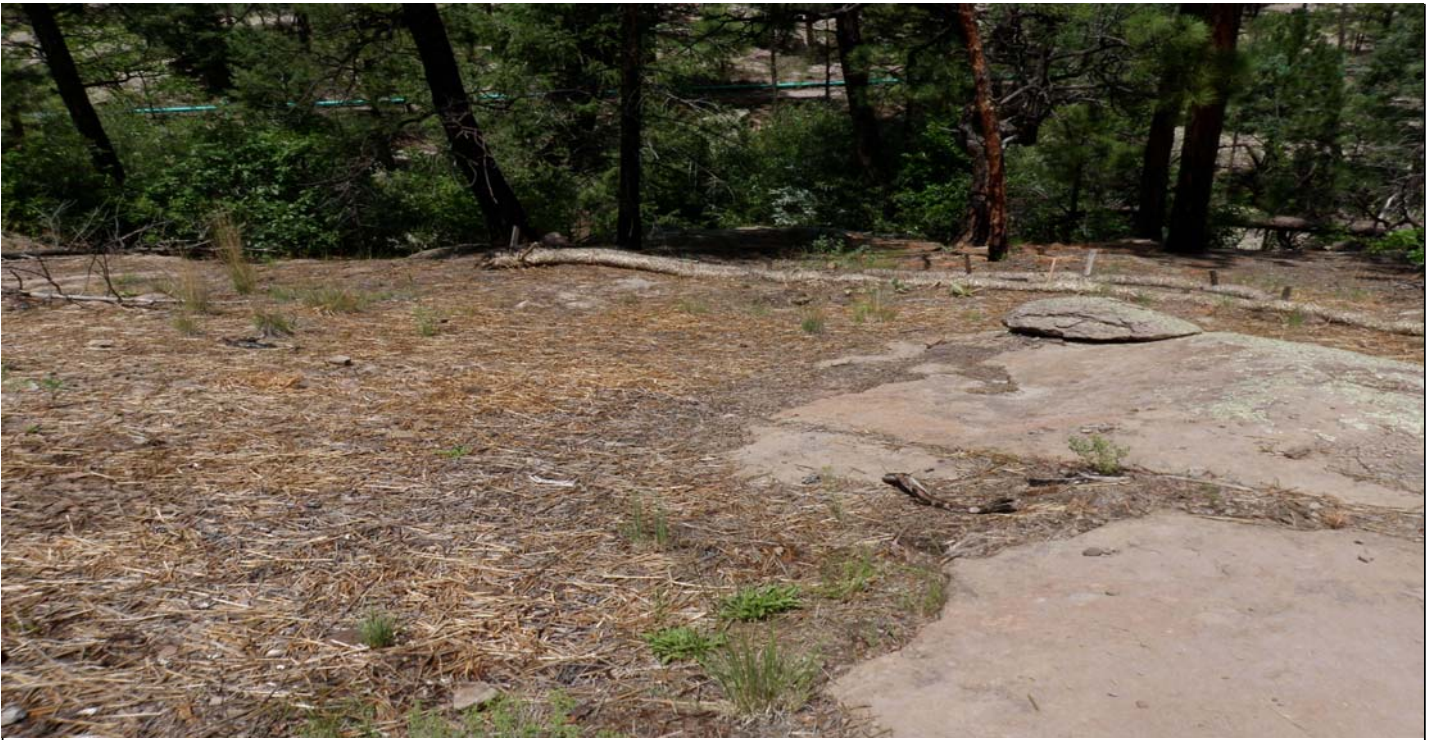
Photo 7465-2.JPG (taken 08/06/10) M01001010001 : Seed and Mulch - Seed and Wood Mulch; M01003060008 : Berms - Straw Wattles.
