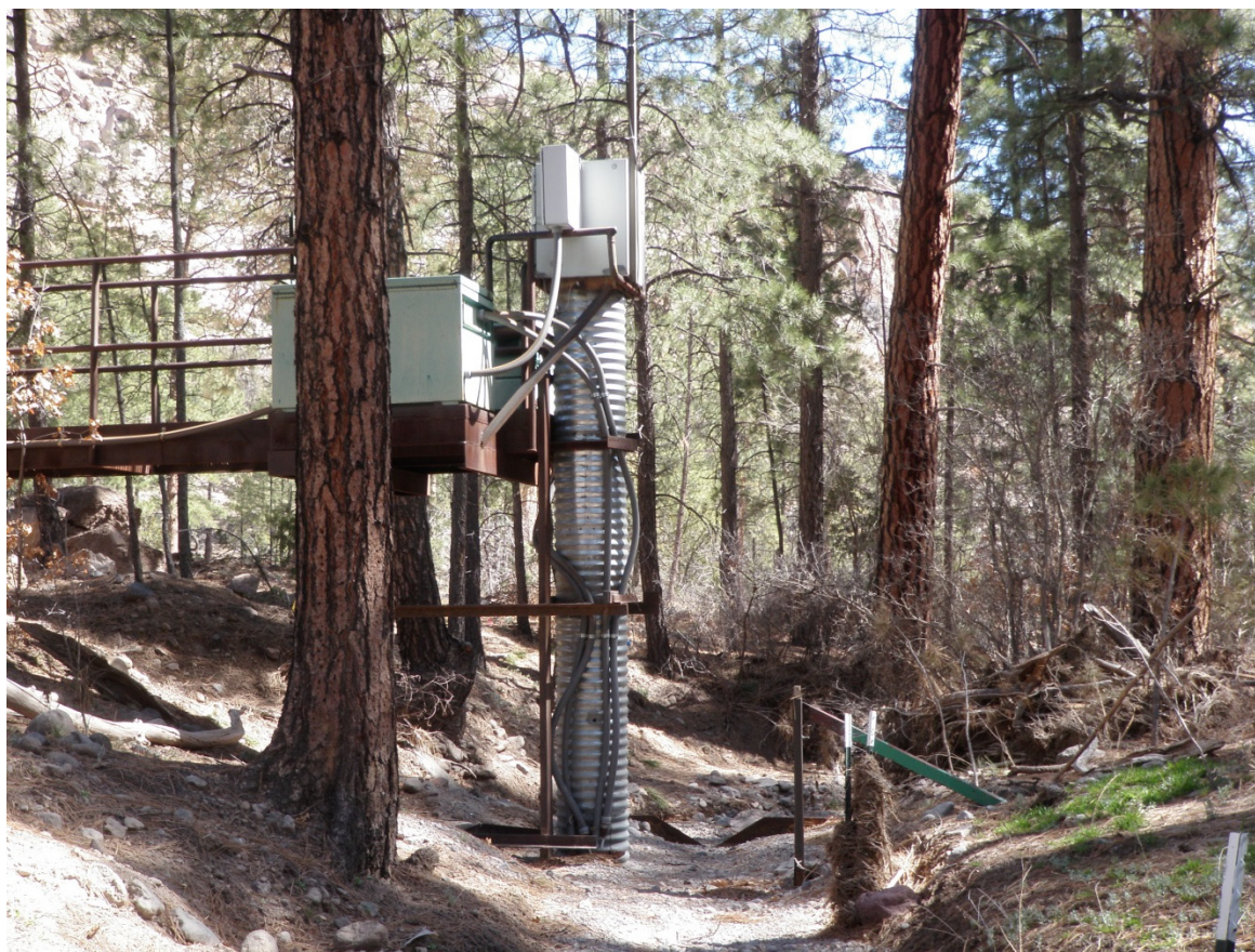
E030 Stream gage downstream view
