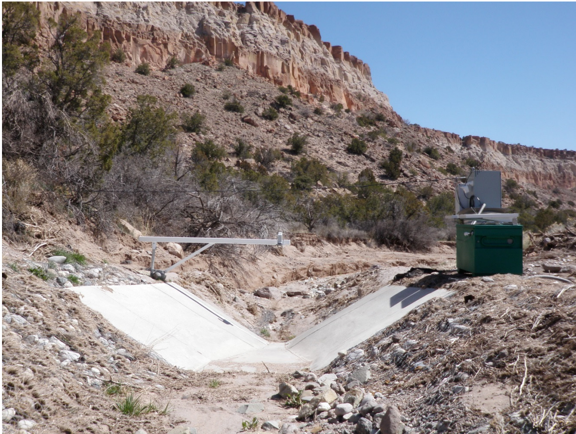
E060.1 Stream gage downstream view
