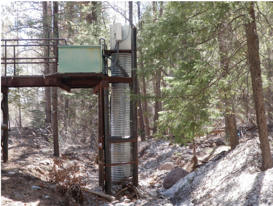
E026 Stream gage downstream view
