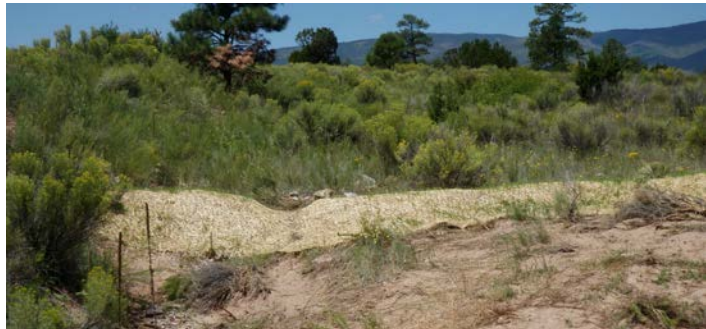
3M-SMA-0.4, Earthen Berm, H00203010003 (photo ID 8517-1)
