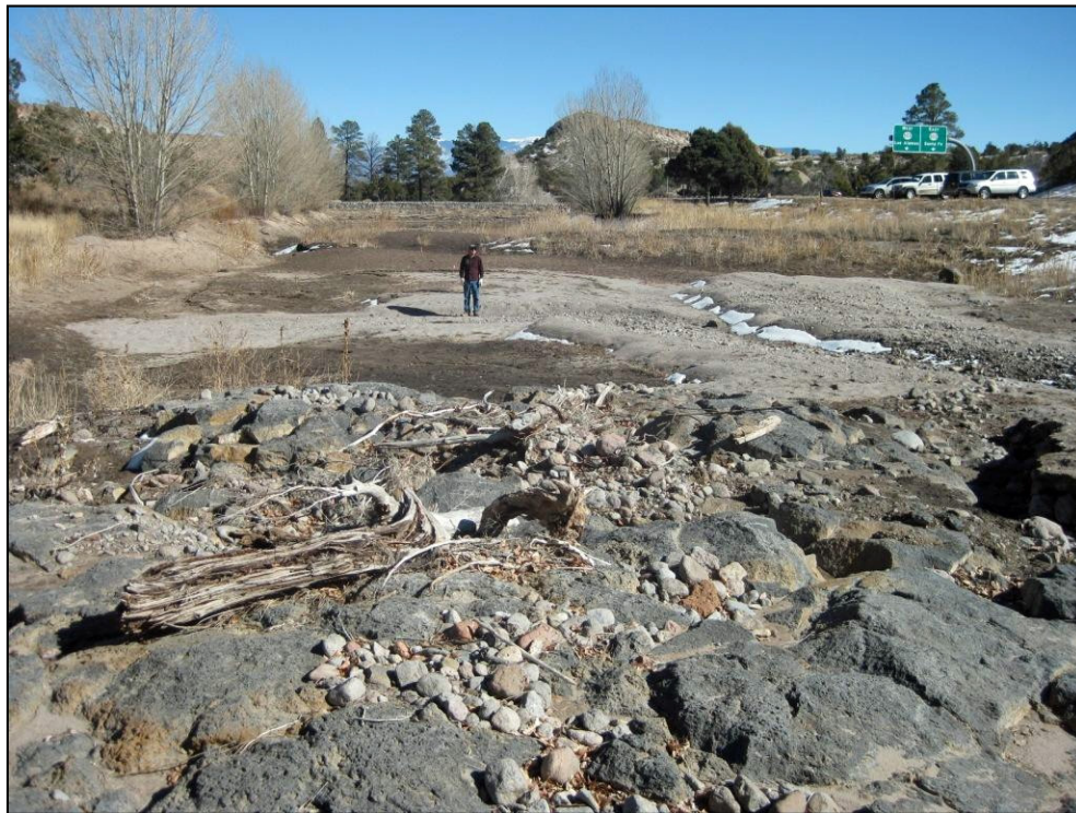
Photo A1-15 January 2015 photograph of sediment accumulation and delta in Basin 2 at the LA Canyon Los Alamos Canyon low-head weir; Basin 3 is visible in the background.
