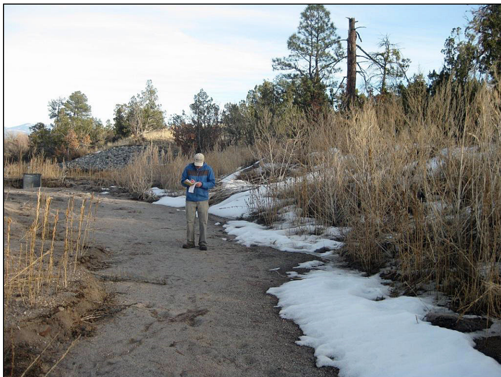
Photo A1-8 February 2015 photograph of area of maximum sediment erosion above the Pueblo Canyon grade-control structure, PUGCS-100, looking downstream. Surface likely modified during excavation of the intake above the PUGCS.
