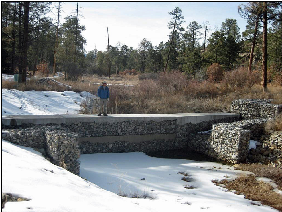
Photo A1-11 February 2015 photographs of the DP Canyon grade-control structure: (a) looking downstream (b) looking upstream
