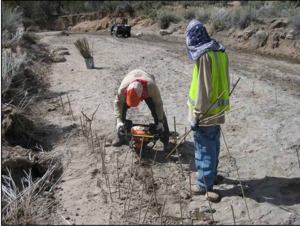
Figure B-2.1-1 Stihl BT 121 auger planting at Coir Bank 2, April 17, 2014
