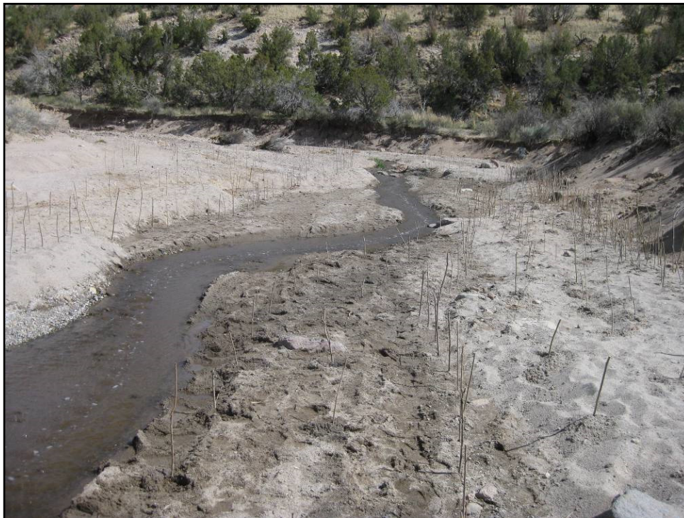
Figure B-2.2-2 Bank 3 (back left) and Bank 4 (front right) with coir Bank 2 shown at the edge of the right of the photo. Note stream channel, overbank, and coir bank willow spacing in RA-2, April 17, 2014.
