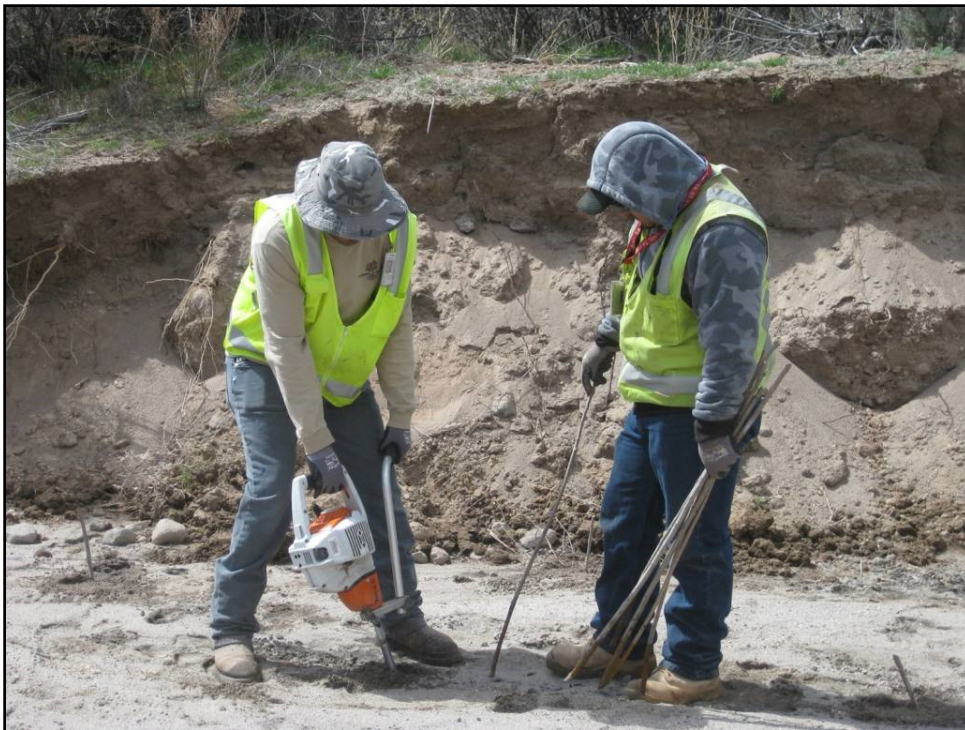
Figure B-2.1-1 Stihl BT 121 auger planting at Coir Bank 2, April 17, 2014
