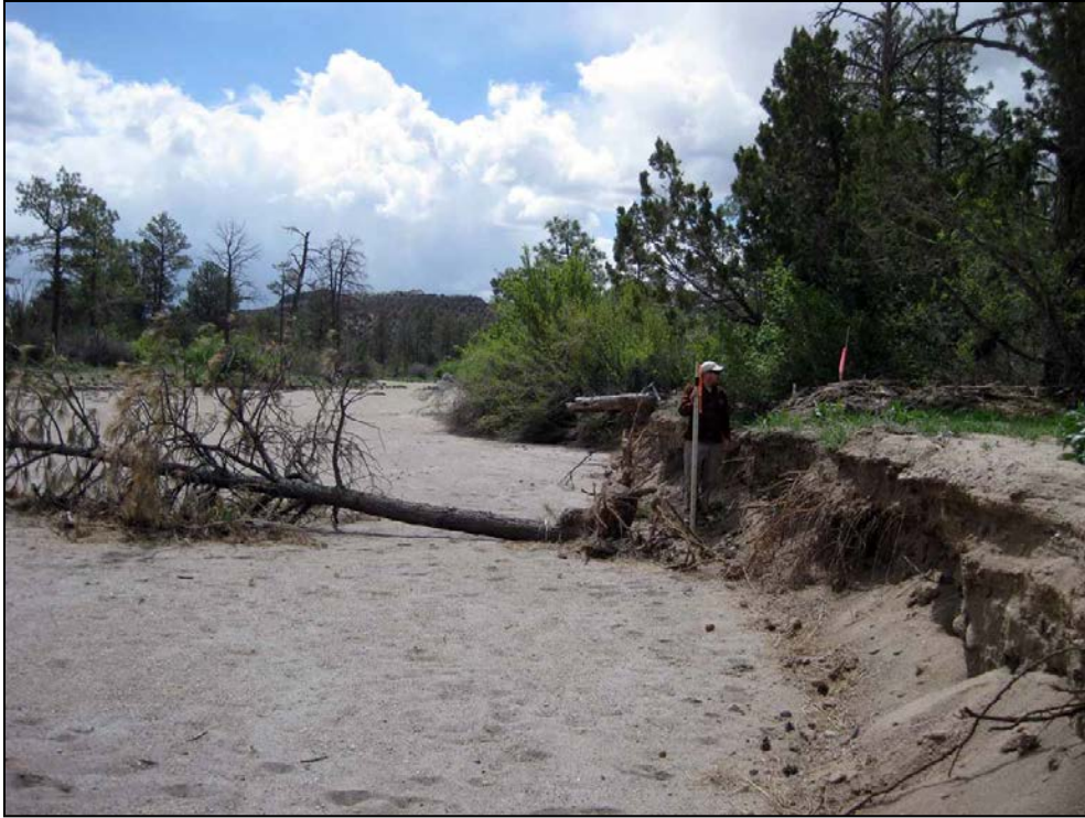
Photo A1-15 May 2014 photograph of area of maximum sediment erosion above the Pueblo Canyon grade-control structure, PUGCS-1400 ft, looking downstream
