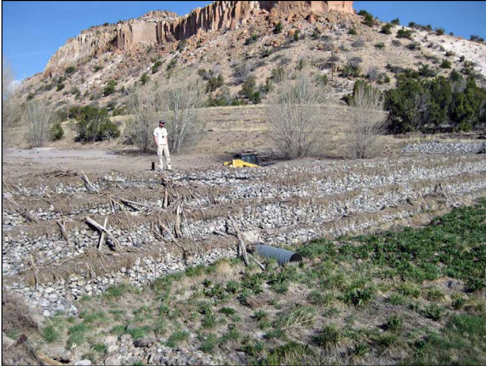
Photo A1-22 April 2014 photograph of the Los Alamos Canyon low-head weir looking upstream
