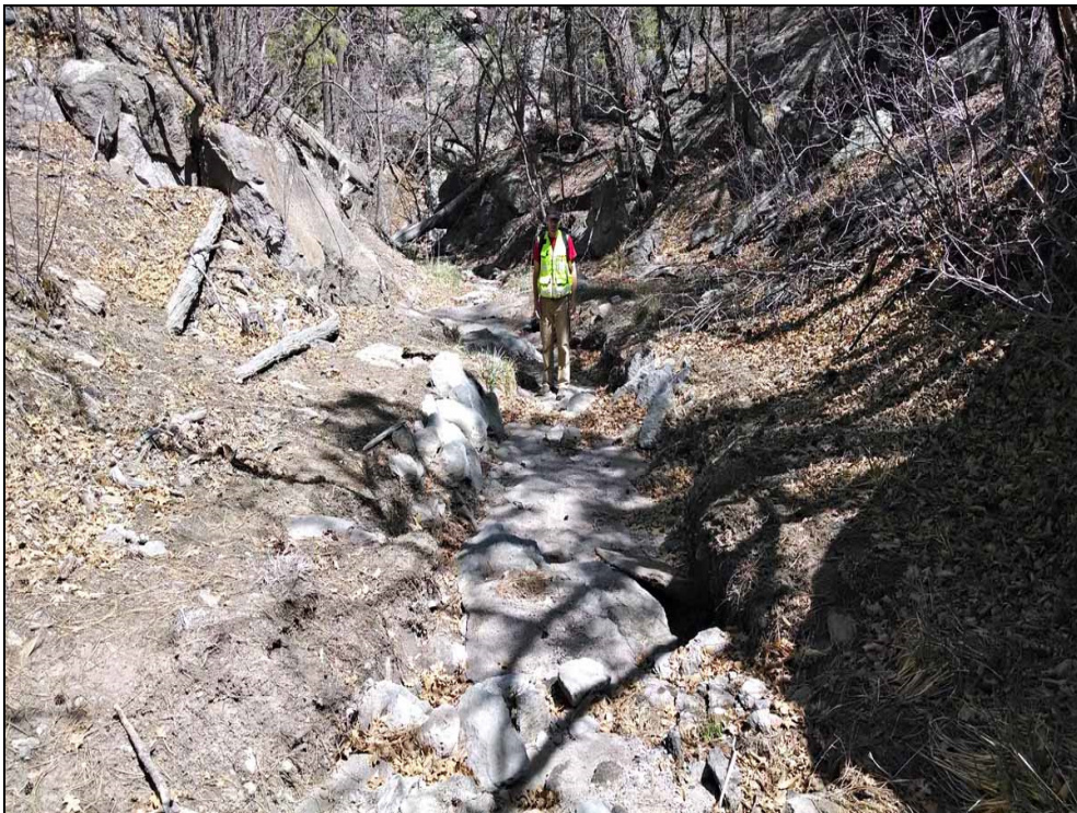
Photo A1-30 April 2014 photograph of rock armoring along stream banks in the south fork of Acid Canyon looking upstream
