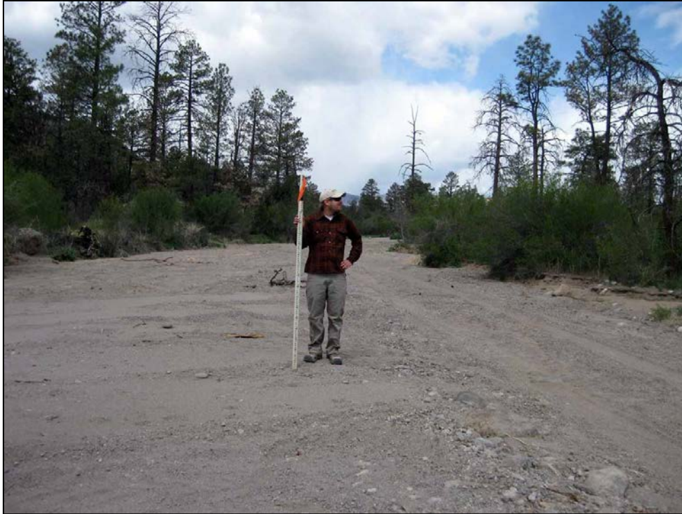
Photo A1-16 May 2014 photograph of area of maximum sediment deposition above the Pueblo Canyon grade control structure, PUGCS-100 ft, looking upstream. Surface modified after surveying during excavation of the intake above the PUGCS.
