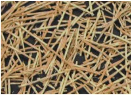
Improper Application Wood Straw at 70% Cover Must Be at 100% Cover
