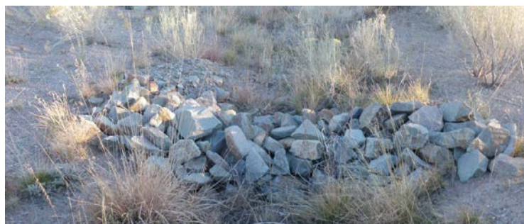
S-SMA-1.1, Rock Check Dam, S00206010008 (photo ID 29464-9)
