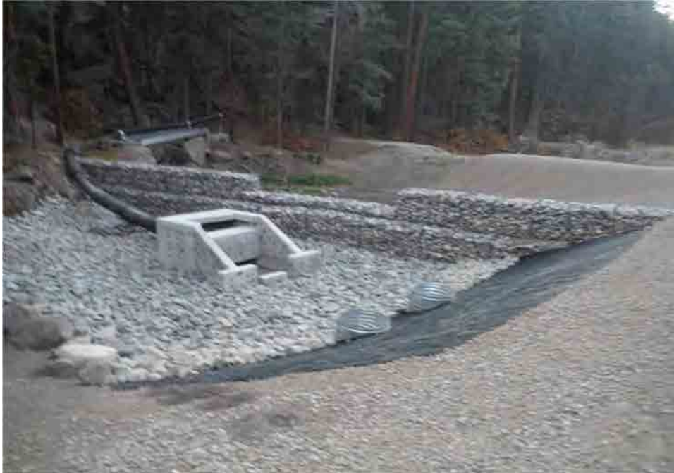
Photo C-3.16-4 Nov 2016 — Filter fabric removed.
