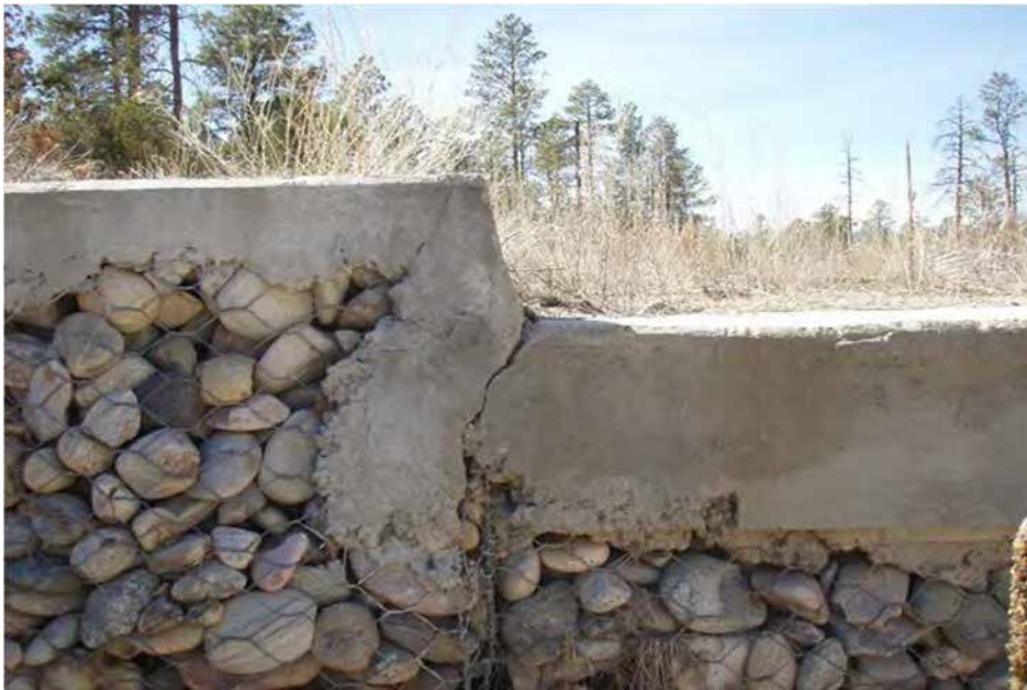
Photo C-5.3-1 March 2016 — Cracking apparent on joints of spillway. No change from previous inspections. Recommend monitoring.
