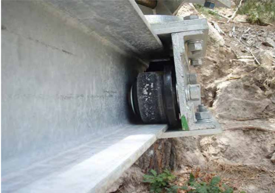
Photo C-3.11-2 June 2016 — Lower rolling pipe support on I-beam with skewed alignment and incorrect bearing. Recommend monitoring I-beam.
