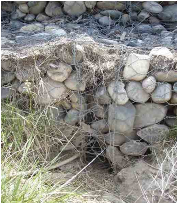
Photo C-4.6-2 June 2016 — Gabion baskets on stream face of weir appear to have undercutting with erosion immediately downstream. Recommend monitoring.
