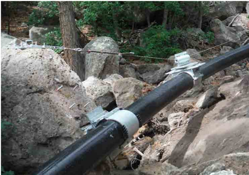
Photo C-3.10-2 Flow Event on August 3, 2016 — Uppermost support cable with fraying and corrosion. Recommend monitoring cables.
