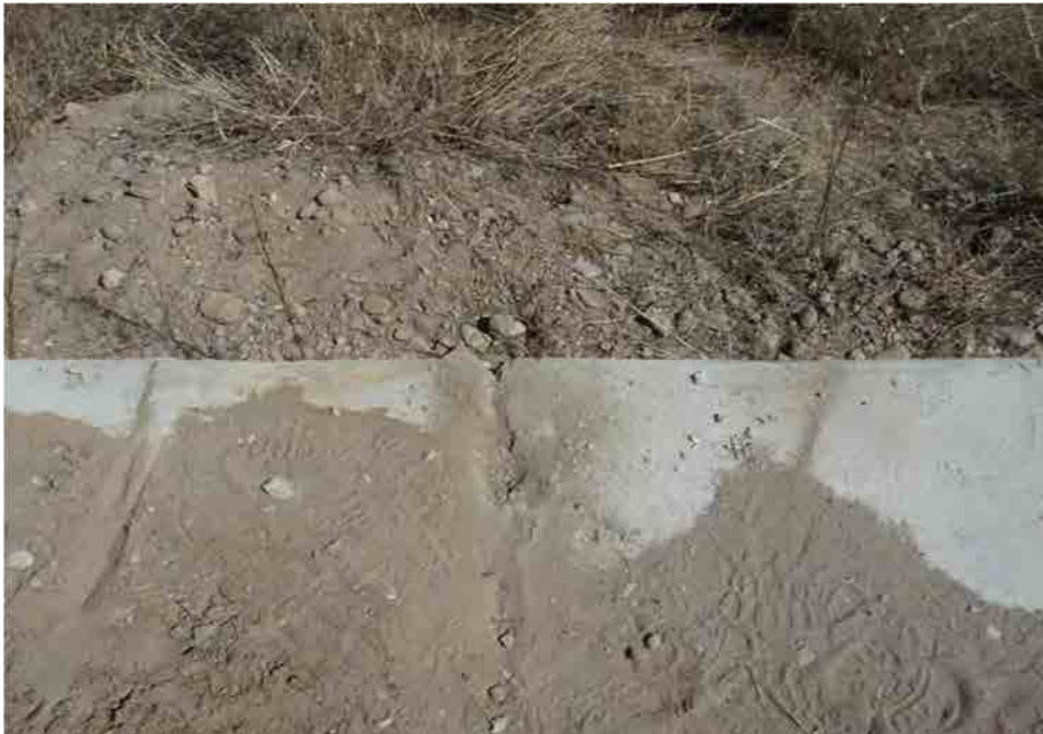
Photo C-5.4-1 March 2016 — Cracking across the concrete crest in a few locations. No change from previous inspection. Recommend monitoring.
