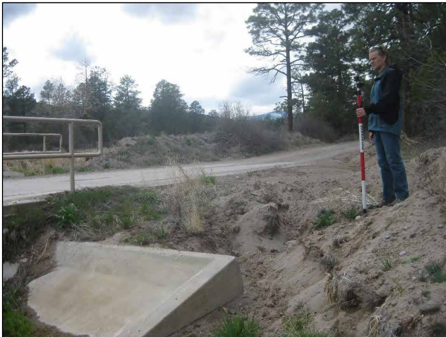
Photo A1-7 Detected erosion (~2.4 ft) around wing ditch culverts/bridge, looking west
