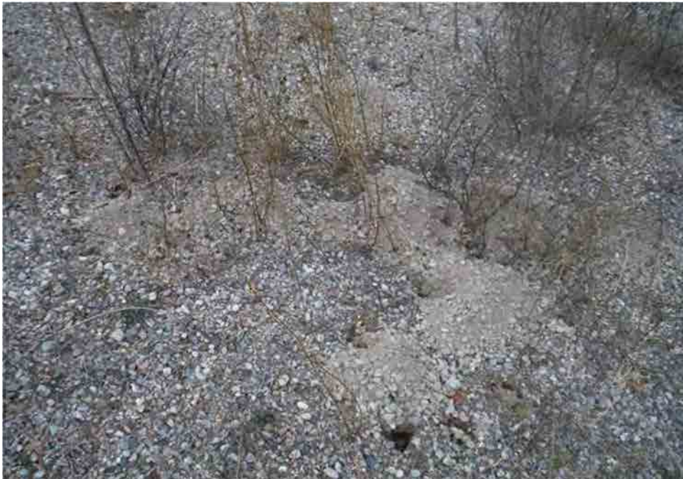
Photo C-3.5-1 March 2016 — Animal burrows in lower embankment south of spillway. Recommend repair of animal burrows.
