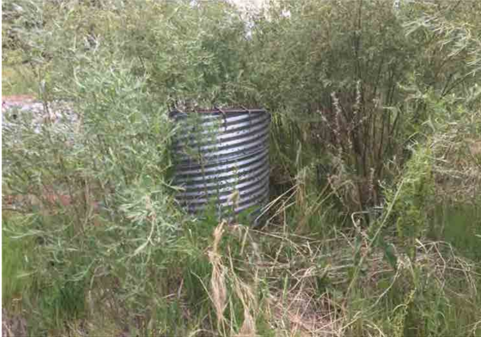
Photo C-2.4-2 June 2016 — Approximate height between channel bed and top of weir is 3.5 ft (no change from previous inspection [Q1 2016]). Tire is still present in the standpipe. Recommend monitoring and removal of tire.
