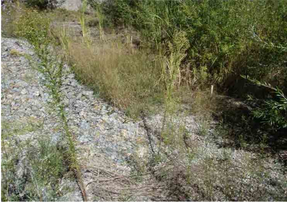
Photo C-3.8-4 Sept 2016 — Deteriorated wattles downstream of lower spillway (consistent with previous inspection). Recommend repairing deteriorated wattles.
