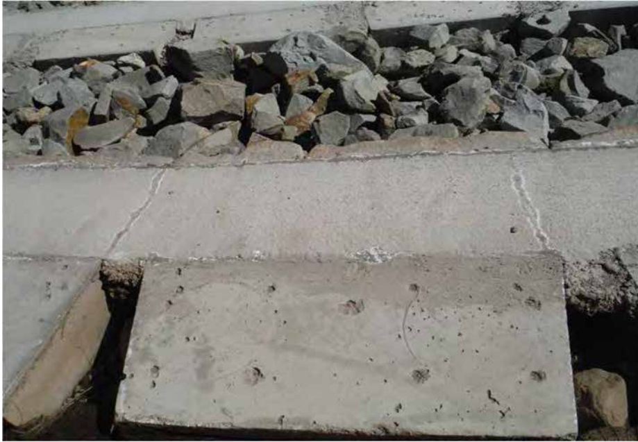
Photo C-6.1-1 March 2016 — Redi-Rock structure shows minor cracks in the concrete. Recommend monitoring cracks.
