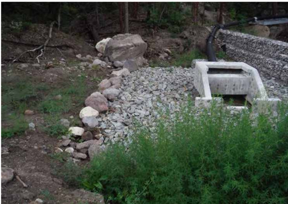
Photo C-3.15-3 Flow Event of August 3, 2016 — Pipe outlet contains trash and debris. Standing water present due to recent rain event. Recommend removal of debris.
