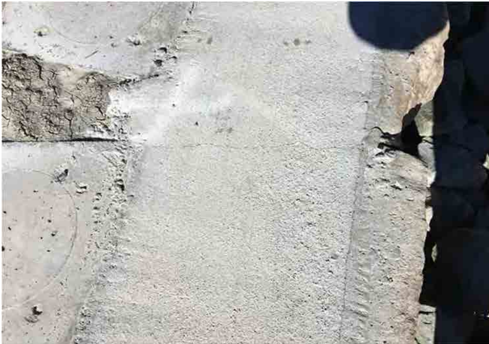
Photo C-6.1-4 Nov 2016 — Shrinkage cracks consistent with previous inspection. Recommend monitoring cracks.
