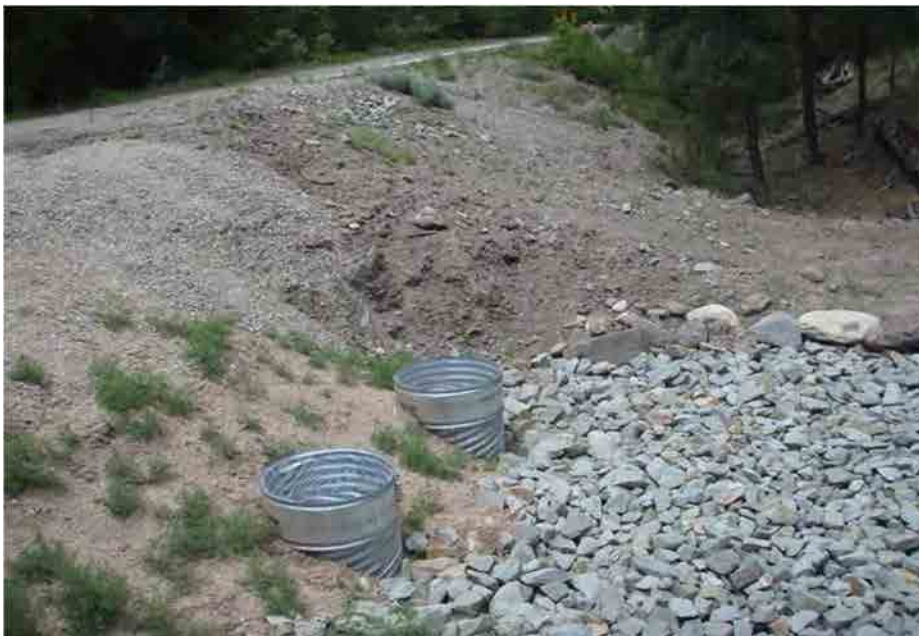
Photo C-3.18-2 June 2016 — Recommend installing trash racks and 3-in.-diameter holes on riser pipes. Bank erosion present.
