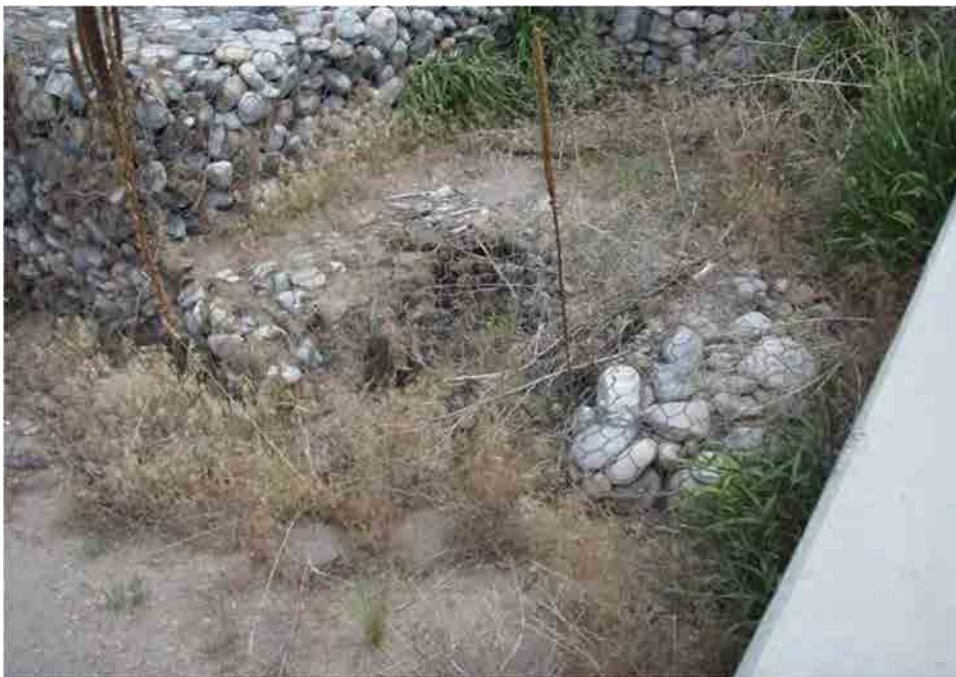
Photo C-5.8-2 June 2016 — Gabion basket settling and missing rocks. Consistent with previous inspections. Recommend monitoring.
