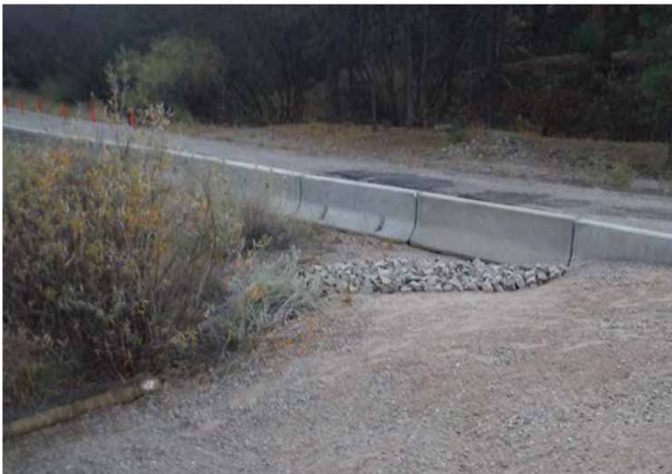
Photo C-3.5-5 Nov 2016 — Lower basin spillway looking east. Animal burrows recently repaired under maintenance work order.
