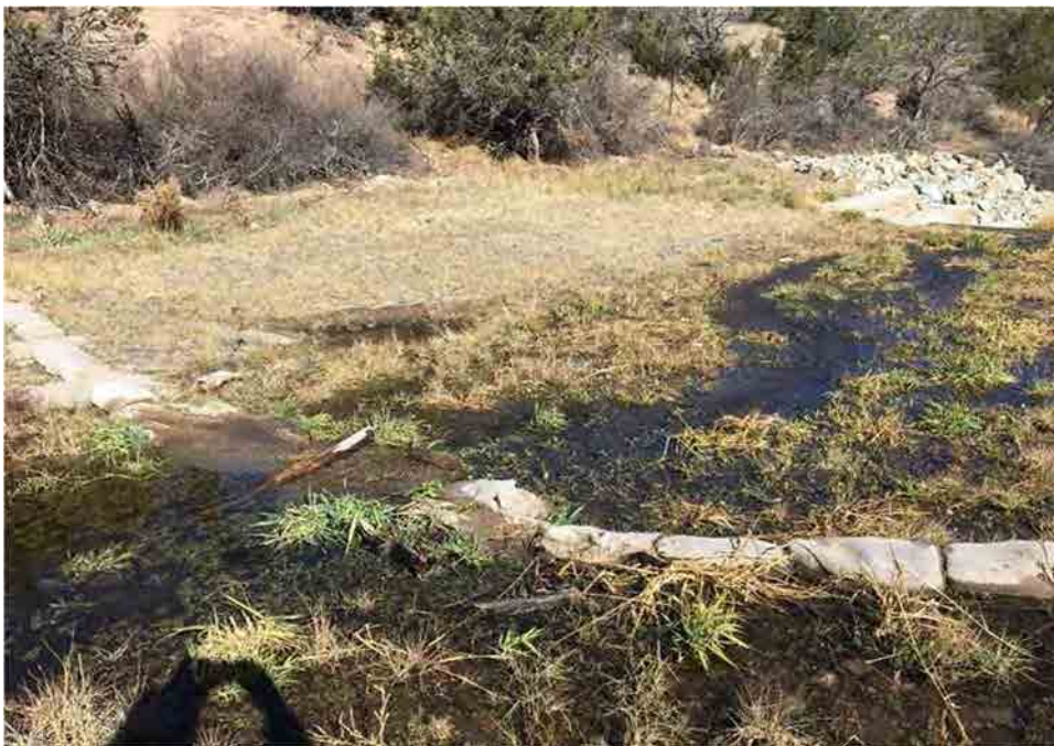
Photo C-6.3-4 Nov 2016 — Channelization present at location of sandbags. Repair sandbags to encourage the spread of water.
