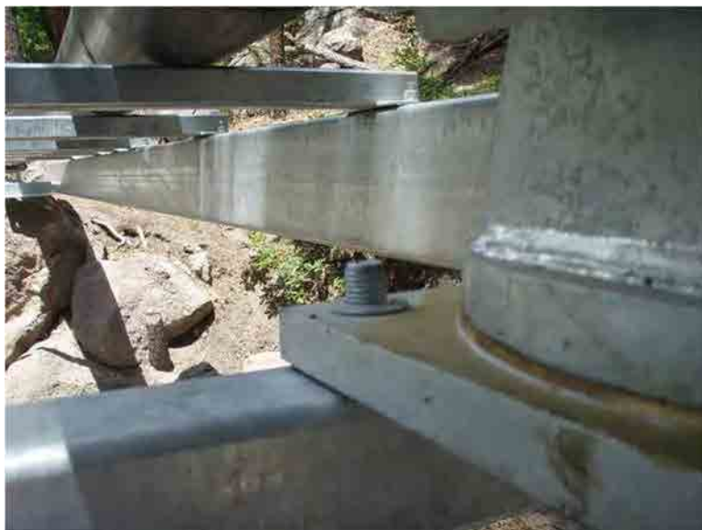
Photo C-3.13-1 June 2016 — Pipe support bolt with missing nut. Recommend installing missing nut.
