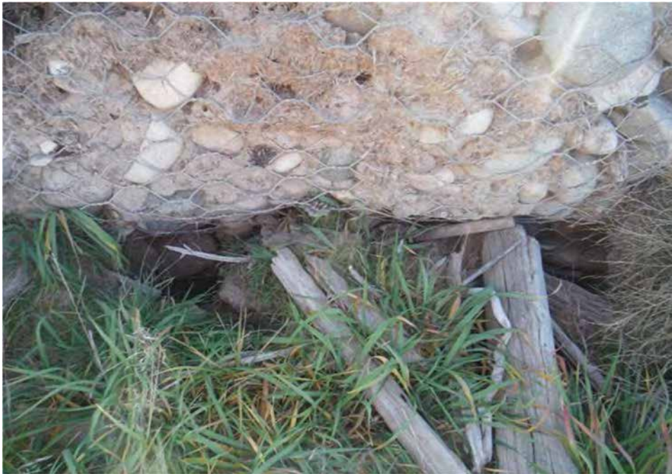
Photo C-4.7-3 Oct 2016 — Occurrences of piping have increased since last inspection. Piping appears to be occurring above the bottom of the weir's lowest level of gabion baskets and mattresses. Estimated 11 locations of piping along the weir. Large voids in gabions could allow fine sediment transport downstream. Recommend monitoring.
