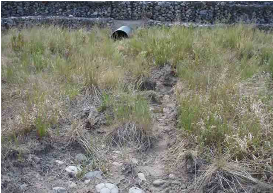
Photo C-4.2-2 June 2016 — Downstream side of outlet pipe shows evidence of erosion. Recommend monitoring.
