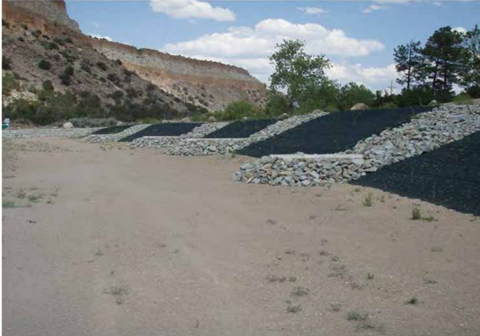
Photo C-5.10-2 June 2016 — Spurs and associated riprap in good condition.
