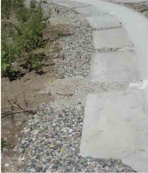
Photo C-6.4-3 Sept 2016 — Monitor area behind Redi-Rock for future erosion. This area was repaired with a mix of gravel and bentonite plugs, which are allowing for a better distribution of flow over the wall in this area.
