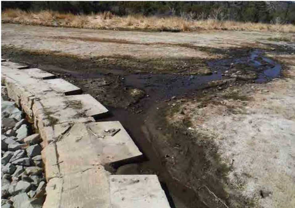
Photo C-6.3-1 March 2016 — Channelization noted, upstream portion of the structure directly behind the Redi-Rock blocks. Recommend monitoring.
