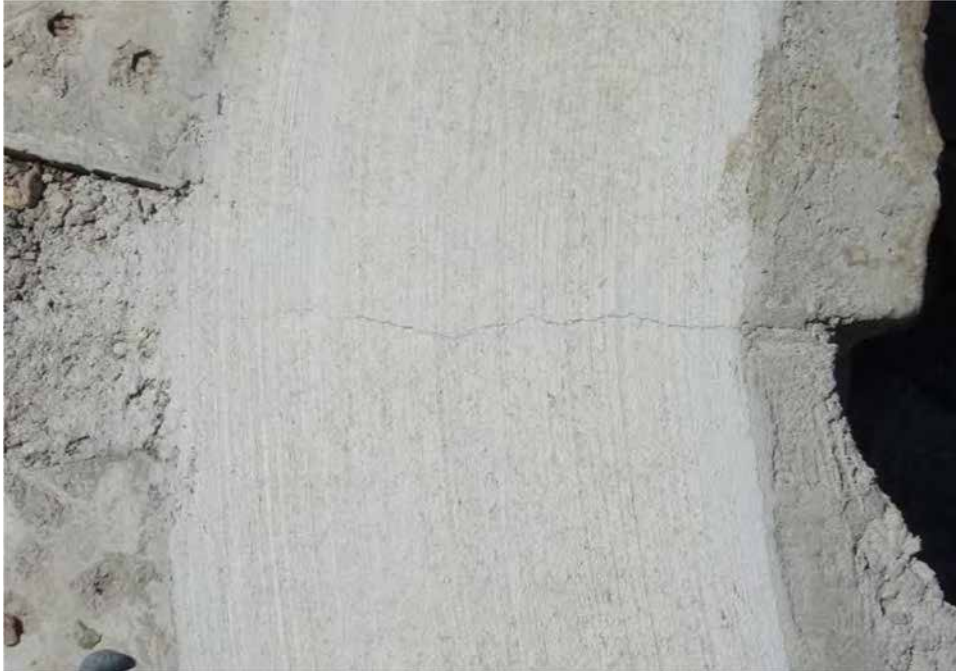
Photo C-6.1-3 Sept 2016 — Shrinkage cracks consistent with previous inspection. Recommend monitoring cracks.
