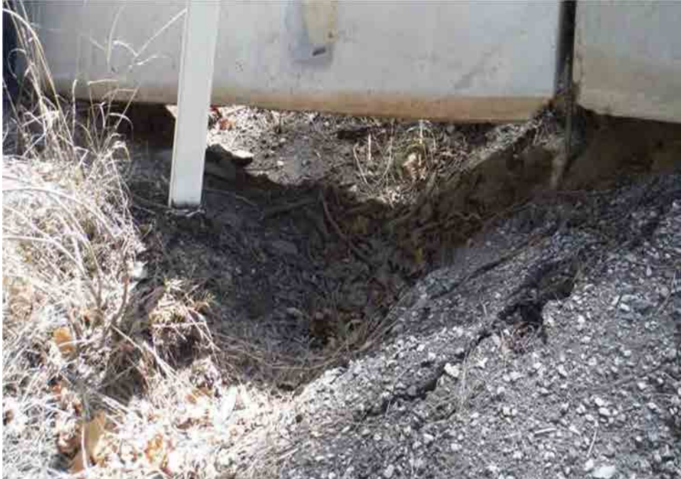
Photo C-3.19-1 March 2016 — Road collapse under Jersey barrier at southeast end of wetland. Recommend repair of road.
