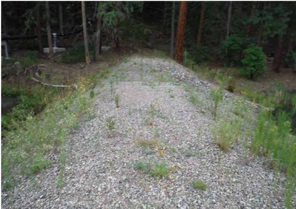
Photo C-3.3-3 Flow Event on August 3, 2016 — Animal burrows present. Slumping failure still present. Recommend repair burrows and slumping.
