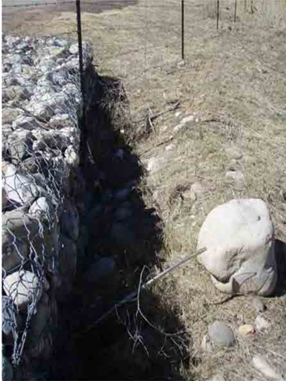
Photo C-4.8-1 March 2016 — Preferential flow path developing on upstream south embankment near the fence. Recommend monitoring.
