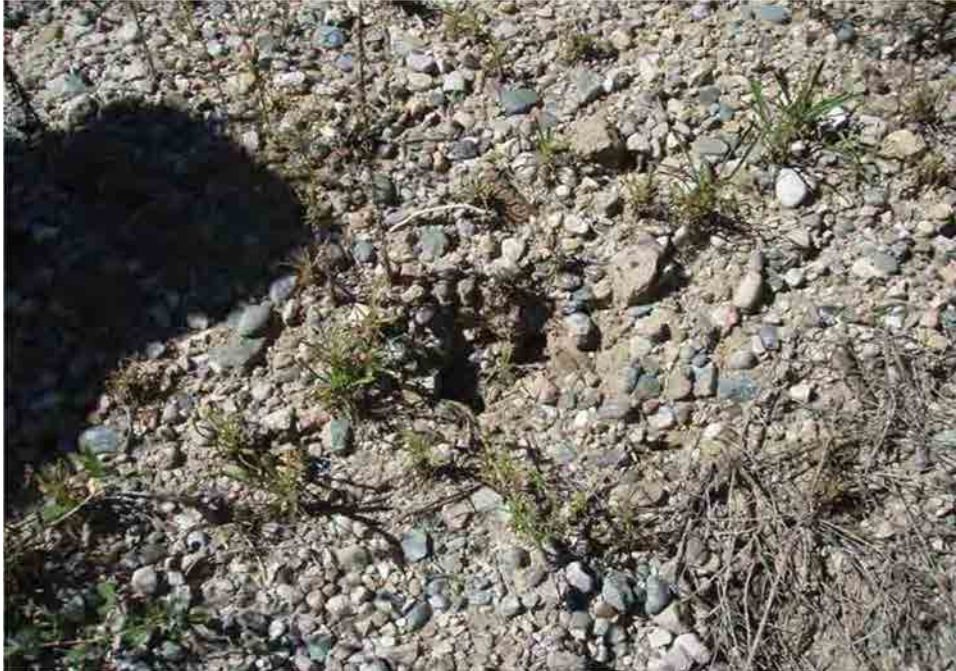
Photo C-3.5-4 Sept 2016 — Animal burrows still present. No change in size and shape since last inspection (flow event on August 3, 2016). No evidence of flow. Recommend repair of animal burrows.
