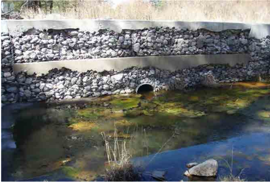
Photo C-2.1-1 March 2016 — Downslope side shows standing water present in pond. The pipe is about \frac{1}{4} full, difficult to determine at the time if sediment is an issue. Recommend monitoring.
