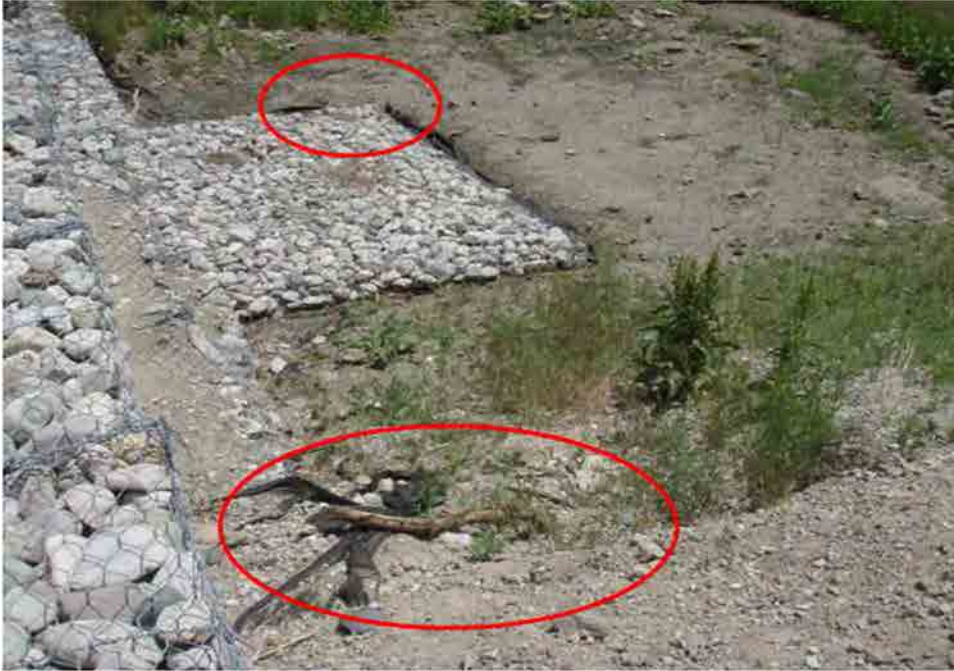
Photo C-3.1-2 June 2016 — Floatable debris found in upper basin marked by red circles. Sloughing on north bank not pictured. Recommend monitoring both.
