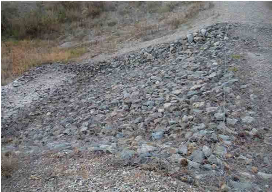
Photo C-3.3-5 Nov 2016 — Spillway wire enclosed riprap repair recently completed under maintenance work order.
