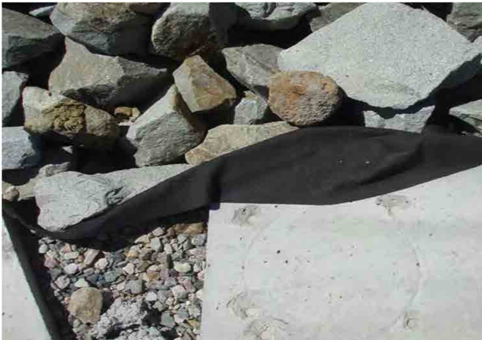
Photo C-6.5-2 Sept 2016 — Some geotextile under riprap has been uncovered. Consistent with previous inspection. Recommend monitoring.
