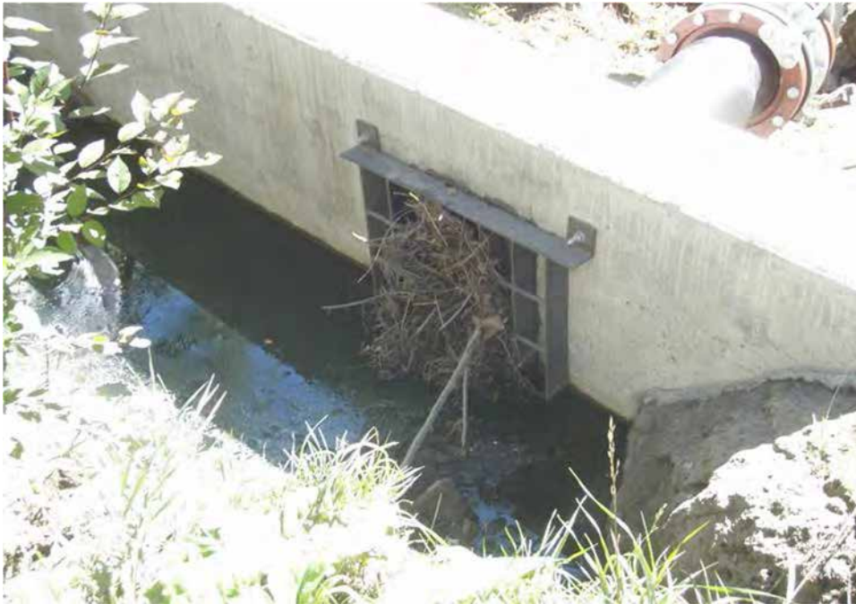
Photo C-3.14-4 Sept 2016 — Pipe inlet still plugged with debris. Recommend removal of debris.
