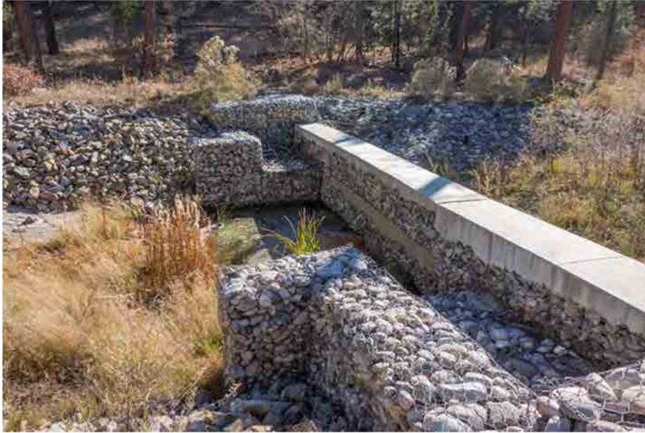
Photo C-2.1-3 Nov 2016 — Standing water in downslope side pond still shows standing water. No visible seepage or piping issue present. Pipe is about 1/8 full and is consistent with the last inspection. Recommend monitoring.
