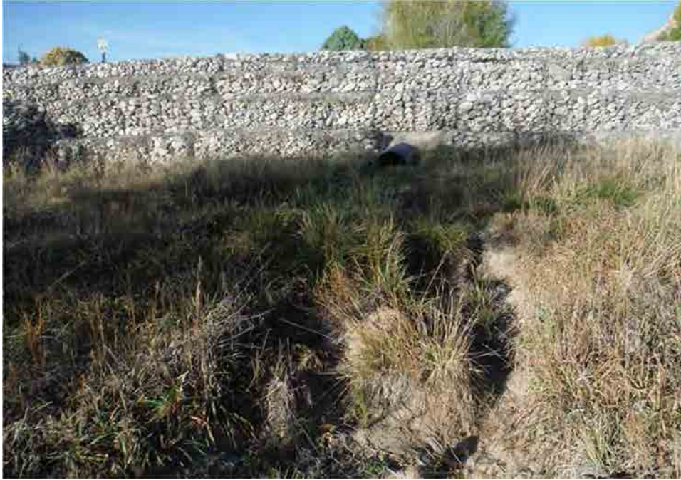
Photo C-4.2-3 Oct 2016 — Downstream side of outlet pipe shows signs of erosion. Recommend monitoring.
