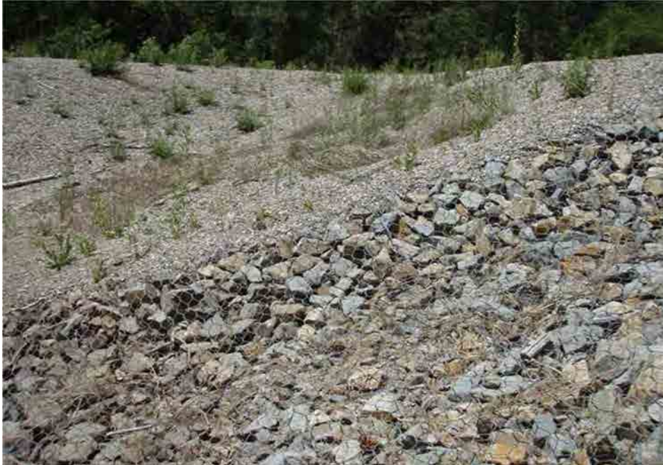
Photo C-3.3-2 June 2016 — Slumping failure of riprap still present. Newly noted animal burrows present. Recommend repair burrows and slumping.
