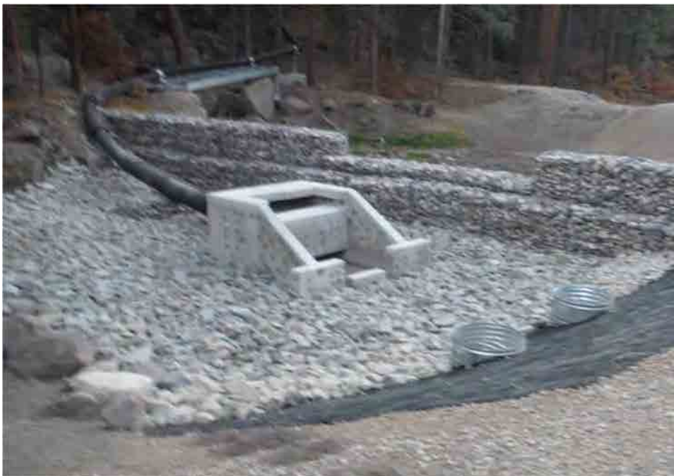
Photo C-3.15-5 Nov 2016 — Pipe outlet looking northeast. Riprap on banks recently installed under maintenance work order. Recent rodent activity on south bank.
