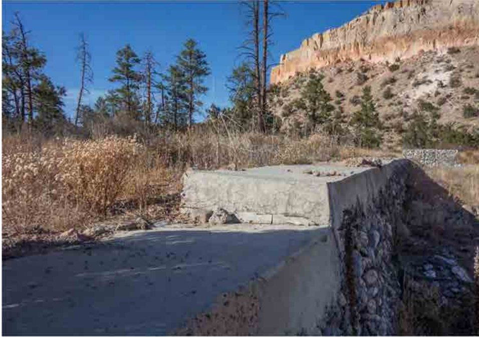
Photo C-5.6-4 Nov 2016 — Gabion baskets adjacent to overflow catchment are bowing out. Consistent with previous inspection. Recommend monitoring.
