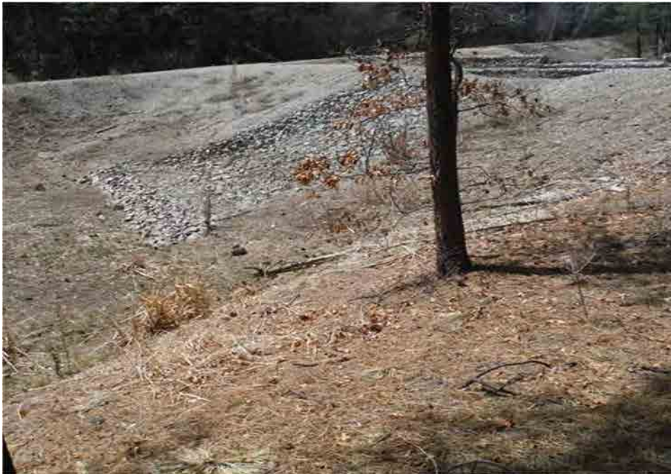
Photo C-3.4-1 March 2016 — Lower basin has sloughing on north bank.
