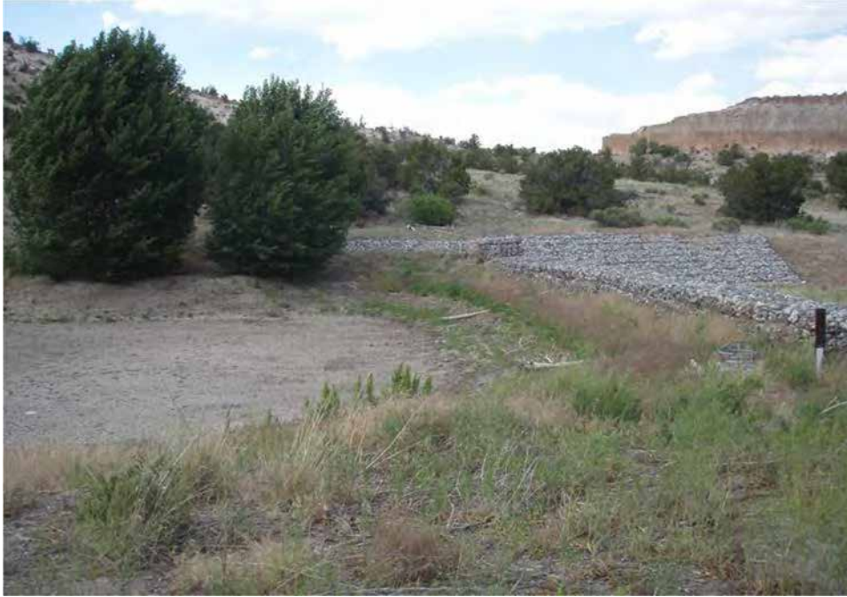
Photo C-4.3-2 June 2016 — Lower pond with estimated 5–6 ft of sediment below top of spillway.
