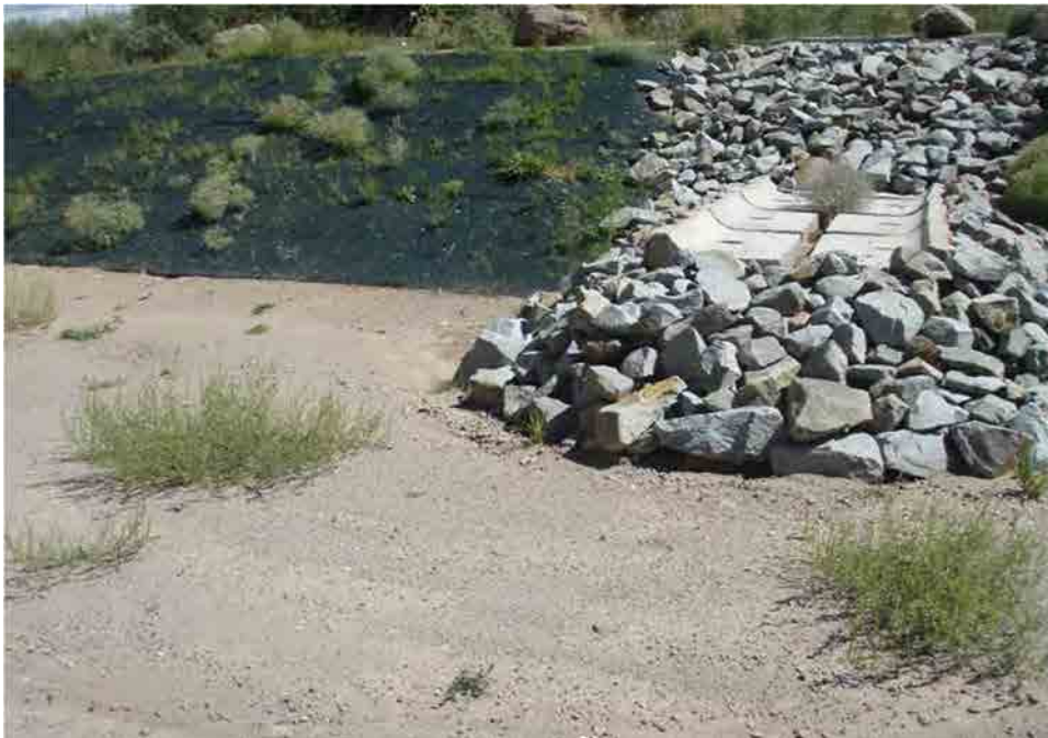
Photo C-5.10-3 Sept 2016 — Rilling occurring at the tip of Spur 4. Recommend monitoring.
