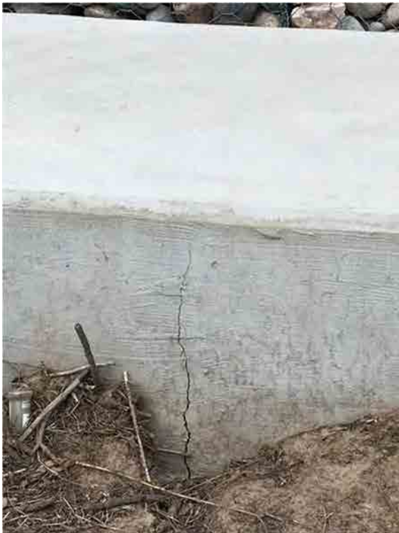
Photo C-2.3-2 June 2016 — Cracks are consistent with previous inspection. Recommend monitoring.
