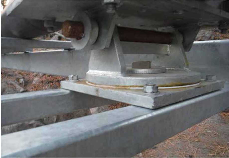
Photo C-3.13-4 Nov 2016 — Previously missing nut recently installed at southwest corner top of plate under maintenance work order.
