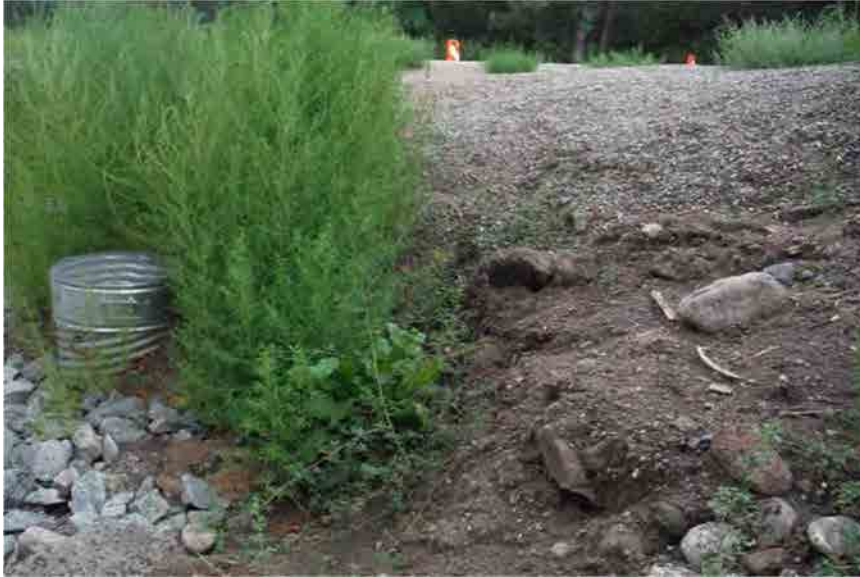
Photo C-3.18-3 Flow Event on August 3, 2016 — Tall vegetation encountered near new culvert pipe inlet risers. Bank erosion present. Recommend installing trash racks and 3-in.-diameter holes on riser pipes.
