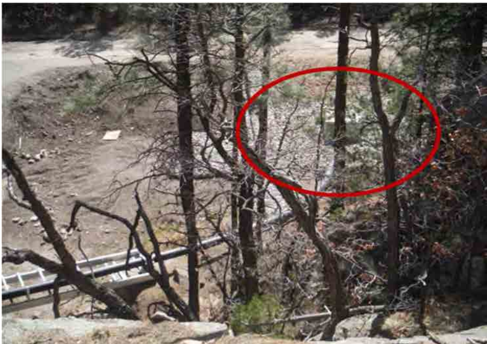
Photo C-3.15-1 March 2016 — Bare soils on steep slopes found on south and north bank upstream of the gabion overflow structure to upper pond. Pipe outlet circled in red above.
