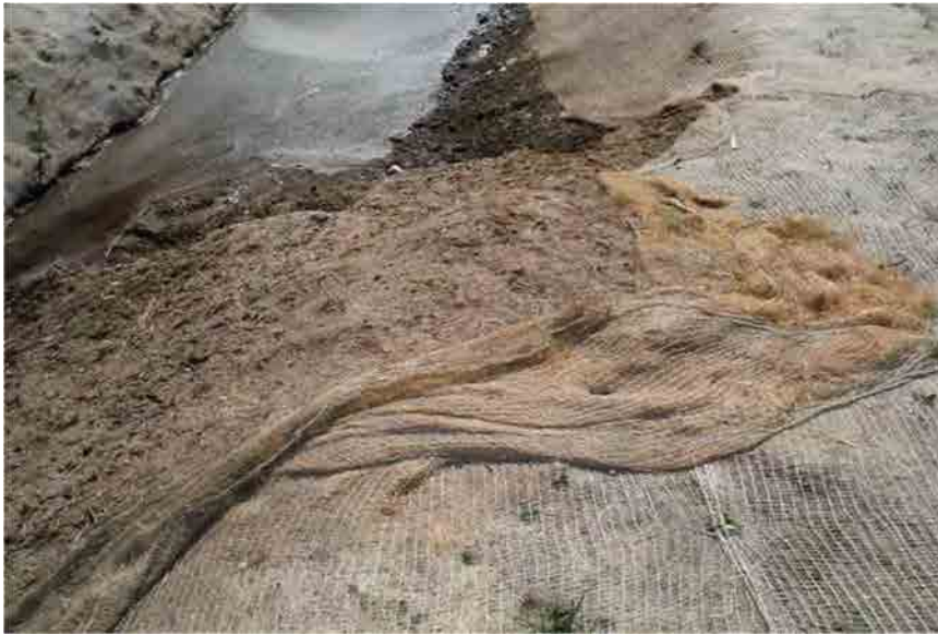
Photo C-6.10-1 March 2016 — TRM is beginning to degrade and has unstapled in a few areas. Recommend re-stapling TRM in this area. Monitor for growth in 2016.
