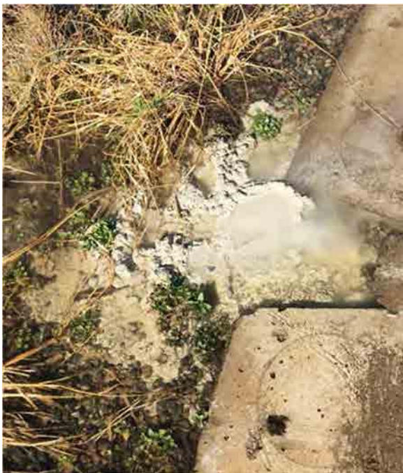
Photo C-6.4-4 Nov 2016 — Monitor behind Redi-Rock for future erosion. Controls previously put in place are allowing for a better distribution of flow over the wall in this area.
