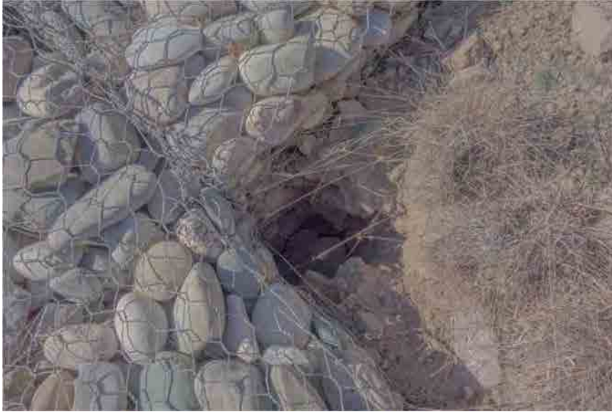
Photo C-2.8-1 Nov 2016 — Erosion feature near northeast corner of spillway. Hole is approximately 2 ft deep and is not described in previous inspection reports.
