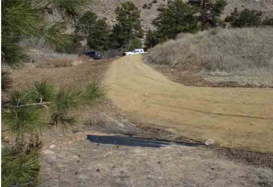
Photo C-4.9-1 March 2016: Borrow pit runoff control berm looking north. The borrow pit runoff control berm appears to be in good hydrologic condition and is functioning correctly to reduce runoff and sediment migration from the area. Recommend monitoring.
