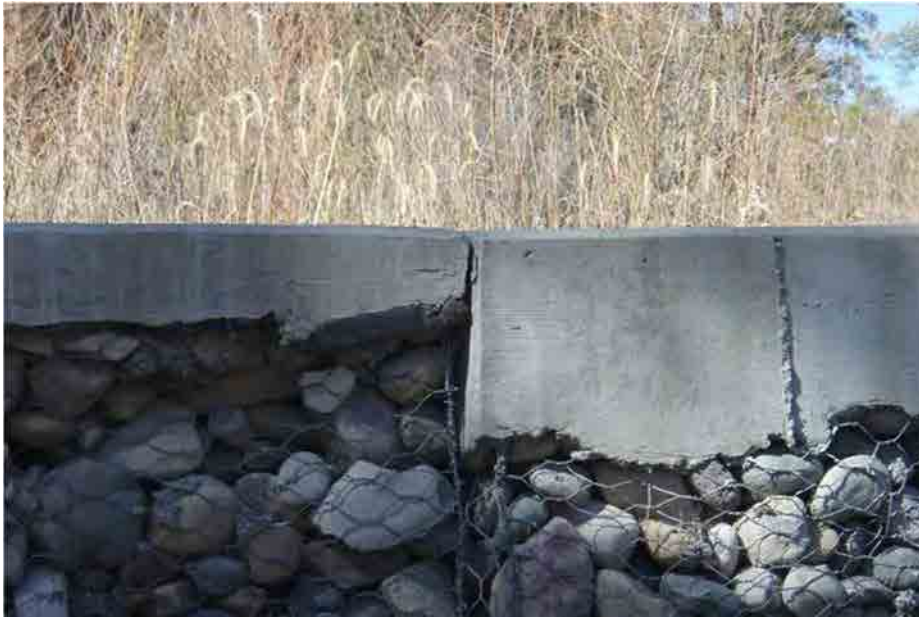
Photo C-2.2-1 March 2016 — The joint located on the northern portion of the crest directly above the bulging gabion basket shows signs of separation (approximately 0.25 in.). No change in condition from the last inspection (Q3 2015). Recommend monitoring.
