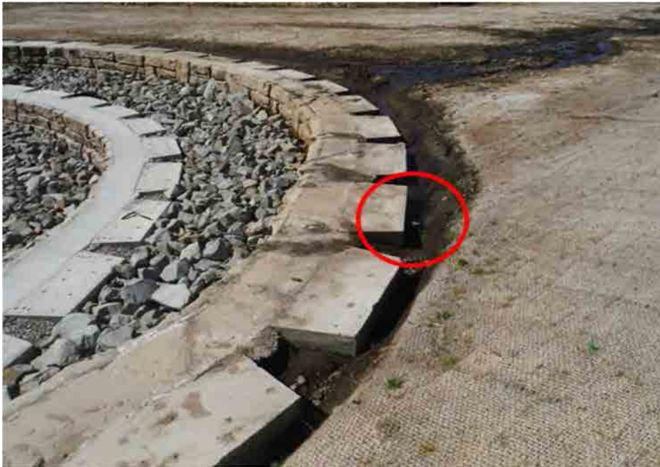
Photo C-6.4-1 March 2016 — Metal debris in T-post section (noted in red circle). Recommend removal.
