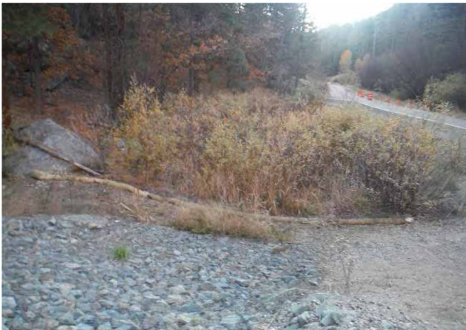
Photo C-3.8-5 Nov 2016 — Straw wattles recently replaced under maintenance work order.
