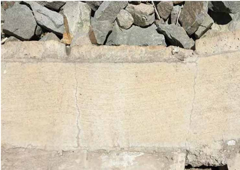
Photo C-6.1-2 June 2016 — Redi-Rock structure shows minor shrinkage cracks. Recommend monitoring cracks.
