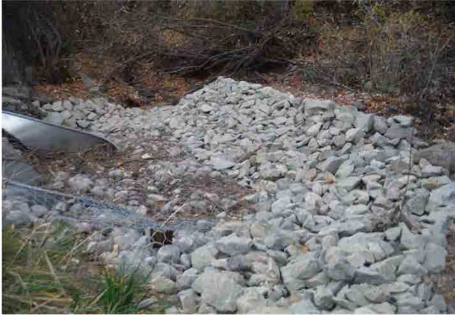
Photo C-3.17-5 Nov 2016 — Culvert outlet riprap extension completed under maintenance order.
