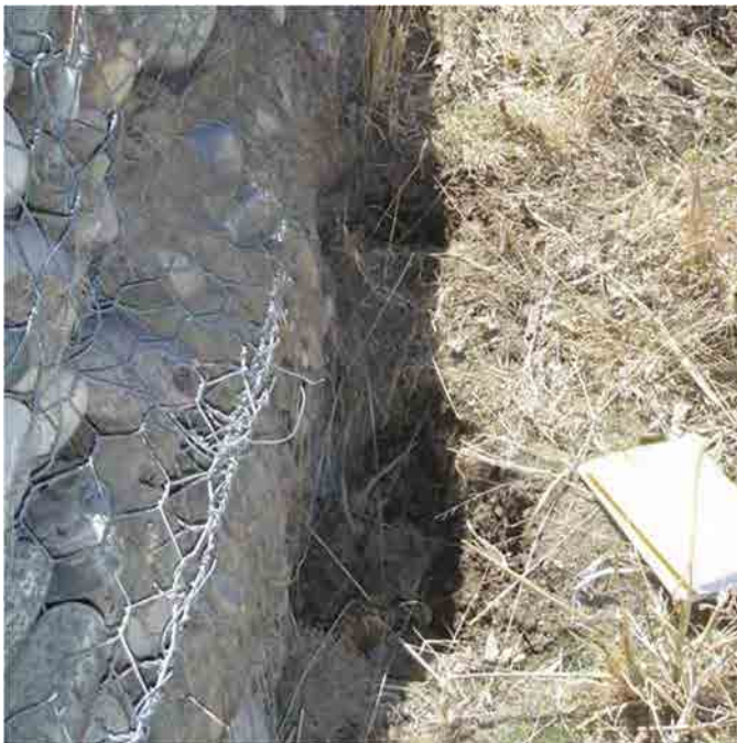
Photo C-4.7-1 March 2016 — Piping on upstream side of weir consistent with previous inspection. Recommend monitoring.
