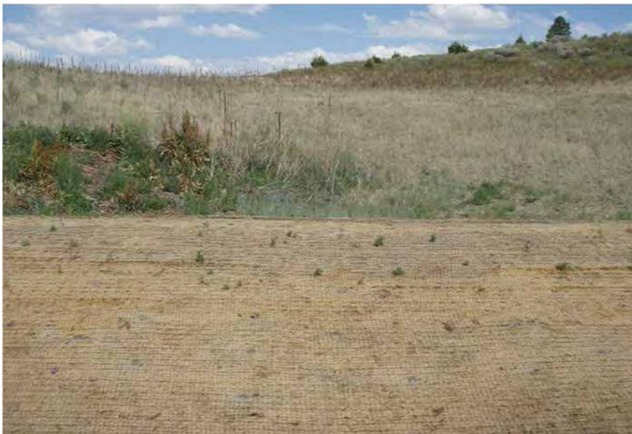
Photo C-4.9-2 June 2016 — Borrow pit runoff control in good condition and is functioning correctly. Recommend monitoring.
