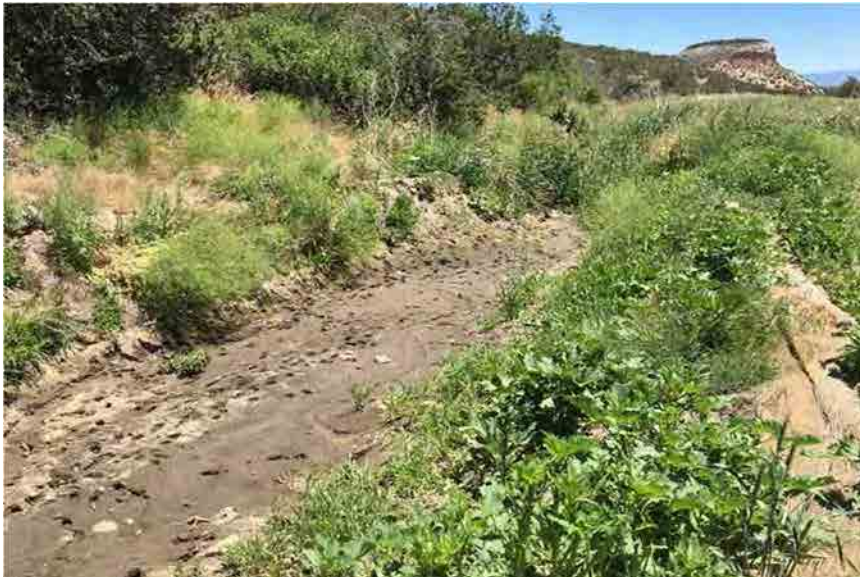
Photo C-6.10-2 June 2016 — The pond has no water in it. ECB has deteriorated on bands and vertical “steps” are present and exposed on interior slopes. ECB is at the end of life and should be retired. Vegetation on side slopes has 100% cover due to broad-leafed foliage. Continue to monitor.
