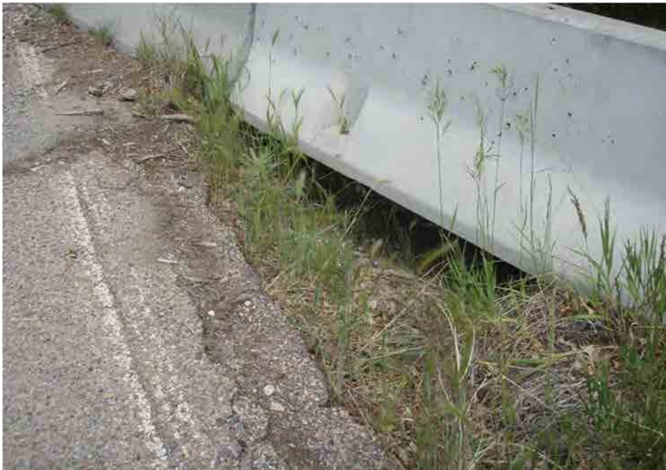
Photo C-3.19-2 June 2016 — Road collapse under Jersey barrier. Recommend repair of road.
