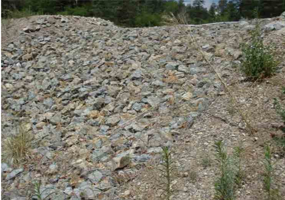
Photo C-3.5-2 June 2016 — Animal burrows on lower basin spillway. Based on visual inspection, number and size of holes appear to be consistent with last inspection (Q1 2016). Recommend repair of animal burrows.
