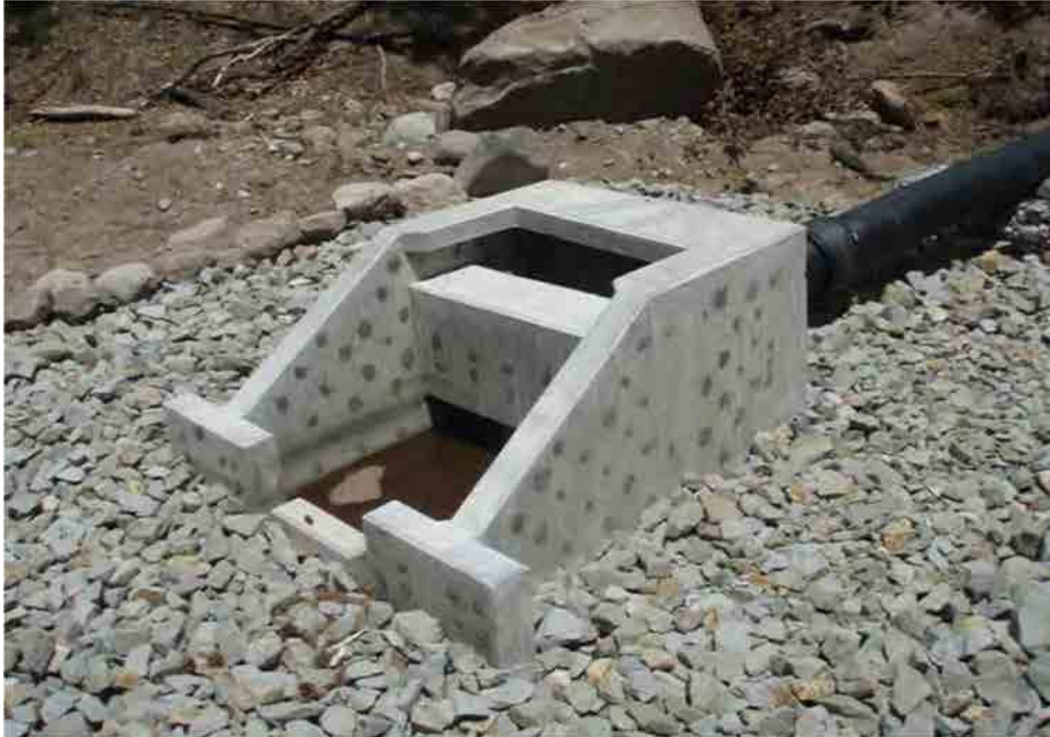
Photo C-3.15-2 June 2016 — Debris around energy dissipater present. Bare soil on south and north banks is exposed and in need of stabilization. Recommend removal of debris.
