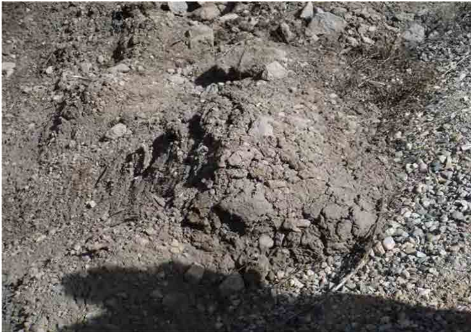
Photo C-3.2-1 March 2016 — Construction excavation spoils found in upper basin. Construction spoils decrease basin capacity. Recommend removal of construction spoils.
