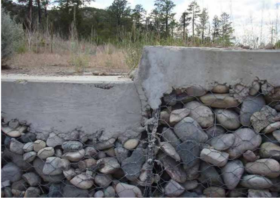
Photo C-5.5-2 June 2016 — Spalling and cracks present on the downstream side of the spillway crest. Consistent with previous inspection. Recommend monitoring.
