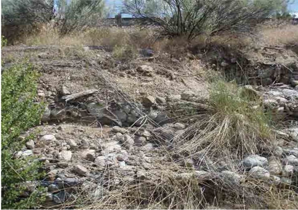
Photo C-4.5-2 June 2016 — Southside of embankment shows erosion approaching NMDOT ROW.
