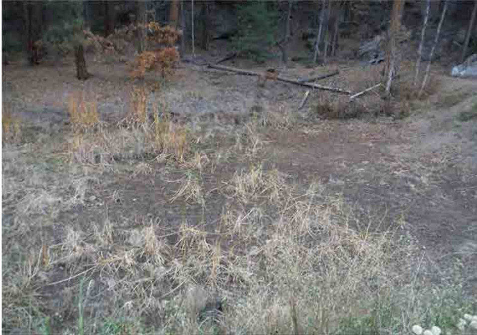
Photo C-3.4-5 Nov 2016 — Debris present in lower basin. Bottom of basin damp from previous flow events. Recommend removal of debris.
