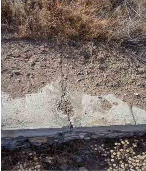
Photo C-5.4-4 Nov 2016 — Cracking across crest in several locations. Consistent with previous inspection. Recommend monitoring.
