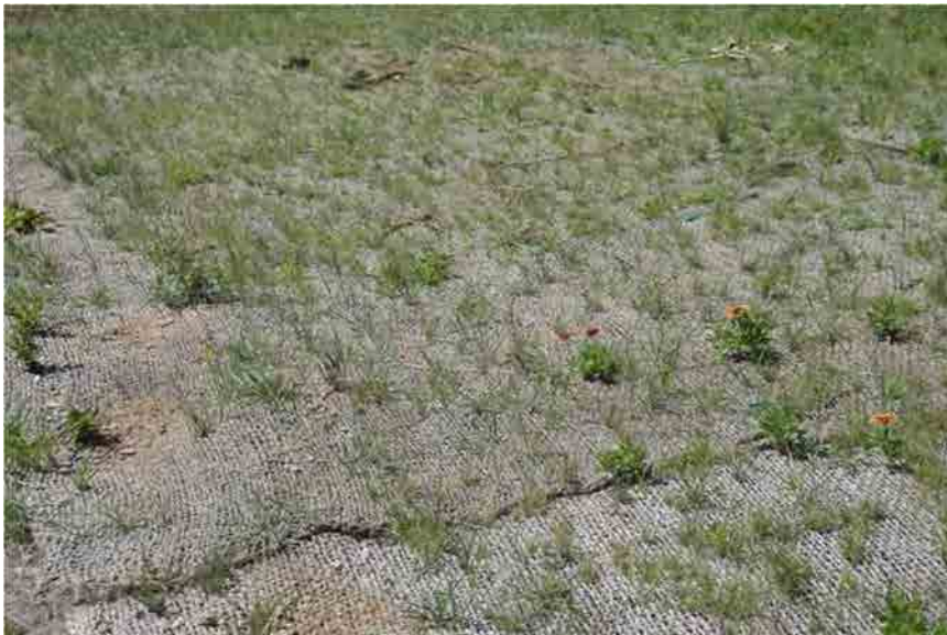
Photo C-6.8-2 Sept 2016 — Geotextile is covered by riprap and TRM except on edges. Vegetative growth becoming established through TRM. Recommend monitoring.
