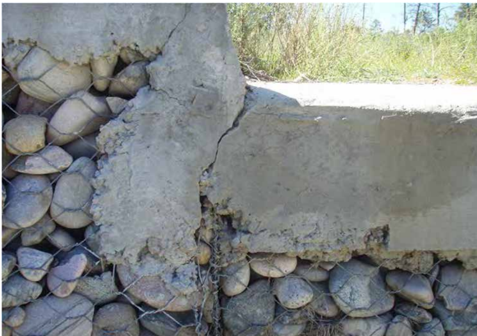
Photo C-5.5-3 Sept 2016 — Spalling and cracks on the downstream face of the spillway. Consistent with previous inspection. Recommend monitoring.
