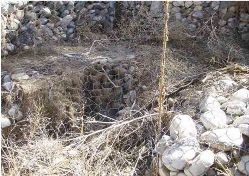
Photo C-5.8-1 March 2016: Gabion basket (located downstream on the south side of spillway) has deteriorated and no longer contains rock supporting the basket. Condition has not changed since previous two inspections. Recommend monitoring.
