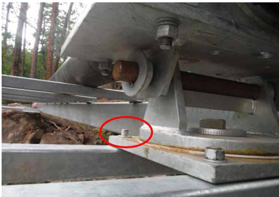
Photo C-3.13-2 Flow Event on August 3, 2016: Pipe support bolt with missing nut (circled in red) consistent with previous inspection. Recommend installing missing nut.
