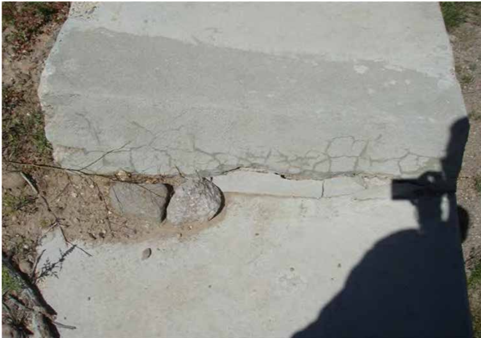
Photo C-5.3-3 Sept 2016 — Cracking occurring at the joints along the spillway. Consistent with previous inspection. Recommend monitoring.
