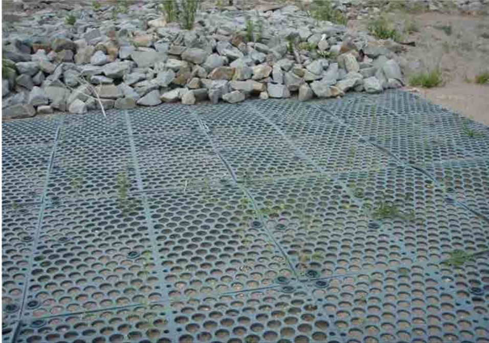
Photo C-5.9-2 June 2016 — ScourStop shows evidence of expansion with minor vegetative growth. Because of expansion, sheets exhibit some bowing but are still anchored to the ground. Recommend monitoring.
