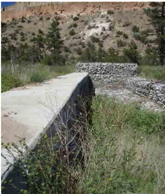
Photo C-5.6-3 Sept 2016 — Gabion baskets adjacent to overflow catchment are bowing out. Consistent with previous inspection. Recommend monitoring.
