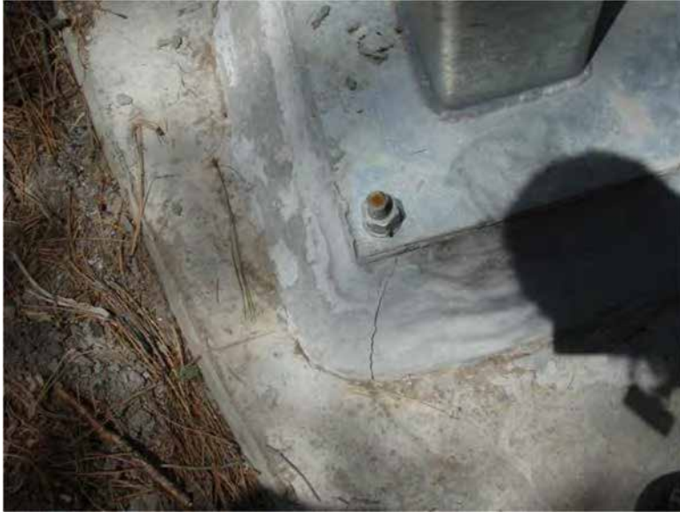
Photo C-3.12-2 June 2016 — Crack found in mortar on southeast corner pipe bridge support. Recommend monitoring crack.
