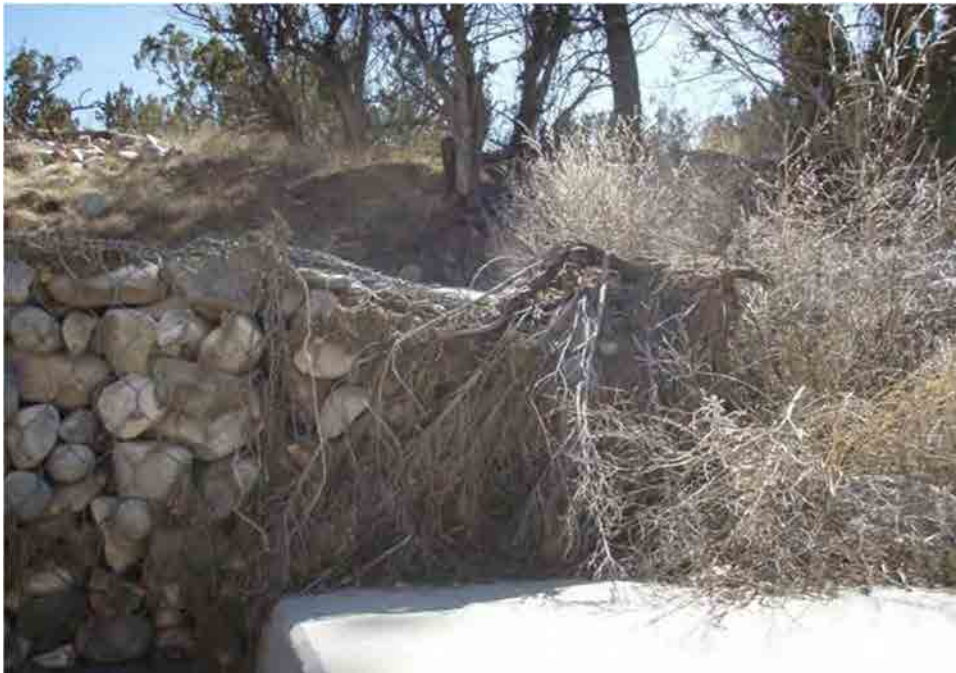
Photo C-5.12-1 March 2016 — Gabion basket on the upstream south side of the spillway appears to be degrading. Recommend monitoring.
