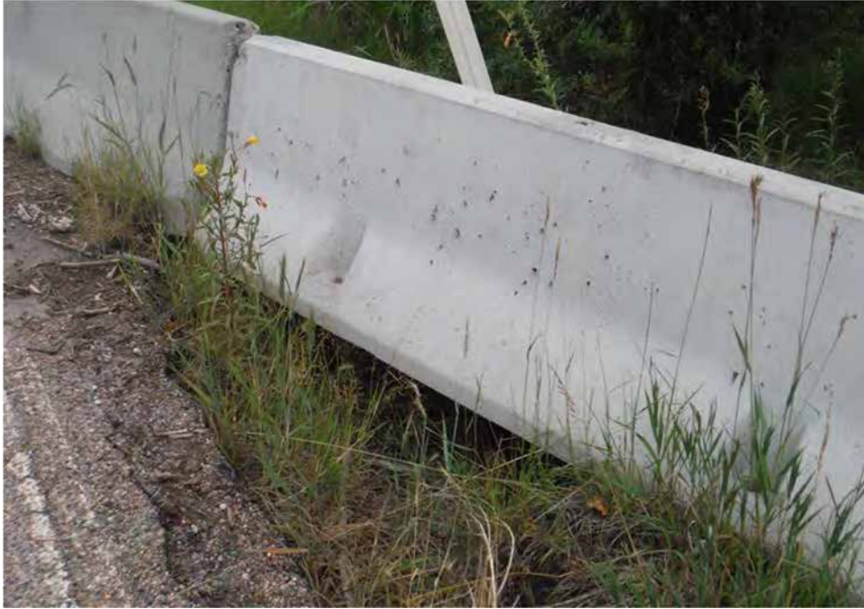
Photo C-3.19-3 Flow Event August 3, 2016 — Road collapse under Jersey barrier. Recommend repair of road.
