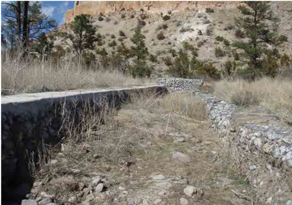
Photo C-5.7-1 March 2016 — The north side of the flow way has sediment accumulation and evidence of standing water (vegetation). Recommend monitoring.
