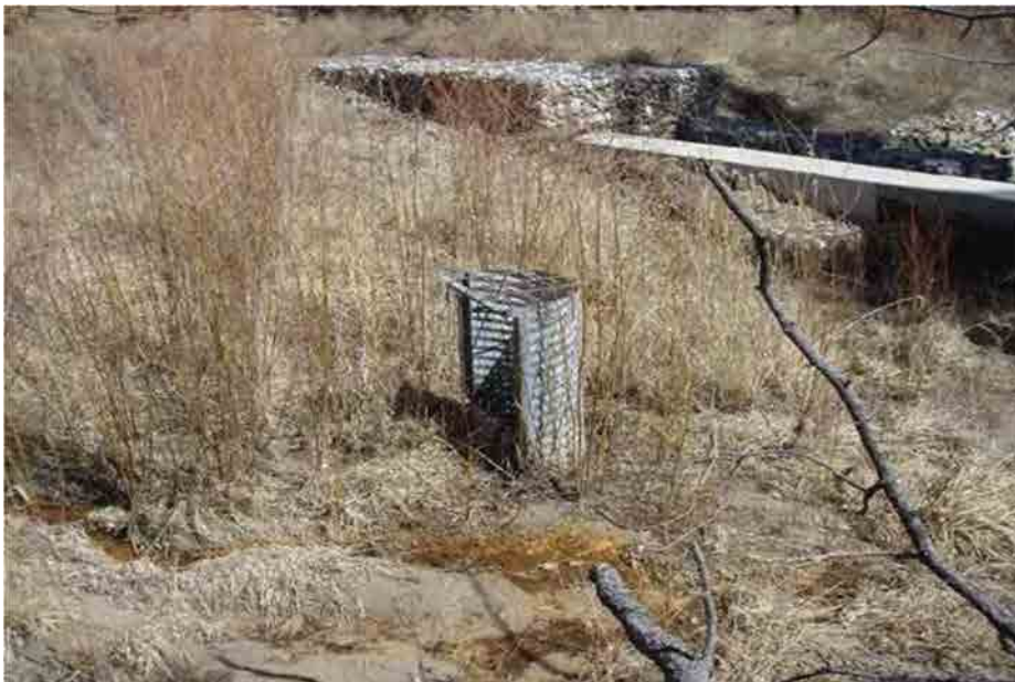
Photo C-2.4-1 March 2016 — Approximate height between channel bed and top of weir is 3.5 ft (no change from the last inspection [Q4 2015]). The height of the standpipe inlet is approximately 1 ft above the soil profile in front of the weir. This may represent a lower height than was present during the last inspection when 1.45 ft was reported. Tire present in standpipe. Recommend monitoring and removal of tire.
