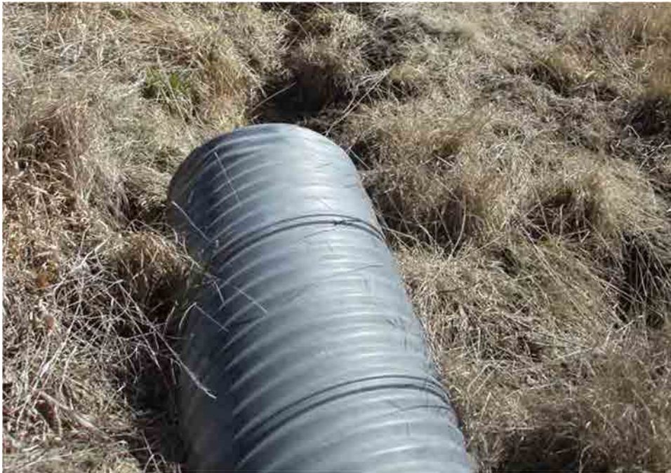
Photo C-4.2-1 March 2016 — Outlet pipe shows evidence of erosion. Recommend monitoring.
