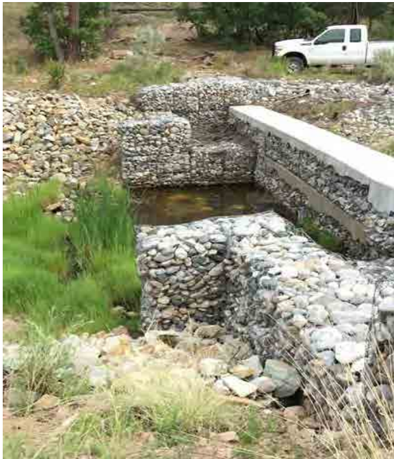
Photo C-2.1-2 June 2016 — Standing water in downslope side pond still shows standing water. No visible seepage or piping issue present. Pipe is about \frac{1}{8} full. Recommend monitoring.
