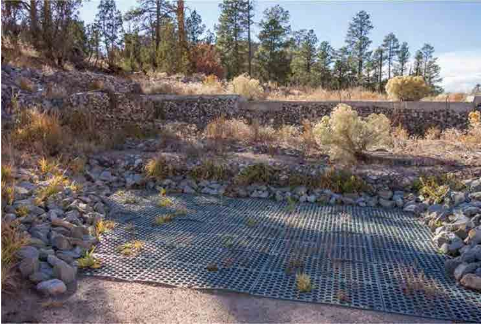
Photo C-5.9-4 Nov 2016 — ScourStop sheets consistent with previous inspection. Recommend monitoring.
