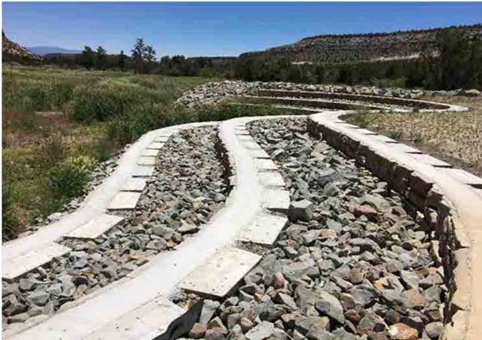
Photo C-6.5-1 June 2016 — Geotextile covered by riprap. Recommend monitoring.
