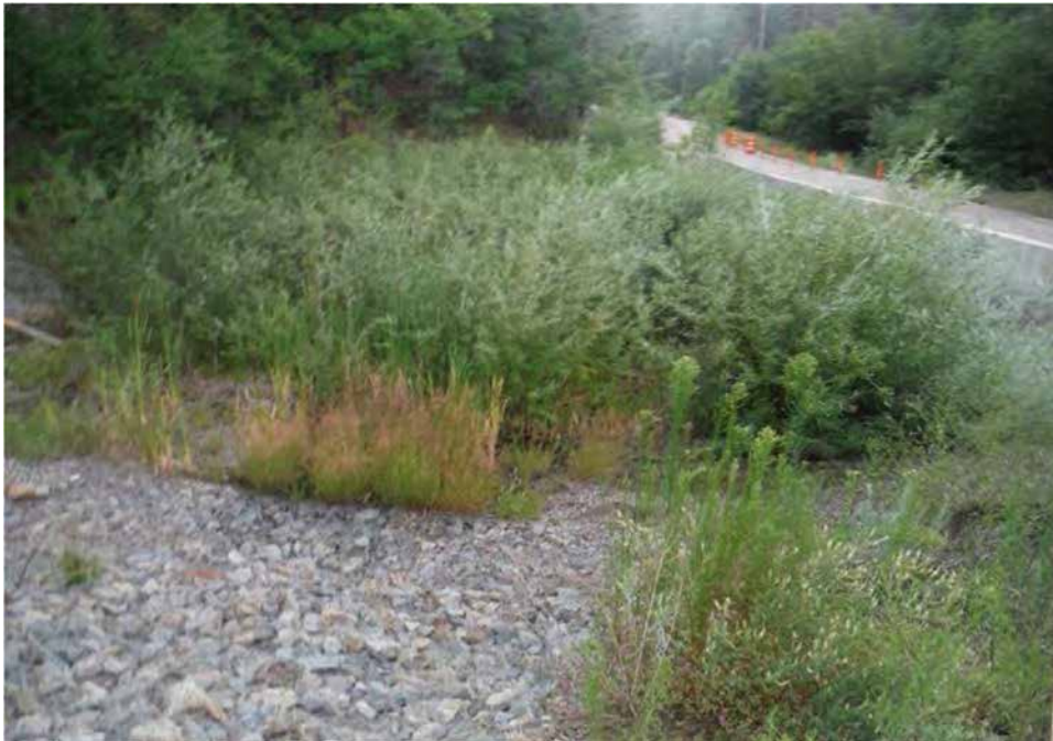
Photo C-3.8-3 Flow Event on August 3, 2016 — Deteriorated wattles. Recommend repairing deteriorated wattles.
