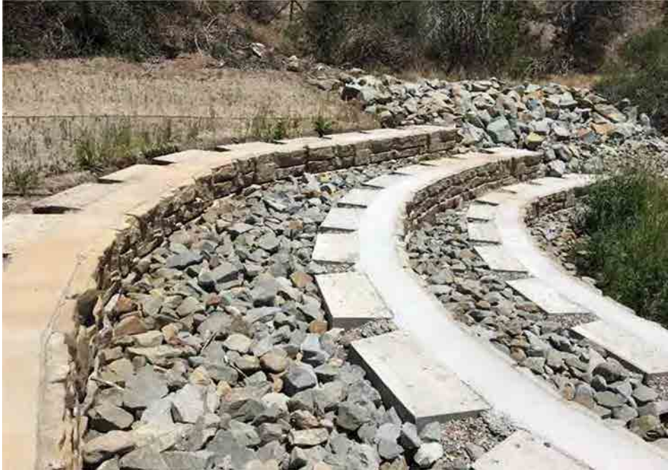
Photo C-6.8-1 June 2016 — Geotextile is covered by riprap except for edges. Recommend monitoring.
