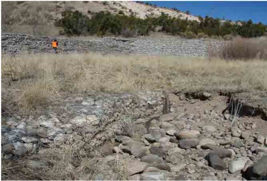
Photo C-4.6-1 March 2016 — Downstream end of gabion basket shows minor erosion and undercutting. Recommend monitoring.
