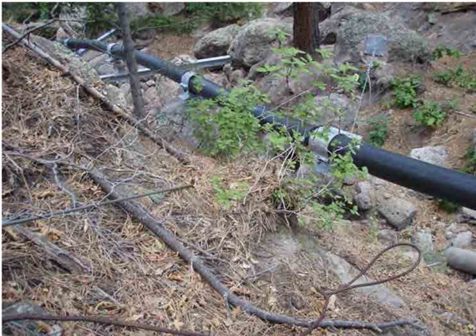
Photo C-3.9-2 June 2016 — Pipeline and supports (nick not pictured). Recommend monitoring nick.
