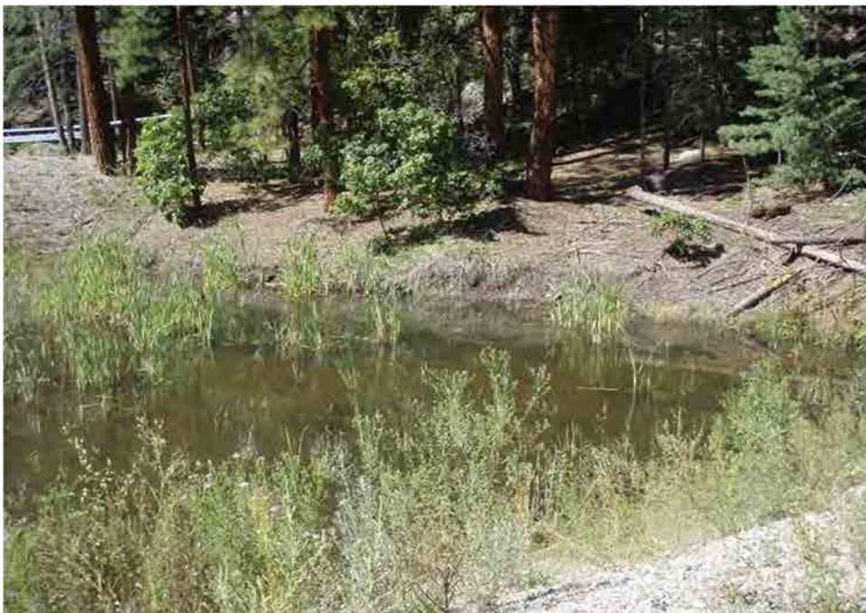
Photo C-3.4-4 Sept 2016 — Sloughing on north bank present (unchanged from previous inspections). Pounded water still present. Battery boxes still present in pond. Recommend removal of debris
