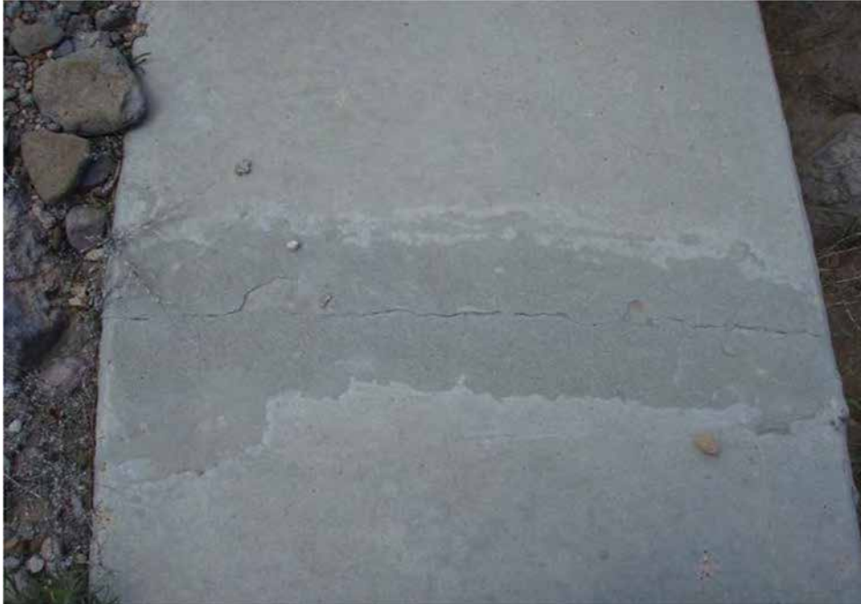
Photo C-5.4-2 June 2016 — Cracking/spalling occurring across the crest in several locations. One significant crack is present; however, no apparent settlement of the crest is noted. Consistent with previous inspection. Recommend monitoring.
