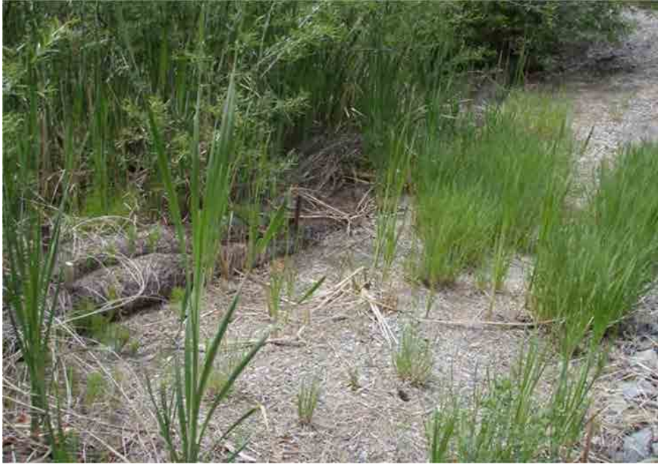
Photo C-3.8-2 June 2016 — Deteriorating wattles downstream of lower spillway at entrance to wetlands. Recommend repairing deteriorated wattles.
