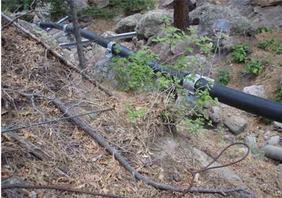
Photo C-3.10-1 June 2016 — Uppermost support cable shows fraying and corrosion (fraying not pictured). Recommend monitoring cables.
