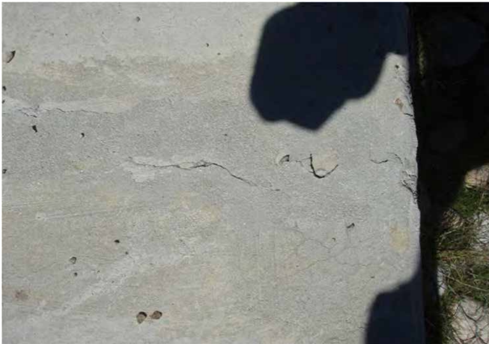
Photo C-5.4-3 Sept 2016 — Cracking across crest in several locations. Consistent with previous inspection. Recommend monitoring.
