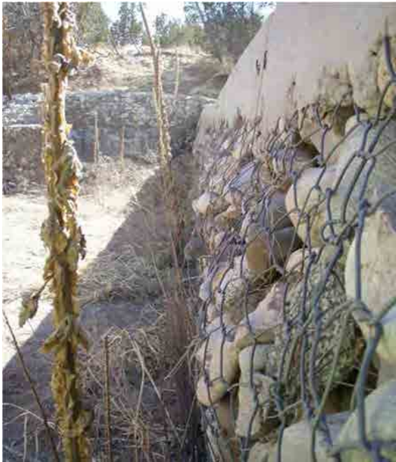
Photo C-5.6-1 March 2016 — Gabion baskets located adjacent to the overflow catchment are bowing out of alignment. No change from last inspection (Sept 2015). Recommend monitoring.
