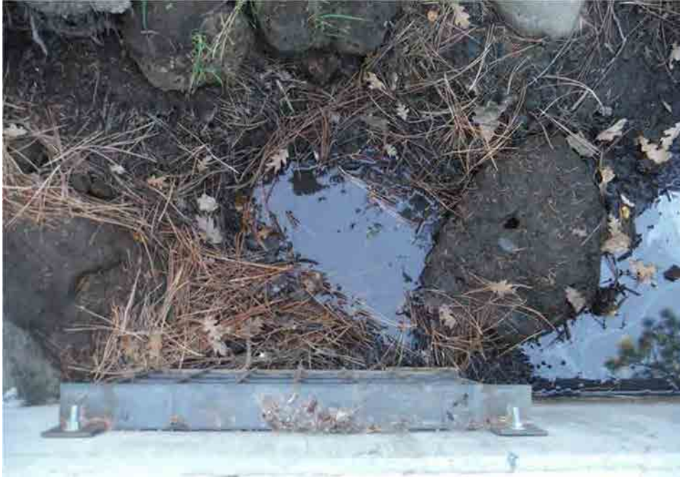
Photo C-3.14-5 Nov 2016 — Debris present at pipe inlet. Recommend removal of debris.
