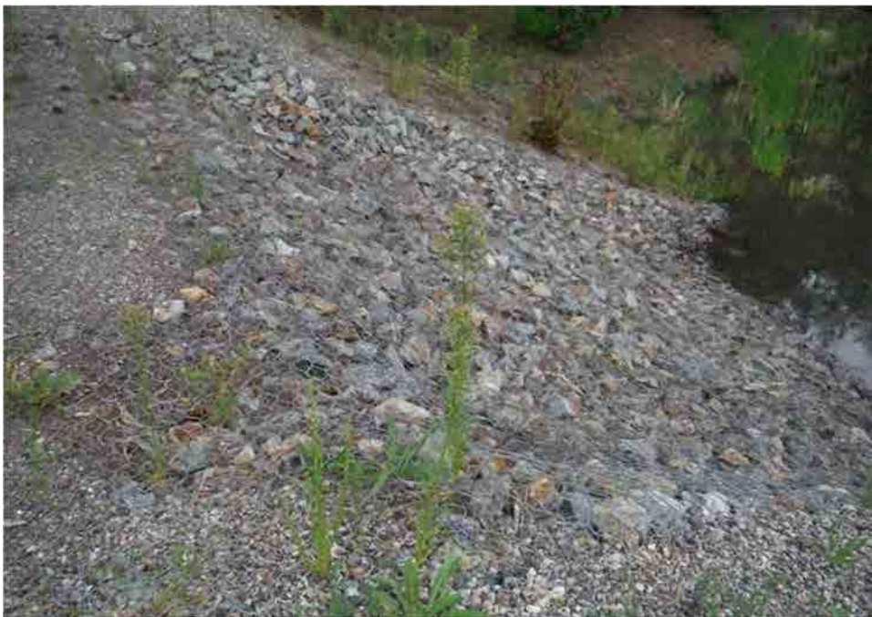
Photo C-3.5-3 Flow Event August 3, 2016 — Animal burrows still present. No change in size and shape since last inspection (Q2 2016). No evidence of flow. Recommend repair of animal burrows.
