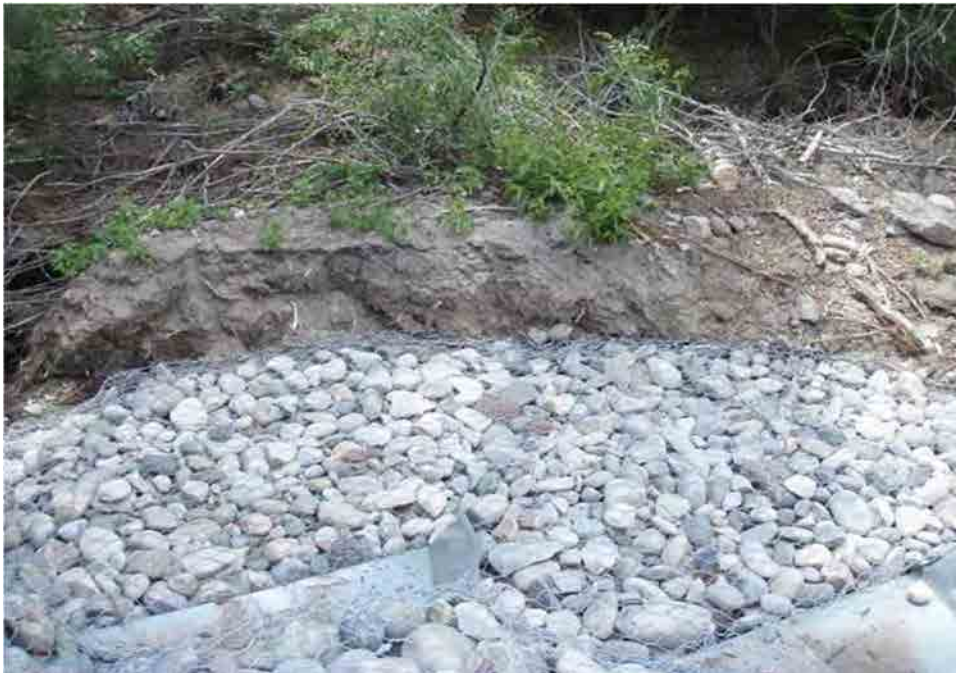
Photo C-3.17-2 June 2016 — Basin outlet area with exposed, unstable bank.
