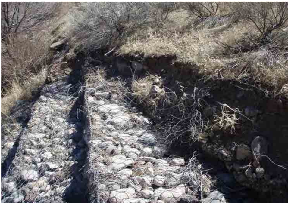
Photo C-4.5-1 March 2016 — Downstream embankments with erosion under former erosion-control blanket (ECB). Erosion could be creeping toward New Mexico Department of Transportation (NMDOT) right of way (ROW).
