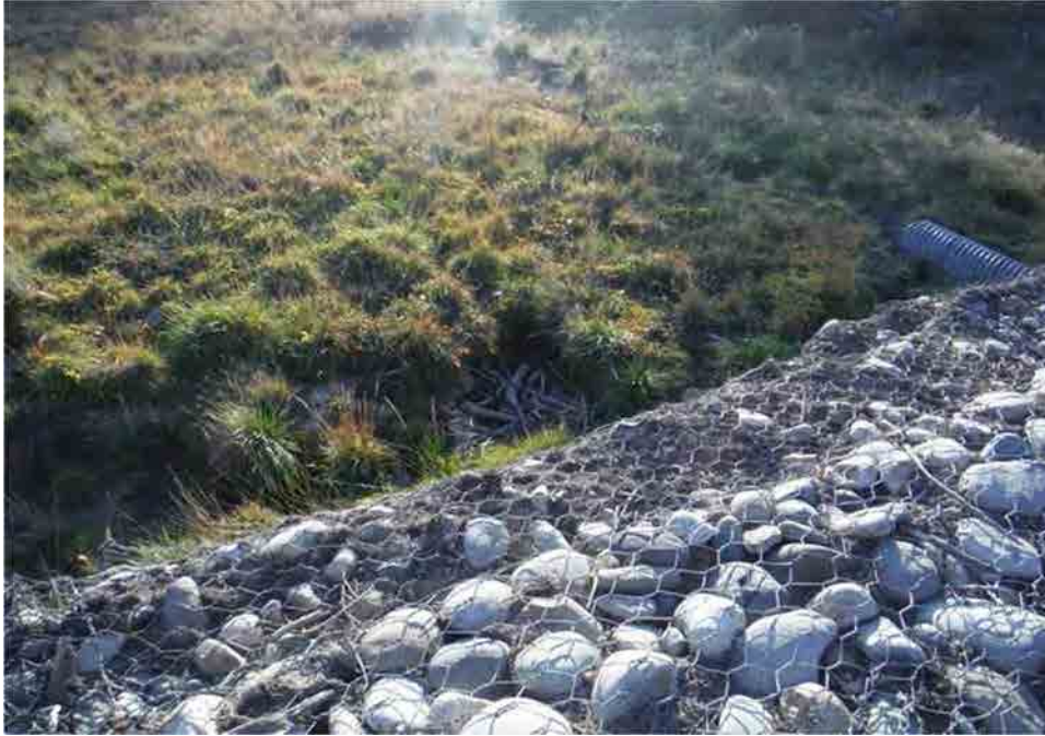
Photo C-4.6-3 Oct 2016 — Gabion baskets show undercutting and erosion immediately downstream. Conditions similar to previous inspections. Recommend monitoring.
