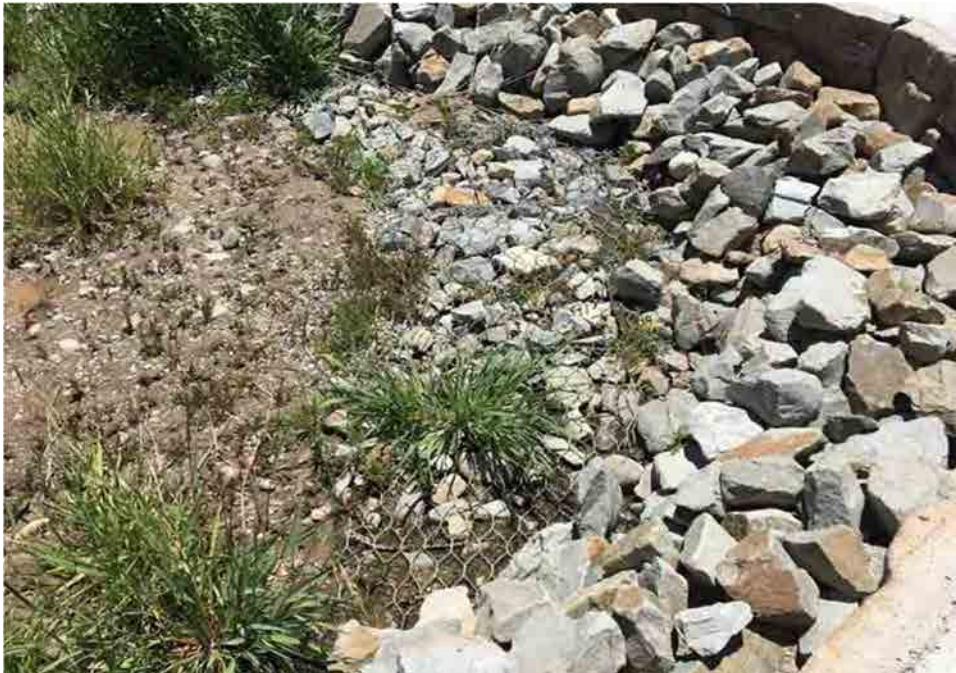
Photo C-6.6-1 March 2016 — Gabions partially covered with sediment. Recommend monitoring.
