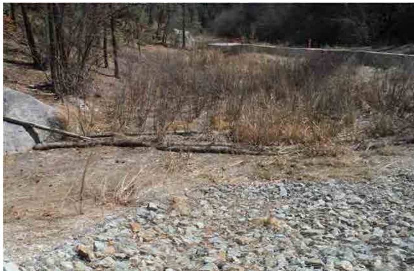
Photo C-3.8-1 March 2016 — Deteriorating wattles downstream of lower spillway at entrance to wetlands. Recommend repairing deteriorated wattles.
