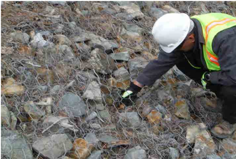
Photo C-3.3-1 March 2016 — Slumping failure of riprap below wire mesh resulting from insufficient number of wire ties to bottom mesh. Recommend repair slumping.
