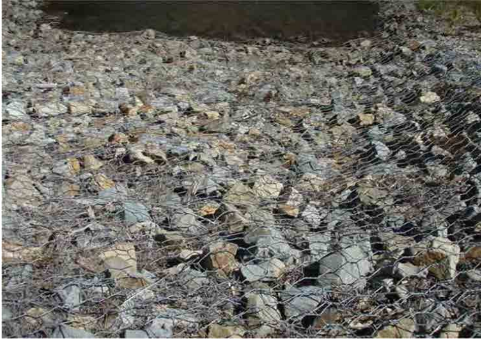
Photo C-3.3-4 Sept 2016 — Slumping on upper portion of spillway still present (consistent with previous inspection). Animal burrows present (consistent with previous inspection). Recommend repair burrows and slumping.
