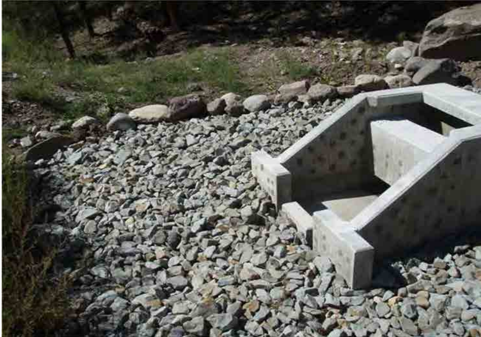
Photo C-3.15-4 Sept 2016 — Banks near pipeline outlet in need of stabilization (consistent with previous inspections). No standing water present. Recommend removal of debris.
