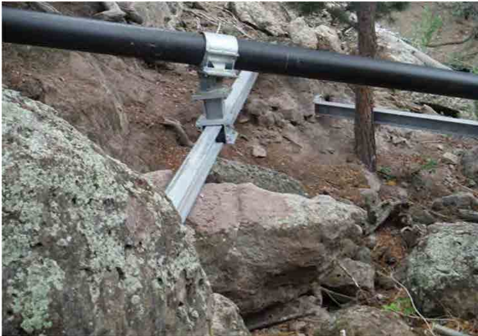
Photo C-3.11-3 Flow Event on August 3, 2016 — Lower rolling pipe support on I-beam with skewed alignment and incorrect bearing. Recommend monitoring I-beam.
