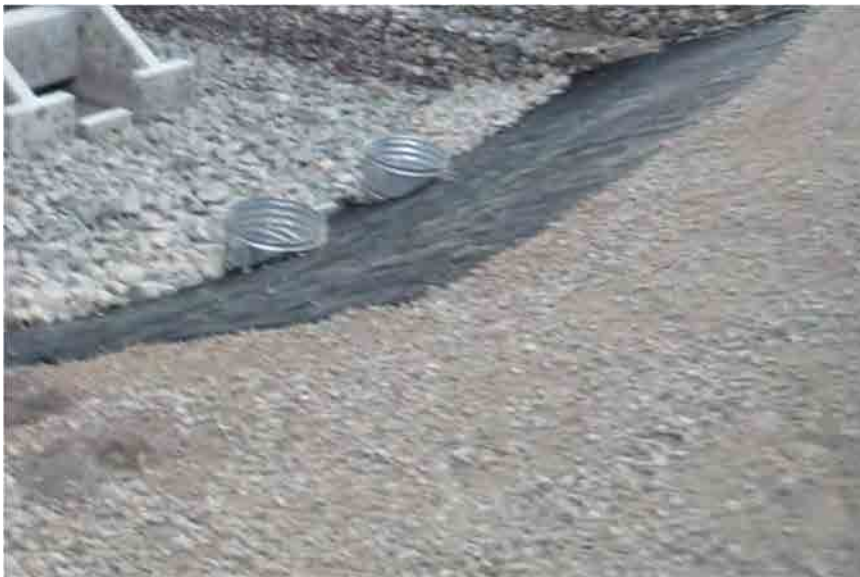
Photo C-3.18-5 Nov 2016 — Riser pipes consistent with previous inspection. Recommend installing trash racks and 3-in.-diameter holes on riser pipes.
