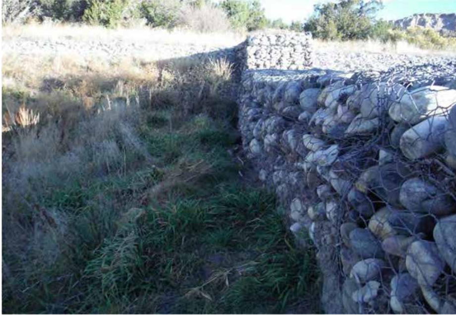
Photo C-4.10-2 Oct 2016 — Bulging gabion baskets found near areas with piping. Recommend monitoring.
