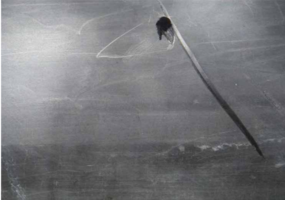
Photo C-3.9-1 March 2016 — Nick in pipe 6 ft east of pipe bridge structure. Recommend monitoring nick.
