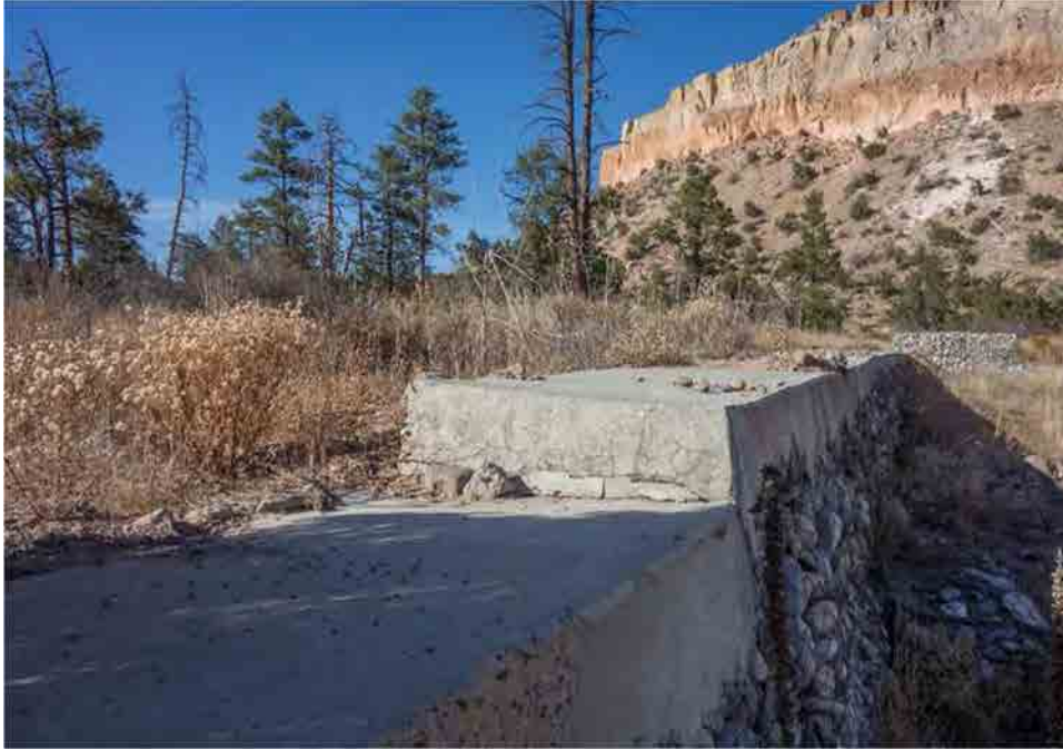
Photo C-5.3-4 Nov 2016 — Joint cracking consistent with previous inspection. Recommend monitoring.
