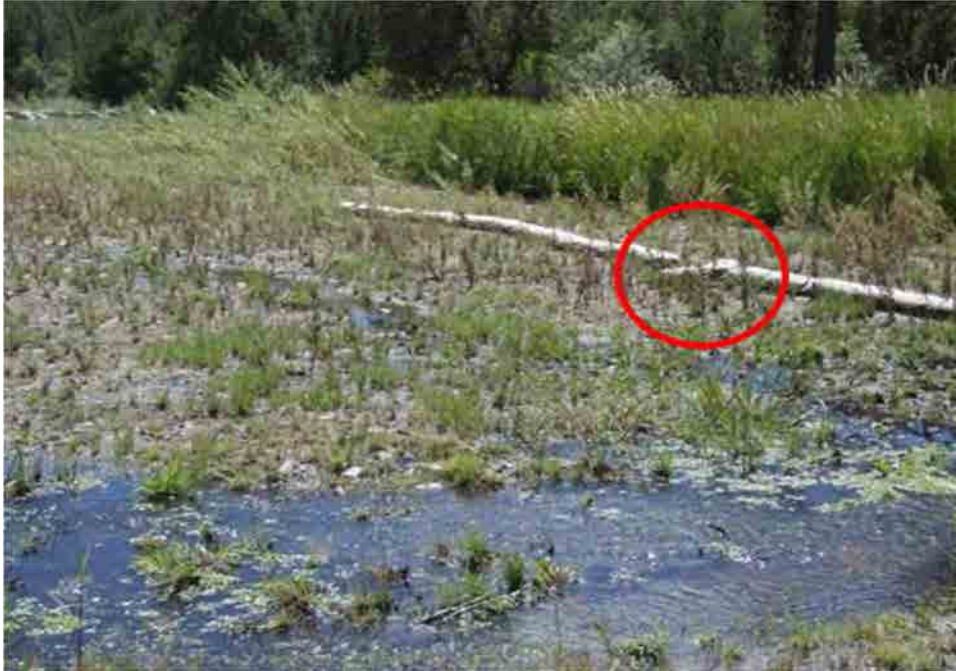
Photo C-6.3-3 Sept 2016 — Spreader sand bags installed since last inspection. Several have been moved, allowing channelization to continue, and one is damaged (noted in red circle). There is evidence of improved sheet flow.
