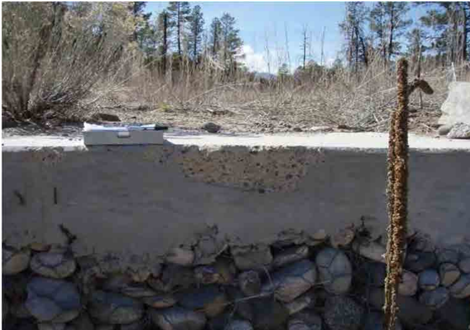
Photo C-5.5-1 March 2016 — Spalling present on the downstream side of the spillway crest. Recommend monitoring.
