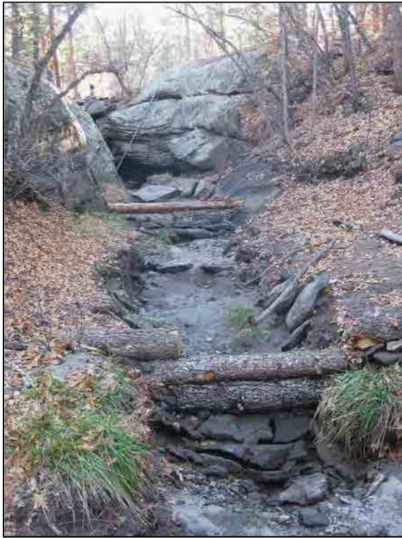
Photo A1-27 Rock armoring along stream banks in the south fork of Acid Canyon: (a) looking upstream in April 2016 and (b) log check dams in November 2016
