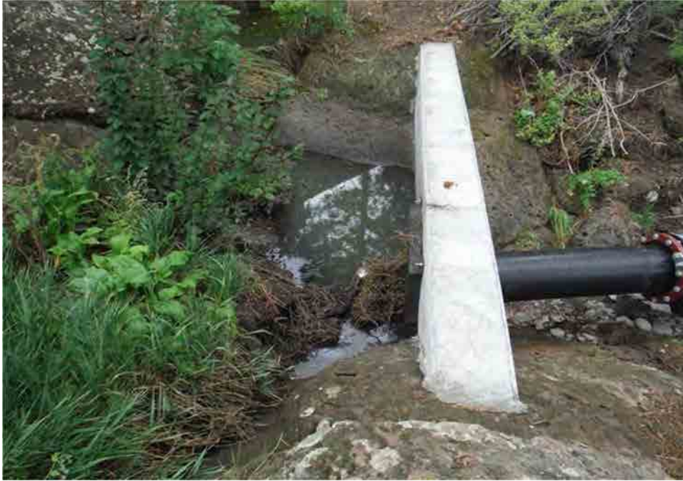
Photo C-3.14-3 Flow Event on August 3, 2016 — Pipe inlet plugged with debris from recent rain event. Recommend removal of debris.
