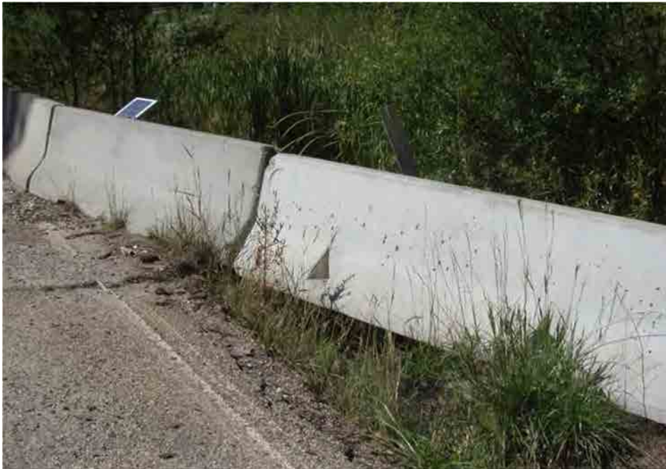
Photo C-3.19-4 Sept 2016 — Road collapse under Jersey barrier (consistent with previous inspection). Recommend repair of road.
