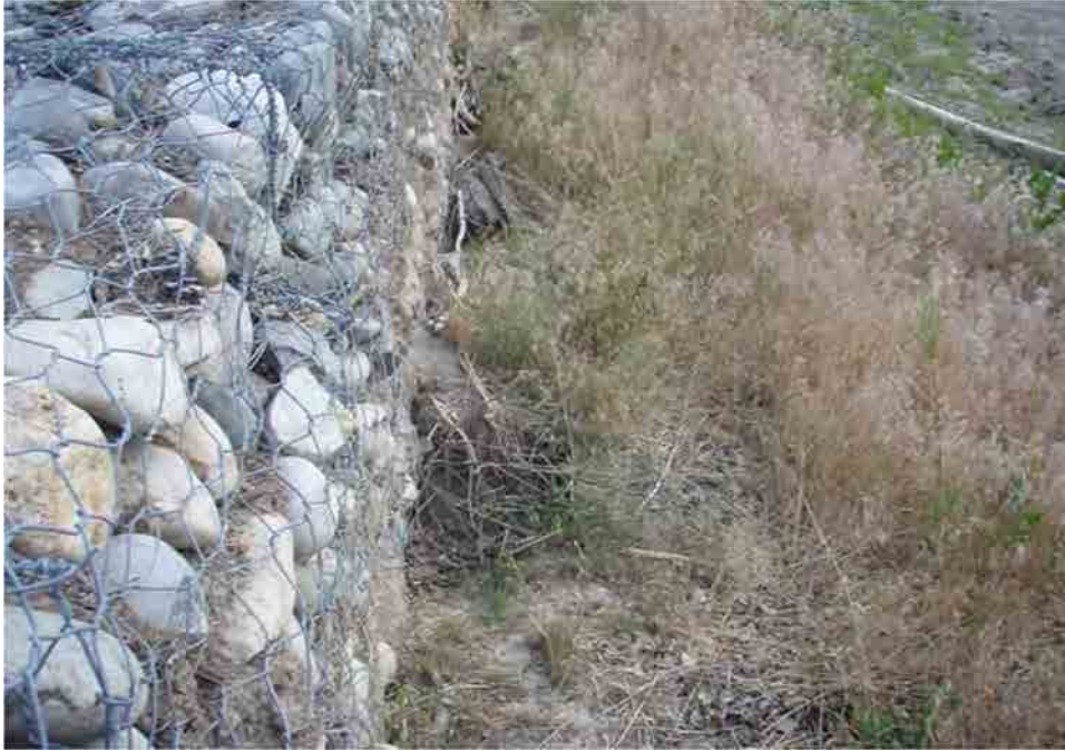
Photo C-4.7-2 June 2016 — Piping erosion consistent with previous inspections. Recommend monitoring.
