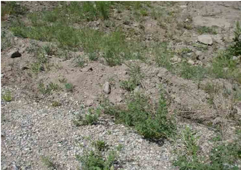
Photo C-3.2-2 June 2016 — Construction spoils remaining from pipeline construction still present. Recommend removal of construction spoils.
