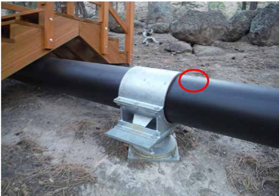
Photo C-3.9-5 Q4 — Nick in pipe found 6 ft east of pipe bridge structure (circled in red). Recommend monitoring nick.
