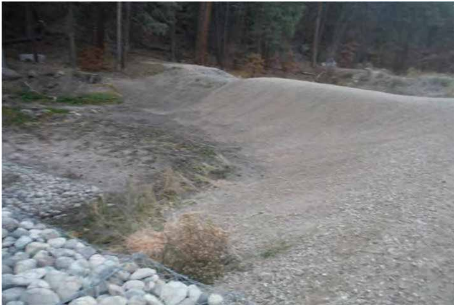
Photo C-3.2-4 Sept 2016 — Recent maintenance removed pipeline construction spoils and placed north of pond with seed and mulch.
