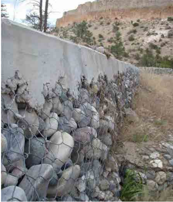
Photo C-5.6-2 June 2016 — Gabion baskets located adjacent to the overflow catchment are bowing out of alignment. No change from last inspection. Recommend monitoring.
