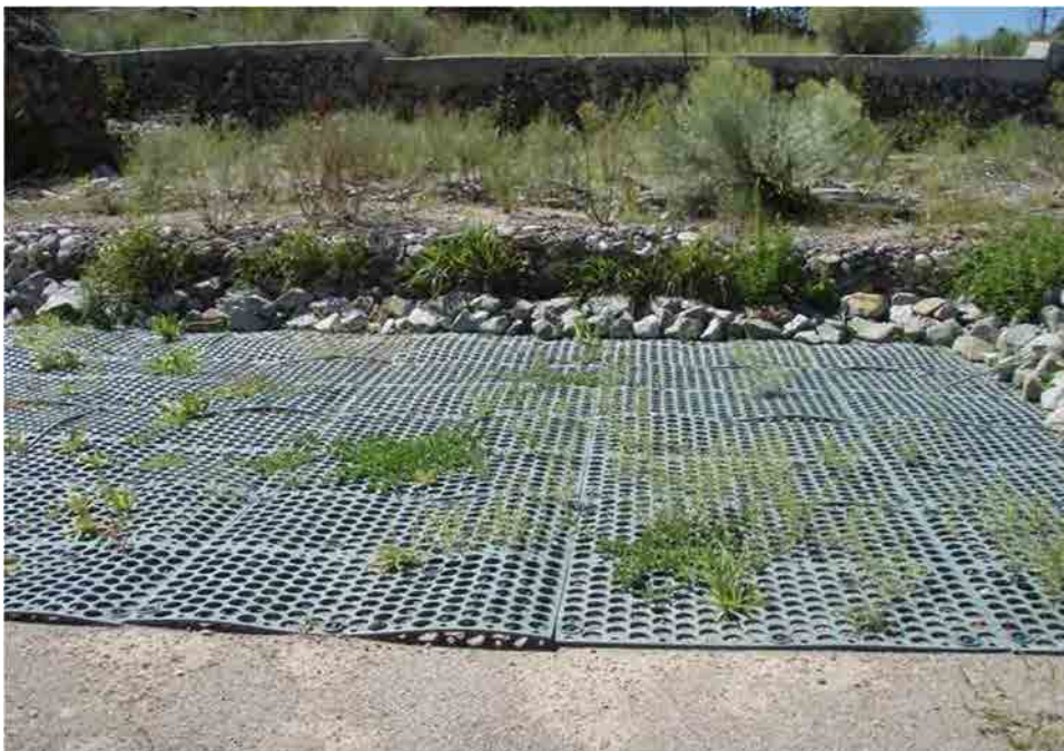
Photo C-5.9-3 Sept 2016 — ScourStop consistent with previous inspection. Recommend monitoring.
