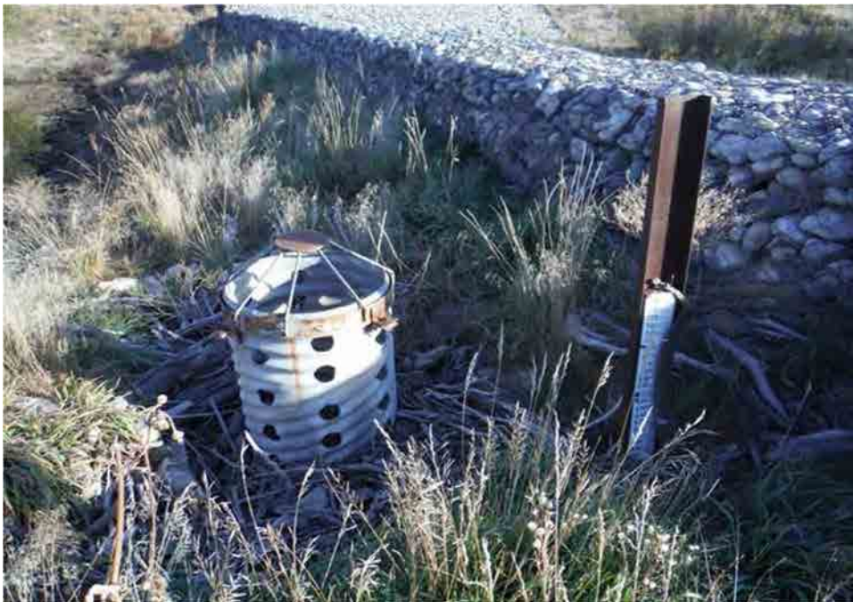
Photo C-4.1-3 Oct 2016 — Standpipe is unobstructed for top four holes. Staff gage reads 5.8 ft. Note: Though piping could be discouraged by clearing debris from around the standpipe, the New Mexico Environment Department wants all water upstream of the weir to filter through the gabions.
