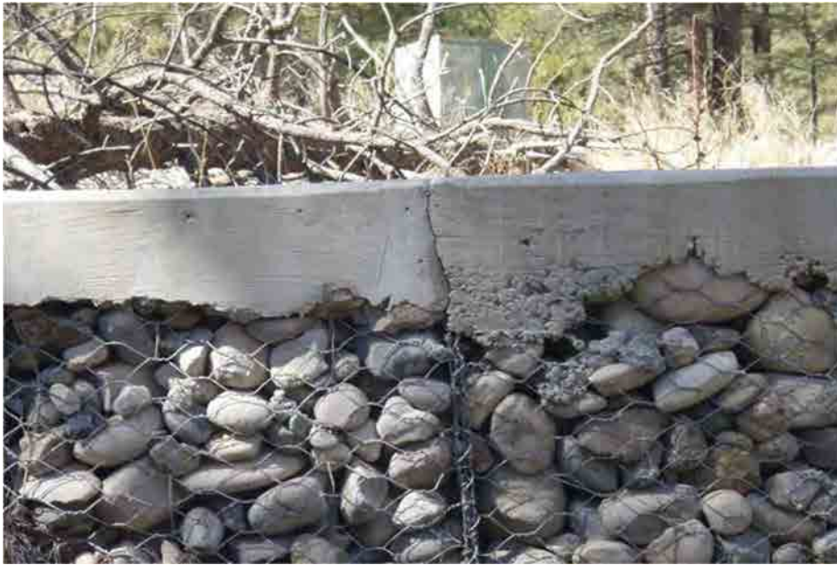
Photo C-2.3-1 March 2016 — Cracks are consistent with previous inspection. Recommend monitoring.
