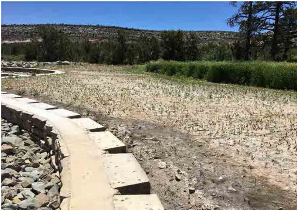
Photo C-6.4-2 June 2016 — Upstream side of upper Redi-Rock structure with settling and erosion. Recommend repairing.
