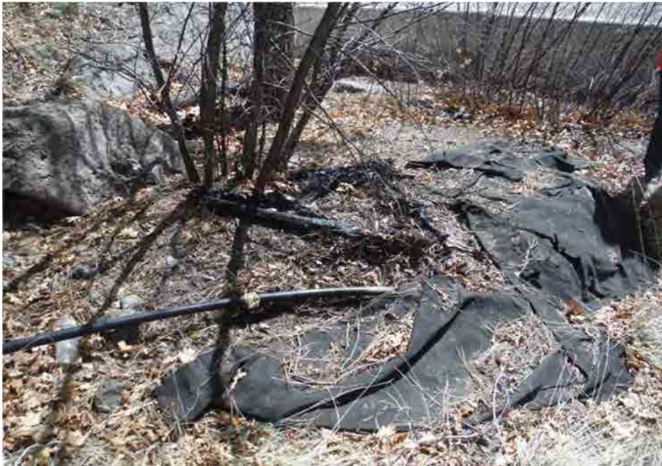
Photo C-3.7-1 March 2016 — Silt fence and pipe materials (construction debris) at southeast side of the wetland pond, near sampler. Recommend removing debris and monitor geotextile.
