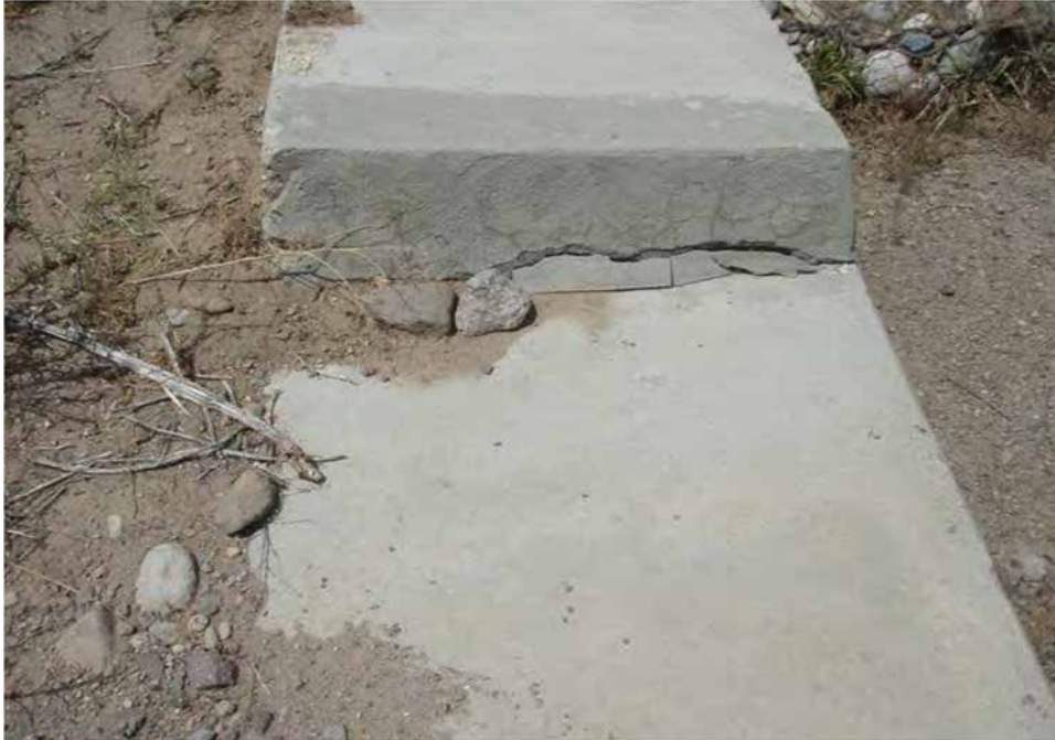
Photo C-5.3-2 June 2016 — Cracking occurring at the joints on the spillway. No change from previous inspection. Recommend monitoring.
