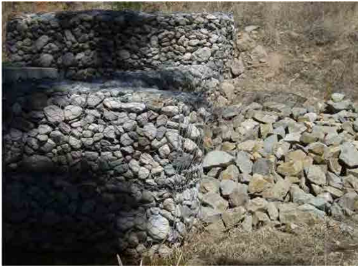
Photo C-2.5-1 March 2016 — Bulging gabion basket located on the downstream face and below crest of weir. Consistent with previous inspection.
