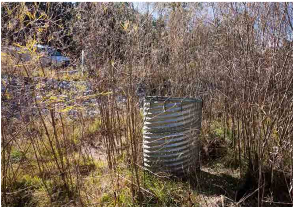
Photo C-2.4-3 Nov 2016 — Approximate height between channel bed and top of weir is 3.5 ft (unchanged from last inspection [Q2 2016]). Tire is still present in the standpipe. Recommend monitoring and removal of tire.
