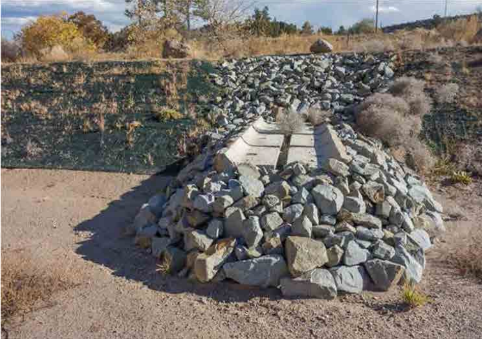
Photo C-5.10-4 Nov 2016 — Rilling occurring at the tip of Spur 4. Consistent with previous inspection. Recommend monitoring.
