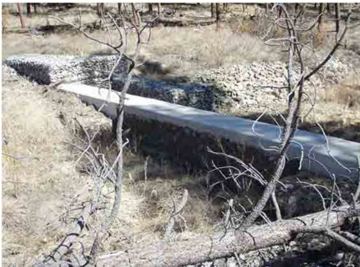
Photo C-2.6-1 March 2016 — Large tree and woody debris shown on upstream slope face of weir. Recommend removal of tree.
