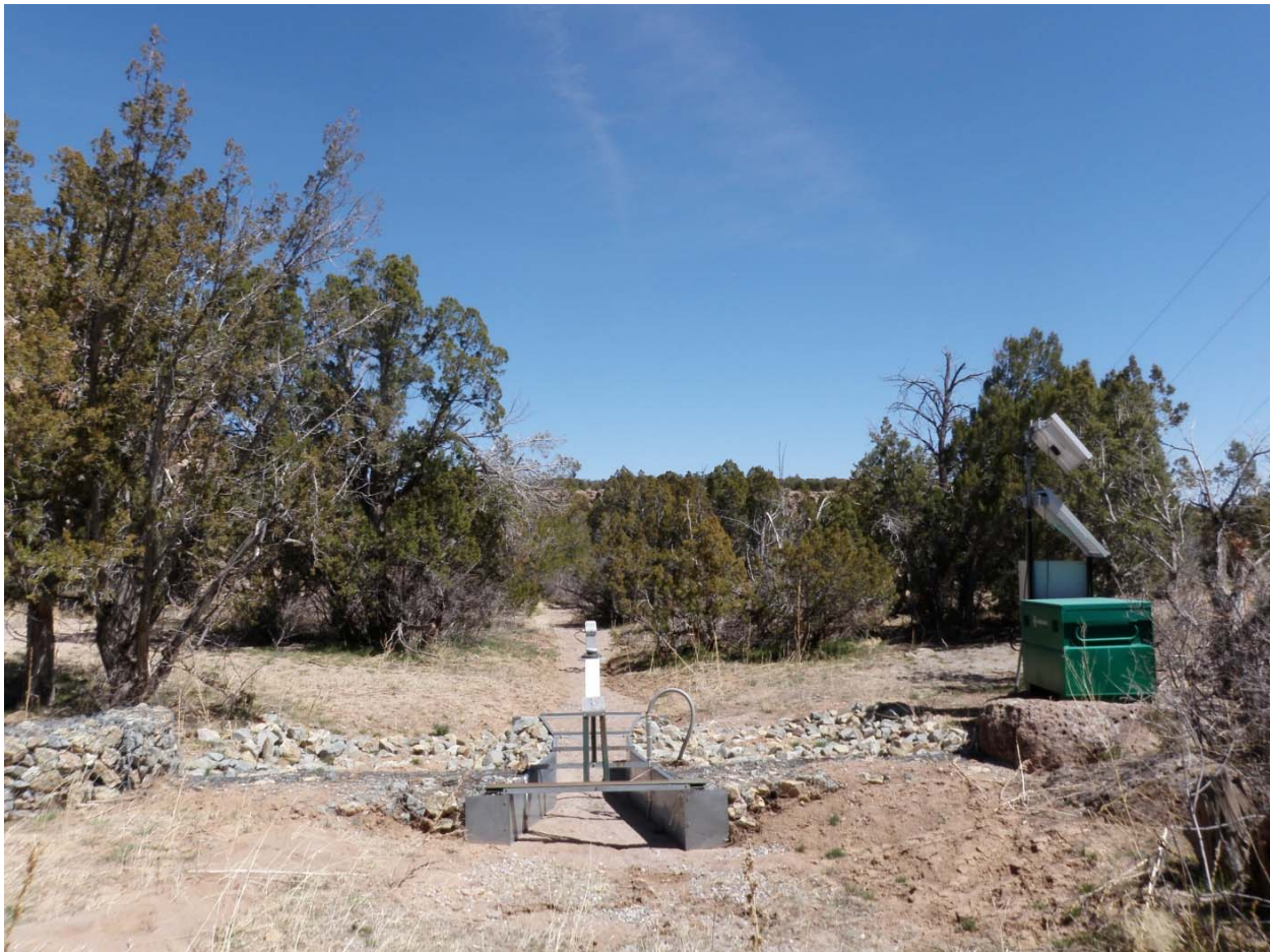
E229.3 Stream gage downstream view
