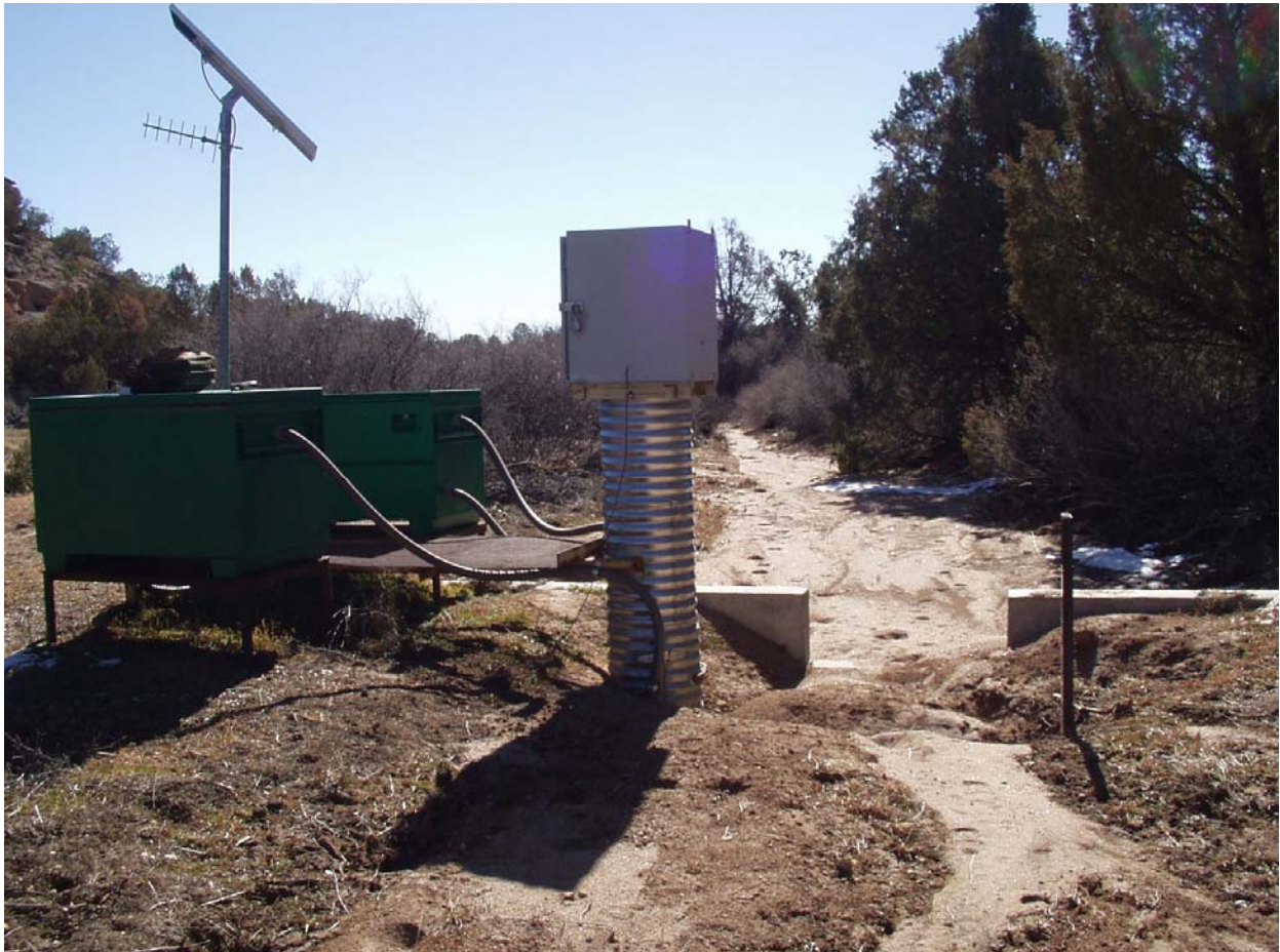
E267 Stream gage downstream view
