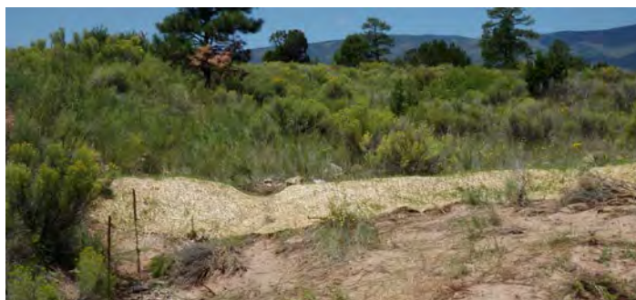
3M-SMA-0.4, Earthen Berm, H00203010003 (photo ID 8517-1)
