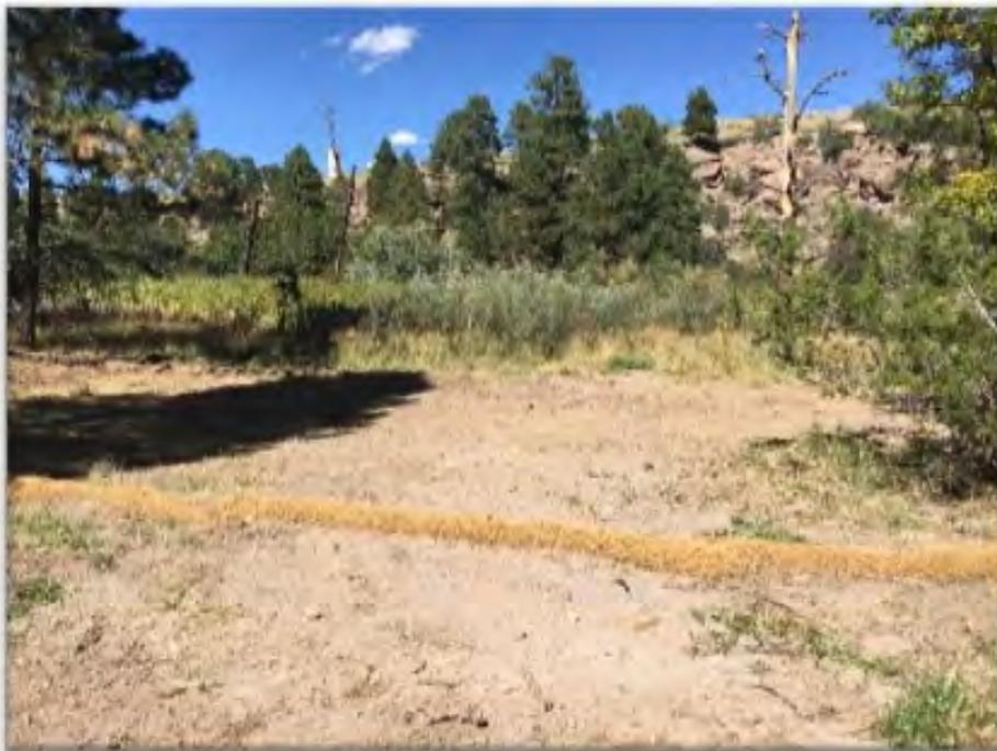
**Figure E-2.1-5** September 2017: A line of coir logs were installed to allow for both velocity dissipation and sediment capture.
