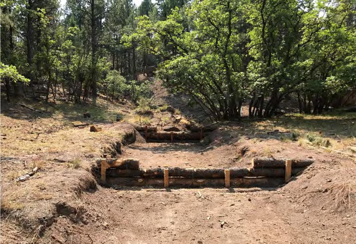
**Figure E-2.1-2 September 2017: View of newly installed log check dams looking upstream**
