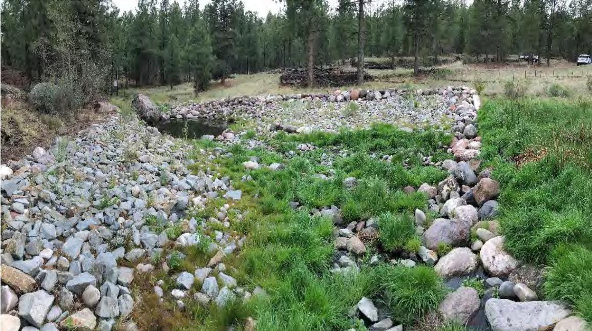
**Figure E-3.6-1 May 2017: Slight vegetation establishment in rip rap. Structure is working as designed with no evidence of channelization.**
