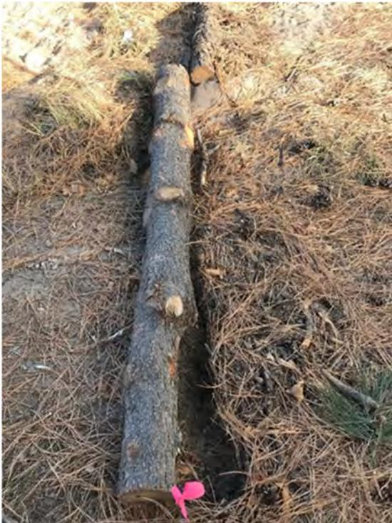
**Figure E-2.1-7** December 2017: Flow spreader logs displaced during flow event. Logs were replaced and keyed in with riprap during January 2018 maintenance. Looking east.
