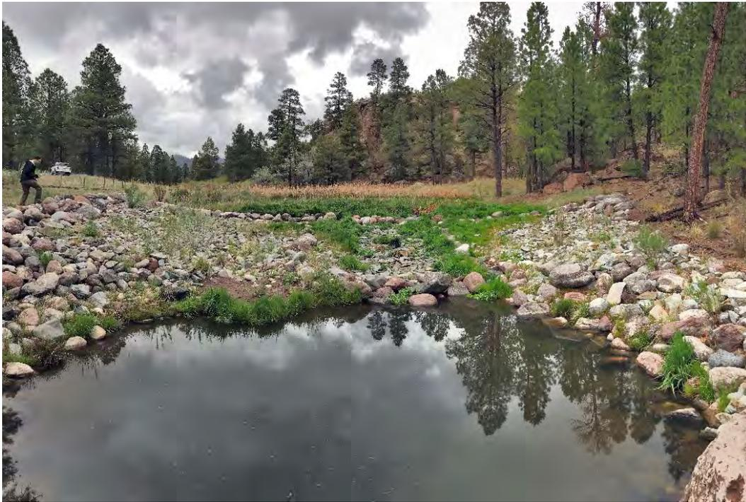
**Figure E-3.7-1** May 2017: Cascade structure working as designed. No evidence of rock displacement. No evidence of erosion in/near cascade pool.
