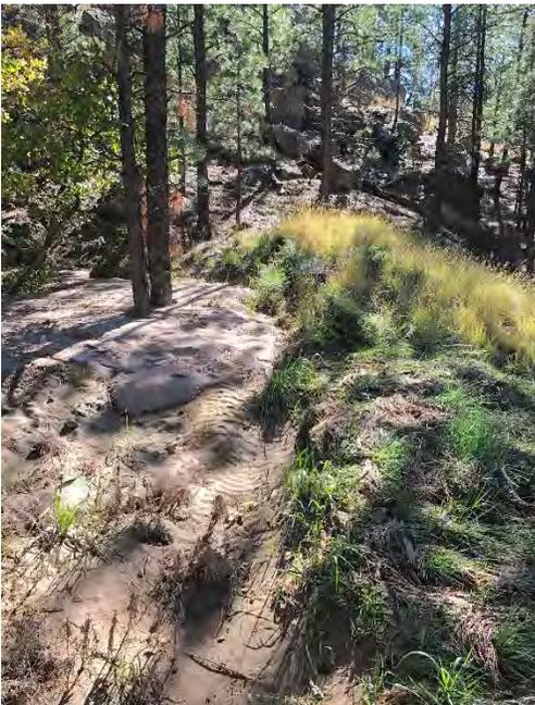
**Figure E-3.8-2 October 2017: Slightly less capacity than last site inspection. Control still has capacity for sediment capture. Better established vegetation on downgradient hill-slope since last visit.**
