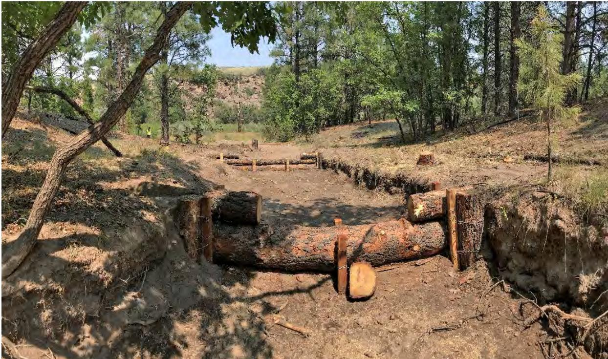
**Figure E-2.1-1** September 2017: The two log check dams were installed to capture sediment originating from an erosion feature upgradient of the controls. Picture looking toward the wetland/downstream.
