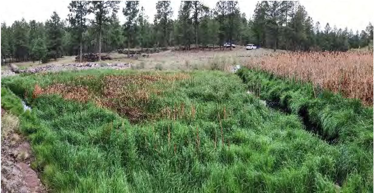
**Figure E-3.5-1** May 2017: Wetland vegetation well established. Dispersing flow evenly throughout GCS. No evidence of channelization. No evidence of cracking or spalling on concrete wall.
