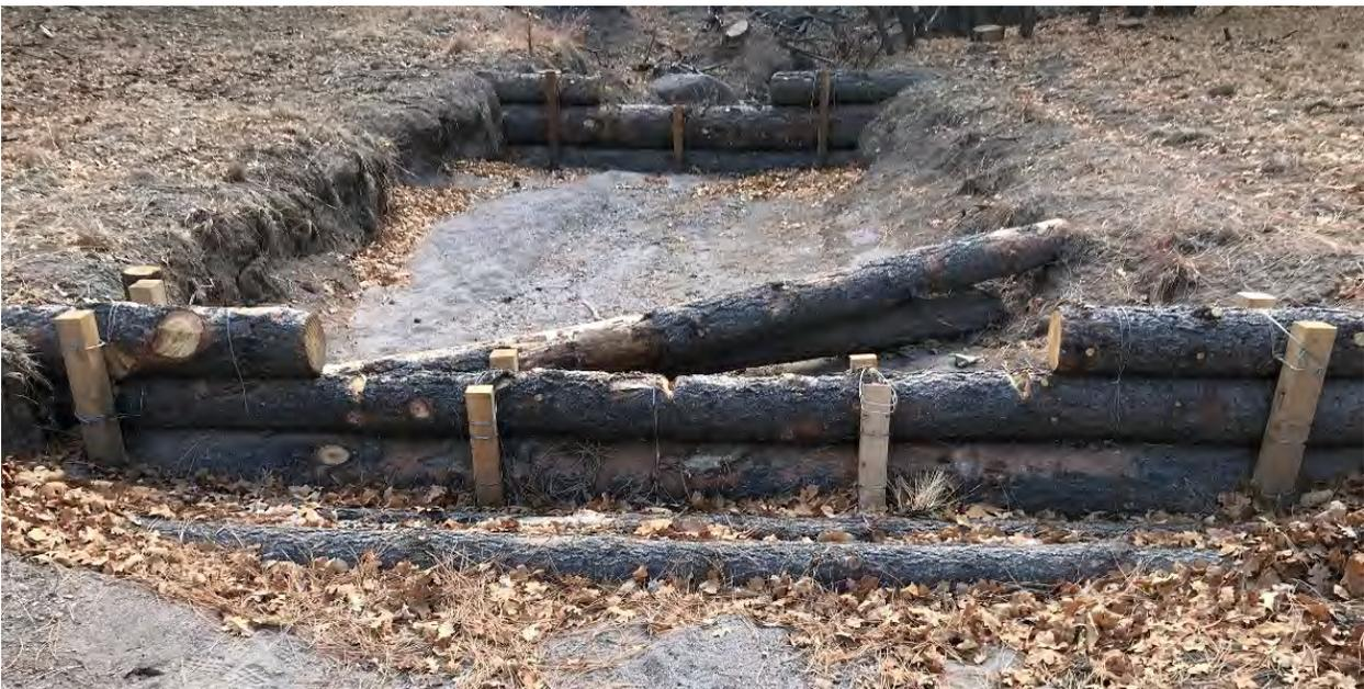
**Figure E-2.1-3 December 2017: View of failed log check dams with displaced scour protection logs. Looking upstream.**
