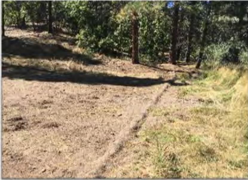
**Figure E-2.1-6** September 2017: Logs were trenched end-to-end to create a flow spreader. This control will encourage sheet flow into the wetland, rather than allowing more erosive concentrated flows. Looking west.
