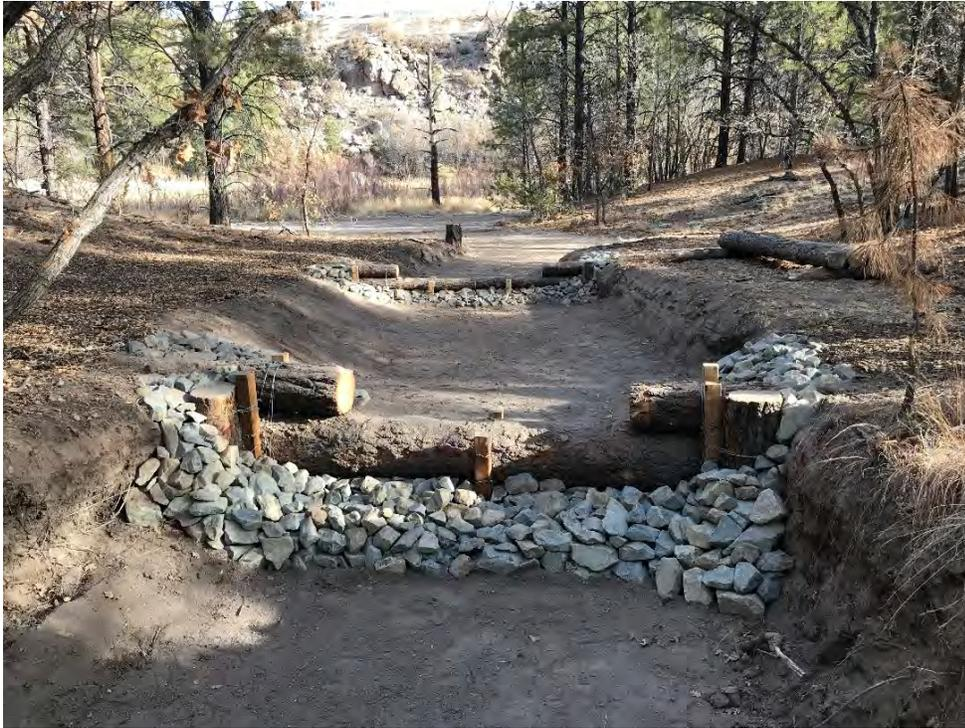
**Figure E-2.1-4** January 2018: View of repaired log check dams with additional riprap erosion protection. Looking downstream.
