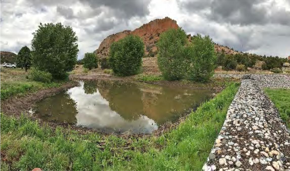
**Photo C-4.7-1 May 2017—Areas where piping was previously noted have been either sedimented in or filled with woody debris. Recommend monitoring.**
