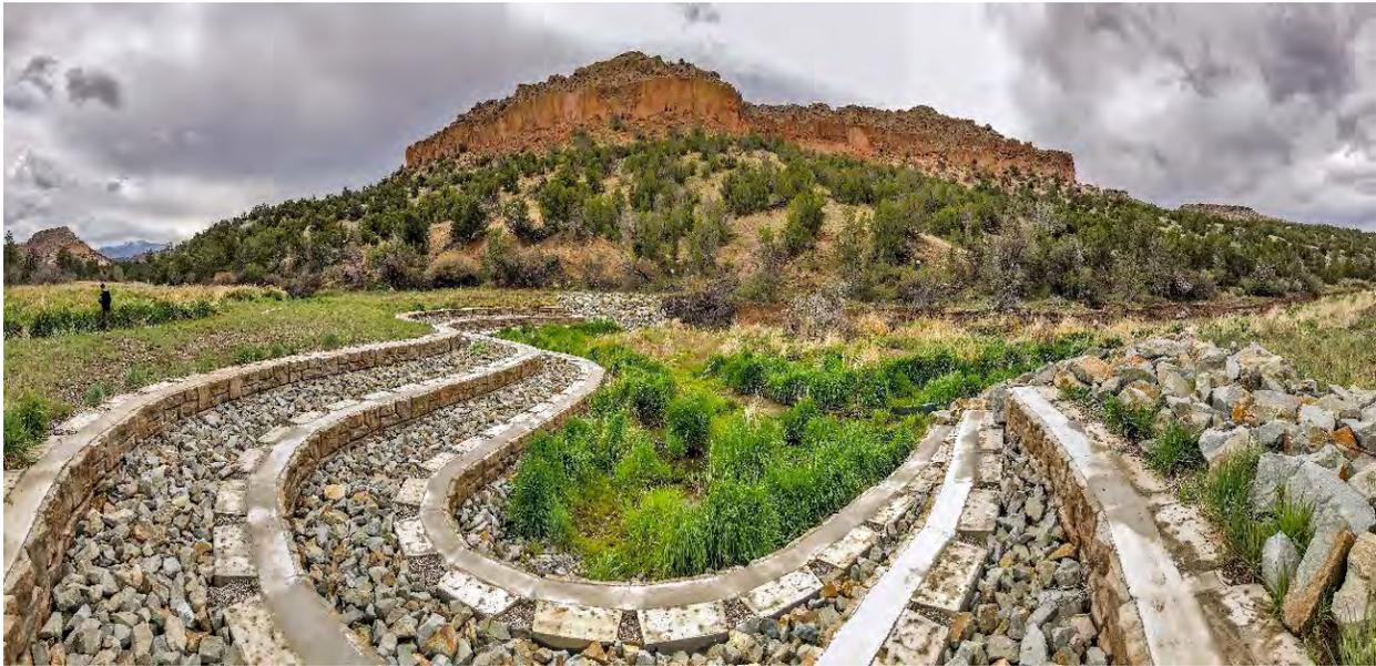
**Photo C-6.1-1 May 2017—Redi-Rock structure shows no evidence of displacement or settling. Reed canary grace is well established both upstream and downstream of control.**
