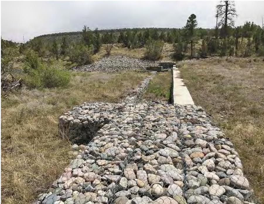
**Photo C-5.2-1 May 2017—Well-established vegetation surrounding control. No presence of trash/debris. Several rodent burrows noticed along control but appear to have no impact on abutment. Continue to monitor.**
