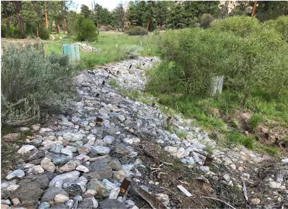
**Photo C-2.1-1** May 2017—Embankment is stable and operating as designed. Well-established vegetation with no erosion occurring from hillslope. Some woody debris located on riprap. Removed debris while on site.
