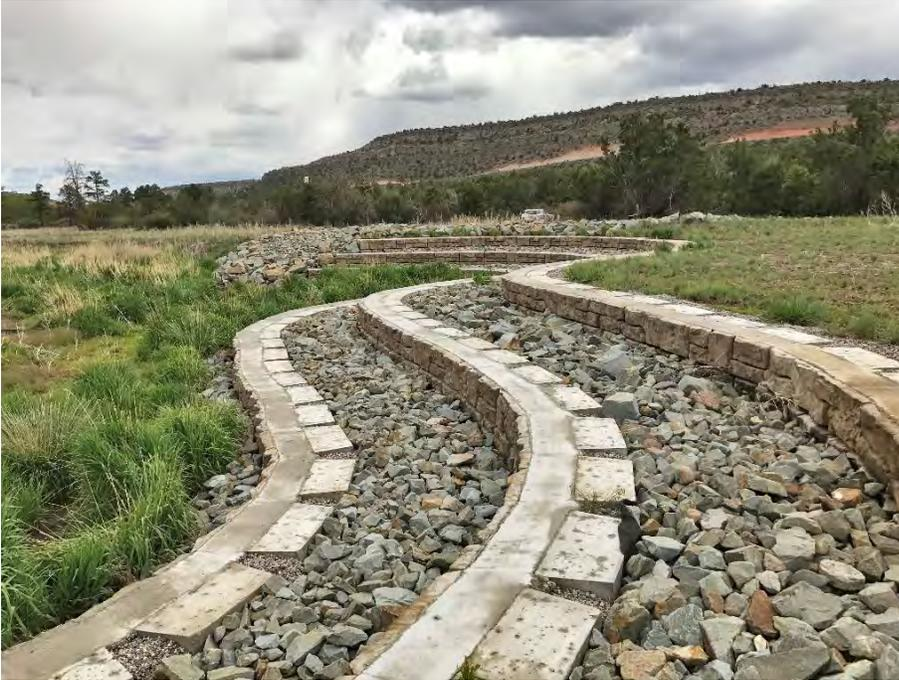
**Photo C-6.4-1 May 2017—Upstream vegetation is minor. Minor channelization occurring from upstream flow. Established vegetation upstream of control would help disperse flow.**
