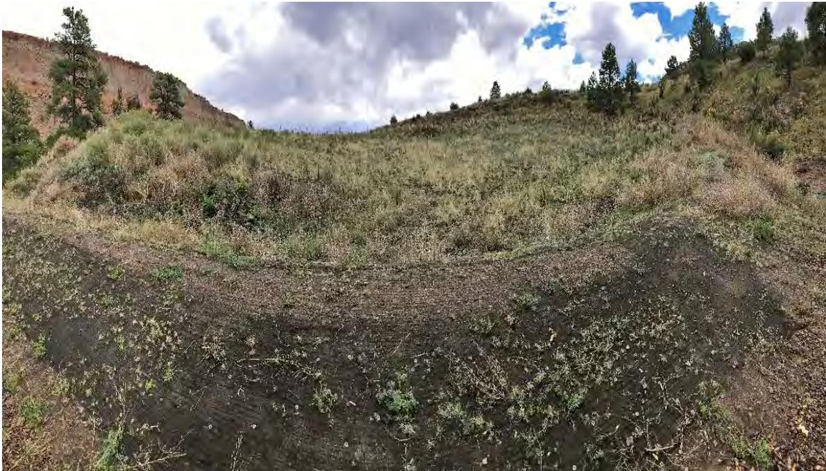
**Photo C-4.9-1 May 2017 —The borrow pit runoff control berm is operating effectively. Sediment accumulated behind berm is stable with thick established vegetation.**
