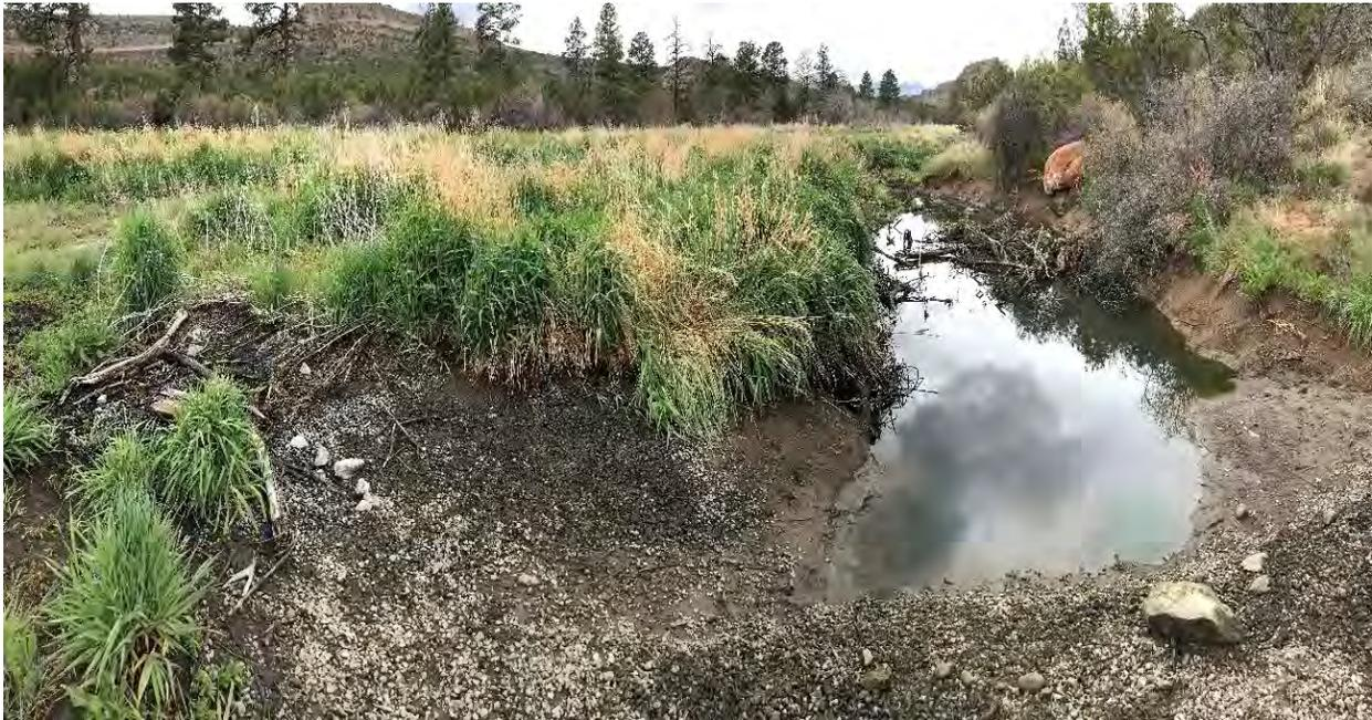
**Photo C-6.5-1** May 2017—Roughly 2 ft of water in upstream wetland area. Sediment capacity at roughly 30 percent.
