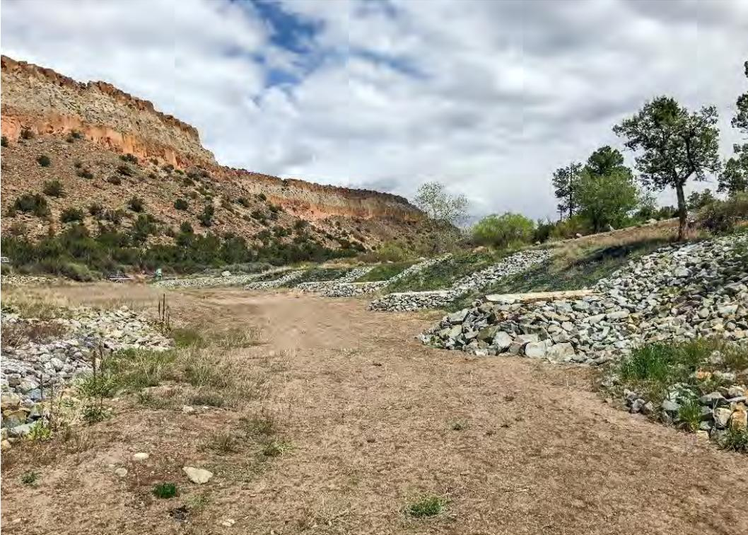
**Photo C-5.5-1 May 2017—Well-established vegetation along all hillslopes. No erosion apparent along slopes or near TRM matting. All structures functioning as designed.**
