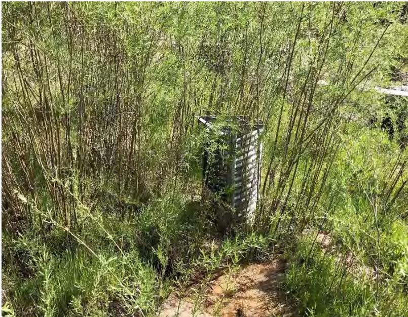
**Photo C-2.6-1** May 2017—No sediment intrusion into standpipe and debris (tire) has been removed from structure. No apparent corrosion to standpipe.
