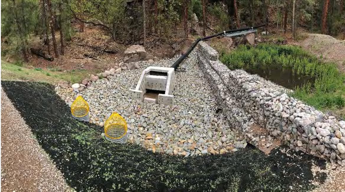
**Photo C-3.7-1** May 2017—Pipeline outlet and energy dissipater is clear of debris with minor established vegetation occurring through turf reinforcement matting (TRM). Culvert outlet and inlets appear functional.
