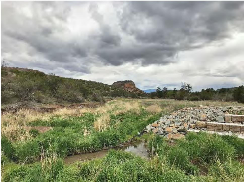
**Photo C-6.3-1 May 2016—Reed canary grass well established. Structure functioning as designed with no evidence of erosion where riprap is located.**
