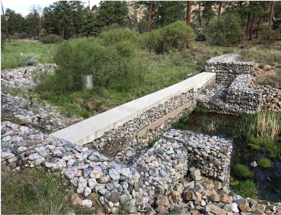
**Photo C-2.5-1 May 2017—Crest of structure is in alignment with no visual deformities.**
