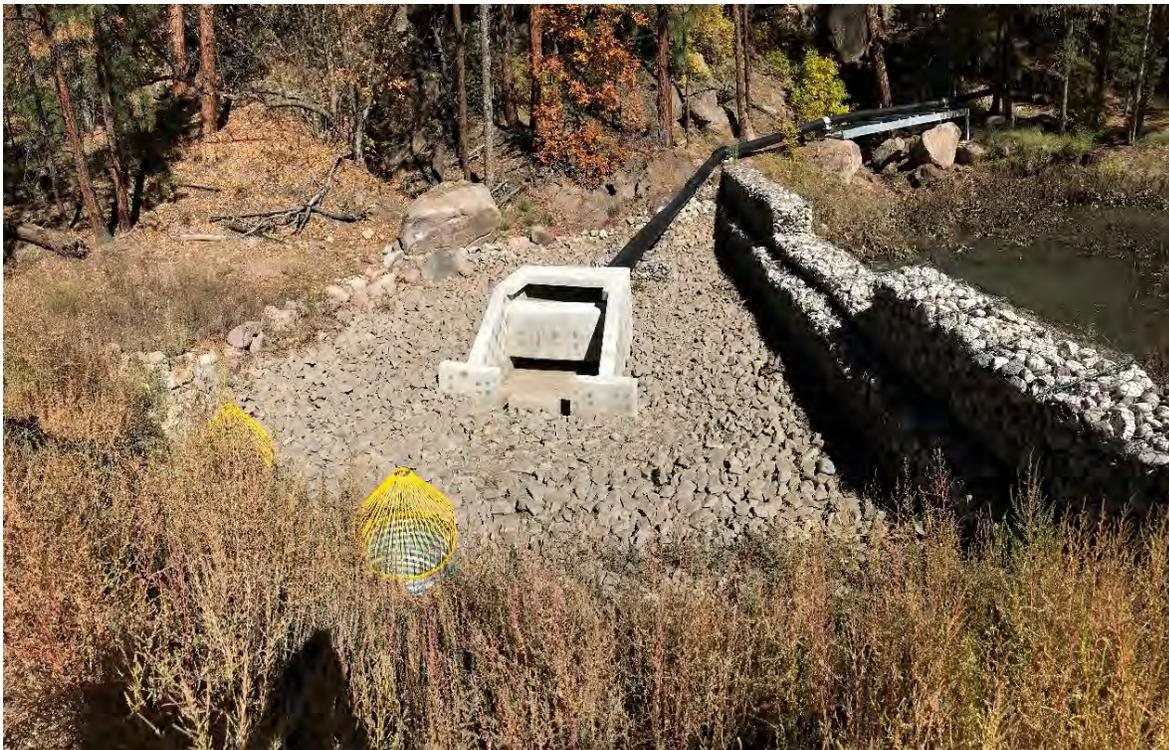
**Photo C-3.7-2** October 2017—Thick established vegetation on TRM-lined slope. Retention area has minor layer of sediment. All outlets and inlets functioning as designed.
