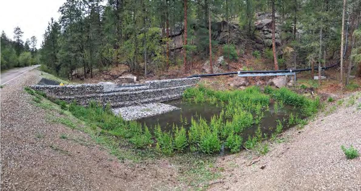
**Photo C-3.2-1 May 2017—No breaching/slides/cracks/sloughs present on embankment and pond. No erosion occurring on slope. No trash or debris present in control.**
