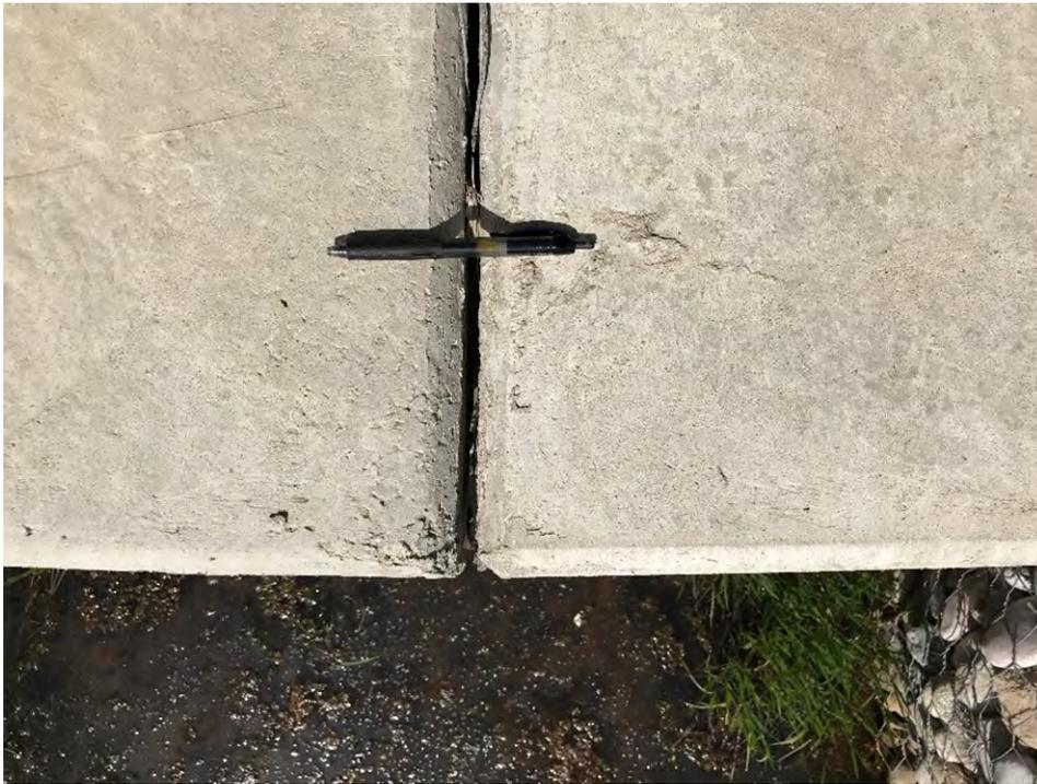
**Photo C-2.4-1** May 2017—Separation of concrete has not changed from inspections conducted in 2016. Will continue to monitor for changes.
