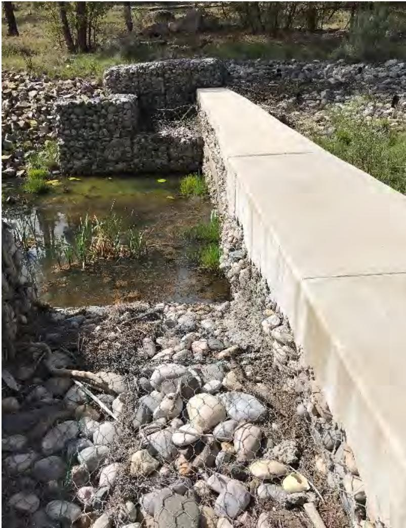
**Photo C-2.3-1** May 2017—No deteriorated joints present on upslope side of weir. Minor bulging of a gabion basket but gabion basket is still structurally intact and in stable condition. Will continue to monitor for changes.
