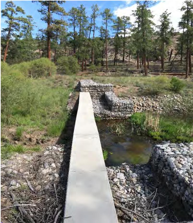
**Photo C-2.7-1 May 2017—Spillway operating as designed. No signs of improper alignment, deterioration, or trash/debris on spillway.**
