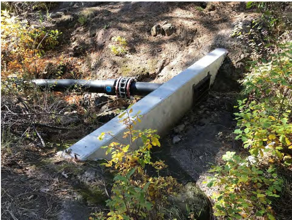
**Photo C-3.5-2** October 2017—Removed needlecast and minor trash buildup behind culvert intake. No change in condition from the last inspection (May 2017).
