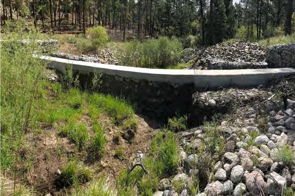
**Photo C-2.2-1 May 2017—Upslope face of weir at roughly 50 percent capacity for sediment storage. Operating effectively. No structural issues identified during inspection.**
