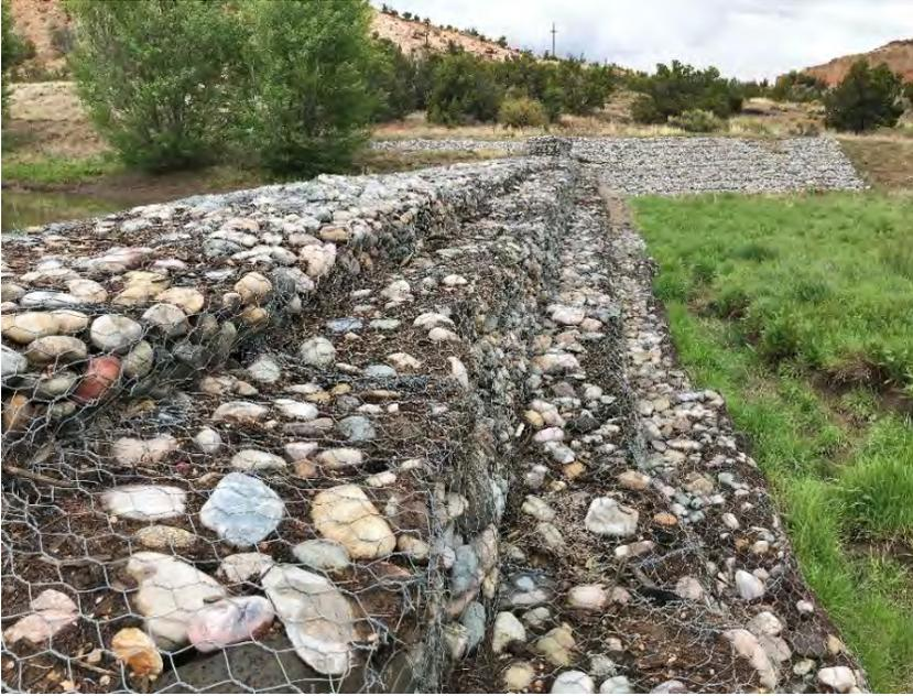
**Photo C-4.3-1** May 2017—No erosion or sloughing of gabion baskets occurring. All gabion baskets appear to be structurally intact and operating as designed. Minor gully forming downgradient of control. Continue to monitor.
