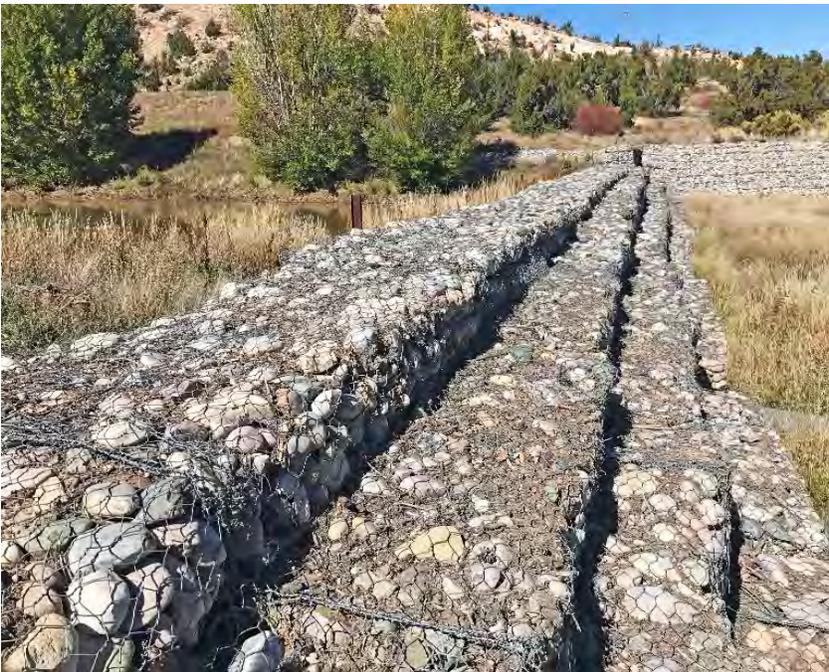
**Photo C-4.3-2** October 2017—Sediment and established vegetation have filled in areas of previously inspected gully. No other changes noted in condition from the last inspection (May 2017).
