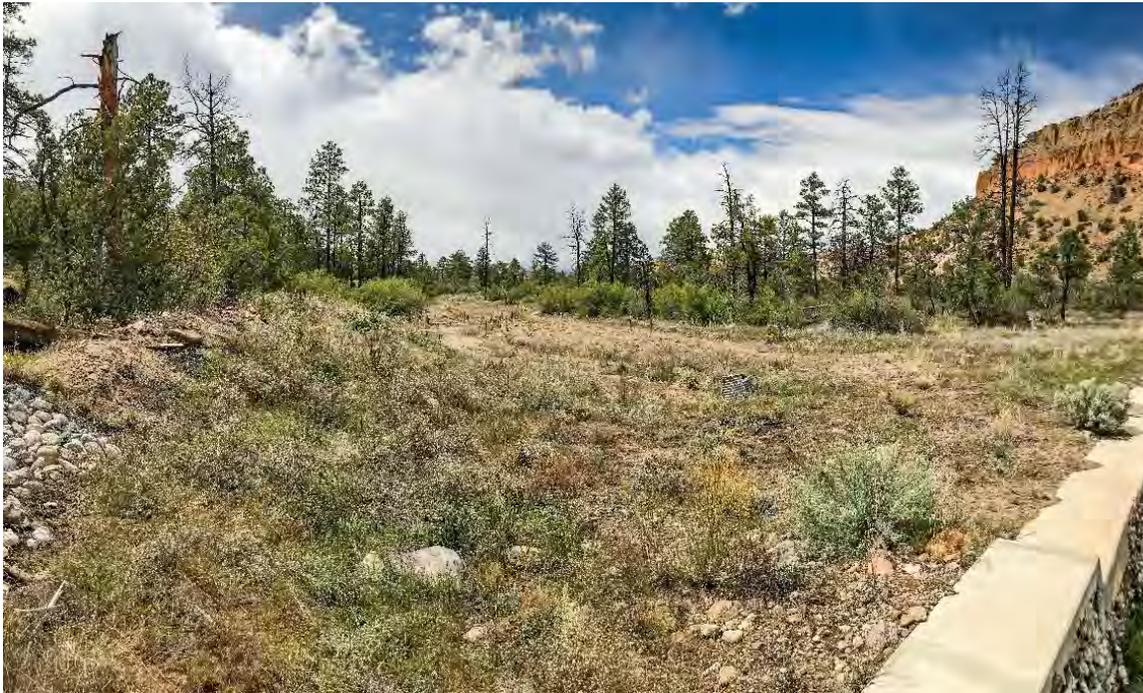
**Photo C-5.1-1 May 2017—Tire present in 2016 inspection was removed from channel. Well-established vegetation on embankment. No signs of erosion or undermining.**
