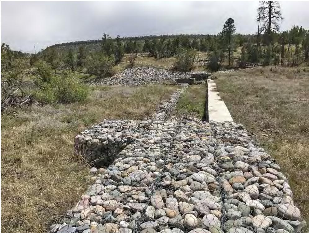
**Photo C-5.4-1** May 2017—No cracks present in concrete. Structure and gabion baskets are in alignment and functioning as designed.
