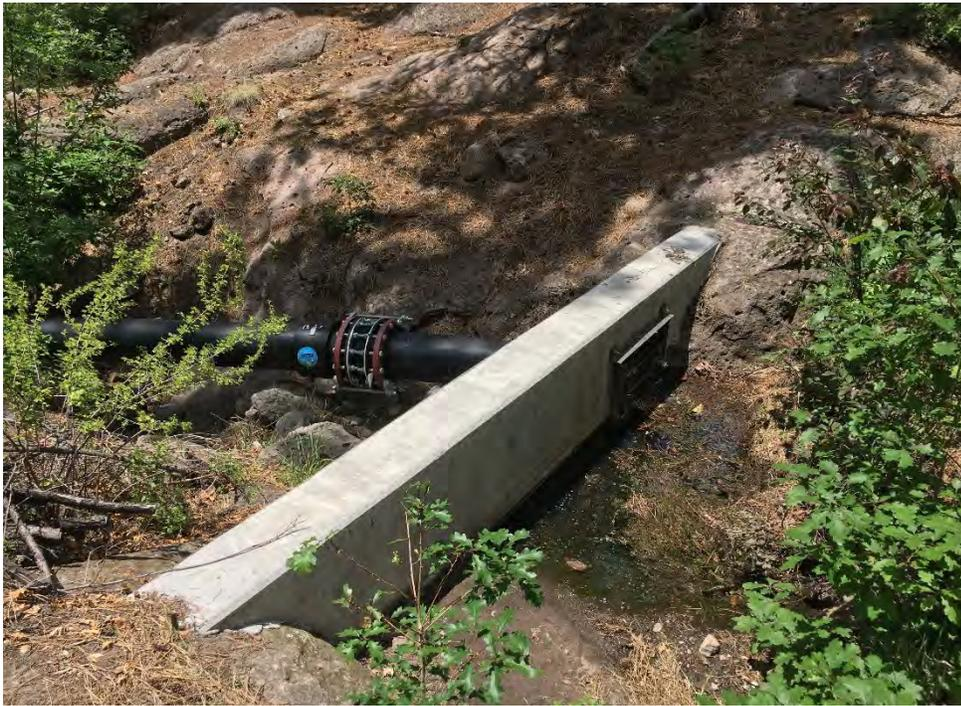
**Photo C-3.5-1** May 2017—Headwall functioning as designed. Removed needlecast and leaf buildup behind intake, as well as some trash.
