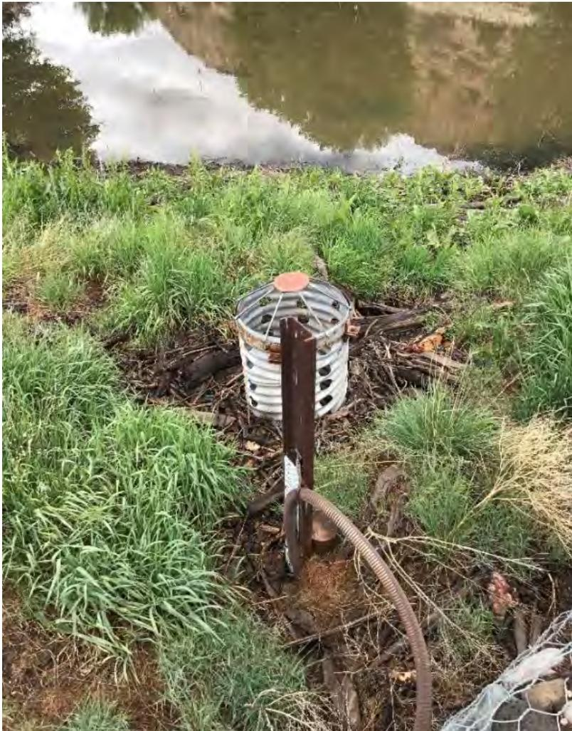
**Photo C-4.8-1** May 2017—Height of inlet is 3½ ft above wood debris. Inlet is clear of debris and functional. Slight erosion from outlet pipe but well vegetated and stable. Continue to monitor.
