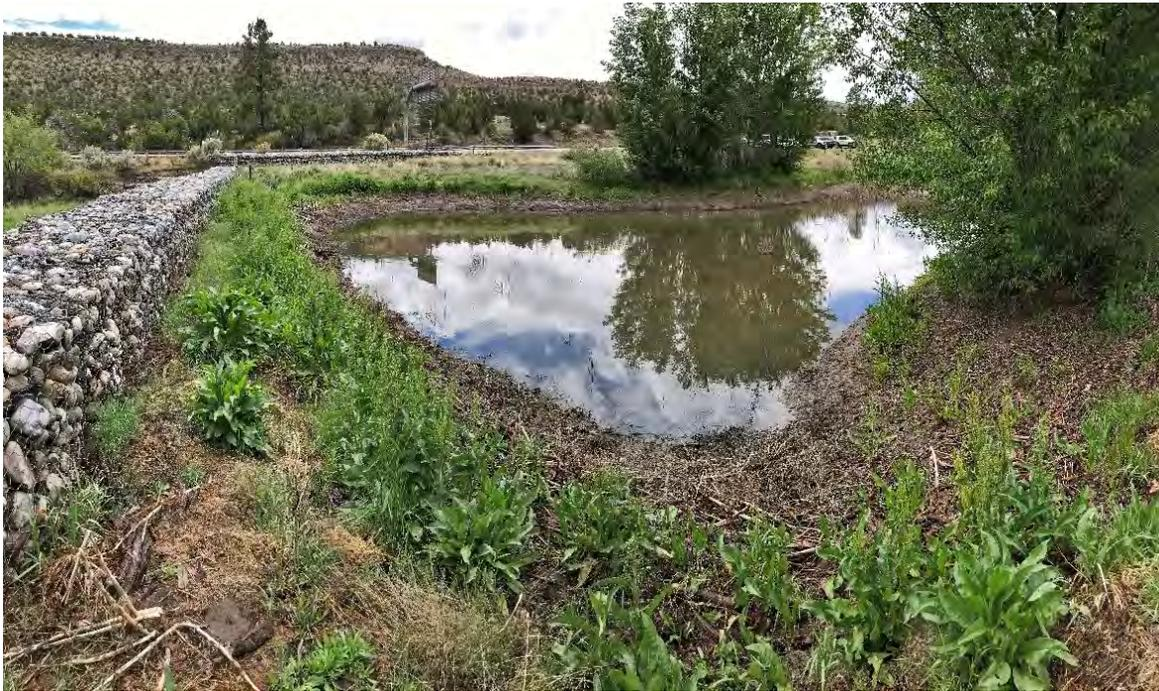
**Photo C-4.2-1** May 2017—Vegetation well established along weir embankment. Sediment loads at approximately 20 percent of total capacity.
