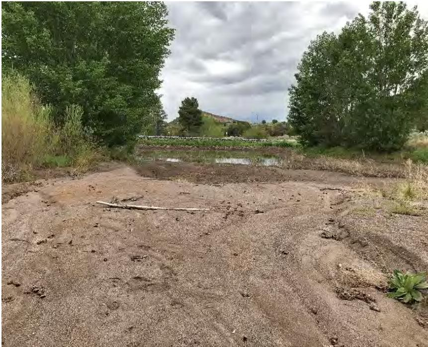
**Photo C-4.6-1 May 2017—Sediment pond level is at approximately 20 percent of total capacity. Pond has approximately 2–3 feet of standing water.**
