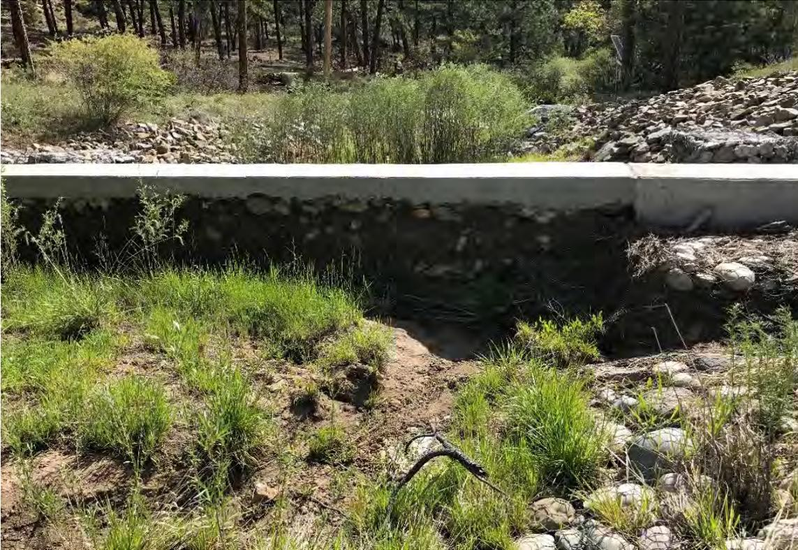
**Photo C-2.8-1 May 2017—Outlet appears to be working as designed. No seepage/piping, undercutting, or erosion occurring near or from outlet.**
