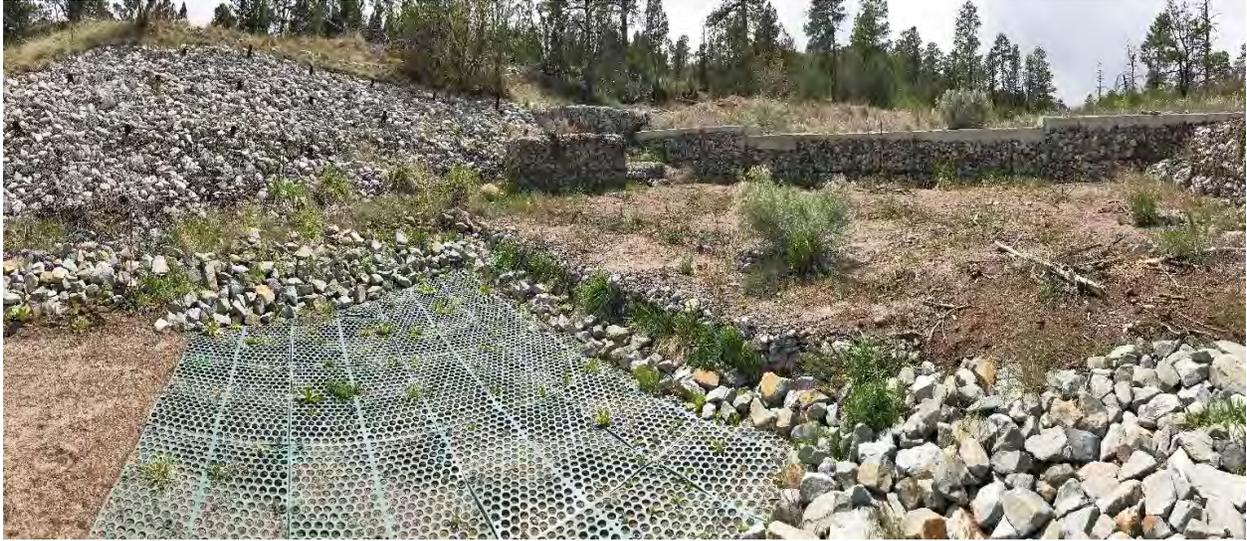
**Photo C-5.3-1 May 2017—Control is operating as designed. No buckling of embankment occurring. Riprap functioning as designed.**
