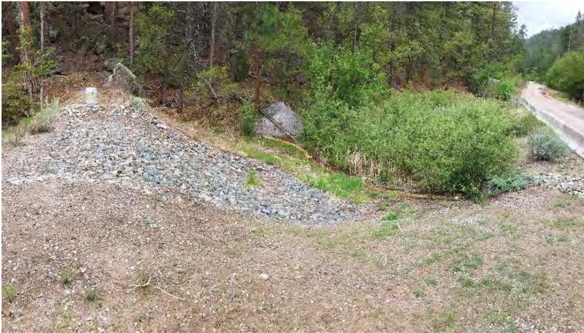
**Photo C-3.3-1 May 2017—No signs of erosion occurring on or near spillway. Spillway is maintaining alignment. No rodent burrows present and control appears stable.**
