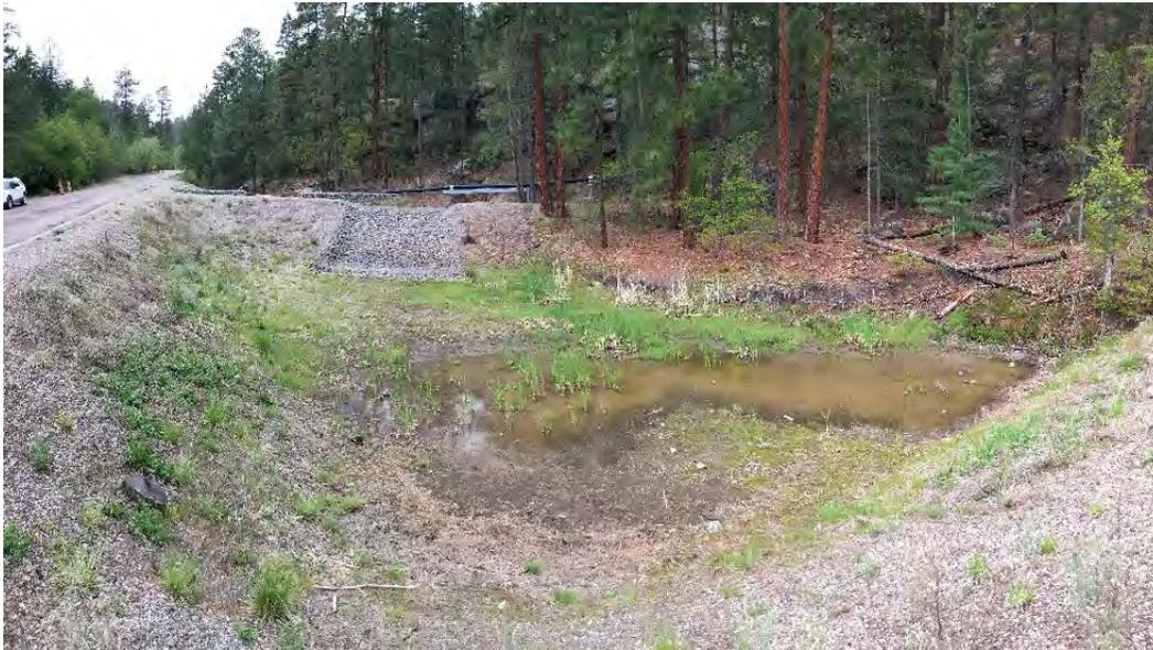
**Photo C-3.1-1 May 2017—No breaching/slides/cracks/sloughs present on embankment and pond. No erosion occurring on slope. No trash or debris present in control.**
