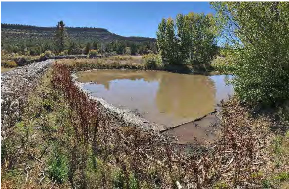
**Photo C-4.2-2** October 2017—No change in condition from the last inspection (May 2017). Control at same sediment capacity and standing water at same level.
