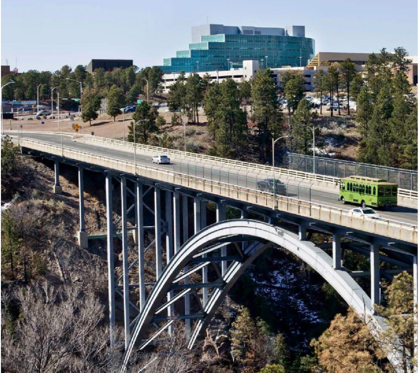
Figure 3-A: Los Alamos Canyon Bridge and National Security Sciences Building at the Core Area
