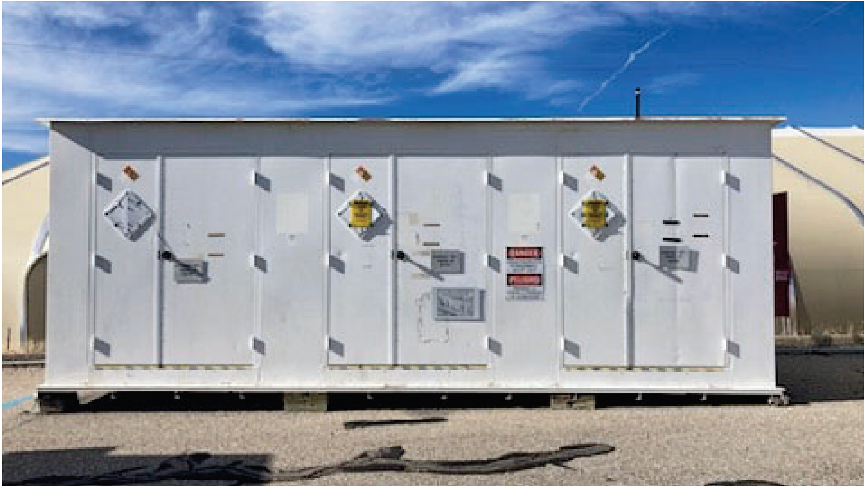
Figure 9: TA-54, Area G, Pad 5, Building 1028 after temporary equipment removal.
