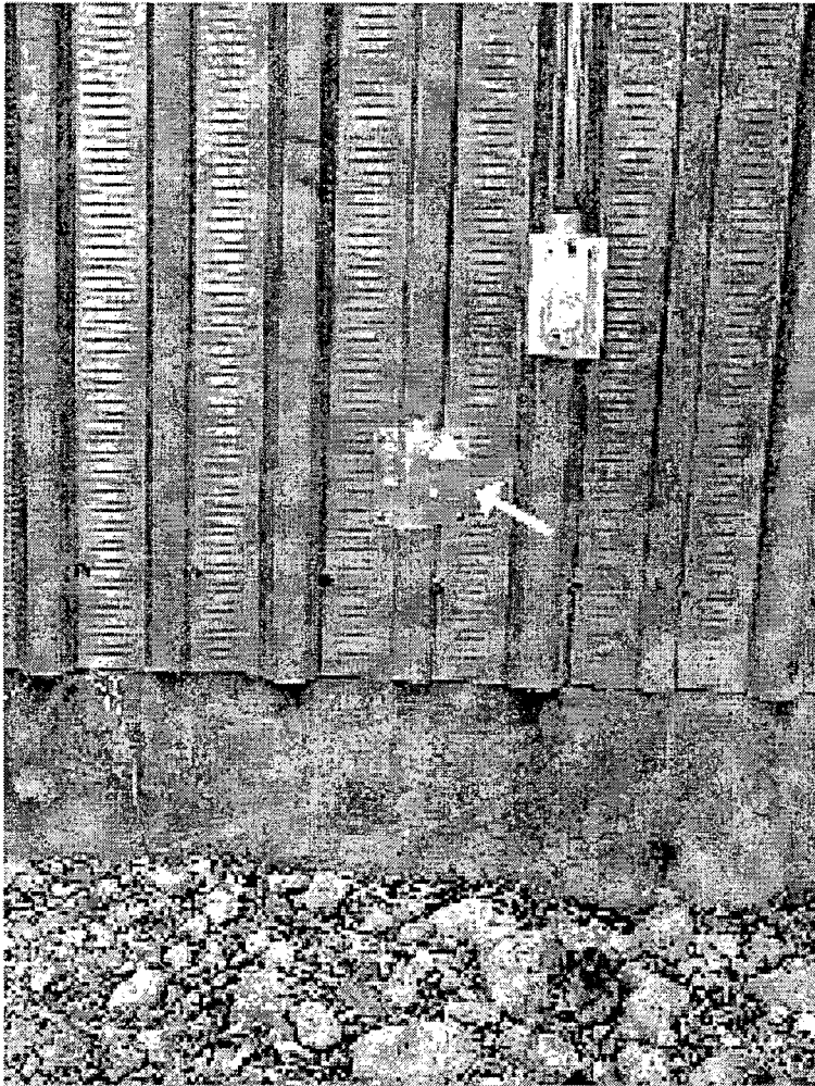
Figure 2.1-1. Eastern exterior wall of Building 46-77 showing metal patch over the location of the former drainpipe
