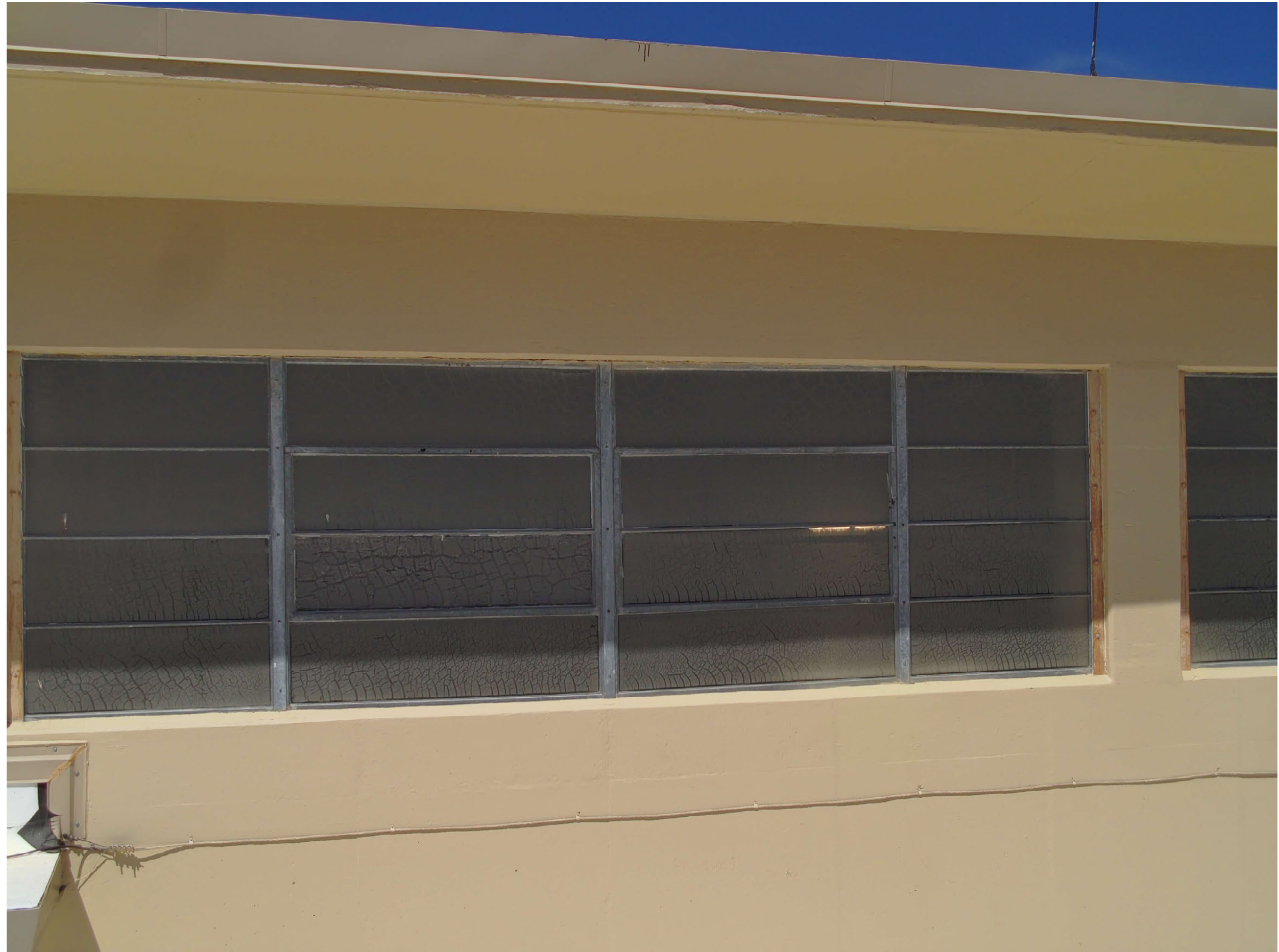
TA-03-0039 center wing, east facade, cracked window coating and delaminated glazing detail
