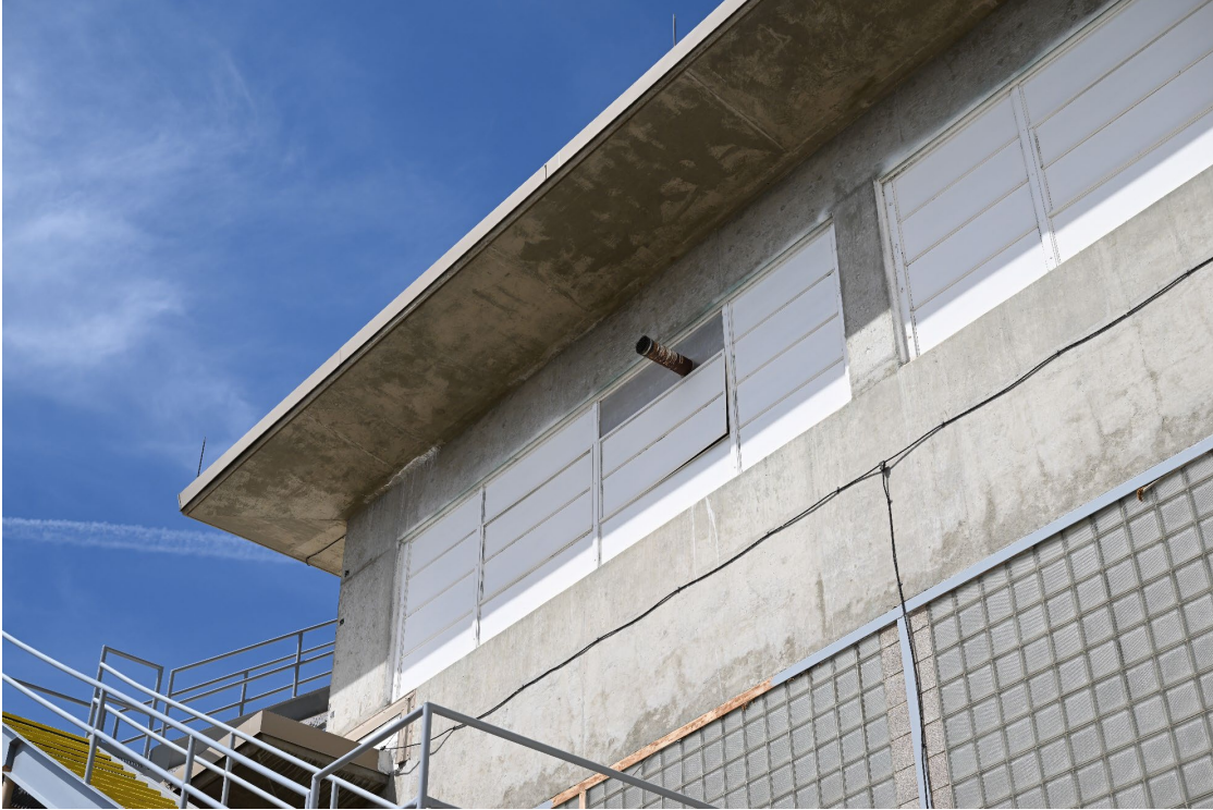
Figure 5-4. Example damaged sash (center) June 6, 2023 (LANL image, image no. DSC_0120).
