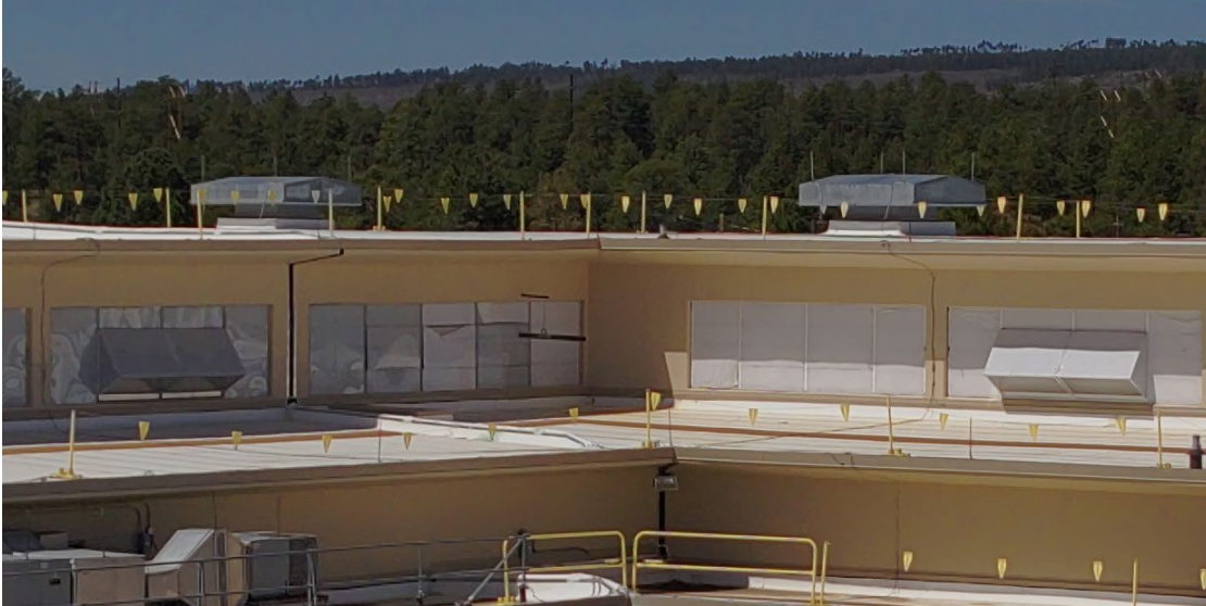
Figure 5-7. Example of broken lites with various ad hoc repairs, May 24, 2024 (LANL image, image no. S1006820).
