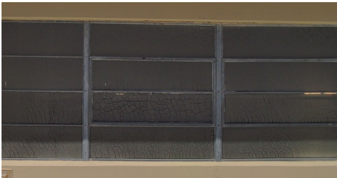
Figure 5-8. Example of delamination to window glazing and caulking, May 24, 2024 (LANL image, image no. S1006820).
