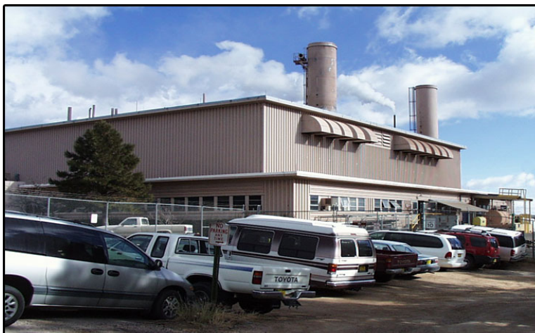
Figure 2.1-1. TA-3 power plant
