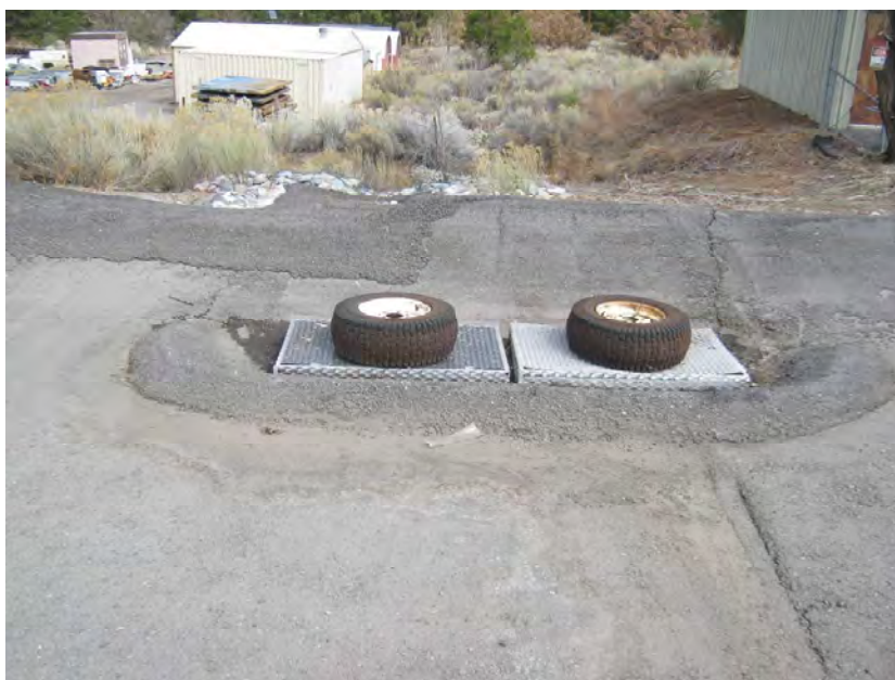
Photograph 10: TA-60-1 parking area storm drains equipped with PetroBarriers™
