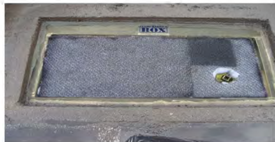
The top layer of filters is placed inside the flanged area including filters around the by-pass valve. The grate is then replaced and the Petro-Barrier-Box is back in service.
