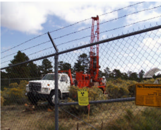
Material Disposal Area U
