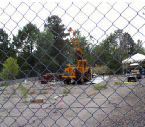
Material Disposal Area B
