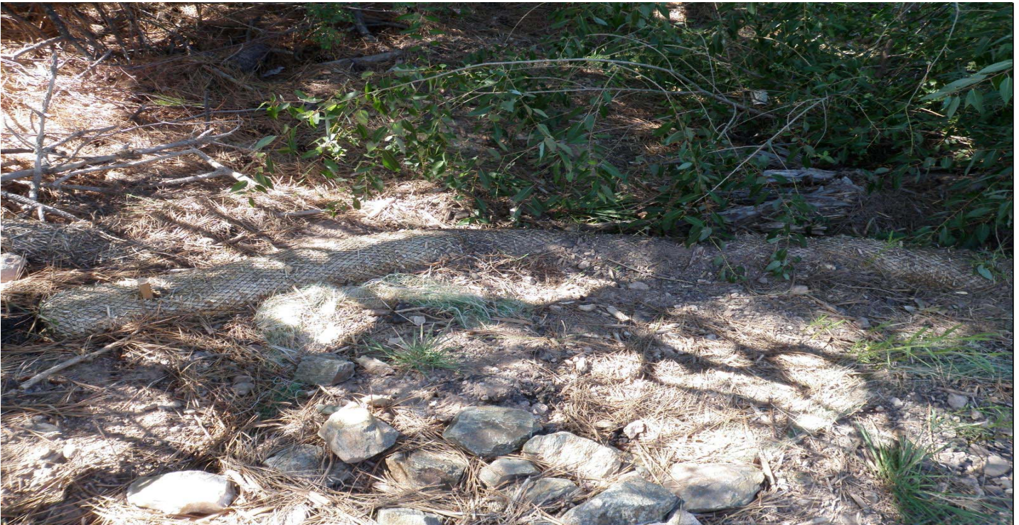
Photo 10561-5r.JPG (taken 09/14/10) L02103060008 : Berms - Straw Wattles.
