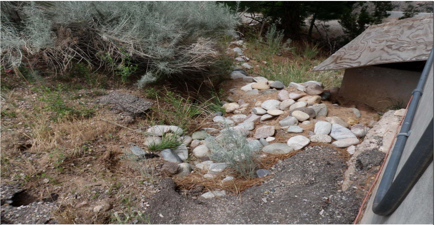
Photo 7417-3.JPG (taken 07/30/10) P00604010001 : Channel/Swale - Earthen Channel/Swale.
