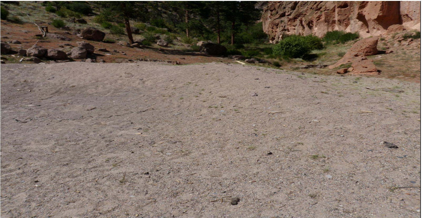
Photo 8791-6r.JPG (taken 09/07/10) A00603010004 : Berms - Earthen Berm.
