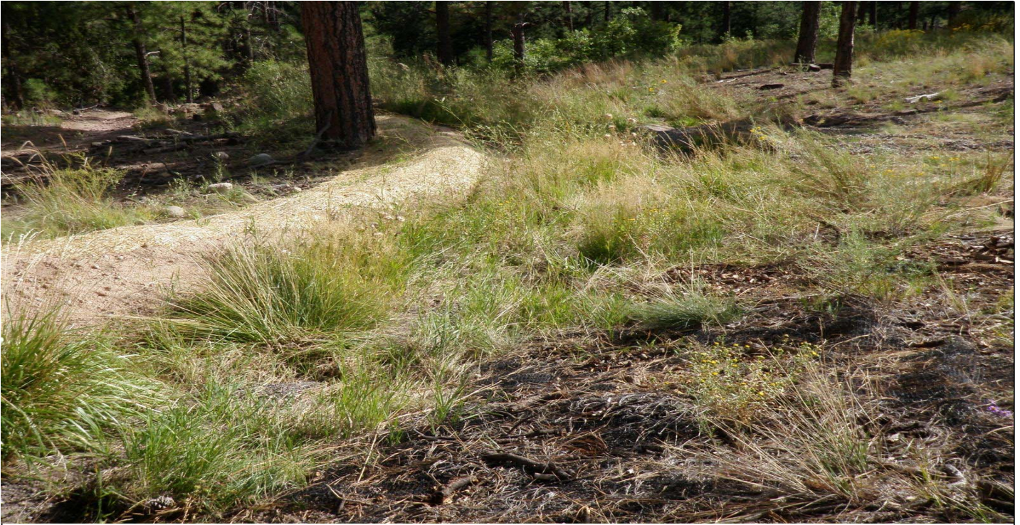
Photo 10554-1r.JPG (taken 09/09/10) E00103010012 : Berms - Earthen Berm.
