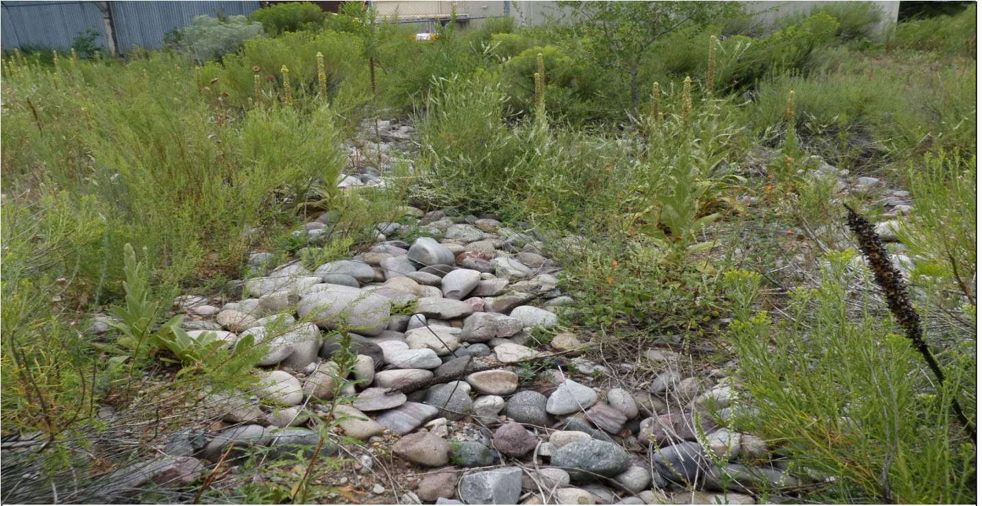
Photo 7451-1.JPG (taken 08/04/10) S00604060011 : Channel/Swale - Rip Rap.
