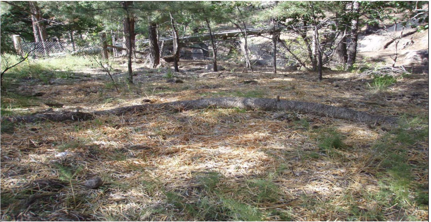
Photo 10871-7.JPG (taken 10/07/10) P00303060005 : Berms - Straw Wattles.
