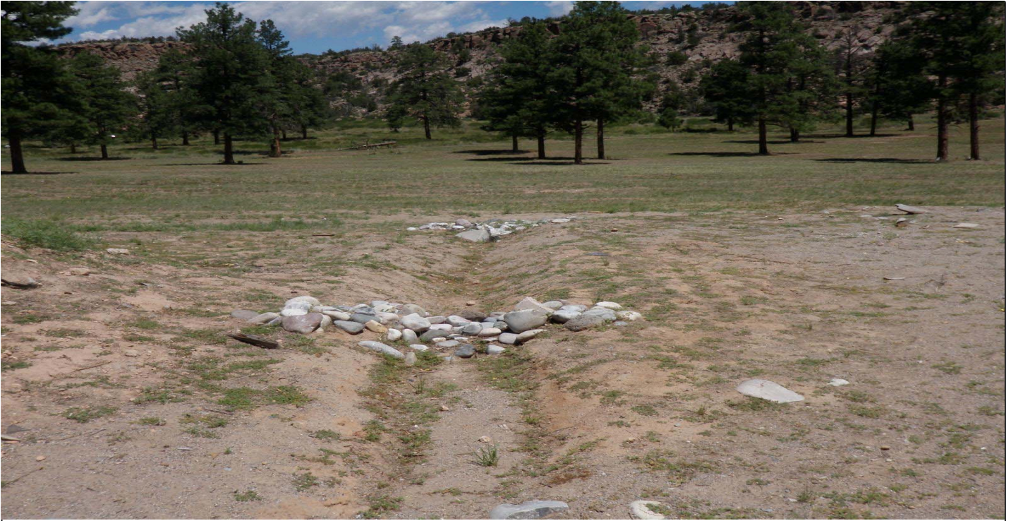
Photo 7596-2r.JPG (taken 08/13/10) I00706010004 : Check Dam - Rock Check Dam.
