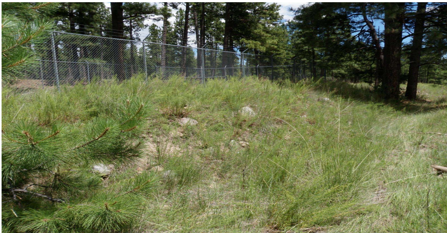
Photo 7499-2r.JPG (taken 08/11/10) J03002010001 : Established Vegetation - Permanent Vegetation Grasses and Shrubs; J03003010003 : Berms - Earthen Berm.
