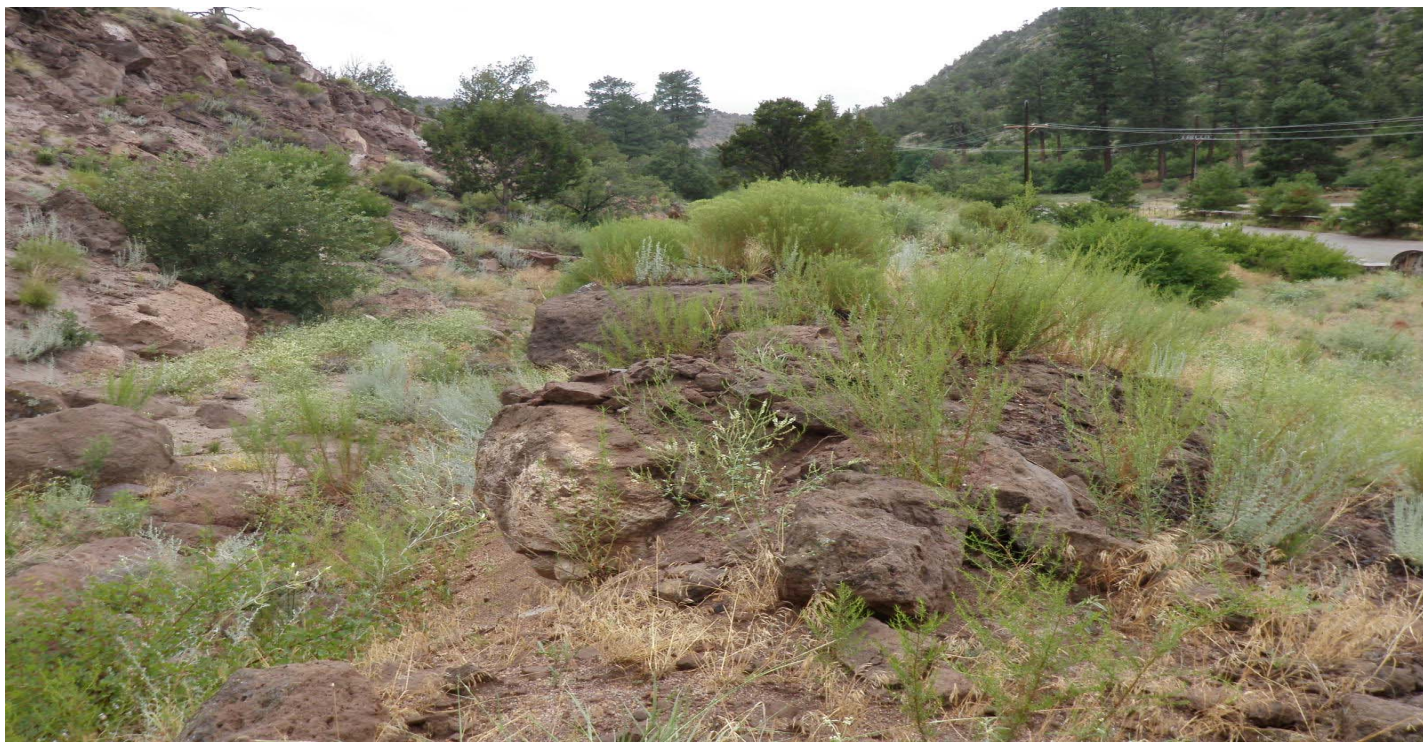
Photo 7345-2.JPG (taken 07/26/10) A00103010005 : Berms - Earthen Berm.
