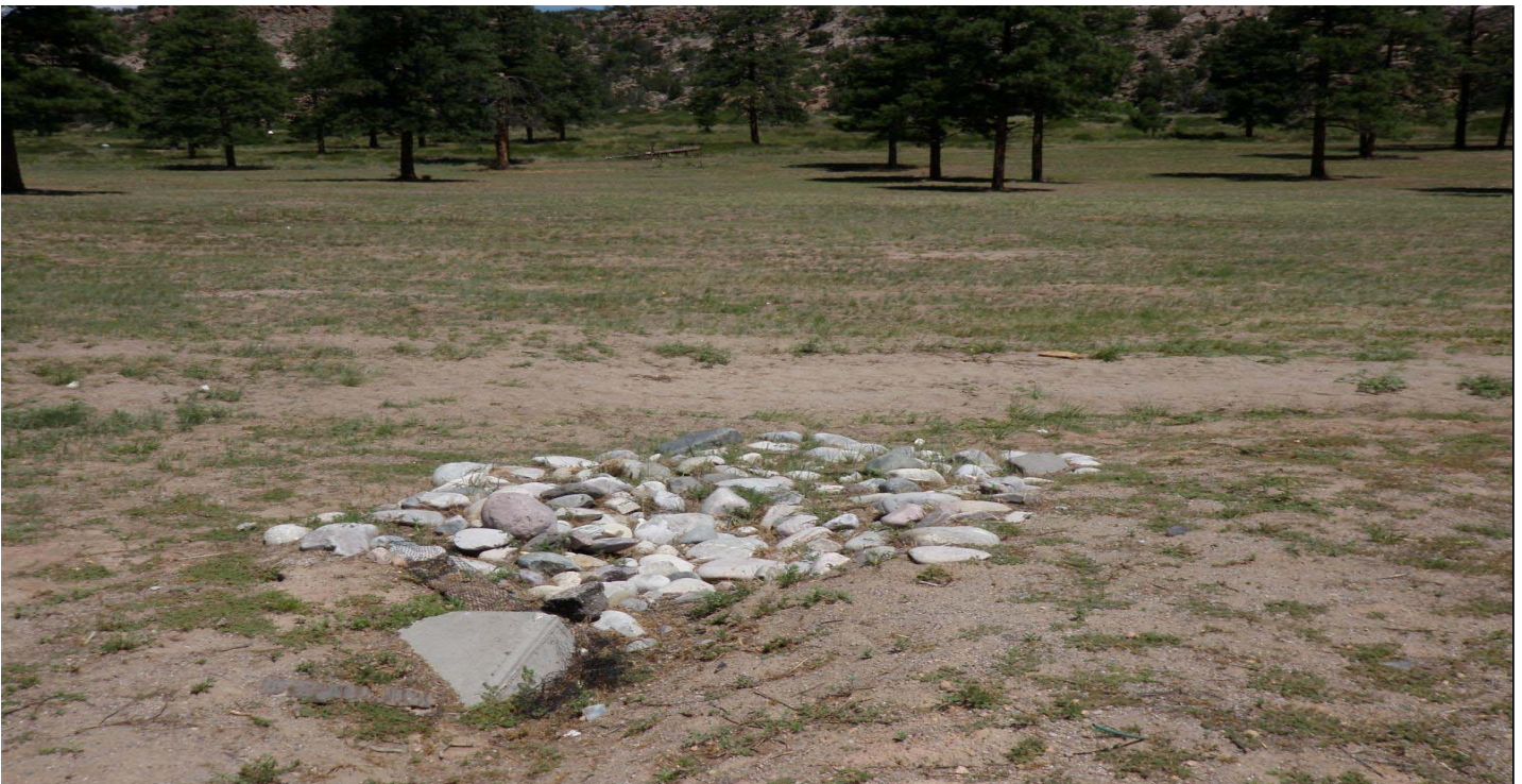
Photo 7596-3r.JPG (taken 08/13/10) I00704060003 : Channel/Swale - Rip Rap.
