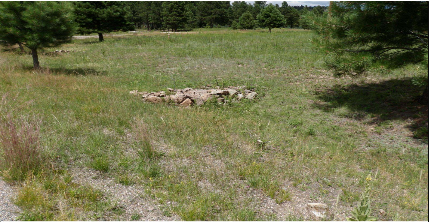
Photo 7497-4r.JPG (taken 08/11/10) J02806010005 : Check Dam - Rock Check Dam.
