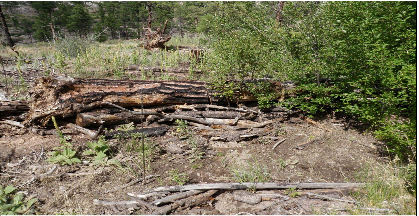
Photo 7484-3r.JPG (taken 08/10/10) C00206020010 : Check Dam - Log Check Dam.
