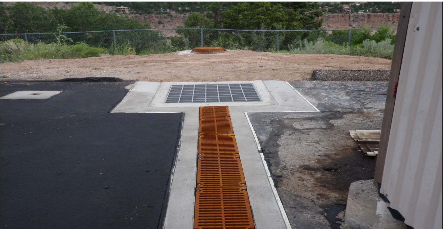
Photo 8653-4.JPG (taken 07/30/10) P00504040016 : Channel/Swale - Culvert.
