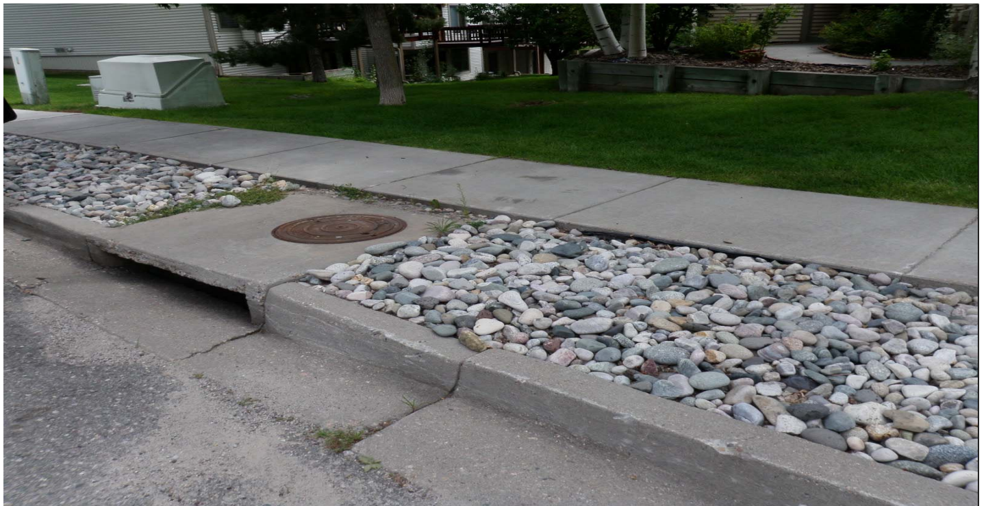
Photo 7422-1.JPG (taken 07/28/10) L00804040004 : Channel/Swale - Culvert.
