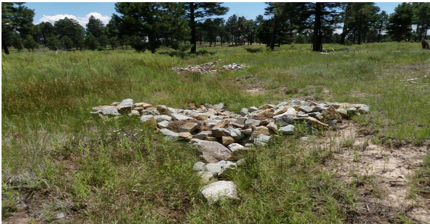
Photo 7594-5r.JPG (taken 08/13/10) W00106010002 : Check Dam - Rock Check Dam.
