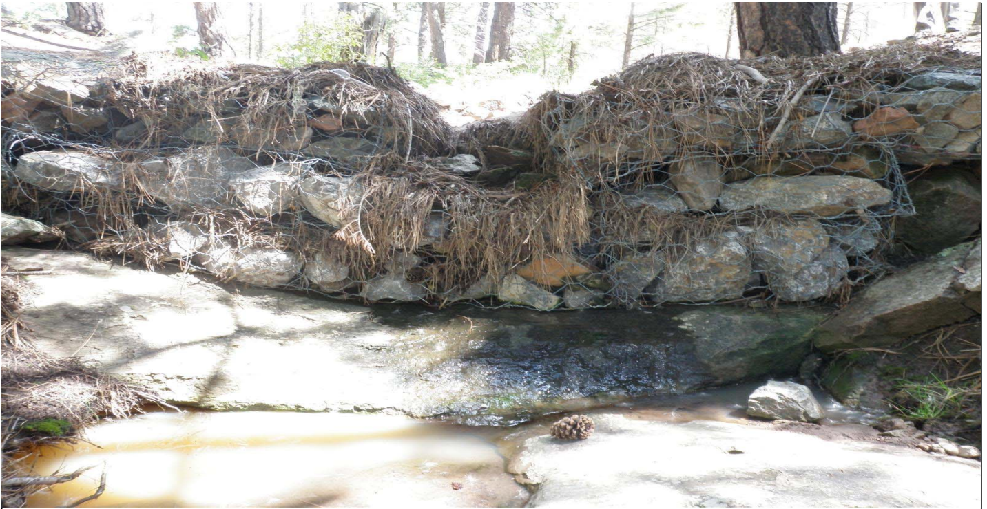
Photo 7516-1r.JPG (taken 08/12/10) E00107010003 : Gabions - Gabions; E00107010004 : Gabions - Gabions.
