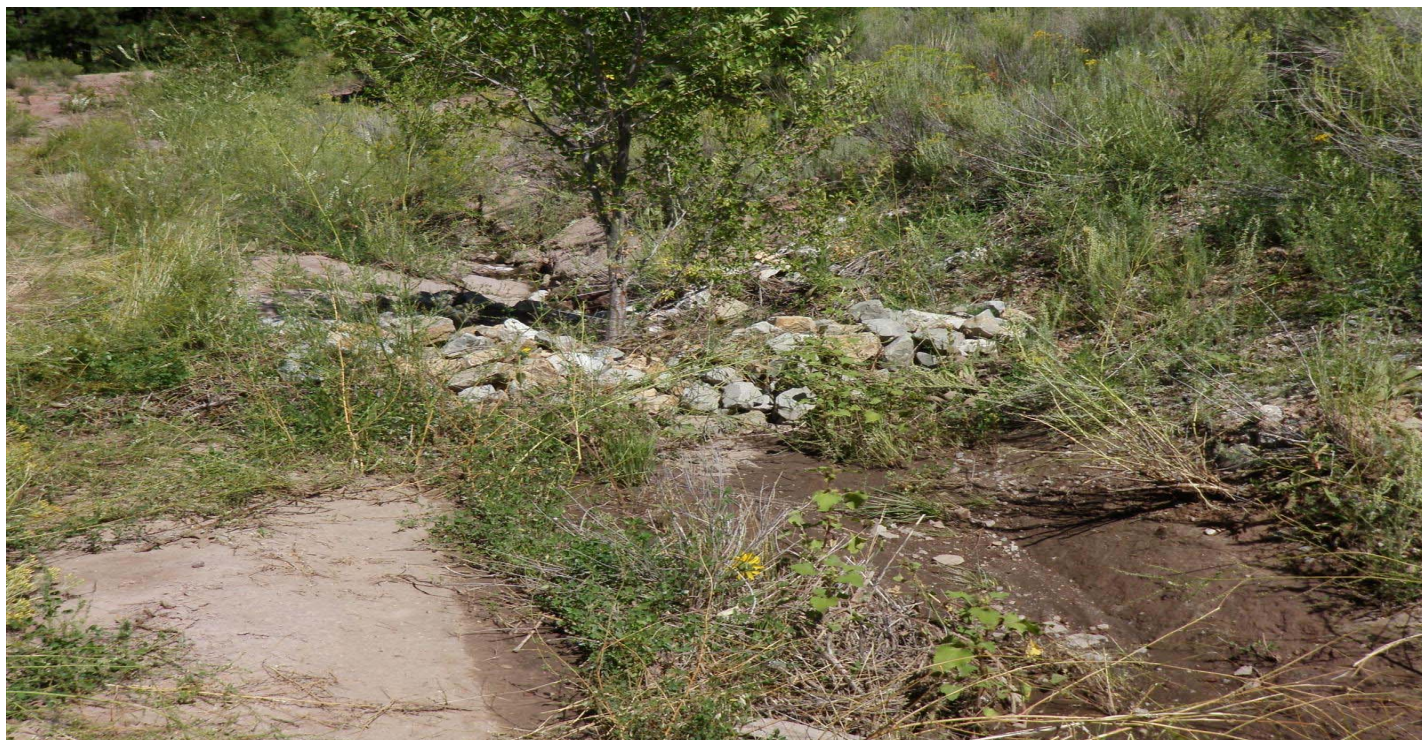
Photo 8513-1r.JPG (taken 08/20/10) S00606010015 : Check Dam - Rock Check Dam.
