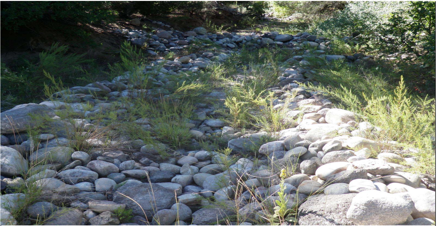
Photo 8505-5r.JPG (taken 08/20/10) J02504060010 : Channel/Swale - Rip Rap; J02506010009 : Check Dam - Rock Check Dam.
