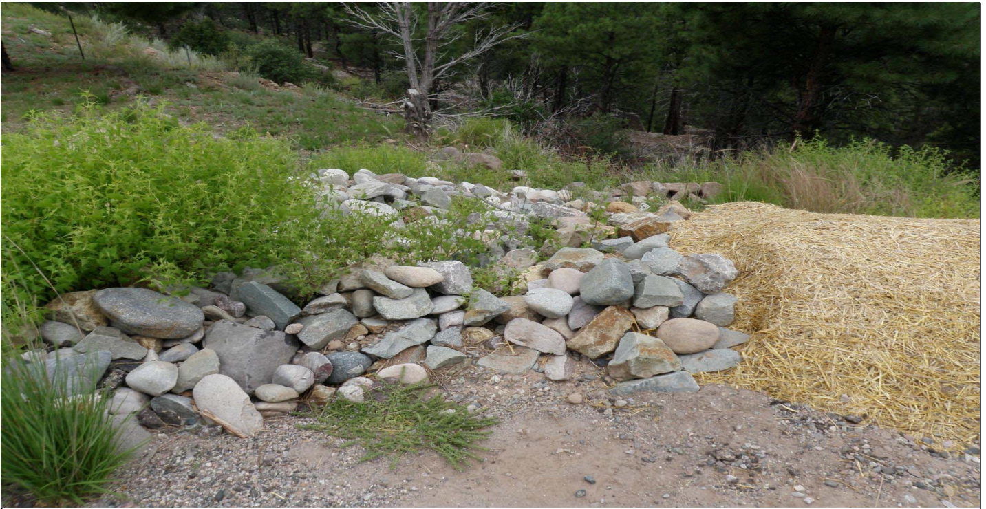
Photo 7511-3r.JPG (taken 08/12/10) J01004060001 : Channel/Swale - Rip Rap; J01006010007 : Check Dam - Rock Check Dam.
