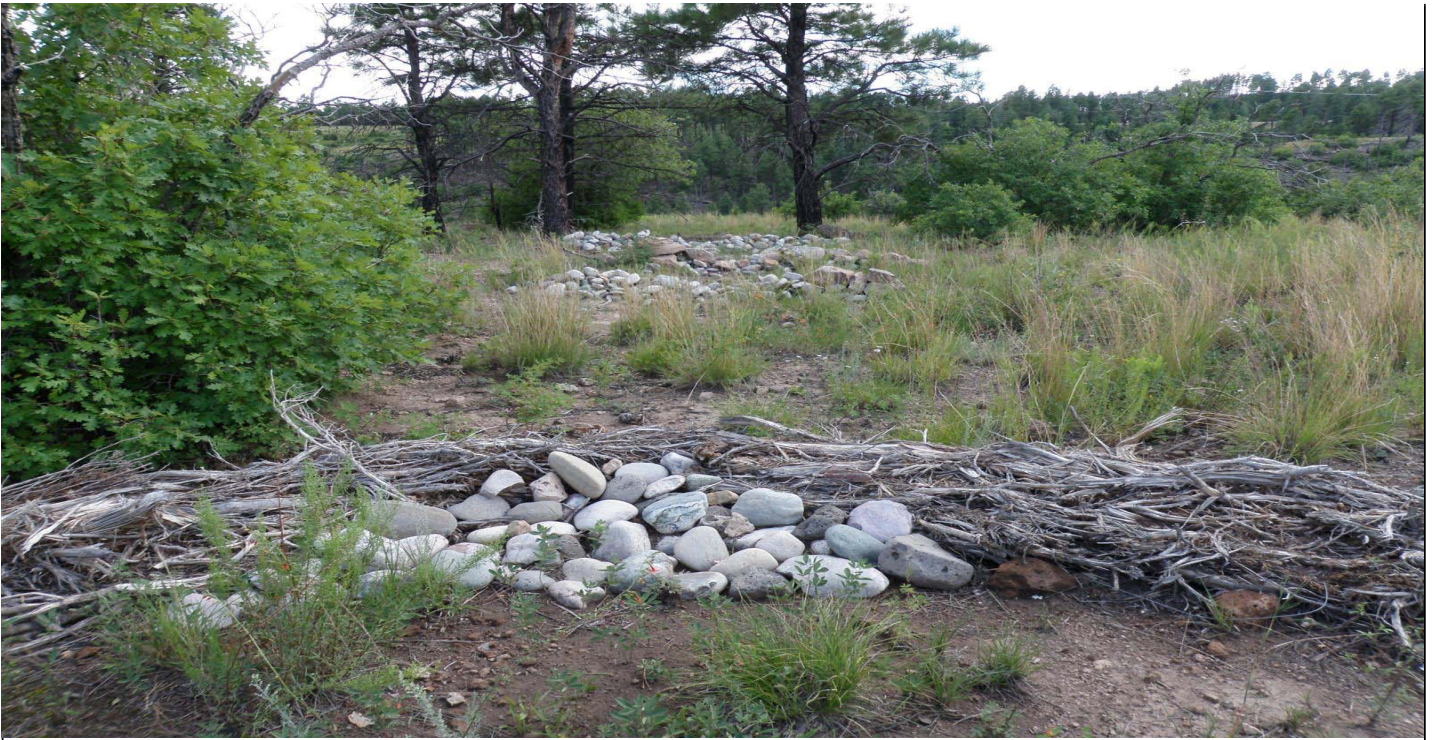
Photo 7509-1r.JPG (taken 08/12/10) J00706010002 : Check Dam - Rock Check Dam; J00706010003 : Check Dam - Rock Check Dam; J00706010004 : Check Dam - Rock Check Dam; J00706030008 : Check Dam - Juniper Bales.
