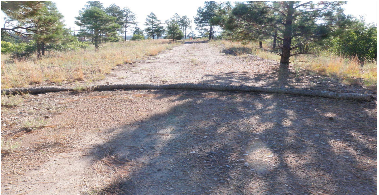
Photo 10874-1r.JPG (taken 10/07/10) W01403060005 : Berms - Straw Wattles.
