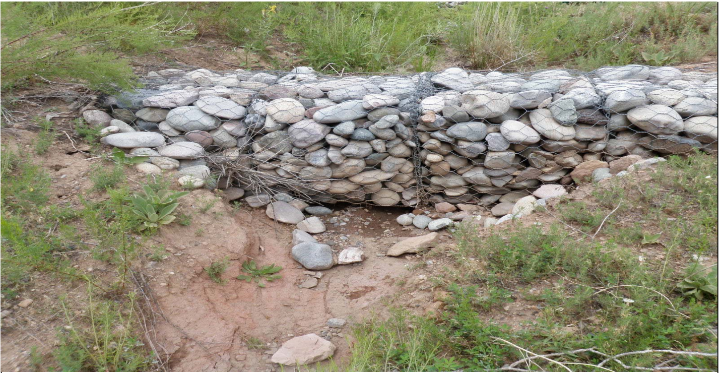
Photo 7451-5.JPG (taken 08/04/10) S00607010008 : Gabions - Gabions.
