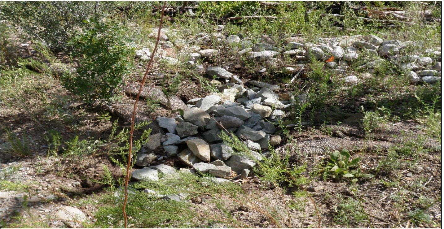
Photo 7481-5r.JPG (taken 08/10/10) C00704060006 : Channel/Swale - Rip Rap.
