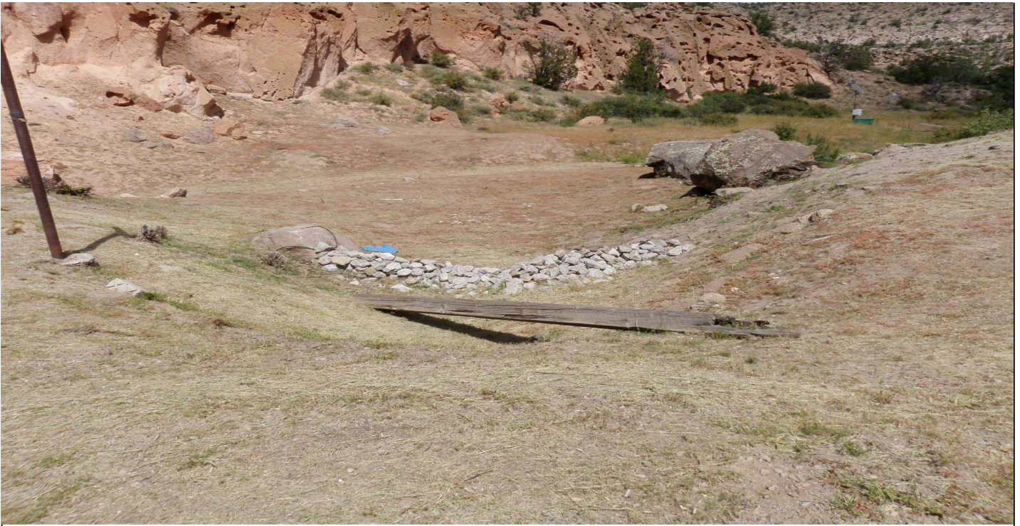
Photo 8791-3r.JPG (taken 09/07/10) A00604010008 : Channel/Swale - Earthen Channel/Swale; A00606010003 : Check Dam - Rock Check Dam.
