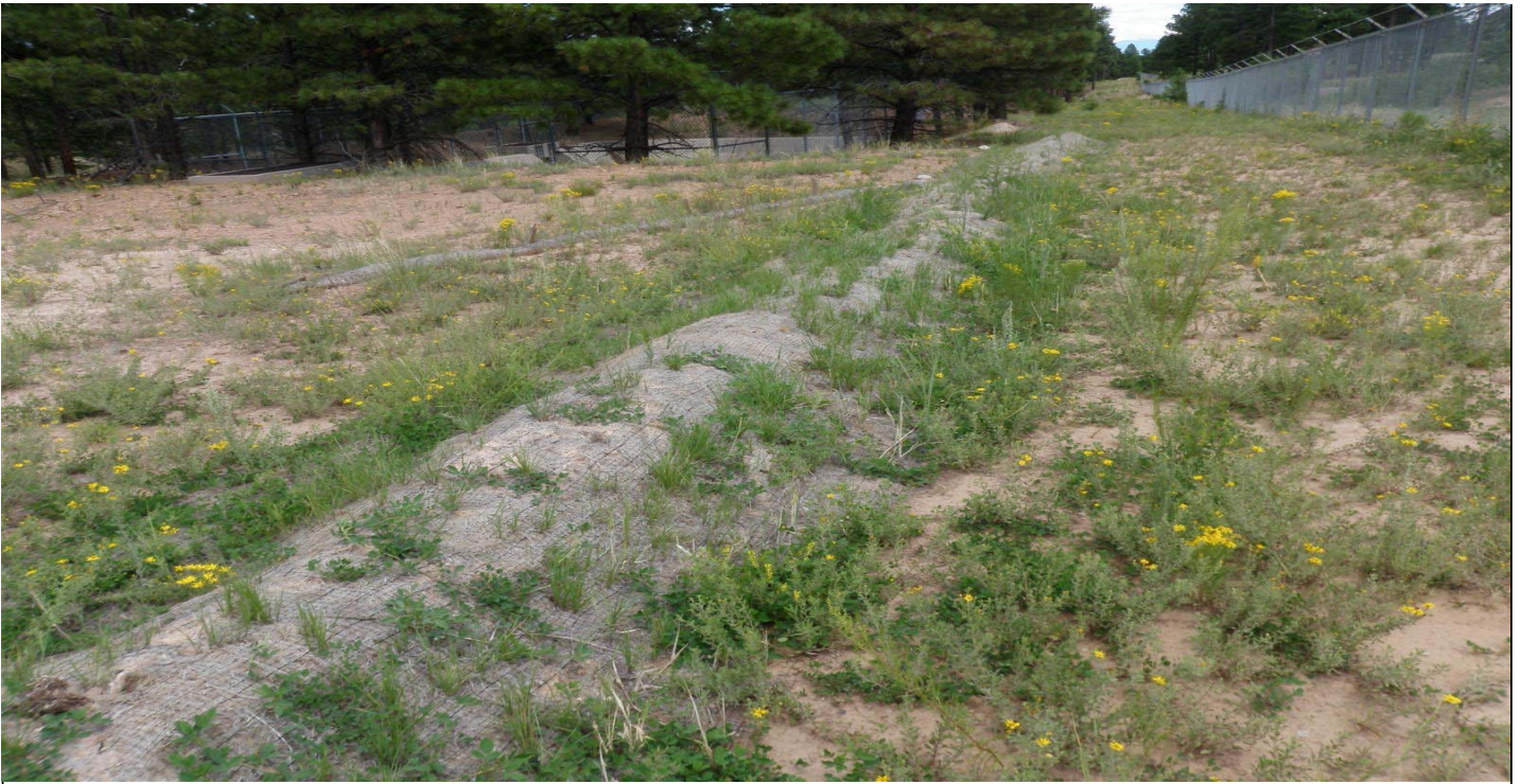
Photo 7503-1r.JPG (taken 08/11/10) J00201060010 : Seed and Mulch - Erosion Control Blanket; J00203010008 : Berms - Earthen Berm.
