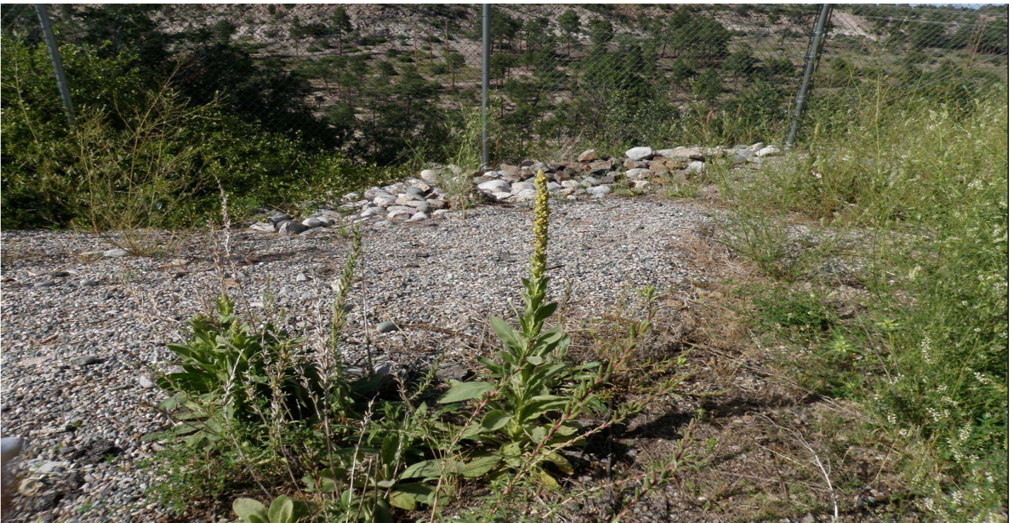
Photo 7484-6r.JPG (taken 08/10/10) C00204060001 : Channel/Swale - Rip Rap.
