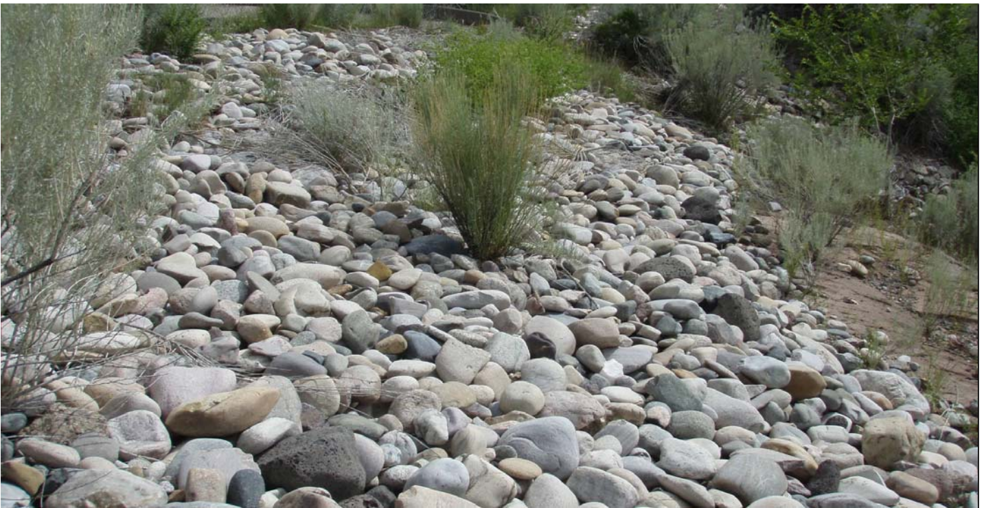
Photo 7600-5.JPG (taken 08/03/10) S00304060010 : Channel/Swale - Rip Rap.
