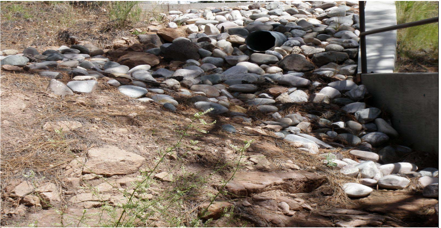
Photo 7516-5r.JPG (taken 08/12/10) E00104060010 : Channel/Swale - Rip Rap.
