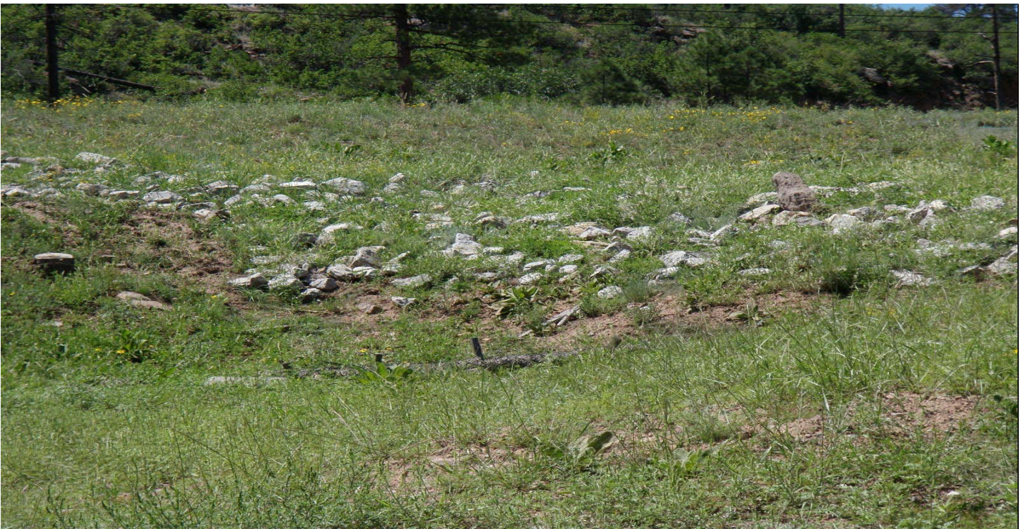
Photo 7595-3r.JPG (taken 08/13/10) I00504060004 : Channel/Swale - Rip Rap.
