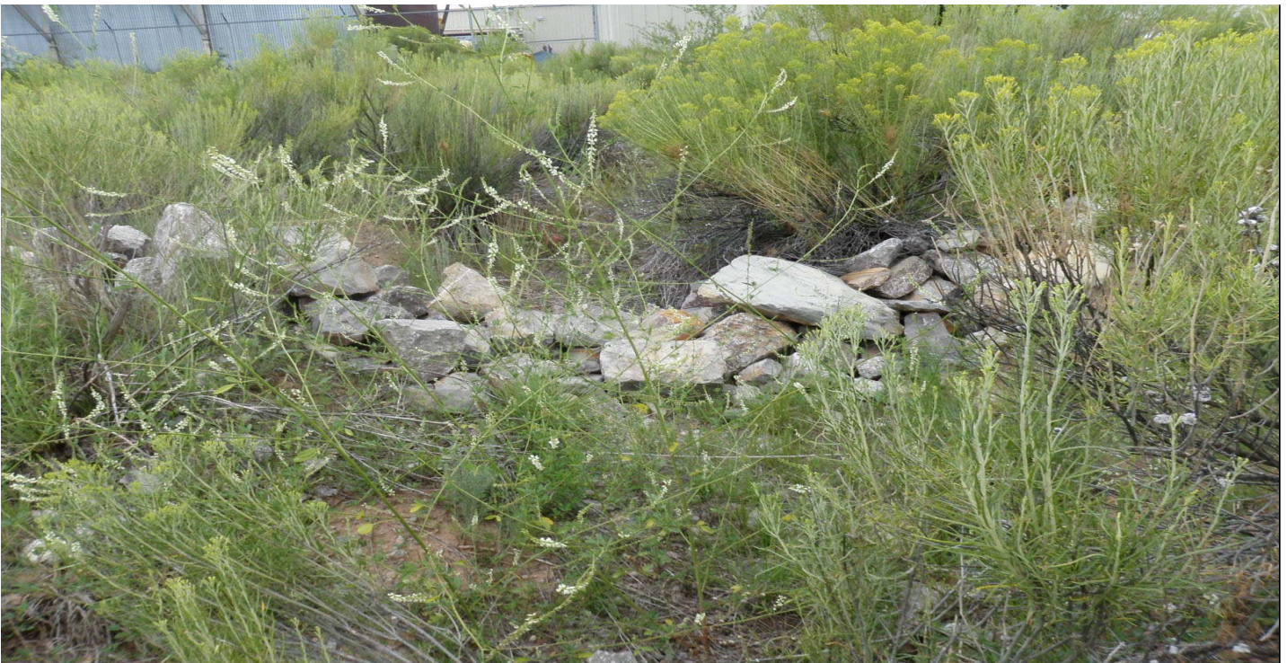
Photo 7451-4.JPG (taken 08/04/10) S00606010012 : Check Dam - Rock Check Dam.
