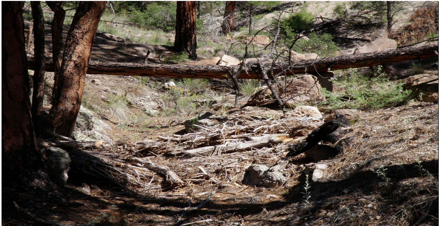
Photo 7443-1.JPG (taken 08/03/10) R00506030003 : Check Dam - Juniper Bales.
