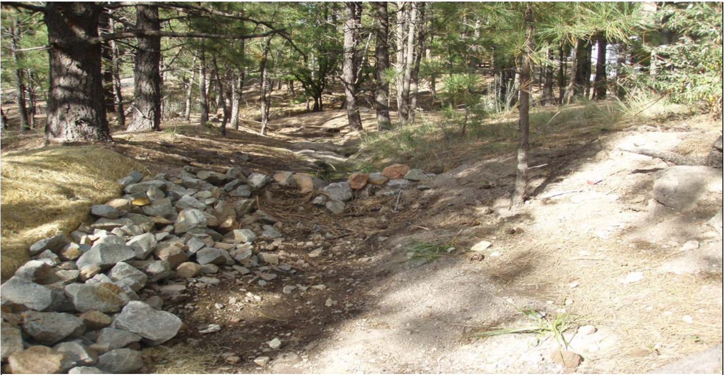
Photo 10871-3.JPG (taken 10/07/10) P00306010004 : Check Dam - Rock Check Dam.
