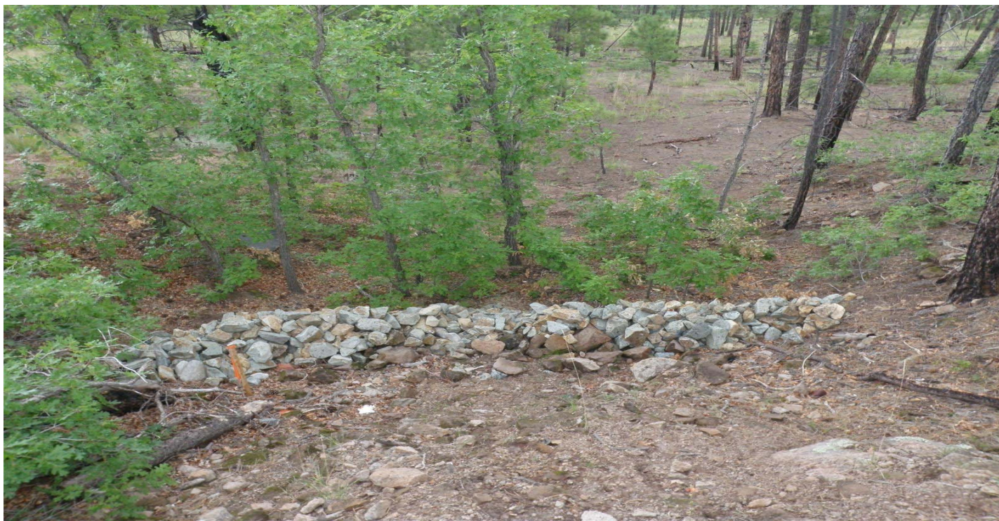
Photo 7515-2r.JPG (taken 08/12/10) H00102020001 : Established Vegetation - Permanent Vegetation Forested/Needle Cast; H00106010002 : Check Dam - Rock Check Dam.
