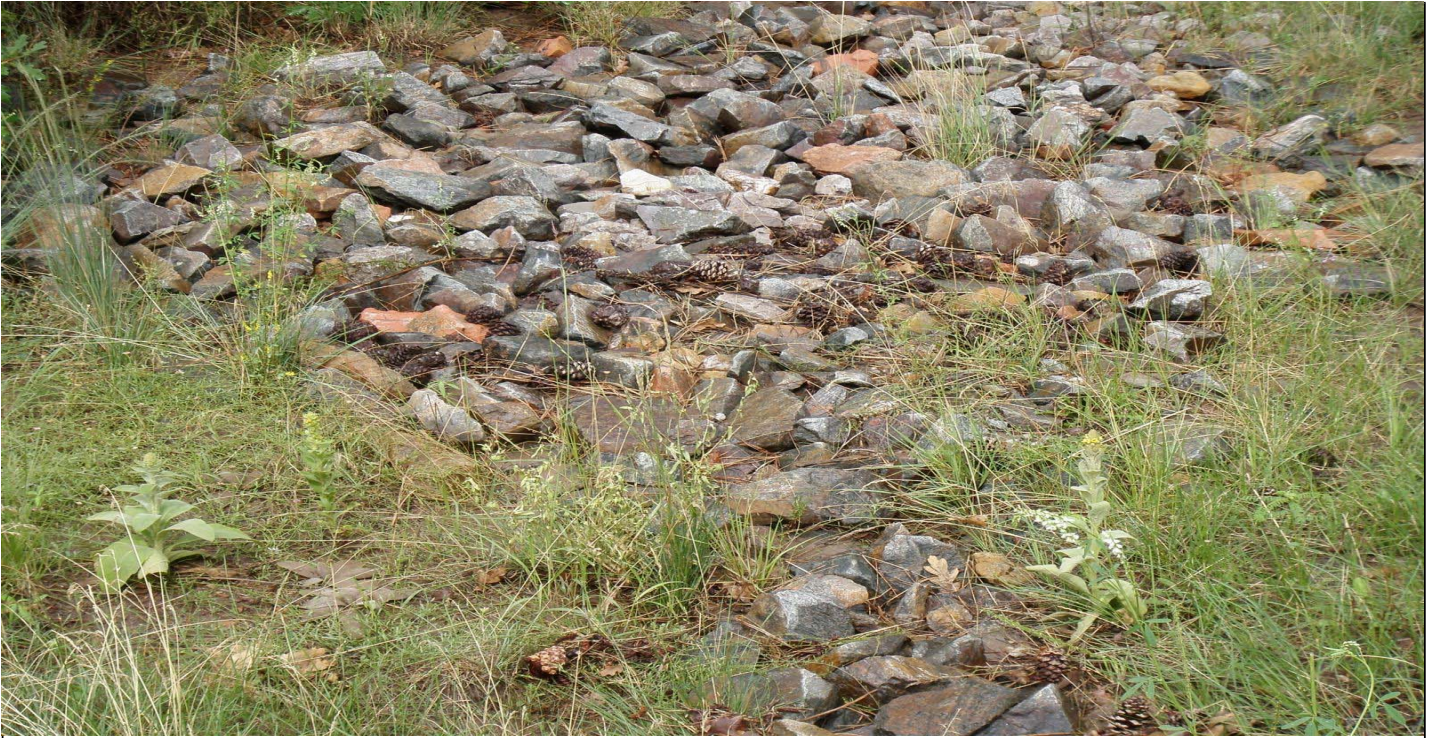
Photo 7489-2r.JPG (taken 08/09/10) M00604060012 : Channel/Swale - Rip Rap.
