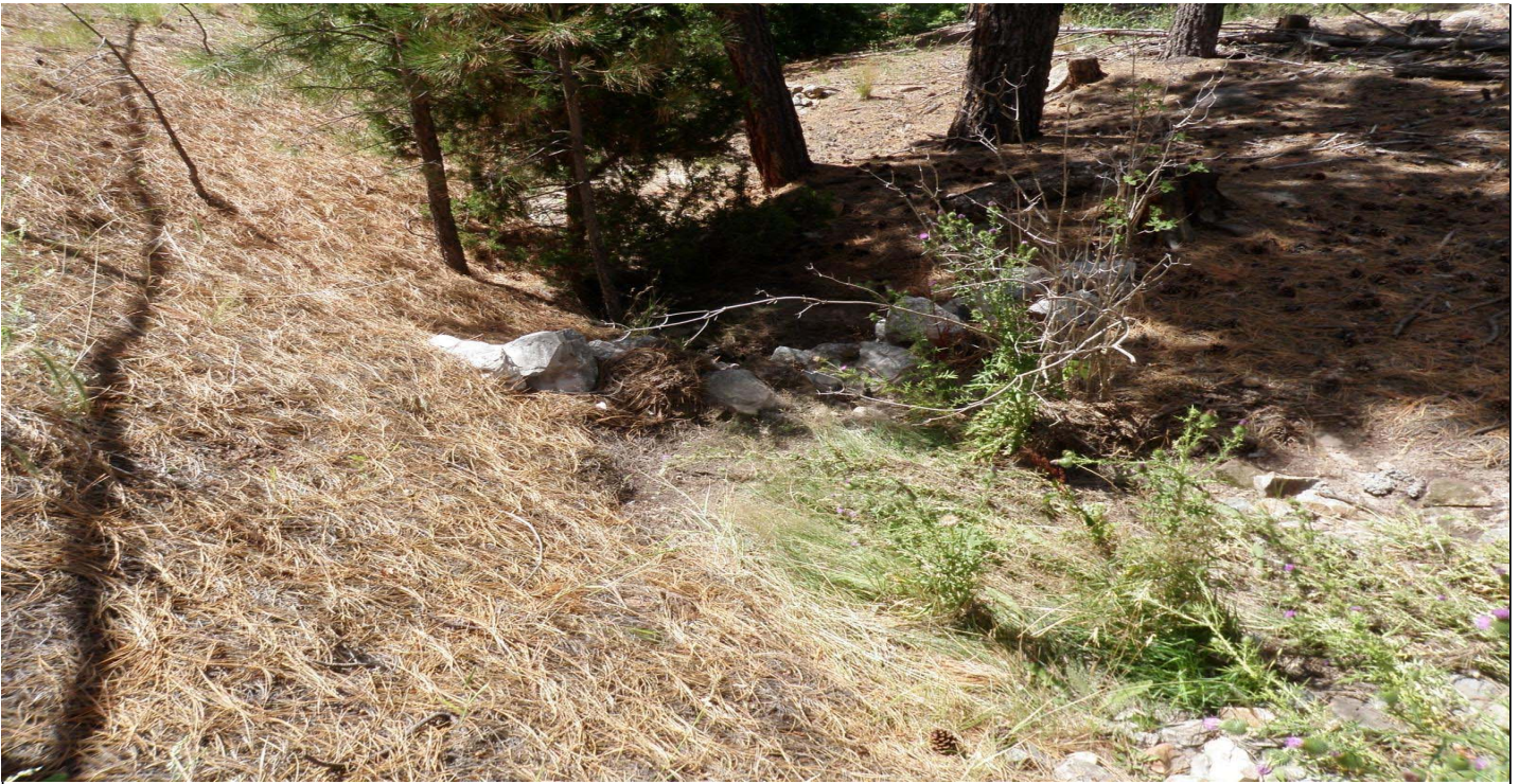
Photo 7516-3r.JPG (taken 08/12/10) E00106010008 : Check Dam - Rock Check Dam.
