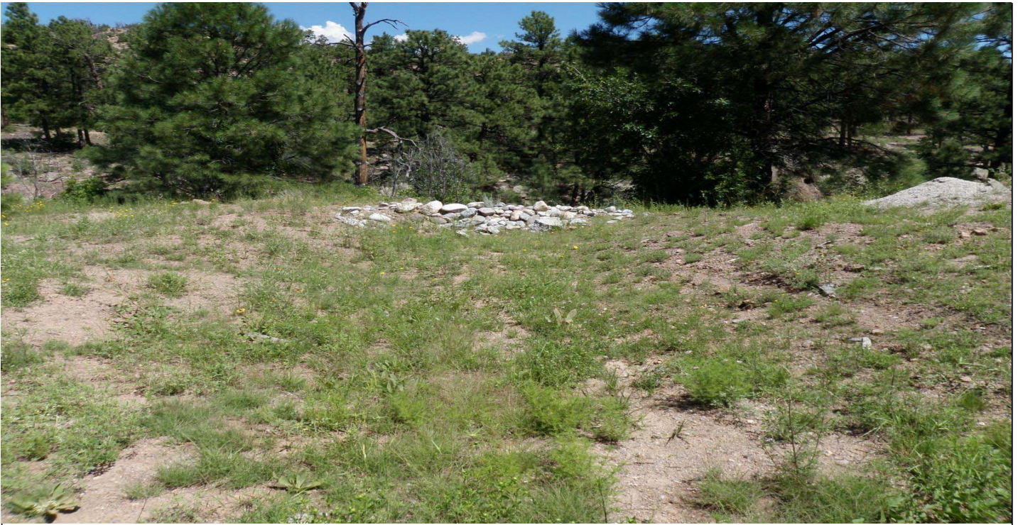
Photo 7595-2r.JPG (taken 08/13/10) I00506010006 : Check Dam - Rock Check Dam.
