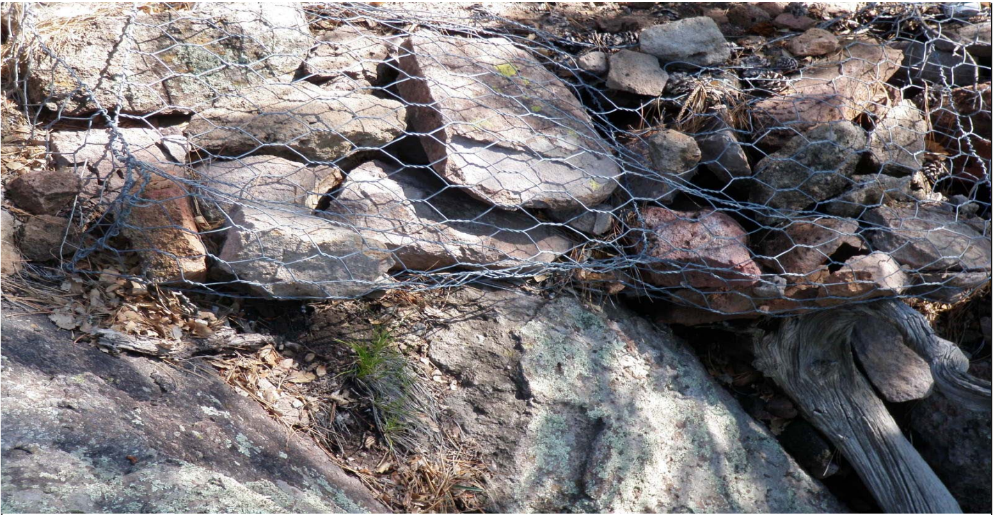
Photo 7420-2.JPG (taken 07/28/10) L00507010002 : Gabions - Gabions.
