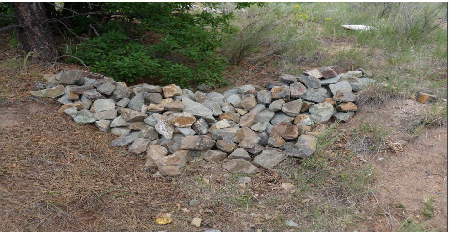
Photo 7451-2.JPG (taken 08/04/10) S00606010014 : Check Dam - Rock Check Dam.
