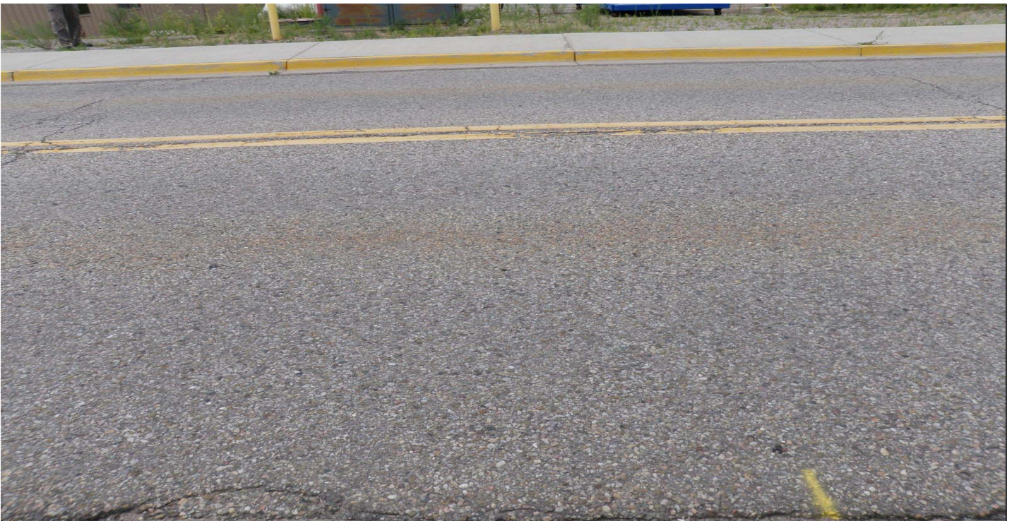
Photo 7522-2r.JPG (taken 08/12/10) E01303090002 : Berms - Curbing.
