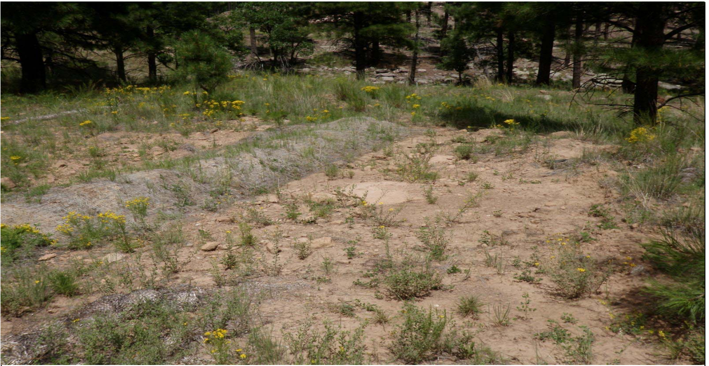
Photo 7503-5r.JPG (taken 08/11/10) J00201060013 : Seed and Mulch - Erosion Control Blanket; J00203010007 : Berms - Earthen Berm.
