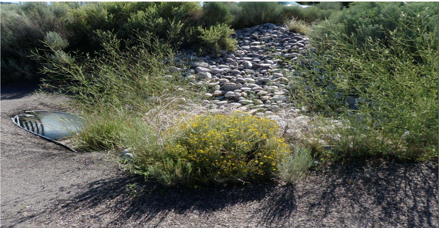
Photo 7356-2.JPG (taken 07/27/10) Q00804060007 : Channel/Swale - Rip Rap.
