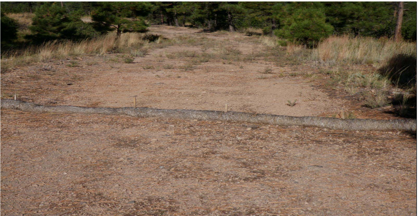
Photo 10874-3r.JPG (taken 10/07/10) W01403060004 : Berms - Straw Wattles.
