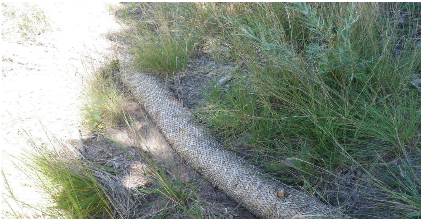
Photo 10561-3r.JPG (taken 09/14/10) L02103060007 : Berms - Straw Wattles.
