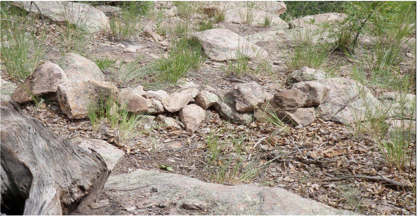
Photo 7509-5r.JPG (taken 08/12/10) J00706010005 : Check Dam - Rock Check Dam.
