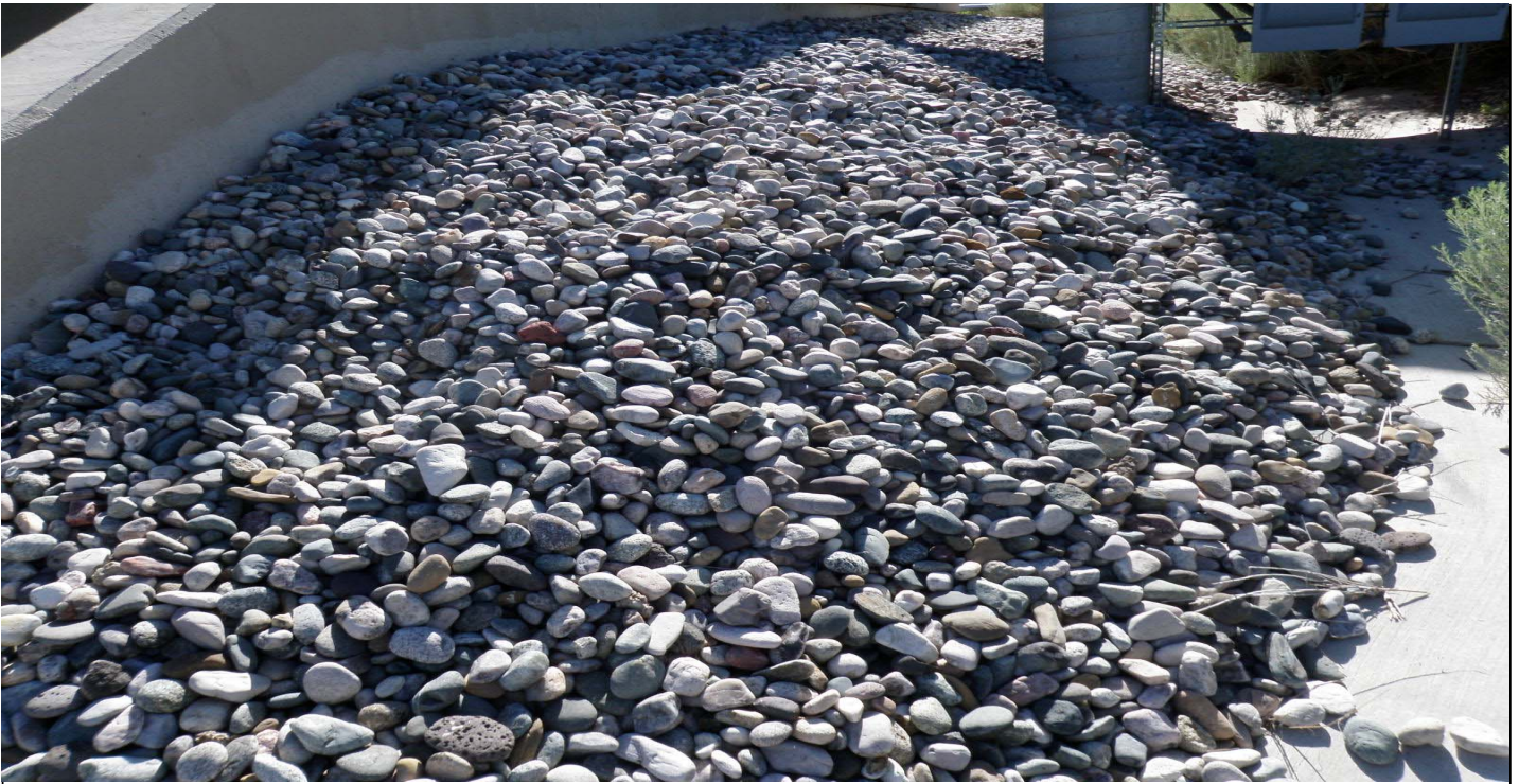
Photo 7356-3.JPG (taken 07/27/10) Q00804060005 : Channel/Swale - Rip Rap.
