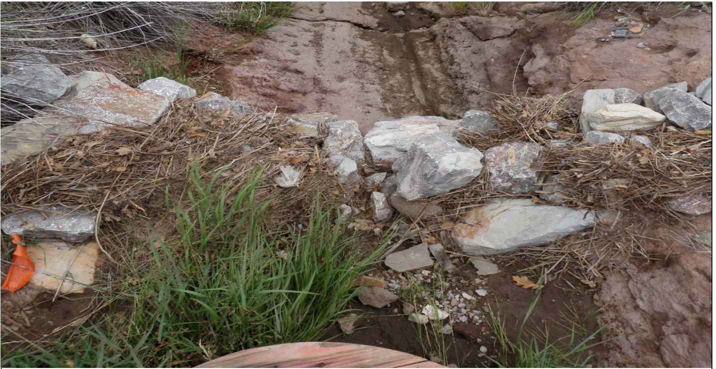
Photo 7451-8.JPG (taken 08/04/10) S00606010001 : Check Dam - Rock Check Dam.
