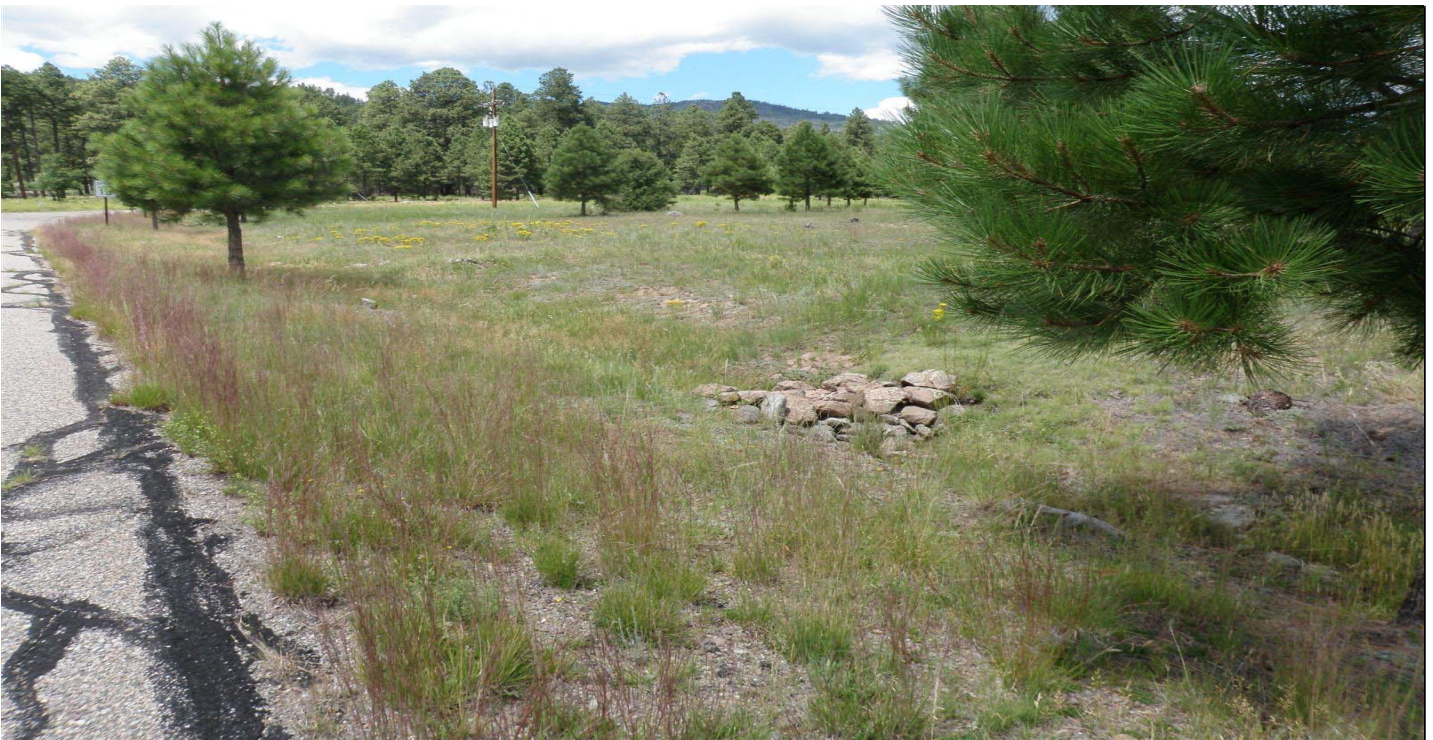
Photo 7497-3r.JPG (taken 08/11/10) J02806010004 : Check Dam - Rock Check Dam.
