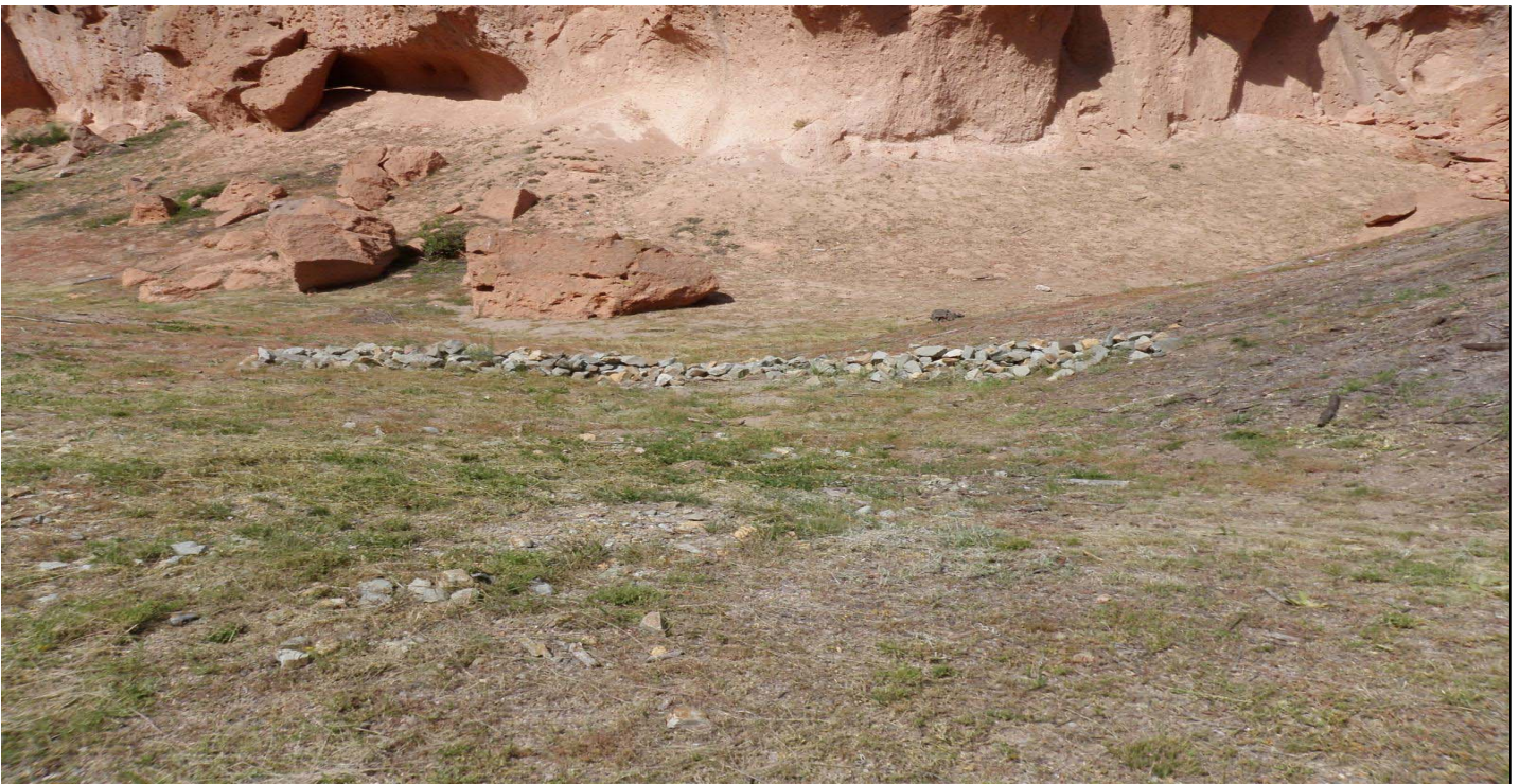
Photo 8791-2r.JPG (taken 09/07/10) A00604010006 : Channel/Swale - Earthen Channel/Swale; A00606010009 : Check Dam - Rock Check Dam.
