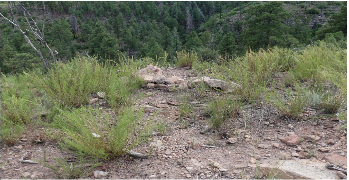
Photo 7509-3r.JPG (taken 08/12/10) J00706010007 : Check Dam - Rock Check Dam.
