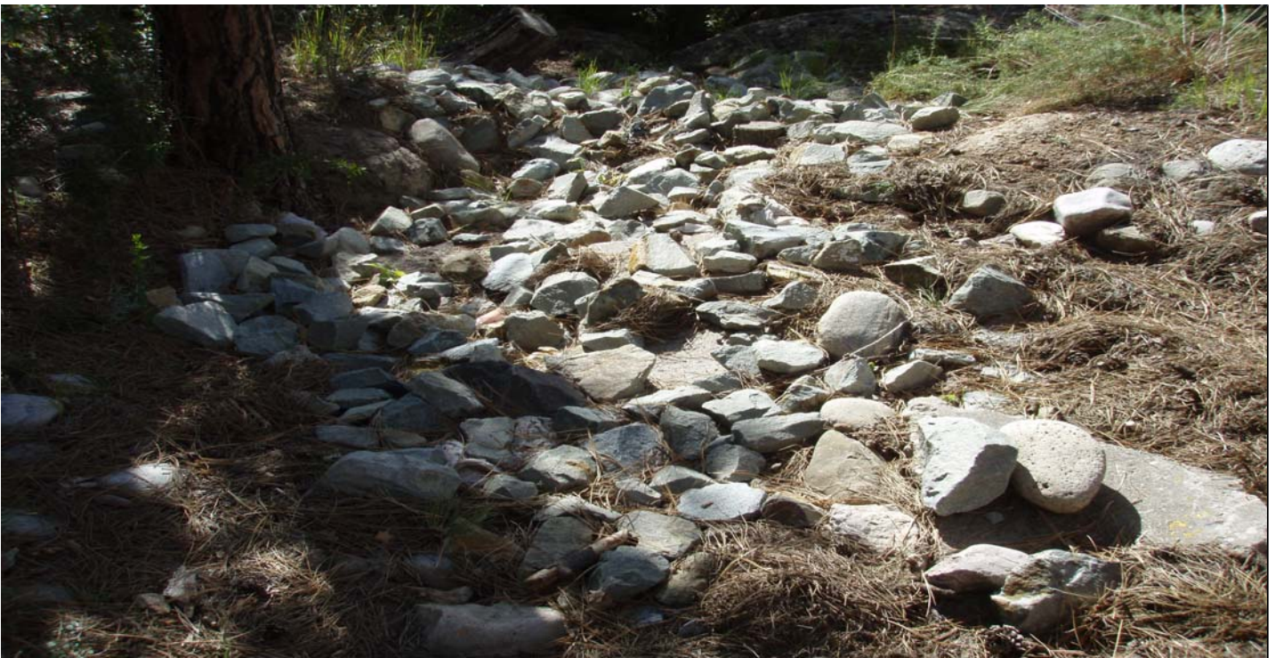
Photo 10871-8.JPG (taken 10/07/10) P00304060011 : Channel/Swale - Rip Rap.
