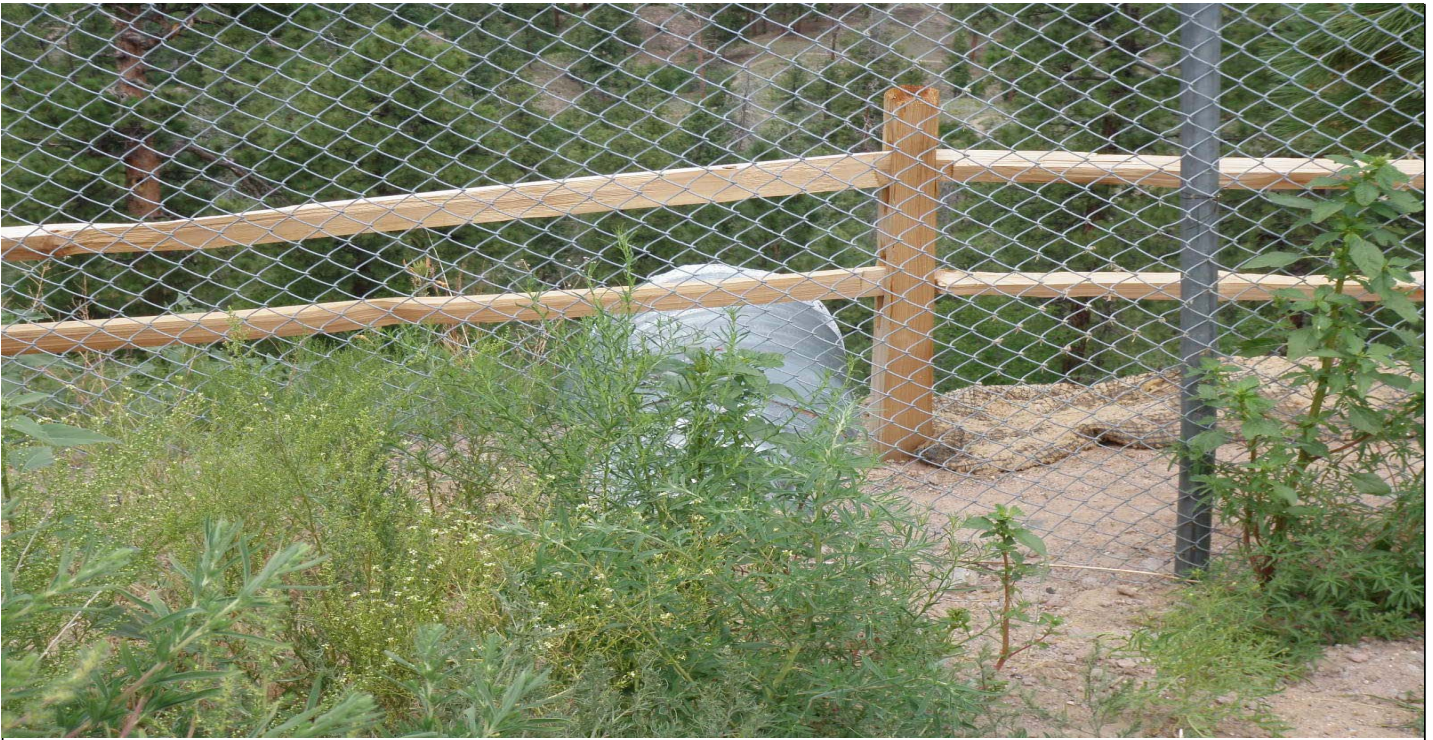
Photo 8653-8.JPG (taken 07/30/10) P00504040004 : Channel/Swale - Culvert.
