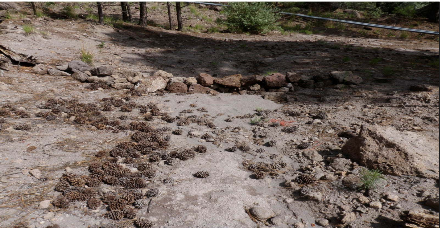
Photo 7424-3.JPG (taken 07/28/10) L01006010008 : Check Dam - Rock Check Dam.
