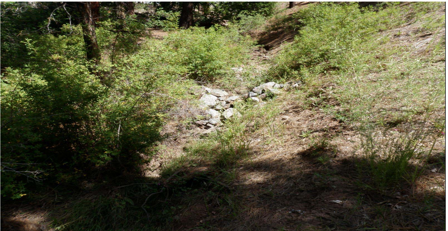
Photo 7516-2r.JPG (taken 08/12/10) E00106010007 : Check Dam - Rock Check Dam.
