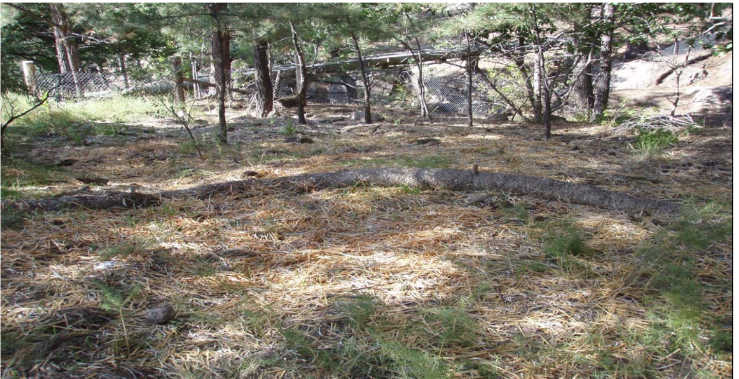
Photo 10870-6.JPG (taken 10/07/10) P00203060011 : Berms - Straw Wattles.
