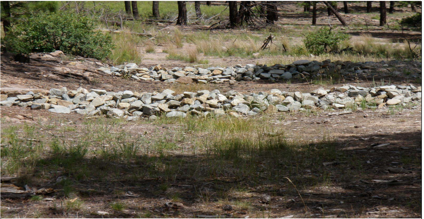
Photo 7506-5r.JPG (taken 08/11/10) J00506010011 : Check Dam - Rock Check Dam; J00506010012 : Check Dam - Rock Check Dam.
