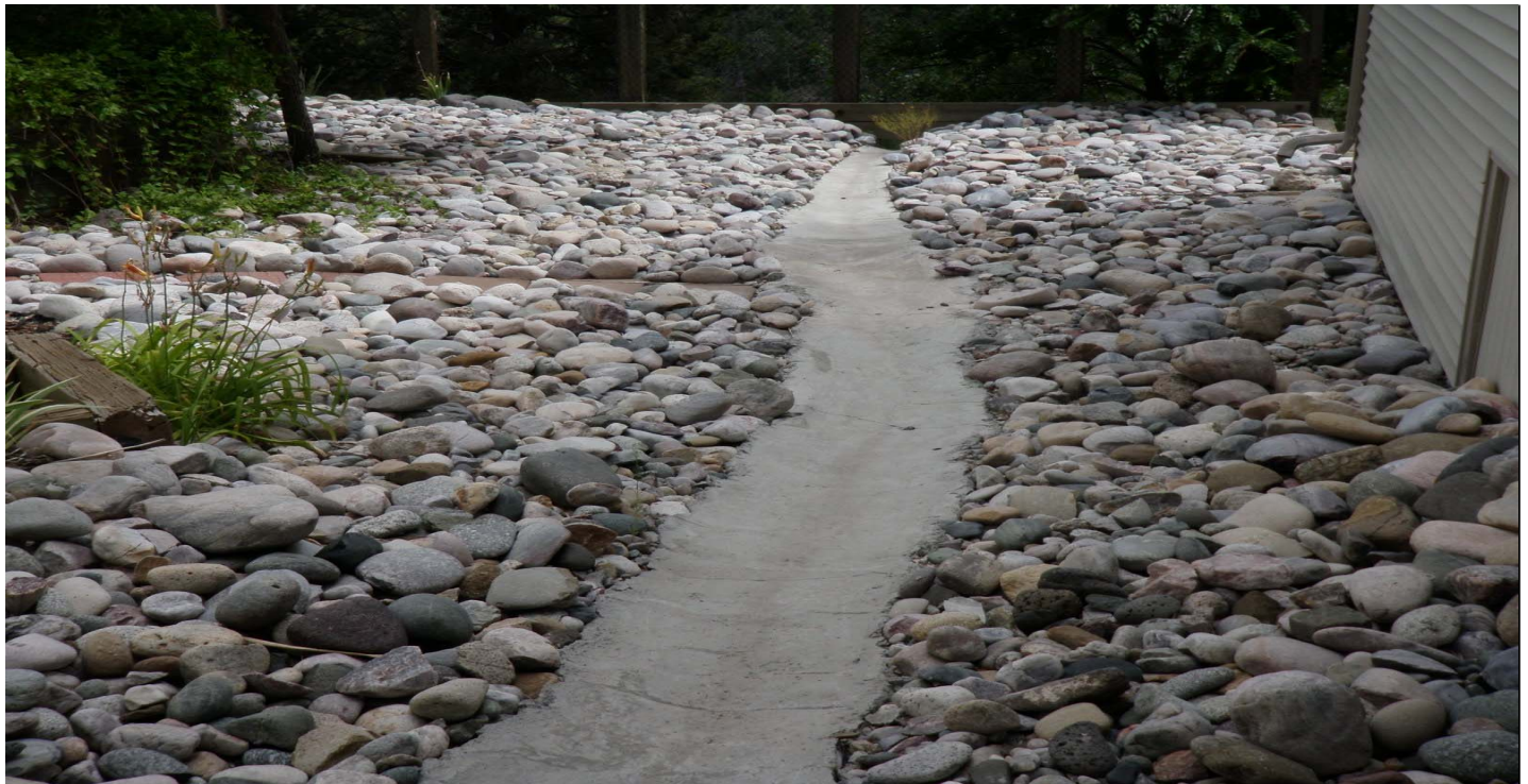
Photo 7424-1.JPG (taken 07/28/10) L01004060004 : Channel/Swale - Rip Rap; L01004060005 : Channel/Swale - Rip Rap.
