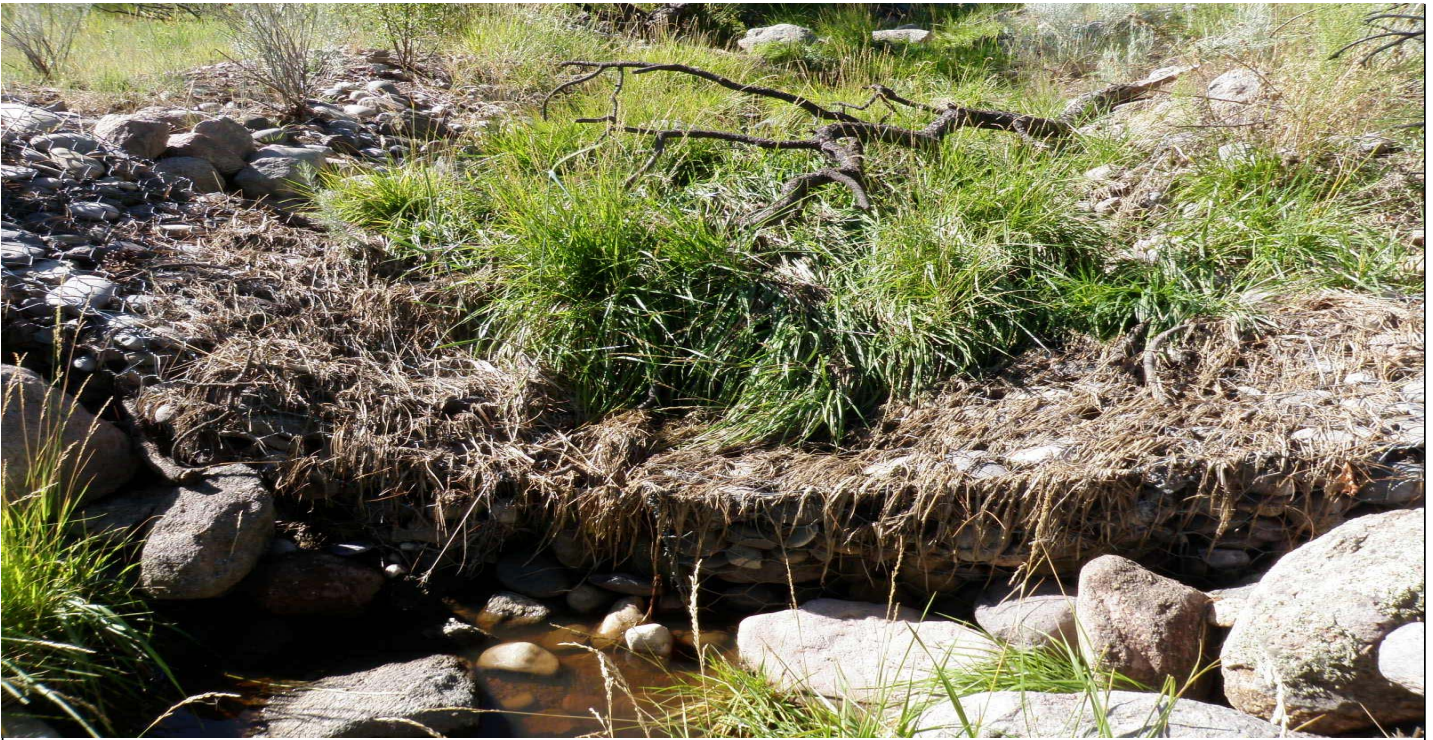
Photo 10552-7.JPG (taken 07/28/10) L00107010005 : Gabions - Gabions.
