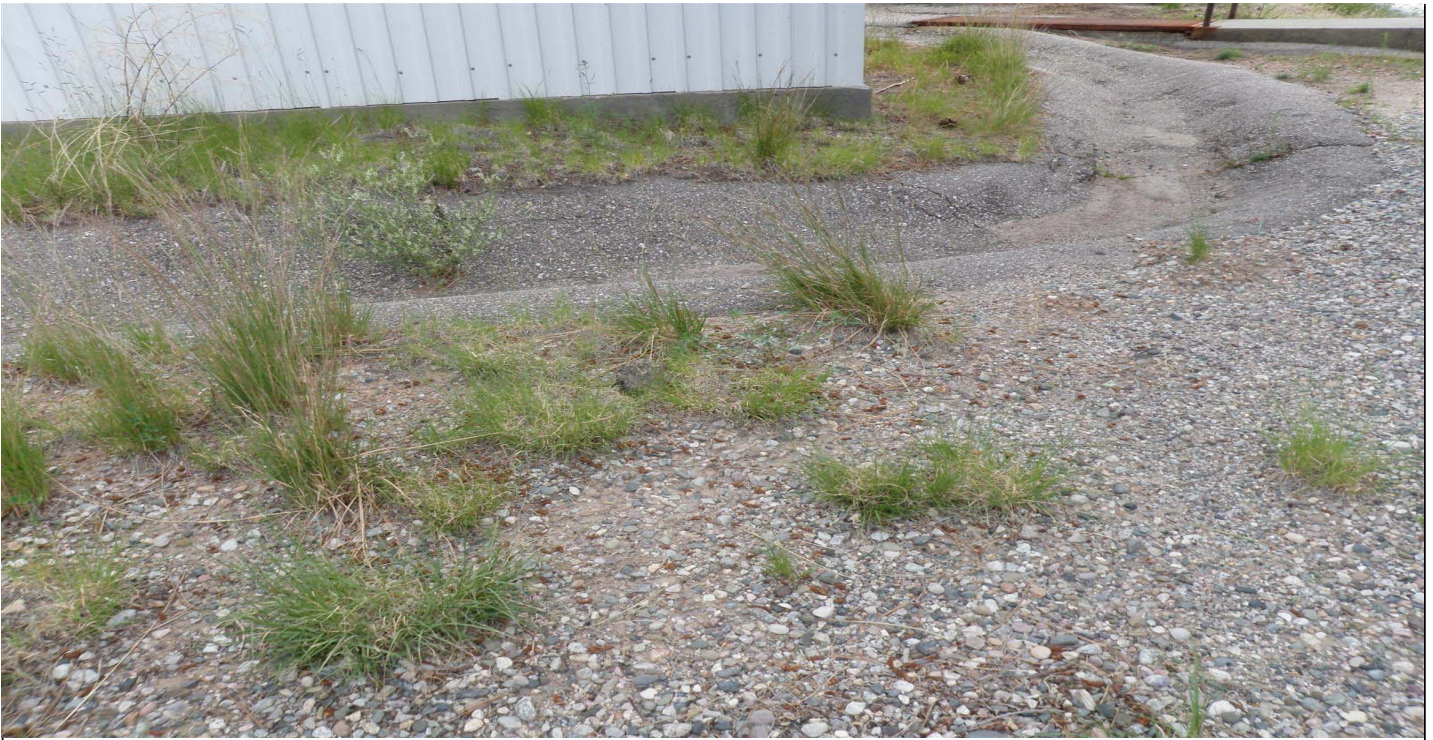
Photo 7522-1r.JPG (taken 08/12/10) E01304020003 : Channel/Swale - Concrete/Asphalt Channel/Swale.
