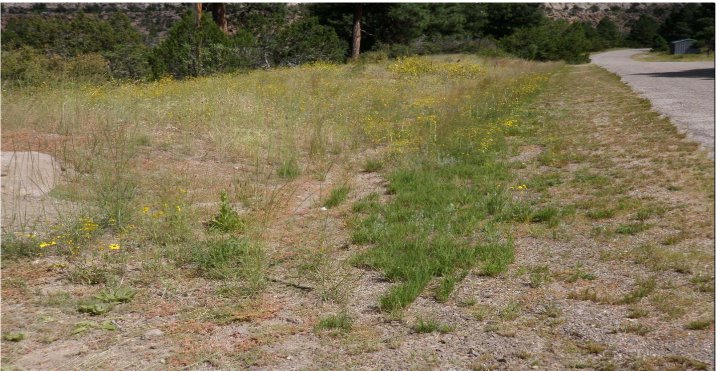
Photo 8791-4r.JPG (taken 09/07/10) A00604010007 : Channel/Swale - Earthen Channel/Swale.
