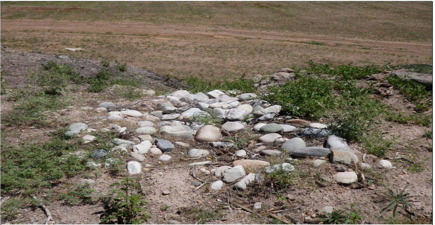
Photo 7596-4r.JPG (taken 08/13/10) I00704060002 : Channel/Swale - Rip Rap.
