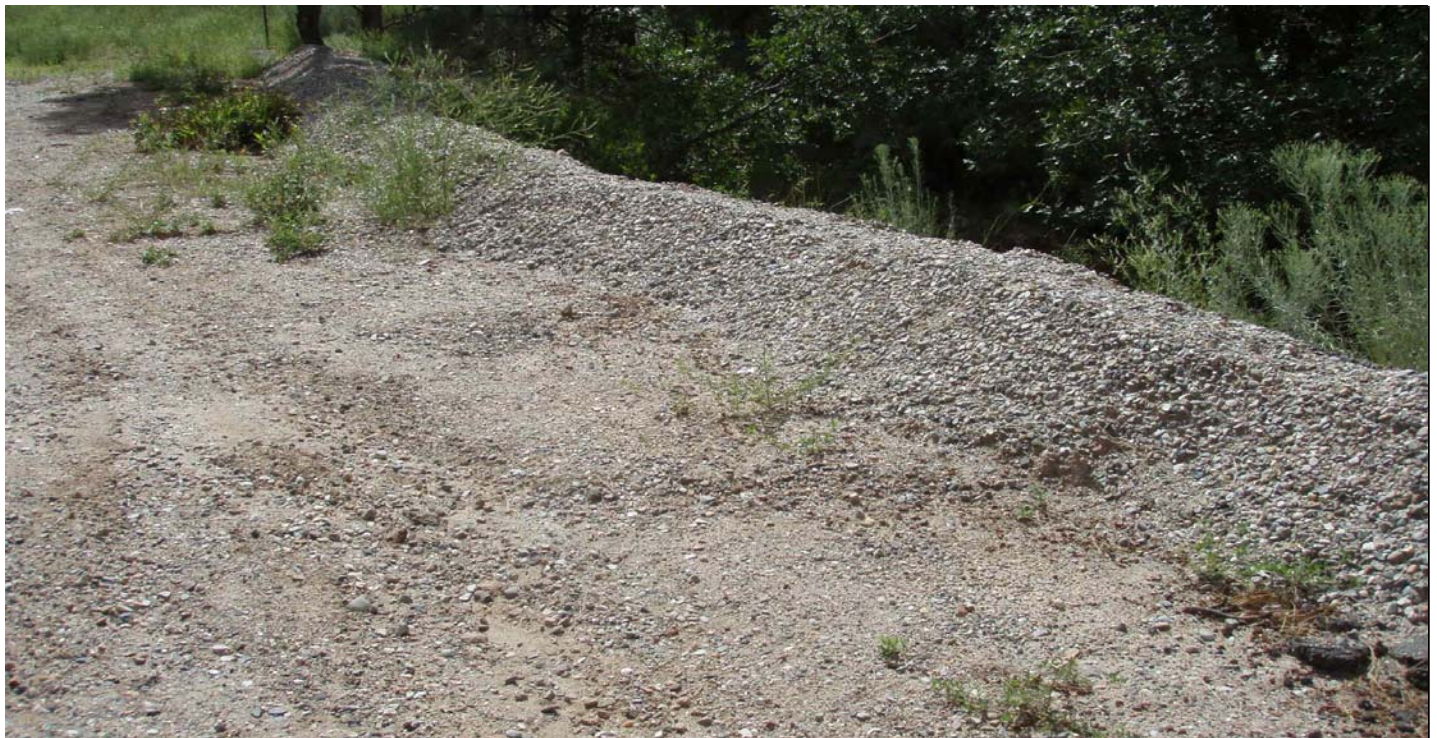
Photo 7600-1.JPG (taken 08/03/10) S00303020008 : Berms - Base Course Berm.
