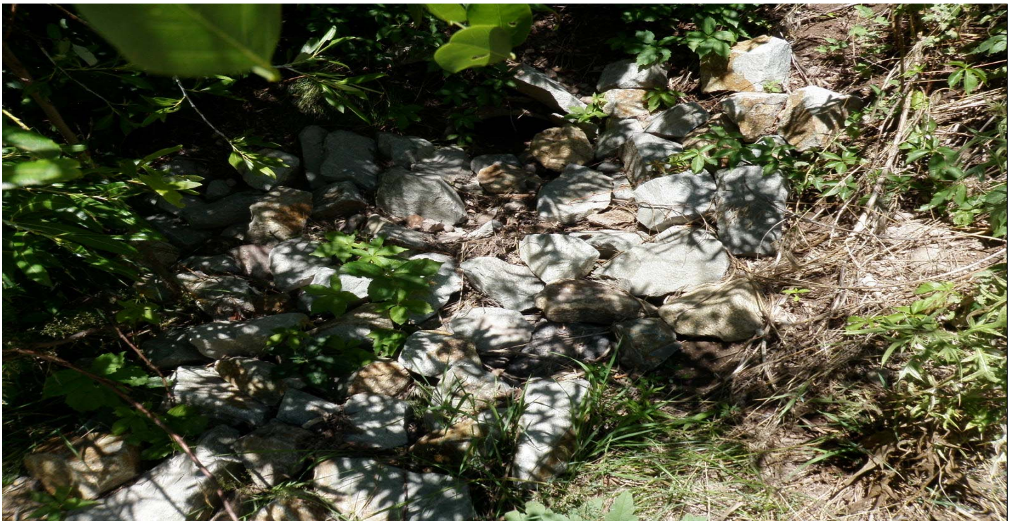
Photo 7427-1.JPG (taken 07/28/10) L01404060007 : Channel/Swale - Rip Rap.
