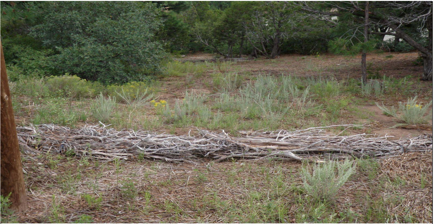
Photo 7485-1r.JPG (taken 08/10/10) C00106030003 : Check Dam - Juniper Bales.
