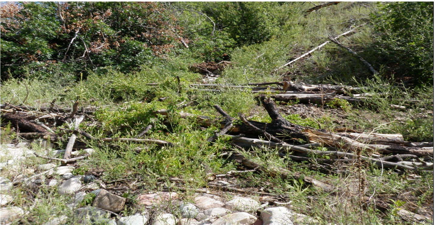
Photo 7481-6r.JPG (taken 08/10/10) C00702010003 : Established Vegetation - Permanent Vegetation Grasses and Shrubs; C00706020015 : Check Dam - Log Check Dam; C00706020016 : Check Dam - Log Check Dam.
