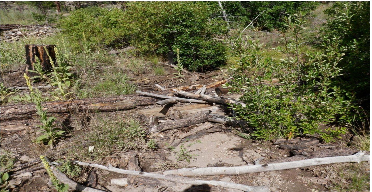
Photo 7484-4r.JPG (taken 08/10/10) C00206020007 : Check Dam - Log Check Dam.
