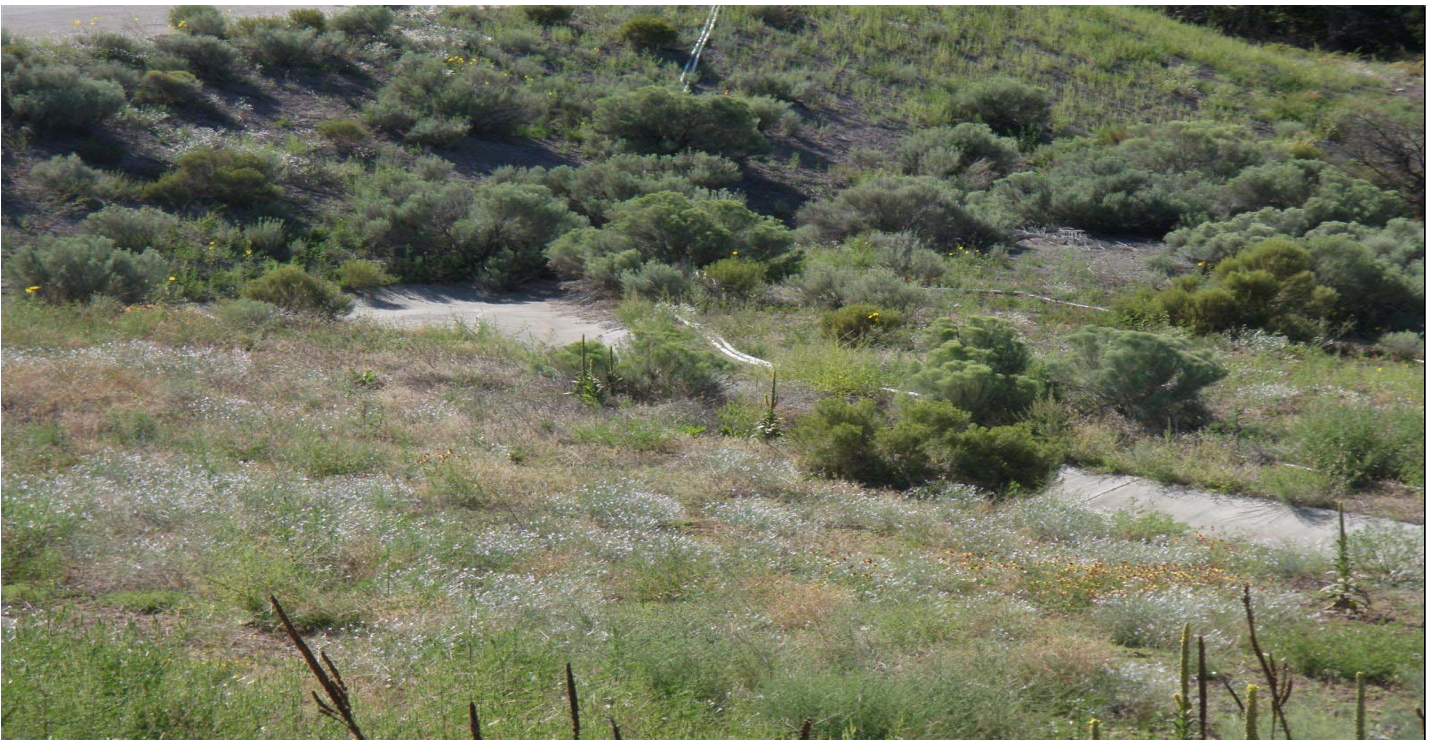
Photo 8505-4r.JPG (taken 08/20/10) J02504020006 : Channel/Swale - Concrete/Asphalt Channel/Swale.
