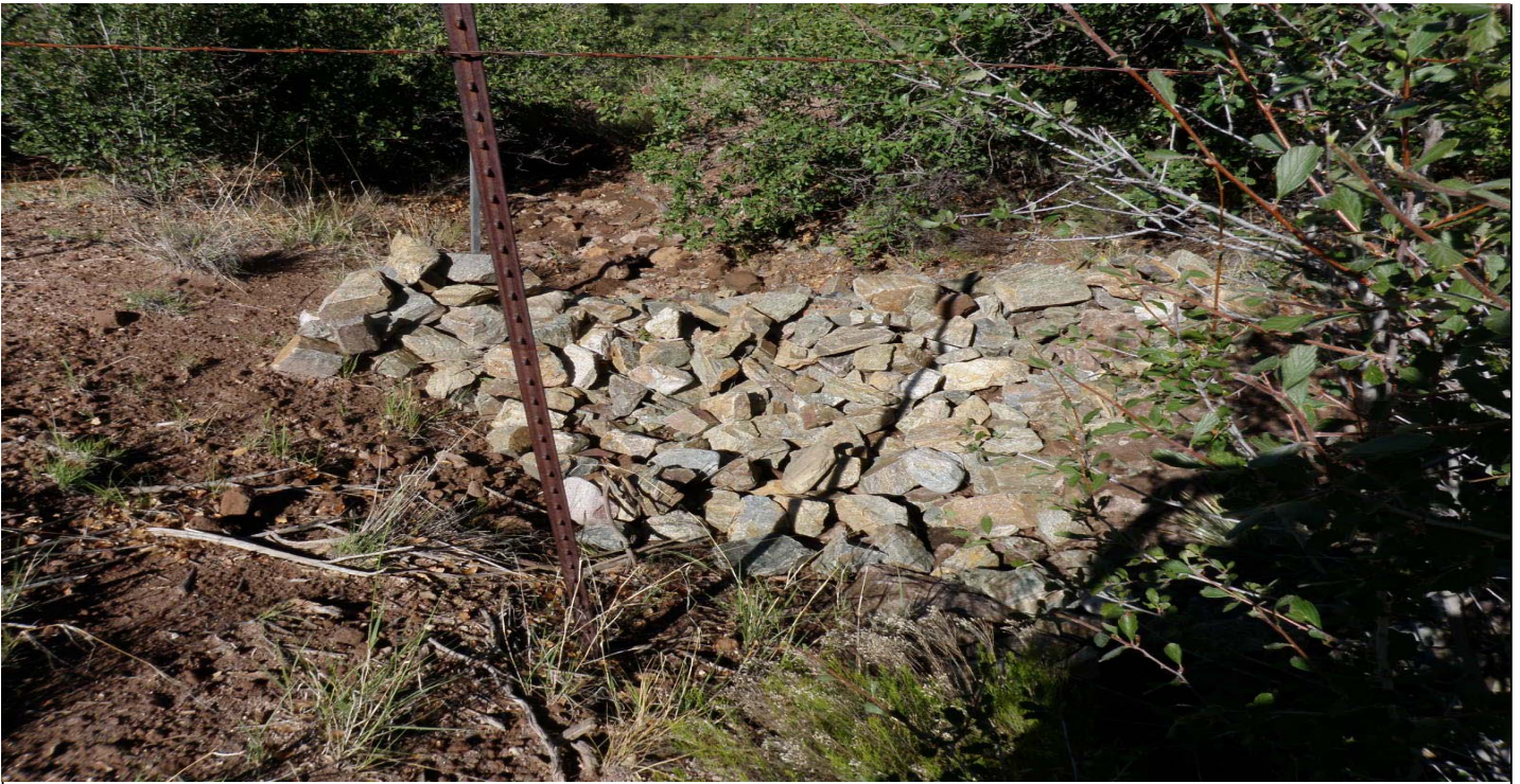
Photo 7356-5.JPG (taken 07/27/10) Q00806010003 : Check Dam - Rock Check Dam.
