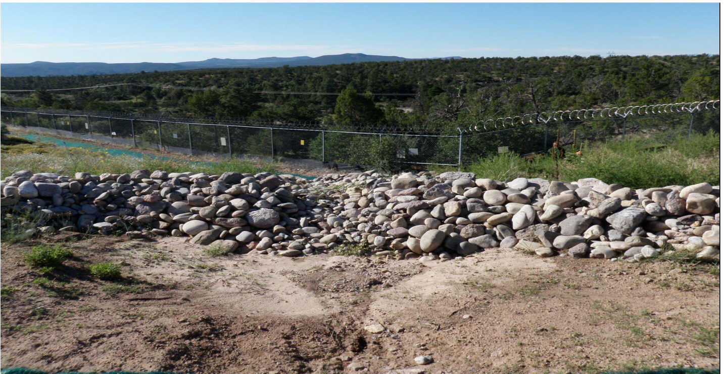
Photo 8504-2r.JPG (taken 08/20/10) J02606010004 : Check Dam - Rock Check Dam.
