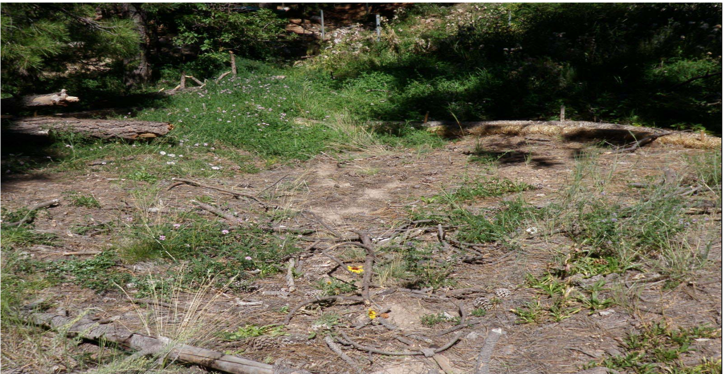
Photo 8661-1r.JPG (taken 09/03/10) S00103060009 : Berms - Straw Wattles.
