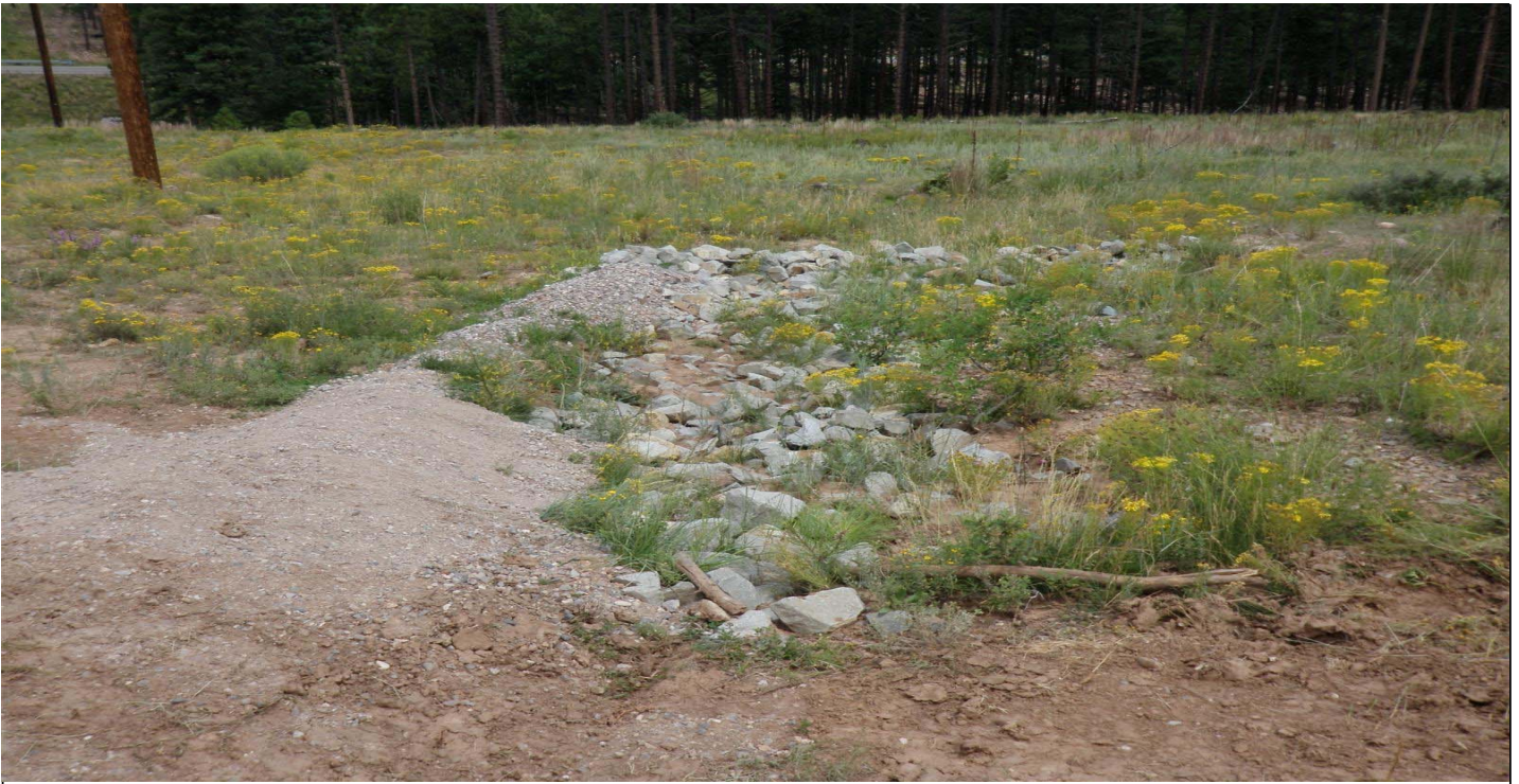
Photo 7501-5r.JPG (taken 08/11/10) J00104060011 : Channel/Swale - Rip Rap; J00106010010 : Check Dam - Rock Check Dam.
