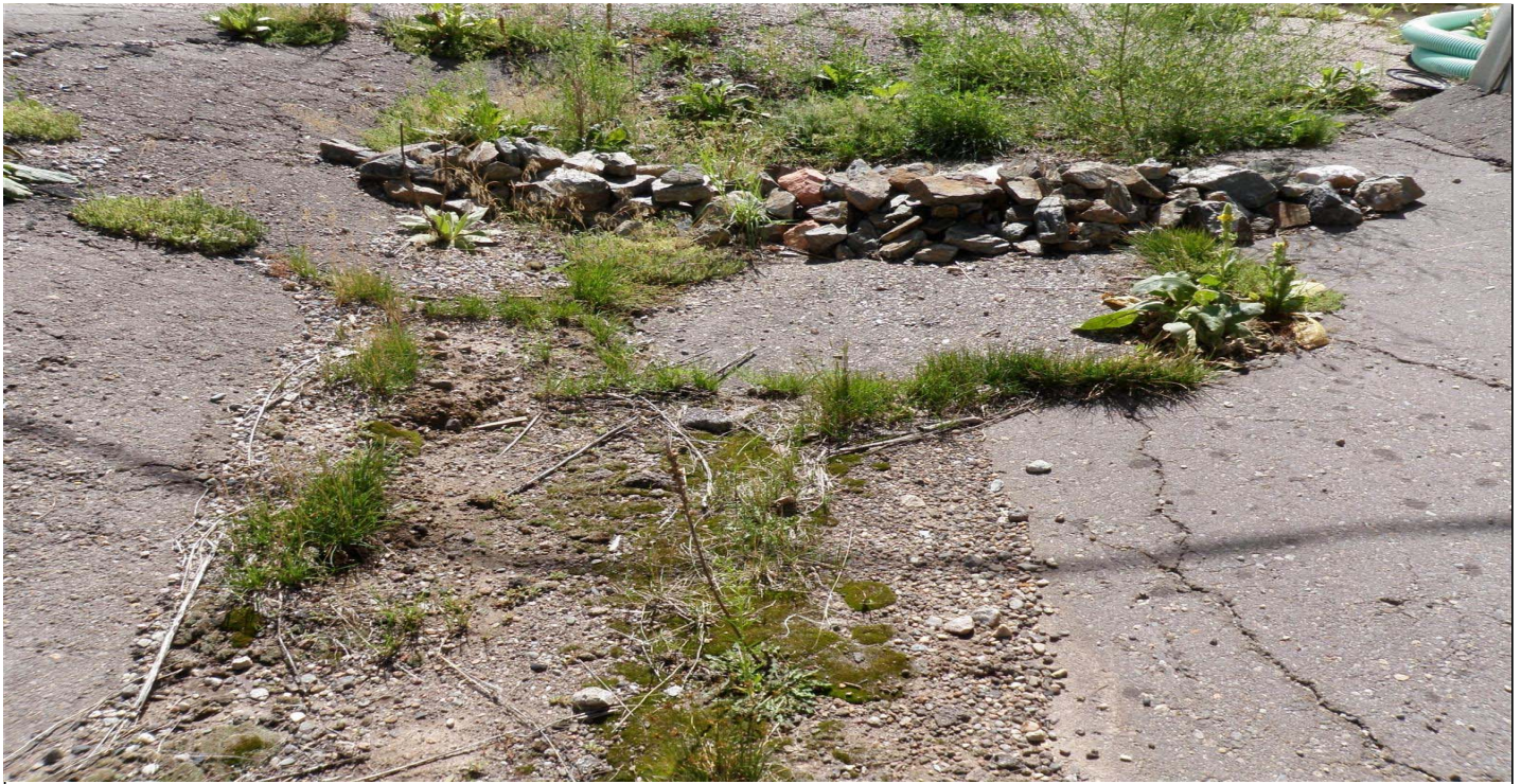
Photo 7526-4r.JPG (taken 08/12/10) J02106010003 : Check Dam - Rock Check Dam.
