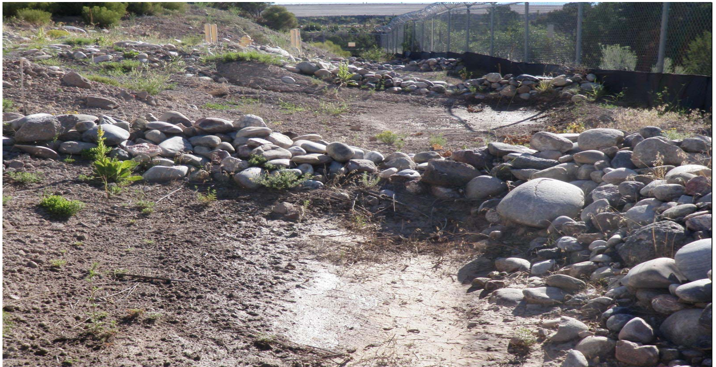
Photo 8507-1r.JPG (taken 08/20/10) J02406010004 : Check Dam - Rock Check Dam.
