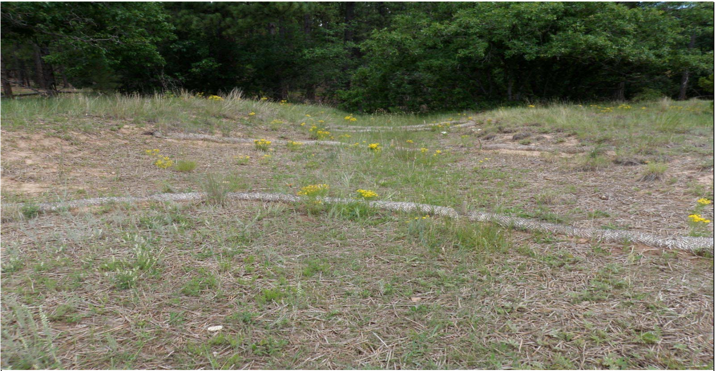
Photo 7498-1r.JPG (taken 08/11/10) J02901010007 : Seed and Mulch - Seed and Wood Mulch; J02902010001 : Established Vegetation - Permanent Vegetation Grasses and Shrubs; J02903060004 : Berms - Straw Wattles; J02903060005 : Berms - Straw Wattles; J02903060006 : Berms - Straw Wattles.
