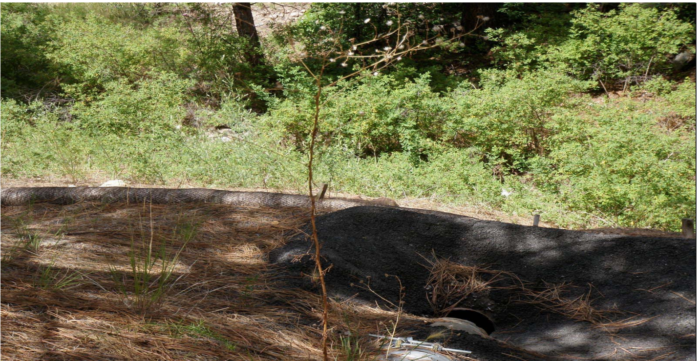
Photo 7516-8r.JPG (taken 08/12/10) E00103060002 : Berms - Straw Wattles.
