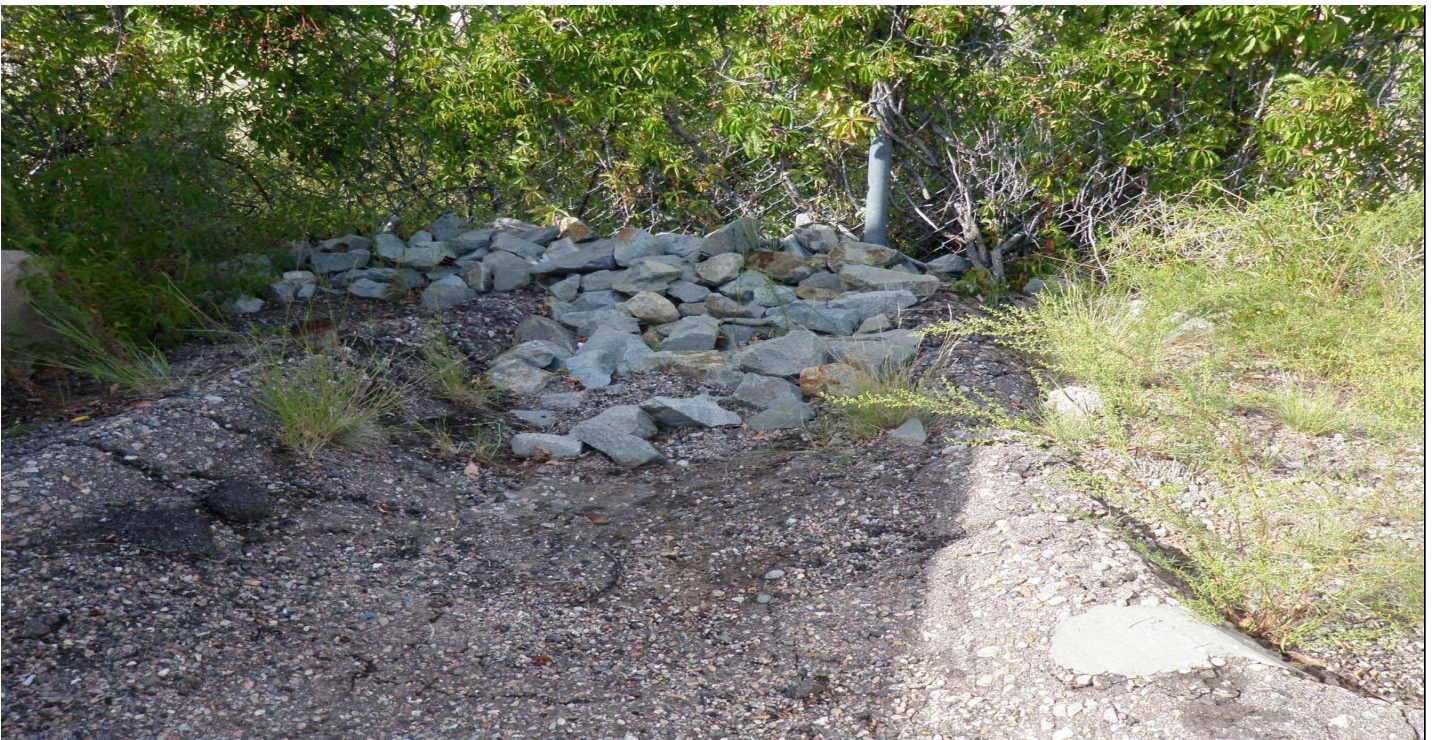
Photo 7483-3r.JPG (taken 08/10/10) C00504060007 : Channel/Swale - Rip Rap.
