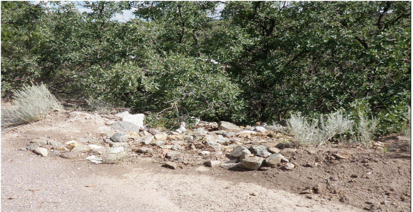
Photo 7480-1r.JPG (taken 08/10/10) C00904010002 : Channel/Swale - Earthen Channel/Swale; C00904060001 : Channel/Swale - Rip Rap.
