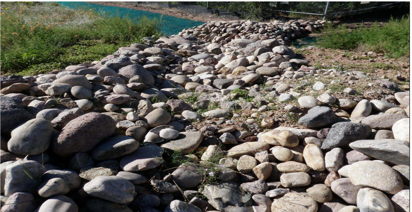
Photo 8504-4r.JPG (taken 08/20/10) J02604060007 : Channel/Swale - Rip Rap.
