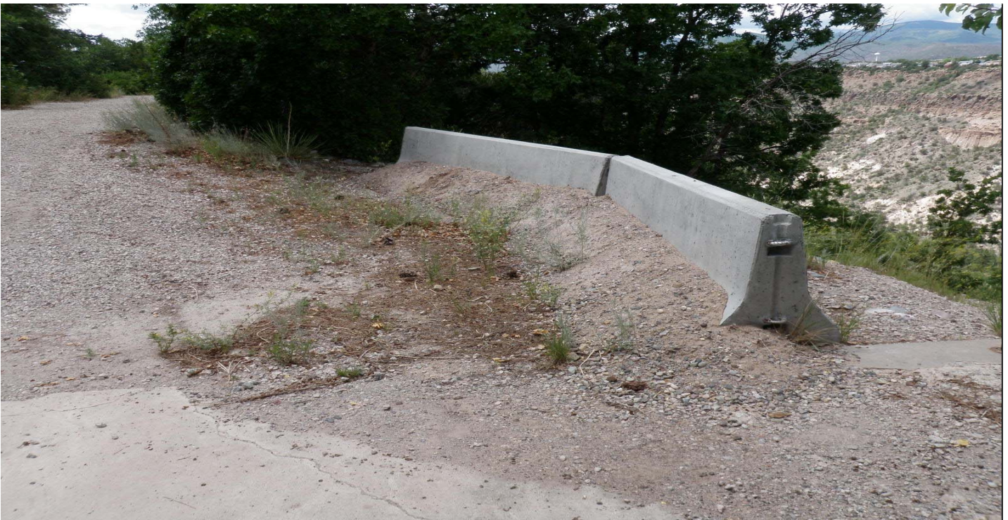
Photo 7417-6.JPG (taken 07/30/10) P00603020009 : Berms - Base Course Berm.
