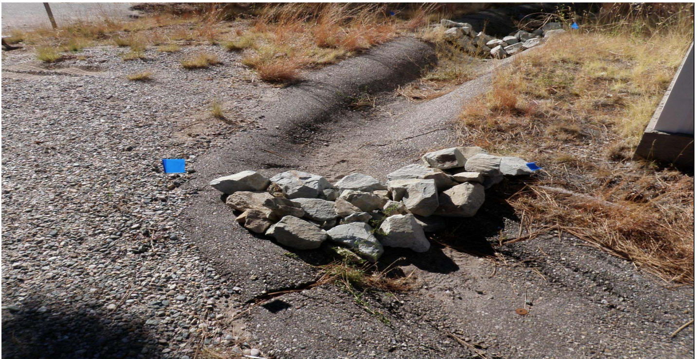
Photo 11698-1r.JPG (taken 11/18/10) E01306010004 : Check Dam - Rock Check Dam; E01306010005 : Check Dam - Rock Check Dam.
