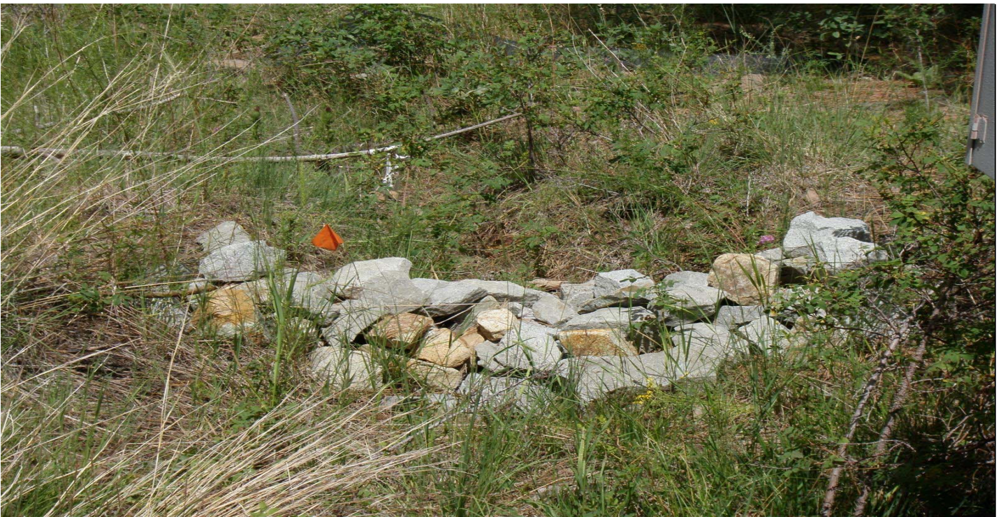
Photo 7503-4r.JPG (taken 08/11/10) J00206010014 : Check Dam - Rock Check Dam.
