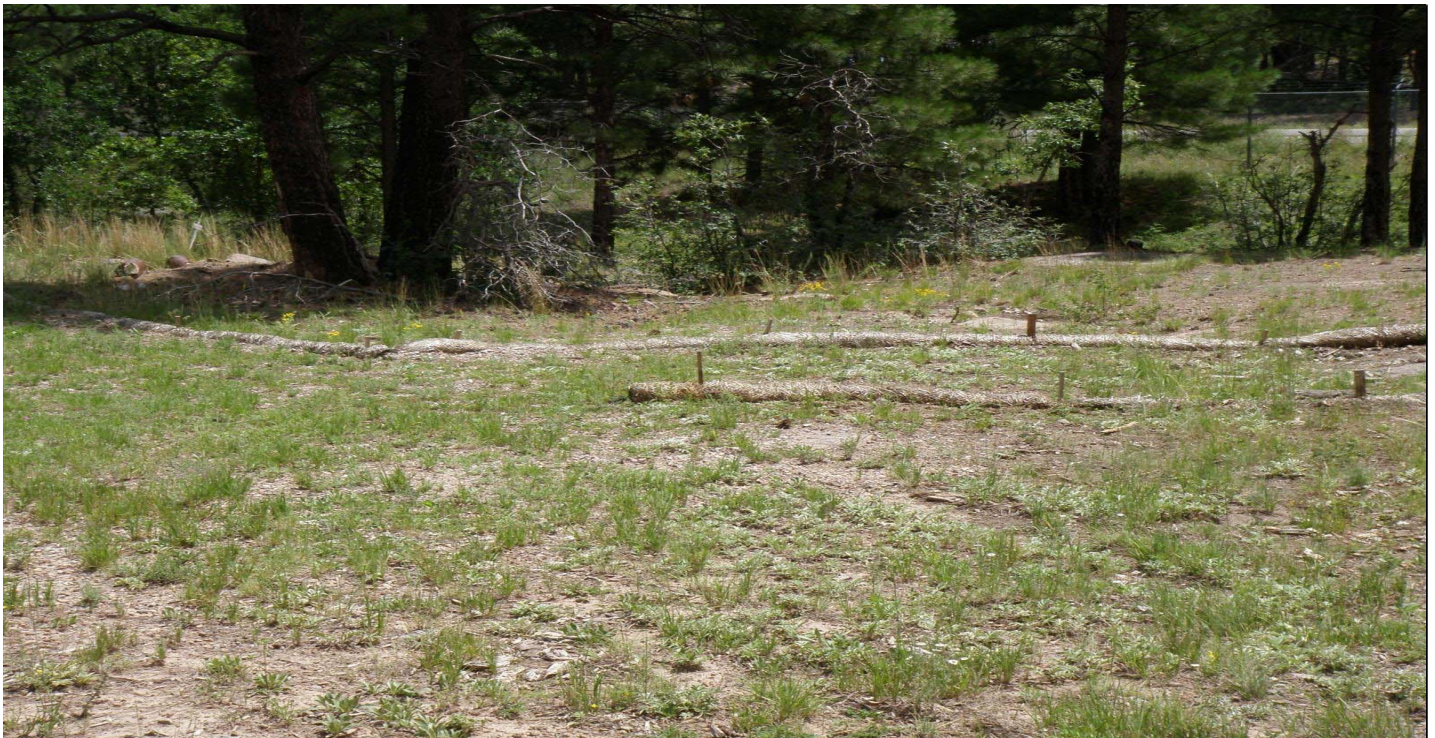
Photo 7502-1r.JPG (taken 08/11/10) J00403060003 : Berms - Straw Wattles; J00403060004 : Berms - Straw Wattles; J00403060005 : Berms - Straw Wattles.
