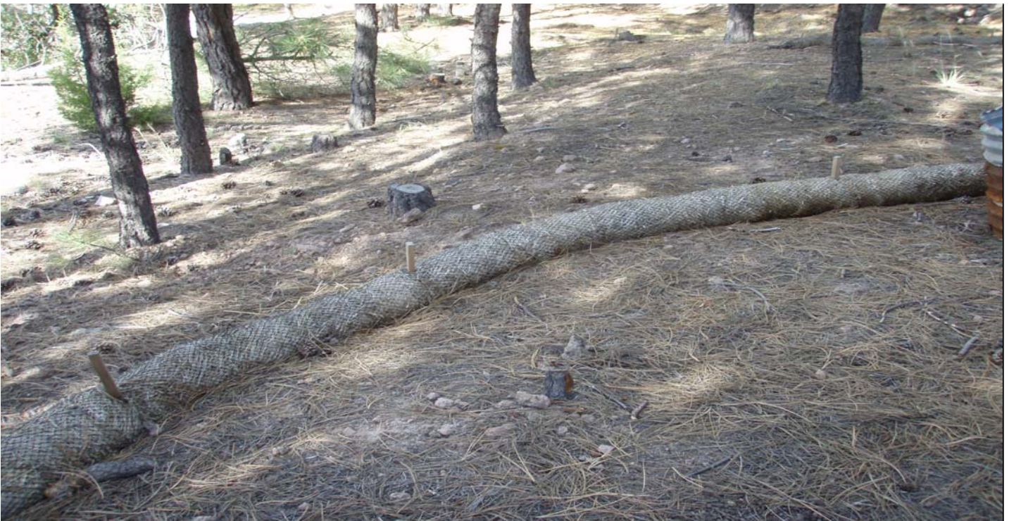
Photo 10870-4.JPG (taken 10/07/10) P00203060009 : Berms - Straw Wattles.
