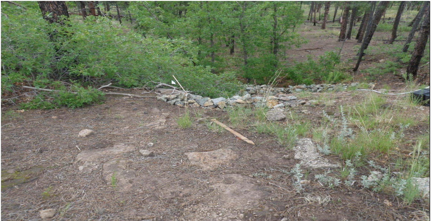
Photo 7515-1r.JPG (taken 08/12/10) H00106010004 : Check Dam - Rock Check Dam.
