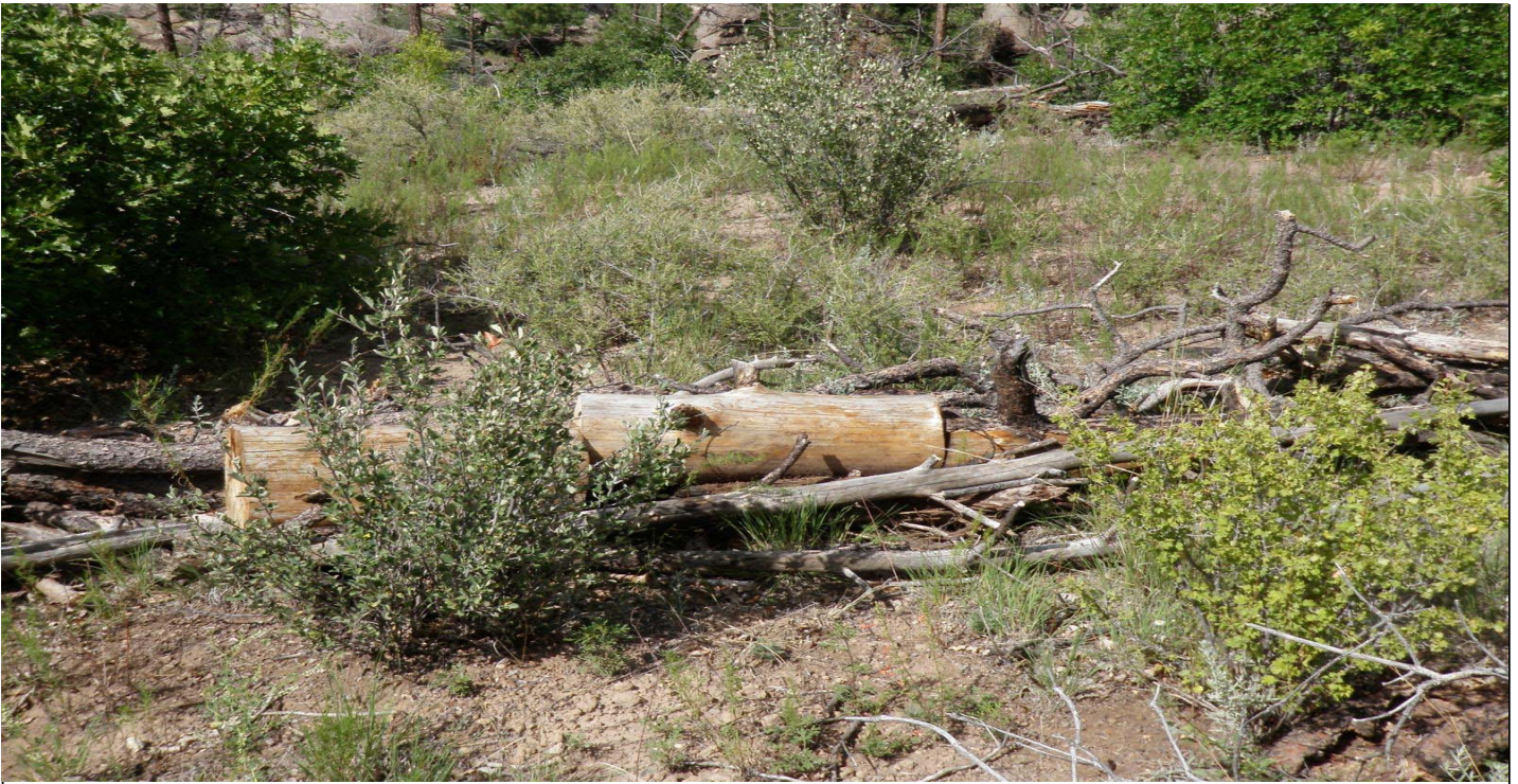
Photo 7481-3r.JPG (taken 08/10/10) C00706020017 : Check Dam - Log Check Dam.
