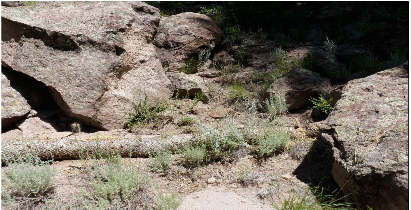
Photo 7430-1.JPG (taken 07/29/10) L02003060005 : Berms - Straw Wattles.
