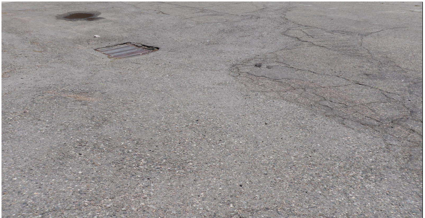
Photo 7596-1r.JPG (taken 08/13/10) I00704040005 : Channel/Swale - Culvert.
