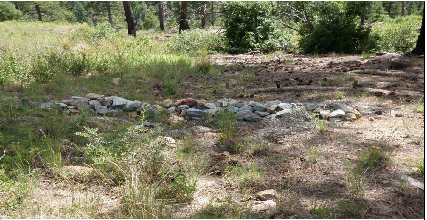
Photo 7506-3r.JPG (taken 08/11/10) J00506010010 : Check Dam - Rock Check Dam.
