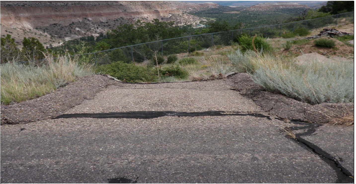
Photo 8653-13.JPG (taken 07/30/10) P00504020005 : Channel/Swale - Concrete/Asphalt Channel/Swale.
