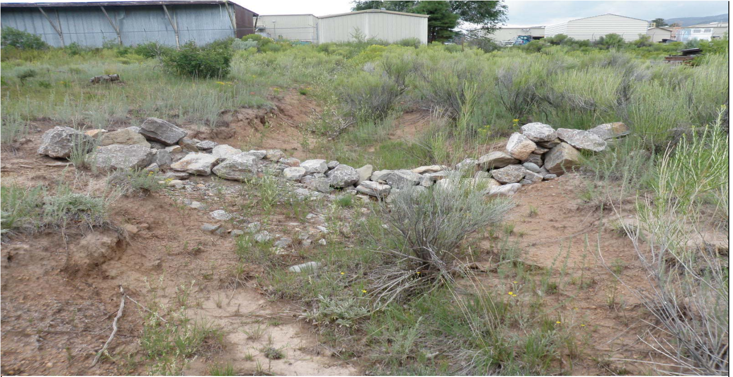
Photo 7451-3.JPG (taken 08/04/10) S00606010013 : Check Dam - Rock Check Dam.
