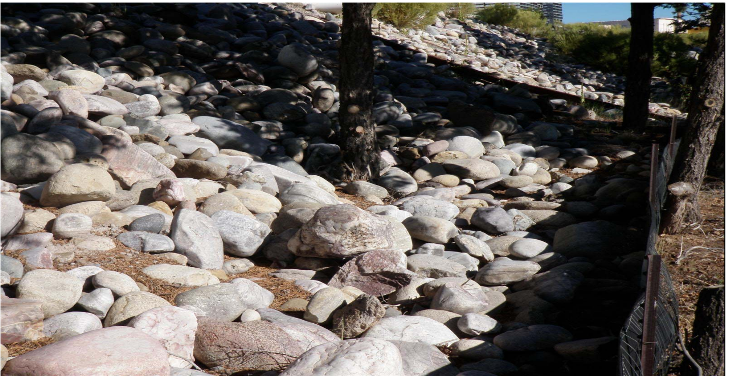
Photo 8507-3r.JPG (taken 08/20/10) J02404060007 : Channel/Swale - Rip Rap.
