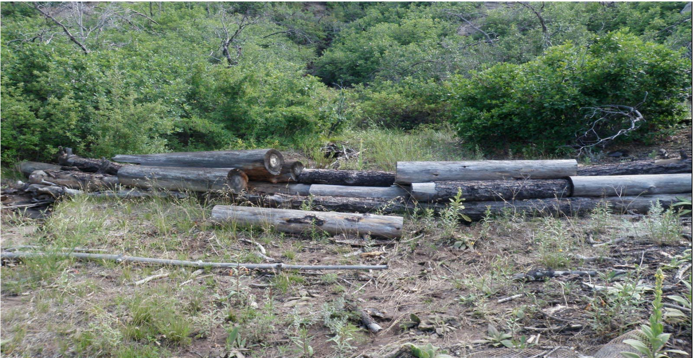
Photo 7484-2r.JPG (taken 08/10/10) C00206020012 : Check Dam - Log Check Dam.
