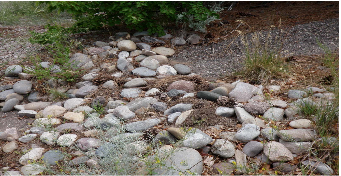
Photo 7417-7.JPG (taken 07/30/10) P00604060002 : Channel/Swale - Rip Rap.
