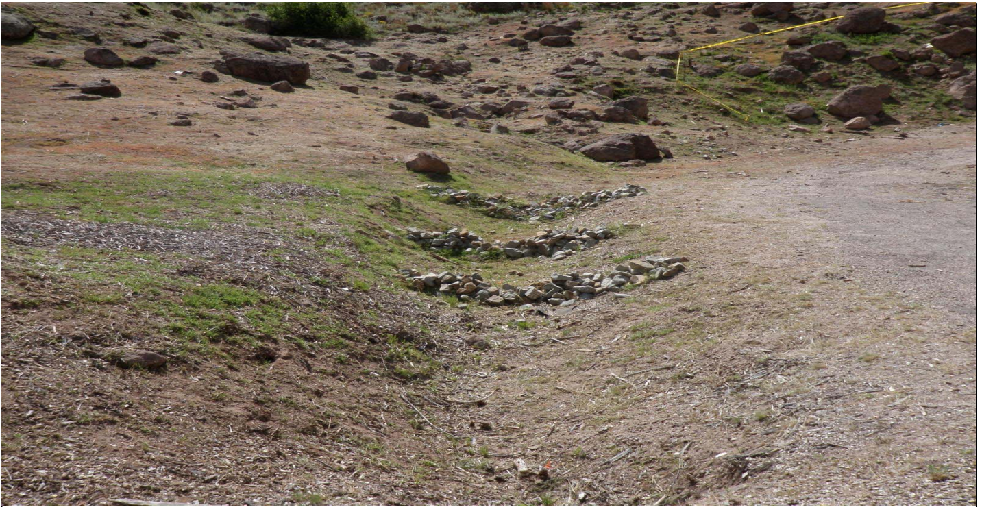
Photo 8791-5r.JPG (taken 09/07/10) A00602010001 : Established Vegetation - Permanent Vegetation Grasses and Shrubs; A00606010010 : Check Dam - Rock Check Dam; A00606010011 : Check Dam - Rock Check Dam; A00606010012 : Check Dam - Rock Check Dam.
