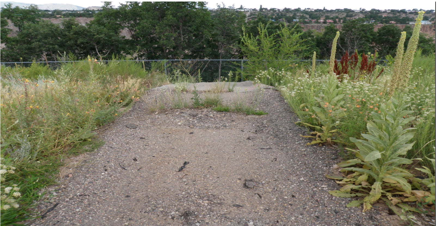
Photo 8653-2.JPG (taken 07/30/10) P00504020011 : Channel/Swale - Concrete/Asphalt Channel/Swale.
