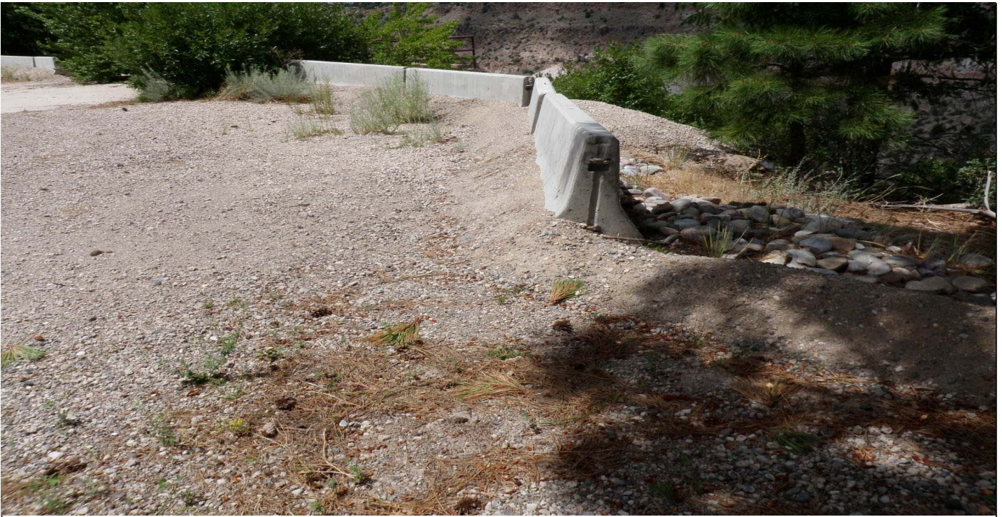
Photo 7417-5.JPG (taken 07/30/10) P00603020010 : Berms - Base Course Berm.
