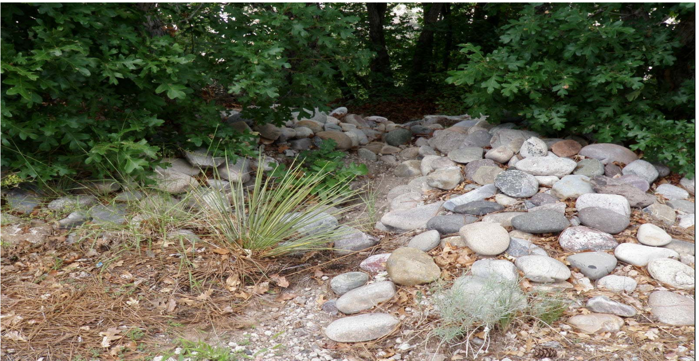
Photo 7417-8.JPG (taken 07/30/10) P00604060003 : Channel/Swale - Rip Rap.
