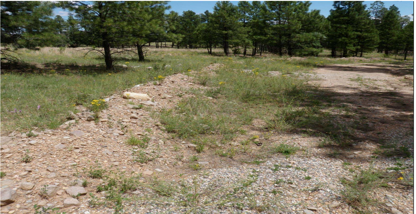
Photo 7500-3r.JPG (taken 08/11/10) J03103020004 : Berms - Base Course Berm.
