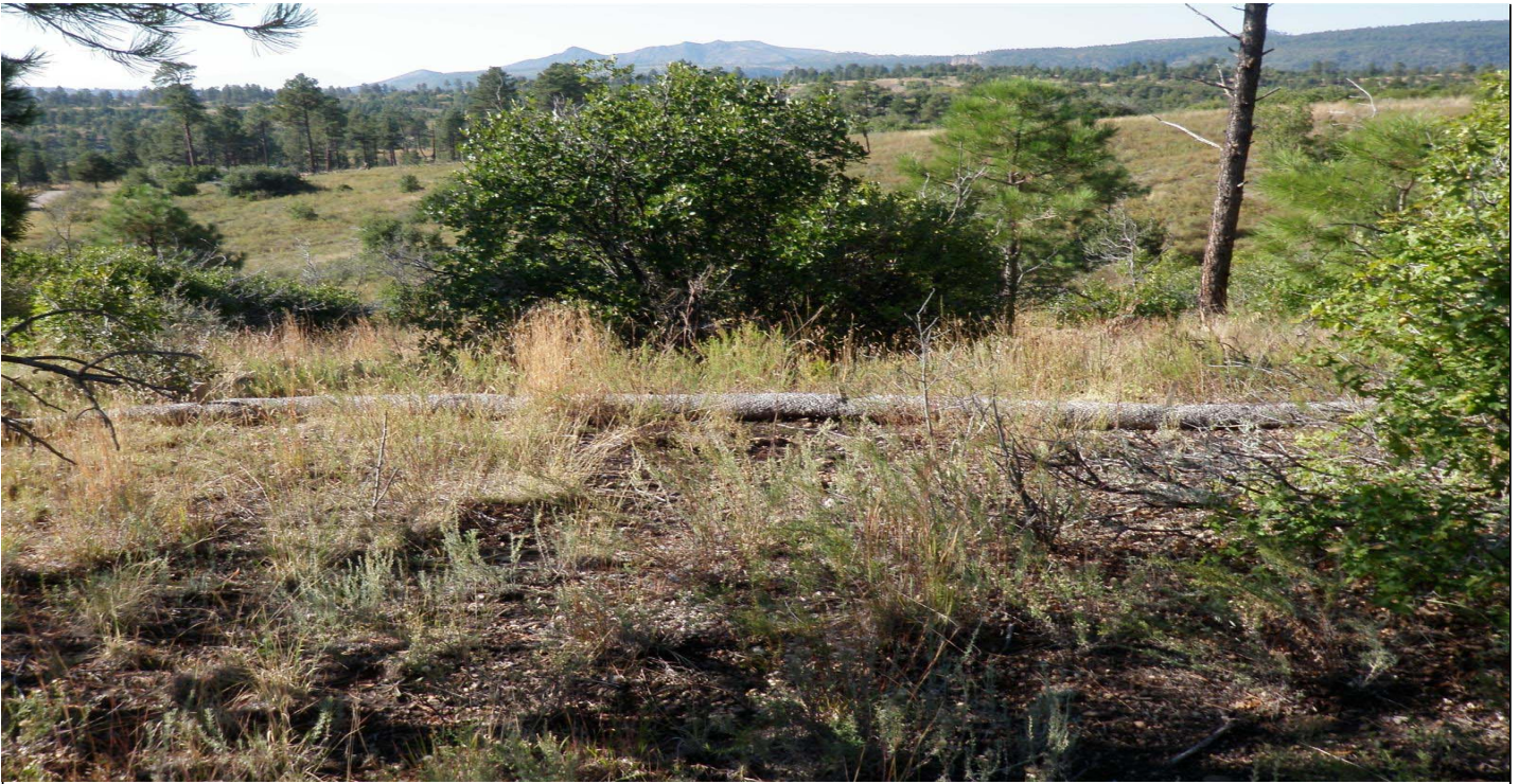
Photo 10874-2r.JPG (taken 10/07/10) W01403060003 : Berms - Straw Wattles.
