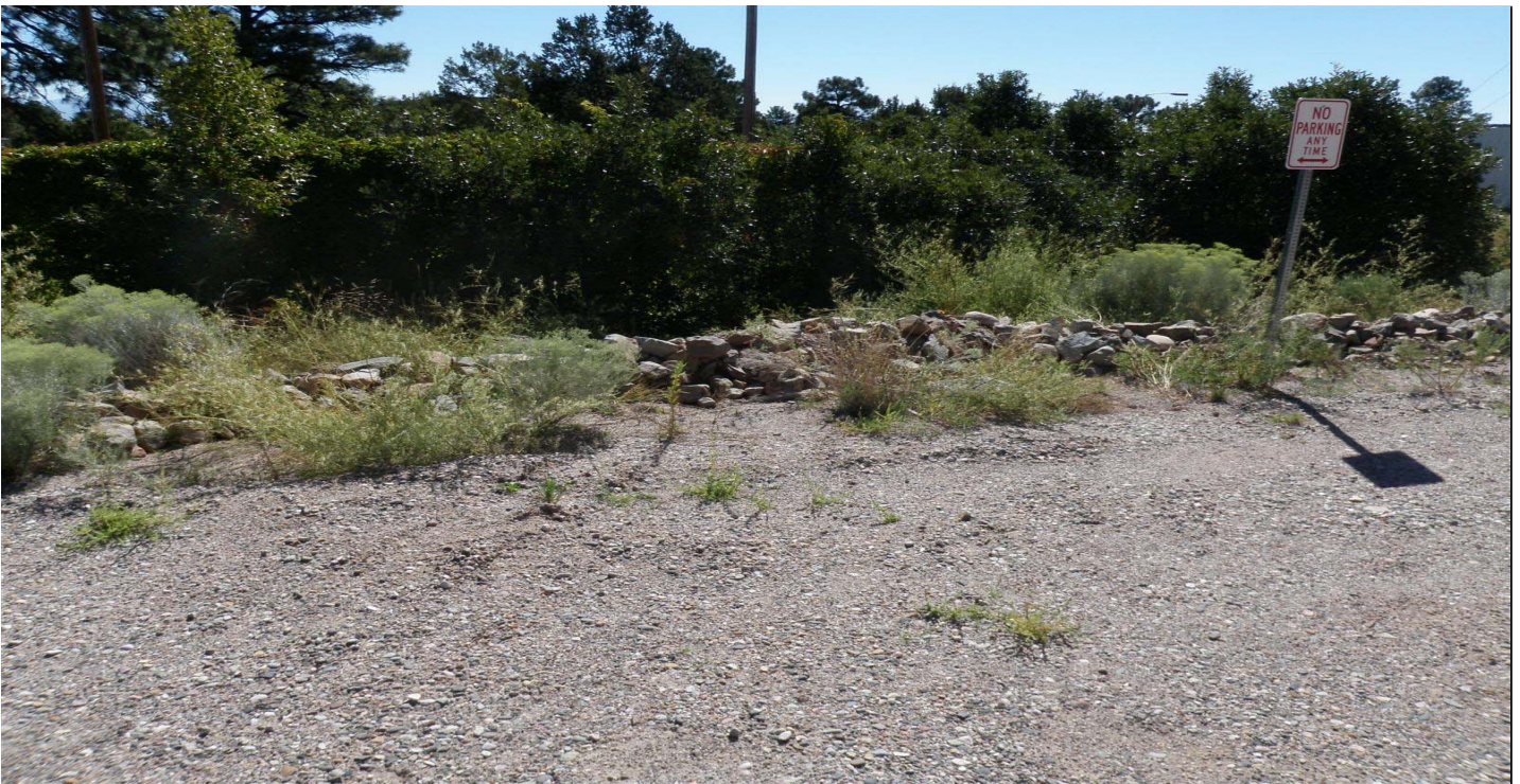
Photo 8670-1r.JPG (taken 09/02/10) C00103120009 : Berms - Rock Berm.
