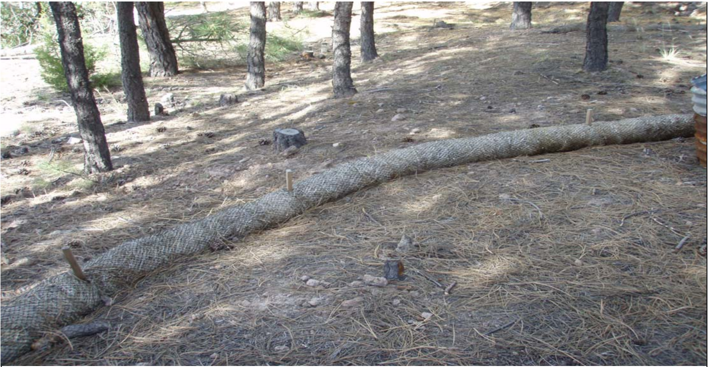
Photo 10871-5.JPG (taken 10/07/10) P00303060007 : Berms - Straw Wattles.
