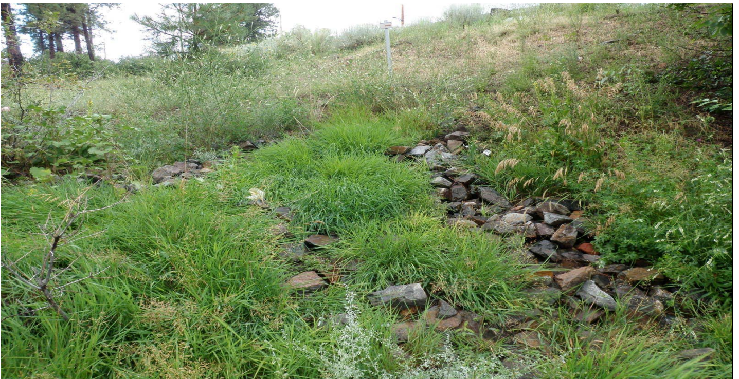
Photo 7489-3r.JPG (taken 08/09/10) M00604060007 : Channel/Swale - Rip Rap.
