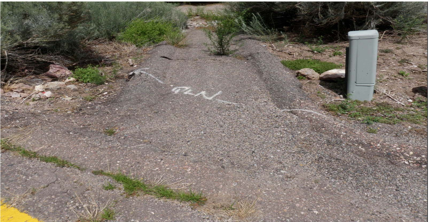
Photo 7417-4.JPG (taken 07/30/10) P00604020006 : Channel/Swale - Concrete/Asphalt Channel/Swale.
