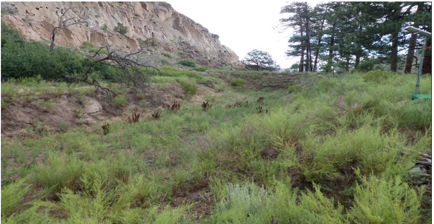
Photo 7471-1.JPG (taken 08/06/10) M02102010002 : Established Vegetation - Permanent Vegetation Grasses and Shrubs; M02105010001 : Sediment Traps and Basins - Sediment Trap.
