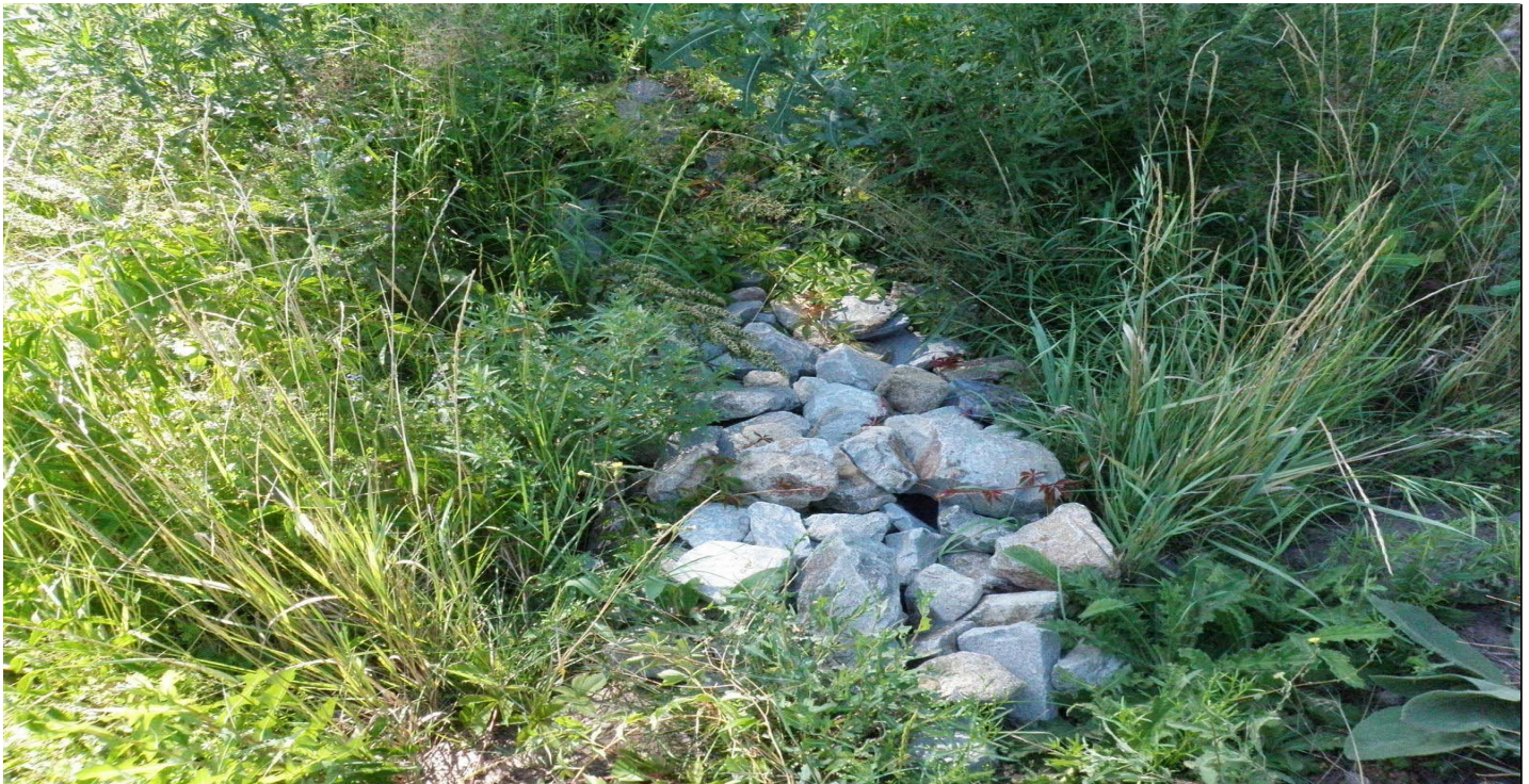
Photo 7524-1r.JPG (taken 08/12/10) J01803120004 : Berms - Rock Berm.
