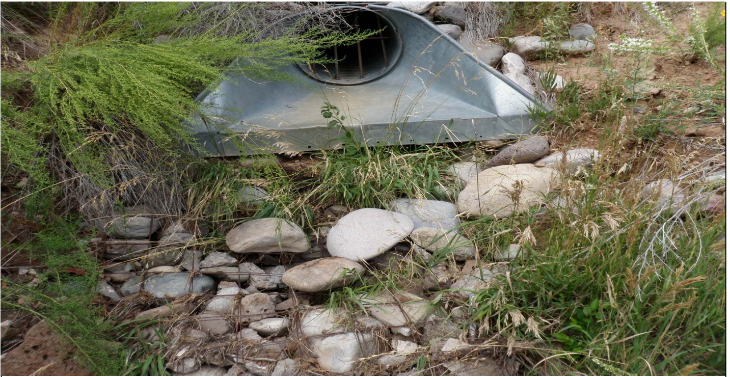
Photo 7424-2.JPG (taken 07/28/10) L01004060007 : Channel/Swale - Rip Rap.
