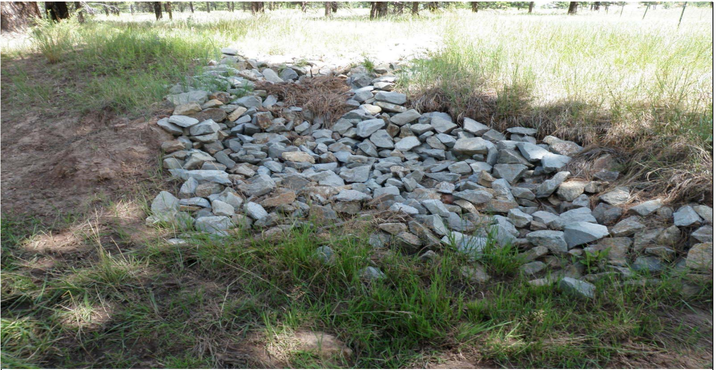
Photo 7594-3r.JPG (taken 08/13/10) W00104060001 : Channel/Swale - Rip Rap.
