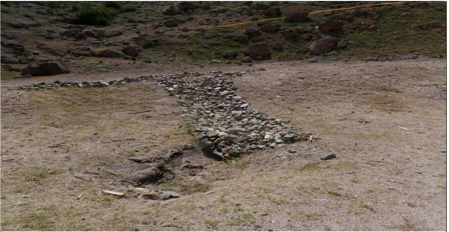
Photo 8791-1r.JPG (taken 09/07/10) A00604060002 : Channel/Swale - Rip Rap.
