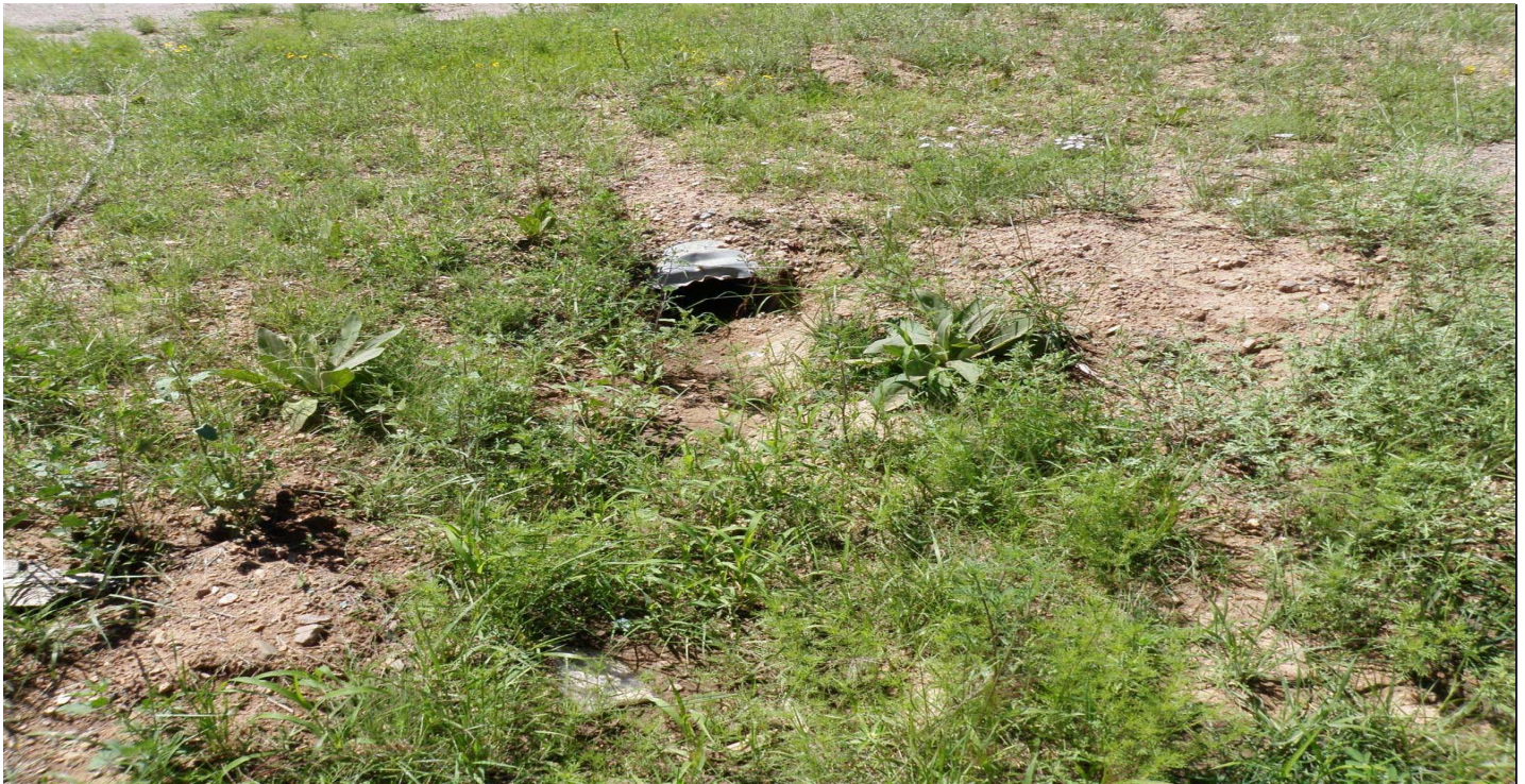
Photo 7595-1r.JPG (taken 08/13/10) I00504040005 : Channel/Swale - Culvert.
