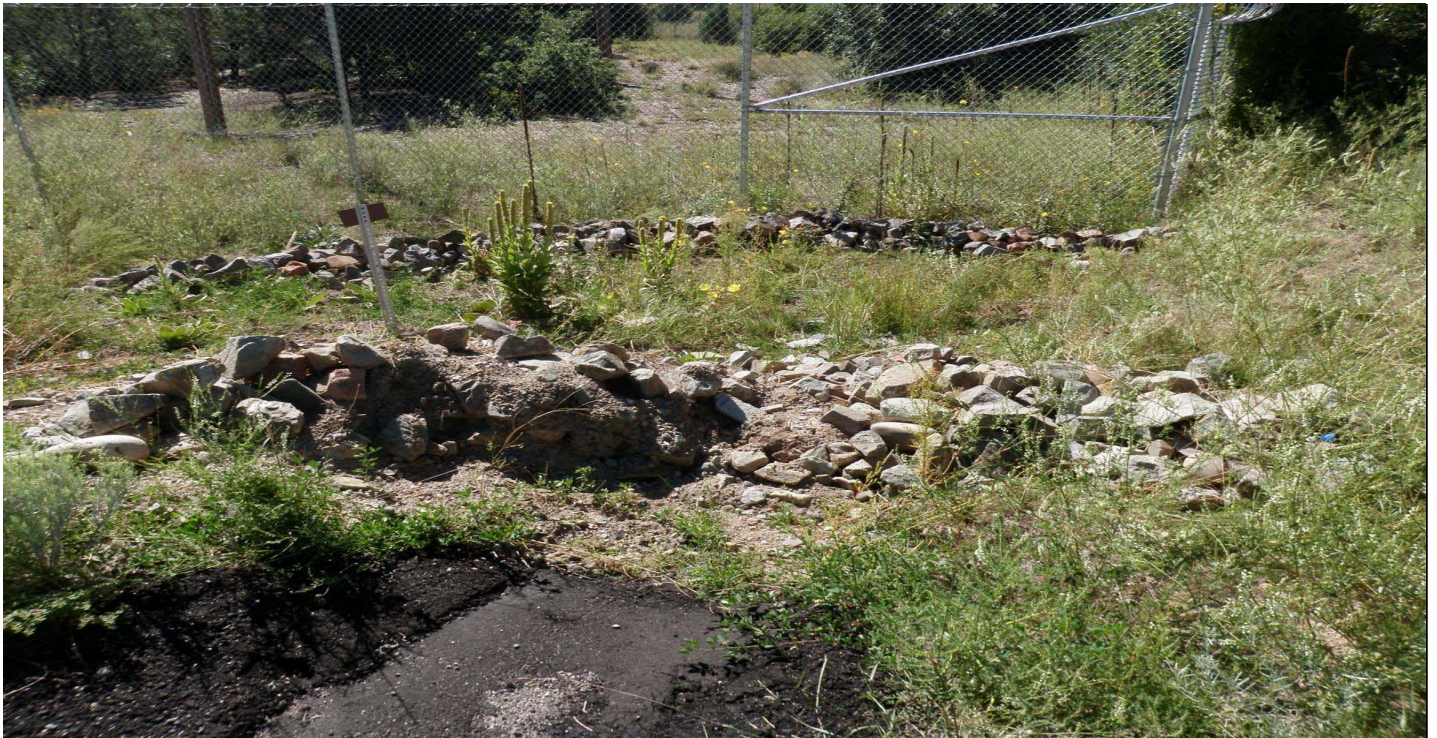
Photo 8670-2r.JPG (taken 09/02/10) C00103120010 : Berms - Rock Berm; C00106010011 : Check Dam - Rock Check Dam.
