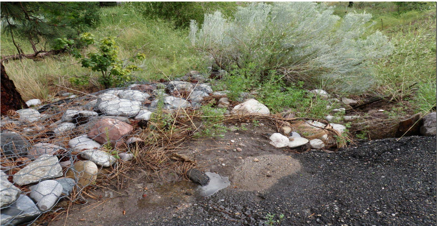
Photo 7489-7r.JPG (taken 08/09/10) M00607010006 : Gabions - Gabions.
