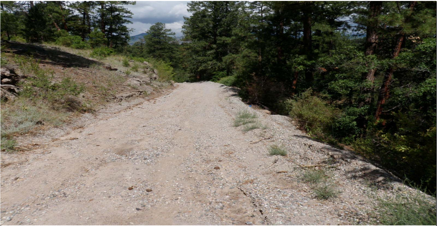
Photo 7414-1.JPG (taken 07/29/10) D00503020003 : Berms - Base Course Berm.
