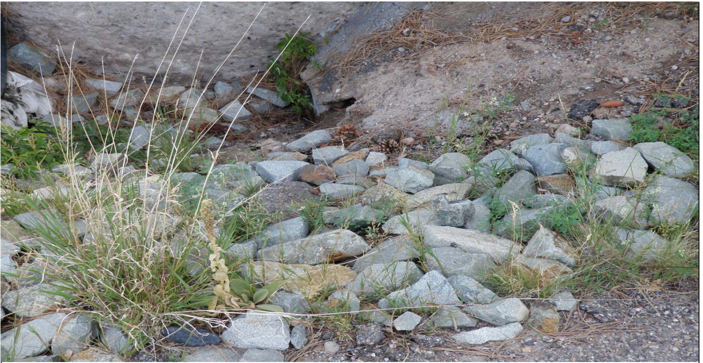
Photo 7482-3r.JPG (taken 08/10/10) C00604060009 : Channel/Swale - Rip Rap.
