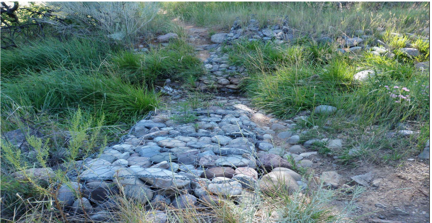
Photo 10552-5.JPG (taken 07/28/10) L00107010001 : Gabions - Gabions.
