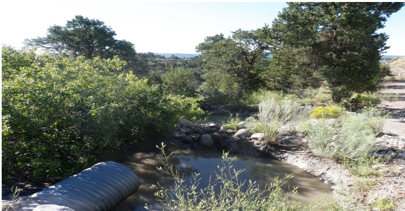
Photo 8507-4r.JPG (taken 08/20/10) J02402010003 : Established Vegetation - Permanent Vegetation Grasses and Shrubs; J02405010005 : Sediment Traps and Basins - Sediment Trap.
