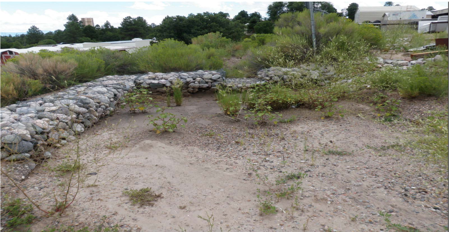
Photo 7451-6.JPG (taken 08/04/10) S00607010007 : Gabions - Gabions.
