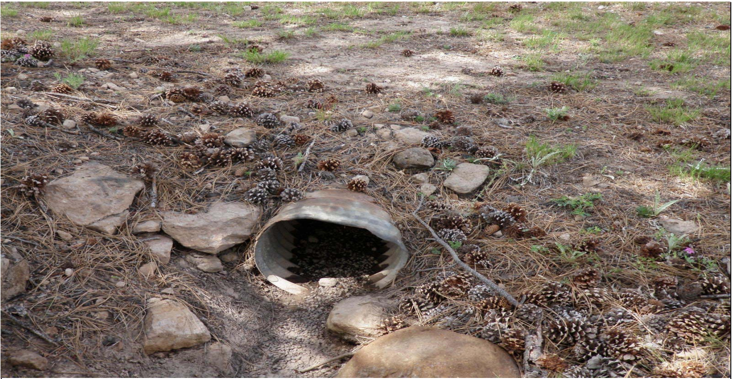
Photo 7508-2r.JPG (taken 08/12/10) J00804040003 : Channel/Swale - Culvert.
