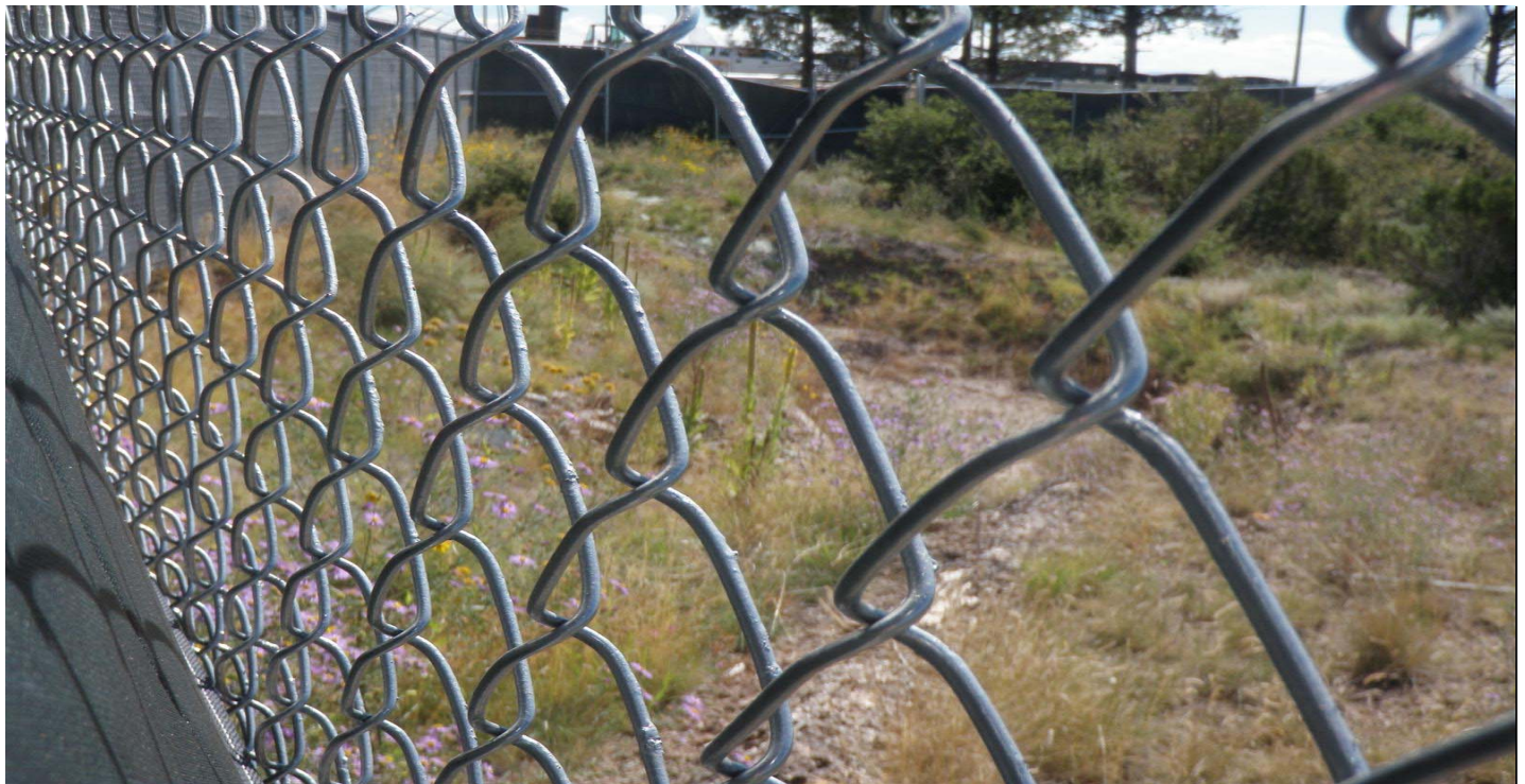
Photo 10547-1r.JPG (taken 09/20/10) L01905020001 : Sediment Traps and Basins - Sediment Basin.
