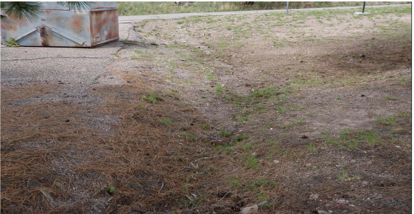
Photo 7508-3r.JPG (taken 08/12/10) J00804010002 : Channel/Swale - Earthen Channel/Swale.
