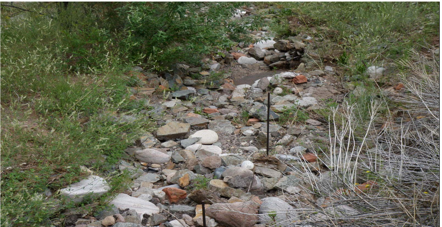
Photo 7451-12.JPG (taken 08/04/10) S00604060010 : Channel/Swale - Rip Rap.
