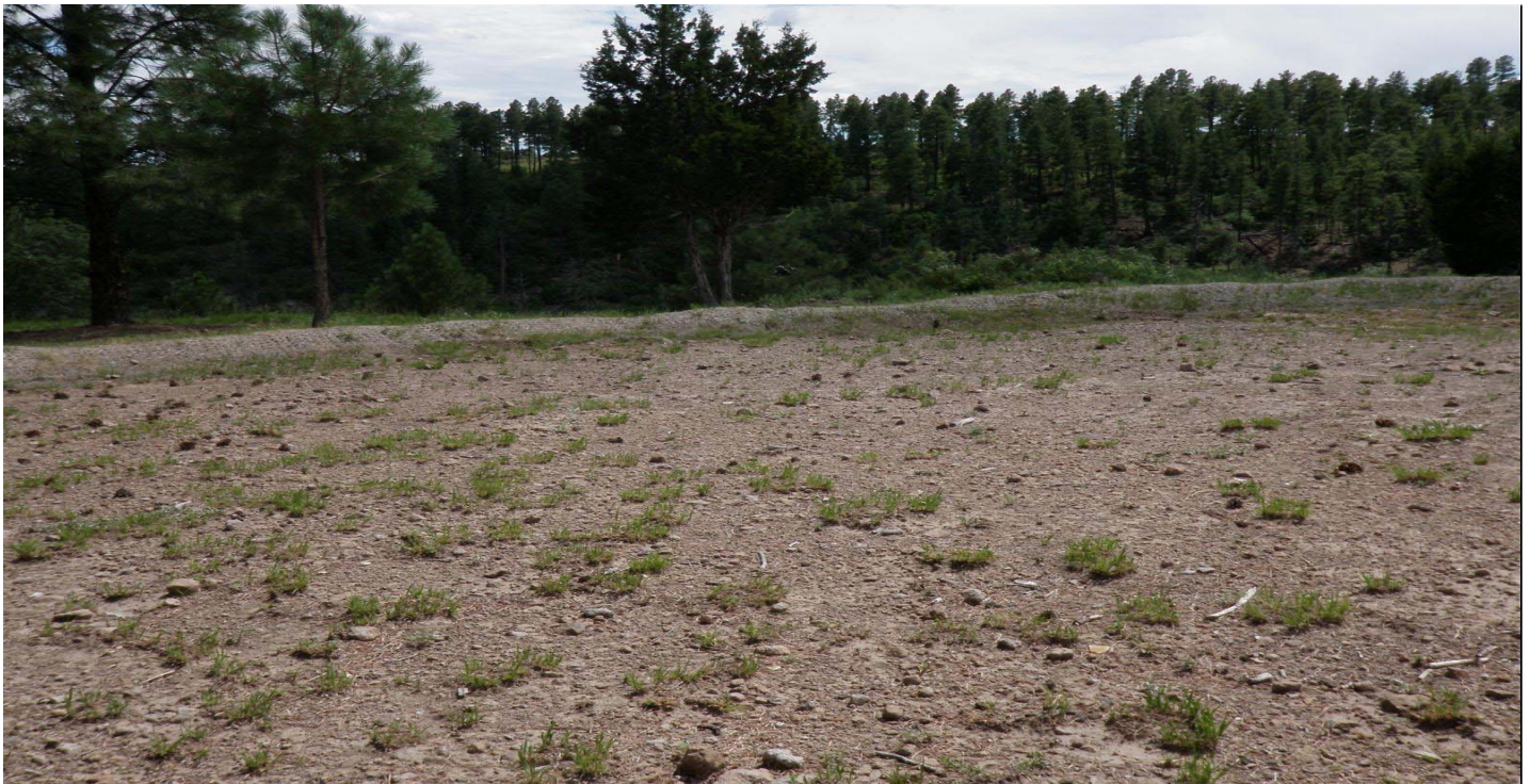
Photo 7508-1r.JPG (taken 08/12/10) J00801060005 : Seed and Mulch - Erosion Control Blanket; J00803010004 : Berms - Earthen Berm.
