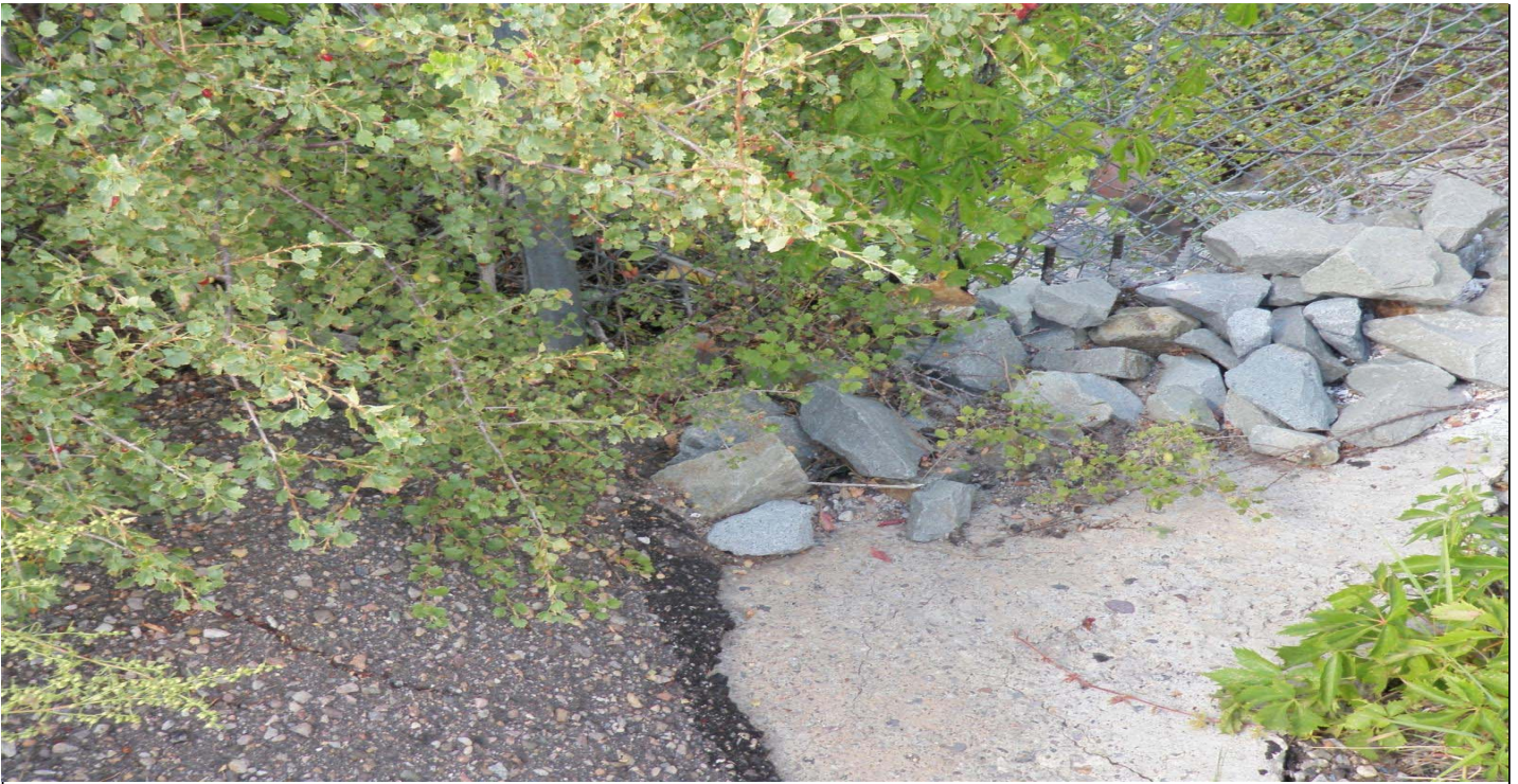
Photo 7483-2r.JPG (taken 08/10/10) C00504060008 : Channel/Swale - Rip Rap.
