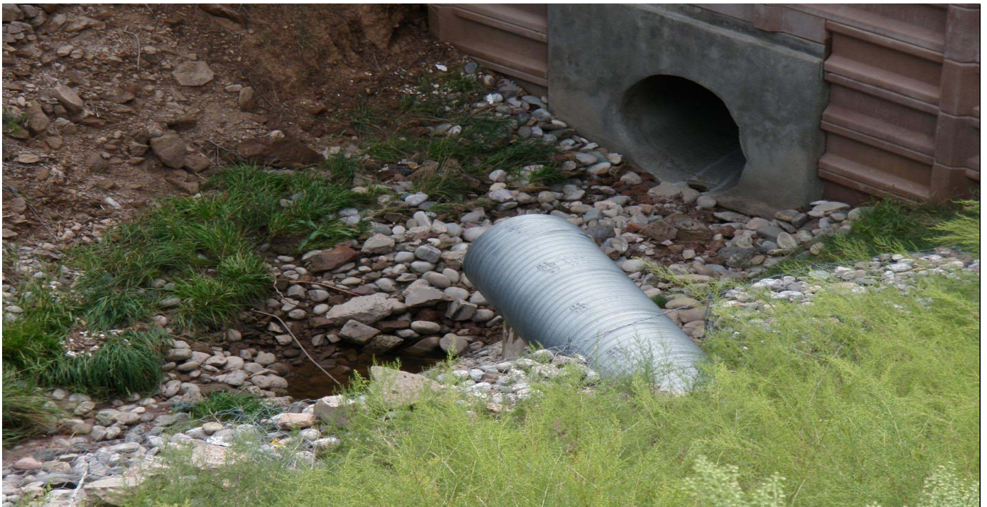
Photo 7493-1r.JPG (taken 08/09/10) M00107010001 : Gabions - Gabions.
