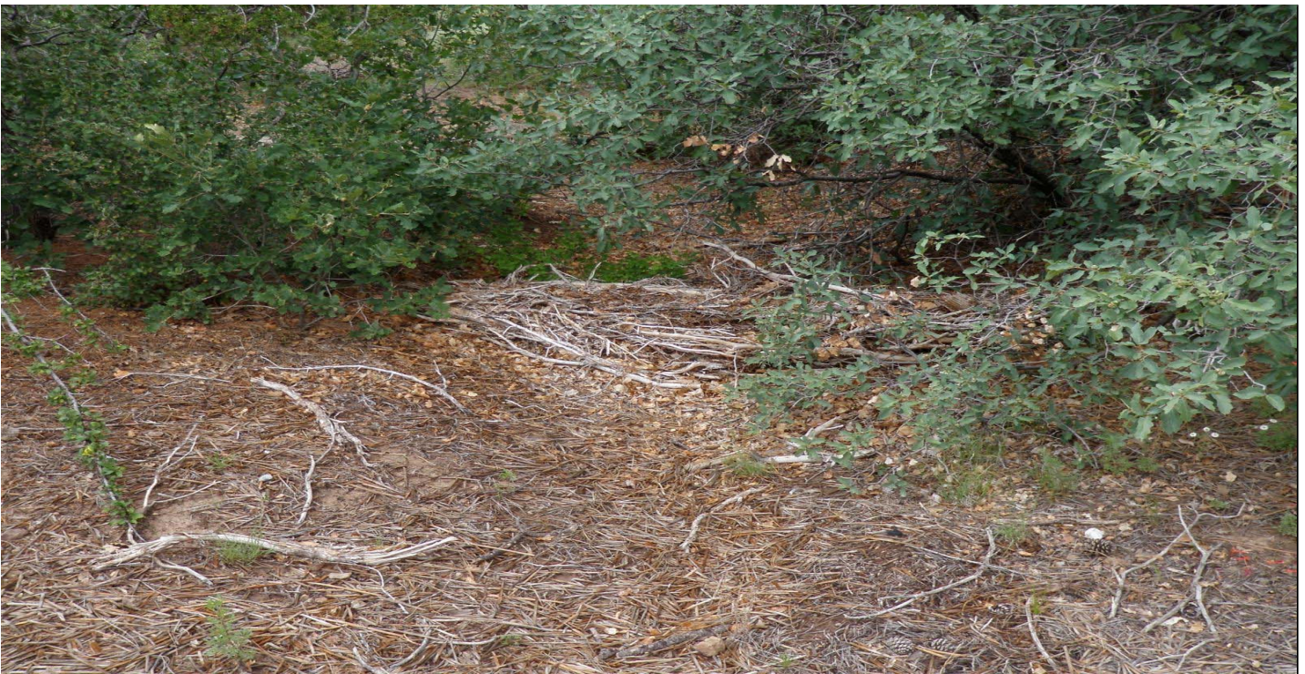
Photo 7485-4r.JPG (taken 08/10/10) C00106030007 : Check Dam - Juniper Bales.
