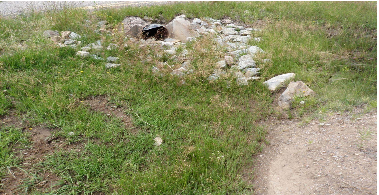
Photo 7497-5r.JPG (taken 08/11/10) J02804060006 : Channel/Swale - Rip Rap.
