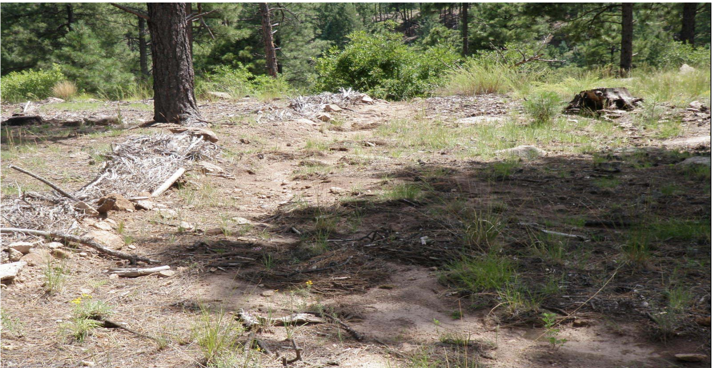
Photo 7506-4r.JPG (taken 08/11/10) J00504010003 : Channel/Swale - Earthen Channel/Swale; J00506030004 : Check Dam - Juniper Bales.
