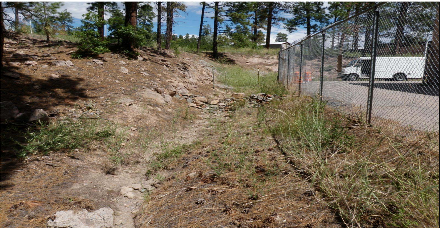
Photo 7516-4r.JPG (taken 08/12/10) E00106010009 : Check Dam - Rock Check Dam.
