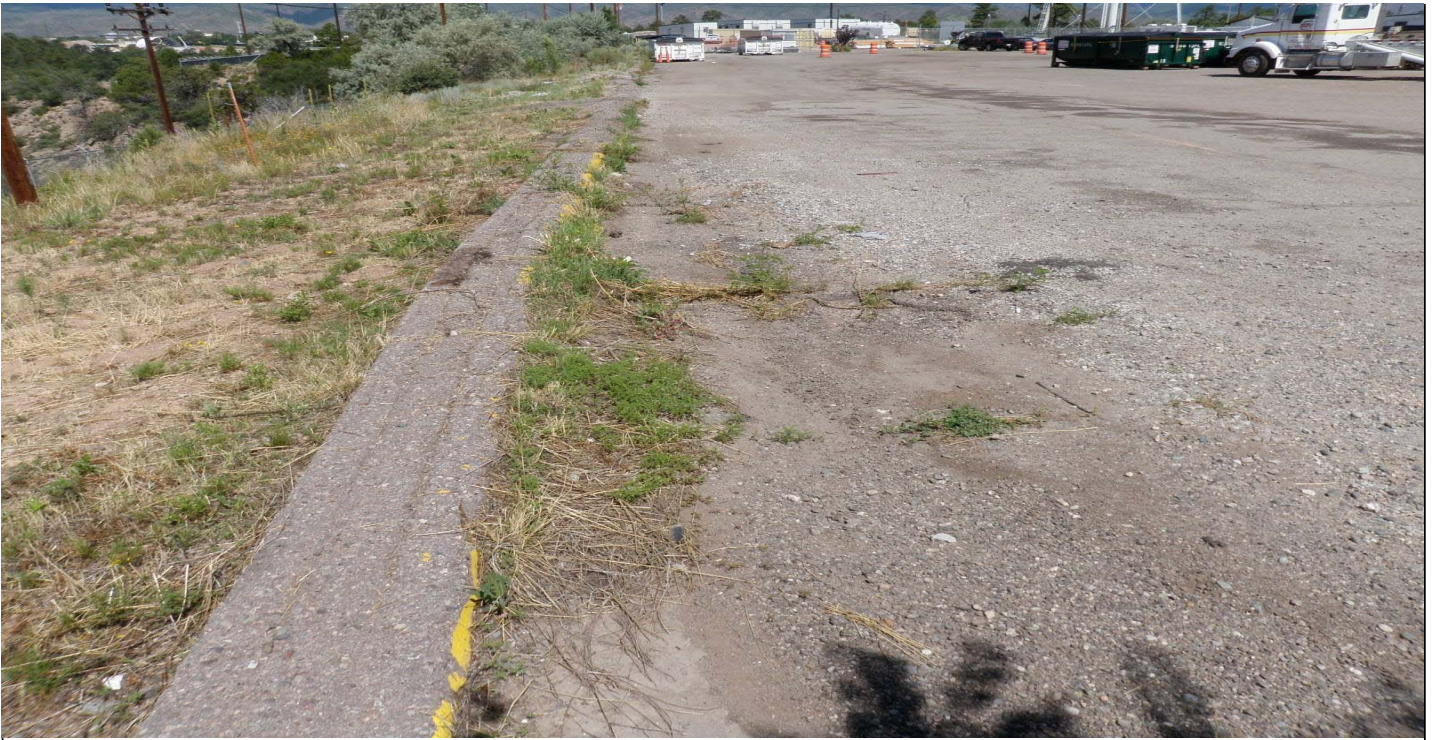
Photo 7430-2.JPG (taken 07/29/10) L02003040002 : Berms - Asphalt Berm.
