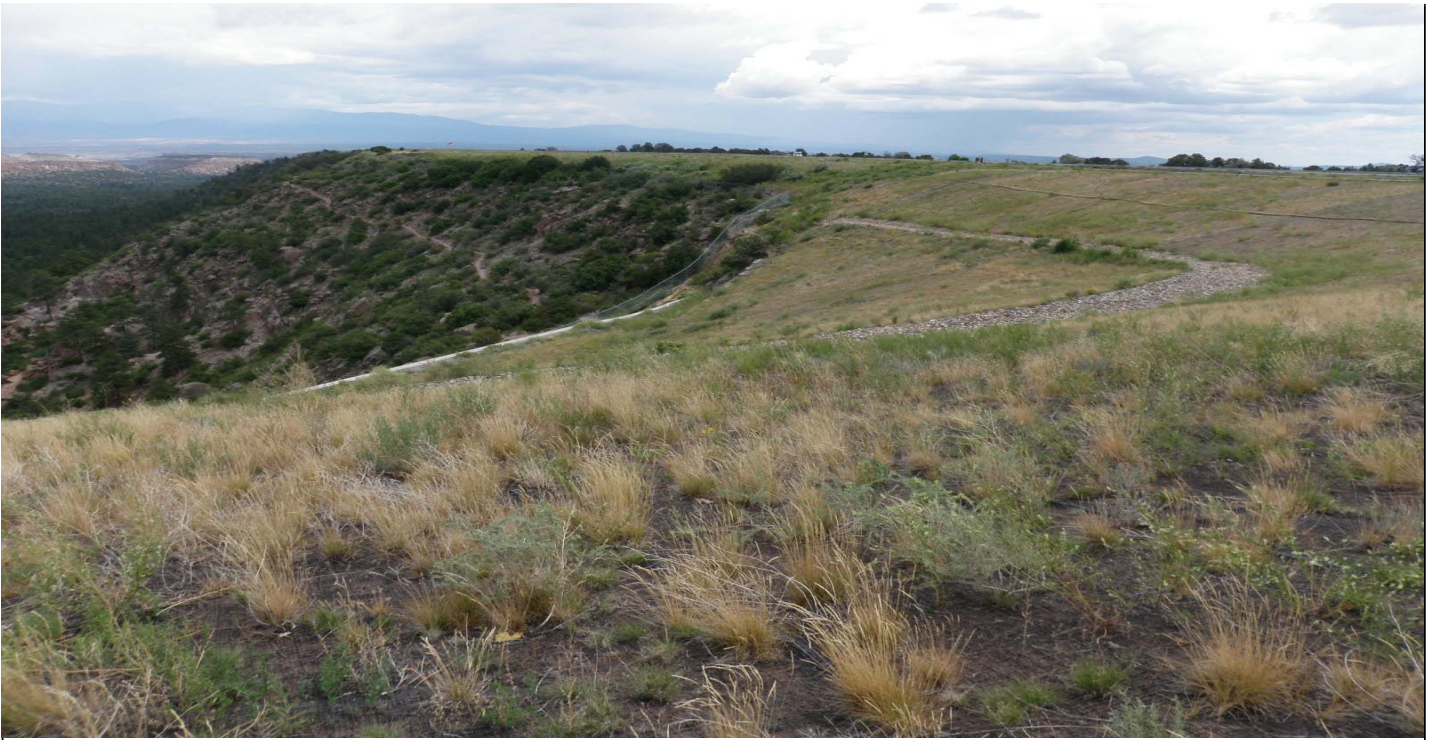
Photo 8653-11.JPG (taken 07/30/10) P00502010001 : Established Vegetation - Permanent Vegetation Grasses and Shrubs; P00503080003 : Berms - Retaining Wall; P00504060002 : Channel/Swale - Rip Rap.
