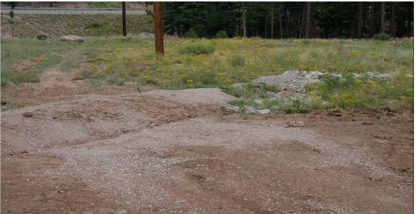
Photo 7501-4r.JPG (taken 08/11/10) J00104050009 : Channel/Swale - Water Bar.
