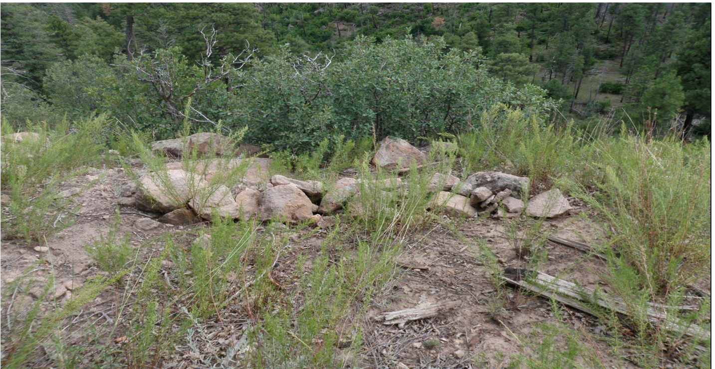
Photo 7509-4r.JPG (taken 08/12/10) J00706010006 : Check Dam - Rock Check Dam.
