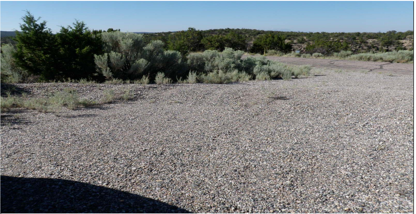
Photo 7356-1.JPG (taken 07/27/10) Q00803020006 : Berms - Base Course Berm.
