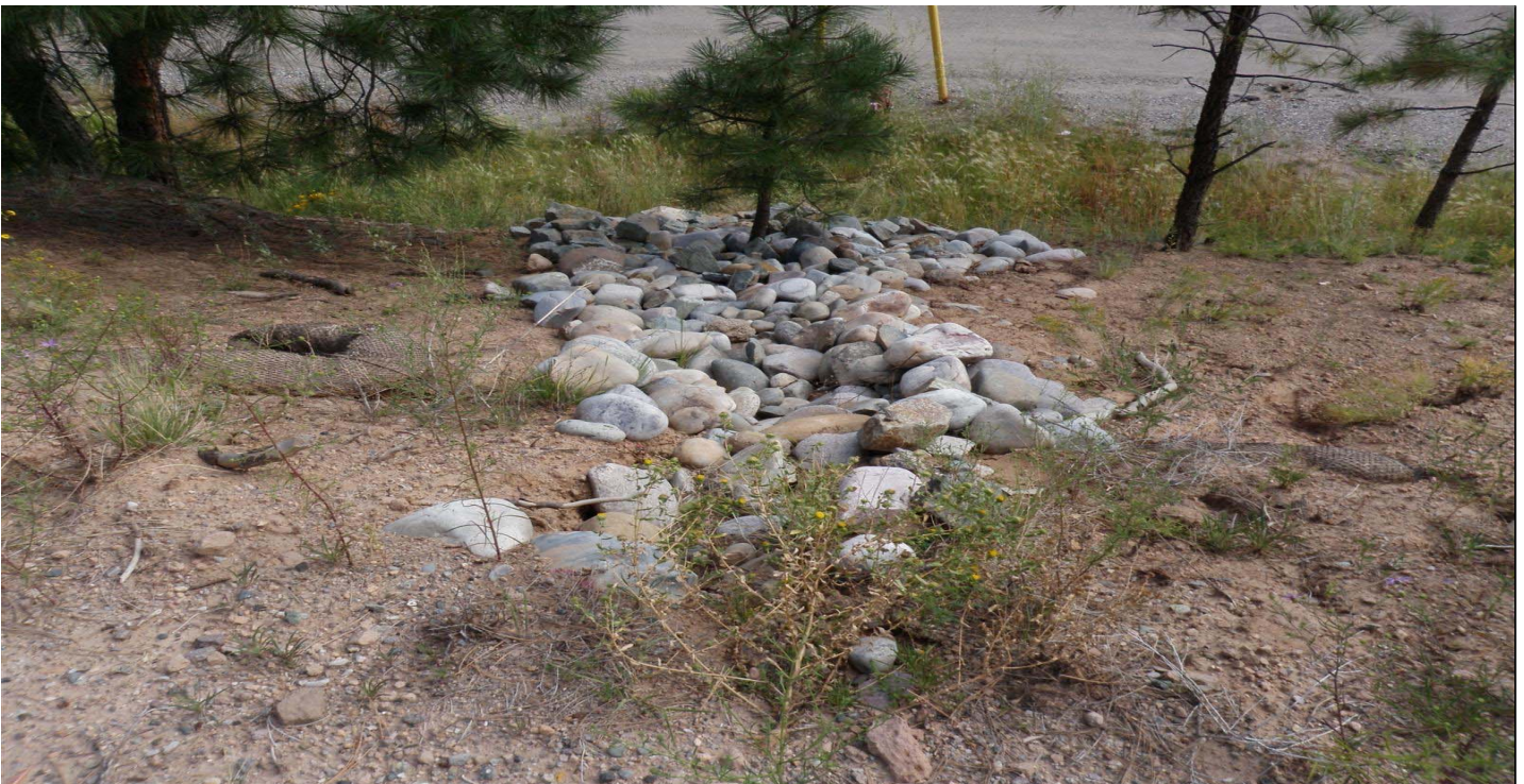
Photo 10554-2r.JPG (taken 09/09/10) E00104060011 : Channel/Swale - Rip Rap.
