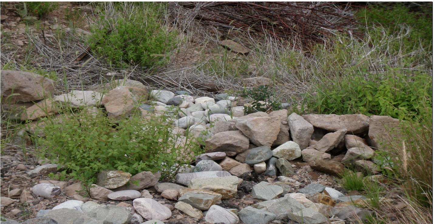
Photo 7511-4r.JPG (taken 08/12/10) J01006010006 : Check Dam - Rock Check Dam.
