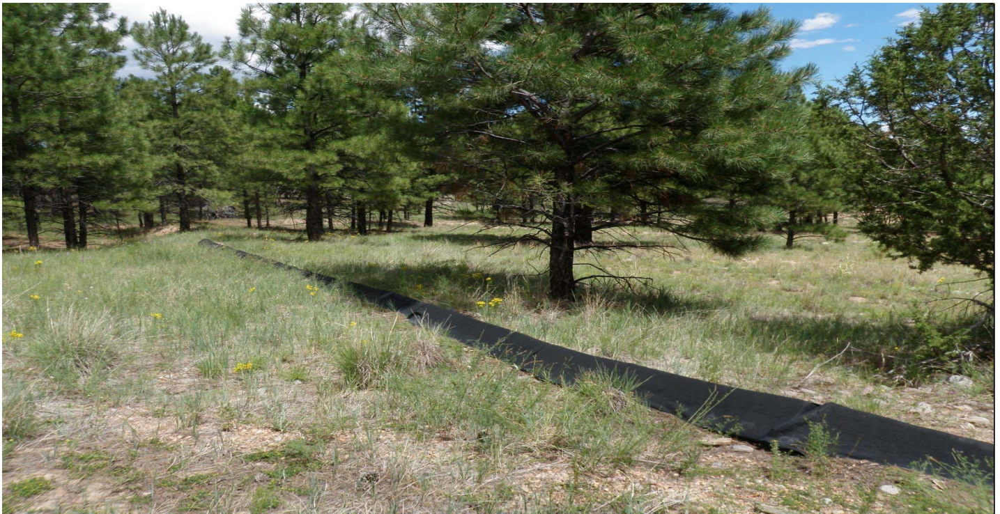
Photo 7500-1r.JPG (taken 08/11/10) J03103050006 : Berms - Silt Dike.
