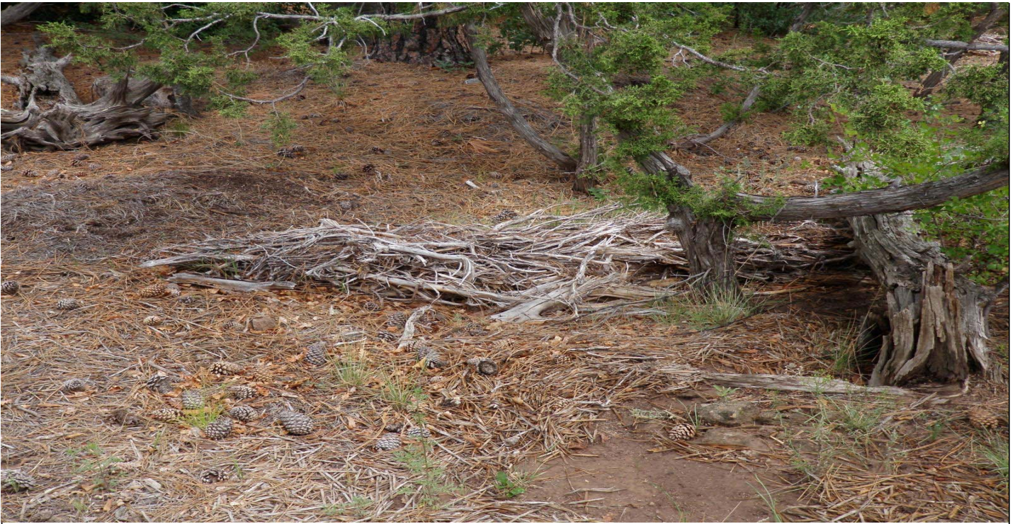
Photo 7485-3r.JPG (taken 08/10/10) C00106030004 : Check Dam - Juniper Bales.
