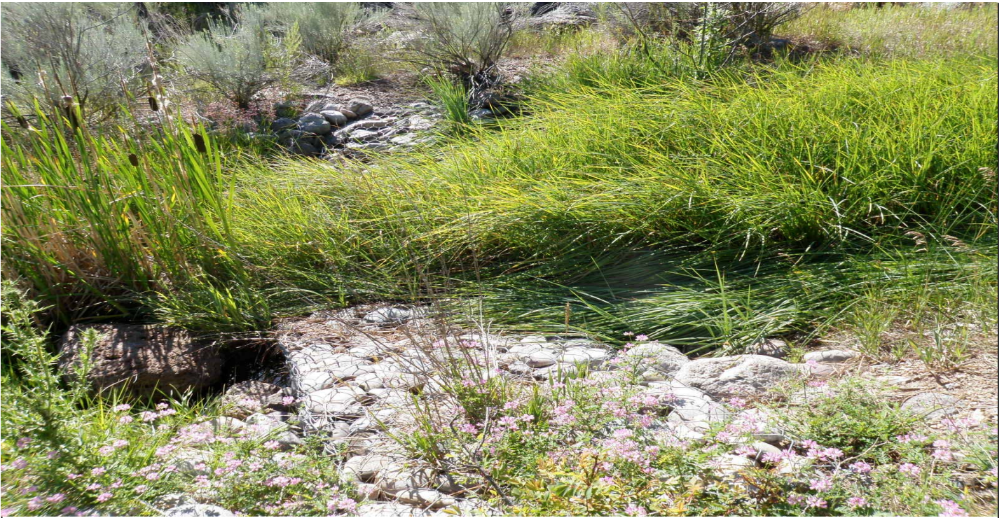
Photo 10552-4.JPG (taken 07/28/10) L00107010004 : Gabions - Gabions.
