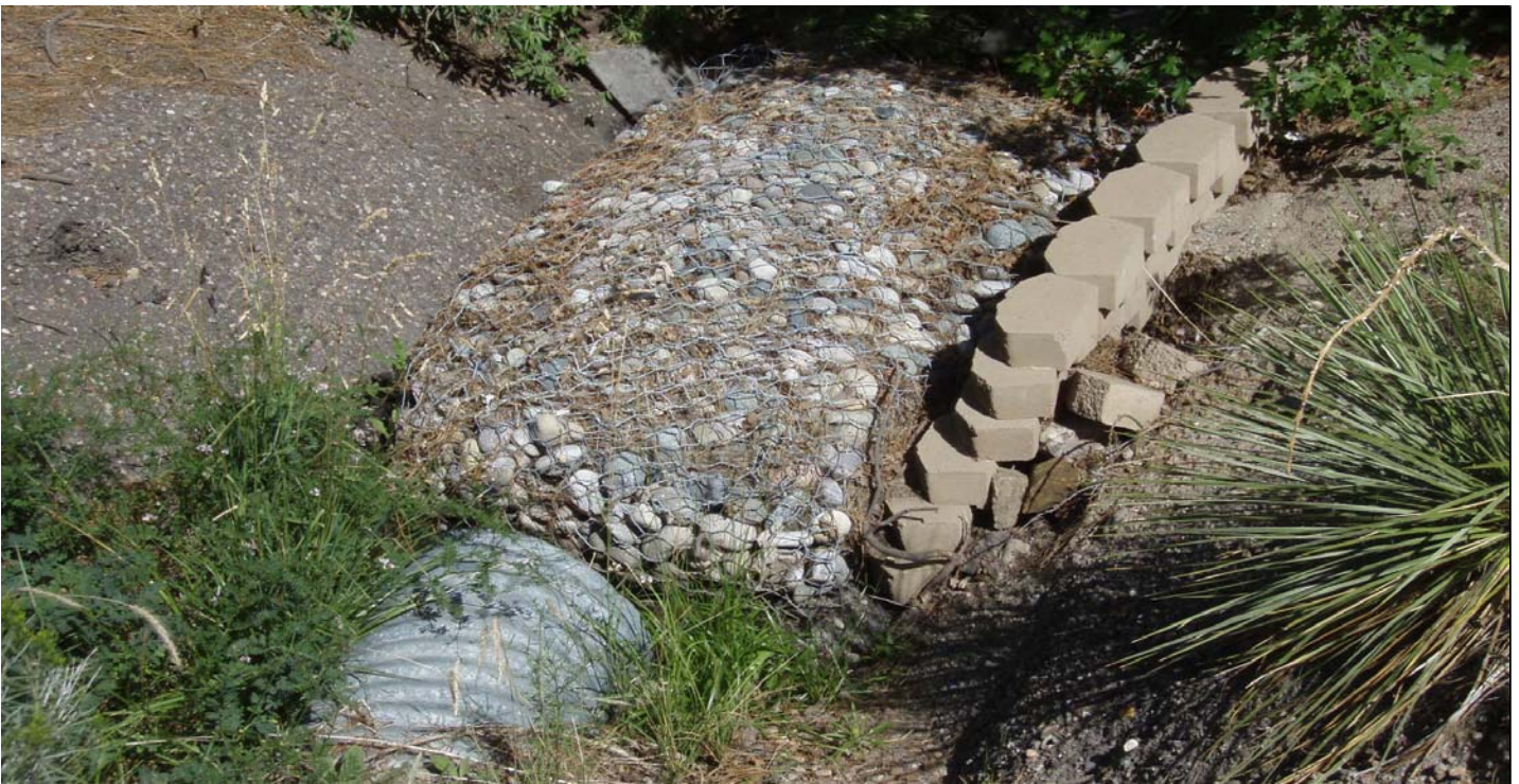
Photo 7599-2.JPG (taken 08/03/10) S00107010008 : Gabions - Gabions.
