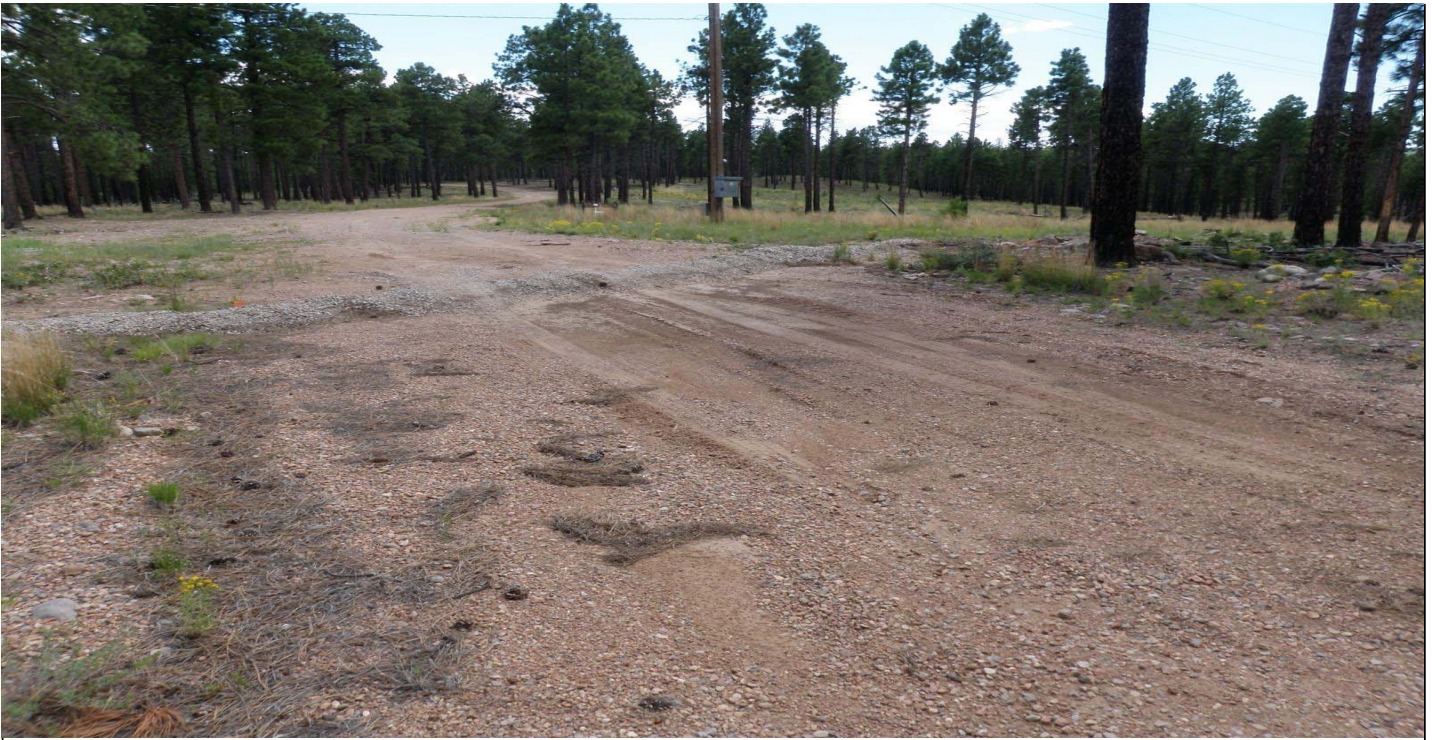
Photo 7501-1r.JPG (taken 08/11/10) J00104050008 : Channel/Swale - Water Bar.
