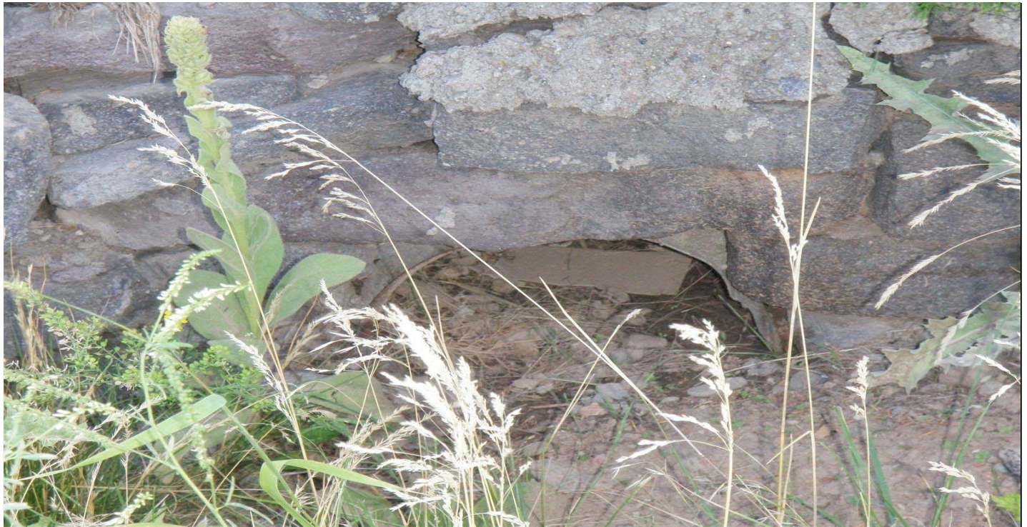
Photo 7505-1r.JPG (taken 08/11/10) E00604040002 : Channel/Swale - Culvert.
