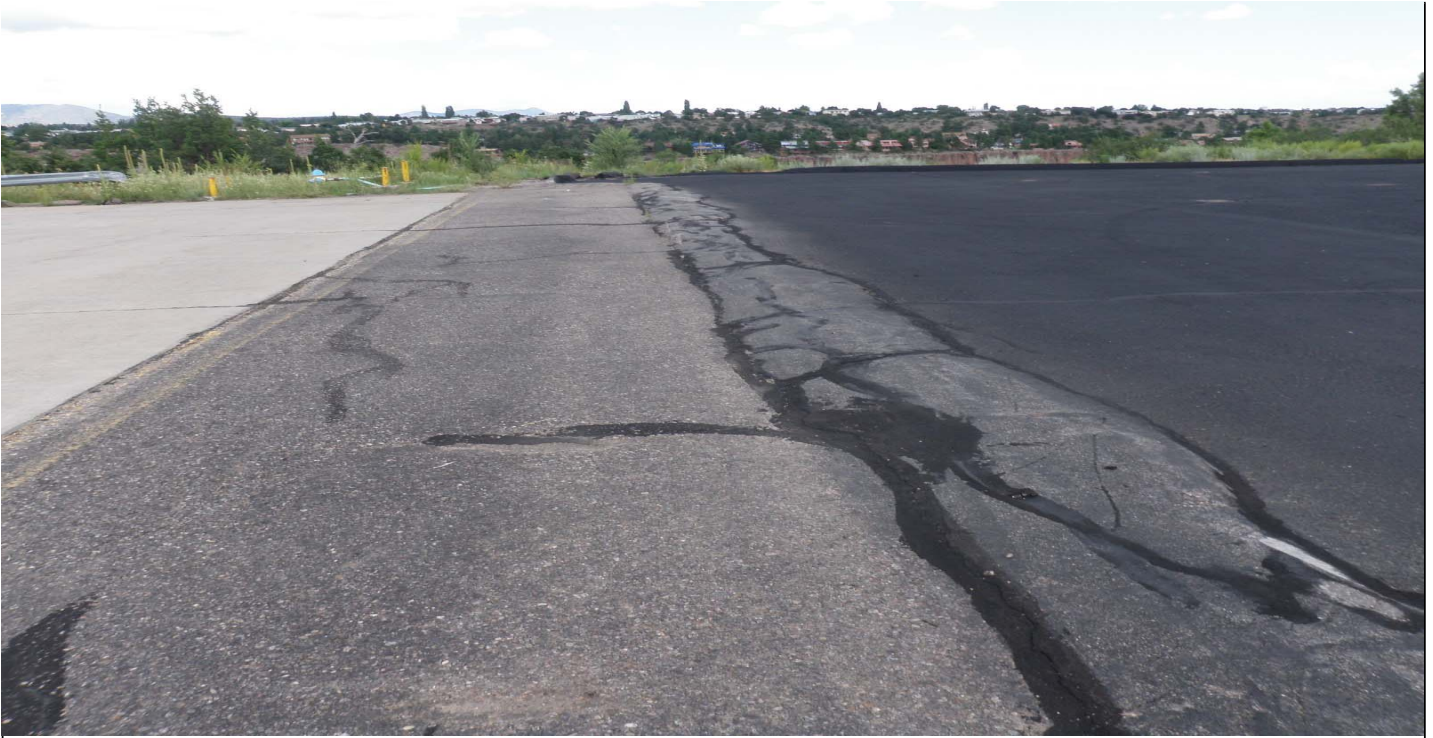
Photo 8653-1.JPG (taken 07/30/10) P00503040010 : Berms - Asphalt Berm.
