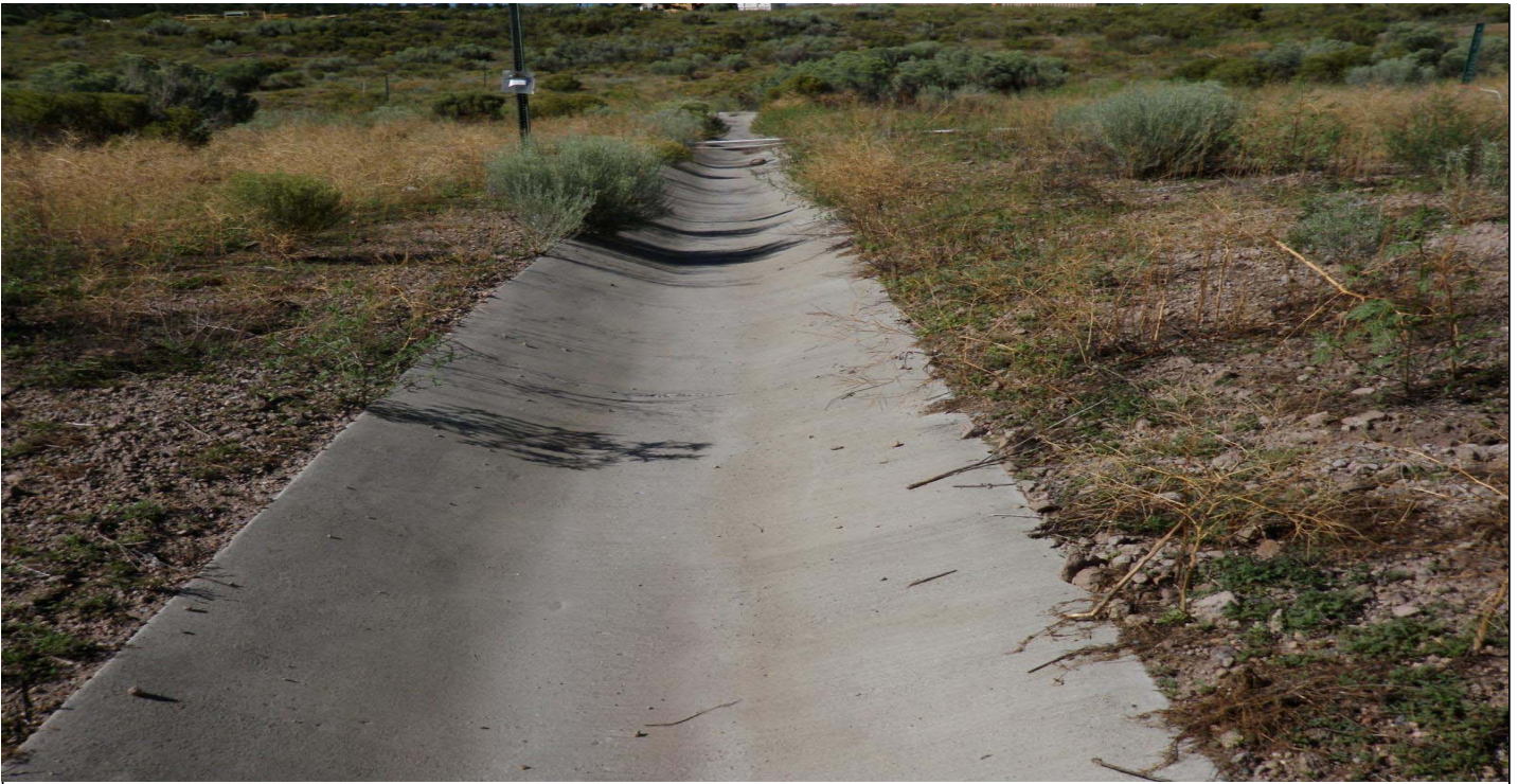
Photo 8505-3r.JPG (taken 08/20/10) J02504020004 : Channel/Swale - Concrete/Asphalt Channel/Swale.
