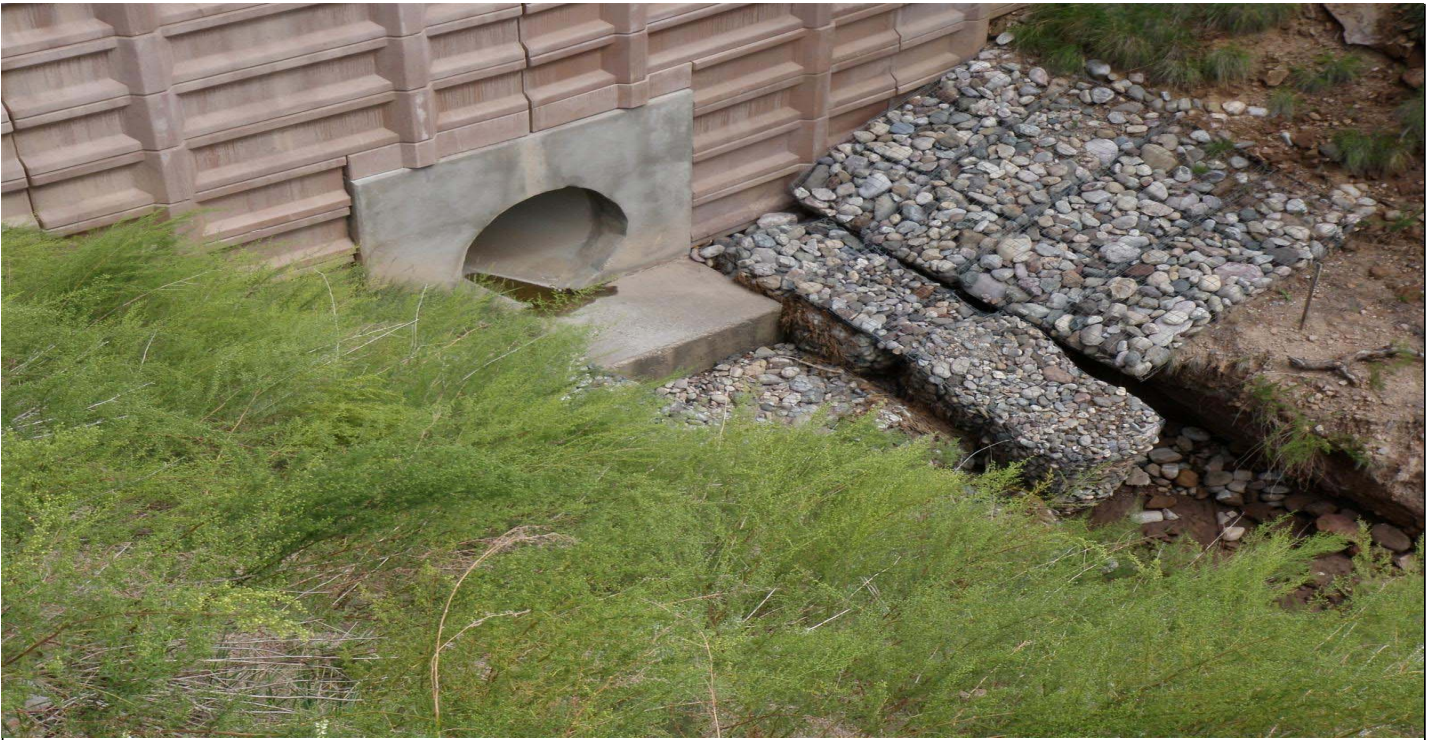
Photo 7493-2r.JPG (taken 08/09/10) M00107010006 : Gabions - Gabions.
