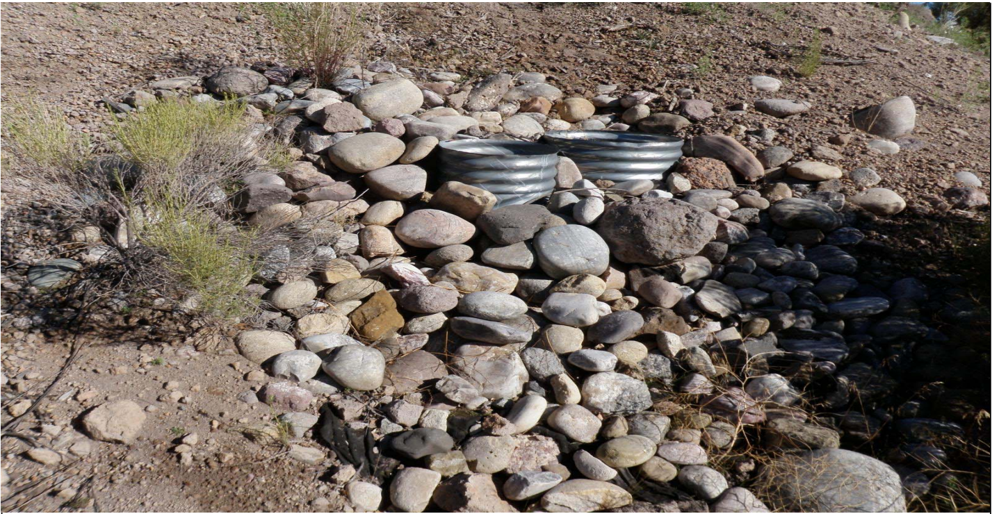
Photo 8507-2r.JPG (taken 08/20/10) J02404060006 : Channel/Swale - Rip Rap.
