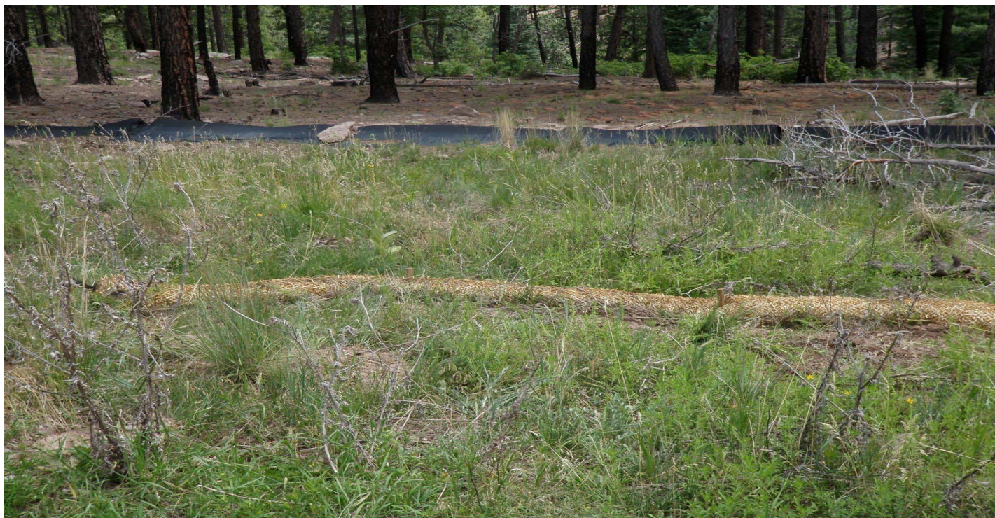
Photo 7500-4r.JPG (taken 08/11/10) J03103050005 : Berms - Silt Dike; J03103060007 : Berms - Straw Wattles.
