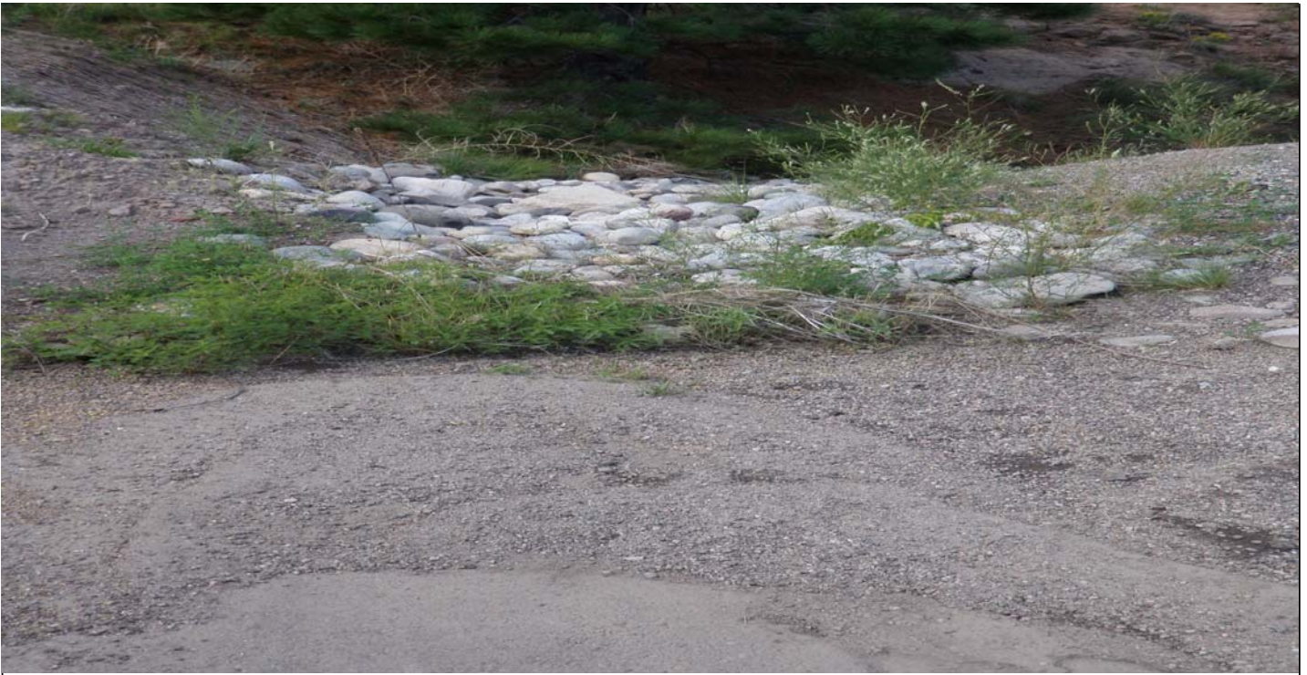
Photo 7484-5.JPG (taken 08/10/10) C00204060009 : Channel/Swale - Rip Rap.
