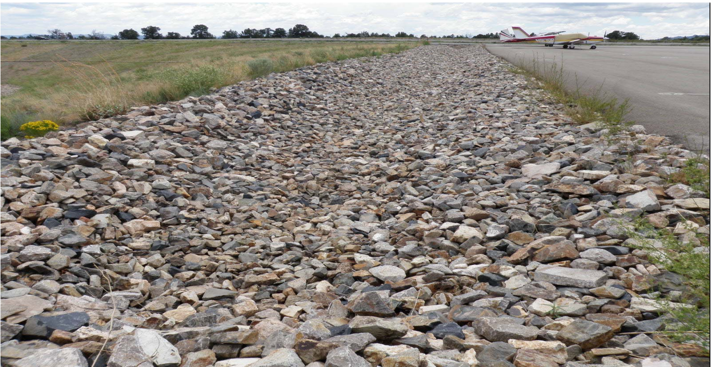
Photo 8653-10.JPG (taken 07/30/10) P00504060013 : Channel/Swale - Rip Rap.
