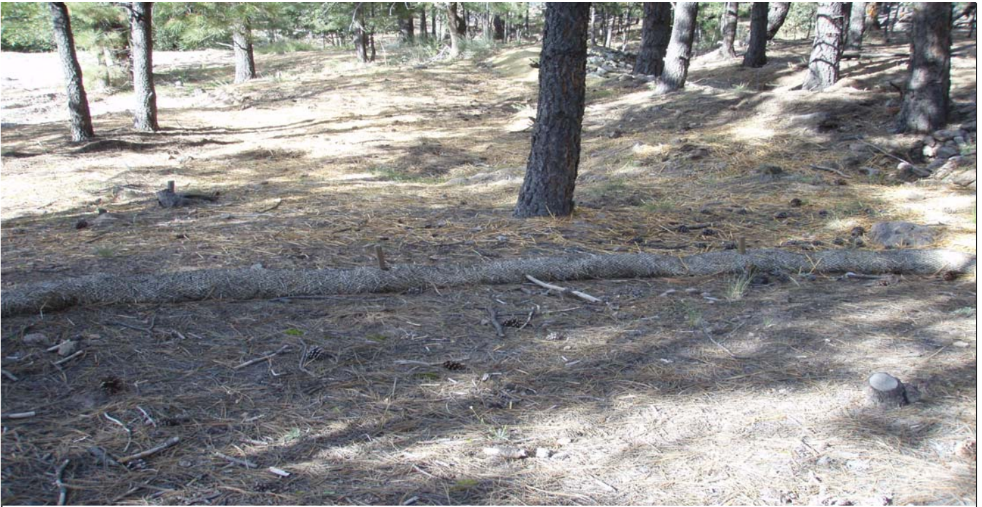
Photo 10870-3.JPG (taken 10/07/10) P00201010014 : Seed and Mulch - Seed and Wood Mulch; P00202020006 : Established Vegetation - Permanent Vegetation Forested/Needle Cast; P00203060010 : Berms - Straw Wattles.
