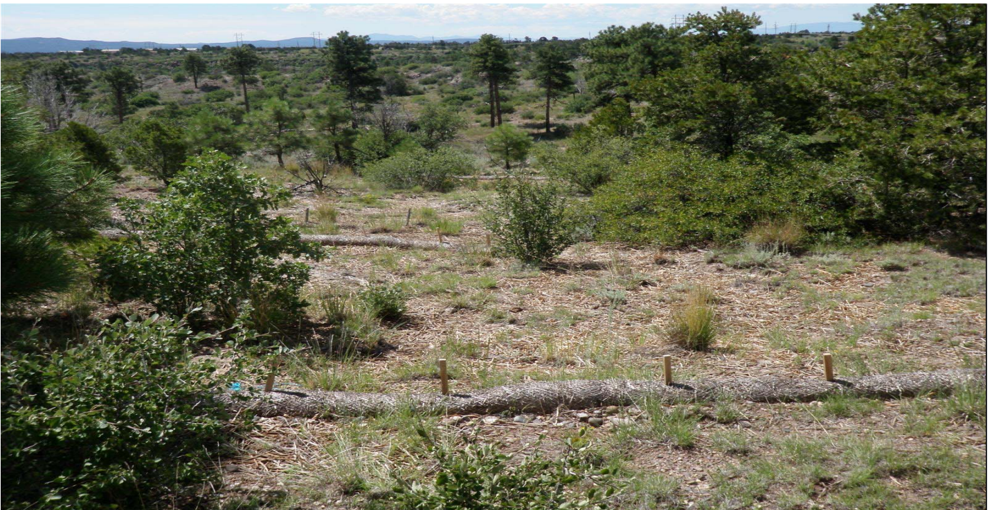
Photo 7486-2r.JPG (taken 08/10/10) M01601010006 : Seed and Mulch - Seed and Wood Mulch; M01602010001 : Established Vegetation - Permanent Vegetation Grasses and Shrubs; M01603060003 : Berms - Straw Wattles; M01603060004 : Berms - Straw Wattles; M01603060005 : Berms - Straw Wattles.
