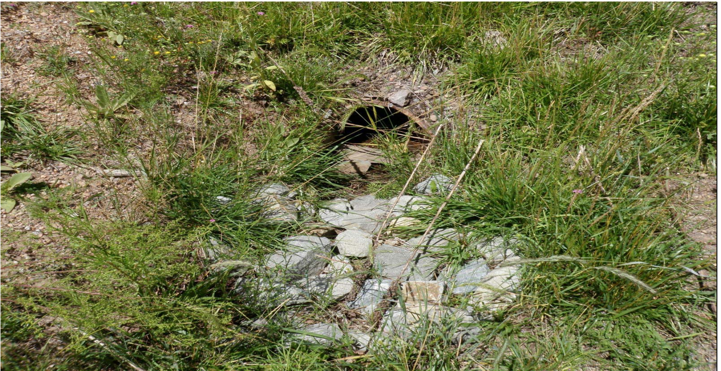
Photo 7594-2r.JPG (taken 08/13/10) W00104060011 : Channel/Swale - Rip Rap.
