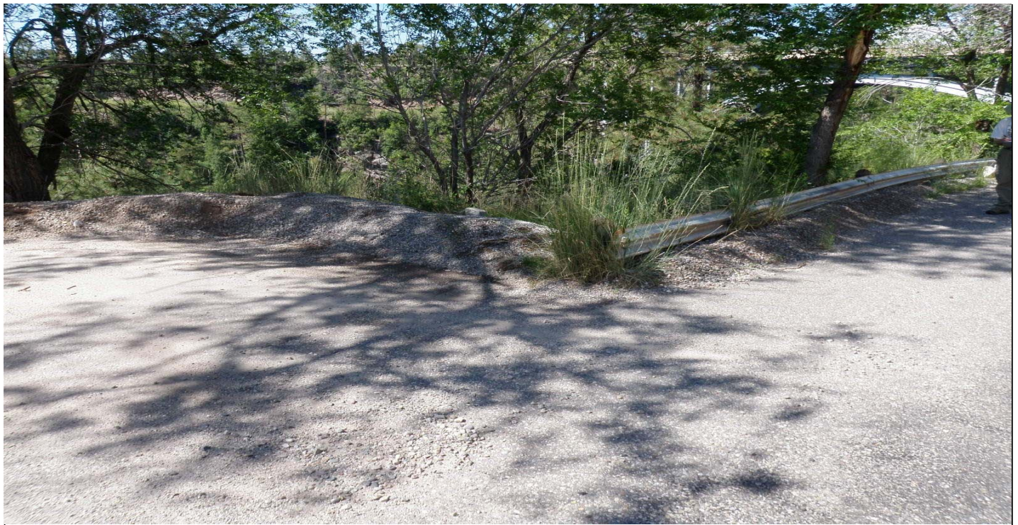
Photo 7420-1.JPG (taken 07/28/10) L00503020001 : Berms - Base Course Berm.
