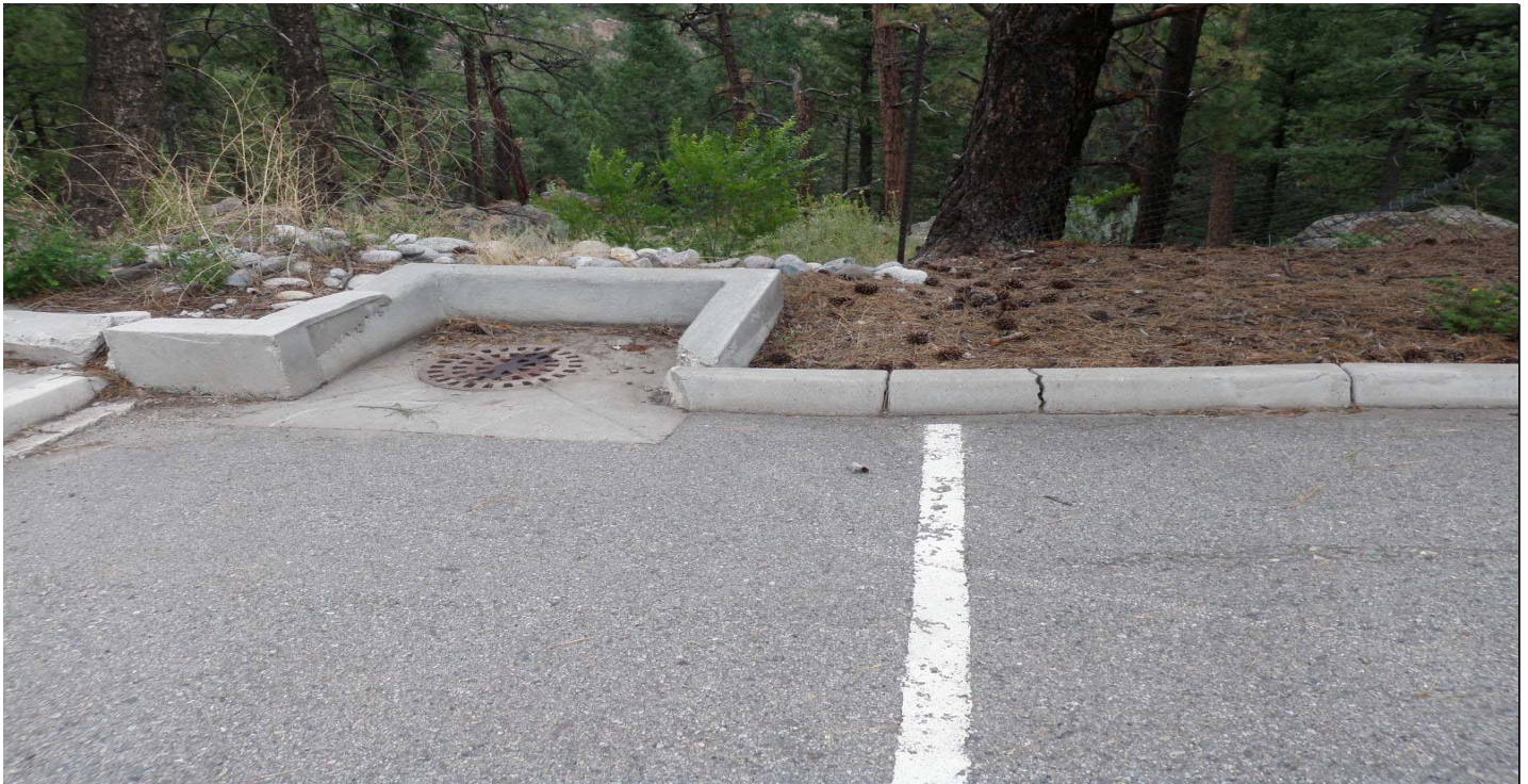
Photo 7409-1.JPG (taken 07/29/10) P00103090003 : Berms - Curbing; P00104040004 : Channel/Swale - Culvert.
