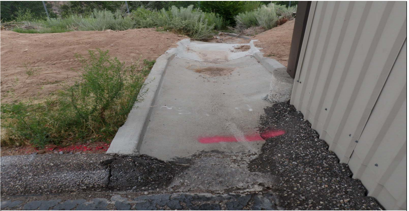
Photo 8653-3.JPG (taken 07/30/10) P00504020009 : Channel/Swale - Concrete/Asphalt Channel/Swale.
