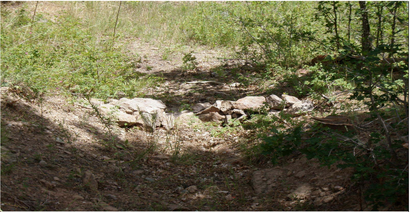
Photo 7502-2r.JPG (taken 08/11/10) J00406010006 : Check Dam - Rock Check Dam.
