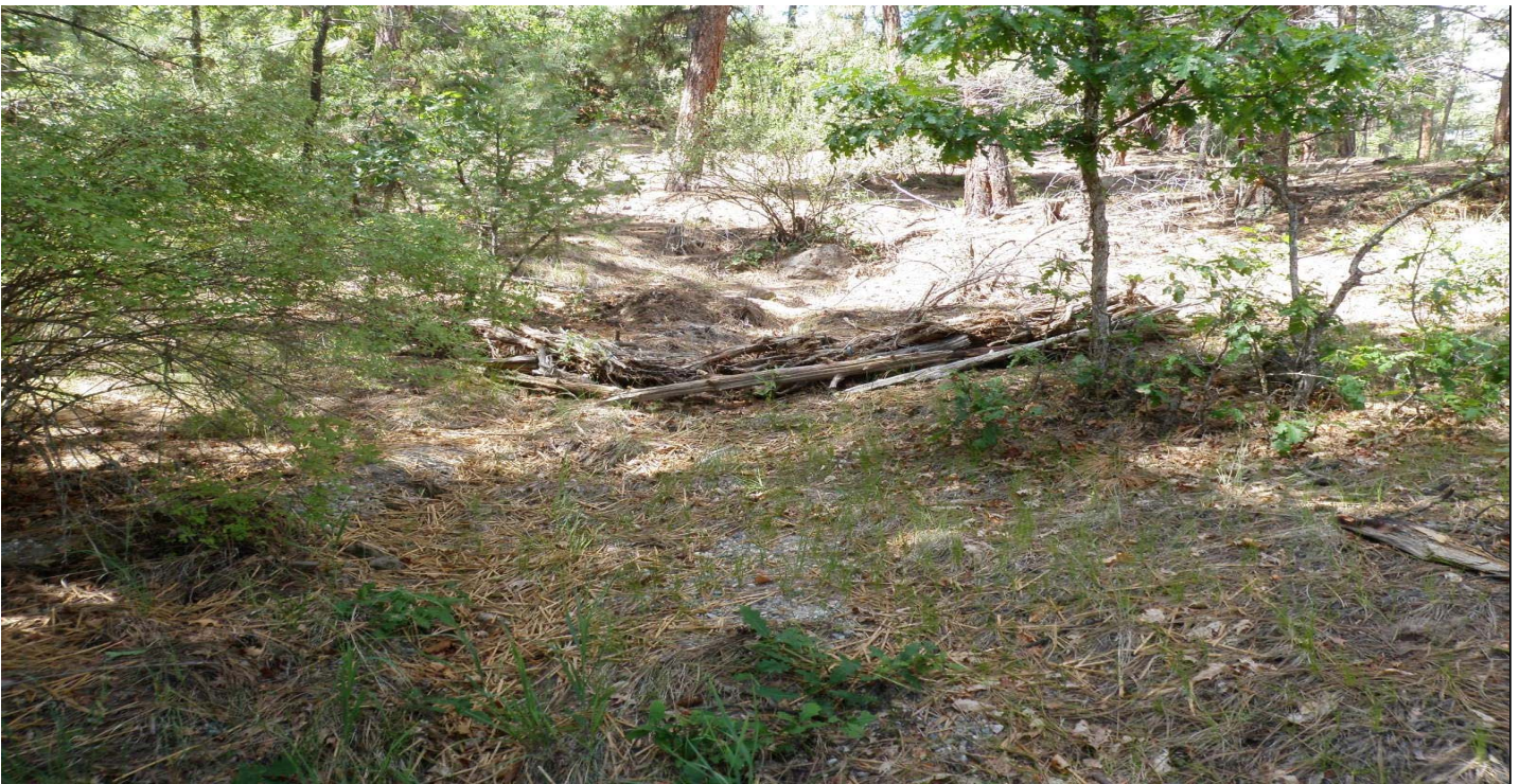
Photo 7414-2.JPG (taken 07/29/10) D00506030009 : Check Dam - Juniper Bales.
