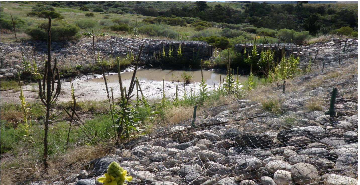
Photo 8505-2r.JPG (taken 08/20/10) J02507010001 : Gabions - Gabions.
