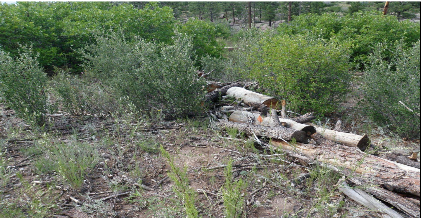
Photo 7481-2r.JPG (taken 08/10/10) C00706020018 : Check Dam - Log Check Dam.
