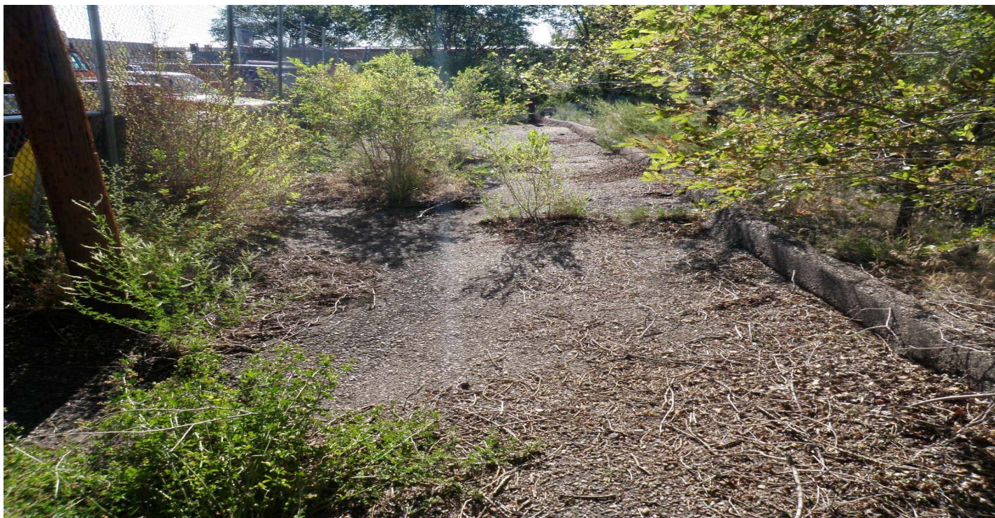
Photo 7427-4.JPG (taken 07/28/10) L01404020001 : Channel/Swale - Concrete/Asphalt Channel/Swale.
