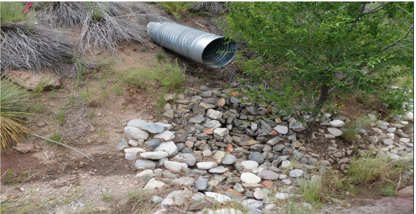
Photo 7451-9.JPG (taken 08/04/10) S00604060002 : Channel/Swale - Rip Rap.
