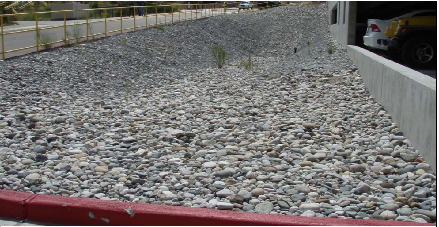
Photo 7599-1.JPG (taken 08/03/10) S00104060007 : Channel/Swale - Rip Rap.
