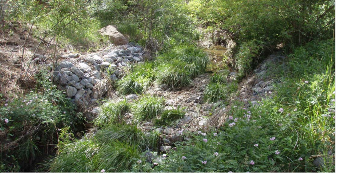
Photo 7599-5.JPG (taken 08/03/10) S00107020003 : Gabions - Gabion Blanket.
