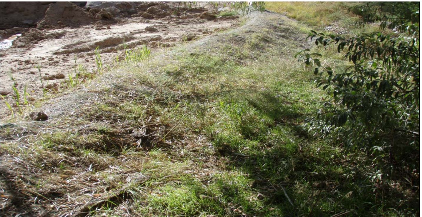
Photo 10871-6.JPG (taken 10/07/10) P00302010001 : Established Vegetation - Permanent Vegetation Grasses and Shrubs; P00303010002 : Berms - Earthen Berm.
