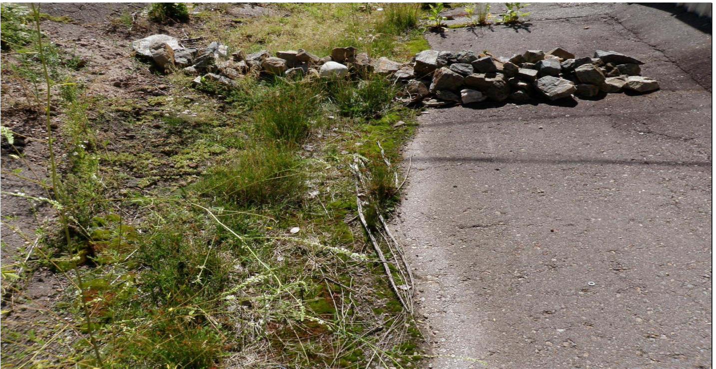
Photo 7526-3r.JPG (taken 08/12/10) J02106010004 : Check Dam - Rock Check Dam.
