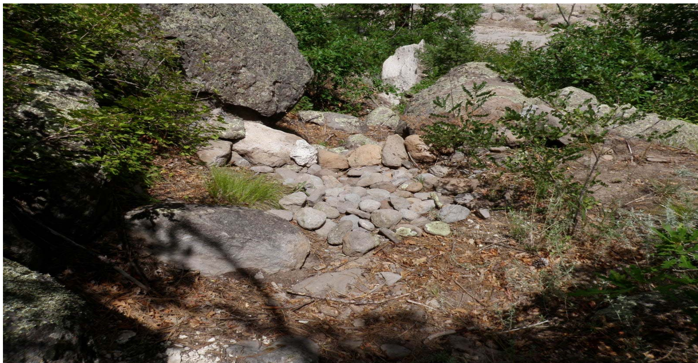
Photo 7460-1.JPG (taken 07/30/10) P00704060006 : Channel/Swale - Rip Rap; P00706010005 : Check Dam - Rock Check Dam.
