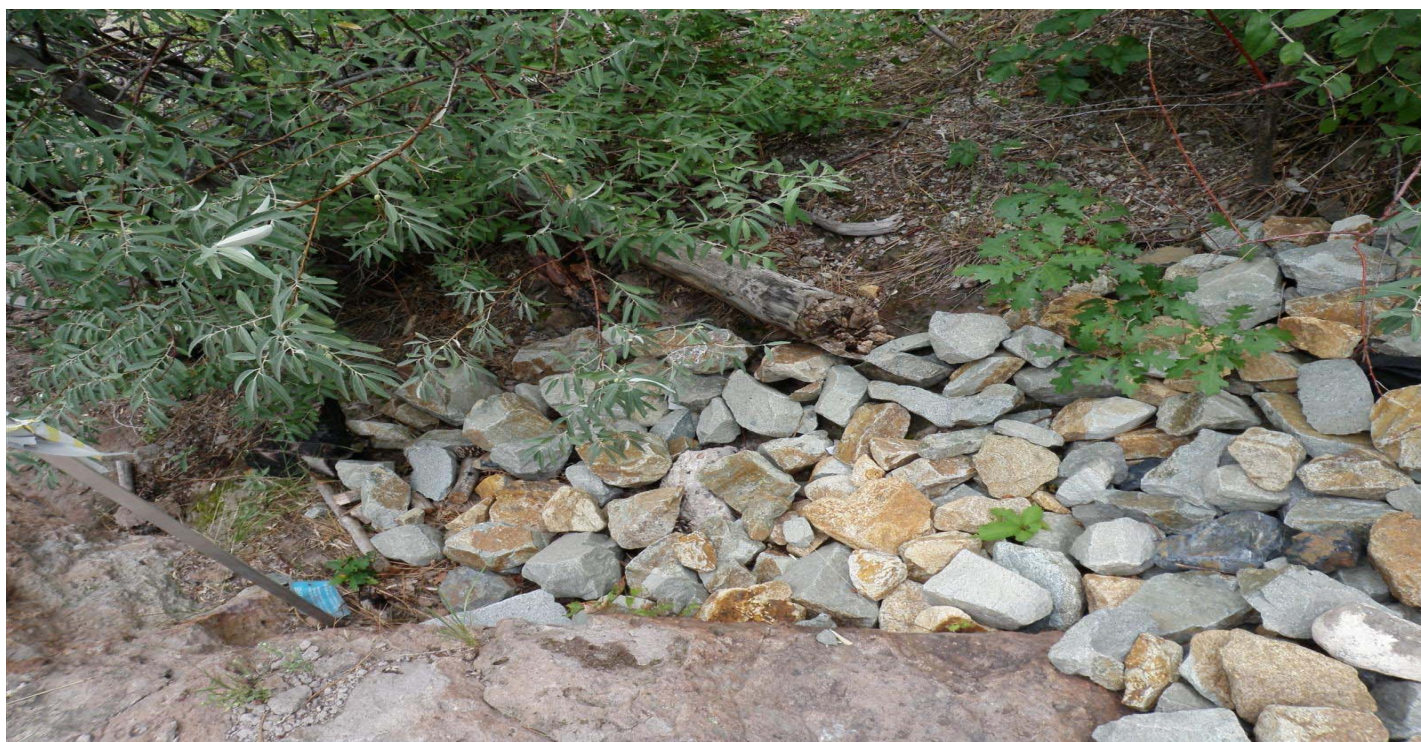
Photo 7488-1r.JPG (taken 08/09/10) M00404060005 : Channel/Swale - Rip Rap.
