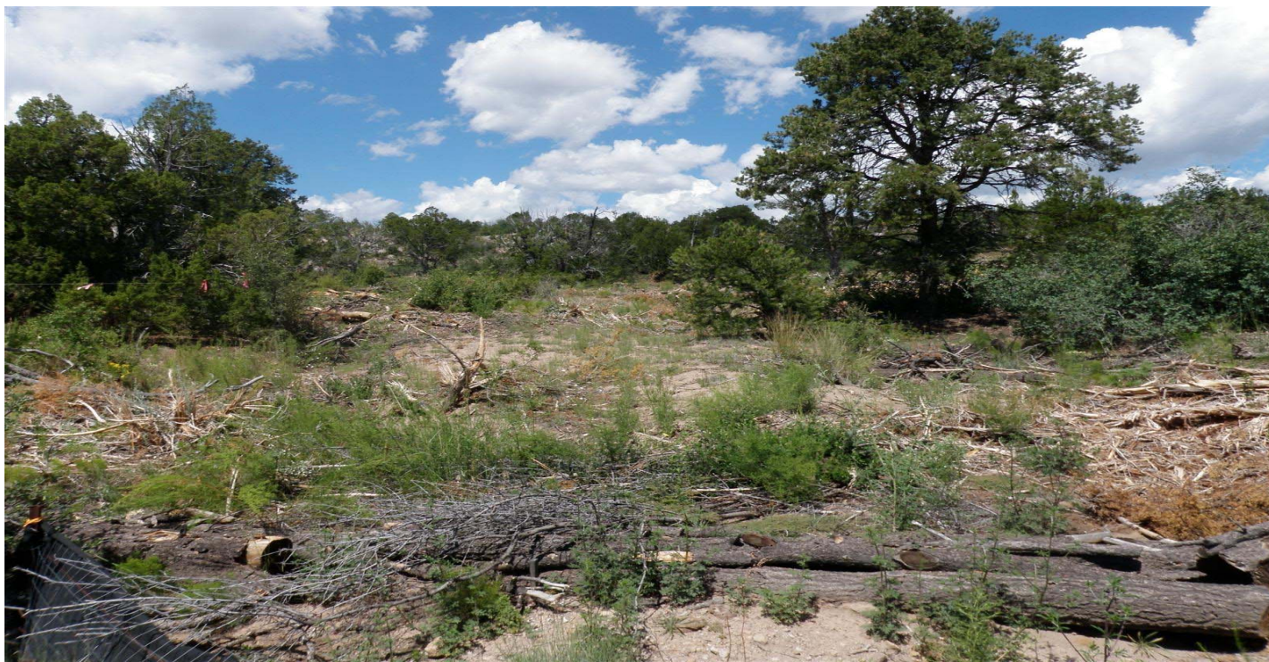
Photo 7476-7r.JPG (taken 08/10/10) M02206020003 : Check Dam - Log Check Dam.
