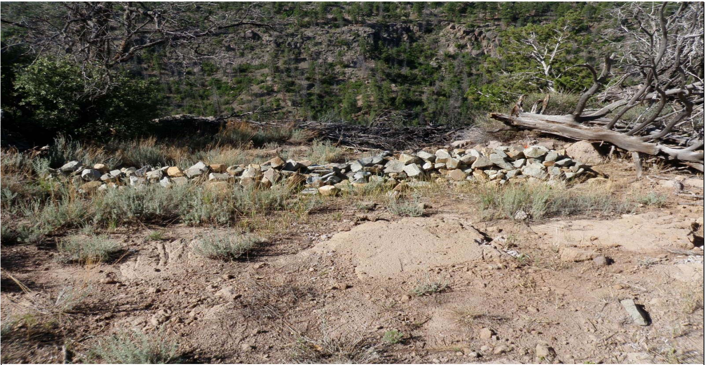
Photo 7437-2.JPG (taken 07/29/10) L02806010002 : Check Dam - Rock Check Dam.
