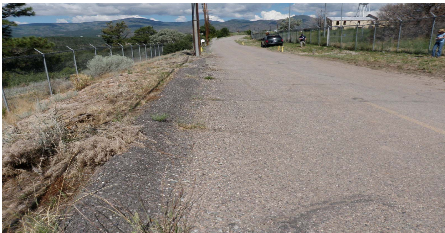
Photo 7432-1.JPG (taken 07/29/10) L02303040002 : Berms - Asphalt Berm.
