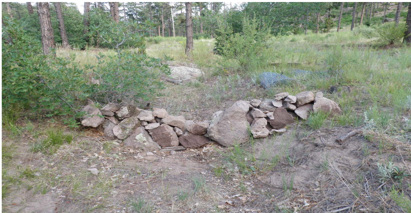
Photo 7412-1.JPG (taken 07/29/10) B00202010001 : Established Vegetation - Permanent Vegetation Grasses and Shrubs; B00206010005 : Check Dam - Rock Check Dam.
