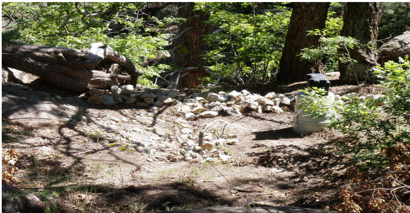
Photo 8510-2r.JPG (taken 08/20/10) M00206010004 : Check Dam - Rock Check Dam.
