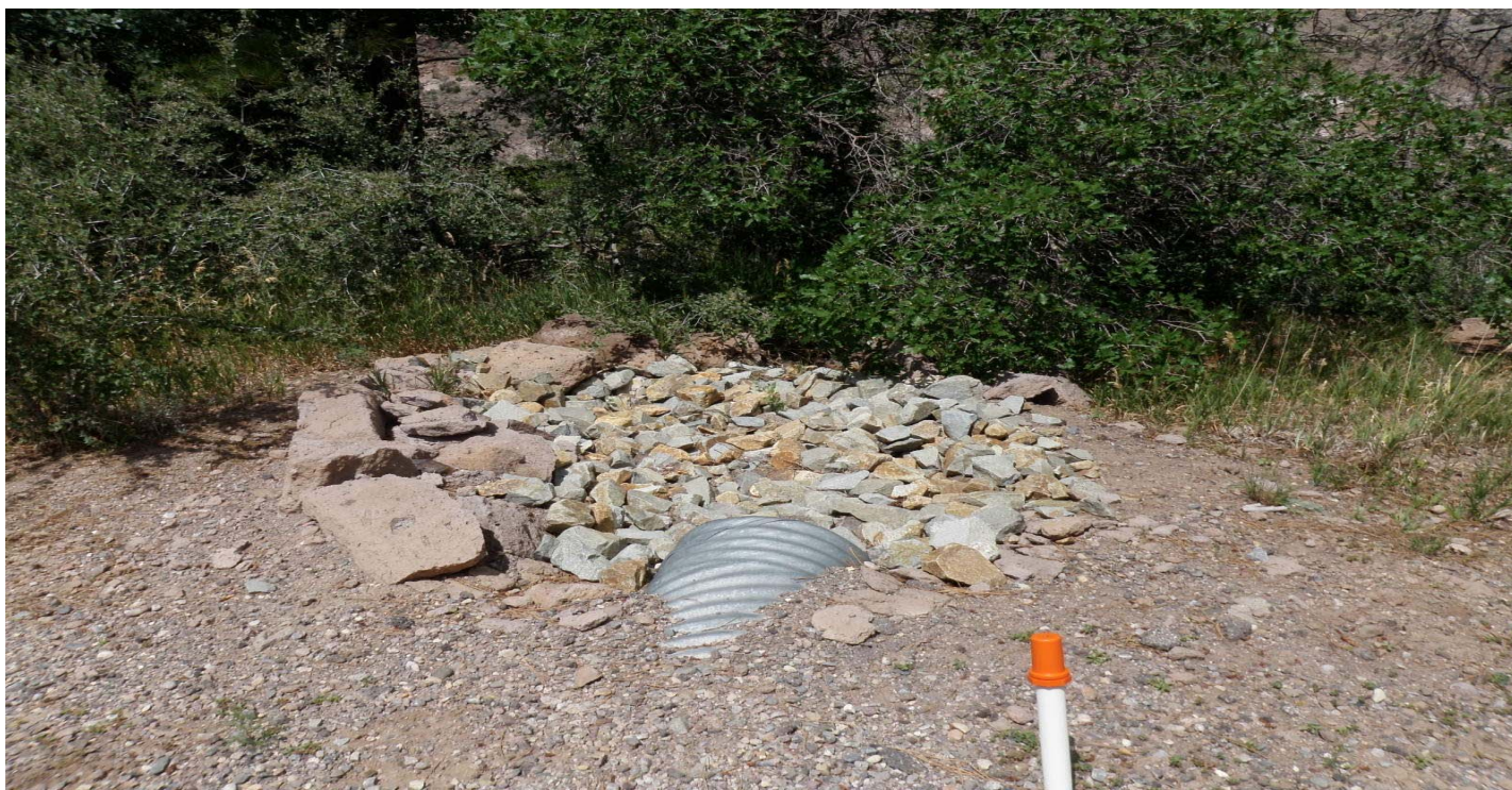
Photo 7460-3.JPG (taken 07/30/10) P00704060003 : Channel/Swale - Rip Rap.
