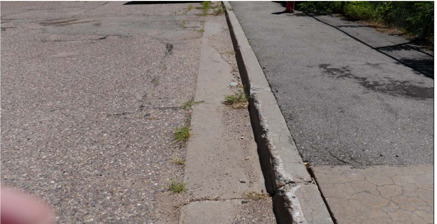
Photo 7469-3.JPG (taken 08/06/10) T00403090004 : Berms - Curbing.
