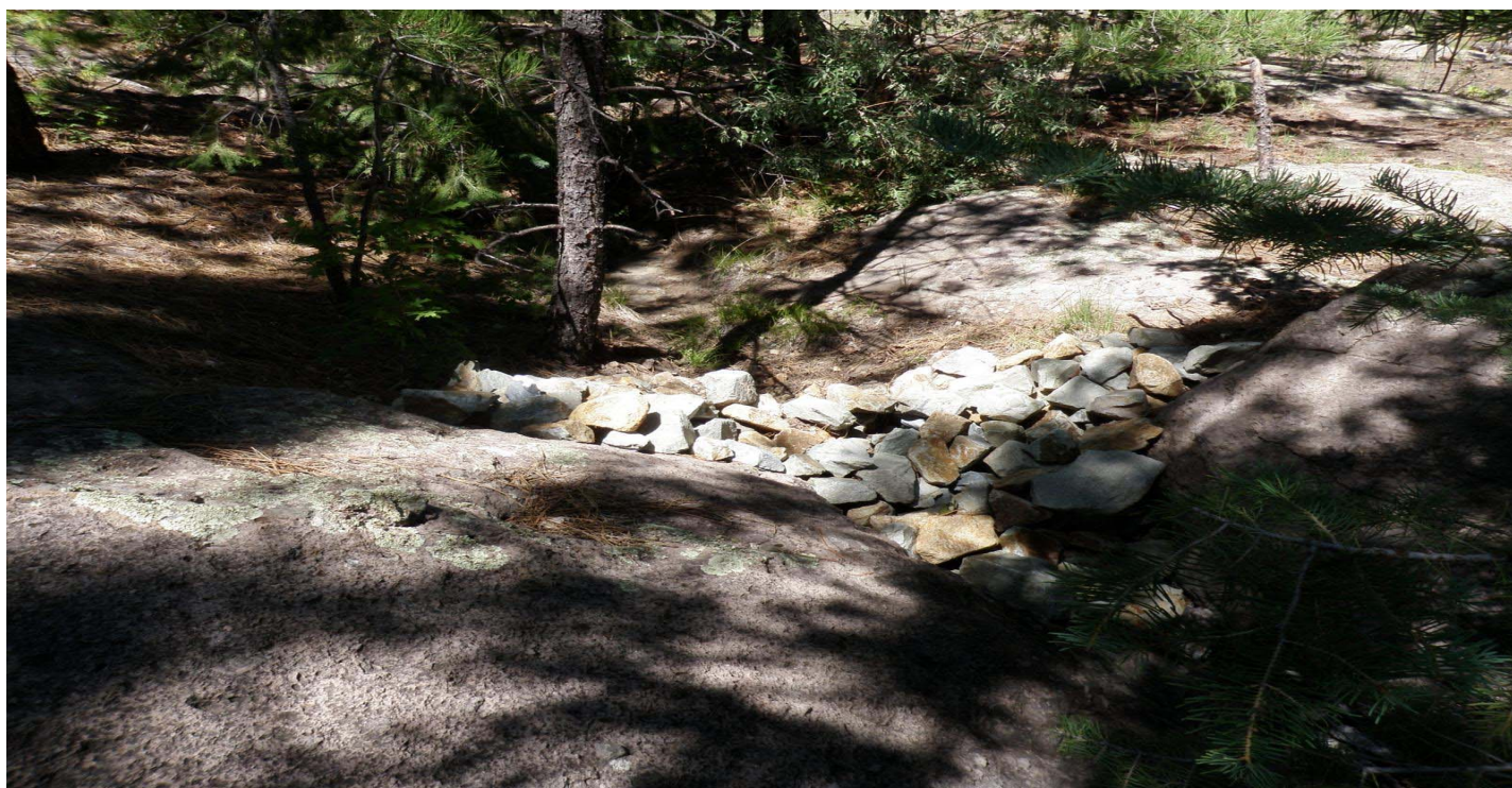
Photo 8510-3r.JPG (taken 08/20/10) M00206010003 : Check Dam - Rock Check Dam.
