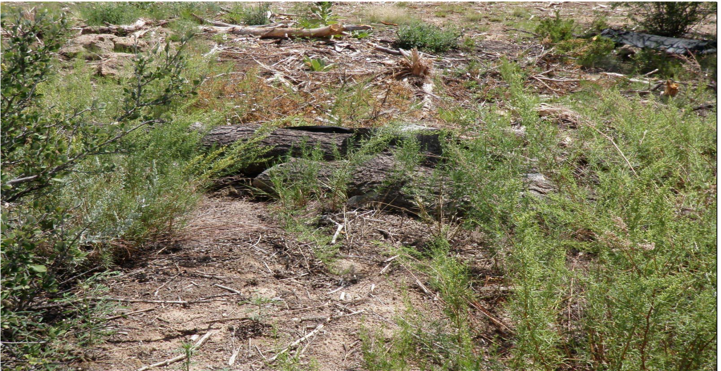
Photo 7476-6r.JPG (taken 08/10/10) M02206020001 : Check Dam - Log Check Dam.
