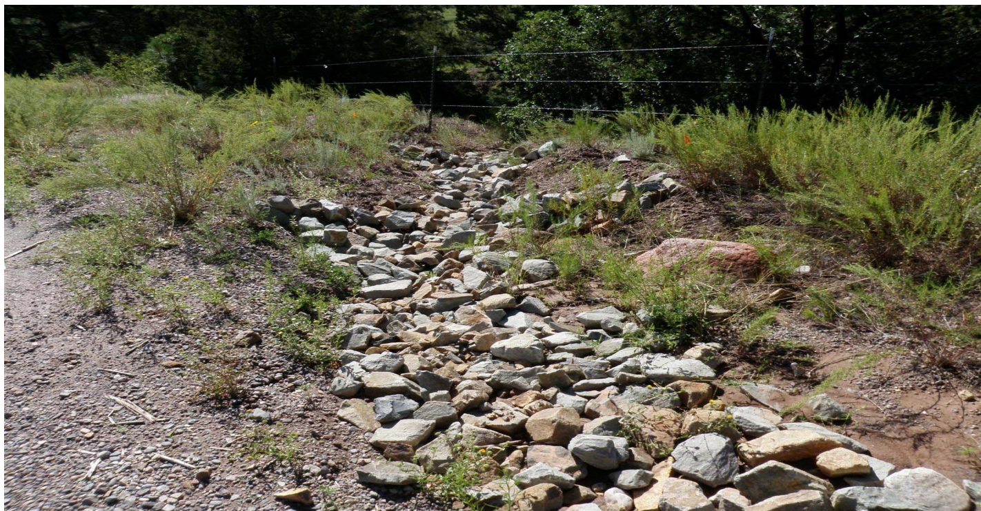
Photo 7598-1r.JPG (taken 08/13/10) R00604060004 : Channel/Swale - Rip Rap; R00606010005 : Check Dam - Rock Check Dam; R00606010006 : Check Dam - Rock Check Dam.
