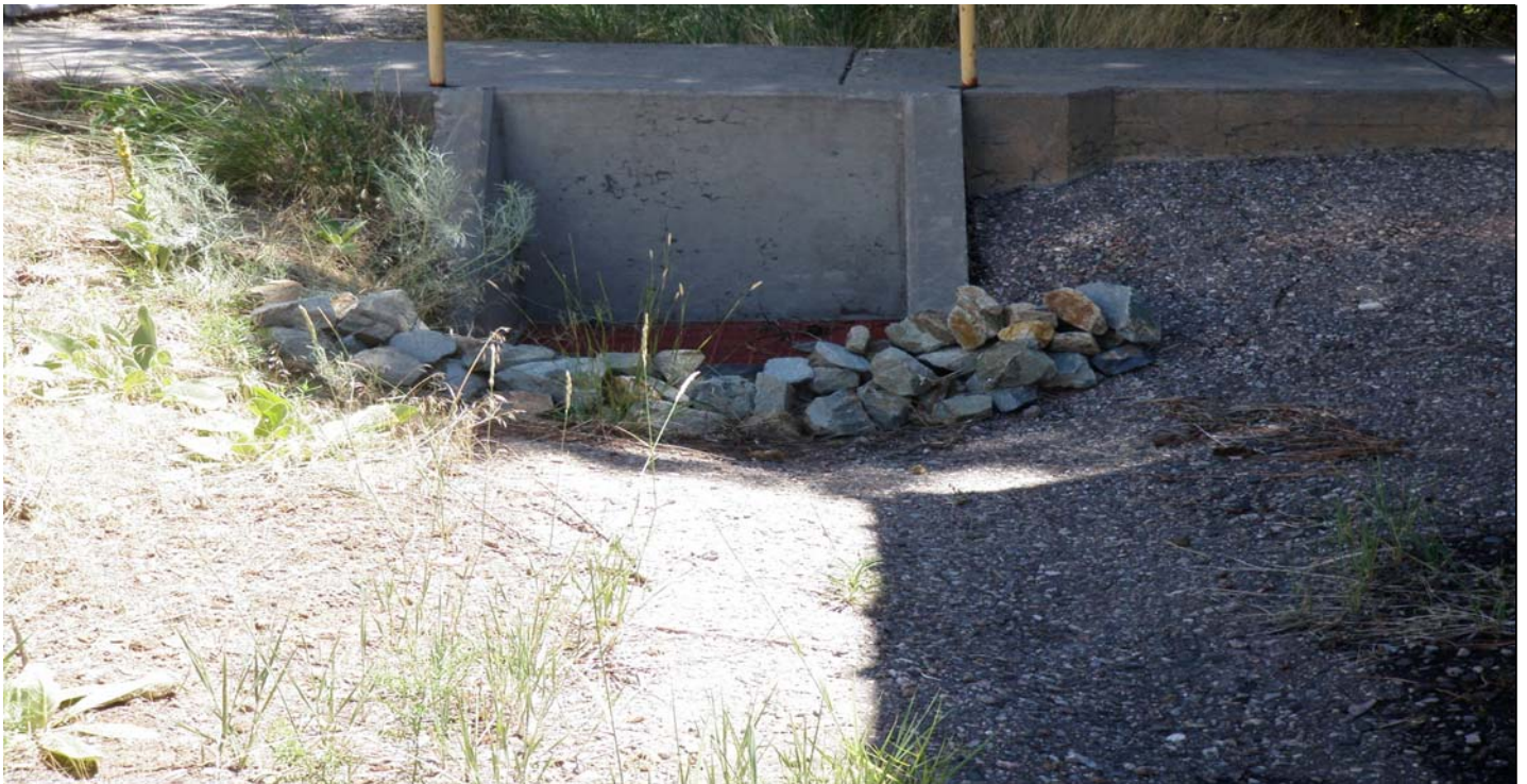
Photo 7469-1.JPG (taken 08/06/10) T00406010006 : Check Dam - Rock Check Dam.
