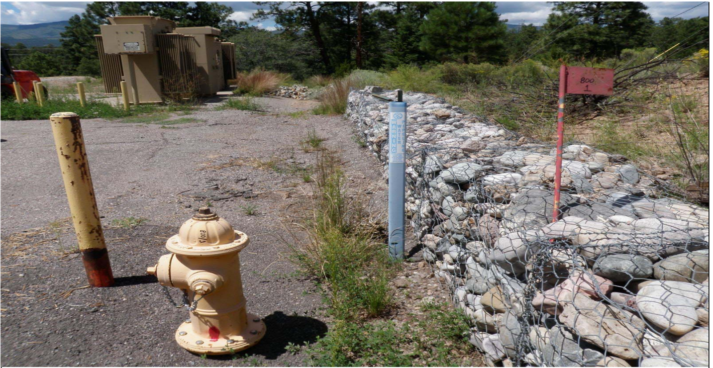
Photo 8515-1r.JPG (taken 08/19/10) S00804020002 : Channel/Swale - Concrete/Asphalt Channel/Swale; S00806010011 : Check Dam - Rock Check Dam; S00807010001 : Gabions - Gabions.
