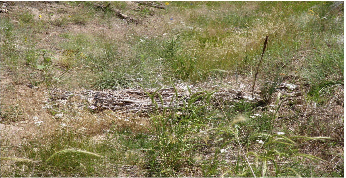
Photo 8656-2.JPG (taken 07/29/10) D00406030007 : Check Dam - Juniper Bales.
