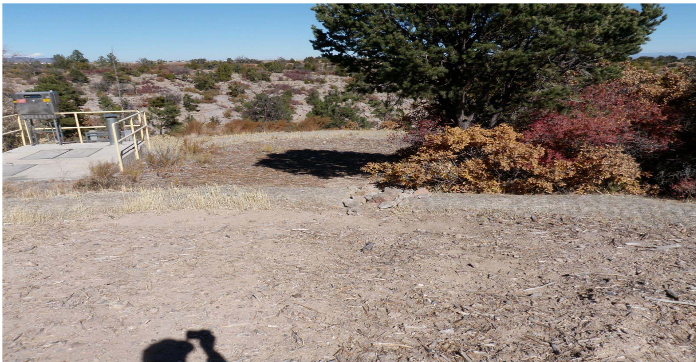
Photo 11656-1r.JPG (taken 11/05/10) D00803010006 : Berms - Earthen Berm; D00803010007 : Berms - Earthen Berm.
