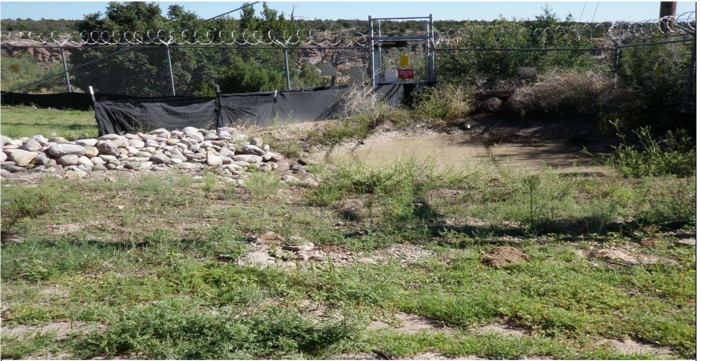
Photo 8509-1r.JPG (taken 08/20/10) C01002010003 : Established Vegetation - Permanent Vegetation Grasses and Shrubs; C01004060007 : Channel/Swale - Rip Rap; C01005010004 : Sediment Traps and Basins - Sediment Trap.
