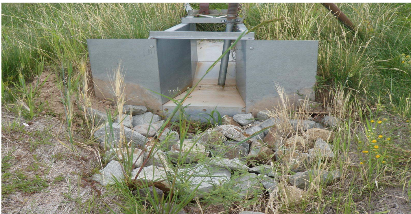
Photo 10553-3r.JPG (taken 09/08/10) S003A04060003 : Channel/Swale - Rip Rap.
