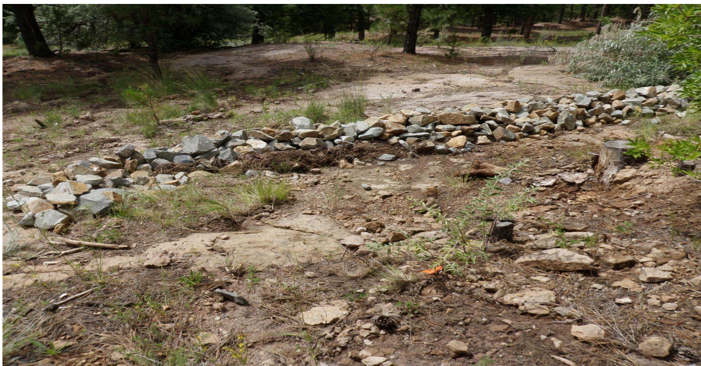
Photo 7494-3r.JPG (taken 08/09/10) M002A03120005 : Berms - Rock Berm.
