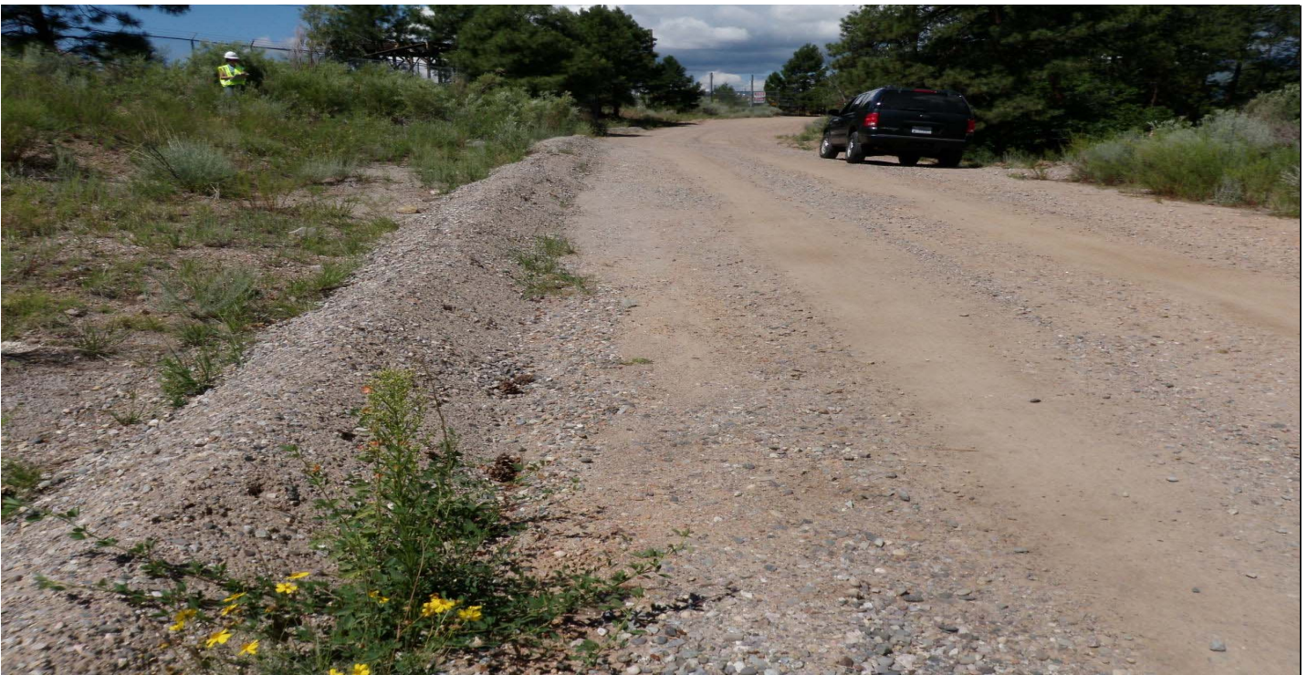
Photo 7415-3.JPG (taken 07/29/10) D00603020002 : Berms - Base Course Berm.
