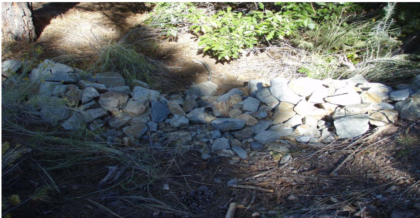
Photo 10869-2.JPG (taken 10/08/10) S005B06010004 : Check Dam - Rock Check Dam.
