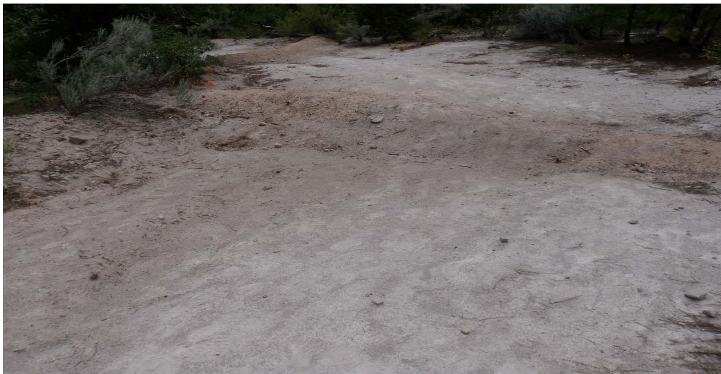
Photo 7452-03.JPG (taken 08/04/10) T00103020014 : Berms - Base Course Berm.
