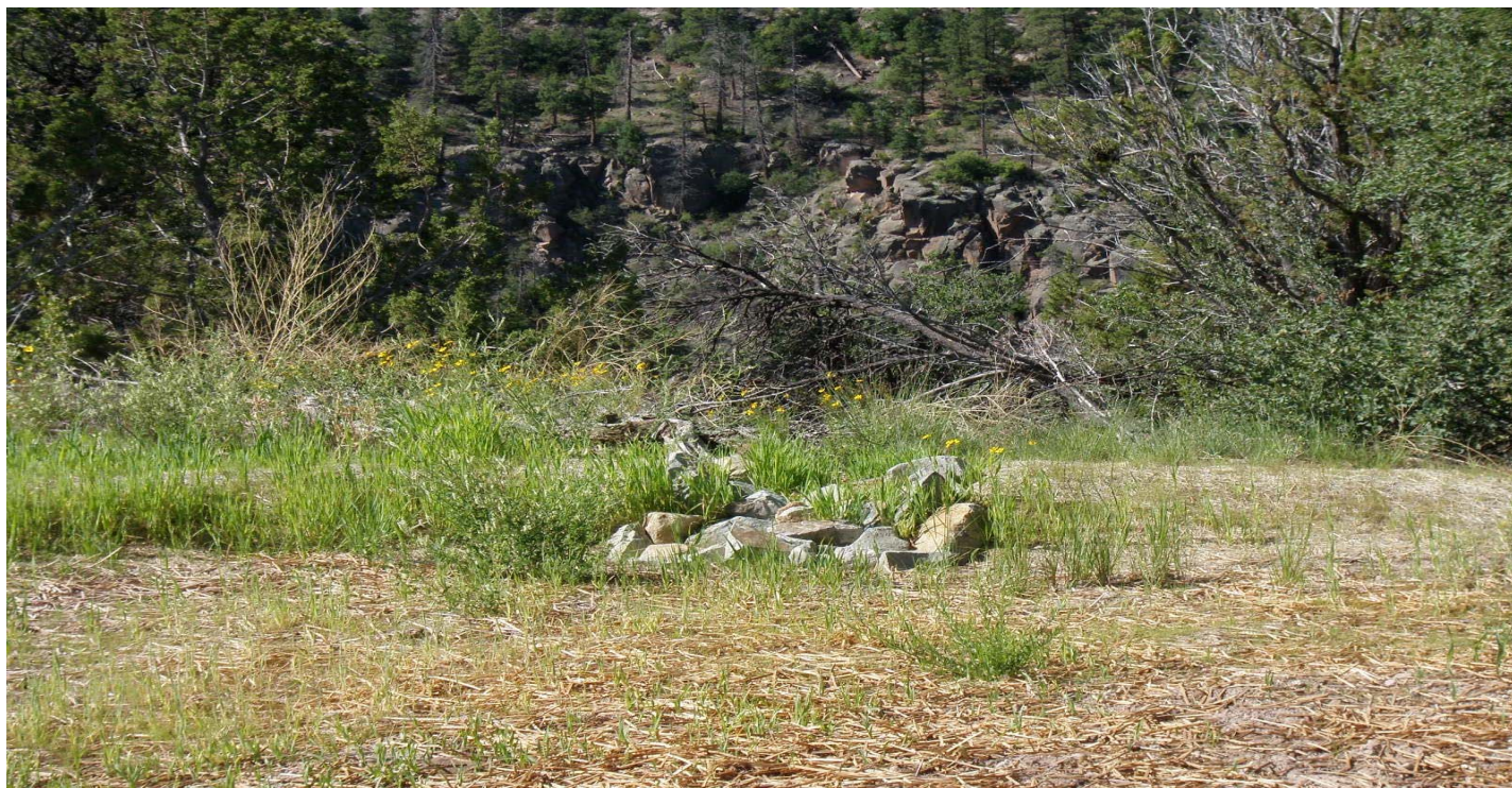
Photo 7436-2.JPG (taken 07/29/10) L02702010001 : Established Vegetation - Permanent Vegetation Grasses and Shrubs; L02703010004 : Berms - Earthen Berm.
