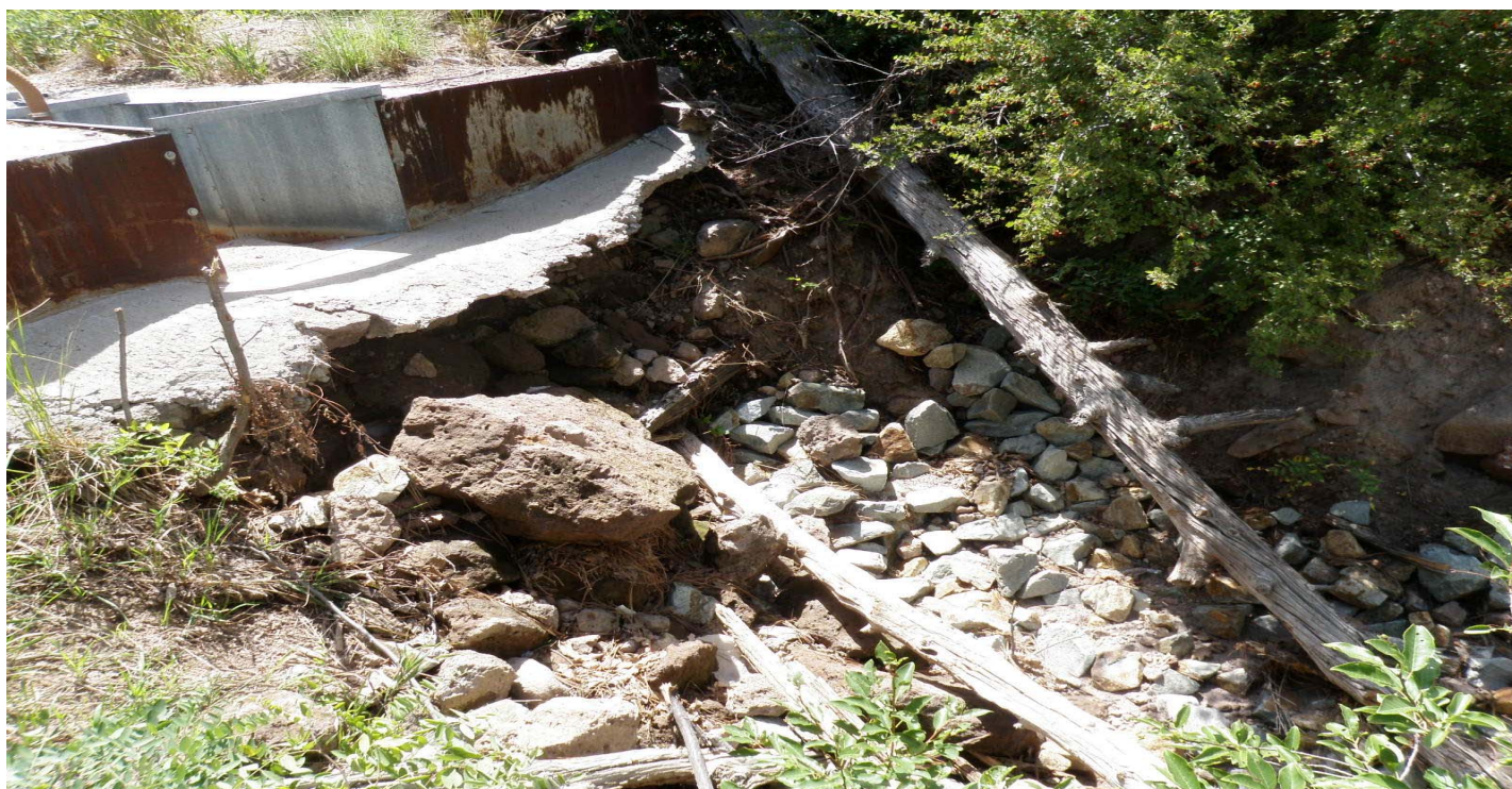
Photo 7454-1.JPG (taken 08/04/10) T00204060006 : Channel/Swale - Rip Rap.
