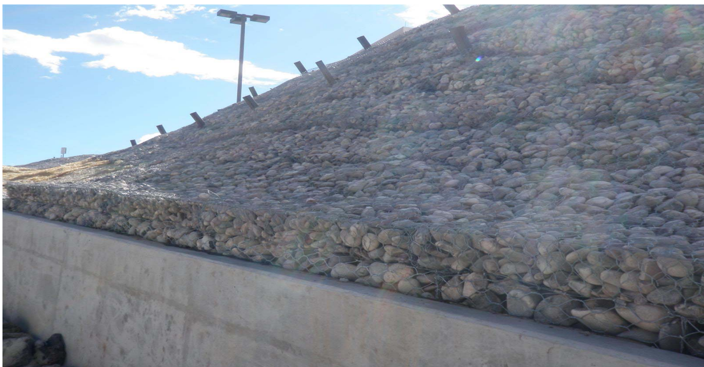
Photo 10550-02r.JPG (taken 09/20/10) M00807020013 : Gabions - Gabion Blanket.
