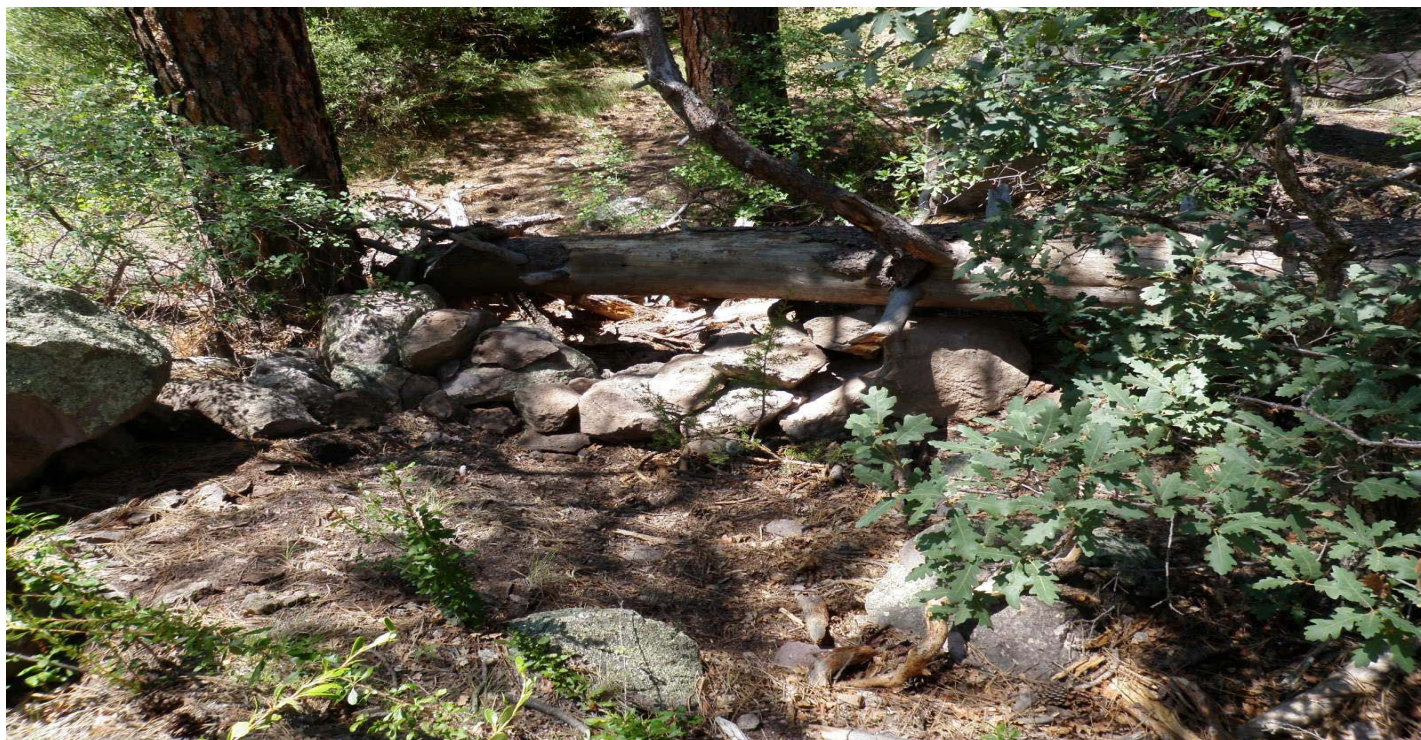
Photo 7433-1.JPG (taken 07/29/10) L02406010005 : Check Dam - Rock Check Dam.
