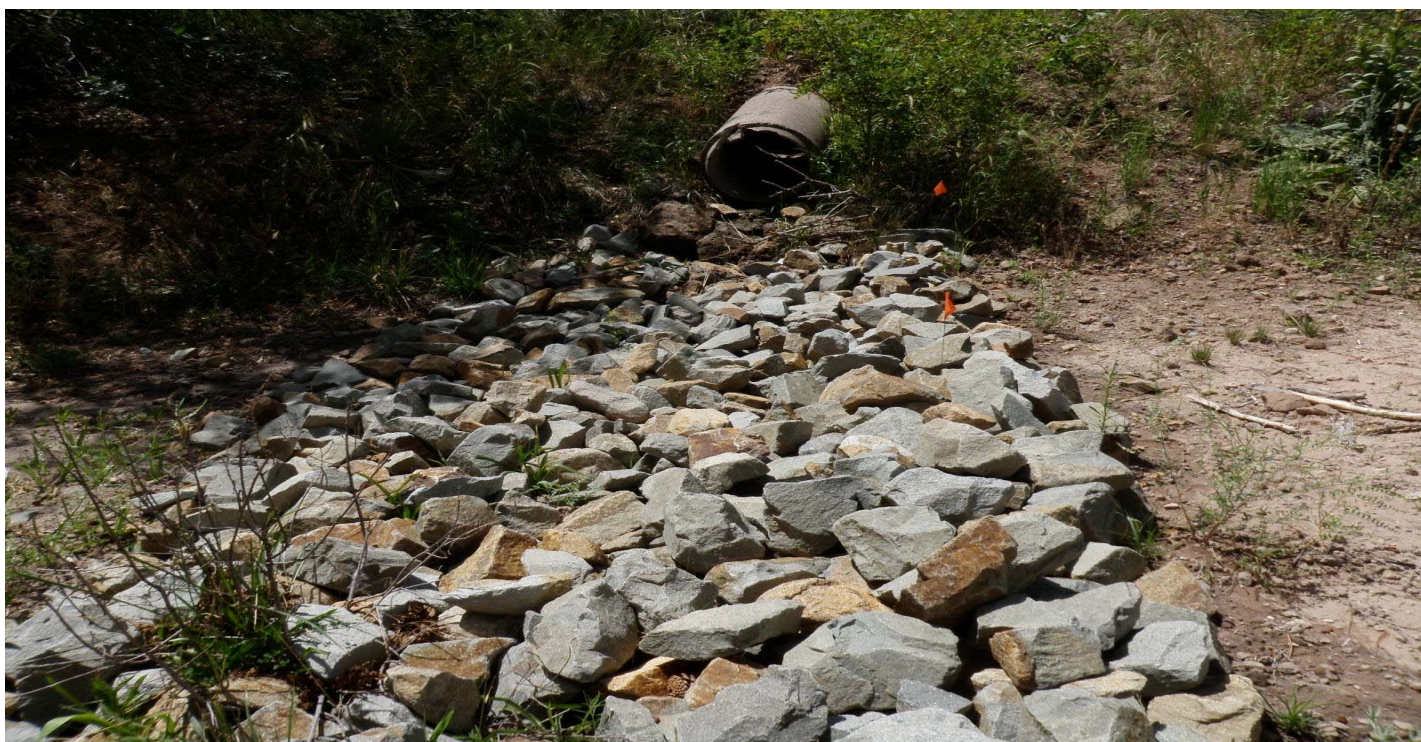
Photo 7413-2.JPG (taken 07/29/10) D00204040003 : Channel/Swale - Culvert; D00204060006 : Channel/Swale - Rip Rap.
