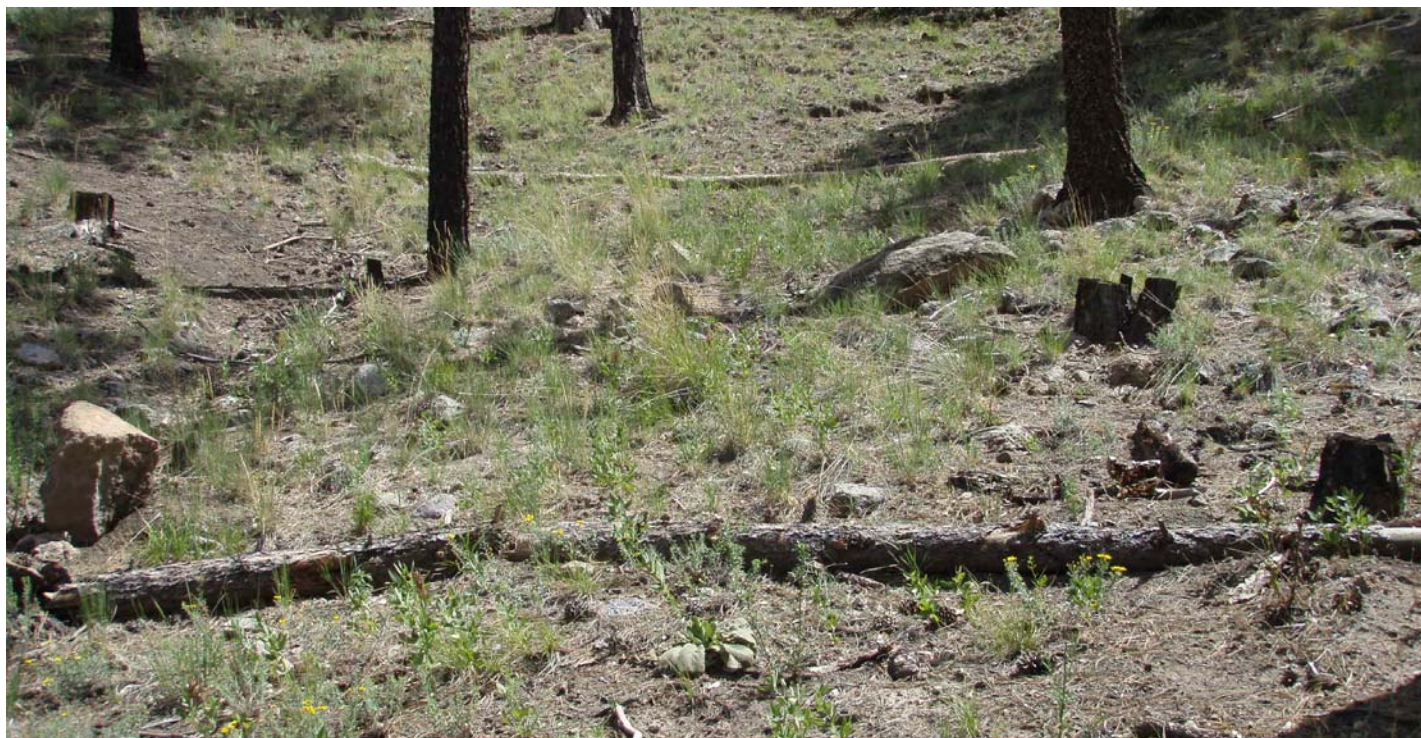
Photo 7441-1.JPG (taken 08/03/10) R00103030004 : Berms - Log Berm; R00103060007 : Berms - Straw Wattles.
