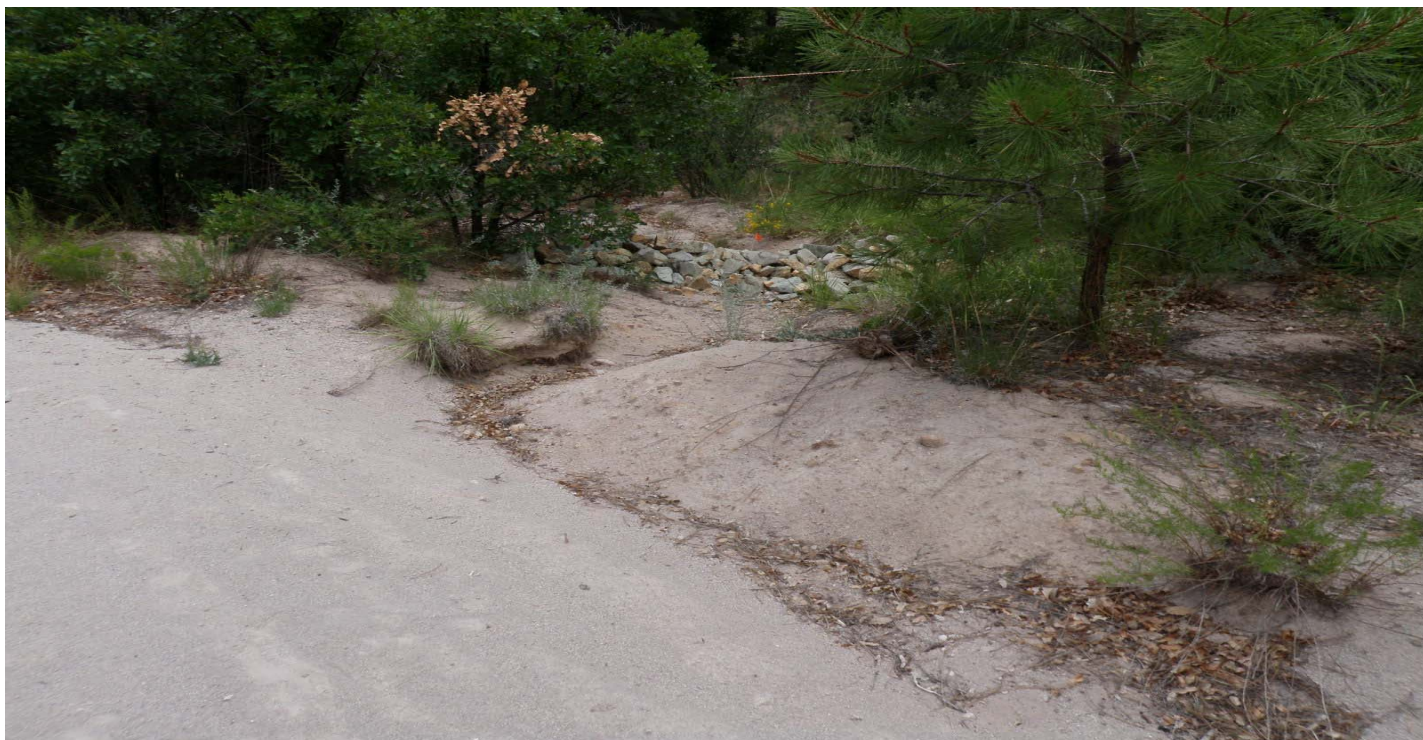
Photo 7452-1.JPG (taken 08/04/10) T00106010012 : Check Dam - Rock Check Dam.
