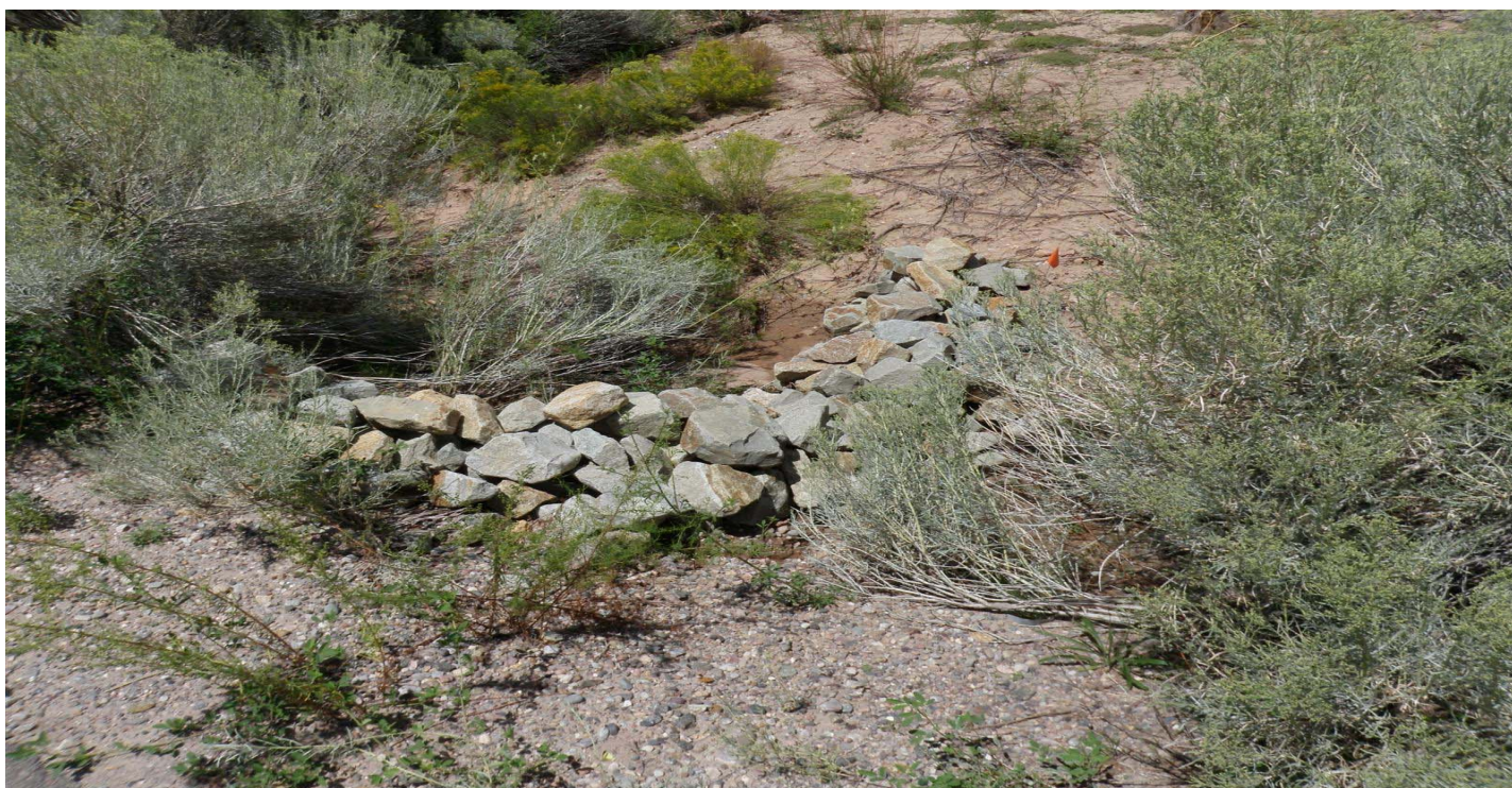
Photo 8500-1r.JPG (taken 08/19/10) S01406010010 : Check Dam - Rock Check Dam.
