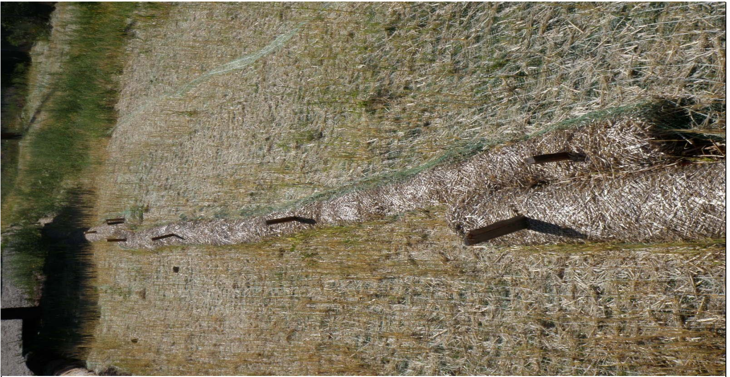
Photo 7435-2.JPG (taken 07/28/10) L02603060007 : Berms - Straw Wattles.
