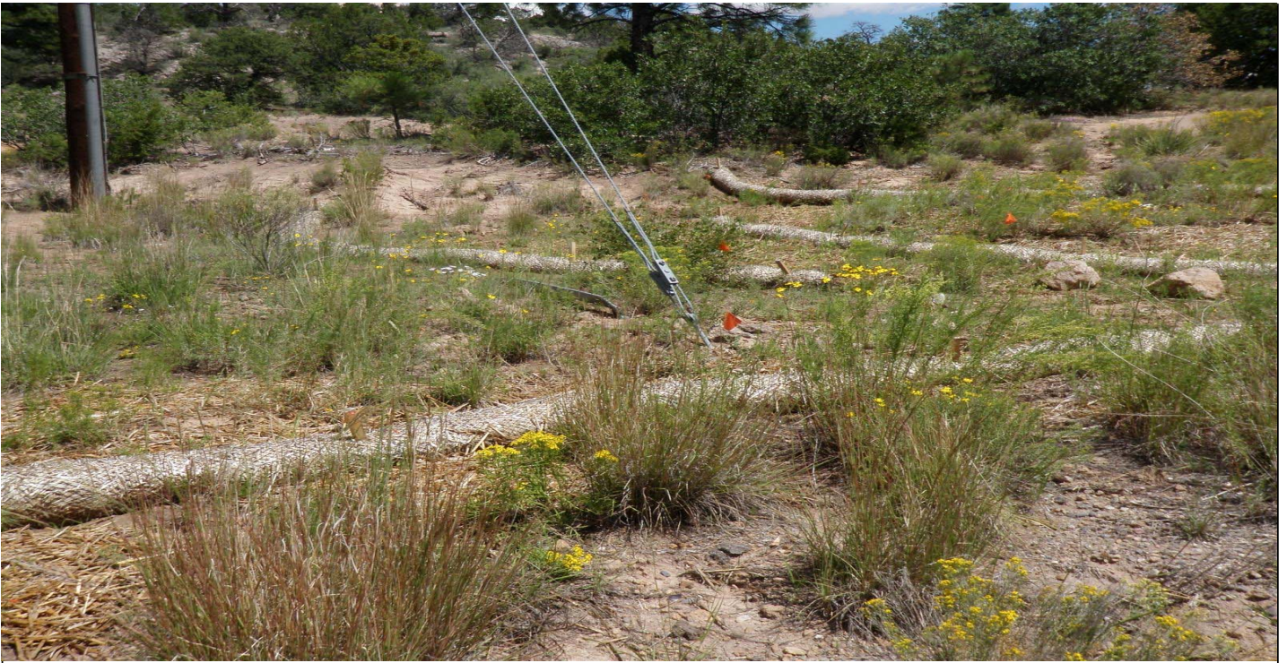
Photo 8515-3r.JPG (taken 08/19/10) S00801010012 : Seed and Mulch - Seed and Wood Mulch; S00802010003 : Established Vegetation - Permanent Vegetation Grasses and Shrubs; S00803060004 : Berms - Straw Wattles; S00803060005 : Berms - Straw Wattles; S00803060006 : Berms - Straw Wattles; S00803060007 : Berms - Straw Wattles.
