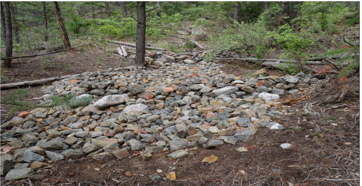
Photo 7466-4.JPG (taken 08/06/10) M01204060007 : Channel/Swale - Rip Rap; M01204060008 : Channel/Swale - Rip Rap; M01206010001 : Check Dam - Rock Check Dam; M01206010005 : Check Dam - Rock Check Dam.
