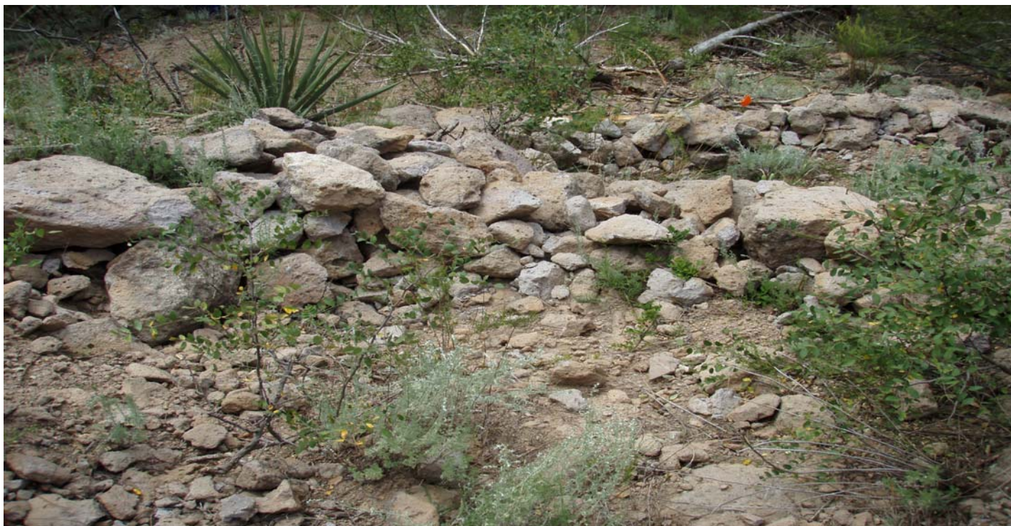
Photo 8532-2.JPG (taken 08/23/10) T00706010011 : Check Dam - Rock Check Dam.
