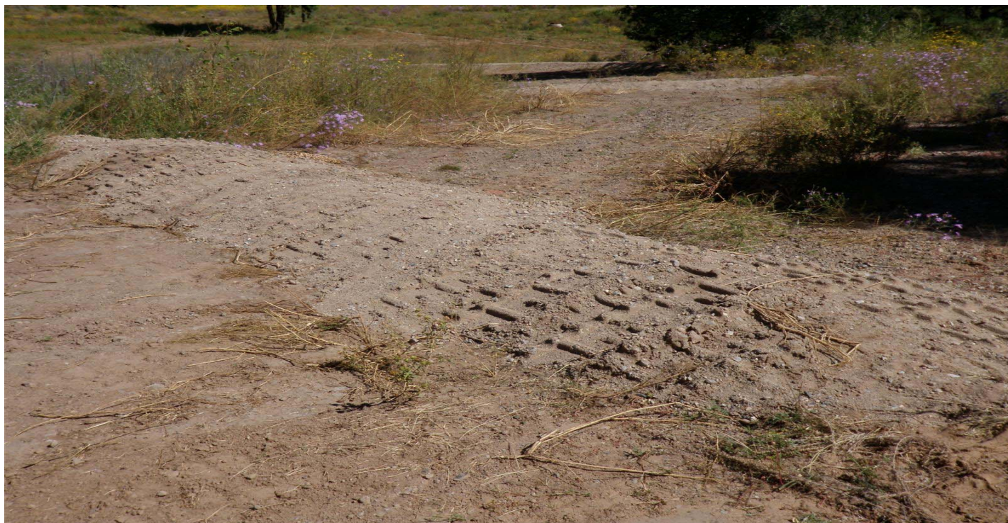
Photo 10559-1r.JPG (taken 09/14/10) P00904050005 : Channel/Swale - Water Bar; P00904050006 : Channel/Swale - Water Bar.
