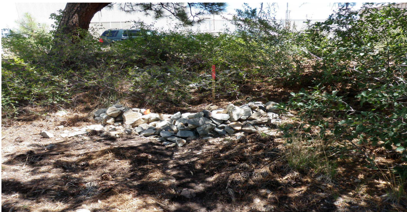
Photo 7453-2.JPG (taken 08/04/10) S00906010005 : Check Dam - Rock Check Dam; S00906010006 : Check Dam - Rock Check Dam.
