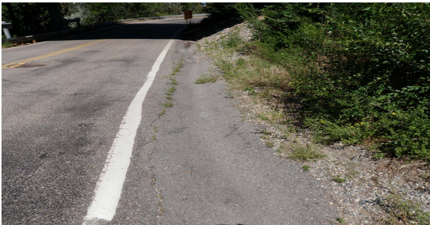
Photo 7418-1.JPG (taken 07/28/10) L00304020005 : Channel/Swale - Concrete/Asphalt Channel/Swale.
