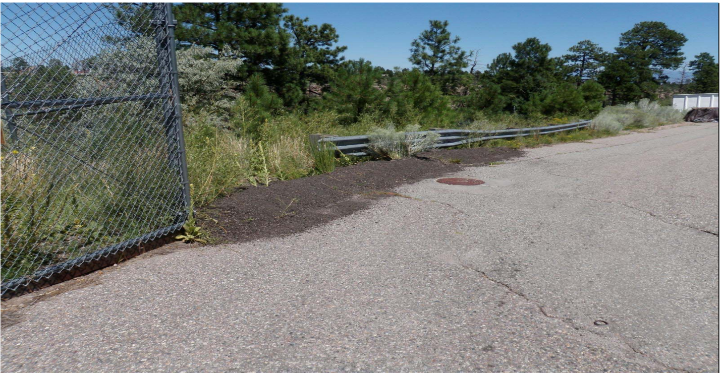
Photo 8511-1r.JPG (taken 08/20/10) M00403040006 : Berms - Asphalt Berm.
