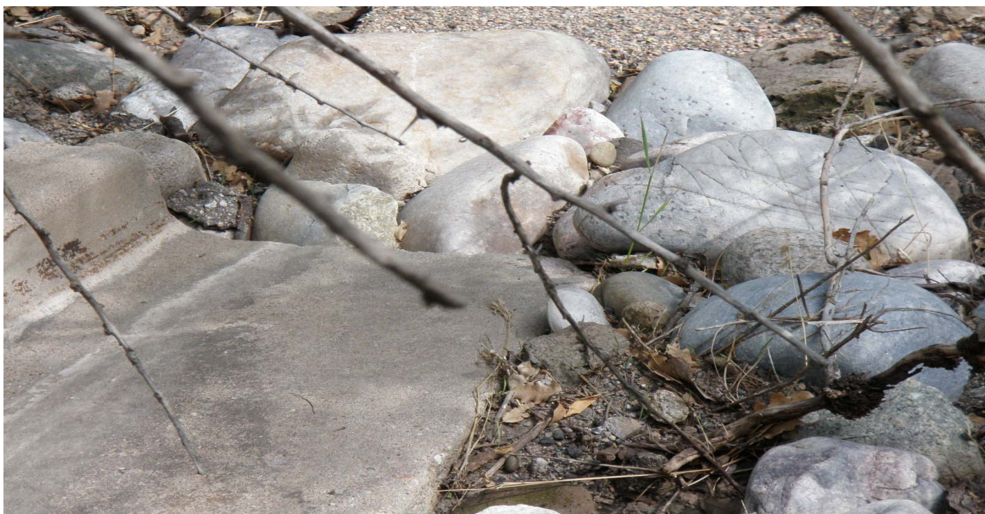
Photo 7458-6.JPG (taken 08/04/10) T00604060004 : Channel/Swale - Rip Rap.
