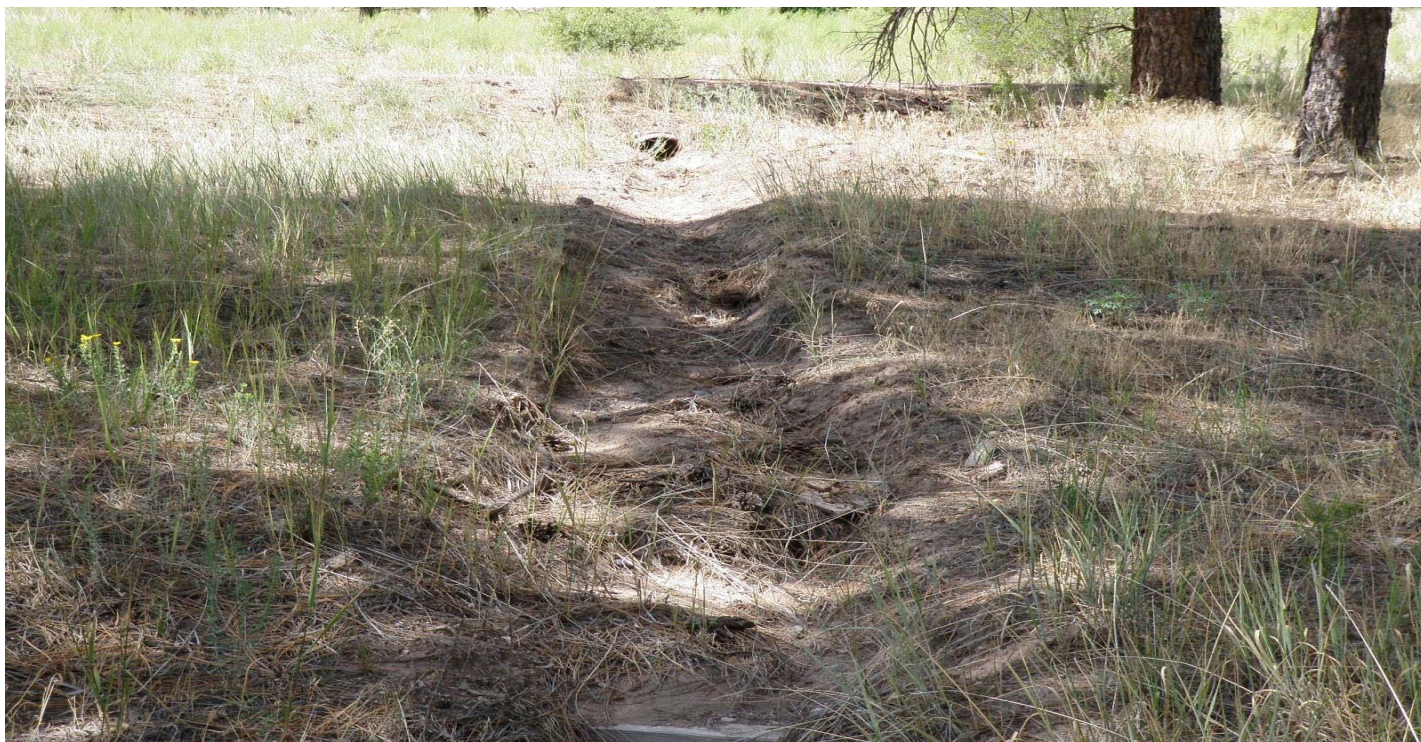
Photo 7411-5.JPG (taken 07/30/10) B00104010005 : Channel/Swale - Earthen Channel/Swale; B00104040003 : Channel/Swale - Culvert.
