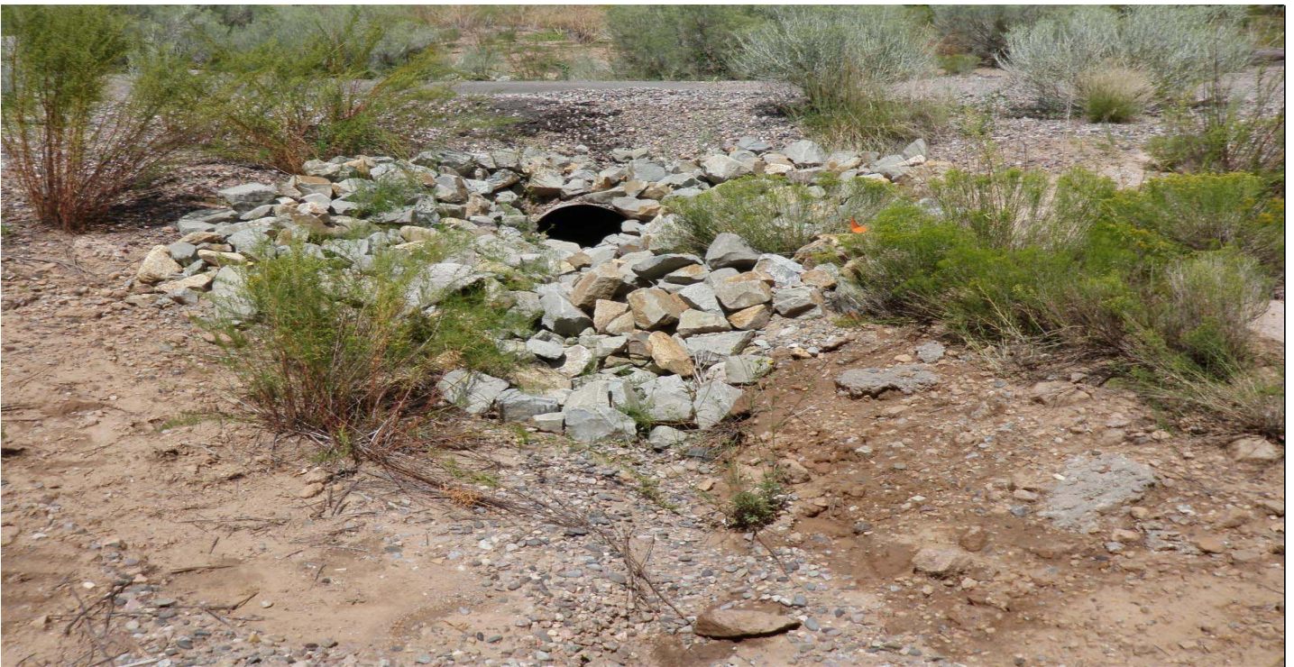
Photo 8500-3r.JPG (taken 08/19/10) S01404060011 : Channel/Swale - Rip Rap; S01406010009 : Check Dam - Rock Check Dam.
