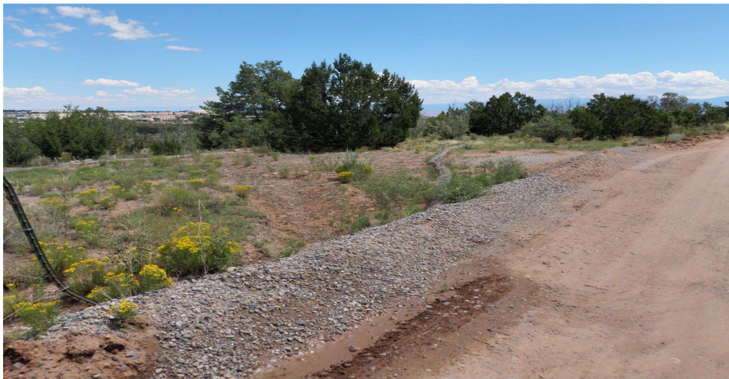
Photo 7477-1r.JPG (taken 08/10/10) M02001010006 : Seed and Mulch - Seed and Wood Mulch; M02003010005 : Berms - Earthen Berm; M02003060003 : Berms - Straw Wattles; M02003060004 : Berms - Straw Wattles.
