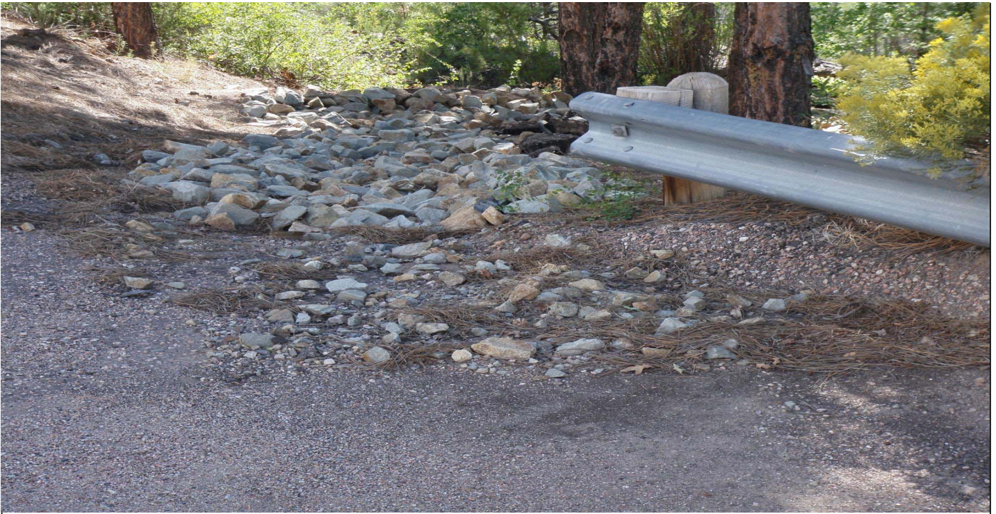
Photo 10555-2r.JPG (taken 09/09/10) S00704030003 : Channel/Swale - Rock Channel/Swale.
