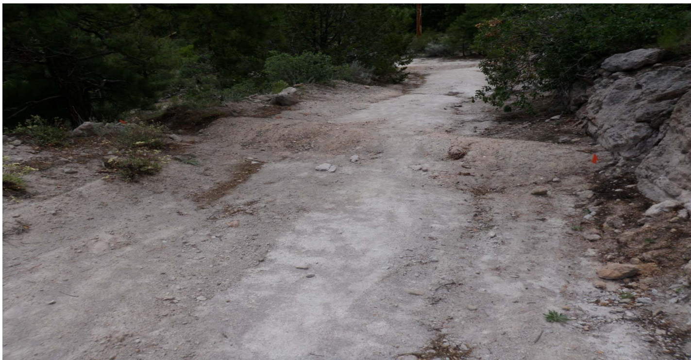
Photo 7452-04.JPG (taken 08/04/10) T00103020015 : Berms - Base Course Berm.
