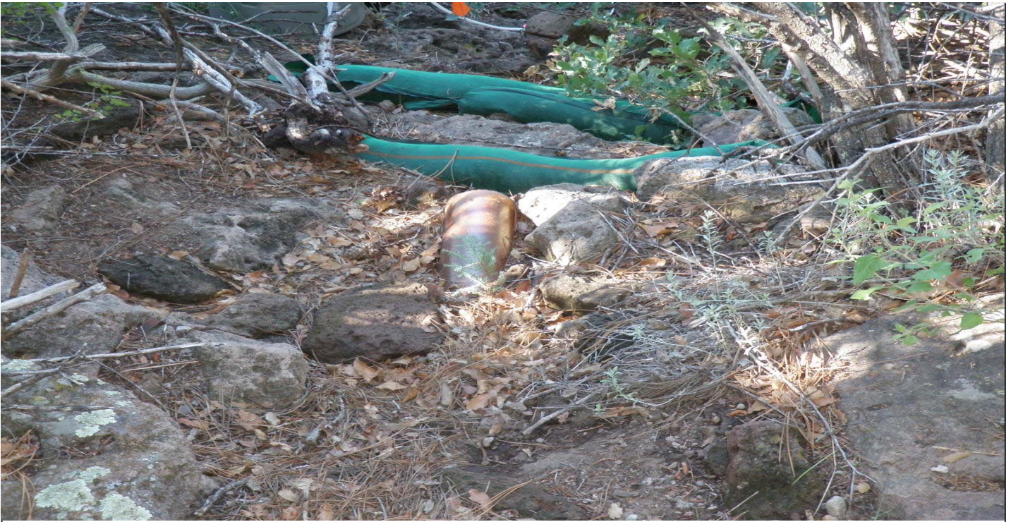
Photo 7447-1.JPG (taken 07/29/10) L01603100005 : Berms - Gravel Bags.
