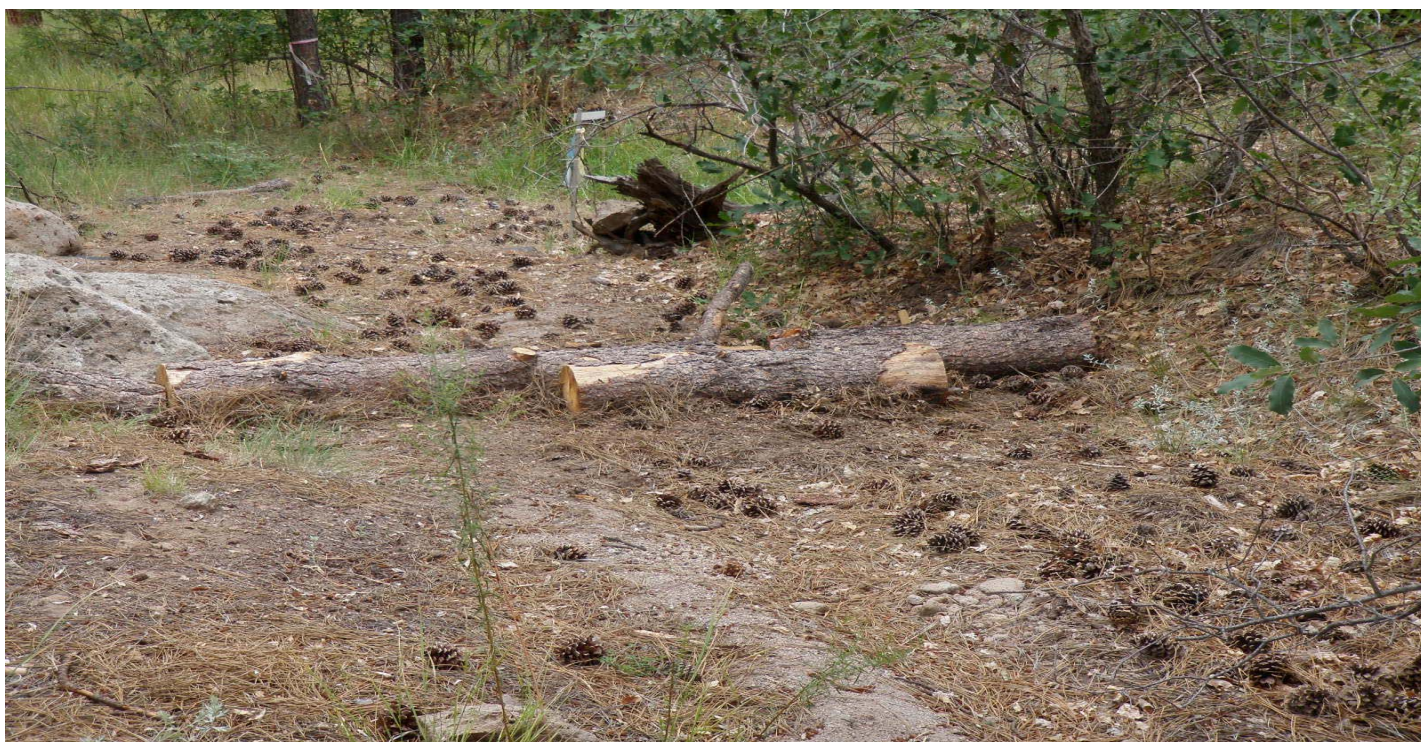
Photo 7458-2.JPG (taken 08/04/10) T00603030010 : Berms - Log Berm.
