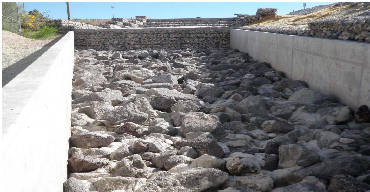
Photo 10550-03r.JPG (taken 09/20/10) M00804060014 : Channel/Swale - Rip Rap.
