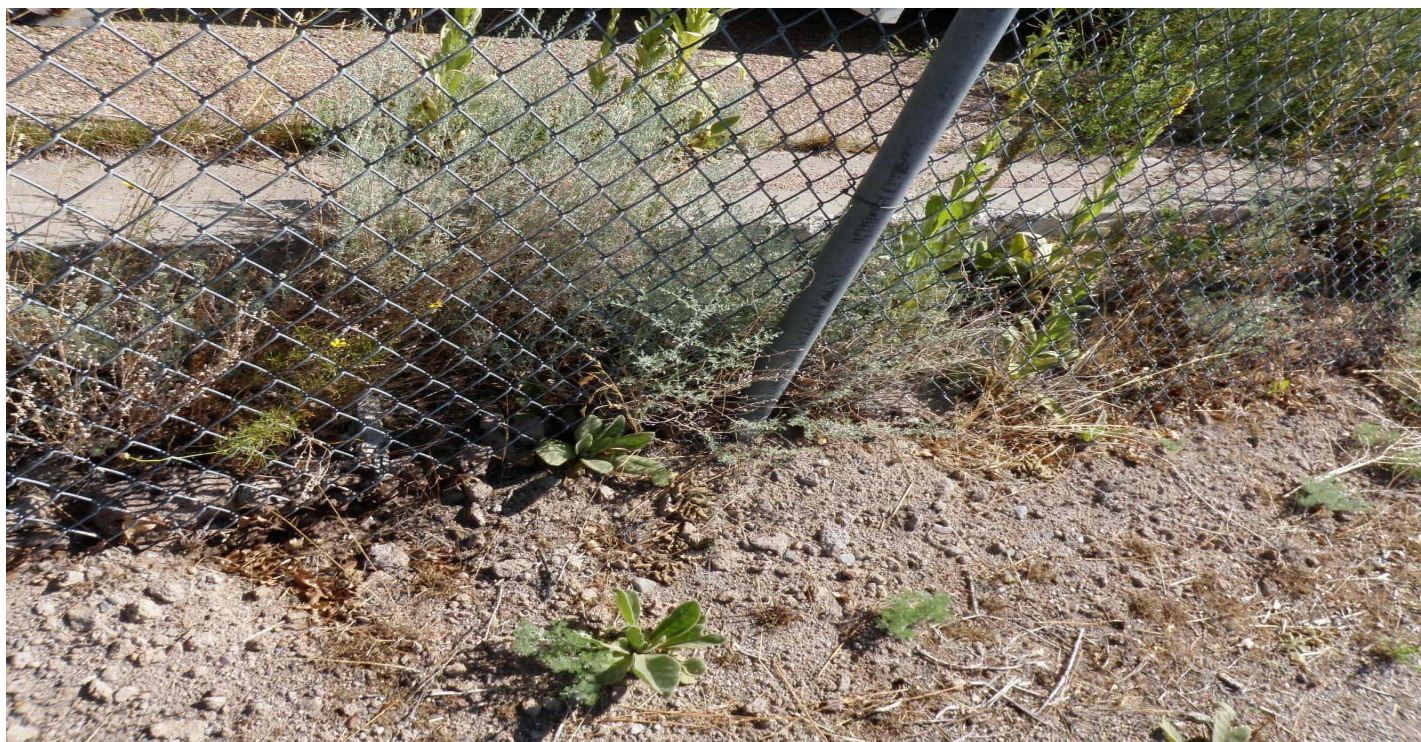
Photo 7434-1.JPG (taken 07/29/10) L02503090004 : Berms - Curbing.
