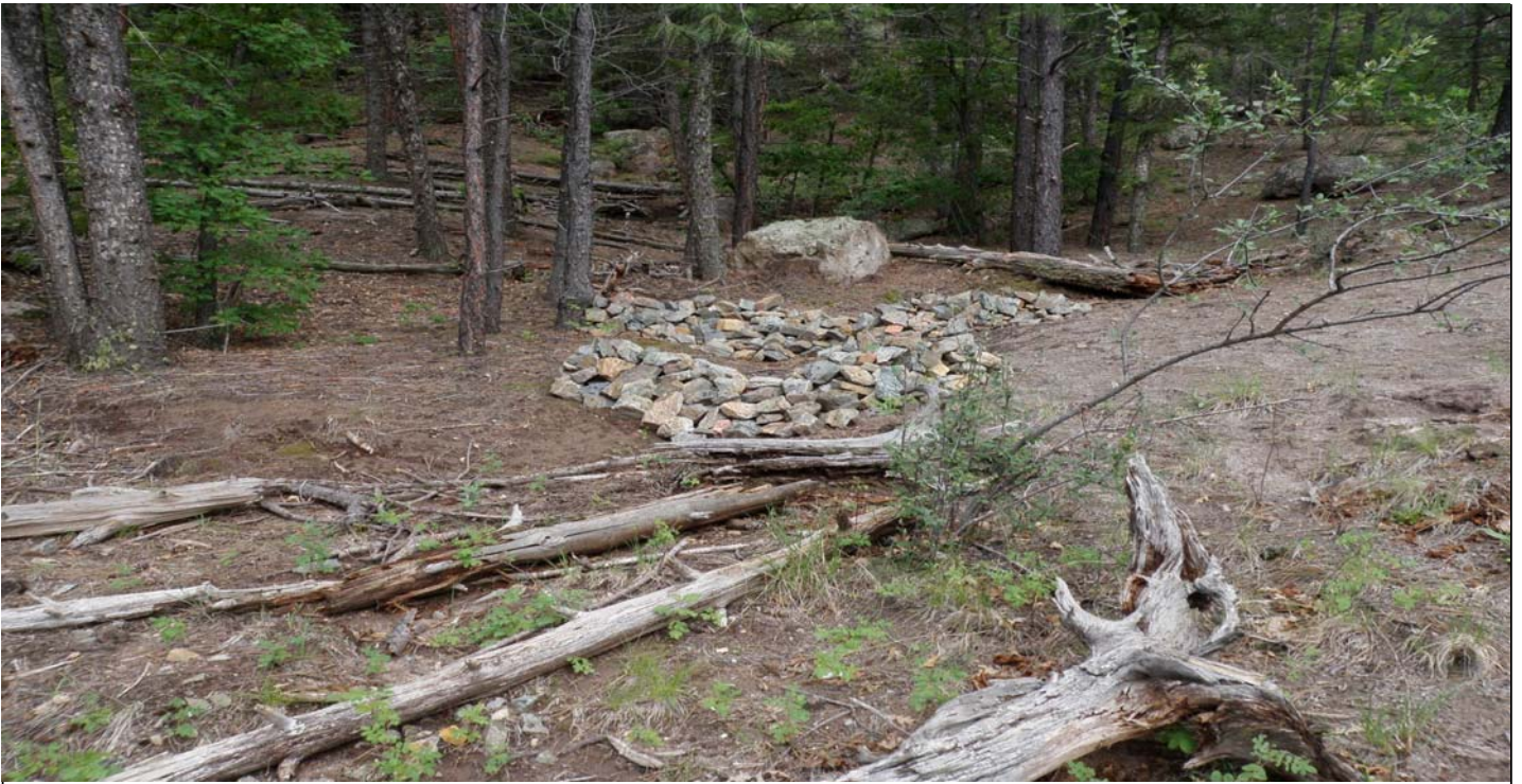
Photo 7466-3.JPG (taken 08/06/10) M01206010006 : Check Dam - Rock Check Dam; M01206010009 : Check Dam - Rock Check Dam.
