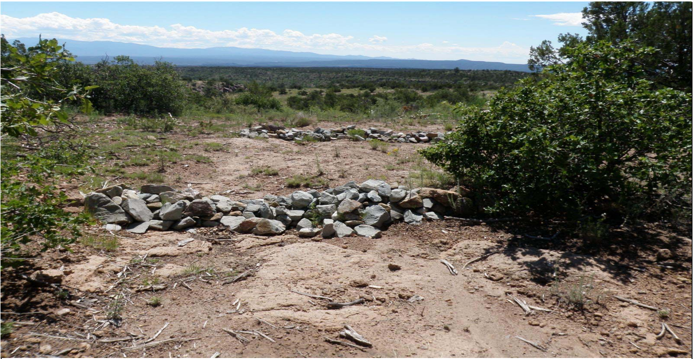
Photo 7476-1r.JPG (taken 08/10/10) M02206010009 : Check Dam - Rock Check Dam; M02206010011 : Check Dam - Rock Check Dam.
