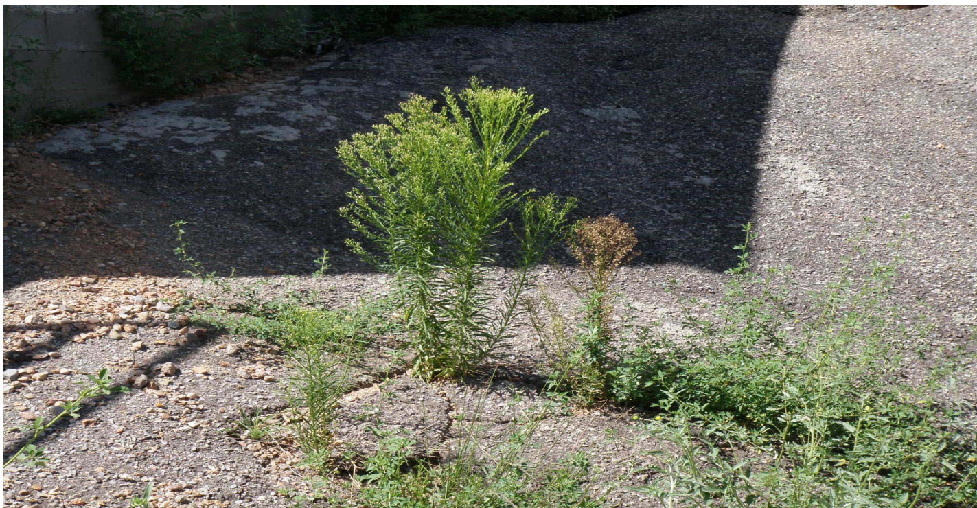
Photo 7452-14.JPG (taken 08/04/10) T00104020006 : Channel/Swale - Concrete/Asphalt Channel/Swale.
