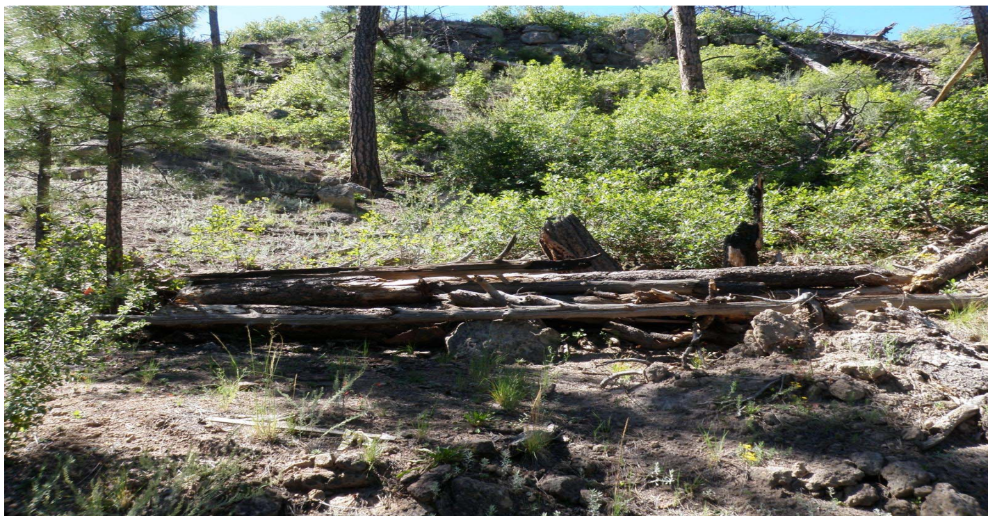
Photo 8664-1r.JPG (taken 09/02/10) T01006020006 : Check Dam - Log Check Dam.
