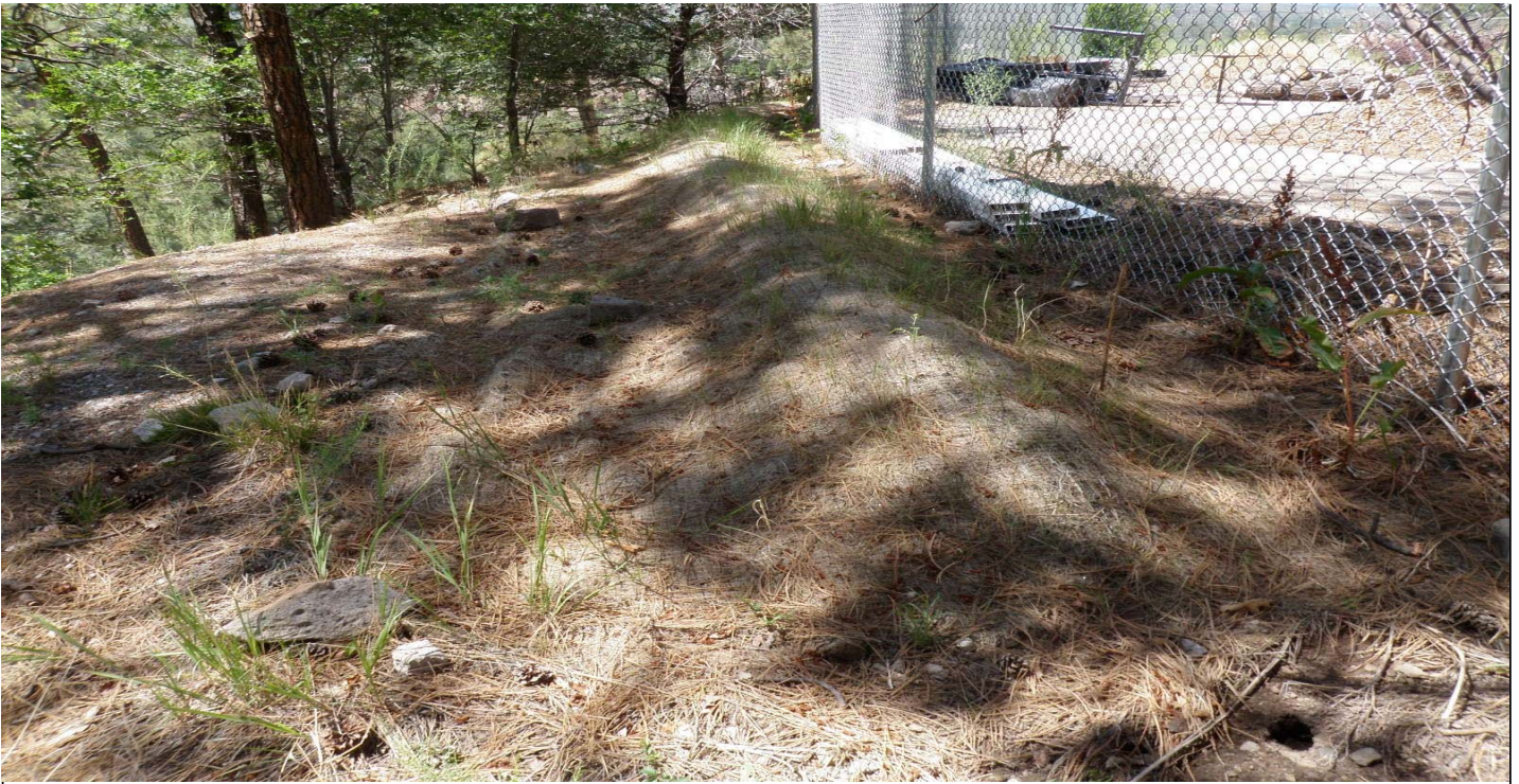
Photo 7410-2.JPG (taken 07/30/10) P002A01060003 : Seed and Mulch - Erosion Control Blanket; P002A03010004 : Berms - Earthen Berm.
