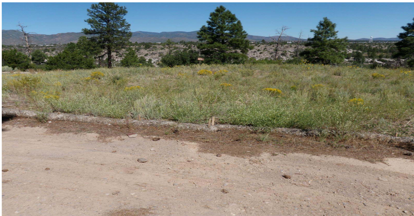
Photo 8665-4r.JPG (taken 09/02/10) T00903060004 : Berms - Straw Wattles.
