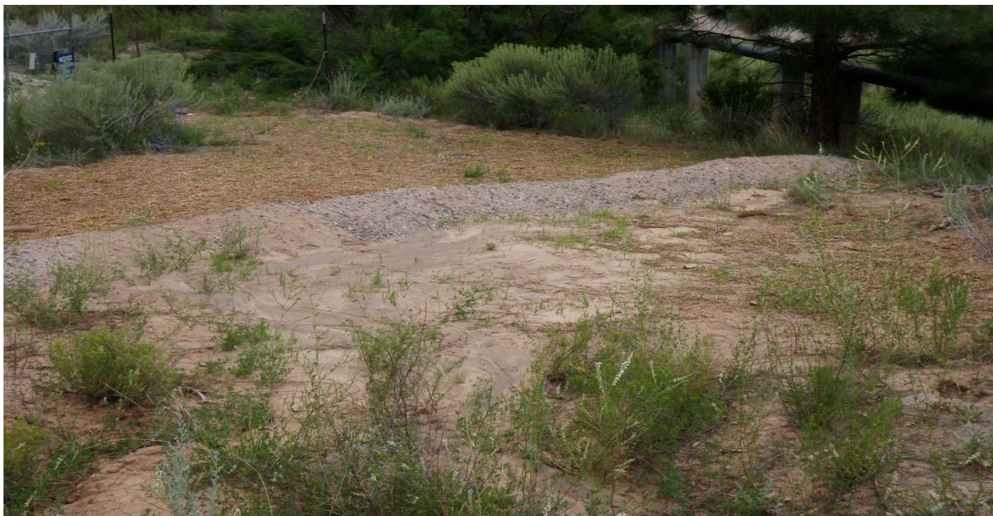
Photo 7452-10.JPG (taken 08/04/10) T00101010019 : Seed and Mulch - Seed and Wood Mulch; T00103020018 : Berms - Base Course Berm.
