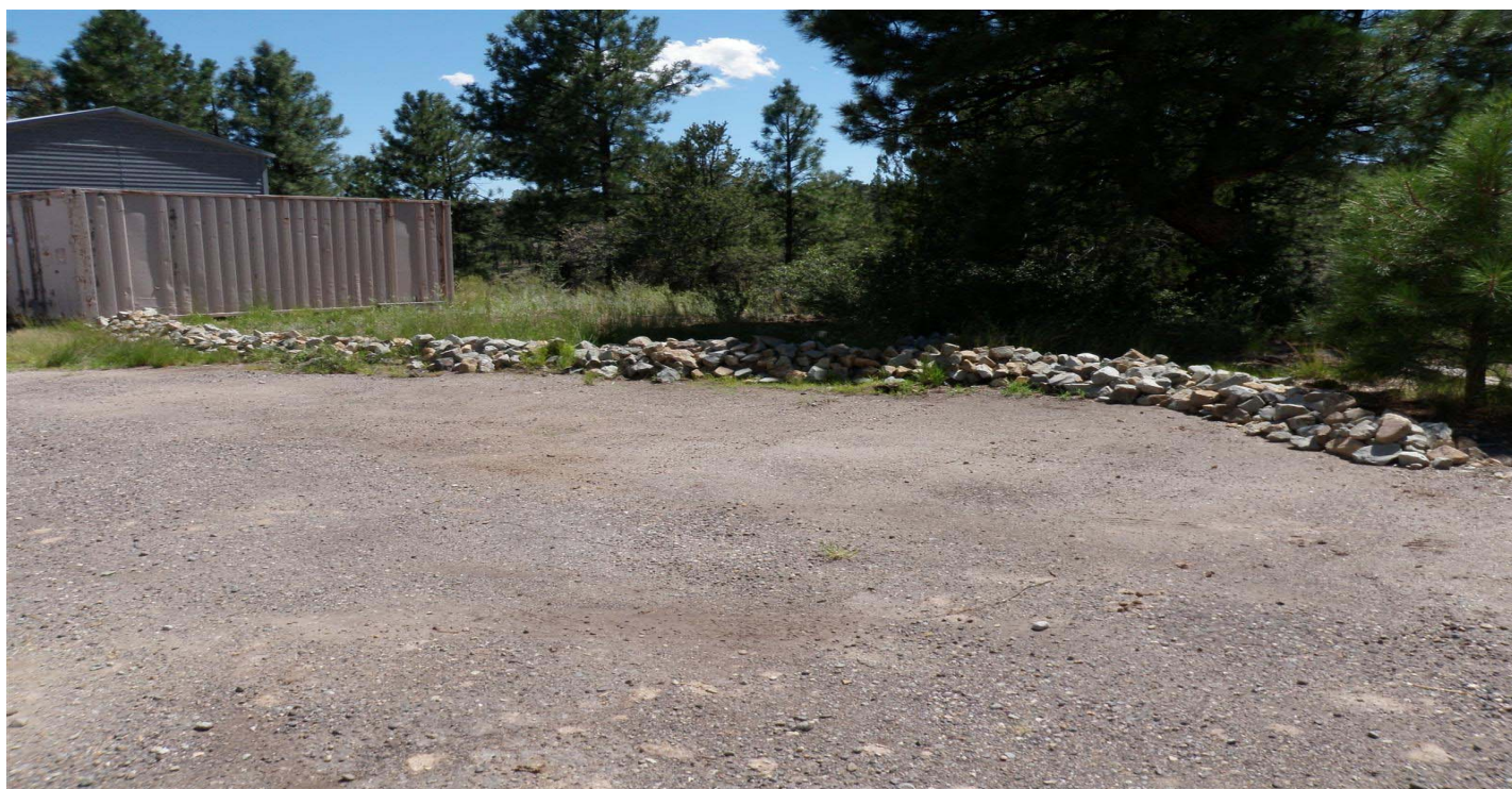
Photo 8512-2r.JPG (taken 08/20/10) S00903120003 : Berms - Rock Berm.
