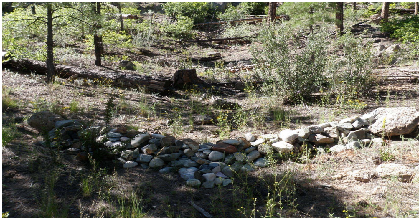
Photo 8665-3r.JPG (taken 09/02/10) T00906010002 : Check Dam - Rock Check Dam; T00906010006 : Check Dam - Rock Check Dam.
