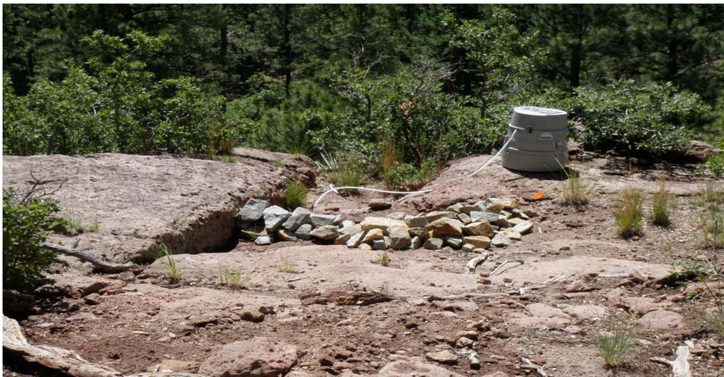
Photo 7470-2.JPG (taken 08/06/10) T00306010005 : Check Dam - Rock Check Dam.
