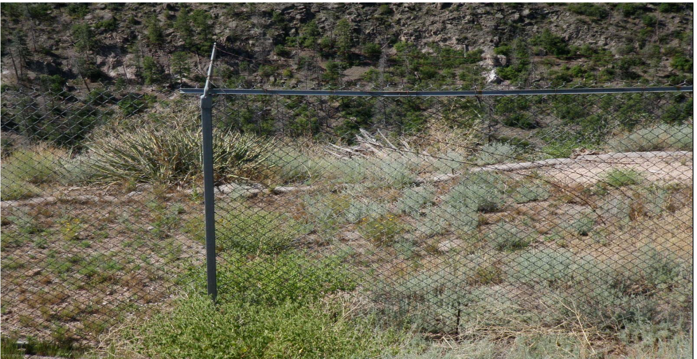
Photo 7431-3.JPG (taken 07/29/10) L022A02010001 : Established Vegetation - Permanent Vegetation Grasses and Shrubs; L022A03060004 : Berms - Straw Wattles.
