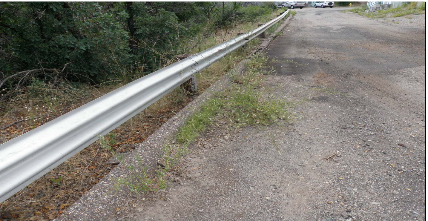
Photo 7458-4.JPG (taken 08/04/10) T00603090005 : Berms - Curbing.
