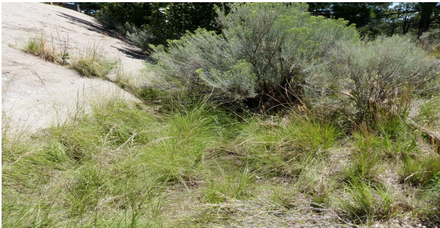
Photo 7470-3.JPG (taken 08/06/10) T00304010002 : Channel/Swale - Earthen Channel/Swale.
