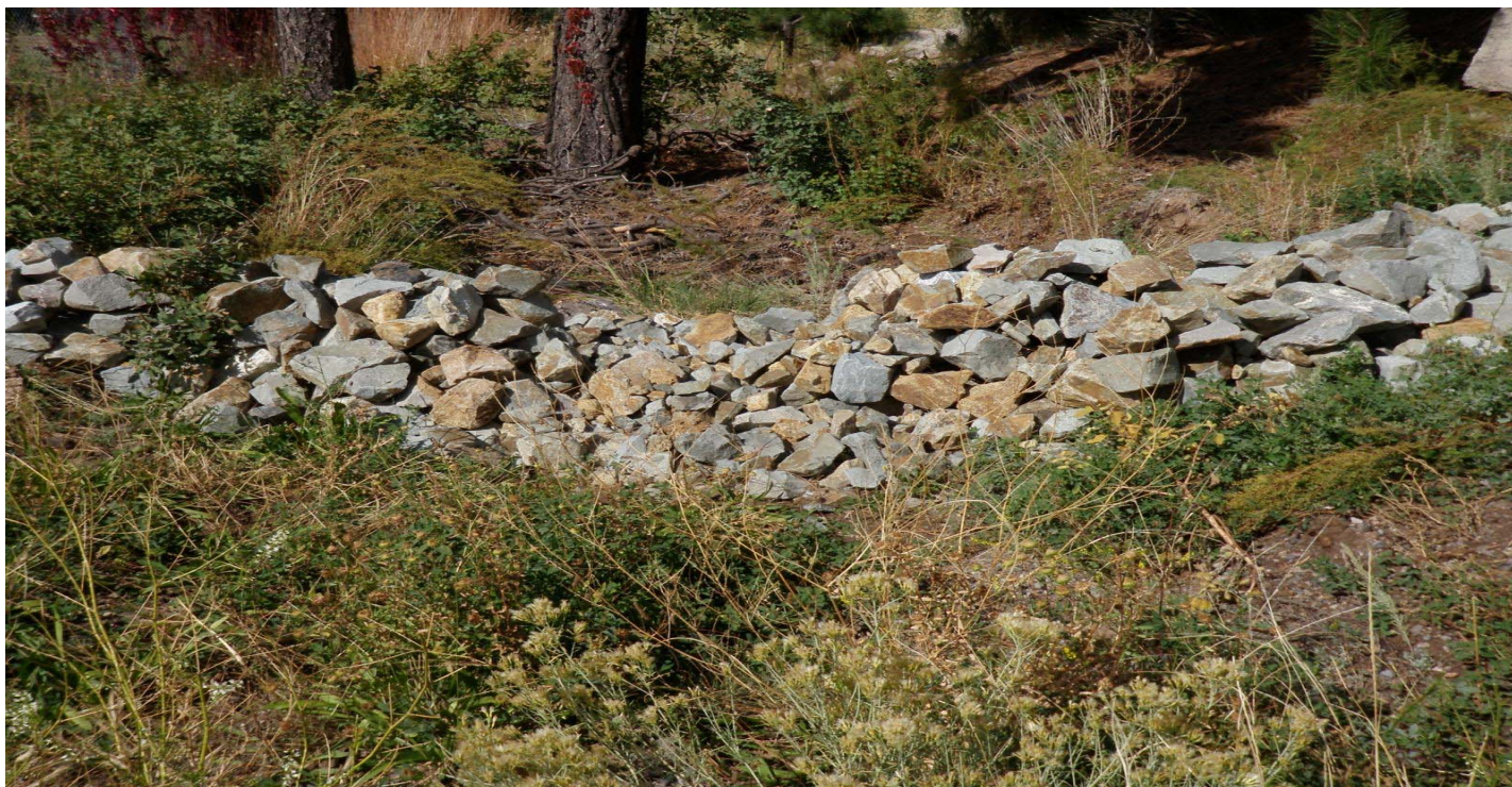
Photo 10890-1r.JPG (taken 10/06/10) S00506010012 : Check Dam - Rock Check Dam.
