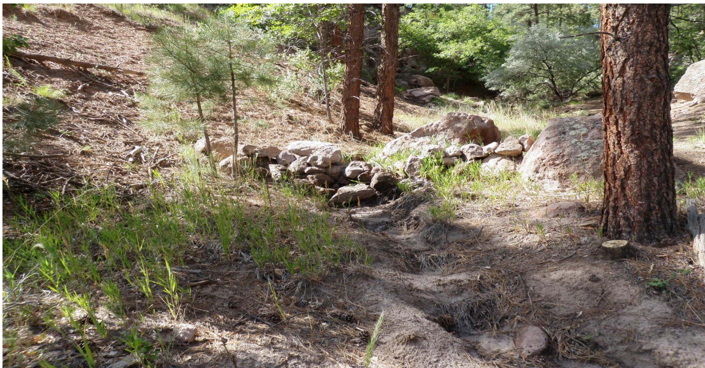
Photo 7412-2.JPG (taken 07/29/10) B00206010003 : Check Dam - Rock Check Dam.
