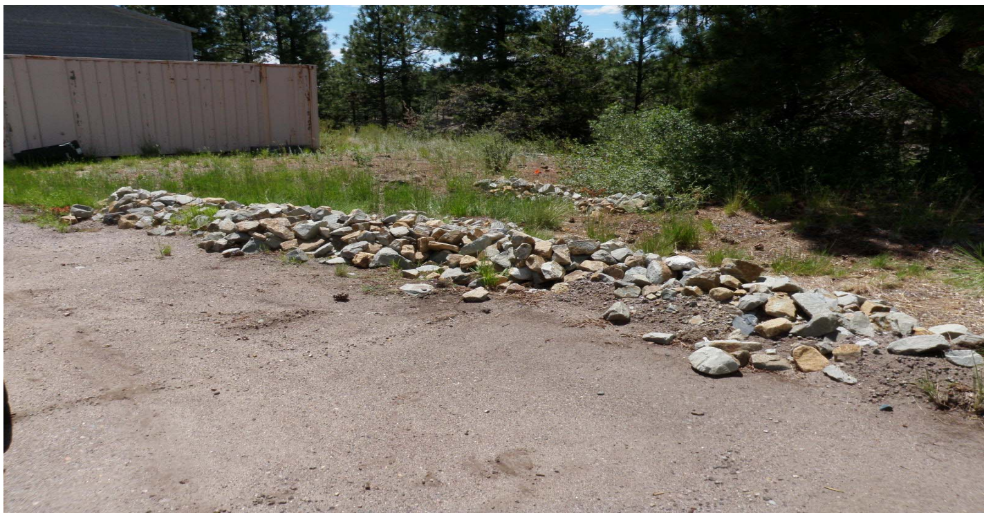
Photo 7453-1.JPG (taken 08/04/10) S00906010007 : Check Dam - Rock Check Dam.
