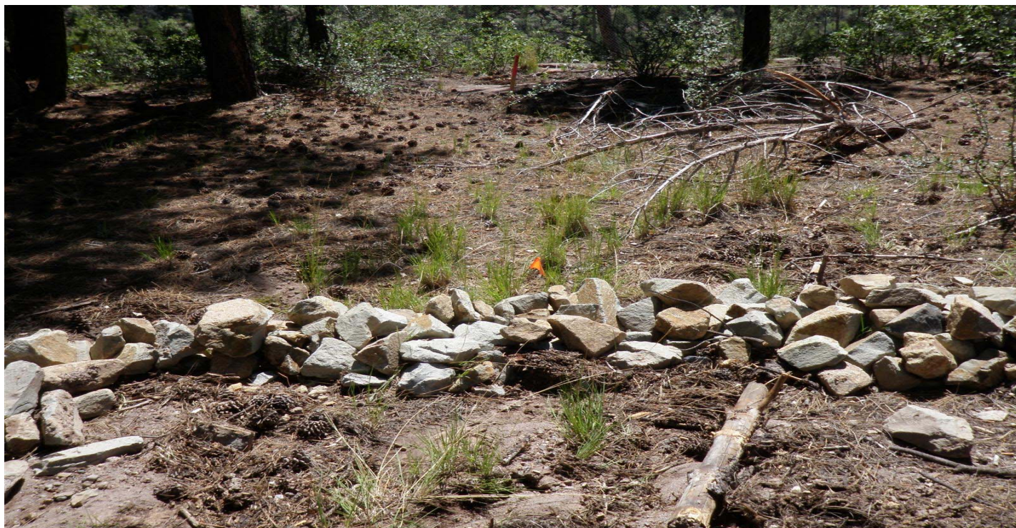
Photo 8512-1r.JPG (taken 08/20/10) S00906010004 : Check Dam - Rock Check Dam.
