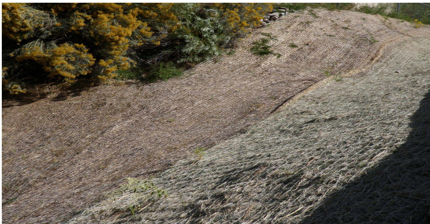
Photo 10550-04r.JPG (taken 09/20/10) M00801060015 : Seed and Mulch - Erosion Control Blanket.
