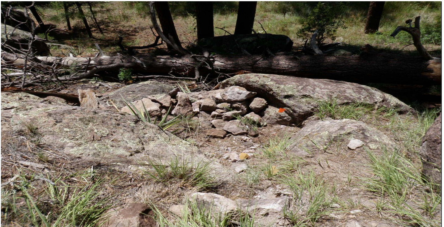
Photo 8655-1.JPG (taken 07/28/10) L02206010004 : Check Dam - Rock Check Dam.
