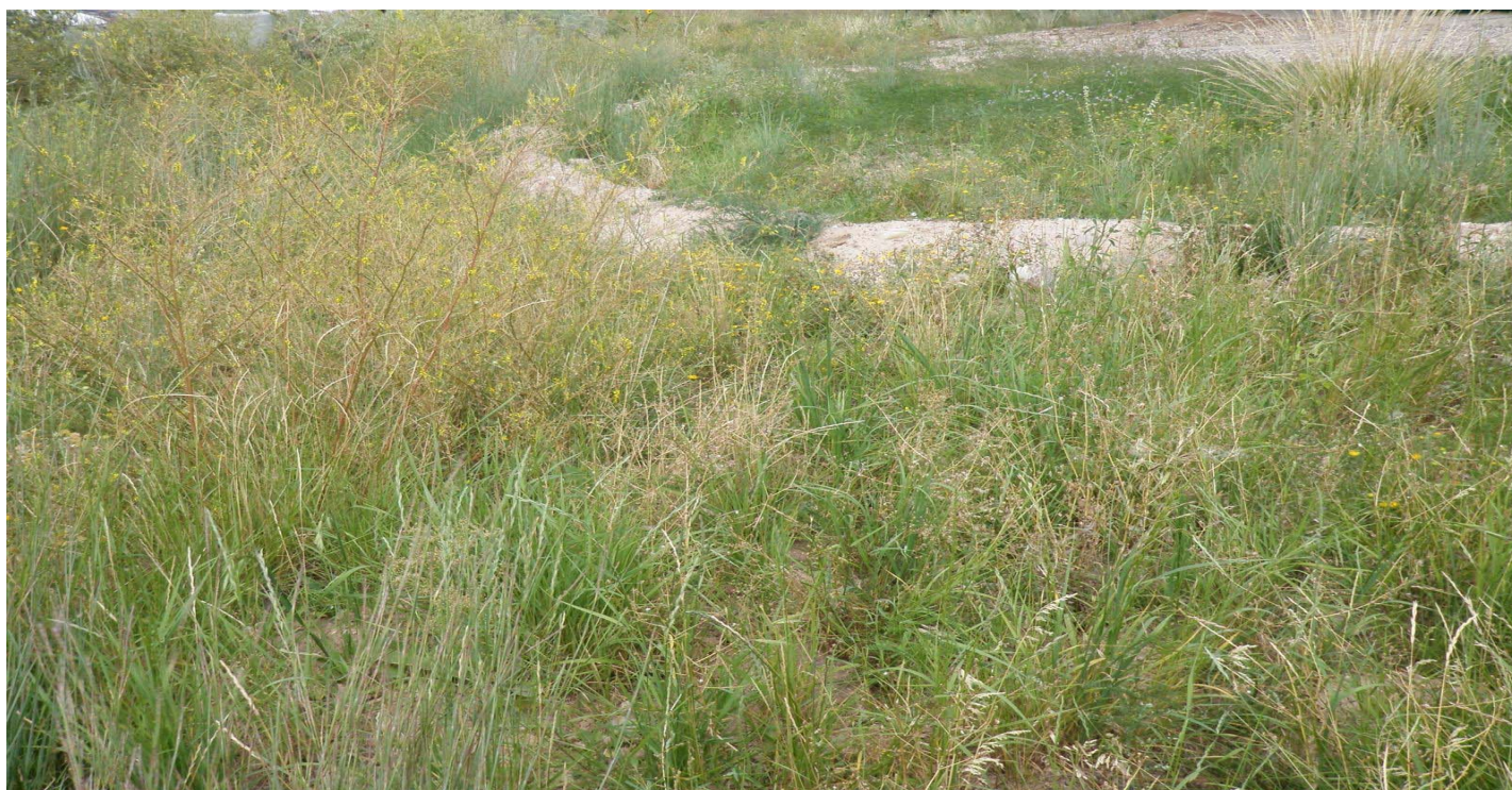
Photo 10553-1r.JPG (taken 09/08/10) S003A03010004 : Berms - Earthen Berm.
