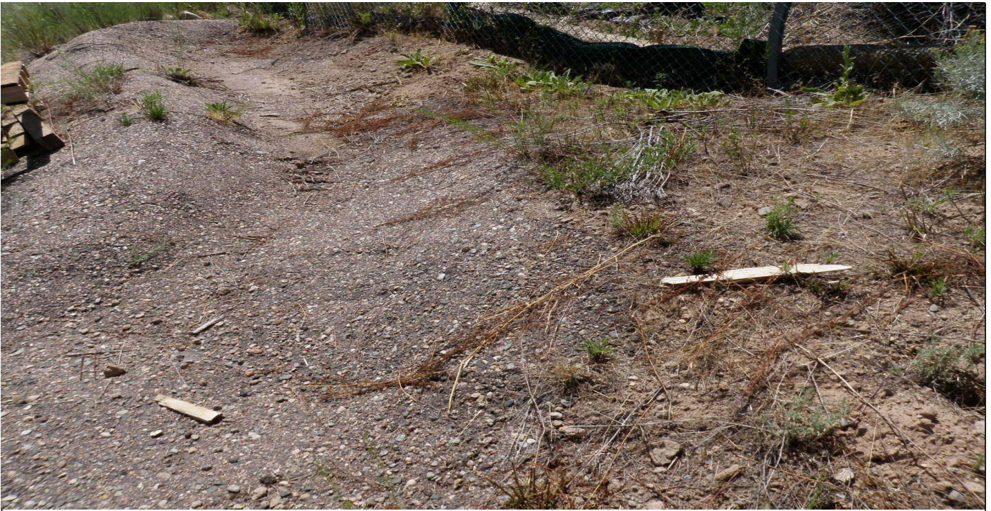
Photo 8656-7.JPG (taken 07/29/10) D00404020005 : Channel/Swale - Concrete/Asphalt Channel/Swale.
