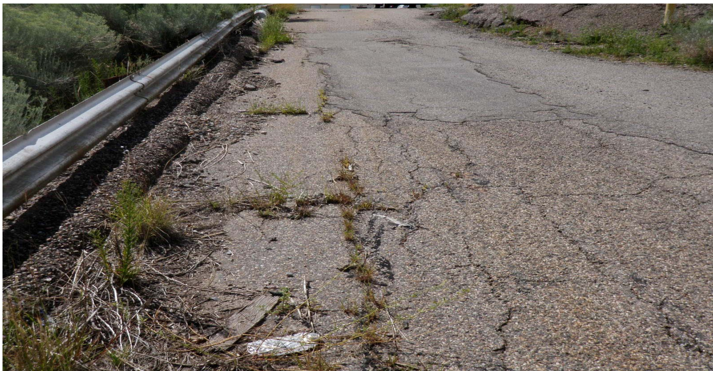
Photo 7452-13.JPG (taken 08/04/10) T00103090004 : Berms - Curbing.
