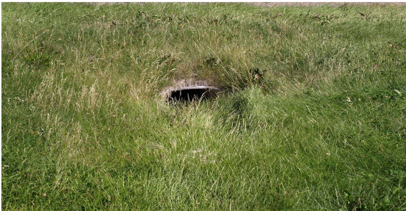
Photo 10553-4.JPG (taken 09/08/10) S003A02030005 : Established Vegetation - Permanent Vegetation Vegetative Buffer Strip.
