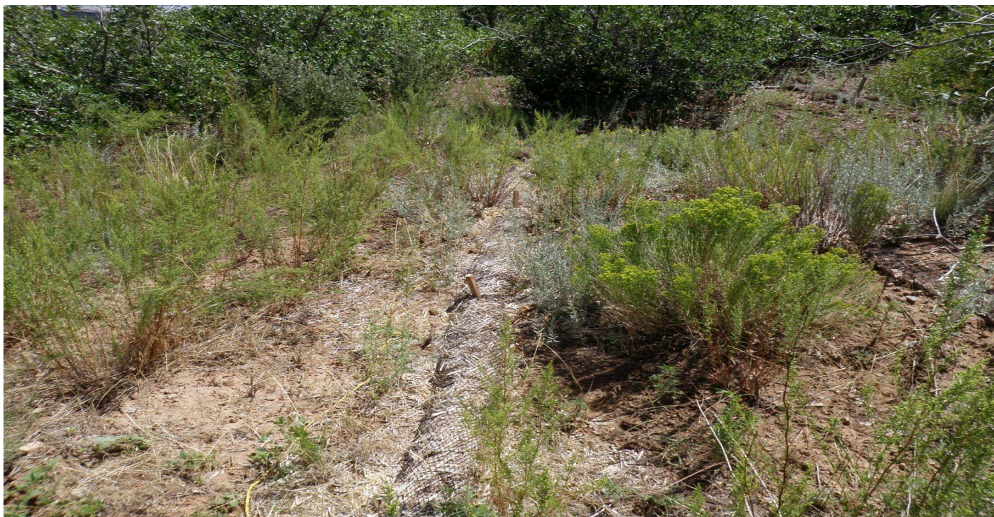
Photo 7479-2r.JPG (taken 08/10/10) M01803060006 : Berms - Straw Wattles.
