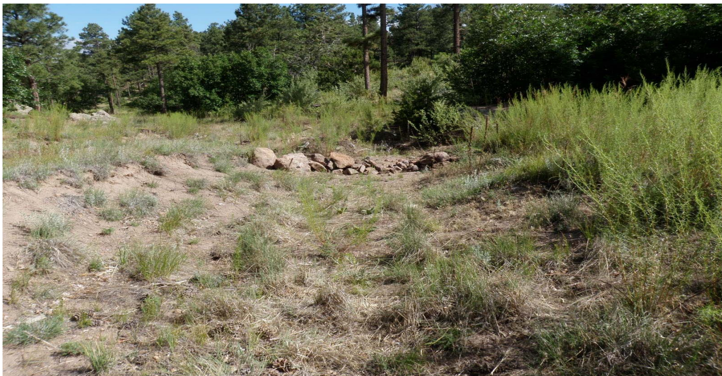
Photo 7412-6.JPG (taken 07/29/10) B00206010007 : Check Dam - Rock Check Dam.
