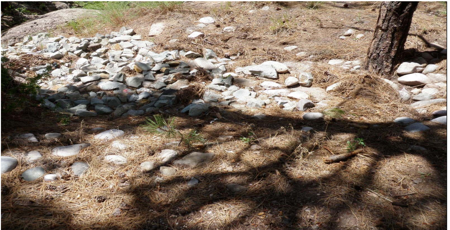
Photo 7410-1.JPG (taken 07/30/10) P002A04060002 : Channel/Swale - Rip Rap.
