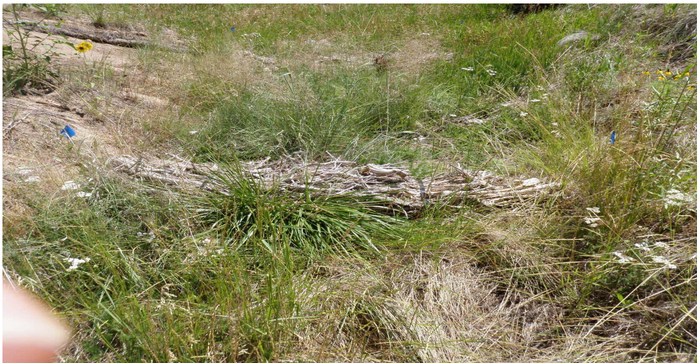
Photo 8656-3.JPG (taken 07/29/10) D00406030006 : Check Dam - Juniper Bales.
