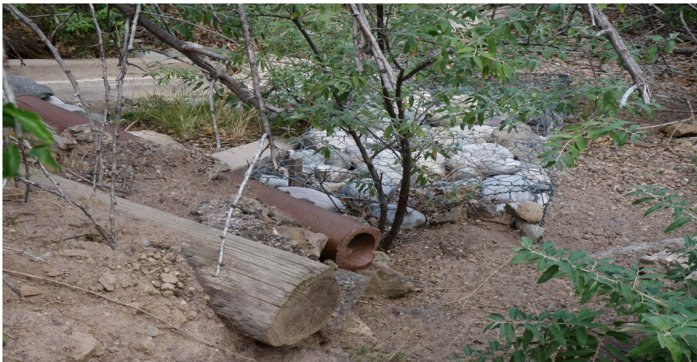
Photo 7458-5.JPG (taken 08/04/10) T00607010003 : Gabions - Gabions.
