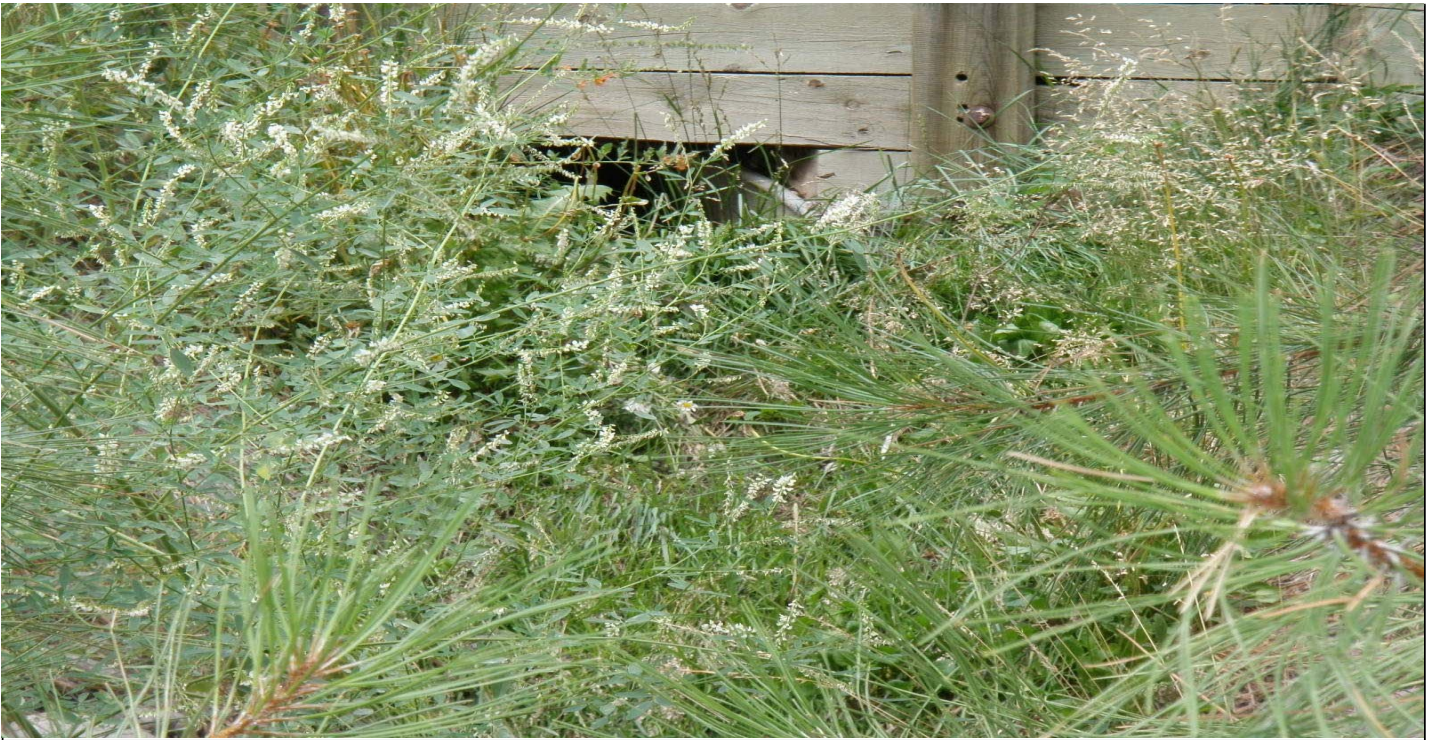
Photo 7423-3.JPG (taken 07/28/10) L00904040002 : Channel/Swale - Culvert.
