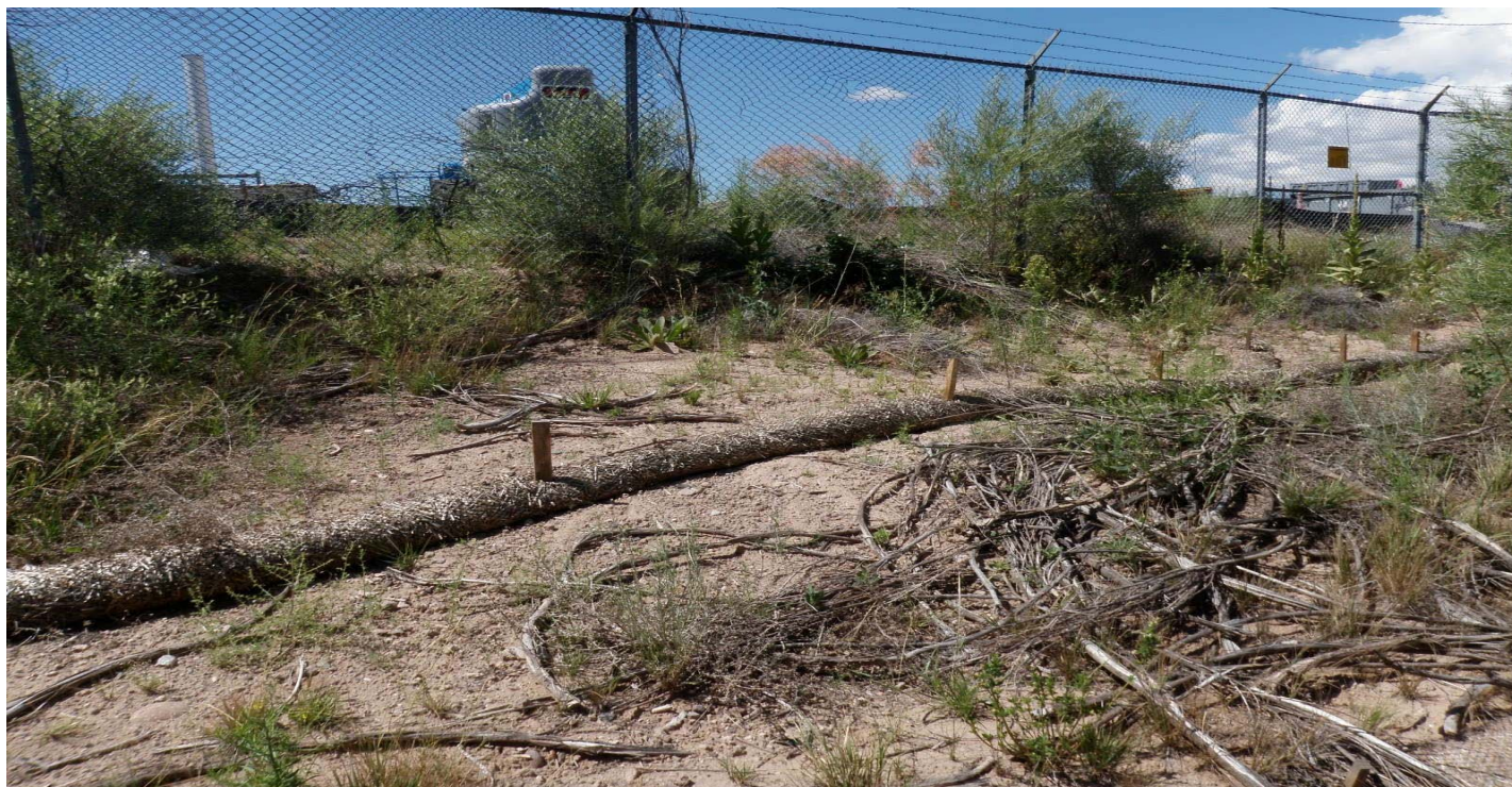
Photo 7415-1.JPG (taken 07/29/10) D00603060003 : Berms - Straw Wattles.
