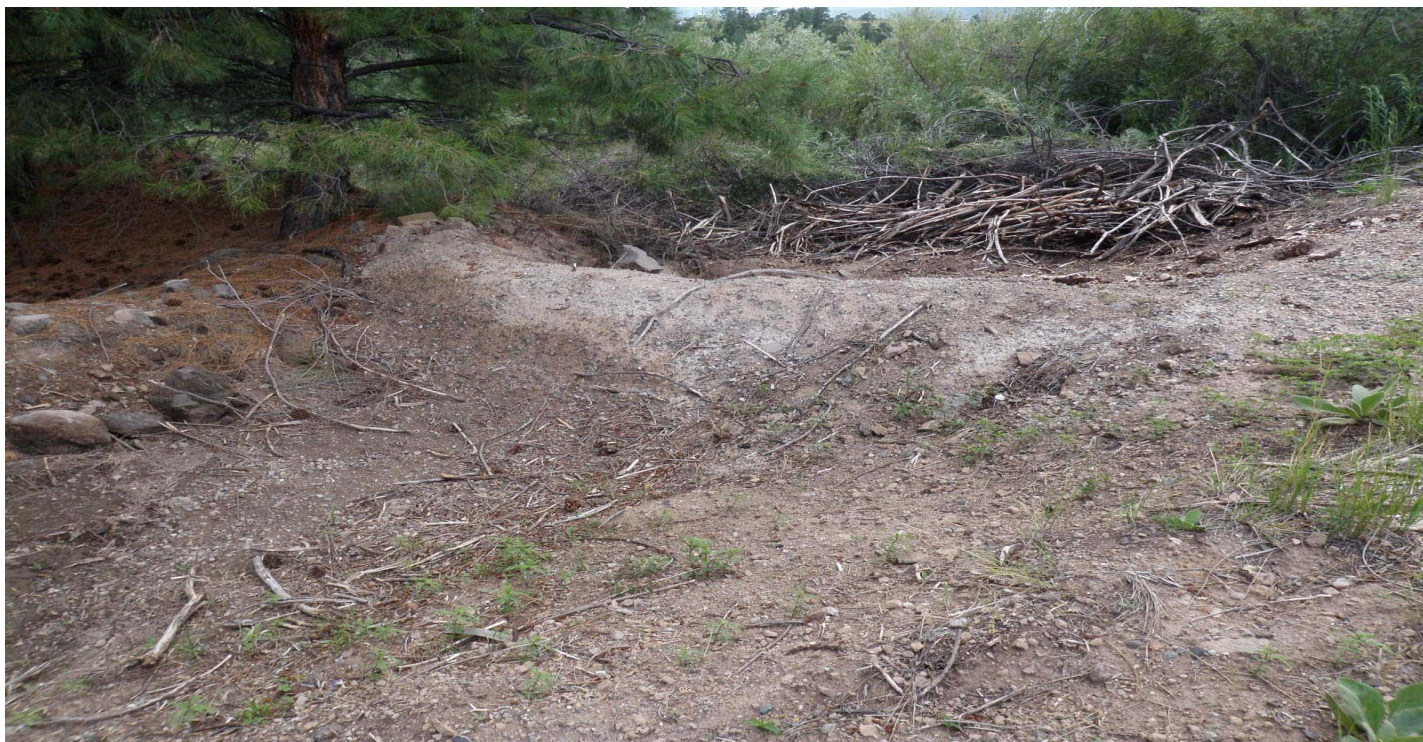
Photo 7450-5.JPG (taken 08/04/10) T00703020003 : Berms - Base Course Berm.
