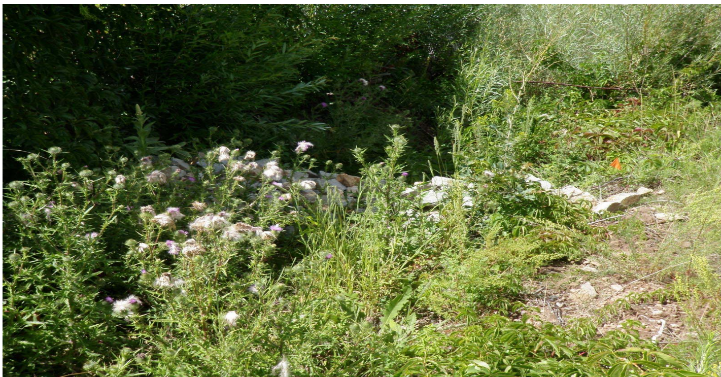
Photo 8501-4r.JPG (taken 08/19/10) S00506010007 : Check Dam - Rock Check Dam.
