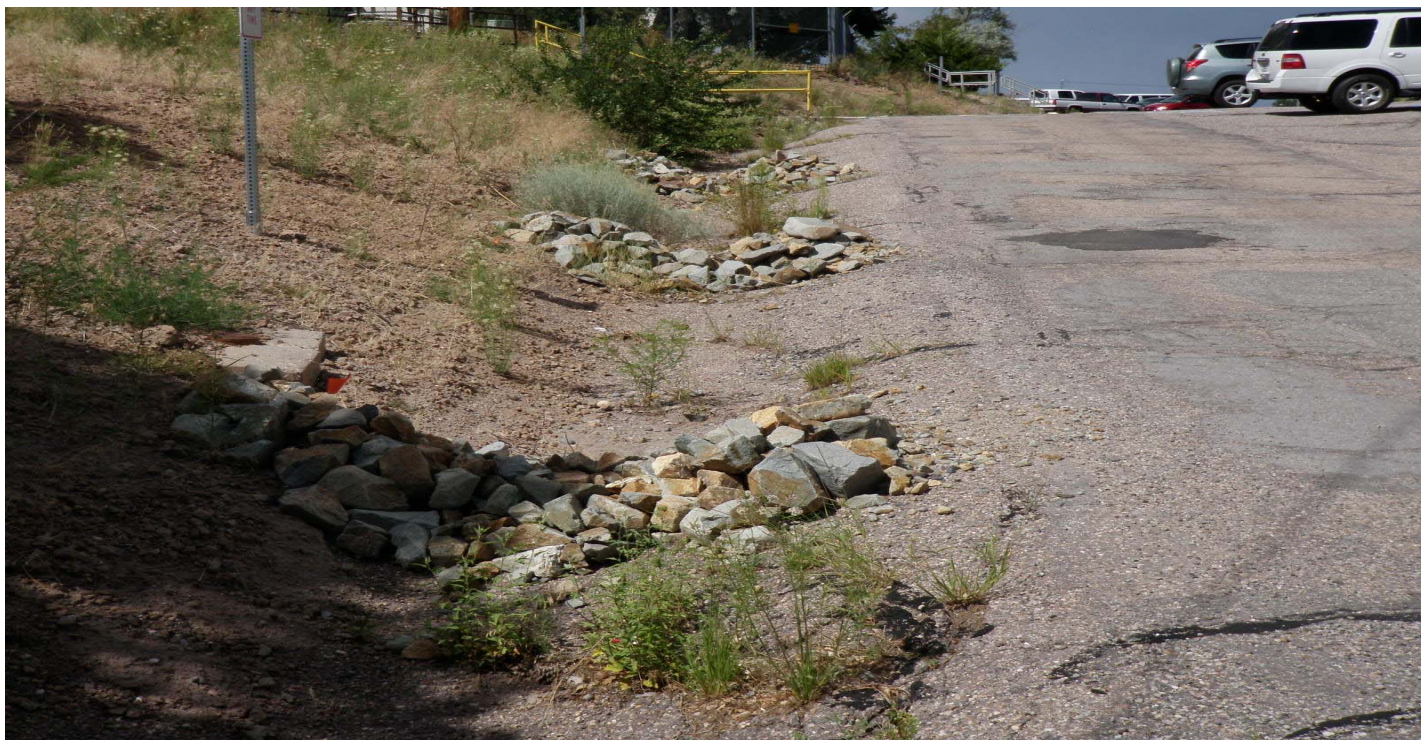
Photo 7458-7.JPG (taken 08/04/10) T00606010006 : Check Dam - Rock Check Dam; T00606010007 : Check Dam - Rock Check Dam; T00606010008 : Check Dam - Rock Check Dam.
