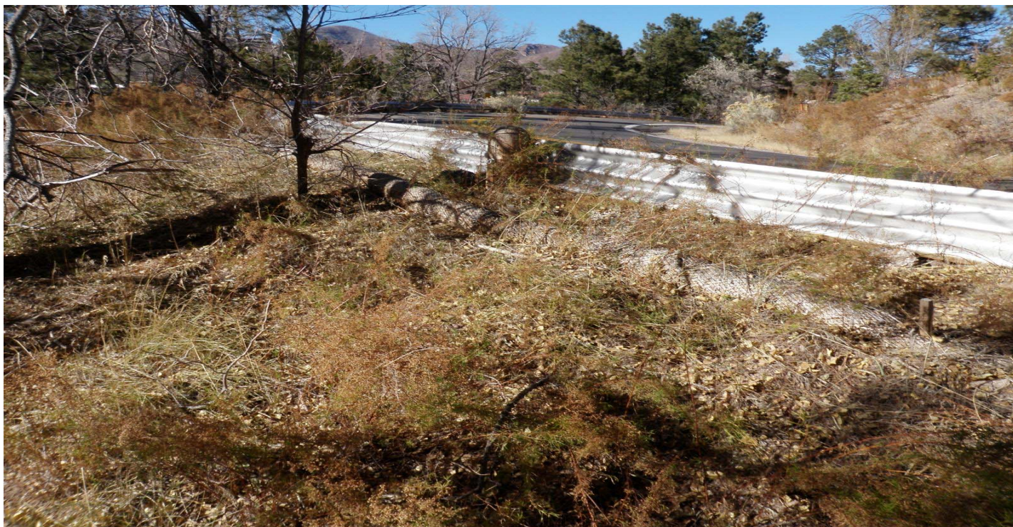
Photo 11806-1r.JPG (taken 07/28/10) L00303060006 : Berms - Straw Wattles; L00303060007 : Berms - Straw Wattles.
