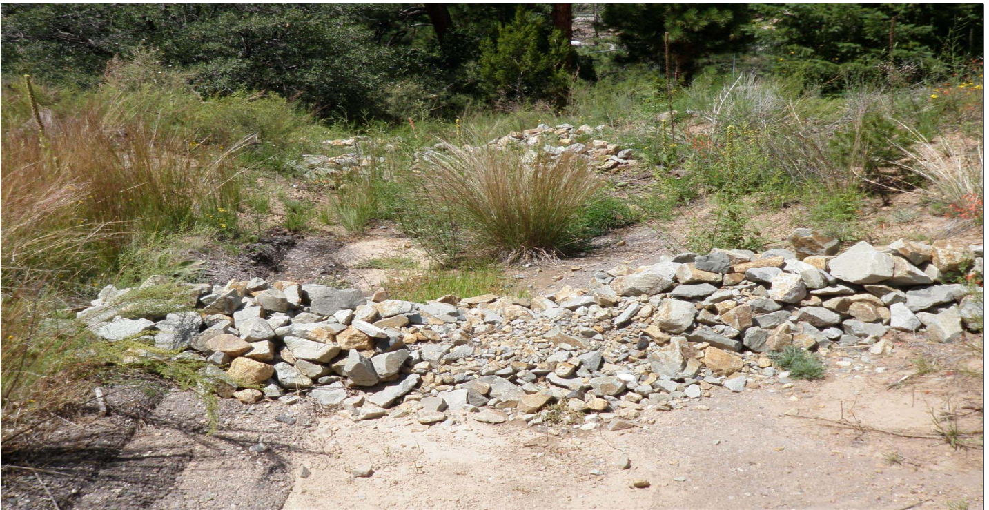
Photo 8515-2r.JPG (taken 08/19/10) S00806010008 : Check Dam - Rock Check Dam; S00806010009 : Check Dam - Rock Check Dam; S00806010010 : Check Dam - Rock Check Dam.
