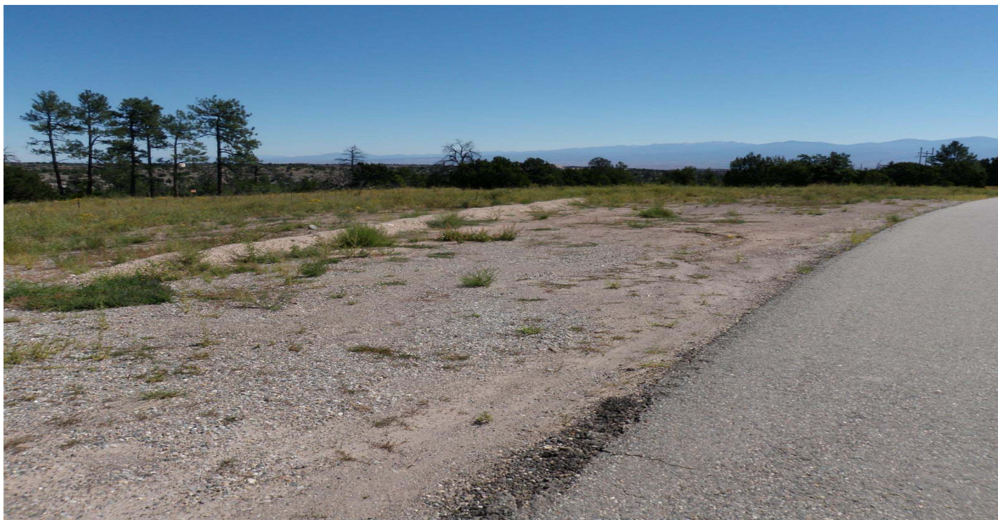
Photo 8664-2r.JPG (taken 09/02/10) T01003020005 : Berms - Base Course Berm.
