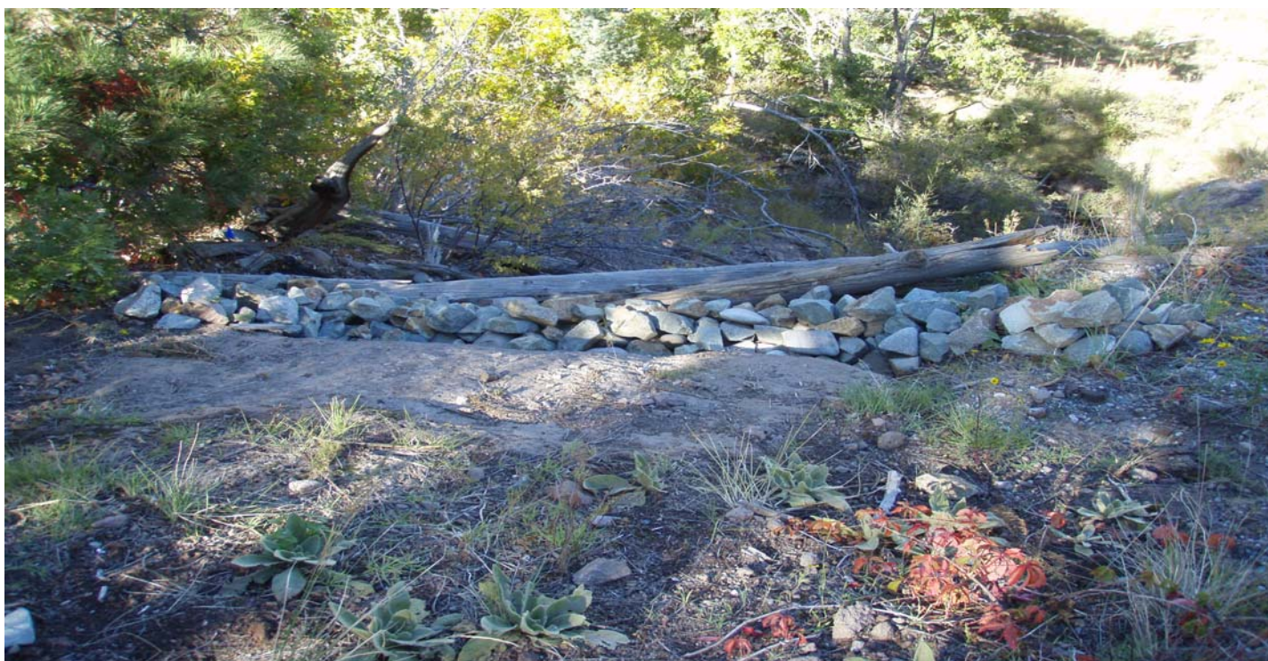
Photo 10869-3.JPG (taken 10/08/10) S005B03120005 : Berms - Rock Berm.
