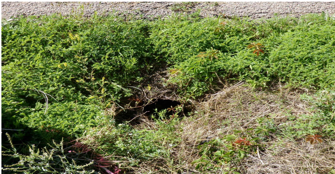
Photo 7434-4.JPG (taken 07/29/10) L02504040005 : Channel/Swale - Culvert.
