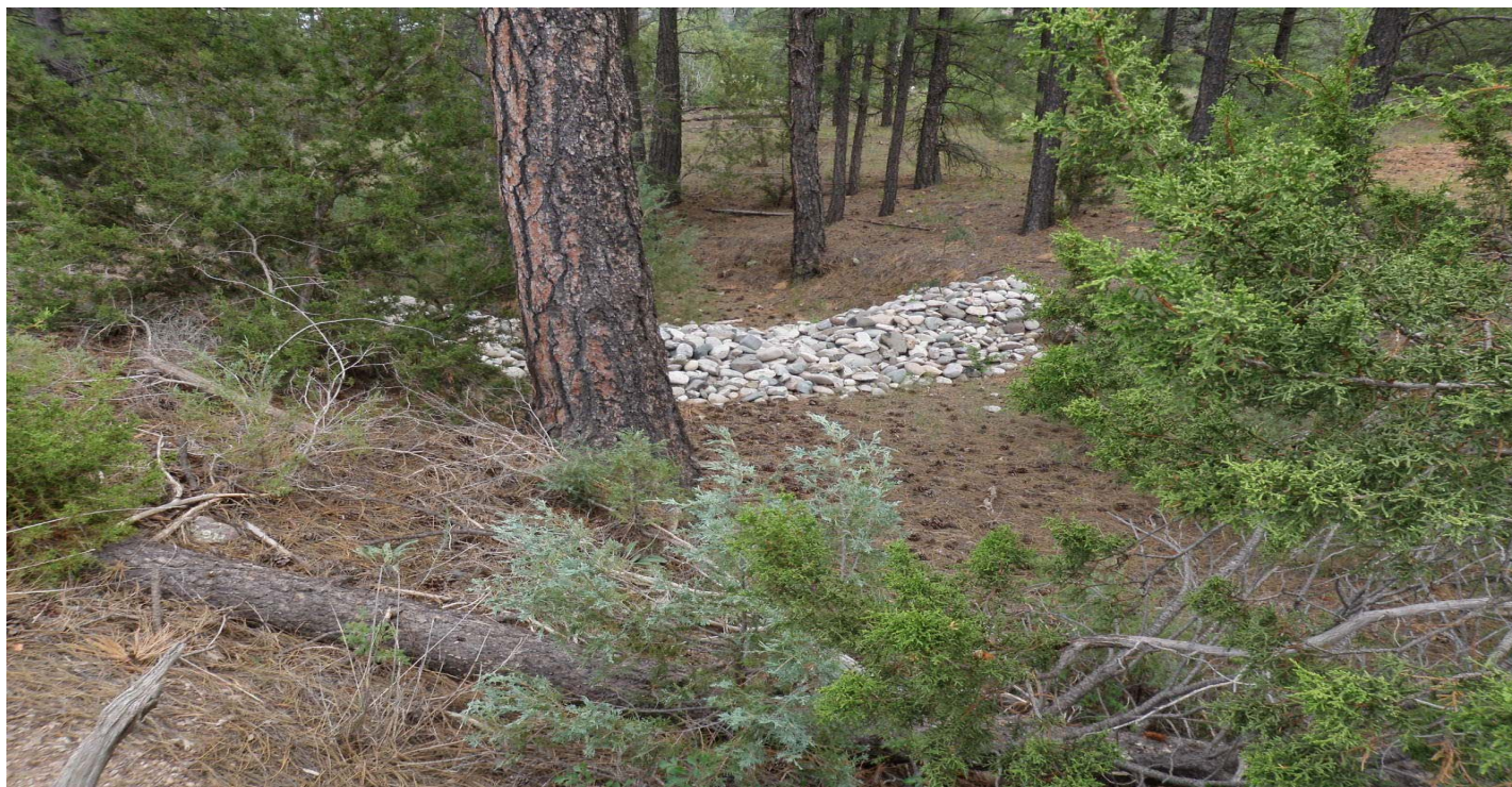
Photo 7446-1.JPG (taken 07/30/10) R00606010003 : Check Dam - Rock Check Dam.
