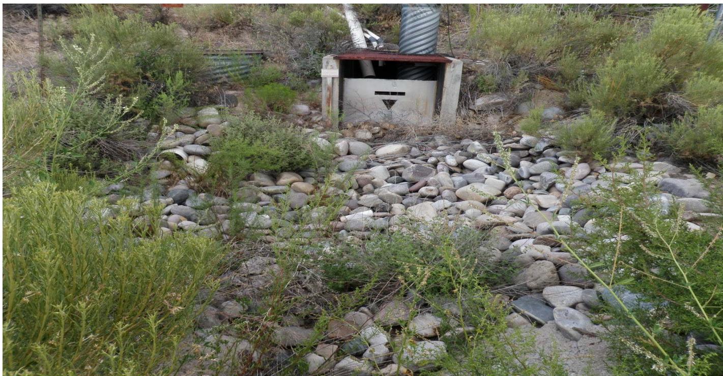
Photo 7439-2.JPG (taken 07/29/10) L03004060003 : Channel/Swale - Rip Rap.
