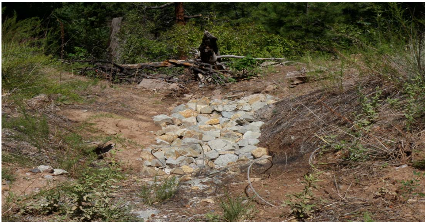
Photo 7466-1.JPG (taken 08/06/10) M01204060004 : Channel/Swale - Rip Rap.
