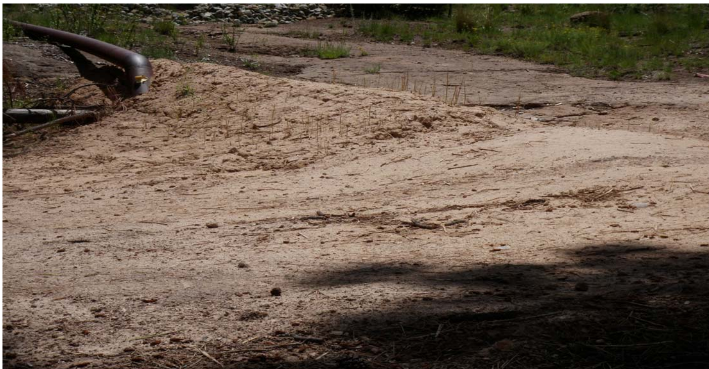
Photo 7465-5.JPG (taken 08/06/10) M01003010004 : Berms - Earthen Berm.
