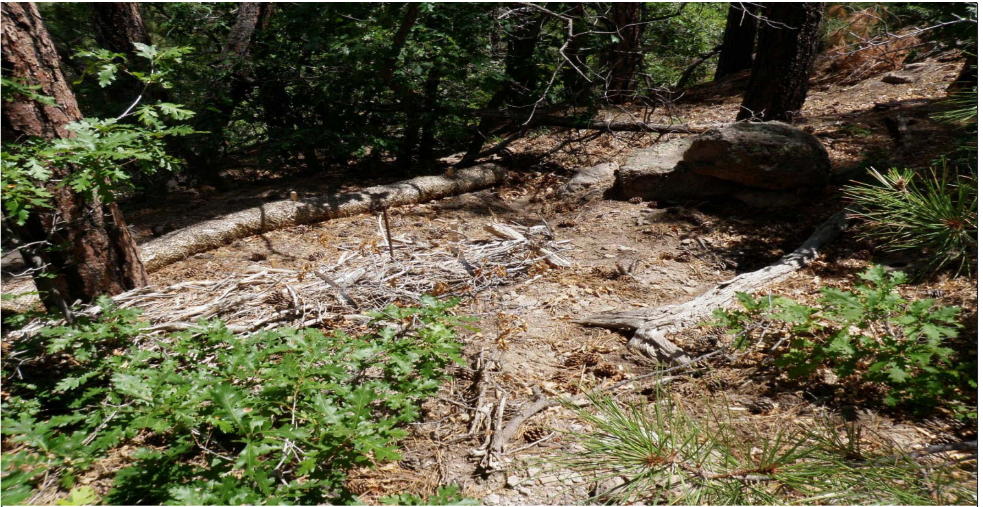
Photo 7413-3.JPG (taken 07/29/10) D00203060005 : Berms - Straw Wattles; D00206030004 : Check Dam - Juniper Bales.
