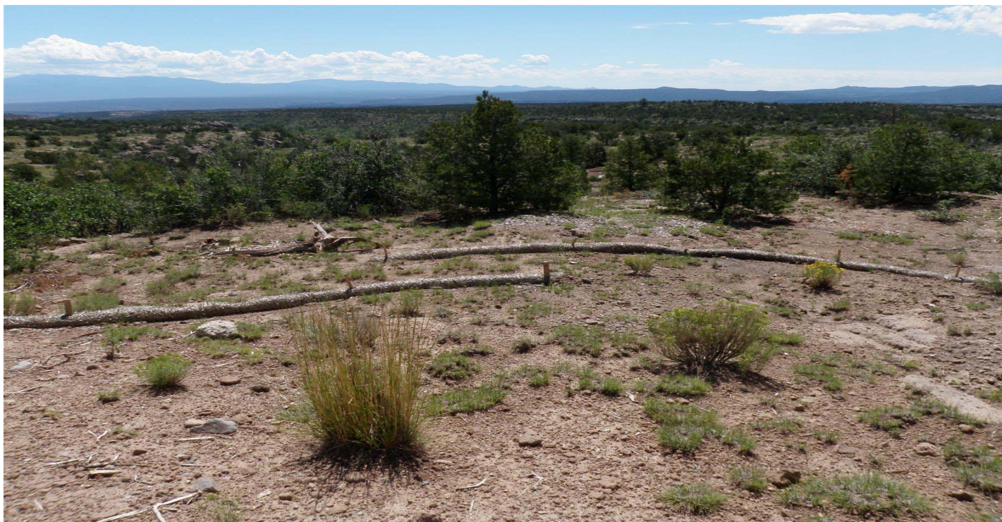
Photo 7476-3r.JPG (taken 08/10/10) M02203060005 : Berms - Straw Wattles; M02203060006 : Berms - Straw Wattles.
