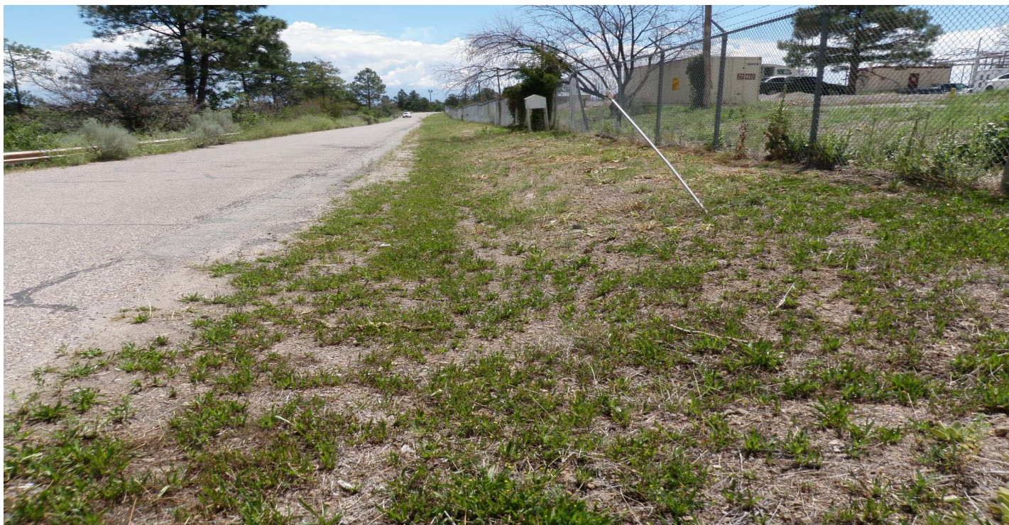
Photo 7413-1.JPG (taken 07/29/10) D00204010002 : Channel/Swale - Earthen Channel/Swale.
