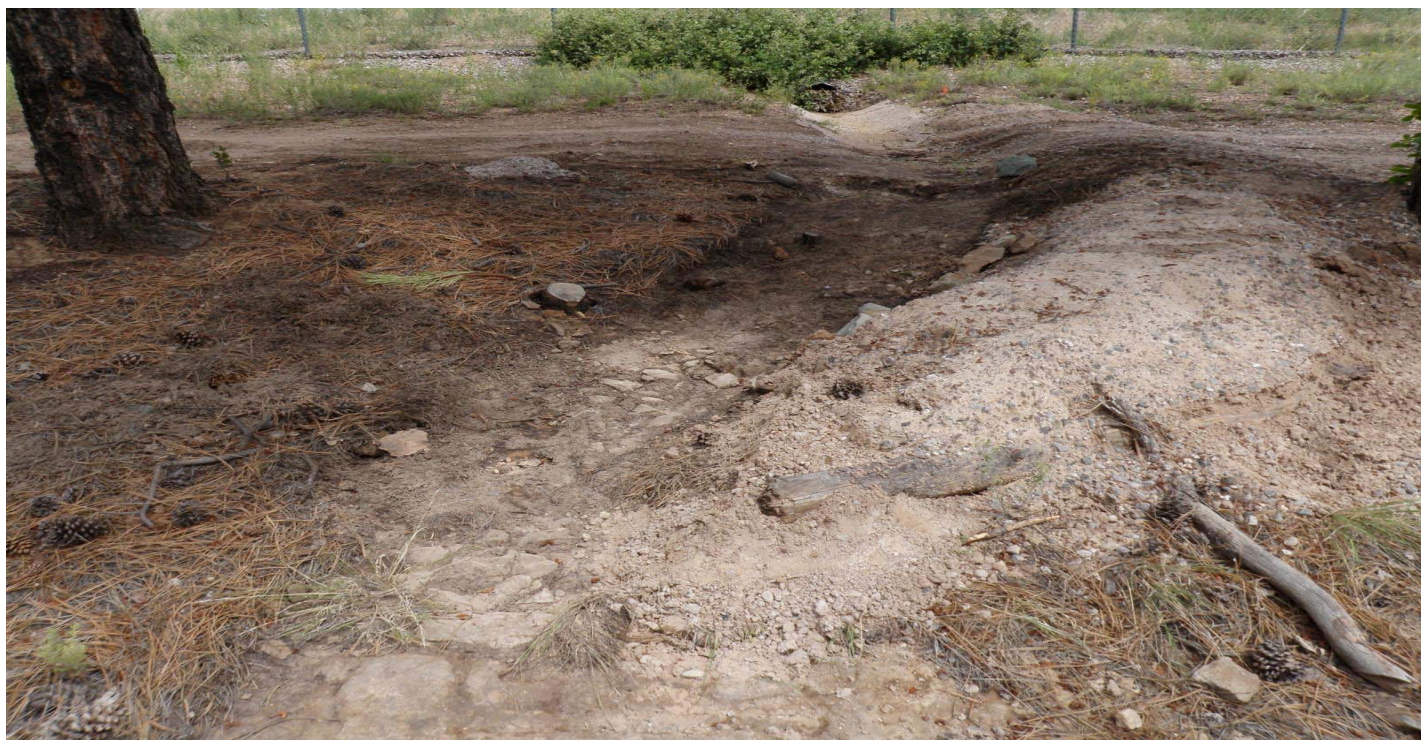
Photo 7494-1r.JPG (taken 08/09/10) M002A03020002 : Berms - Base Course Berm.
