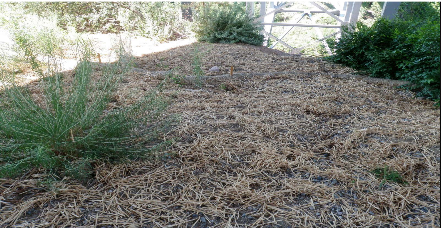
Photo 7418-3.JPG (taken 07/28/10) L00301010009 : Seed and Mulch - Seed and Wood Mulch; L00303060008 : Berms - Straw Wattles.
