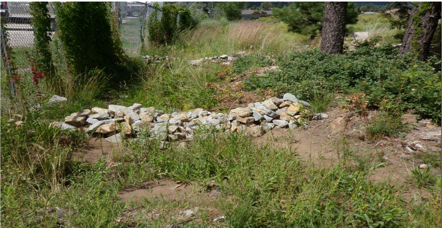
Photo 8501-2r.JPG (taken 08/19/10) S00506010009 : Check Dam - Rock Check Dam; S00506010010 : Check Dam - Rock Check Dam.
