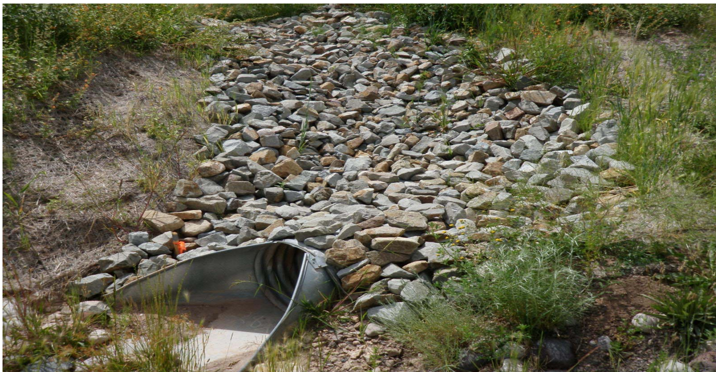
Photo 10553-2r.JPG (taken 09/08/10) S003A04060002 : Channel/Swale - Rip Rap.
