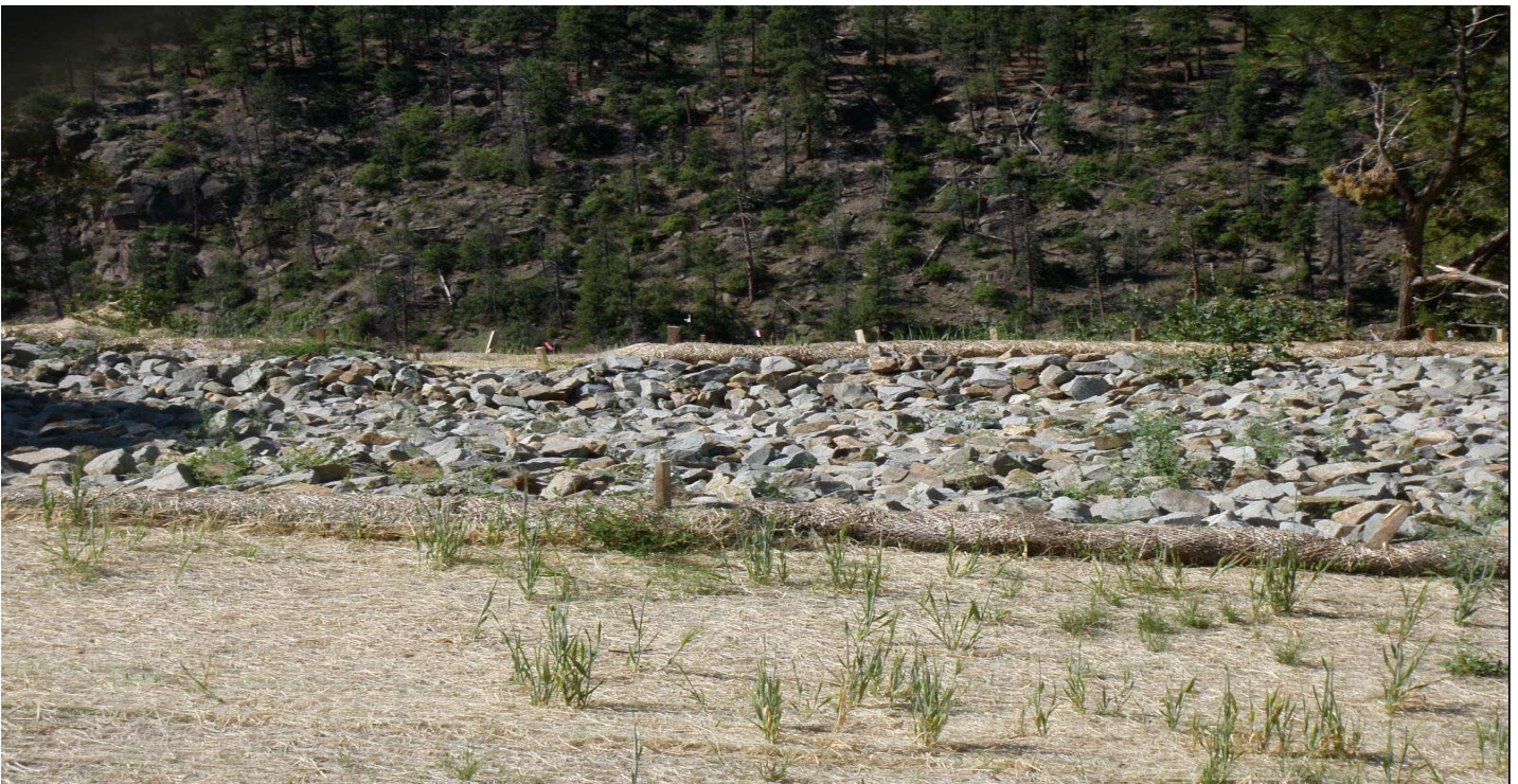
Photo 7435-3.JPG (taken 07/28/10) L02603060005 : Berms - Straw Wattles; L02604060006 : Channel/Swale - Rip Rap.
