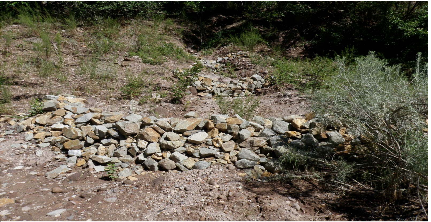
Photo 7418-6.JPG (taken 07/28/10) L00303120012 : Berms - Rock Berm; L00306010010 : Check Dam - Rock Check Dam; L00306010011 : Check Dam - Rock Check Dam.
