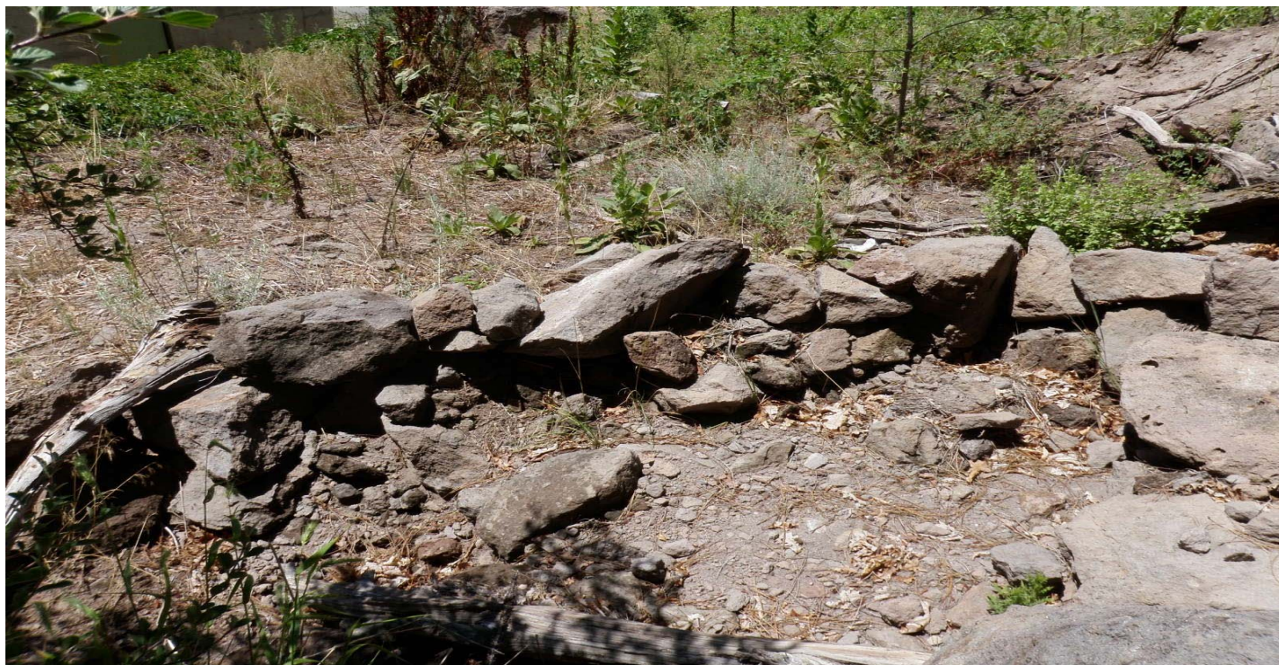
Photo 7426-1.JPG (taken 07/28/10) L01506010002 : Check Dam - Rock Check Dam.
