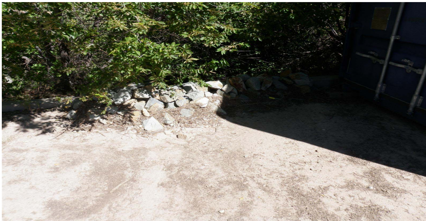
Photo 8669-1r.JPG (taken 09/02/10) S01106010004 : Check Dam - Rock Check Dam.
