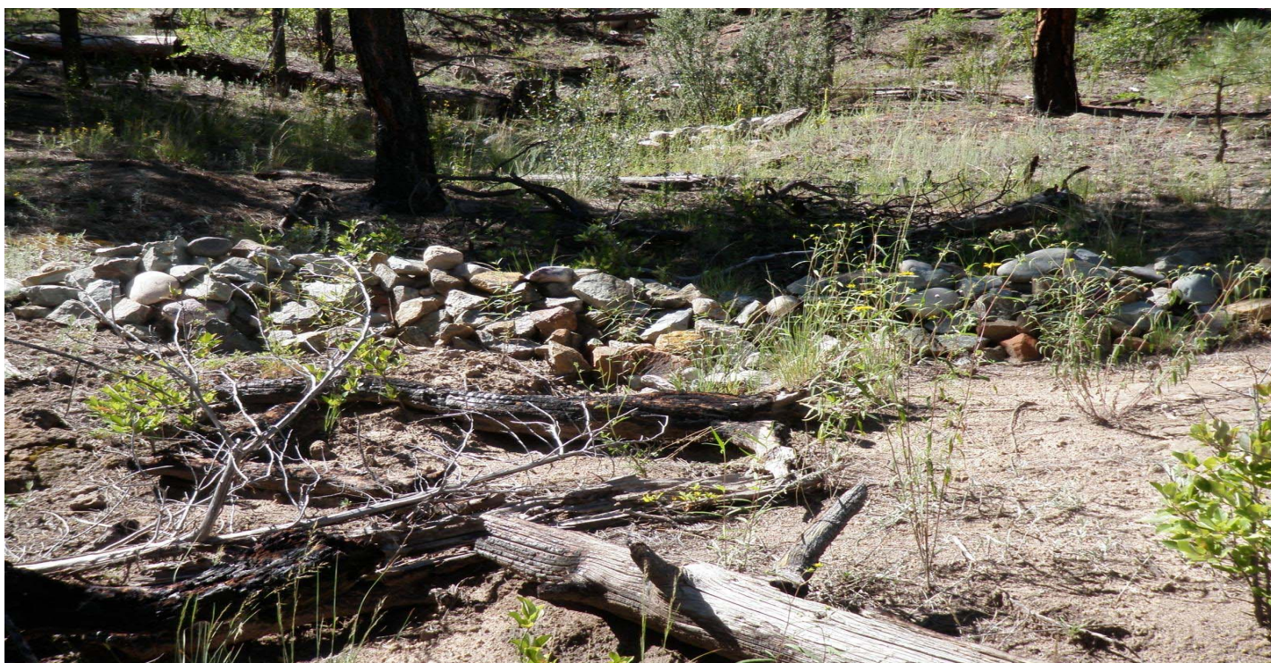
Photo 8665-2r.JPG (taken 09/02/10) T00906010003 : Check Dam - Rock Check Dam.
