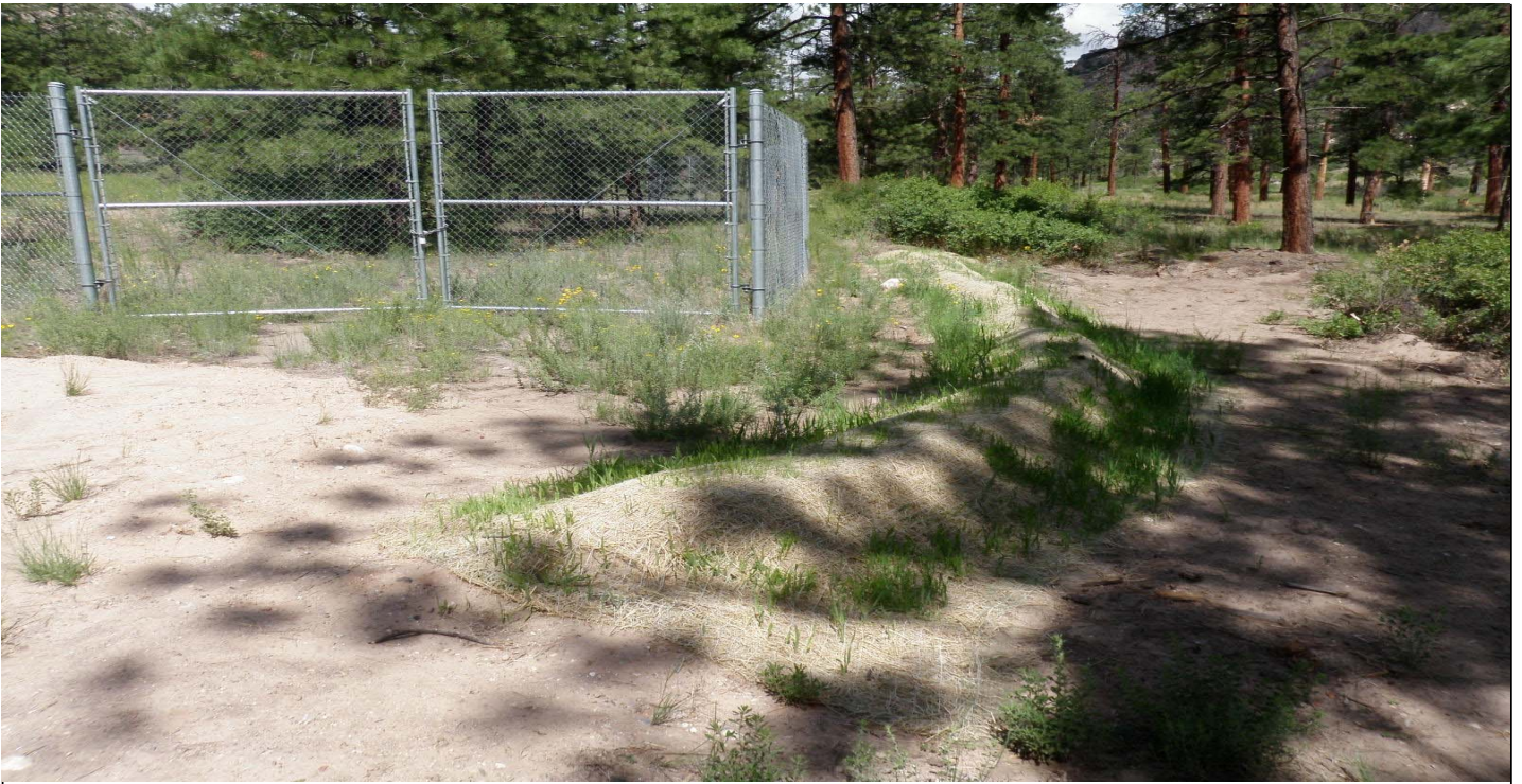
Photo 7411-1.JPG (taken 07/30/10) B00103010007 : Berms - Earthen Berm.
