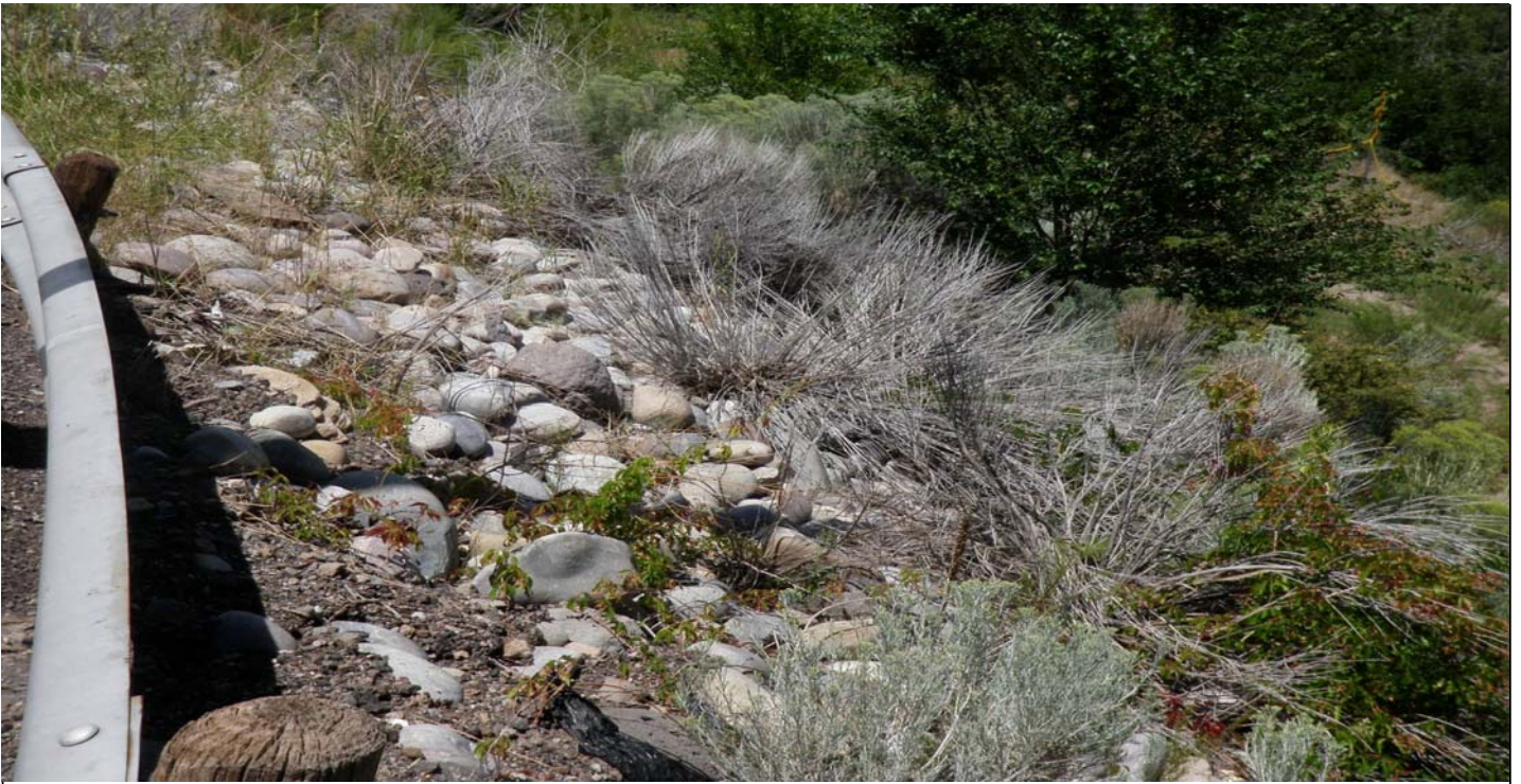
Photo 7463-2.JPG (taken 08/06/10) M01404060001 : Channel/Swale - Rip Rap.
