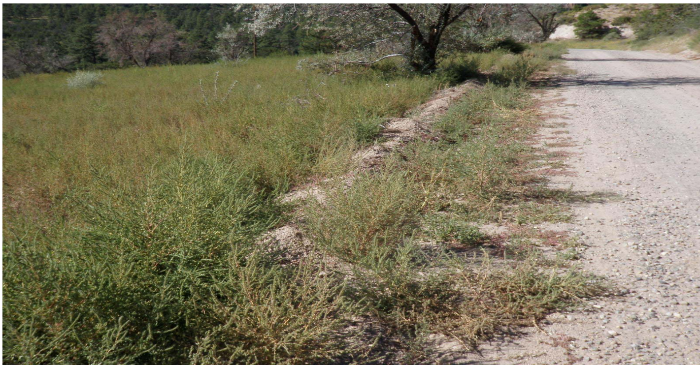
Photo 10560-6r.JPG (taken 09/14/10) P00403010002 : Berms - Earthen Berm.
