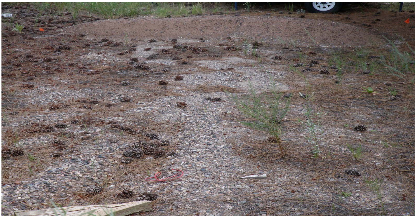
Photo 7450-3.JPG (taken 08/04/10) T00703020008 : Berms - Base Course Berm.
