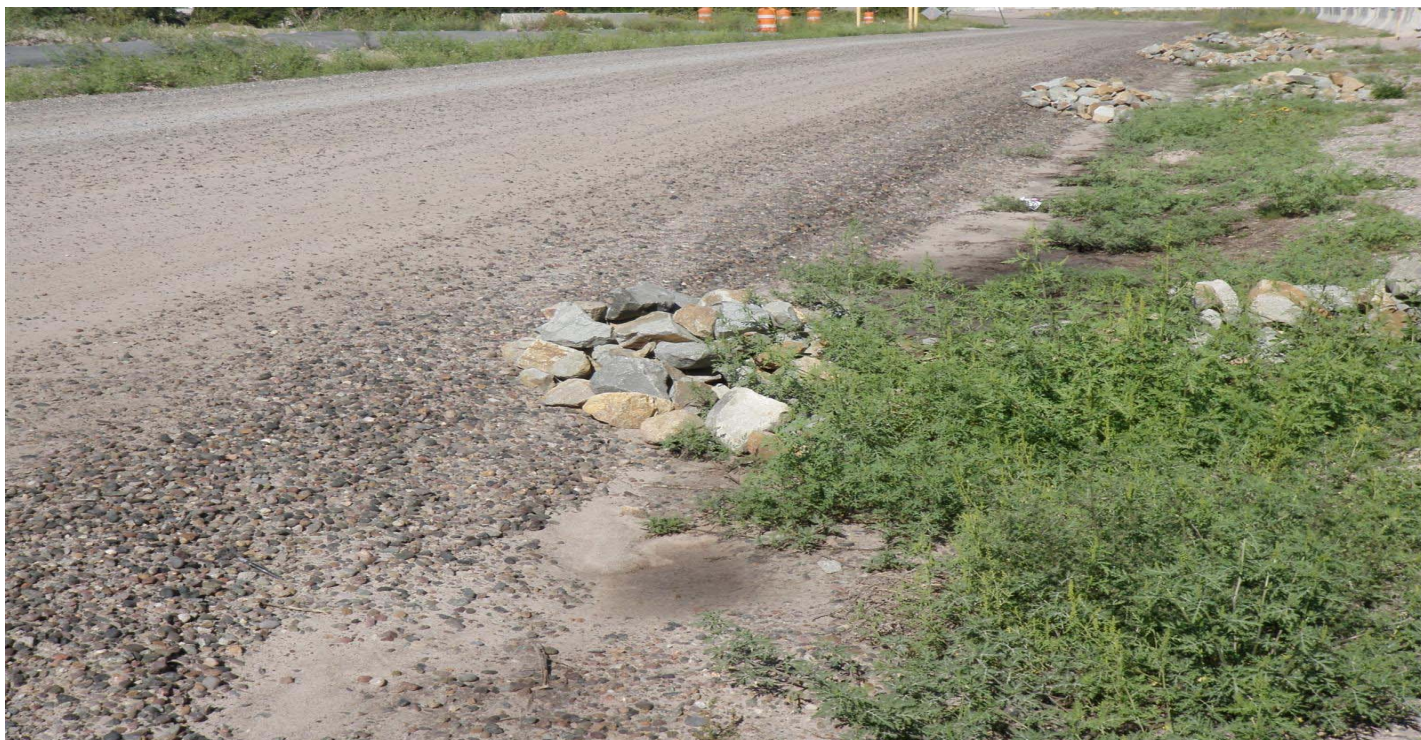
Photo 8509-3r.JPG (taken 08/20/10) C01006010008 : Check Dam - Rock Check Dam; C01006010009 : Check Dam - Rock Check Dam; C01006010010 : Check Dam - Rock Check Dam; C01006010011 : Check Dam - Rock Check Dam.
