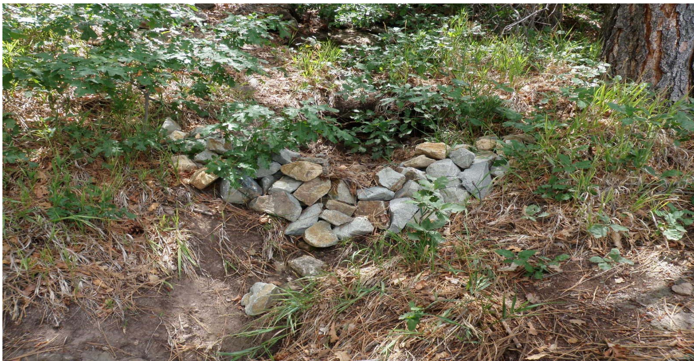
Photo 7460-4.JPG (taken 07/30/10) P00706010004 : Check Dam - Rock Check Dam.
