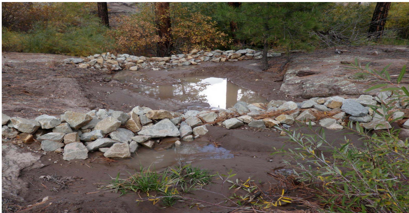
Photo 11026-2r.JPG (taken 10/21/10) M00806010011 : Check Dam - Rock Check Dam; M00806010012 : Check Dam - Rock Check Dam.
