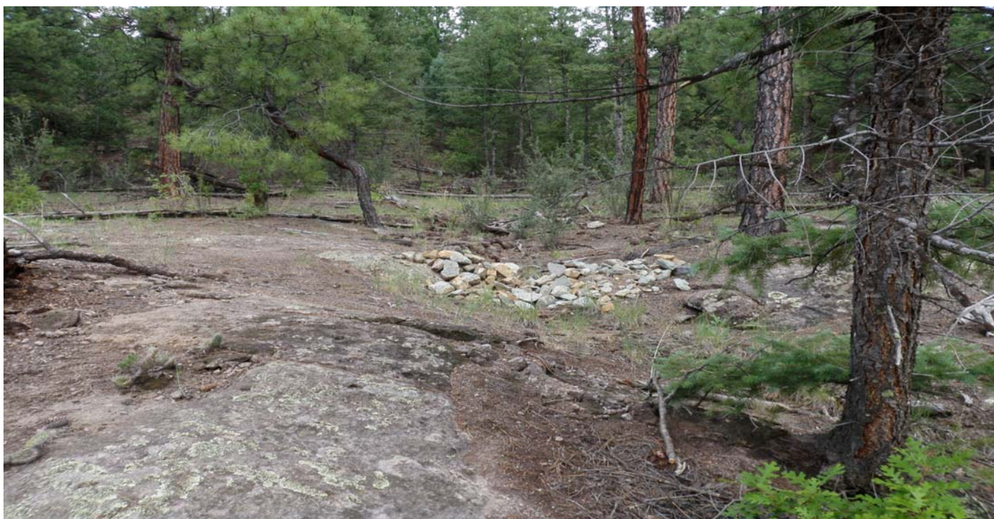
Photo 7464-3.JPG (taken 08/06/10) M012A06010003 : Check Dam - Rock Check Dam.
