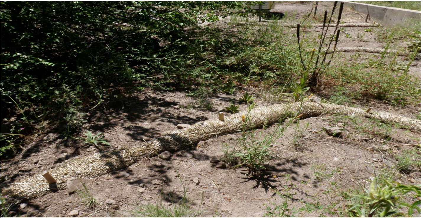
Photo 7426-4.JPG (taken 07/28/10) L01503060004 : Berms - Straw Wattles; L01503060005 : Berms - Straw Wattles; L01503060006 : Berms - Straw Wattles.
