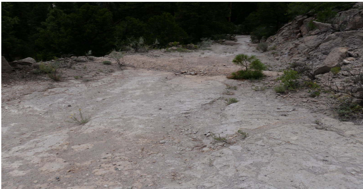
Photo 7452-05.JPG (taken 08/04/10) T00103020016 : Berms - Base Course Berm.
