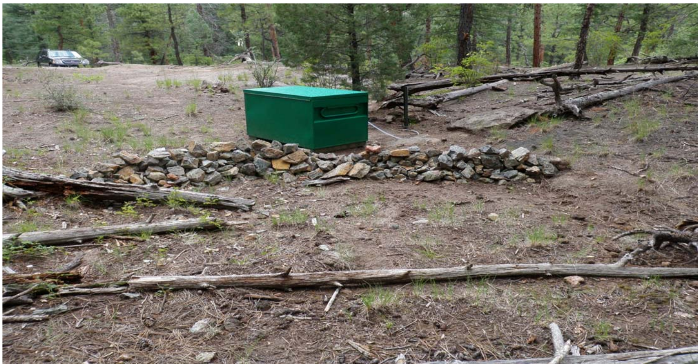
Photo 7466-5.JPG (taken 08/06/10) M01206010010 : Check Dam - Rock Check Dam.
