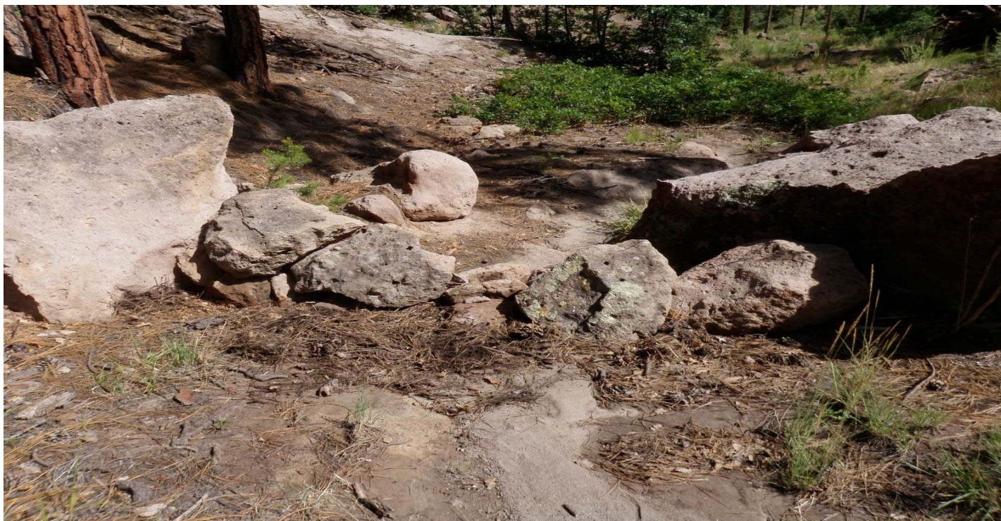
Photo 7412-3.JPG (taken 07/29/10) B00206010004 : Check Dam - Rock Check Dam.
