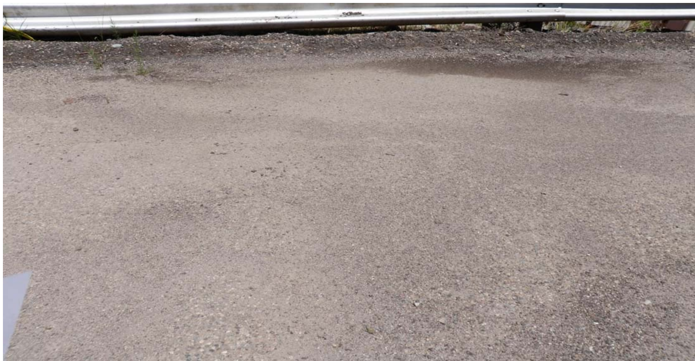
Photo 7463-1.JPG (taken 08/06/10) M01403090005 : Berms - Curbing.
