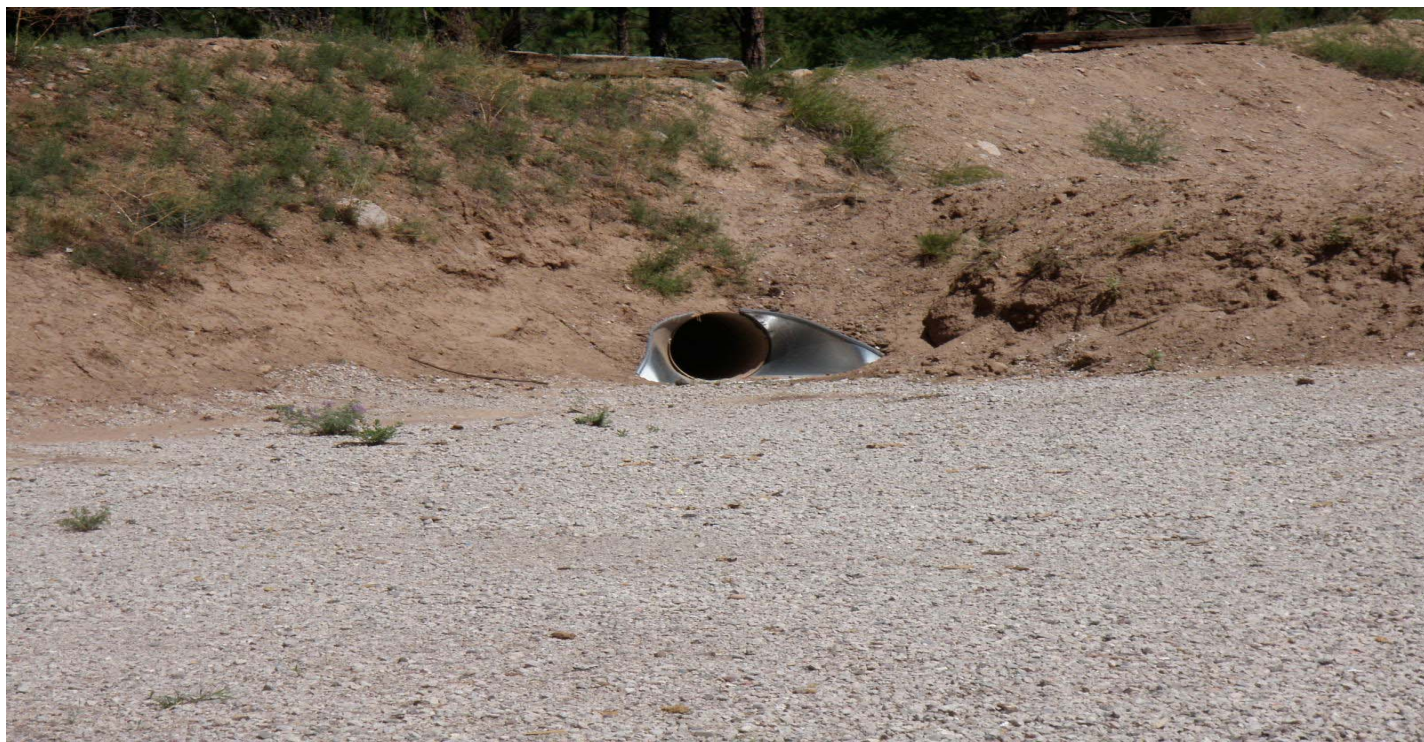
Photo 7442-4.JPG (taken 08/03/10) R00304040002 : Channel/Swale - Culvert.
