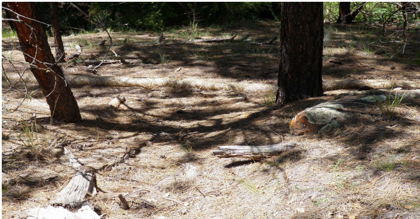
Photo 7435-1.JPG (taken 07/28/10) L02603060004 : Berms - Straw Wattles.
