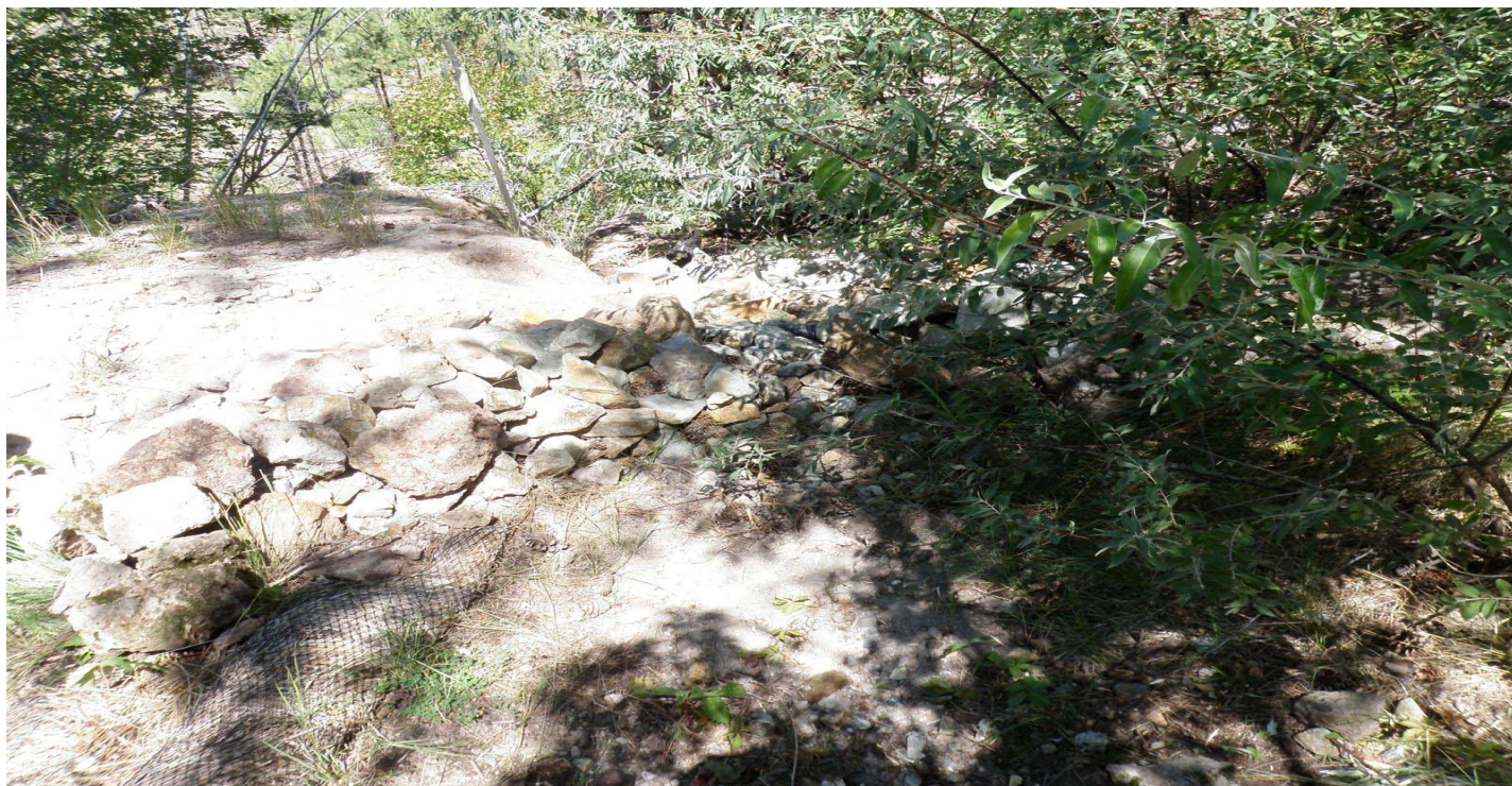
Photo 8511-2r.JPG (taken 08/20/10) M00406010004 : Check Dam - Rock Check Dam.
