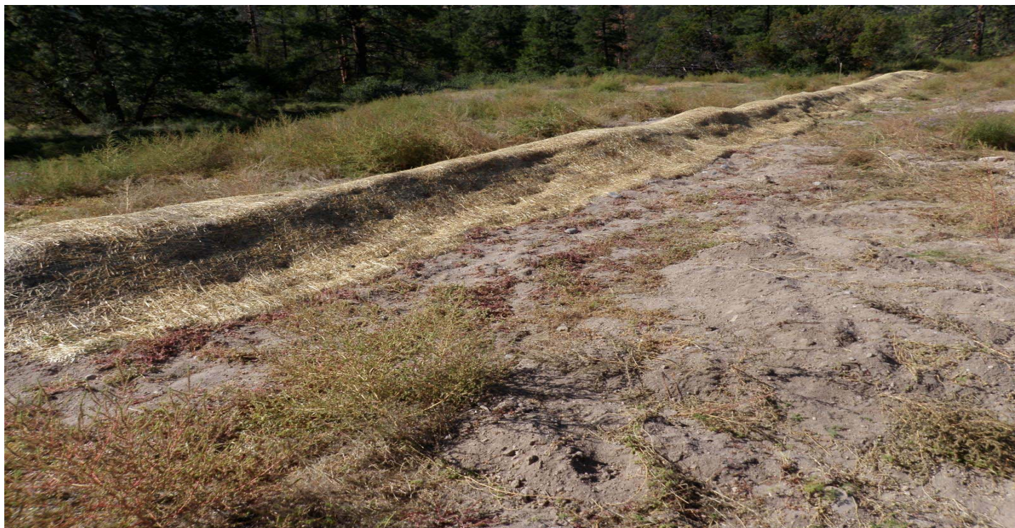
Photo 10560-1r.JPG (taken 09/14/10) P00403010006 : Berms - Earthen Berm.
