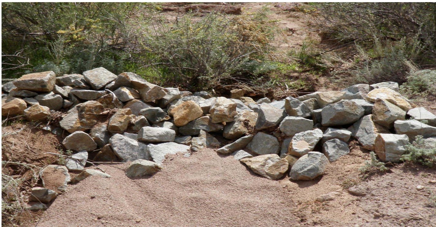
Photo 10886-1r.JPG (taken 10/06/10) S01406010012 : Check Dam - Rock Check Dam.
