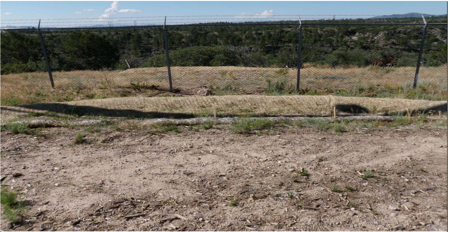
Photo 7434-2.JPG (taken 07/29/10) L02503010008 : Berms - Earthen Berm; L02503010009 : Berms - Earthen Berm.
