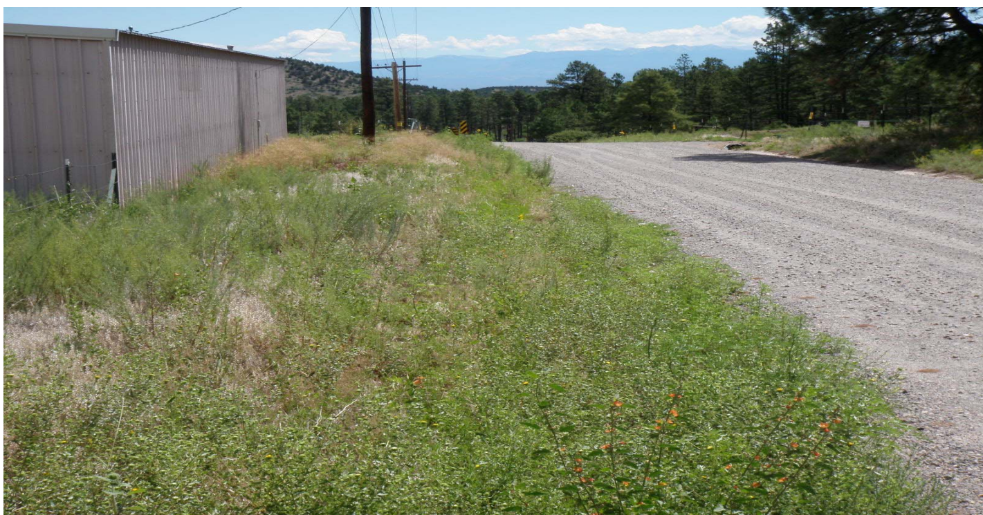
Photo 7442-3.JPG (taken 08/03/10) R00304010003 : Channel/Swale - Earthen Channel/Swale.
