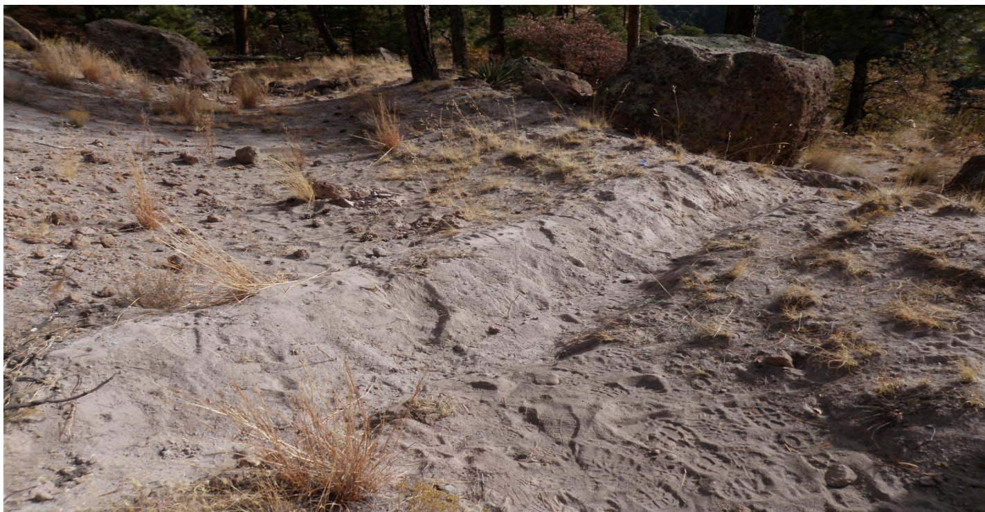
Photo 12128-2r.JPG (taken 12/06/10) L01204050009 : Channel/Swale - Water Bar.
