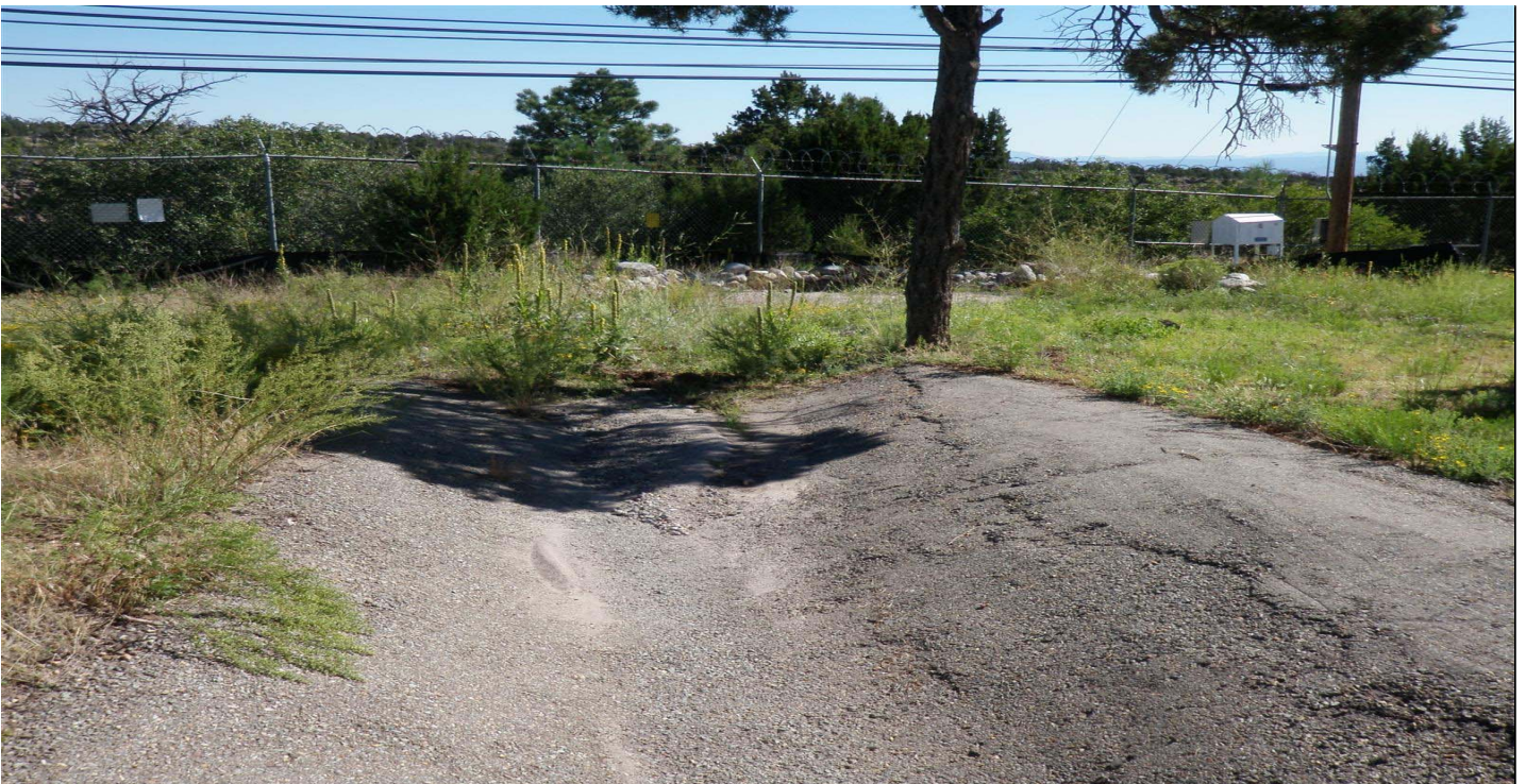
Photo 8509-2r.JPG (taken 08/20/10) C01004020005 : Channel/Swale - Concrete/Asphalt Channel/Swale; C01006010006 : Check Dam - Rock Check Dam.
