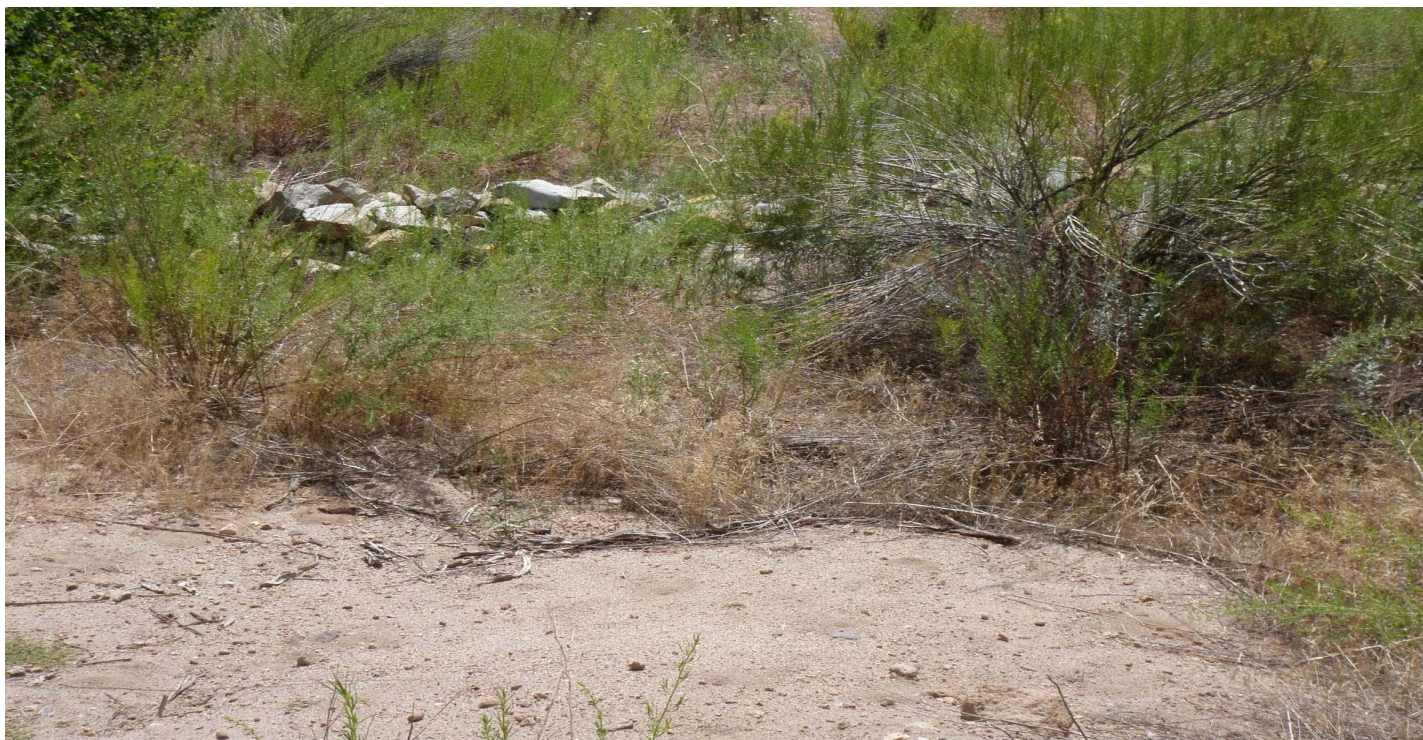
Photo 7411-4.JPG (taken 07/30/10) B00106010008 : Check Dam - Rock Check Dam.
