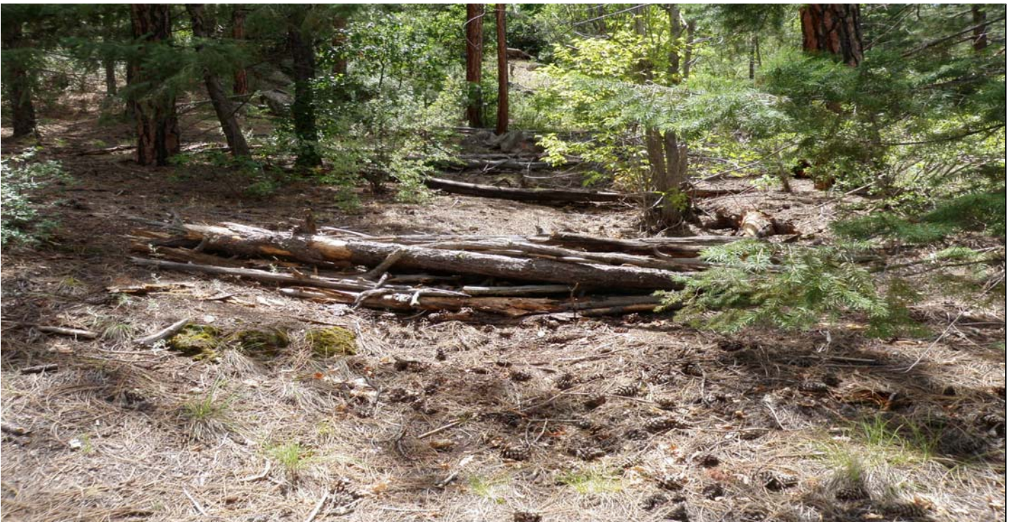
Photo 7463-3.JPG (taken 08/06/10) M01402010003 : Established Vegetation - Permanent Vegetation Grasses and Shrubs; M01402020004 : Established Vegetation - Permanent Vegetation Forested/Needle Cast; M01406020006 : Check Dam - Log Check Dam.
