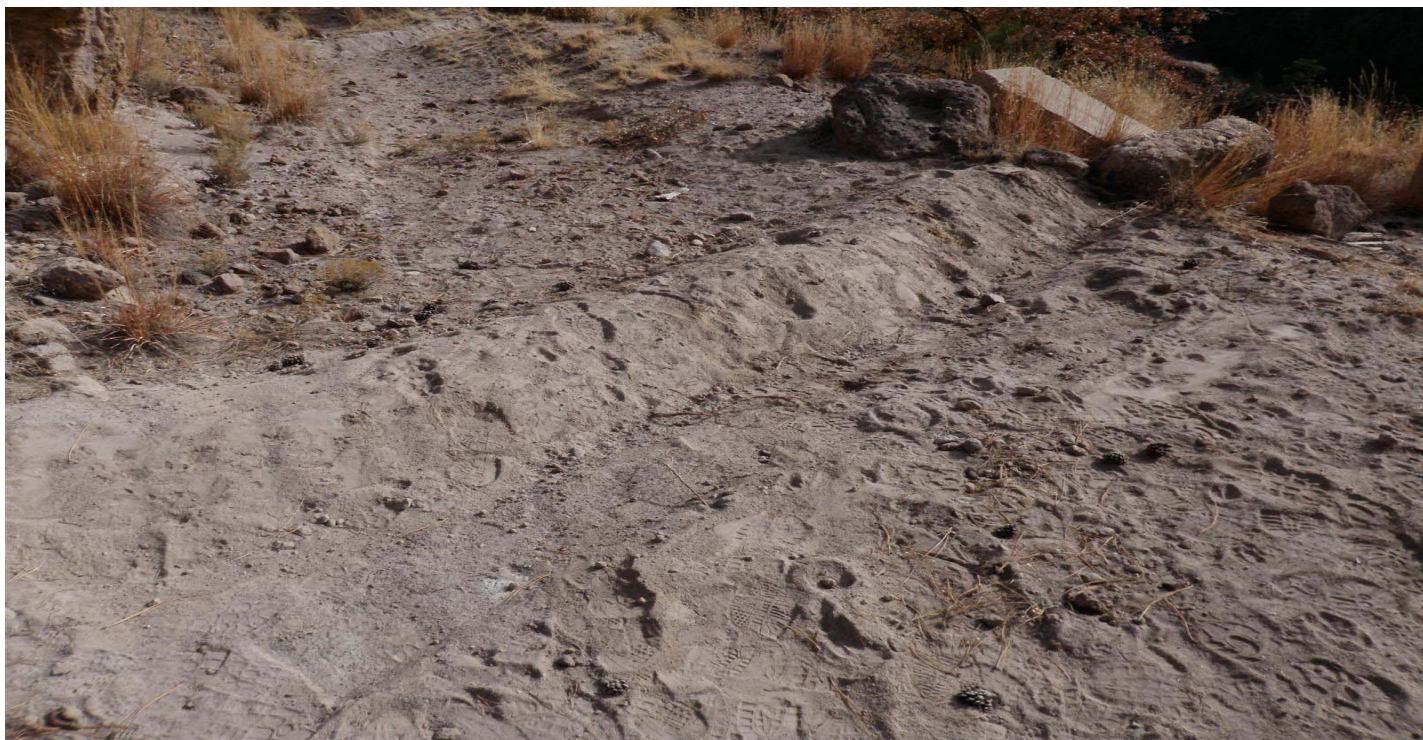
Photo 12128-3r.JPG (taken 12/06/10) L01204050008 : Channel/Swale - Water Bar.
