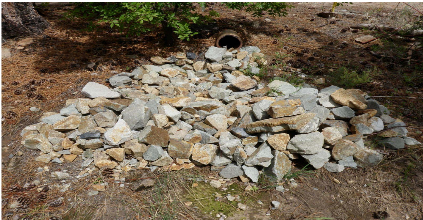
Photo 7494-2r.JPG (taken 08/09/10) M002A04060003 : Channel/Swale - Rip Rap; M002A06010004 : Check Dam - Rock Check Dam.
