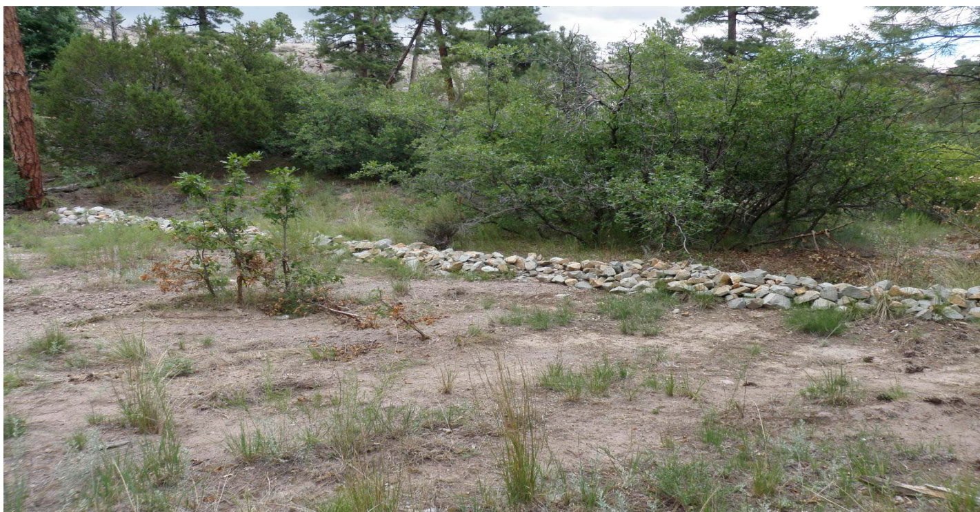
Photo 7452-6.JPG (taken 08/04/10) T00103120008 : Berms - Rock Berm.
