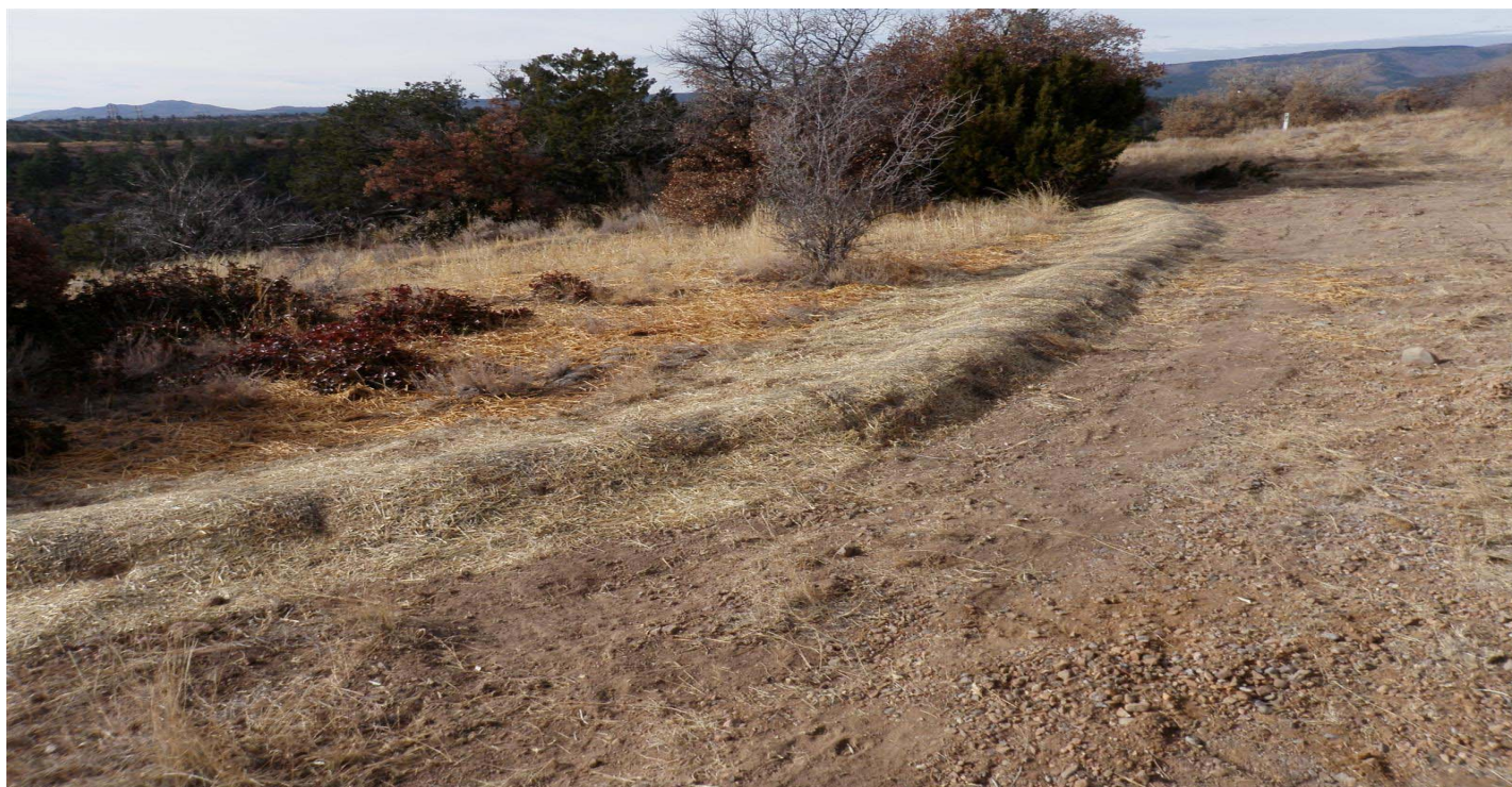
Photo 12127-1r.JPG (taken 12/06/10) L02803010006 : Berms - Earthen Berm.
