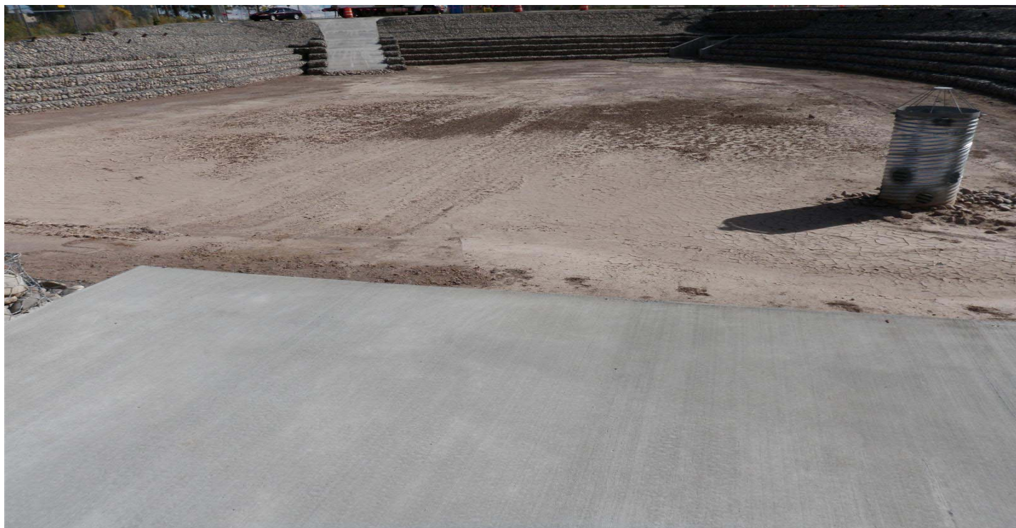
Photo 10550-05r.JPG (taken 09/20/10) M00805020016 : Sediment Traps and Basins - Sediment Basin.
