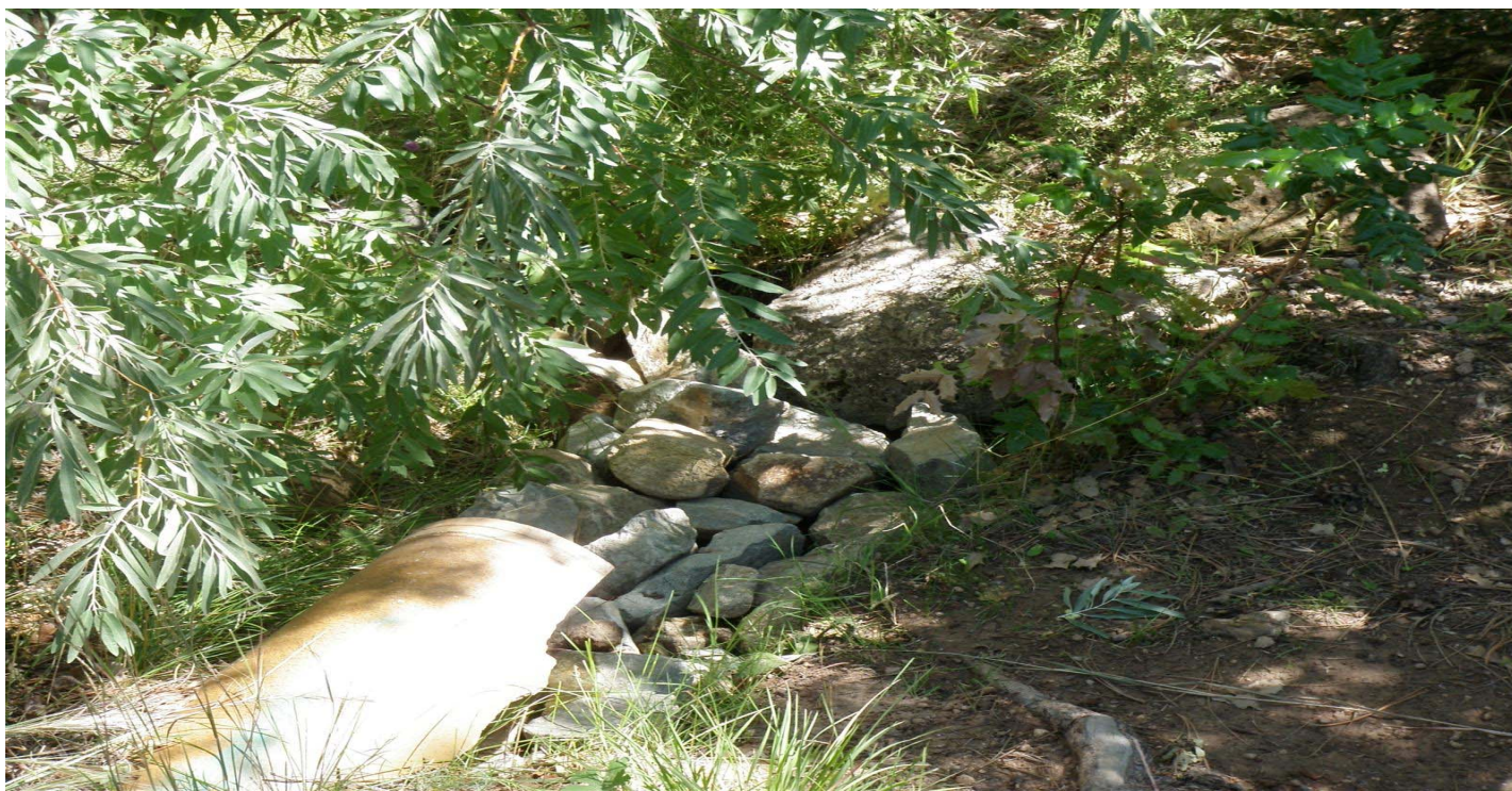
Photo 8510-1r.JPG (taken 08/20/10) M00204060008 : Channel/Swale - Rip Rap.
