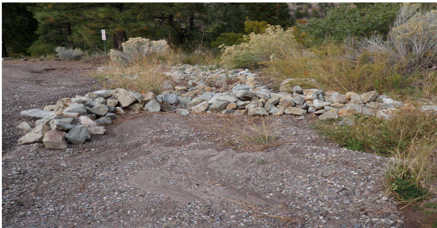
Photo 11026-3r.JPG (taken 10/21/10) M00806010007 : Check Dam - Rock Check Dam.
