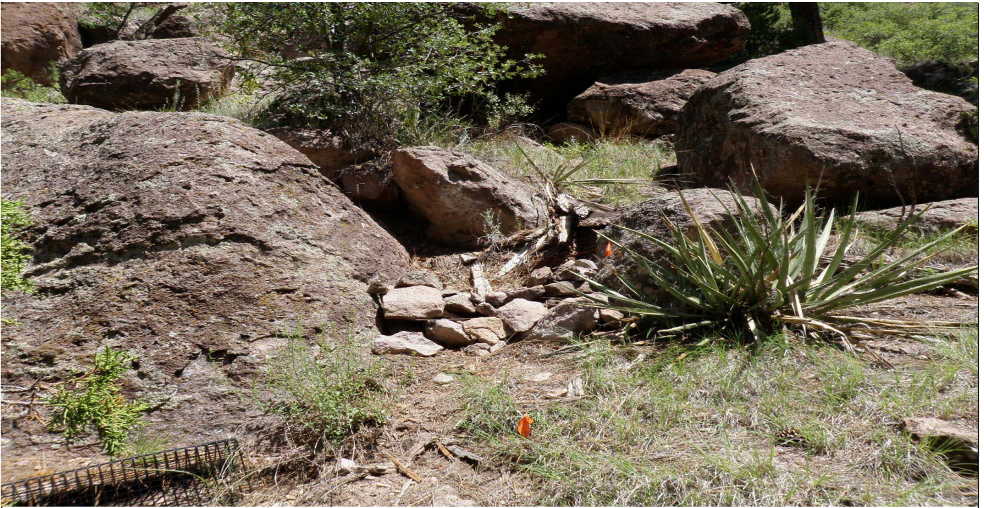
Photo 8655-2.JPG (taken 07/28/10) L02206010001 : Check Dam - Rock Check Dam.
