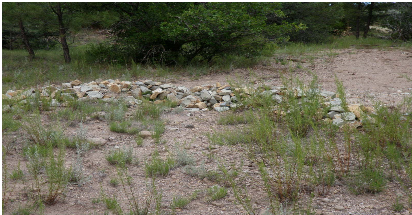
Photo 7452-8.JPG (taken 08/04/10) T00106010011 : Check Dam - Rock Check Dam.
