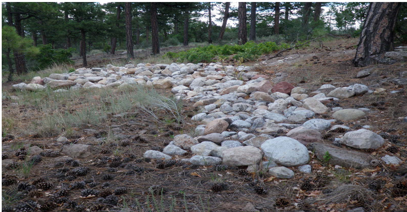
Photo 8656-9.JPG (taken 07/29/10) D00404060004 : Channel/Swale - Rip Rap.
