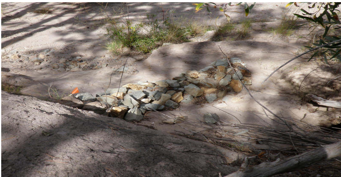
Photo 10550-09r.JPG (taken 09/20/10) M00806010010 : Check Dam - Rock Check Dam.
