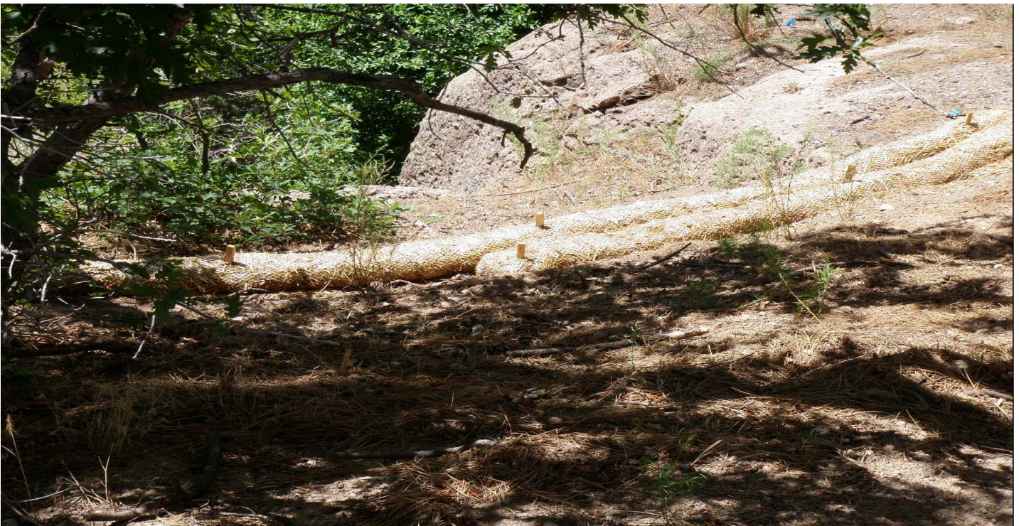
Photo 7410-3.JPG (taken 07/30/10) P002A03060005 : Berms - Straw Wattles.
