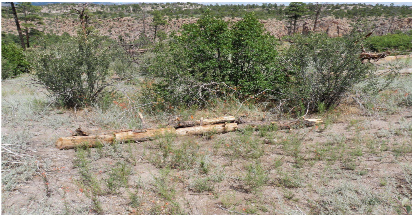
Photo 7478-2r.JPG (taken 08/10/10) M01906020006 : Check Dam - Log Check Dam.
