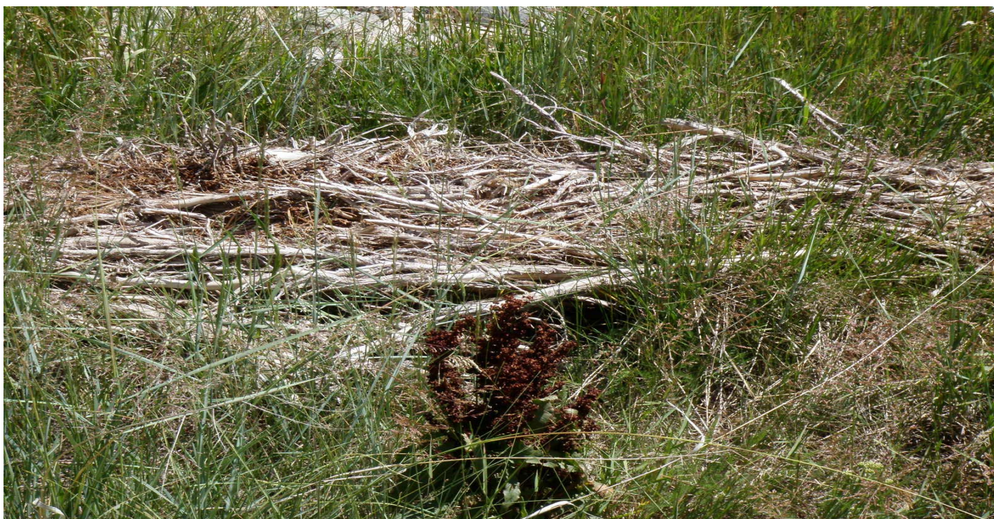
Photo 8656-4.JPG (taken 07/29/10) D00406030008 : Check Dam - Juniper Bales.
