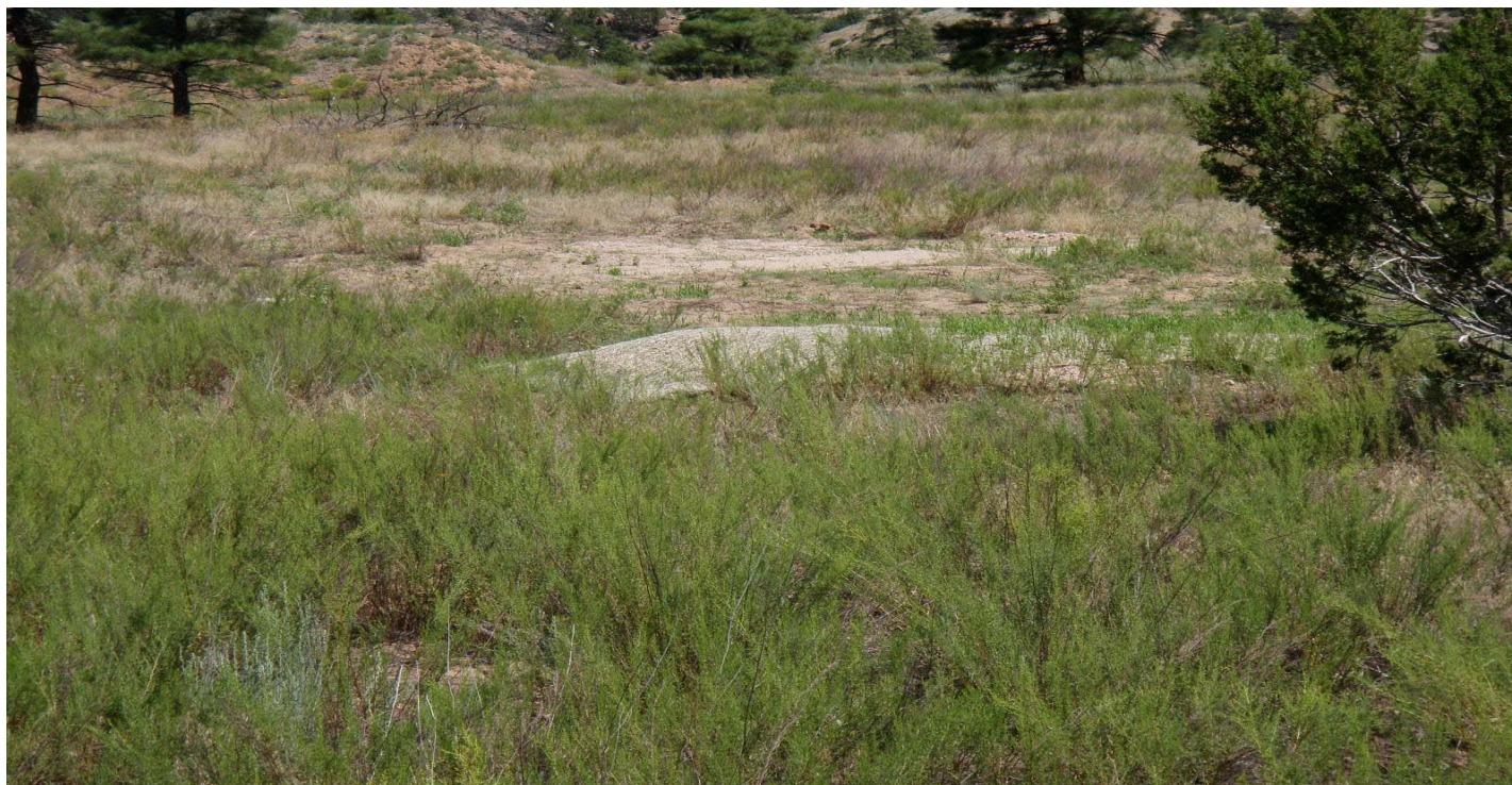
Photo 7442-1.JPG (taken 08/03/10) R00303010006 : Berms - Earthen Berm.
