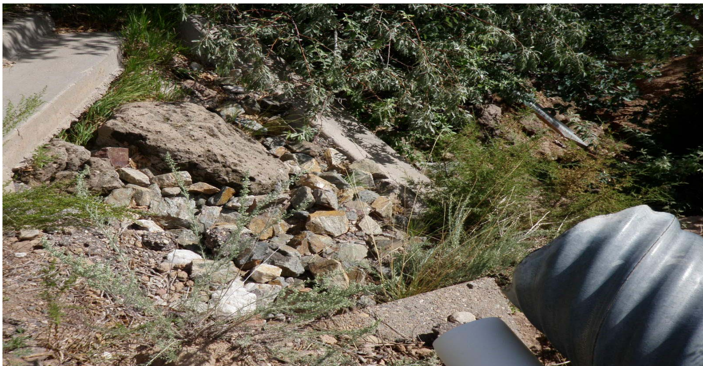
Photo 7459-4.JPG (taken 08/04/10) T00504060001 : Channel/Swale - Rip Rap.
