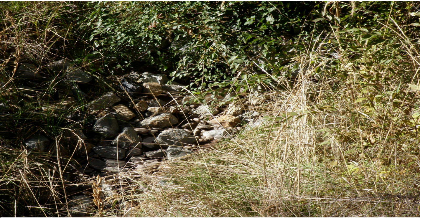
Photo 11612-2r.JPG (taken 10/28/10) L00404060003 : Channel/Swale - Rip Rap.
