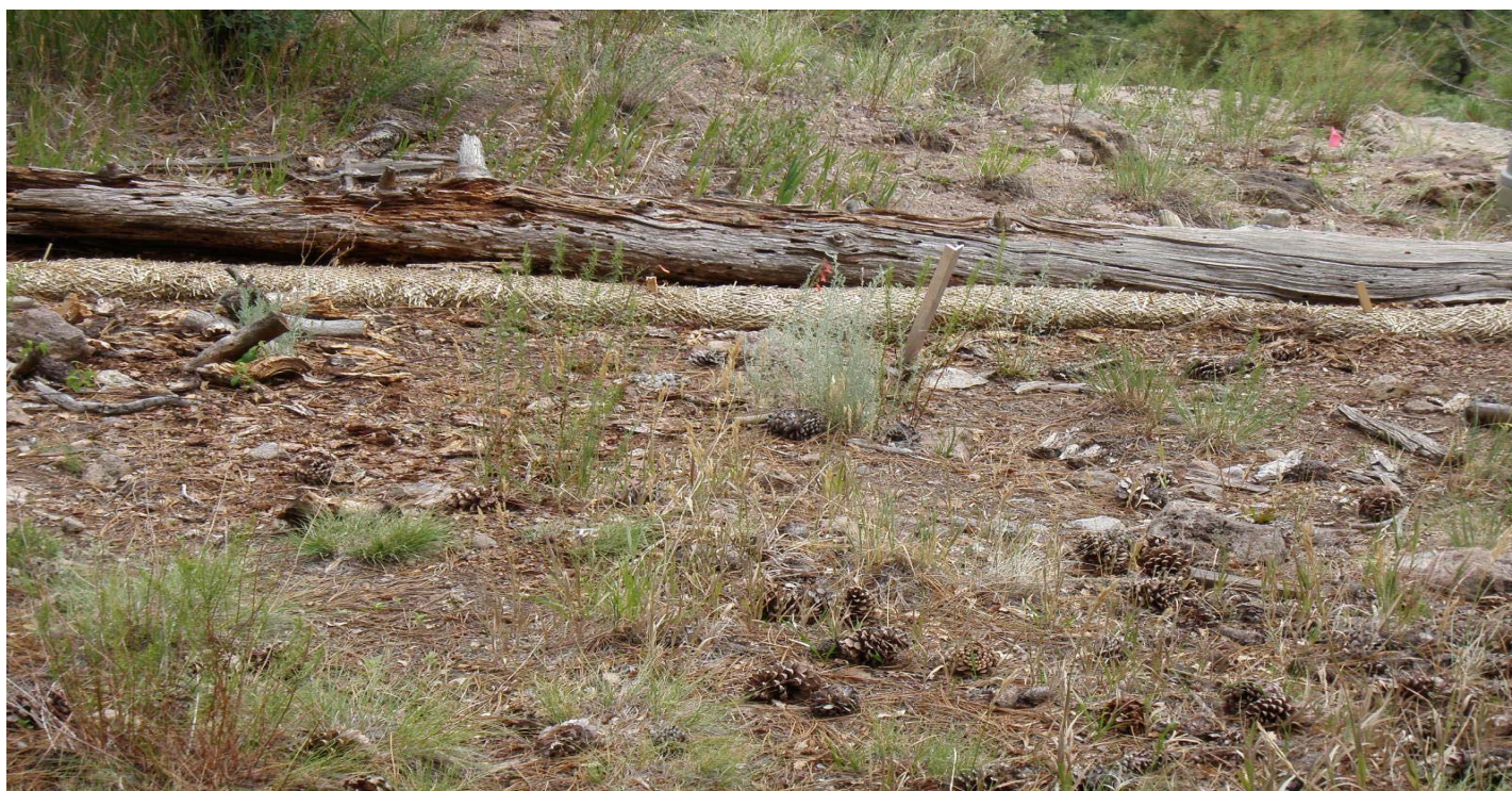
Photo 7423-1.JPG (taken 07/28/10) L00903060003 : Berms - Straw Wattles.
