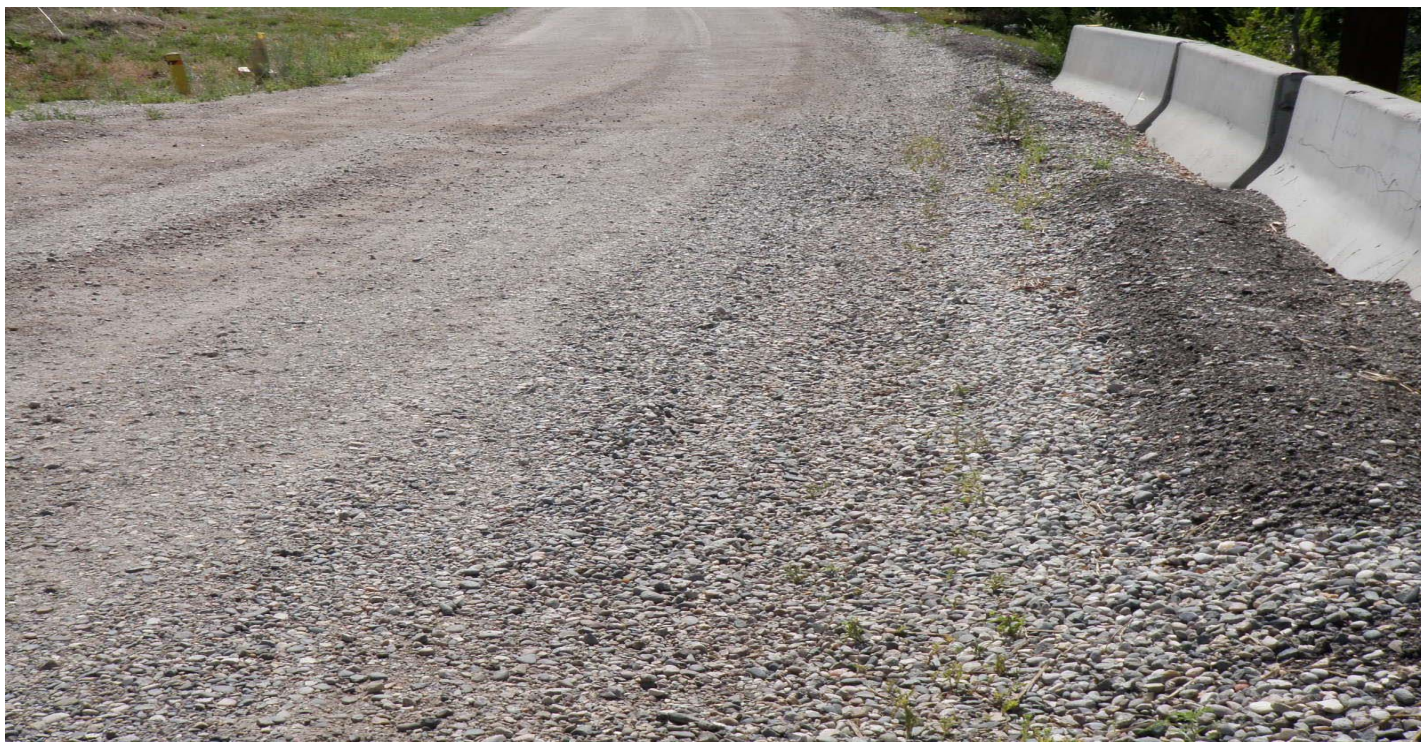
Photo 8655-4.JPG (taken 07/28/10) L02203040005 : Berms - Asphalt Berm.
