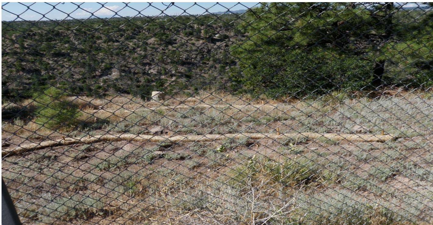
Photo 7432-2.JPG (taken 07/29/10) L02302010001 : Established Vegetation - Permanent Vegetation Grasses and Shrubs; L02303060003 : Berms - Straw Wattles; L02303060004 : Berms - Straw Wattles.
