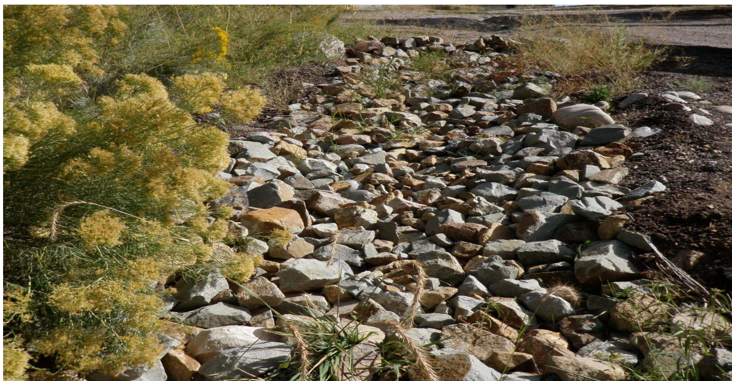
Photo 10550-06r.JPG (taken 09/20/10) M00804060001 : Channel/Swale - Rip Rap.
