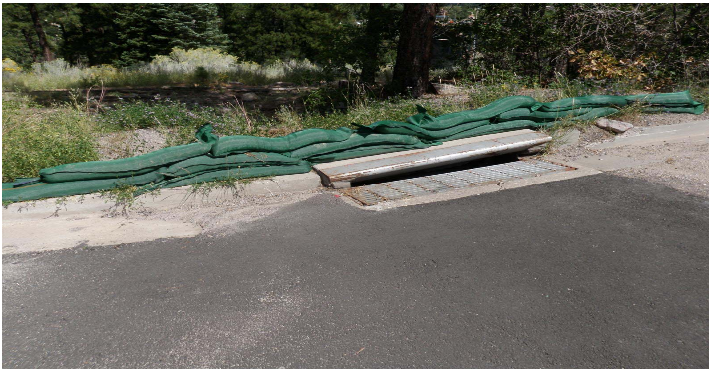
Photo 10562-5r.JPG (taken 09/14/10) L00203090002 : Berms - Curbing; L00203100010 : Berms - Gravel Bags; L00204040004 : Channel/Swale - Culvert.
