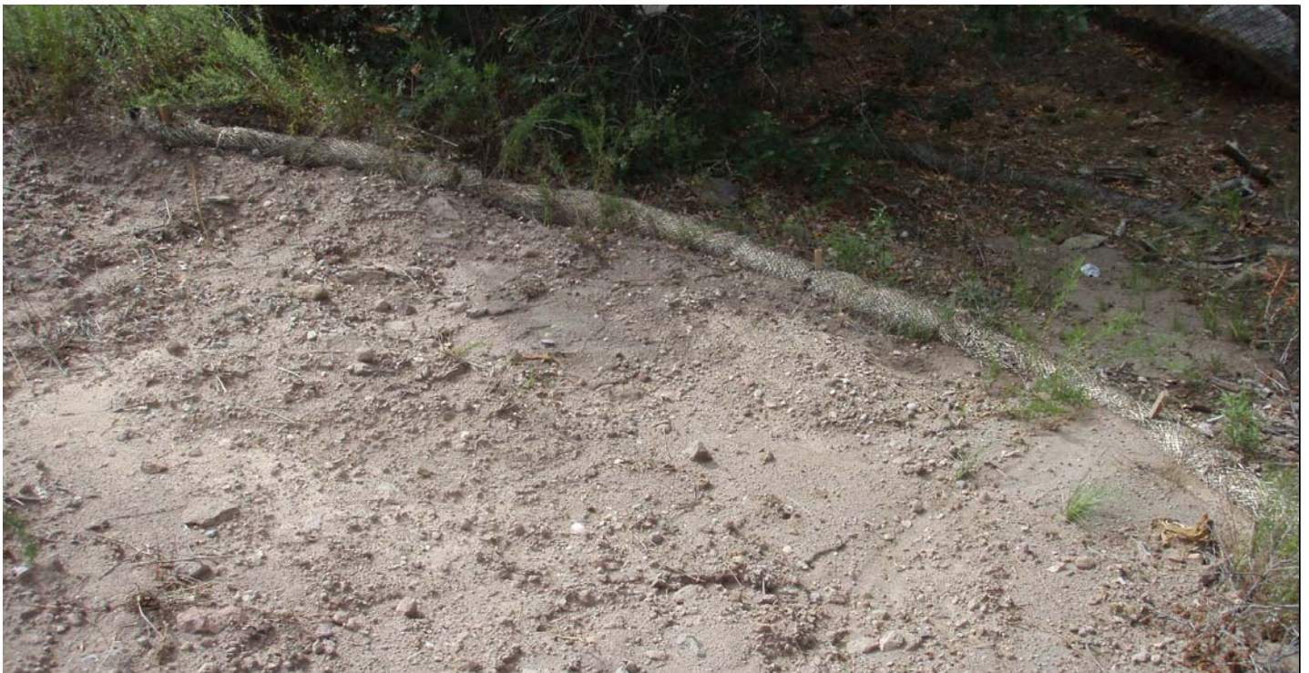
Photo 7518-1.JPG (taken 08/12/10) S00403060002 : Berms - Straw Wattles.
