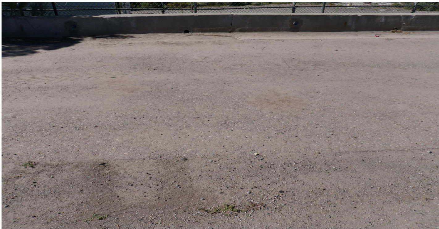
Photo 8508-2r.JPG (taken 08/20/10) J02703090001 : Berms - Curbing.
