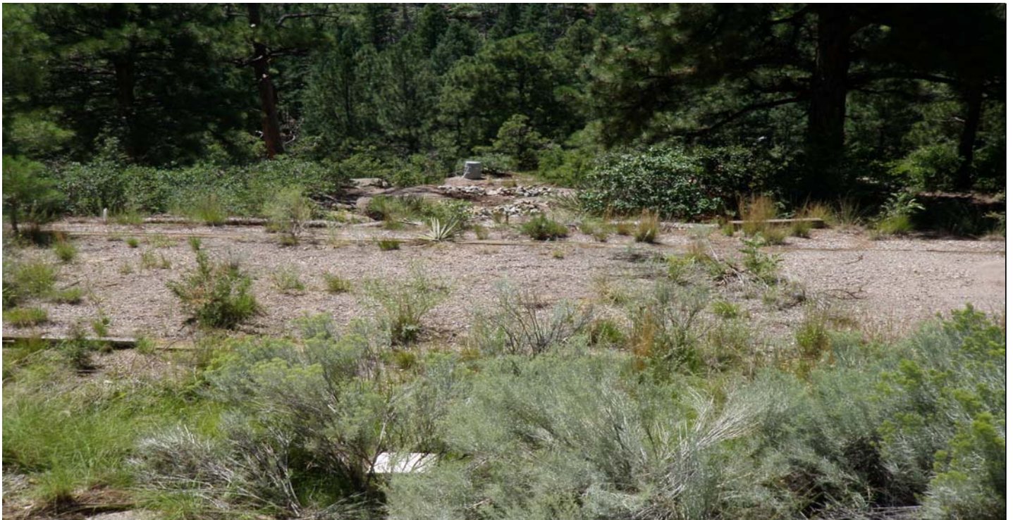
Photo 7470-1.JPG (taken 08/06/10) T00306010003 : Check Dam - Rock Check Dam; T00306010004 : Check Dam - Rock Check Dam; T00308020001 : Cap - Rock Cap.
