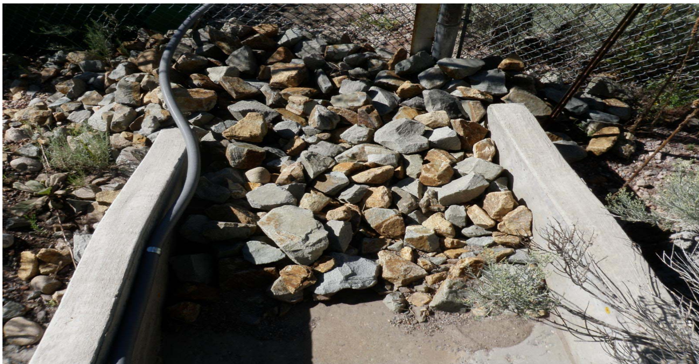
Photo 8508-3r.JPG (taken 08/20/10) J02704060006 : Channel/Swale - Rip Rap.
