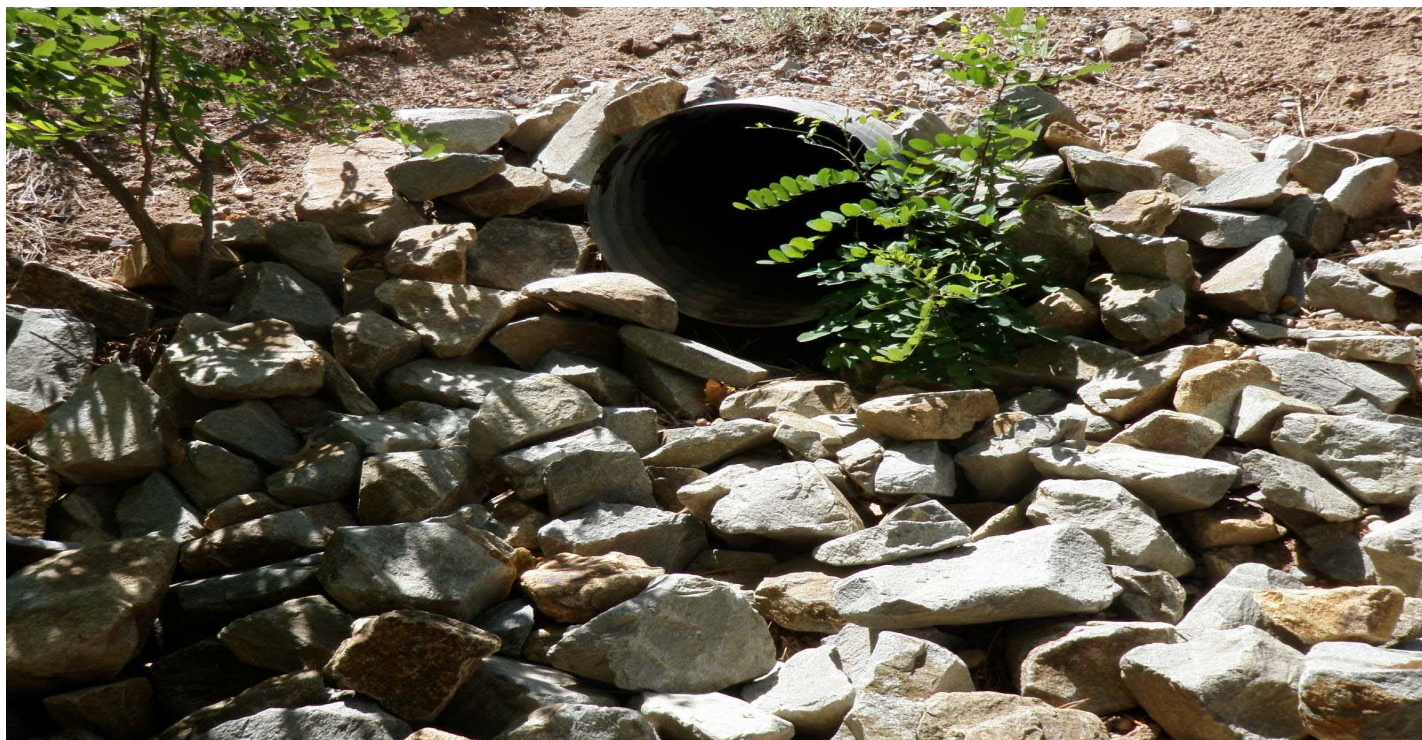
Photo 7415-4.JPG (taken 07/29/10) D00604060004 : Channel/Swale - Rip Rap.
