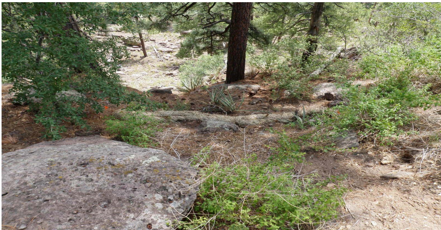
Photo 7421-2.JPG (taken 07/28/10) L00703060004 : Berms - Straw Wattles.
