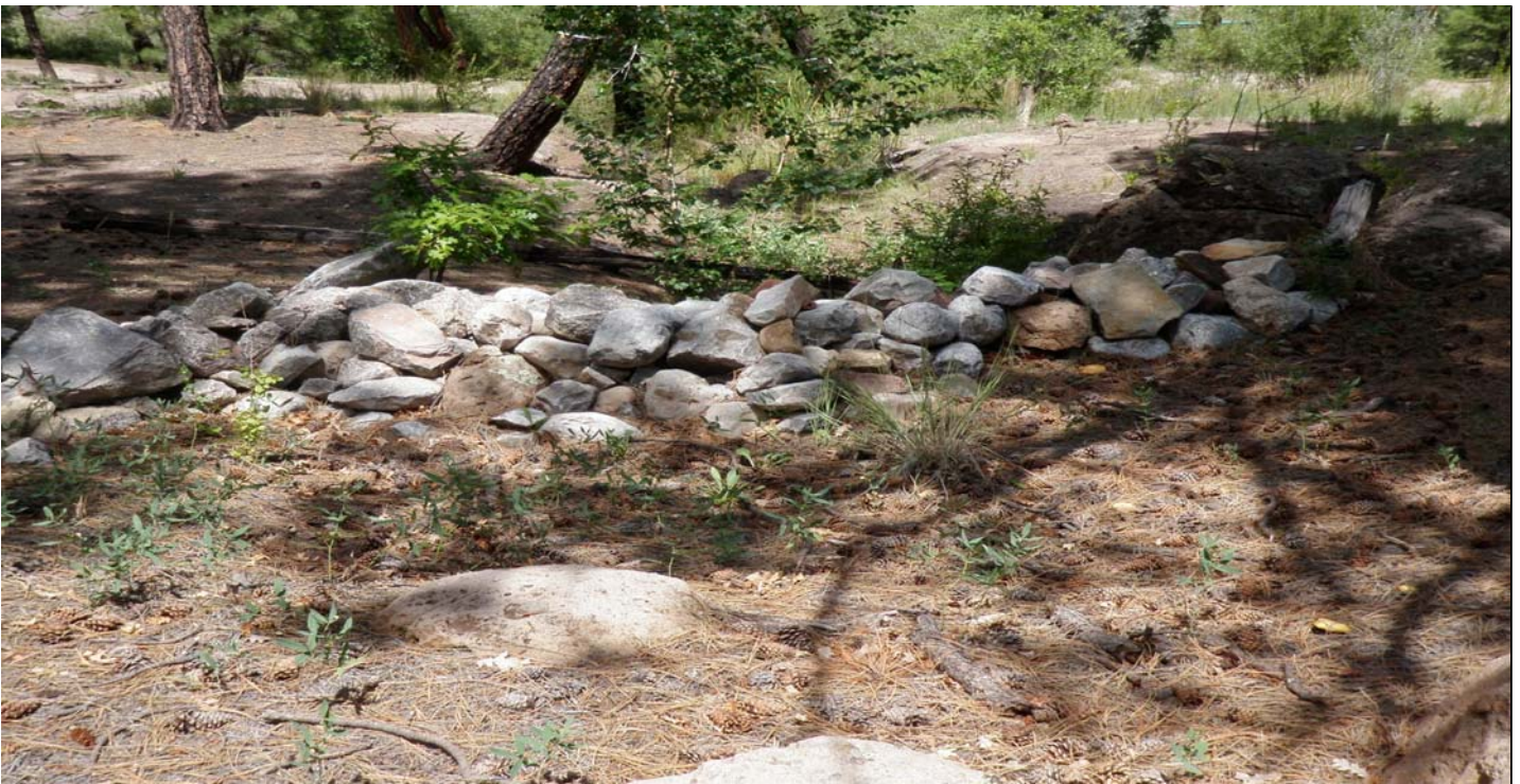
Photo 7468-3.JPG (taken 08/06/10) M00902020002 : Established Vegetation - Permanent Vegetation Forested/Needle Cast; M00906010003 : Check Dam - Rock Check Dam.
