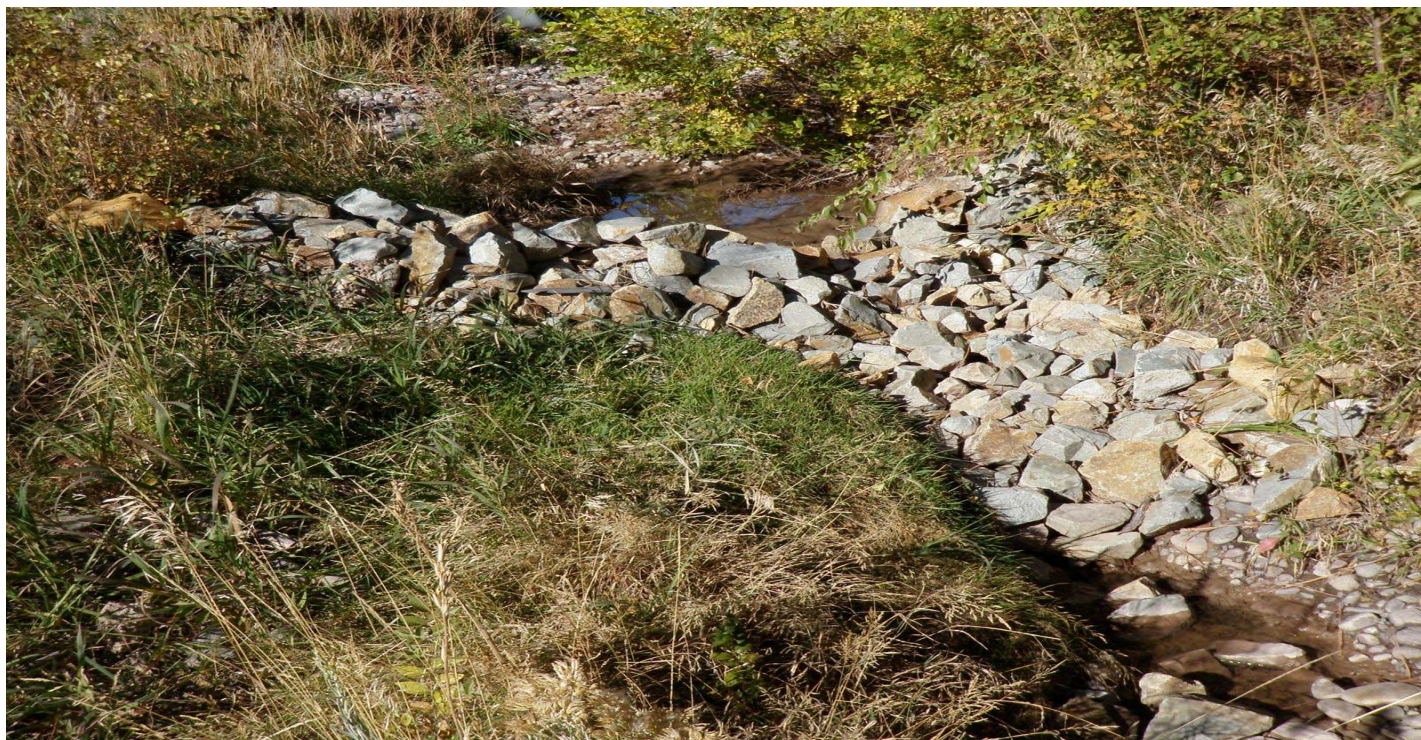
Photo 11612-1r.JPG (taken 10/28/10) L00406010004 : Check Dam - Rock Check Dam.
