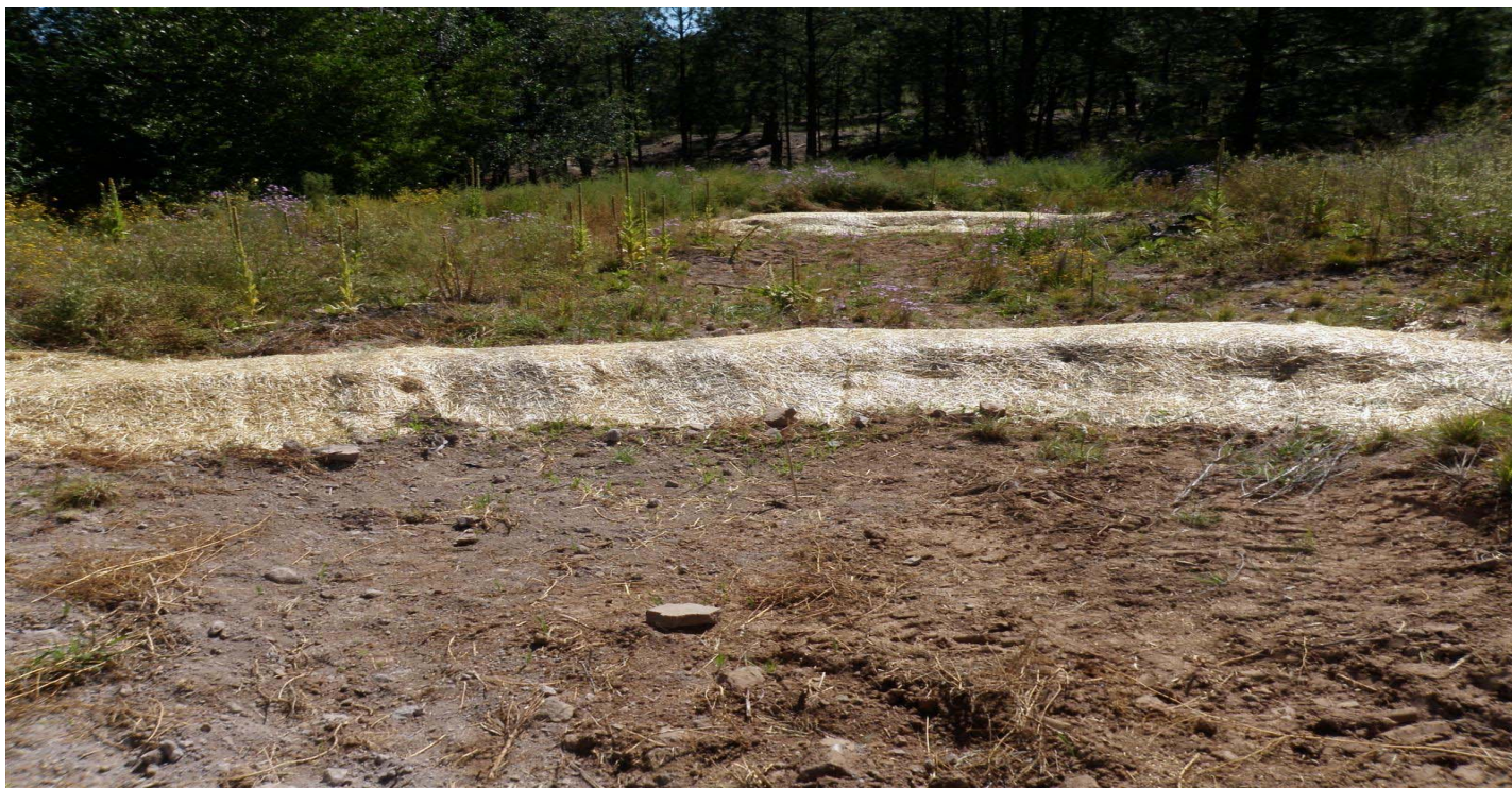
Photo 10559-4r.JPG (taken 09/14/10) P00903010008 : Berms - Earthen Berm; P00903010009 : Berms - Earthen Berm.
