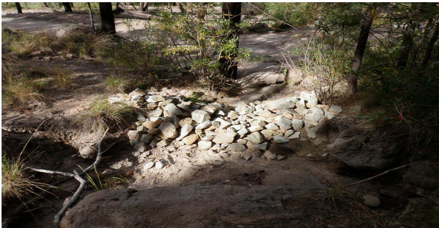
Photo 10550-07r.JPG (taken 09/20/10) M00806010008 : Check Dam - Rock Check Dam.
