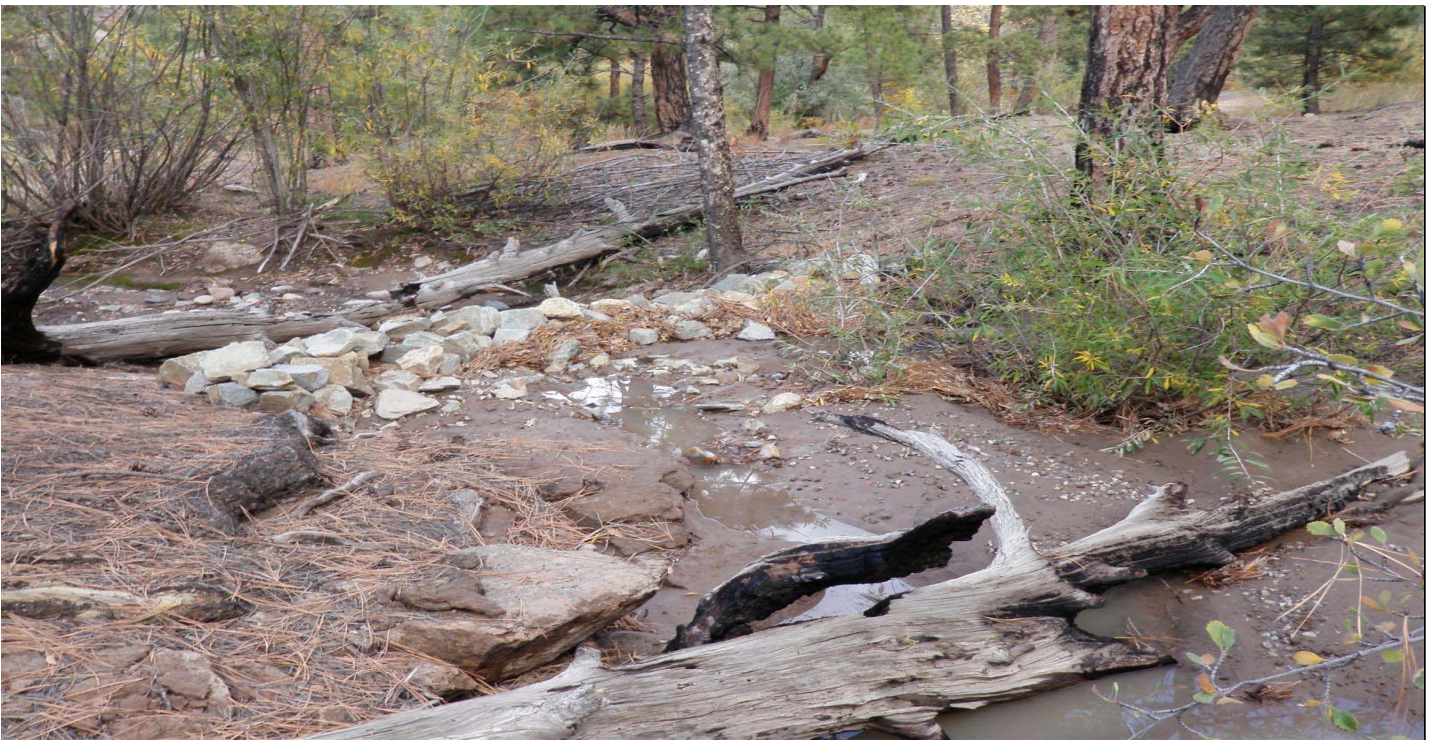
Photo 11026-1r.JPG (taken 10/21/10) M00806010009 : Check Dam - Rock Check Dam.
