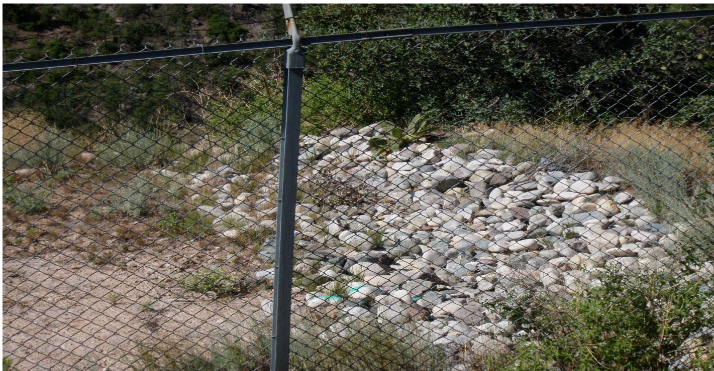
Photo 7431-4.JPG (taken 07/29/10) L022A04030003 : Channel/Swale - Rock Channel/Swale.
