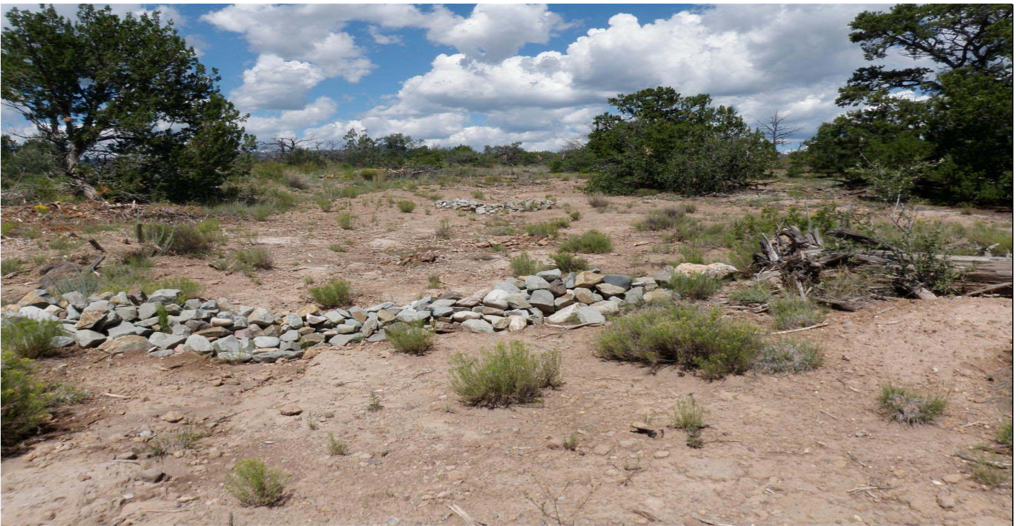
Photo 7476-2r.JPG (taken 08/10/10) M02206010008 : Check Dam - Rock Check Dam; M02206010010 : Check Dam - Rock Check Dam.
