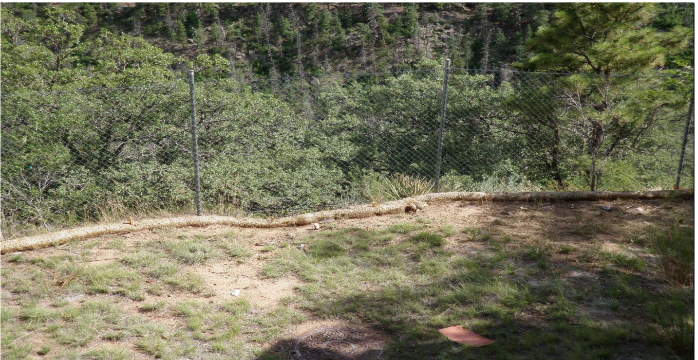
Photo 7425-5.JPG (taken 07/28/10) L01203060002 : Berms - Straw Wattles.
