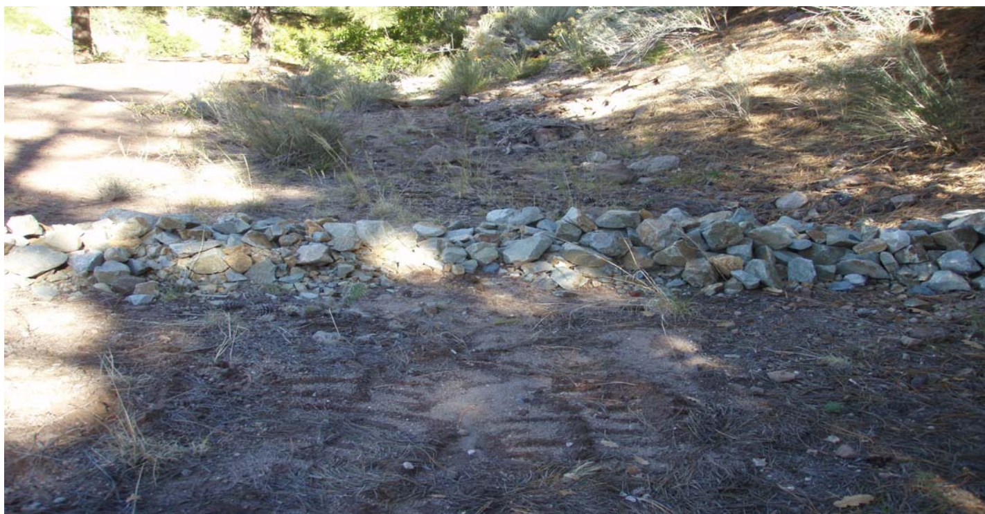
Photo 10869-1.JPG (taken 10/08/10) S005B06010003 : Check Dam - Rock Check Dam.
