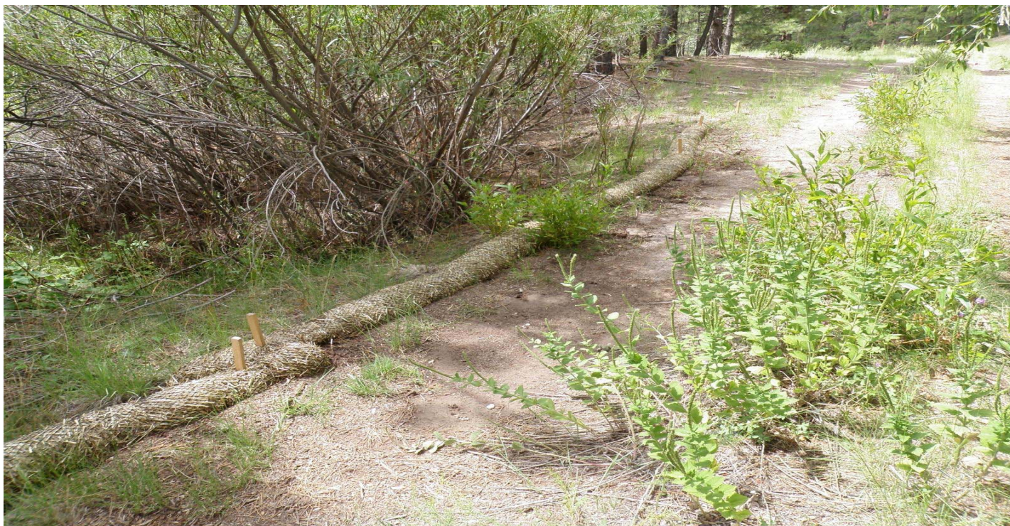
Photo 7495-1r.JPG (taken 08/09/10) M00203060006 : Berms - Straw Wattles.
