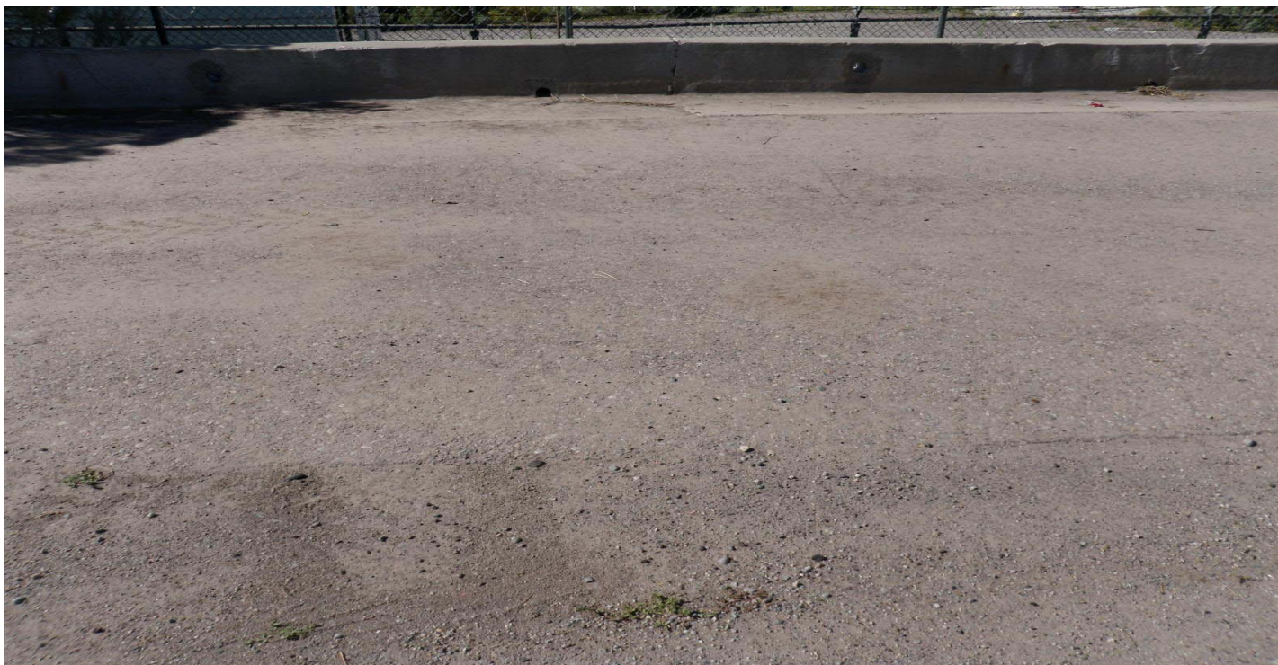
Photo 8508-2r.JPG (taken 08/20/10) J02703090001 : Berms - Curbing.
