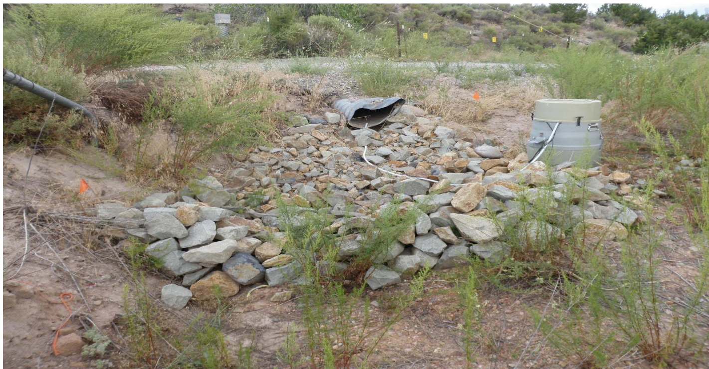
Photo 7439-1.JPG (taken 07/29/10) L03004060009 : Channel/Swale - Rip Rap; L03006010001 : Check Dam - Rock Check Dam.
