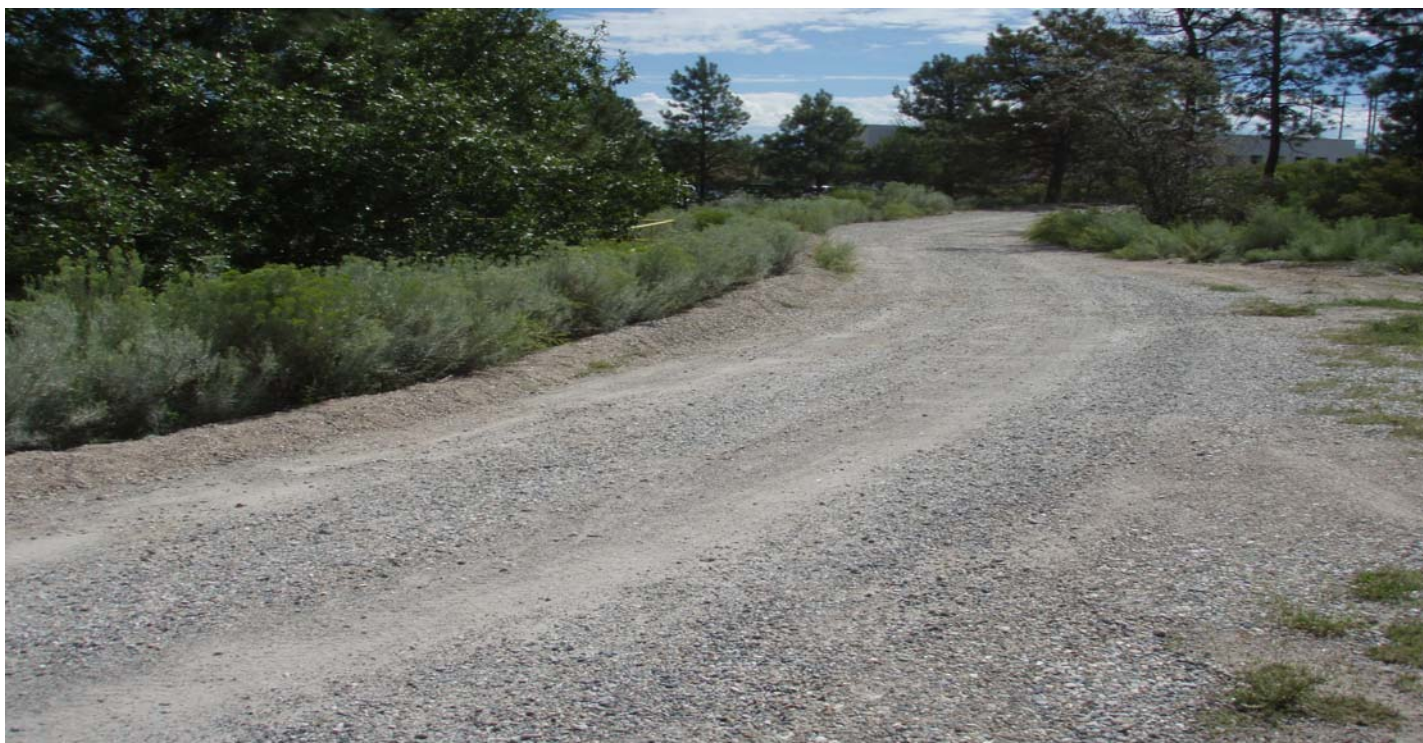
Photo 7518-3.JPG (taken 08/12/10) S00403020004 : Berms - Base Course Berm.
