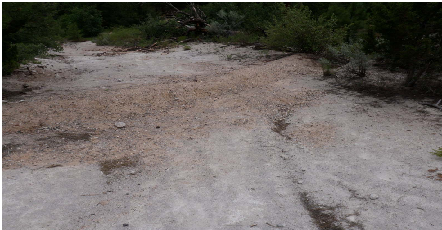
Photo 7452-02.JPG (taken 08/04/10) T00103020013 : Berms - Base Course Berm.
