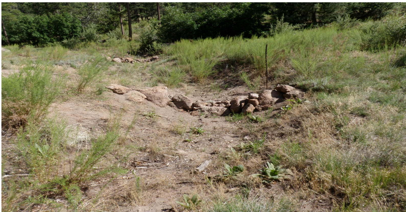
Photo 7412-5.JPG (taken 07/29/10) B00206010006 : Check Dam - Rock Check Dam.
