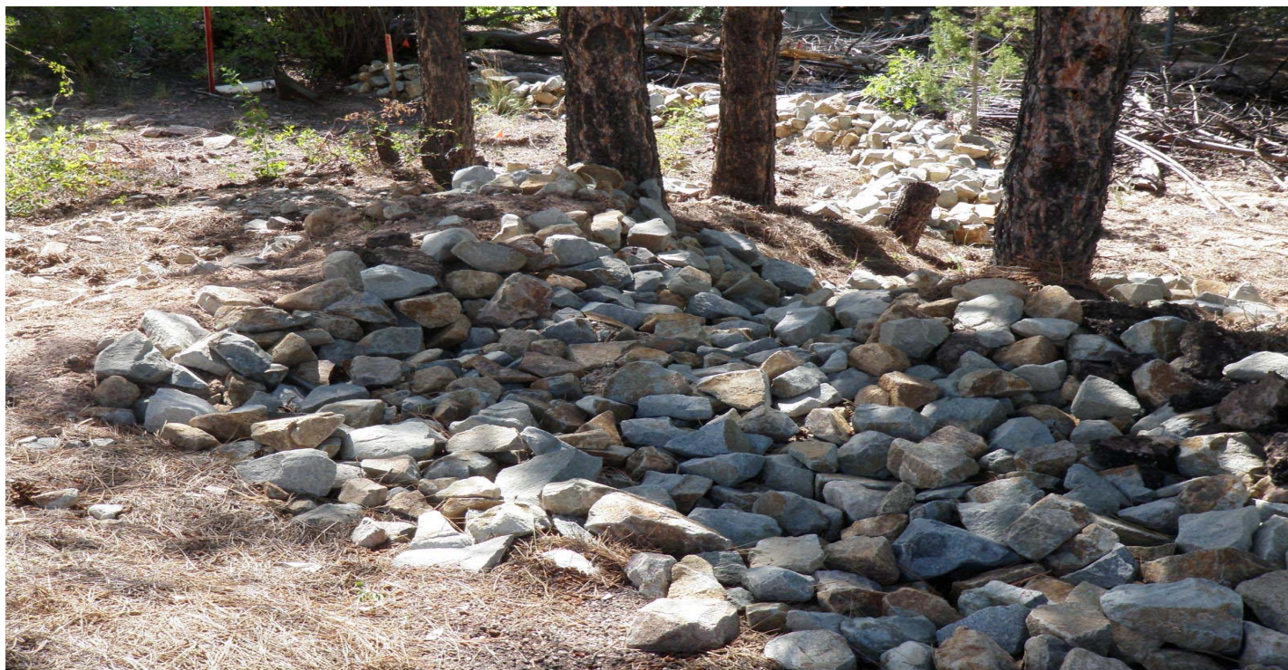
Photo 10555-1r.JPG (taken 09/09/10) S00703120004 : Berms - Rock Berm.
