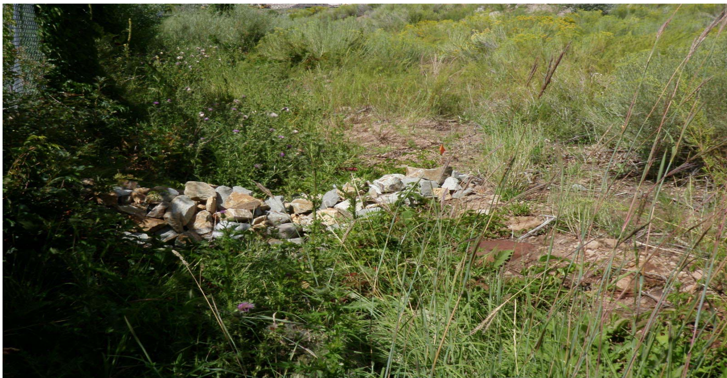
Photo 8501-3r.JPG (taken 08/19/10) S00502010003 : Established Vegetation - Permanent Vegetation Grasses and Shrubs; S00506010008 : Check Dam - Rock Check Dam.
