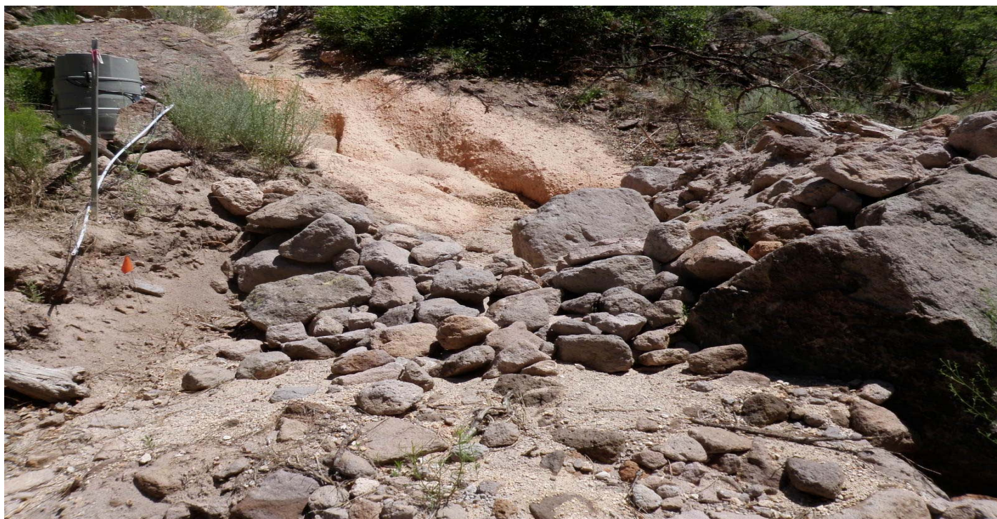
Photo 7431-1.JPG (taken 07/29/10) L022A06010005 : Check Dam - Rock Check Dam.
