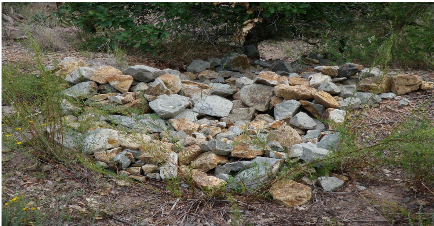
Photo 7450-4.JPG (taken 08/04/10) T00706010009 : Check Dam - Rock Check Dam.
