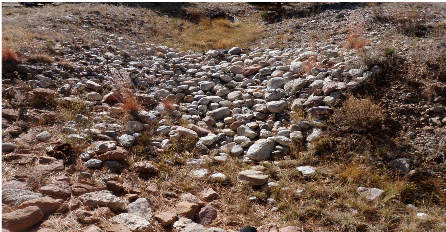
Photo 11699-5r.JPG (taken 11/15/10) V00504060015 : Channel/Swale - Rip Rap.
