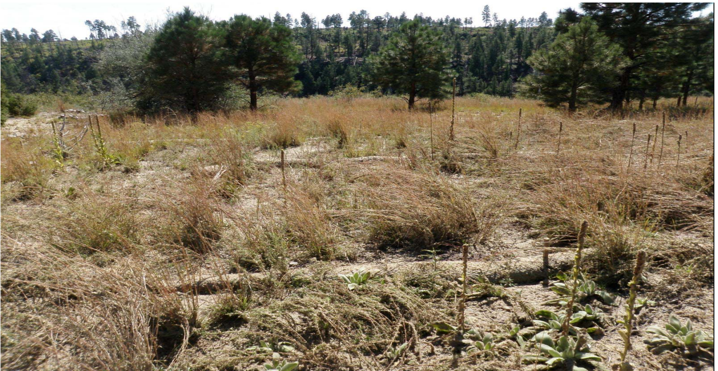
Photo 10864-4r.JPG (taken 10/07/10) J01303060009 : Berms - Straw Wattles; J01303060010 : Berms - Straw Wattles; J01303060011 : Berms - Straw Wattles.
