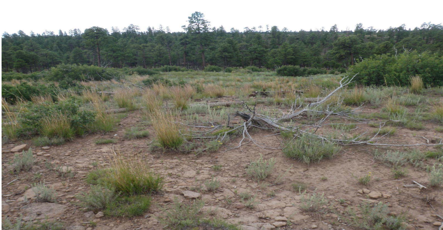
Photo 7513-4r.JPG (taken 08/12/10) E01403060009 : Berms - Straw Wattles.
