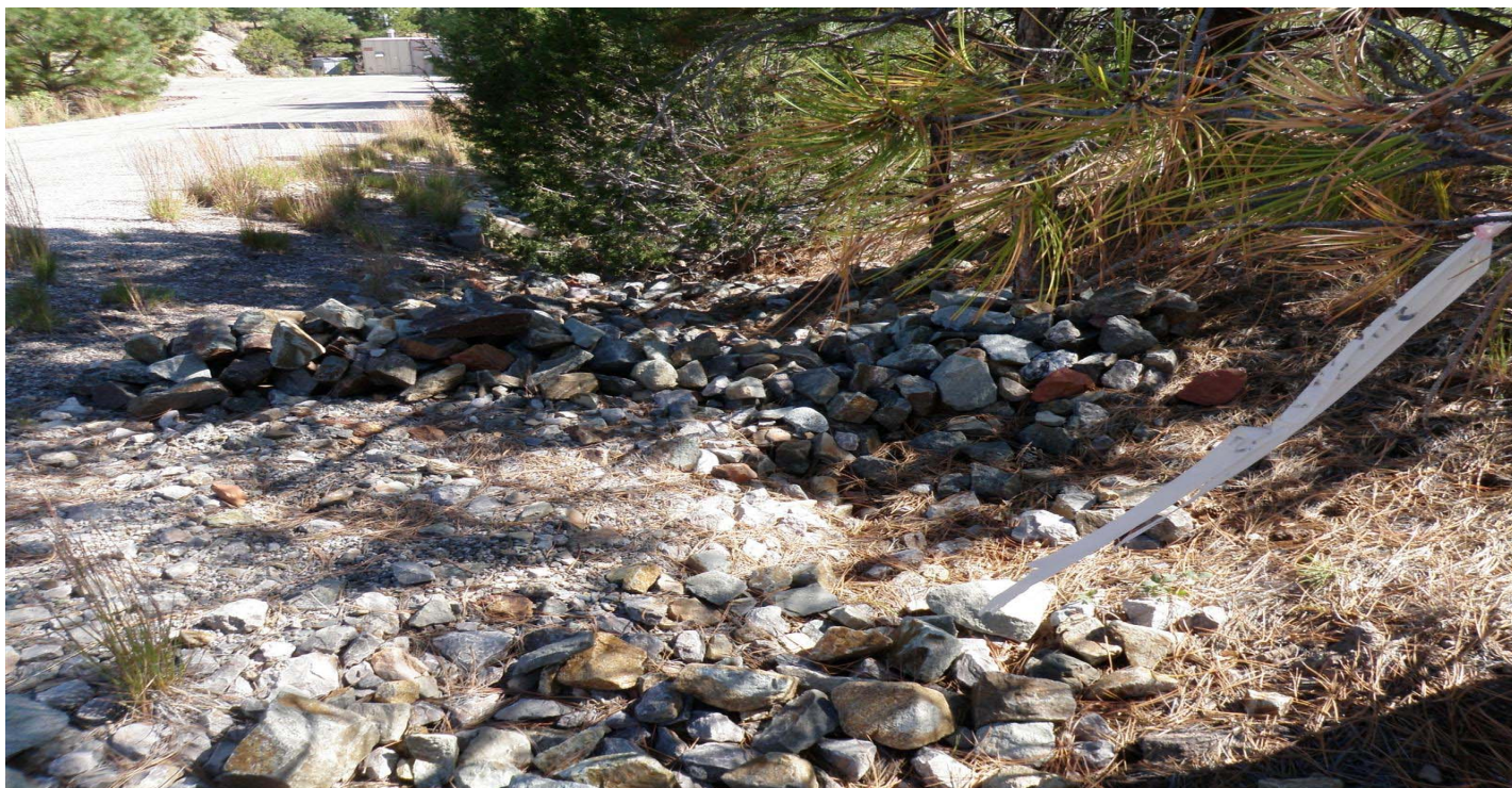
Photo 10873-13r.JPG (taken 10/07/10) H00306010016 : Check Dam - Rock Check Dam.
