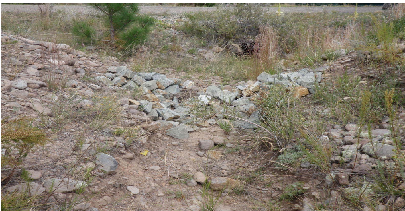
Photo 10885-2r.JPG (taken 10/01/10) V00506010009 : Check Dam - Rock Check Dam.
