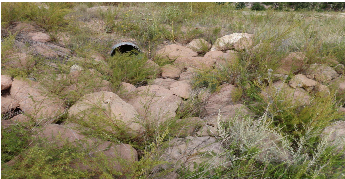
Photo 8793-1r.JPG (taken 09/07/10) V00804040011 : Channel/Swale - Culvert; V00804060009 : Channel/Swale - Rip Rap.
