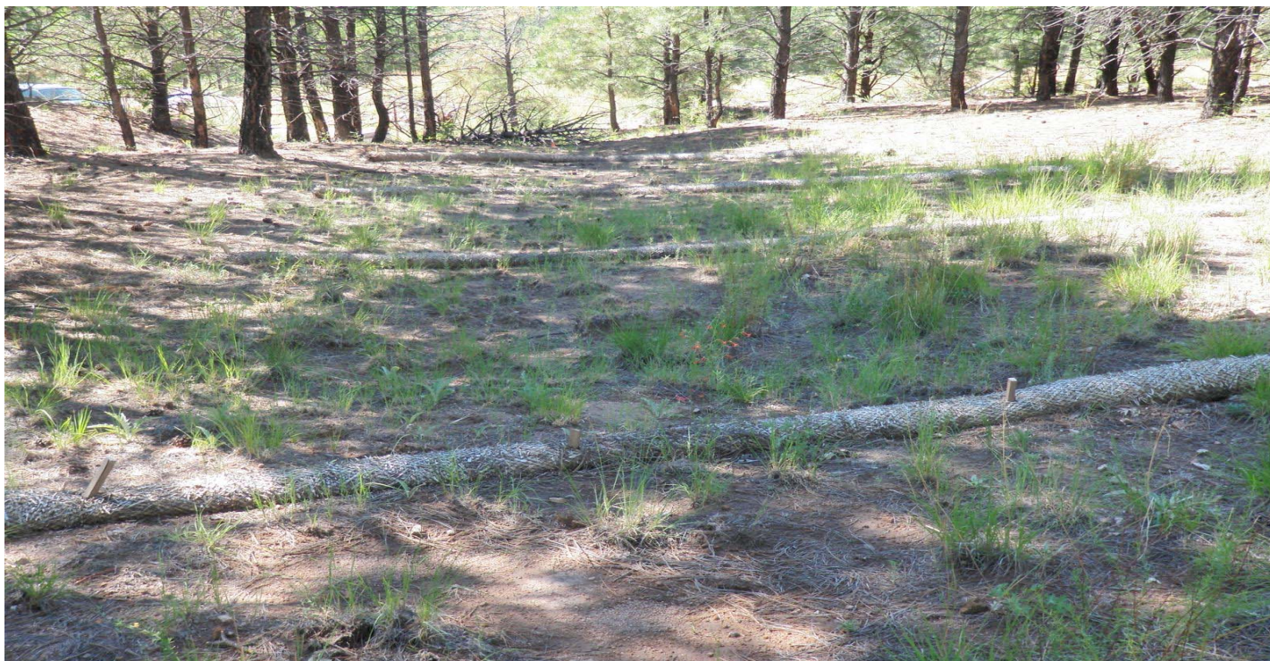
Photo 8525-03r.JPG (taken 08/18/10) V009A03060018 : Berms - Straw Wattles; V009A03060019 : Berms - Straw Wattles; V009A03060020 : Berms - Straw Wattles; V009A03060021 : Berms - Straw Wattles.
