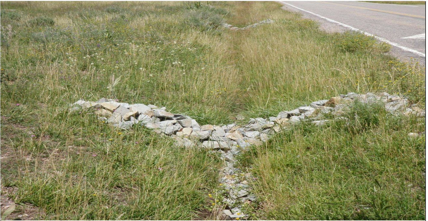
Photo 7800-1r.JPG (taken 08/17/10) W00206010008 : Check Dam - Rock Check Dam; W00206010009 : Check Dam - Rock Check Dam.
