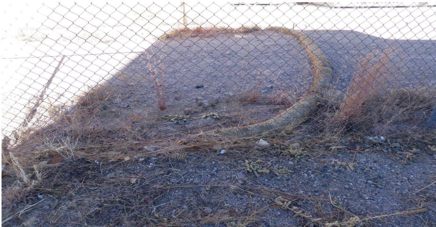
Photo 12126-5r.JPG (taken 12/02/10) E01203060008 : Berms - Straw Wattles.
