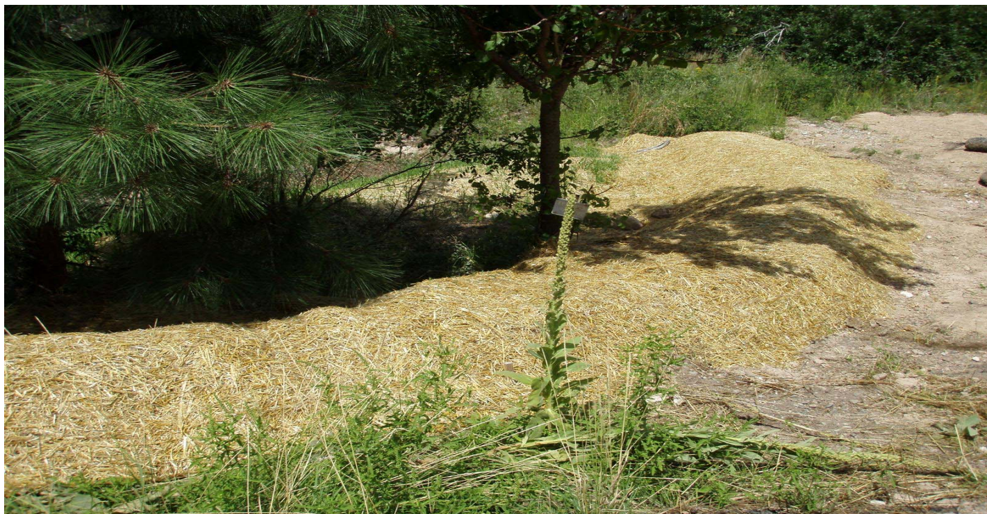
Photo 8536-1r.JPG (taken 08/23/10) V01502010001 : Established Vegetation - Permanent Vegetation Grasses and Shrubs; V01503010005 : Berms - Earthen Berm.
