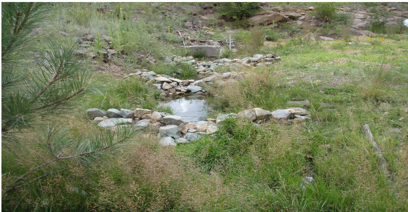
Photo 8531-07r.JPG (taken 08/23/10) W00606010003 : Check Dam - Rock Check Dam.
