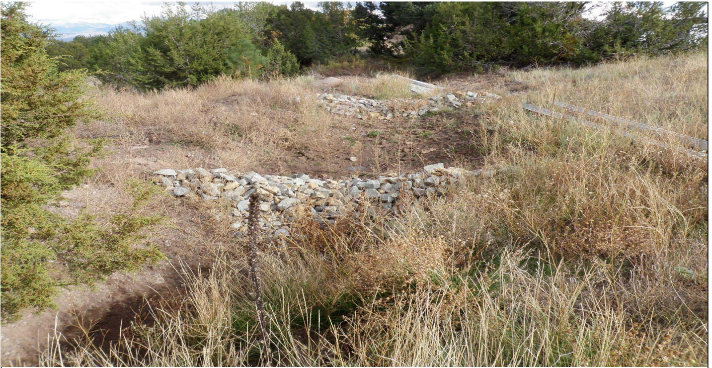
Photo 11025-1r.JPG (taken 10/21/10) C00406010004 : Check Dam - Rock Check Dam; C00406010013 : Check Dam - Rock Check Dam.
