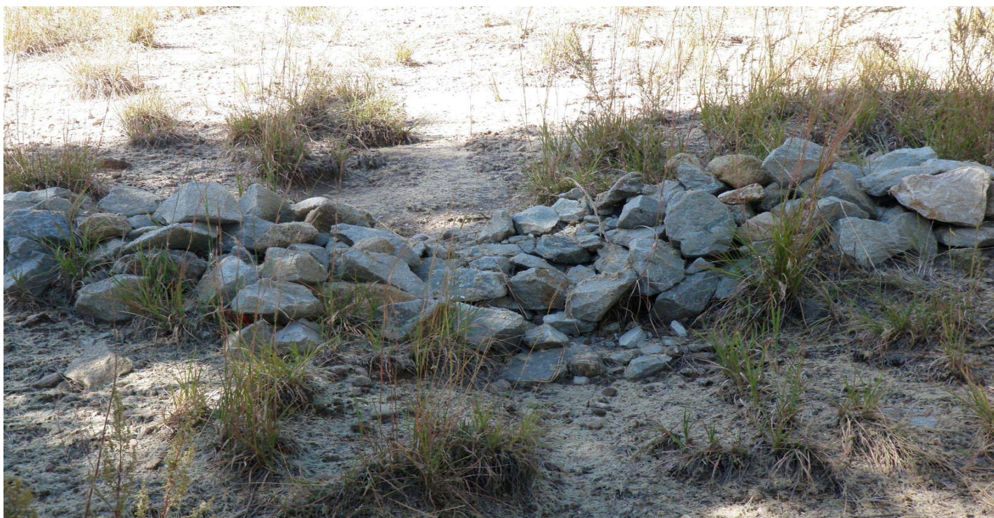
Photo 10865-4r.JPG (taken 10/07/10) J01406010012 : Check Dam - Rock Check Dam.
