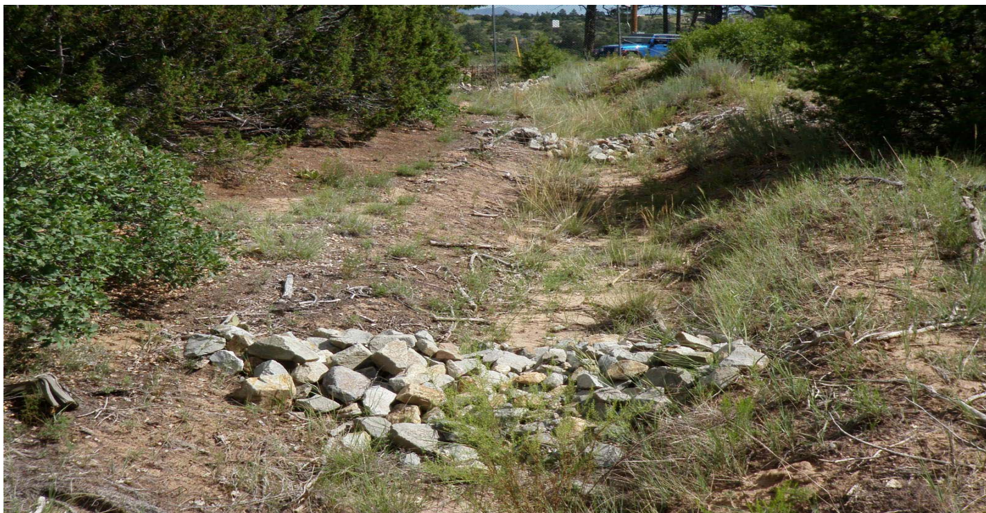
Photo 8519-16.JPG (taken 08/04/10) W01906010003 : Check Dam - Rock Check Dam; W01906010004 : Check Dam - Rock Check Dam; W01906010005 : Check Dam - Rock Check Dam.
