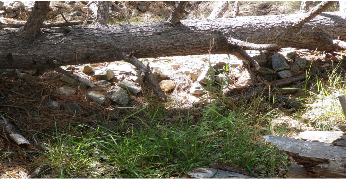
Photo 8522-08r.JPG (taken 08/18/10) V00306010011 : Check Dam - Rock Check Dam.
