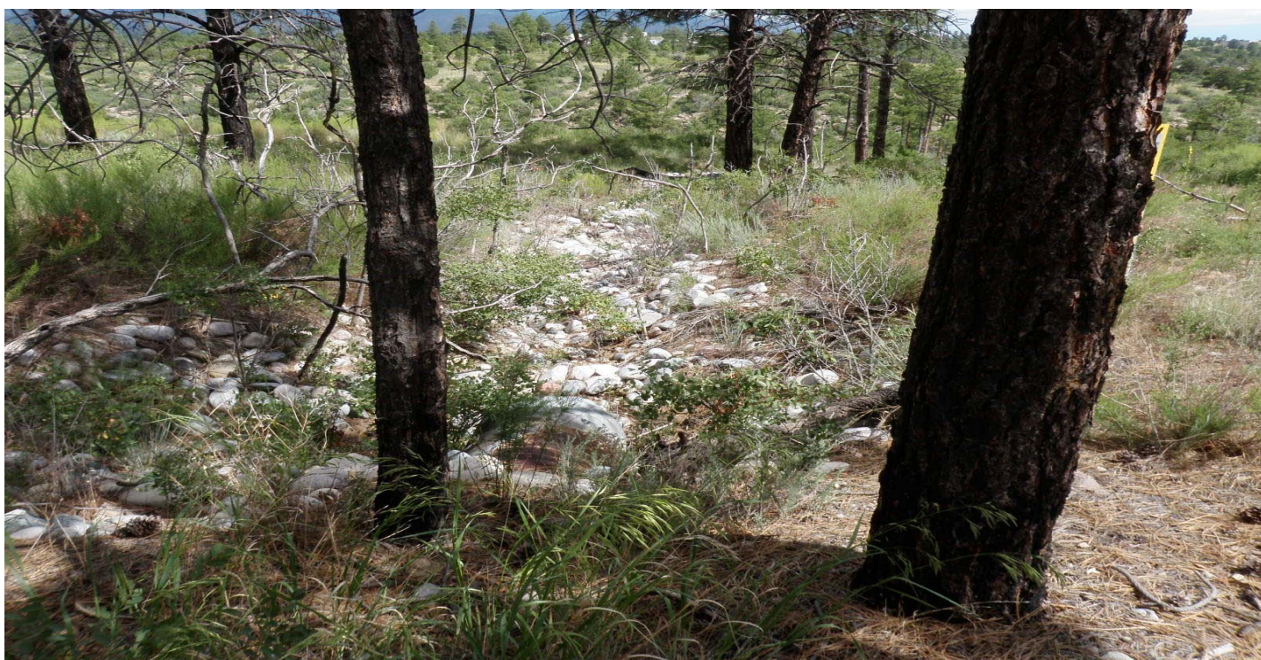
Photo 8519-17.JPG (taken 08/04/10) W01904060002 : Channel/Swale - Rip Rap.
