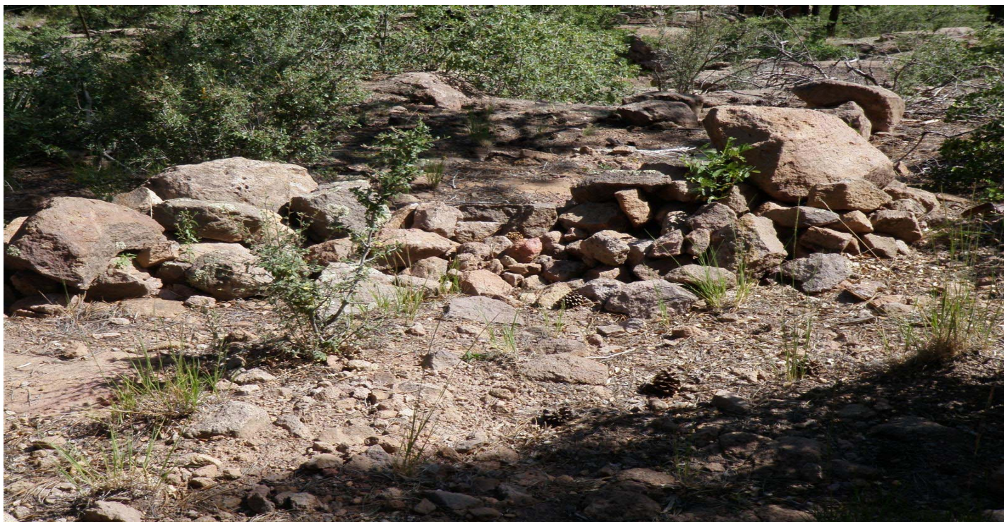
Photo 7801-5r.JPG (taken 08/17/10) W00906010007 : Check Dam - Rock Check Dam.
