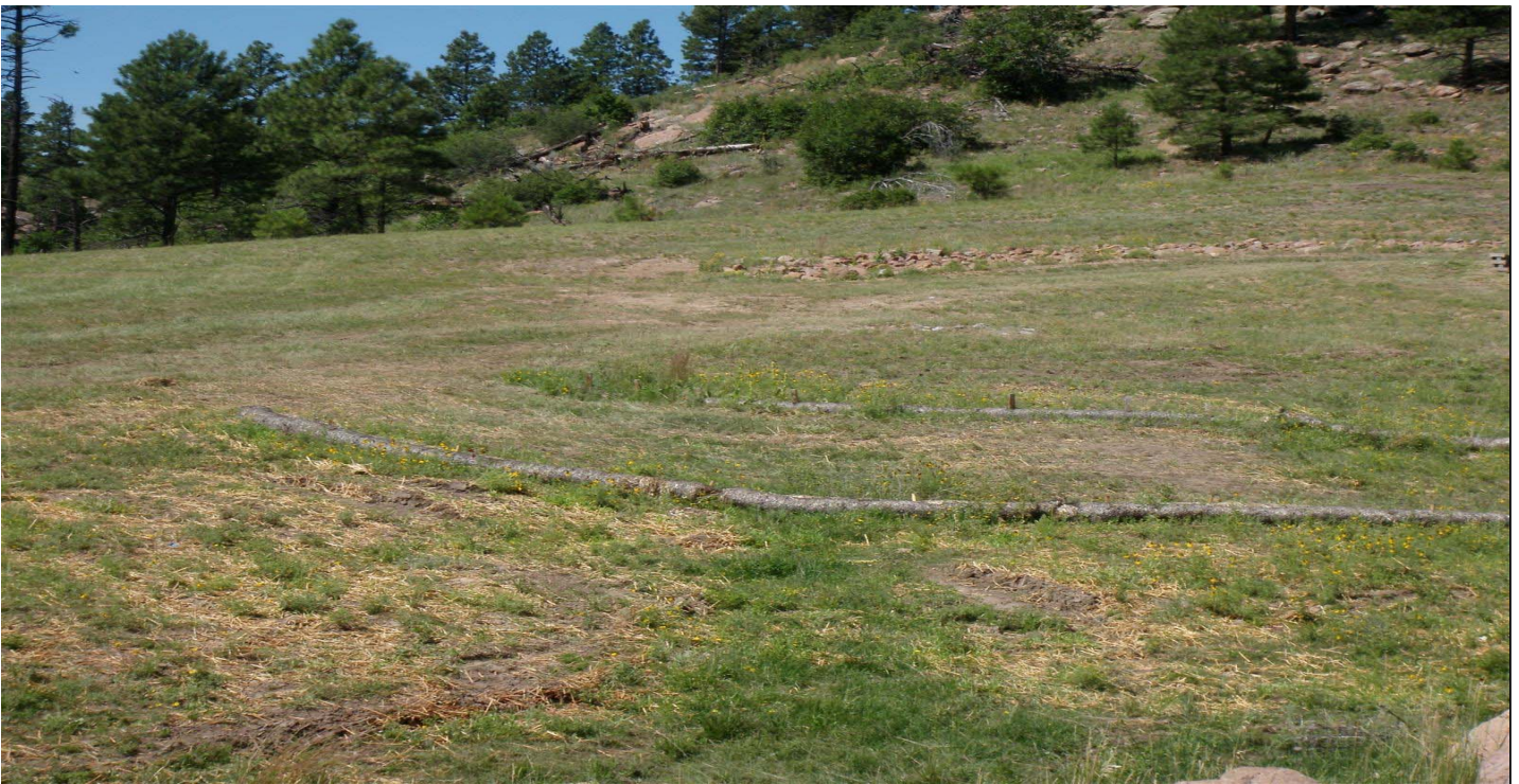
Photo 8524-02r.JPG (taken 08/18/10) V00901010003 : Seed and Mulch - Seed and Wood Mulch; V00902010012 : Established Vegetation - Permanent Vegetation Grasses and Shrubs; V00903060020 : Berms - Straw Wattles; V00903060021 : Berms - Straw Wattles.
