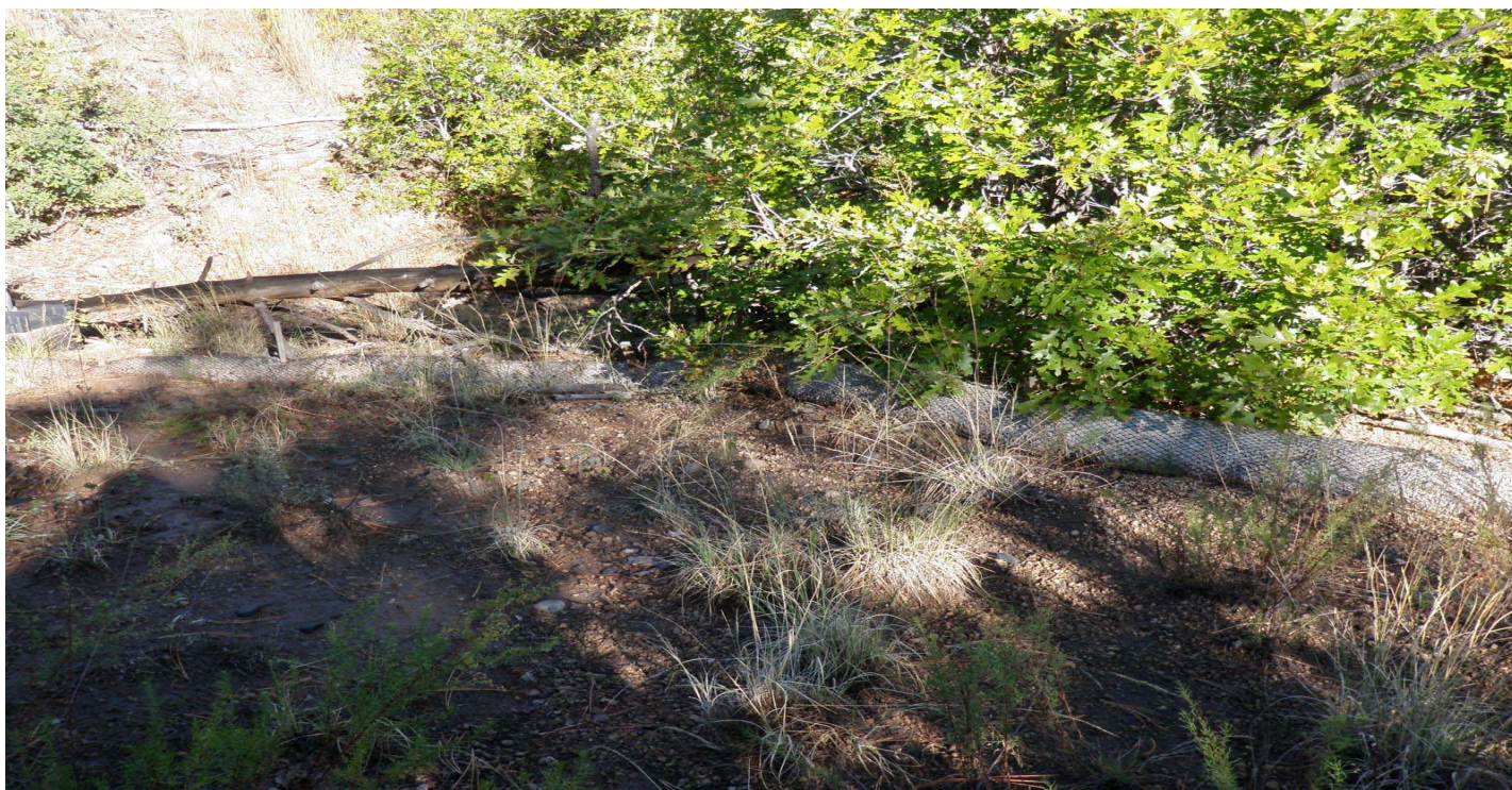
Photo 10875-3r.JPG (taken 10/07/10) W01503060003 : Berms - Straw Wattles.
