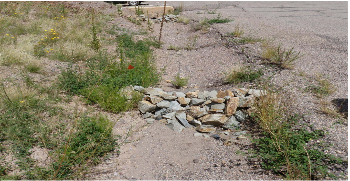
Photo 8503-1r.JPG (taken 08/19/10) C00306010019 : Check Dam - Rock Check Dam; C00306010020 : Check Dam - Rock Check Dam.
