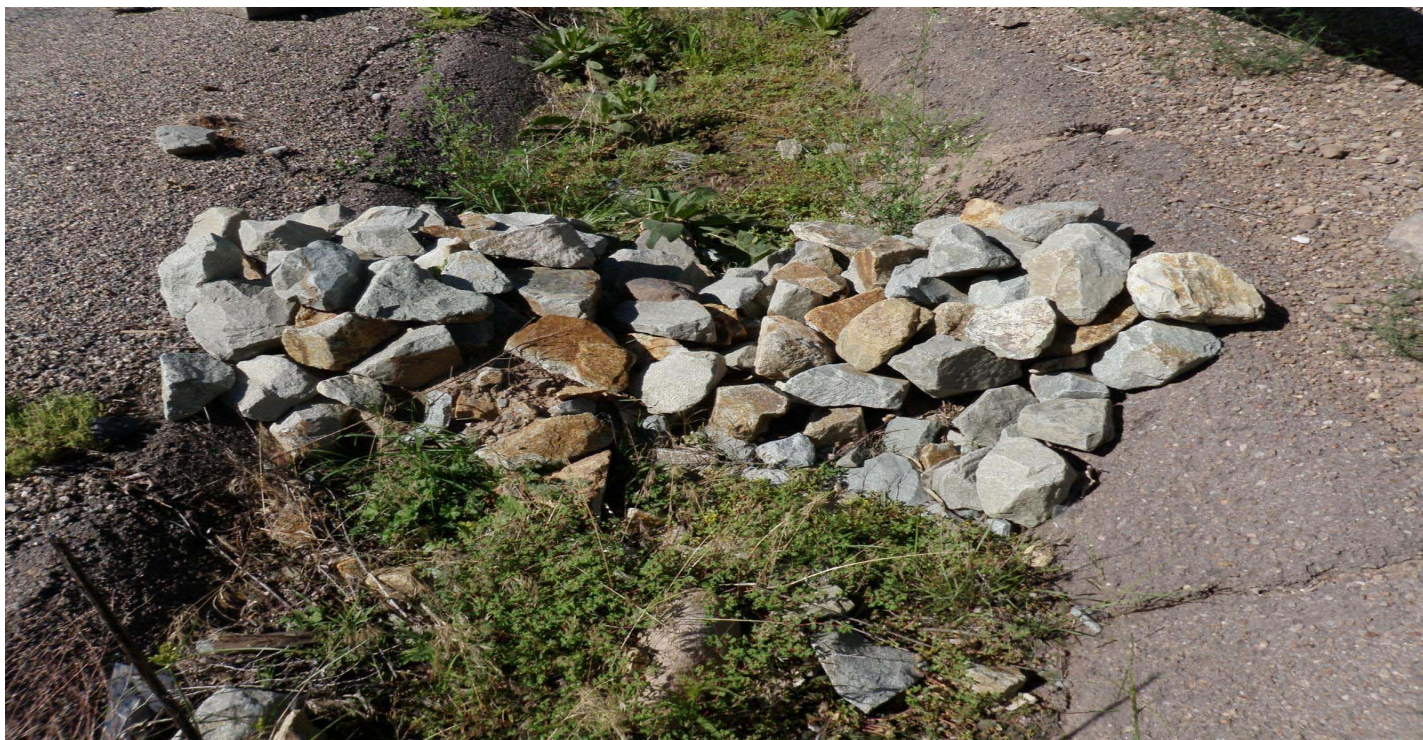
Photo 7523-1r.JPG (taken 08/12/10) J01606010007 : Check Dam - Rock Check Dam.
