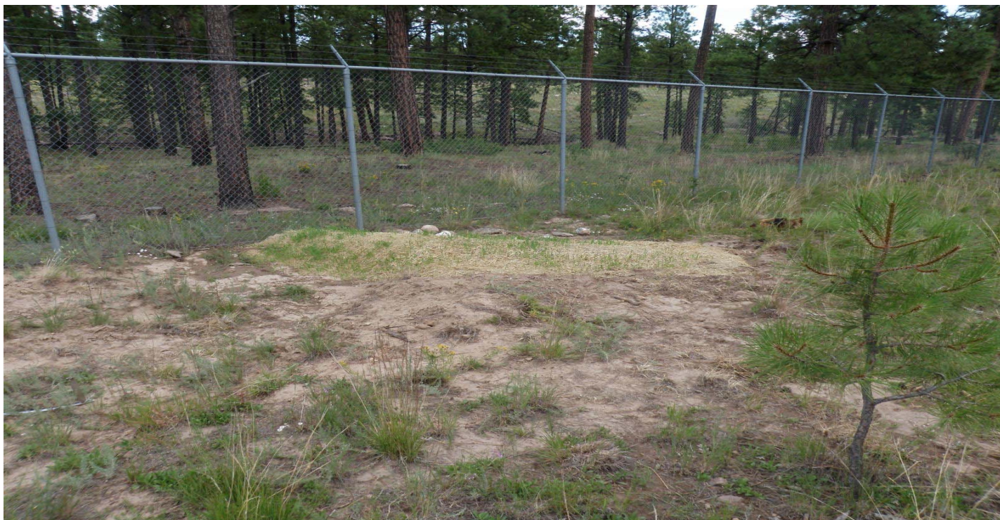
Photo 8518-1r.JPG (taken 08/13/10) E00203010010 : Berms - Earthen Berm.
