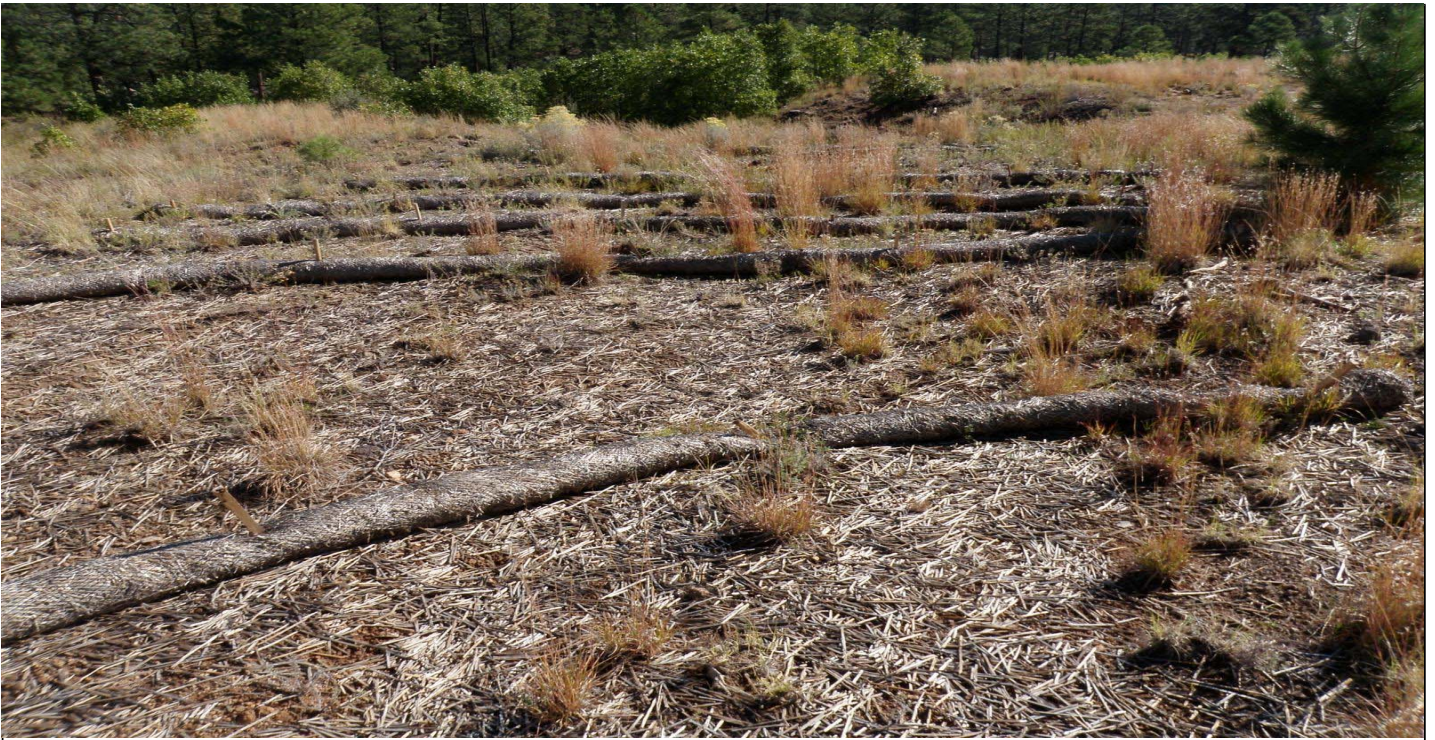
Photo 10877-1r.JPG (taken 10/07/10) W01701010006 : Seed and Mulch - Seed and Wood Mulch; W01703060009 : Berms - Straw Wattles; W01703060010 : Berms - Straw Wattles; W01703060011 : Berms - Straw Wattles; W01703060012 : Berms - Straw Wattles; W01703060015 : Berms - Straw Wattles.
