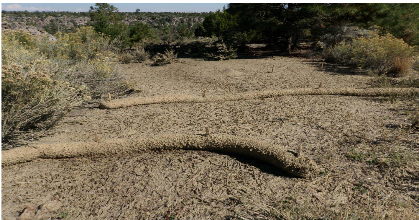
Photo 10872-07r.JPG (taken 10/07/10) H00403060022 : Berms - Straw Wattles; H00403060023 : Berms - Straw Wattles.
