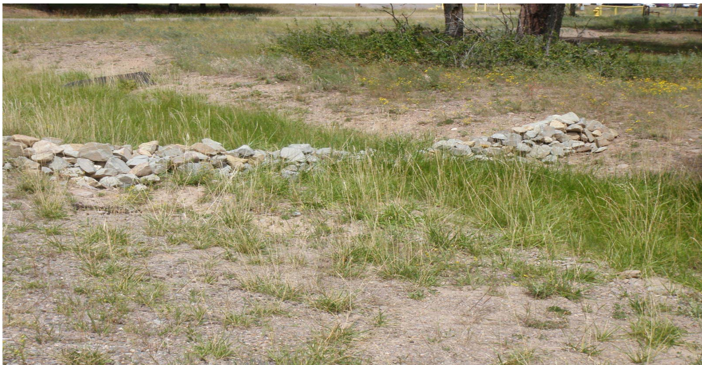
Photo 8788-1r.JPG (taken 09/07/10) W00206010011 : Check Dam - Rock Check Dam.
