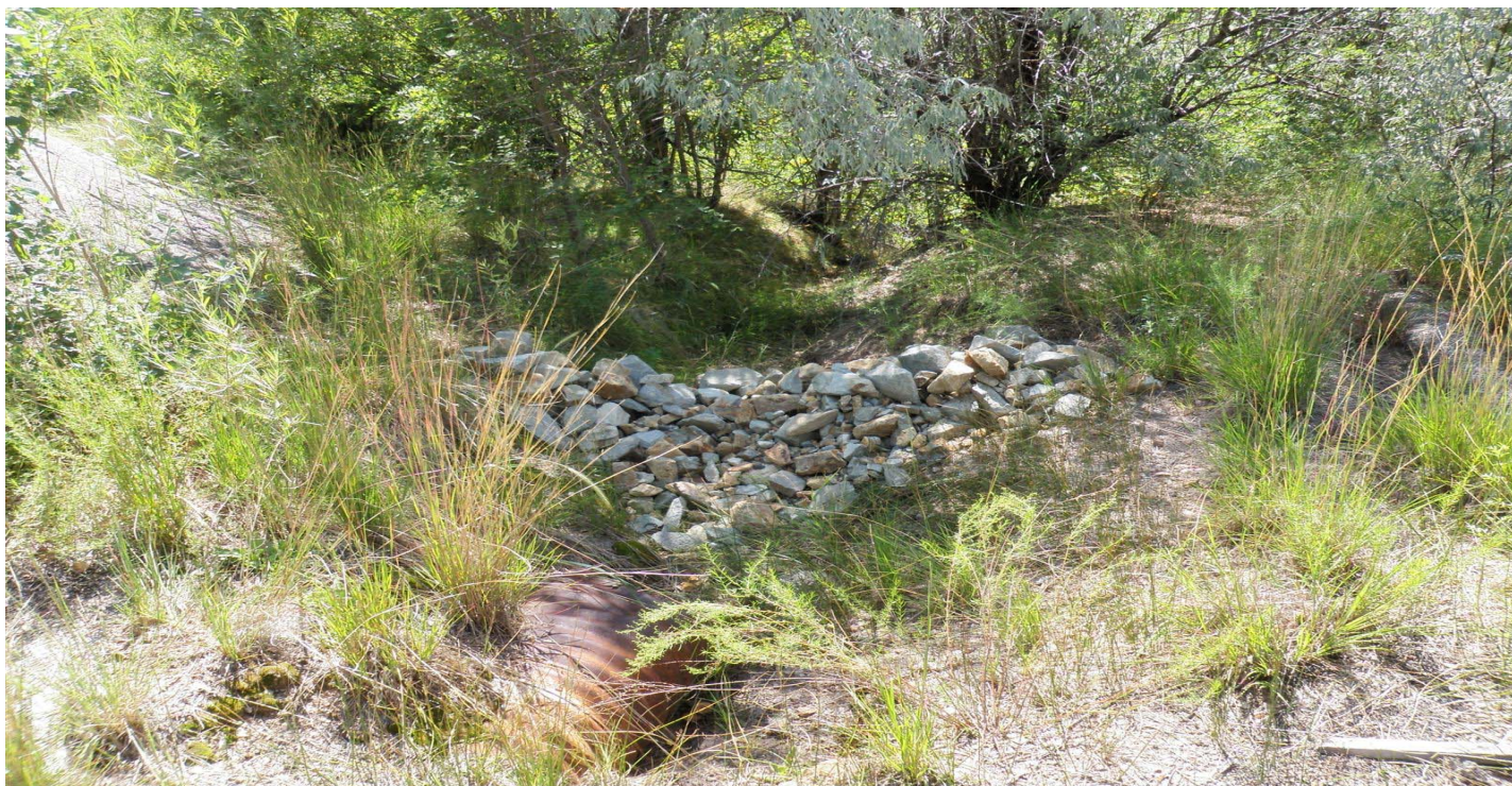
Photo 8529-3r.JPG (taken 08/18/10) V01406010006 : Check Dam - Rock Check Dam.
