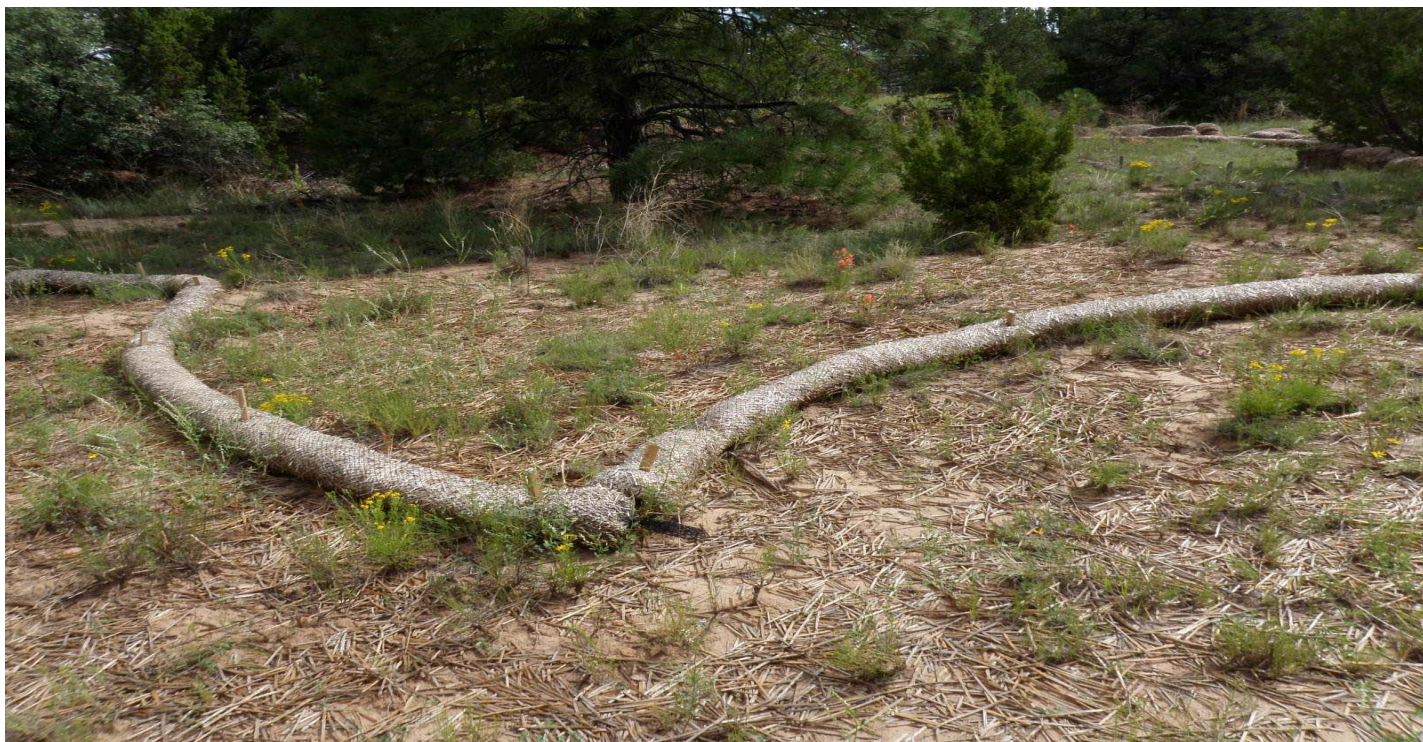
Photo 8519-12.JPG (taken 08/04/10) W01903060012 : Berms - Straw Wattles.
