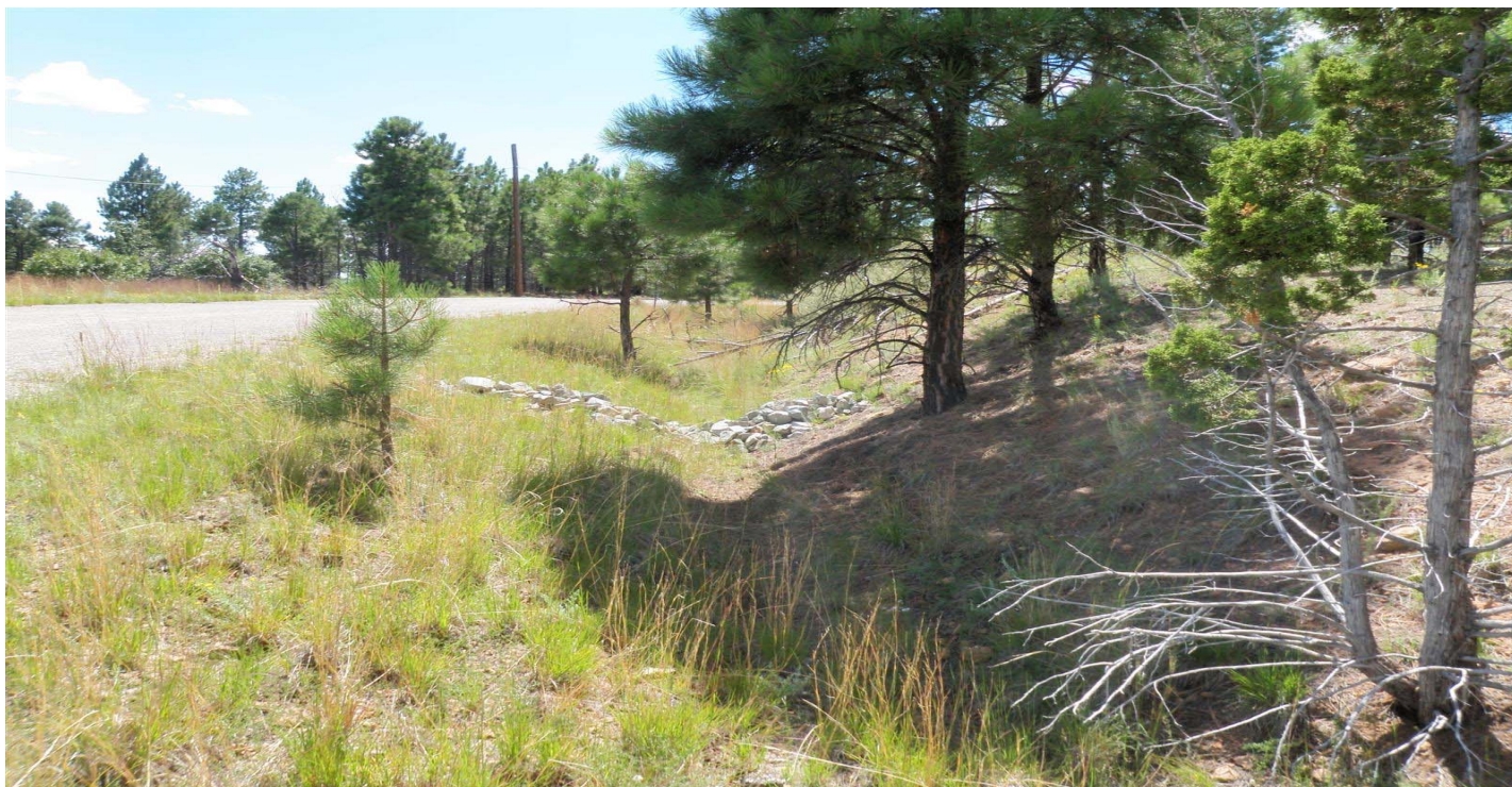
Photo 8530-4r.JPG (taken 08/18/10) W01206010006 : Check Dam - Rock Check Dam.
