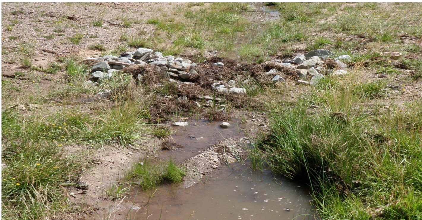
Photo 7800-3r.JPG (taken 08/17/10) W00206010010 : Check Dam - Rock Check Dam.
