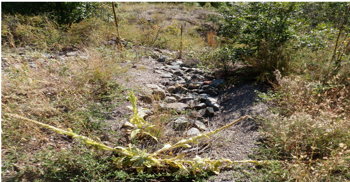
Photo 10878-3r.JPG (taken 10/07/10) W01804060006 : Channel/Swale - Rip Rap.
