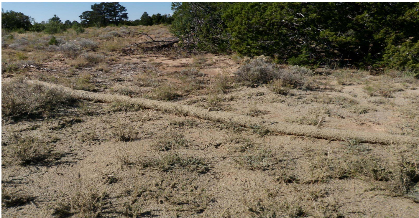
Photo 10872-08r.JPG (taken 10/07/10) H00403060002 : Berms - Straw Wattles.
