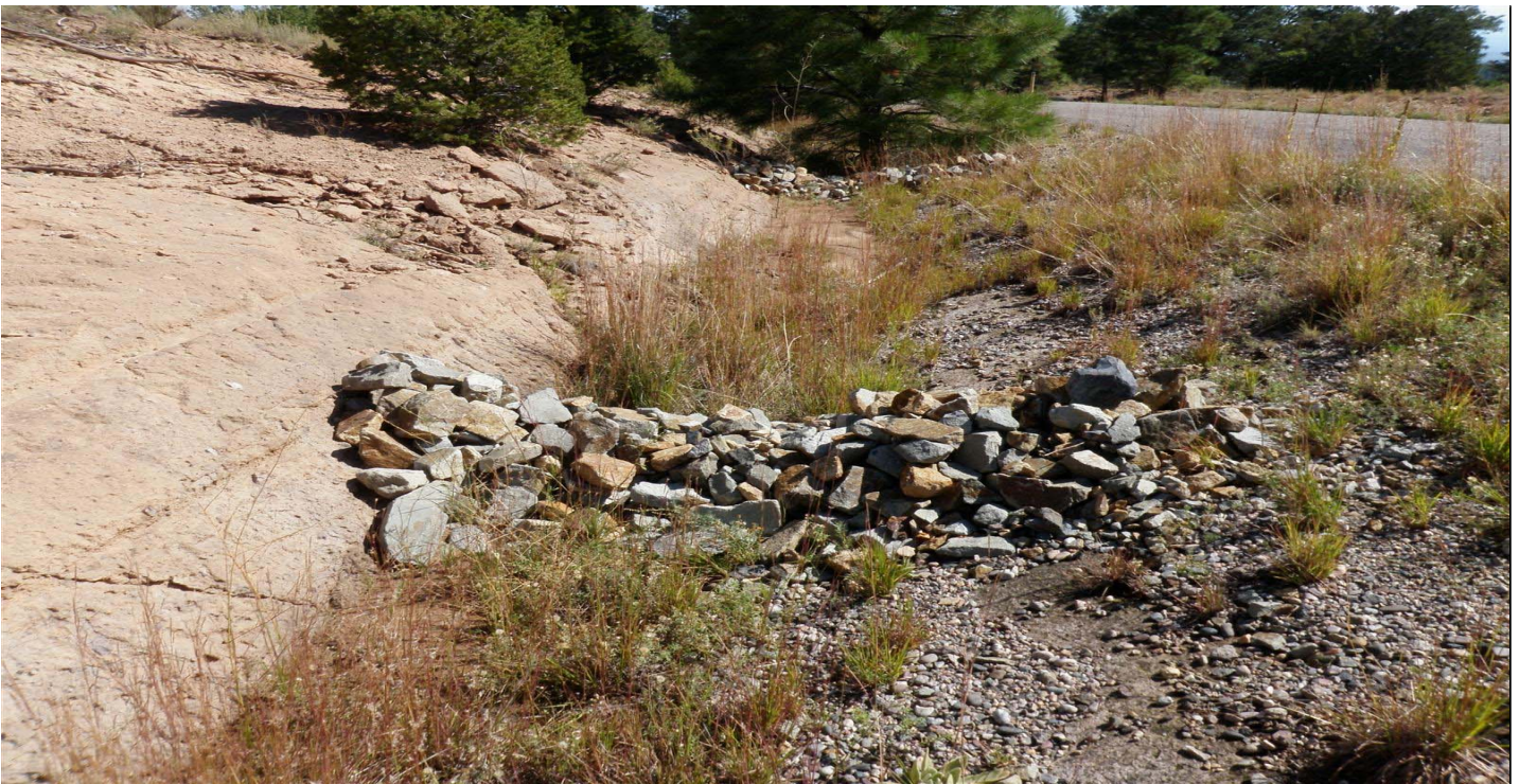
Photo 10873-06r.JPG (taken 10/07/10) H00306010007 : Check Dam - Rock Check Dam; H00306010008 : Check Dam - Rock Check Dam.
