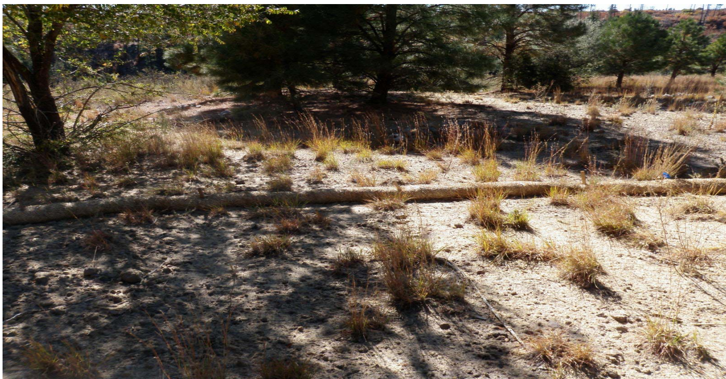
Photo 11459-1r.JPG (taken 10/26/10) J01403060014 : Berms - Straw Wattles.
