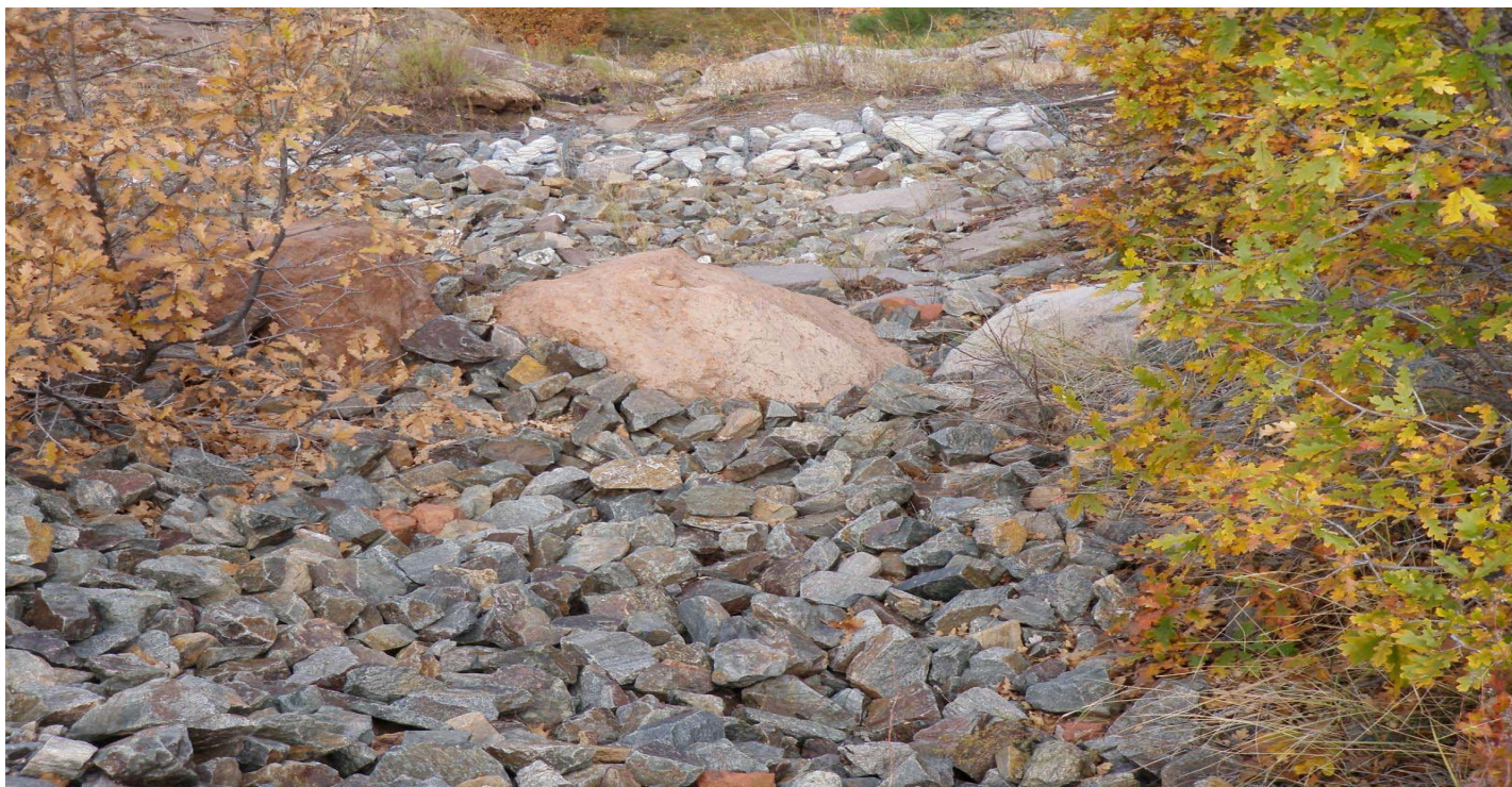
Photo 11465-7r.JPG (taken 10/22/10) V008A04060005 : Channel/Swale - Rip Rap; V008A07010003 : Gabions - Gabions.
