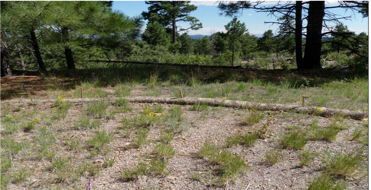
Photo 7802-2r.JPG (taken 08/17/10) W00803060013 : Berms - Straw Wattles.
