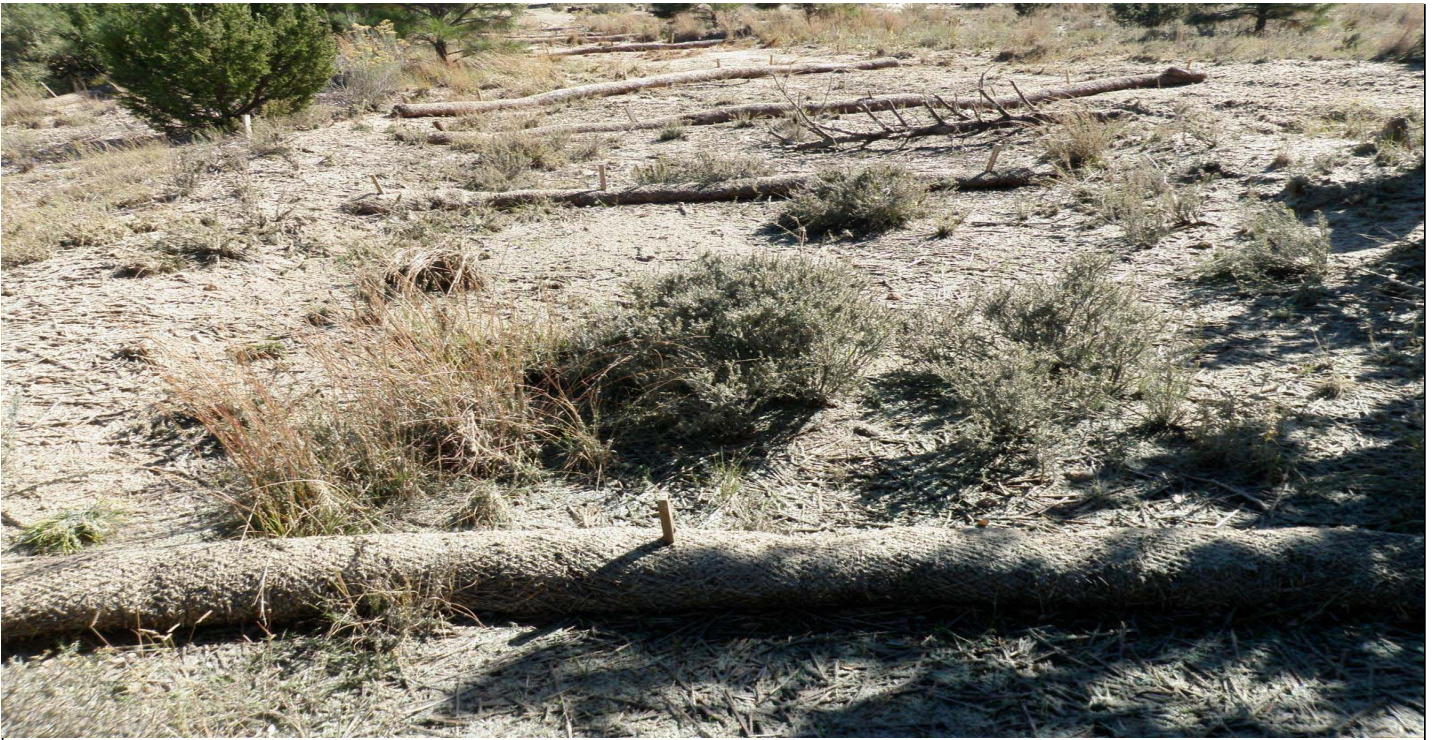
Photo 10872-10r.JPG (taken 10/07/10) H00403060004 : Berms - Straw Wattles; H00403060005 : Berms - Straw Wattles; H00403060006 : Berms - Straw Wattles.
