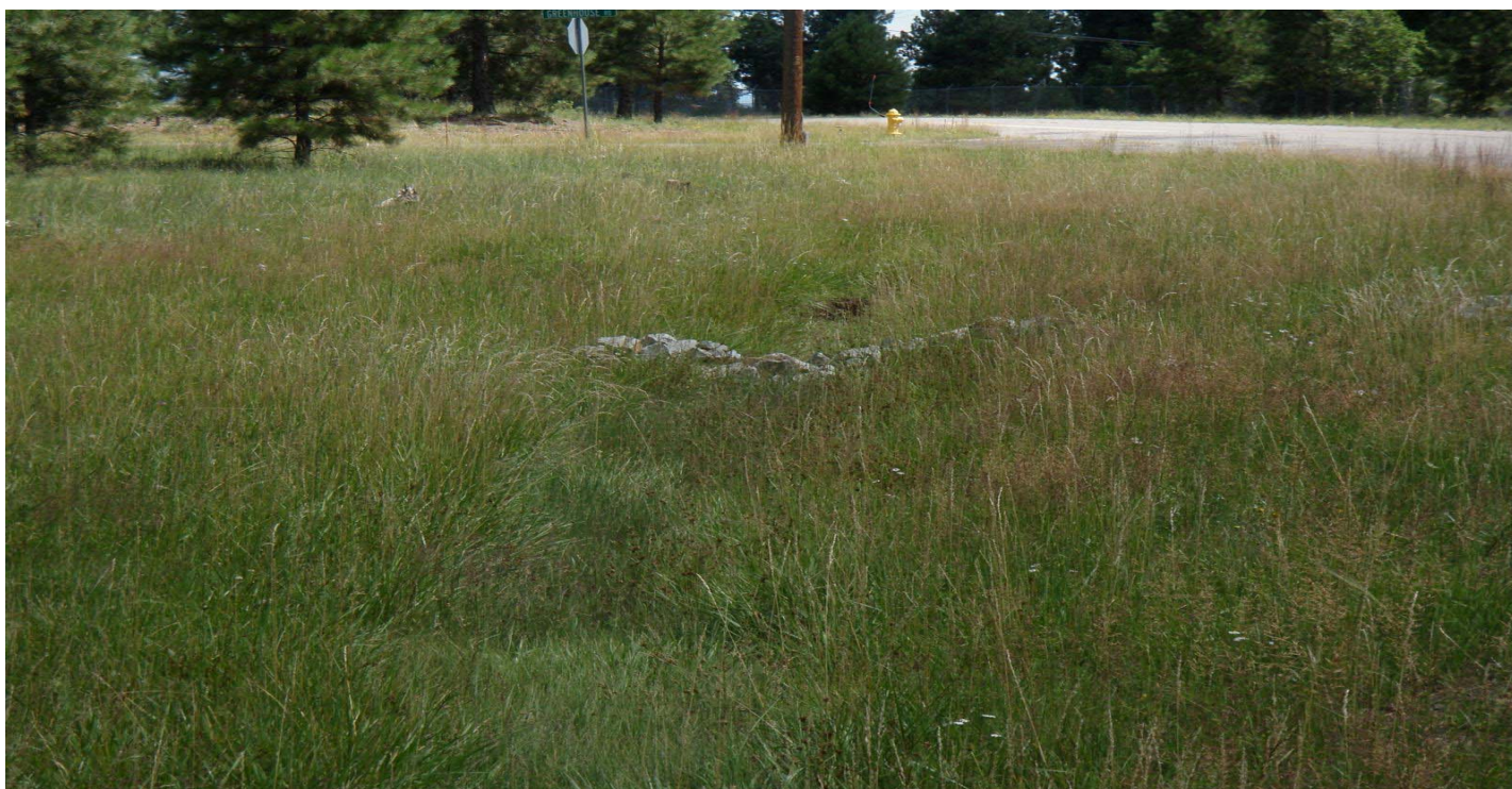
Photo 7800-5r.JPG (taken 08/17/10) W00206010012 : Check Dam - Rock Check Dam.
