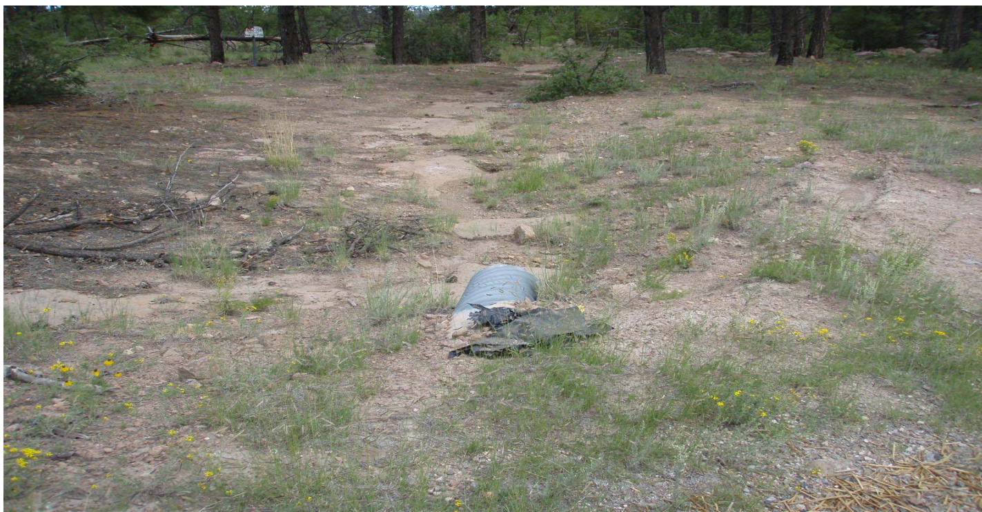
Photo 8531-10r.JPG (taken 08/23/10) W00604040011 : Channel/Swale - Culvert.
