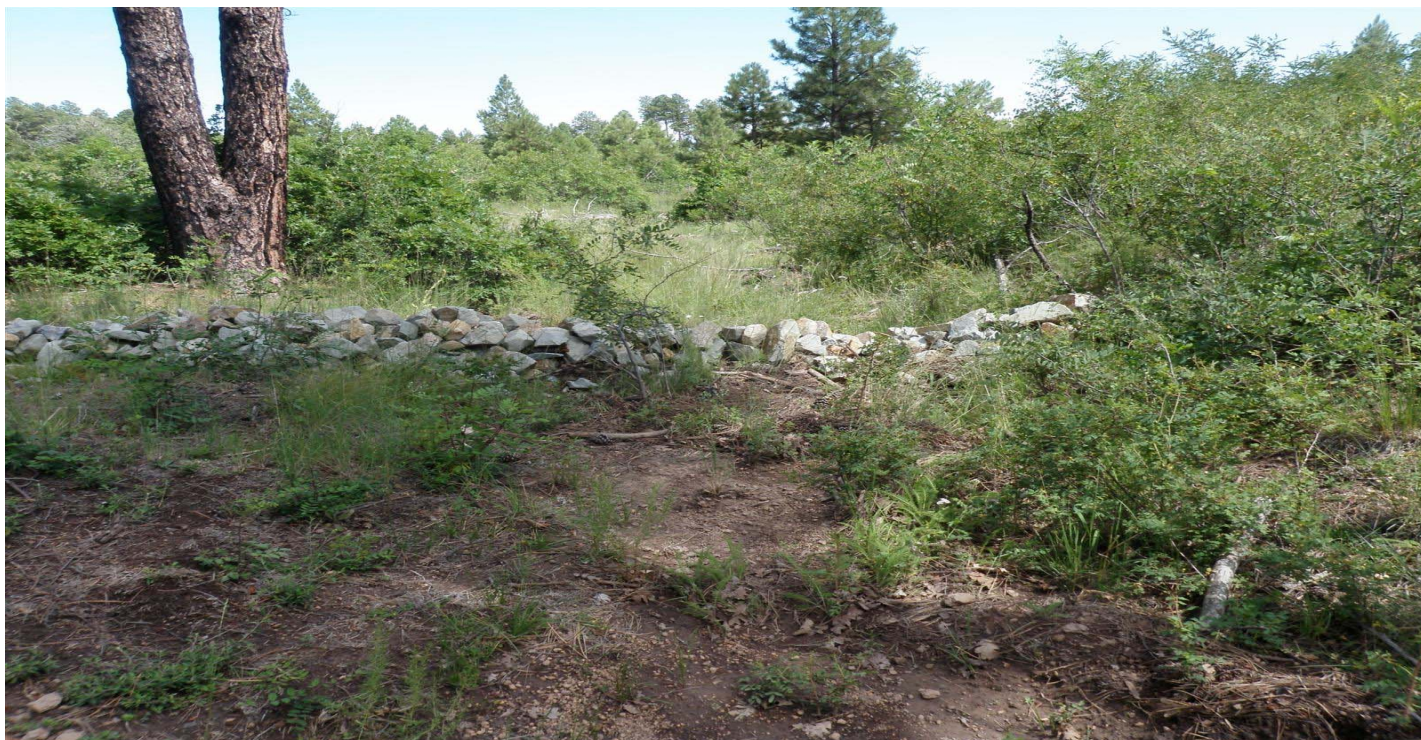
Photo 7807-2r.JPG (taken 08/17/10) W00306010005 : Check Dam - Rock Check Dam.
