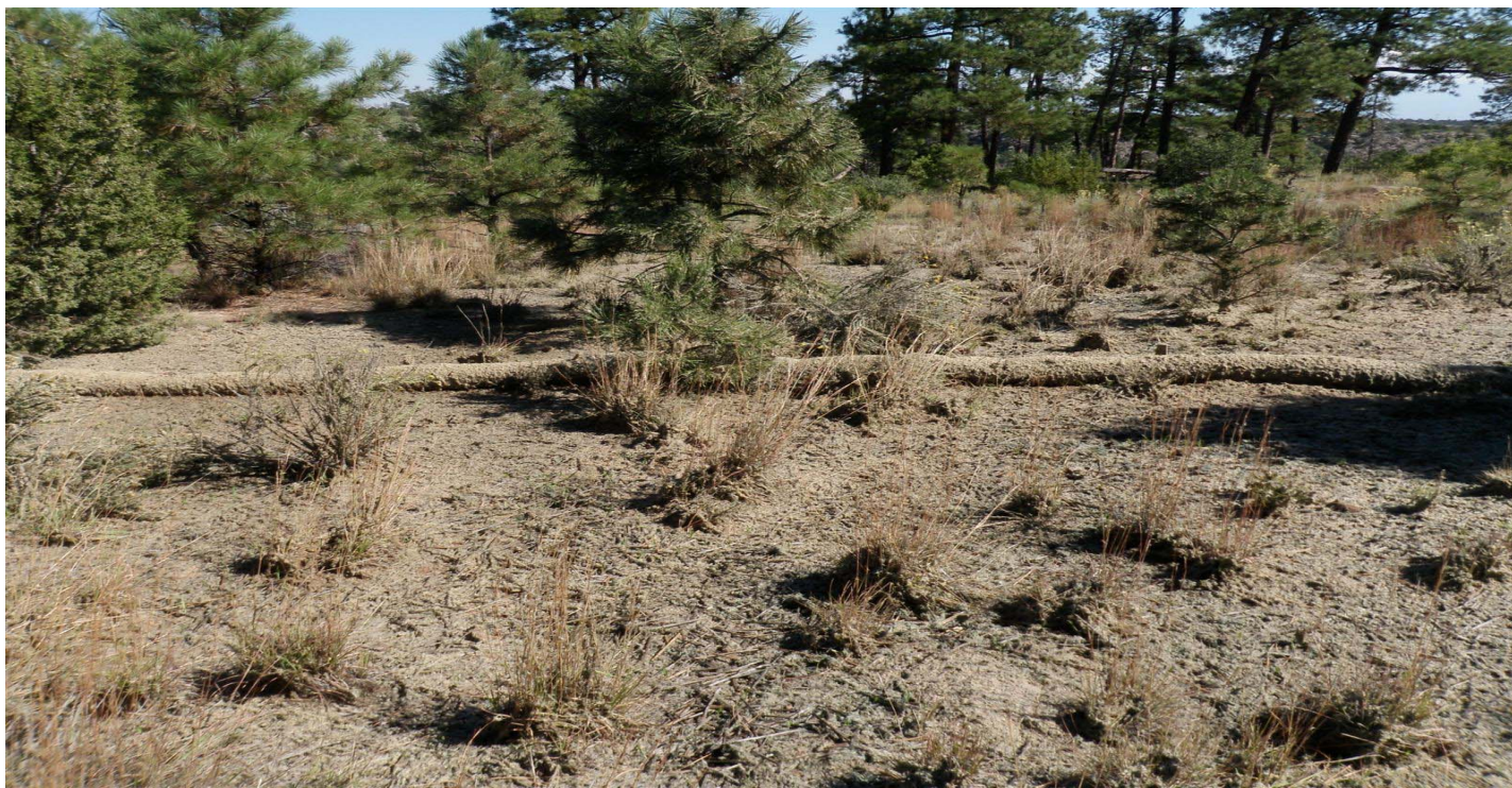
Photo 10872-02r.JPG (taken 10/07/10) H00403060019 : Berms - Straw Wattles.
