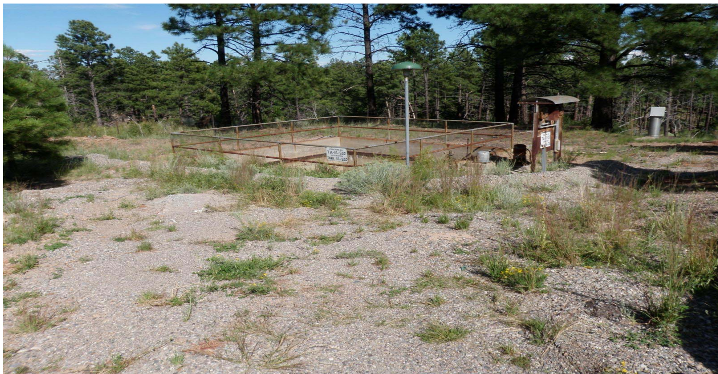
Photo 7804-1r.JPG (taken 08/17/10) W012A03020003 : Berms - Base Course Berm.
