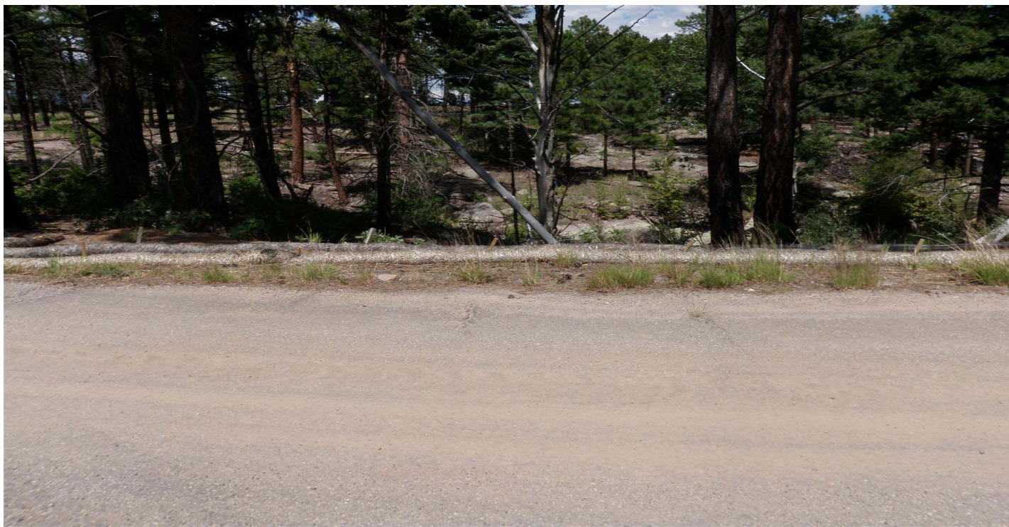
Photo 8527-5r.JPG (taken 08/18/10) V00703060007 : Berms - Straw Wattles.
