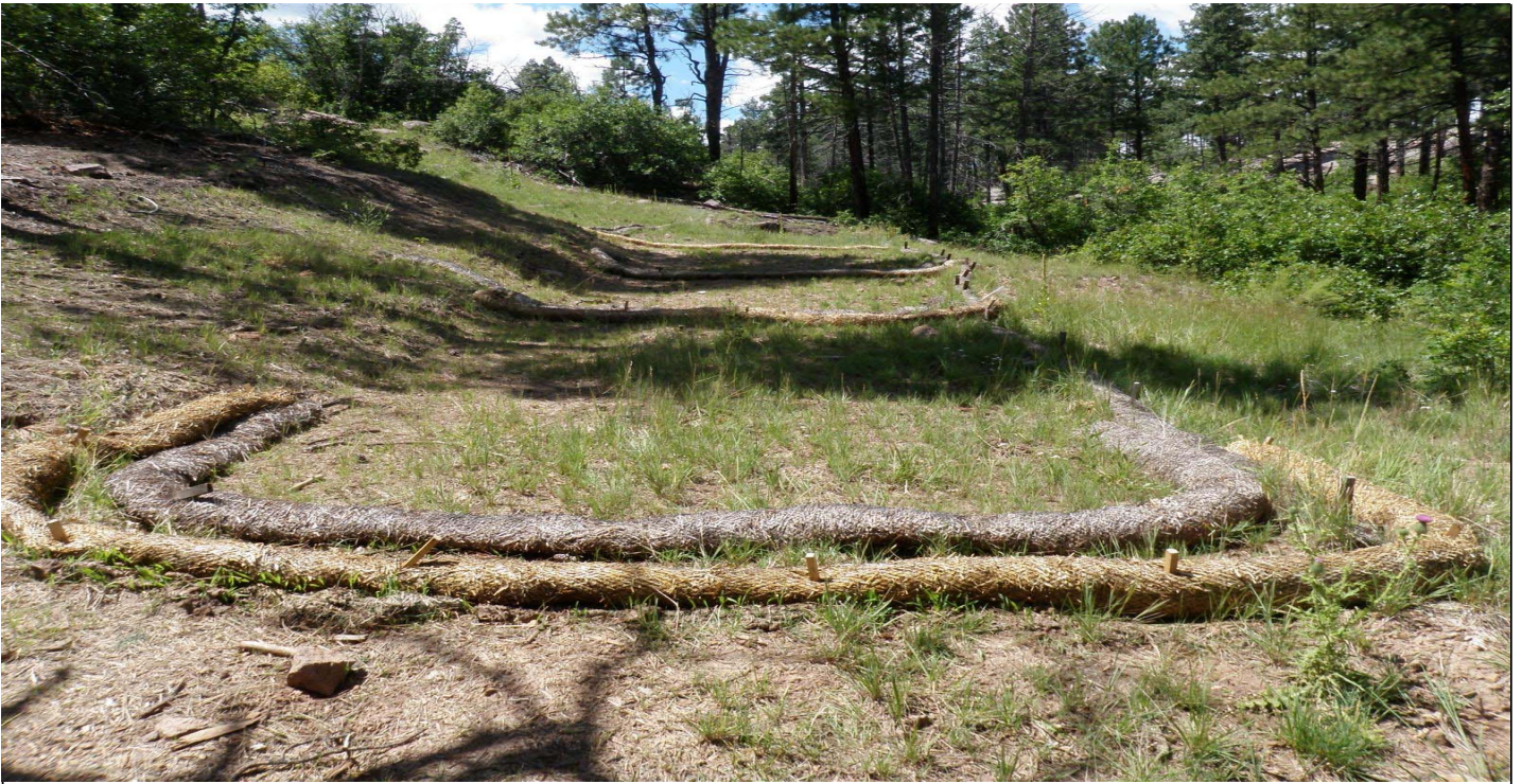
Photo 8527-1r.JPG (taken 08/18/10) V00703060012 : Berms - Straw Wattles; V00703060013 : Berms - Straw Wattles; V00703060014 : Berms - Straw Wattles; V00703060015 : Berms - Straw Wattles.
