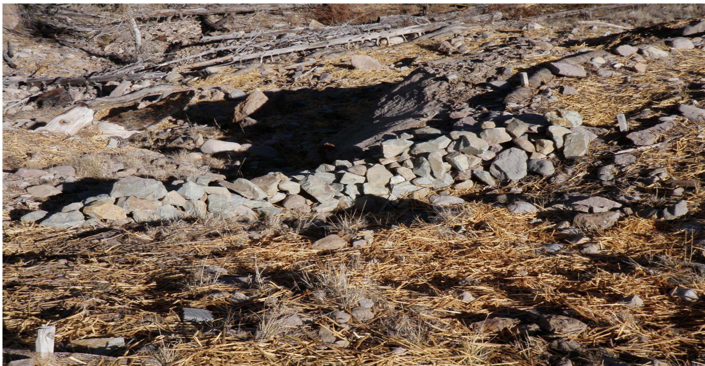
Photo 11699-2r.JPG (taken 11/15/10) V00506010011 : Check Dam - Rock Check Dam.
