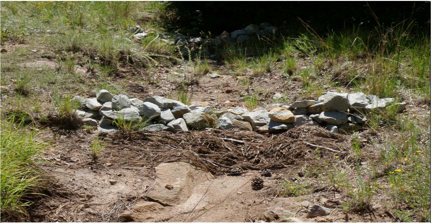
Photo 8524-06r.JPG (taken 08/18/10) V00906010015 : Check Dam - Rock Check Dam; V00906010016 : Check Dam - Rock Check Dam.
