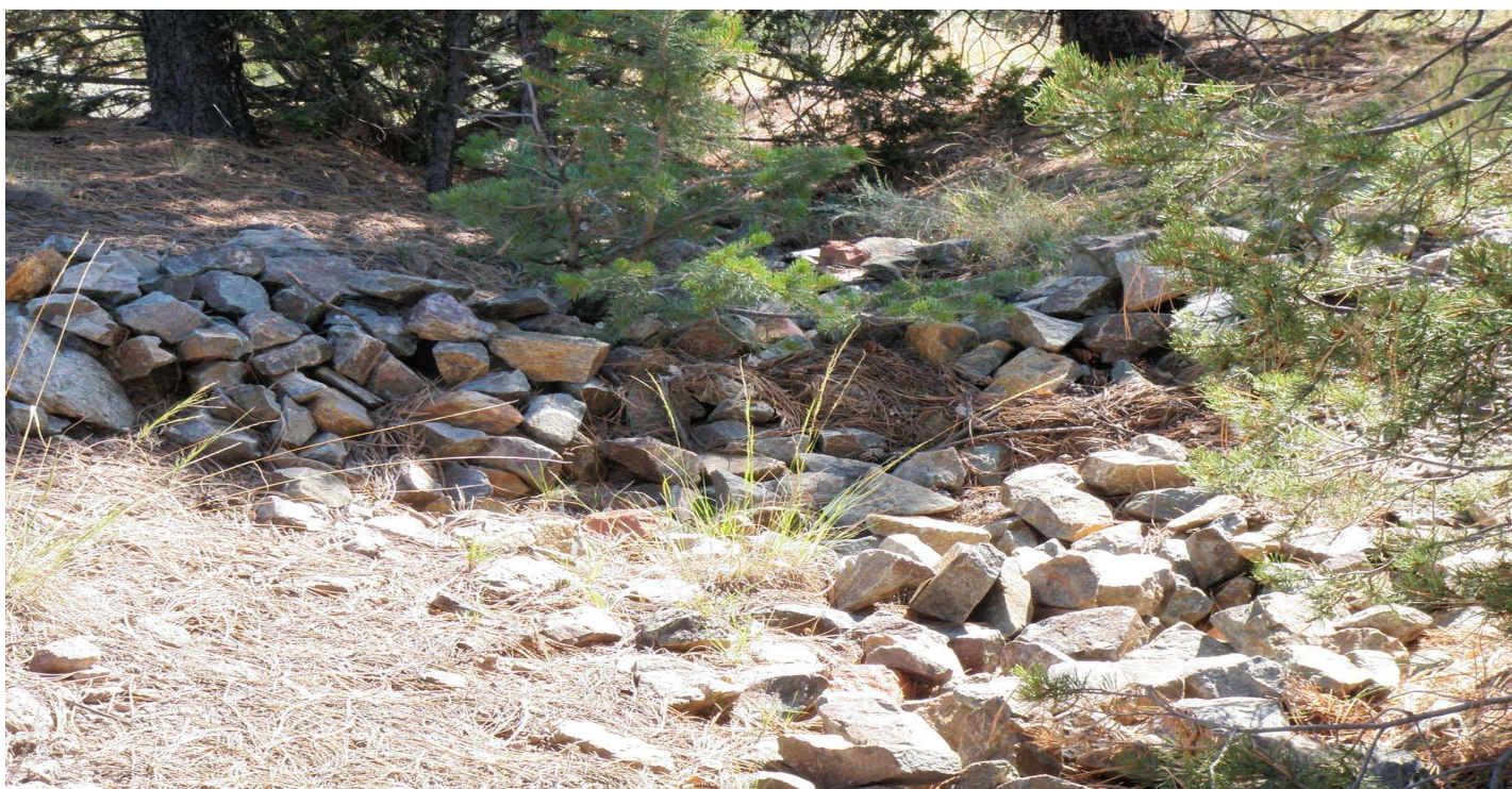
Photo 10873-10r.JPG (taken 10/07/10) H00306010002 : Check Dam - Rock Check Dam.
