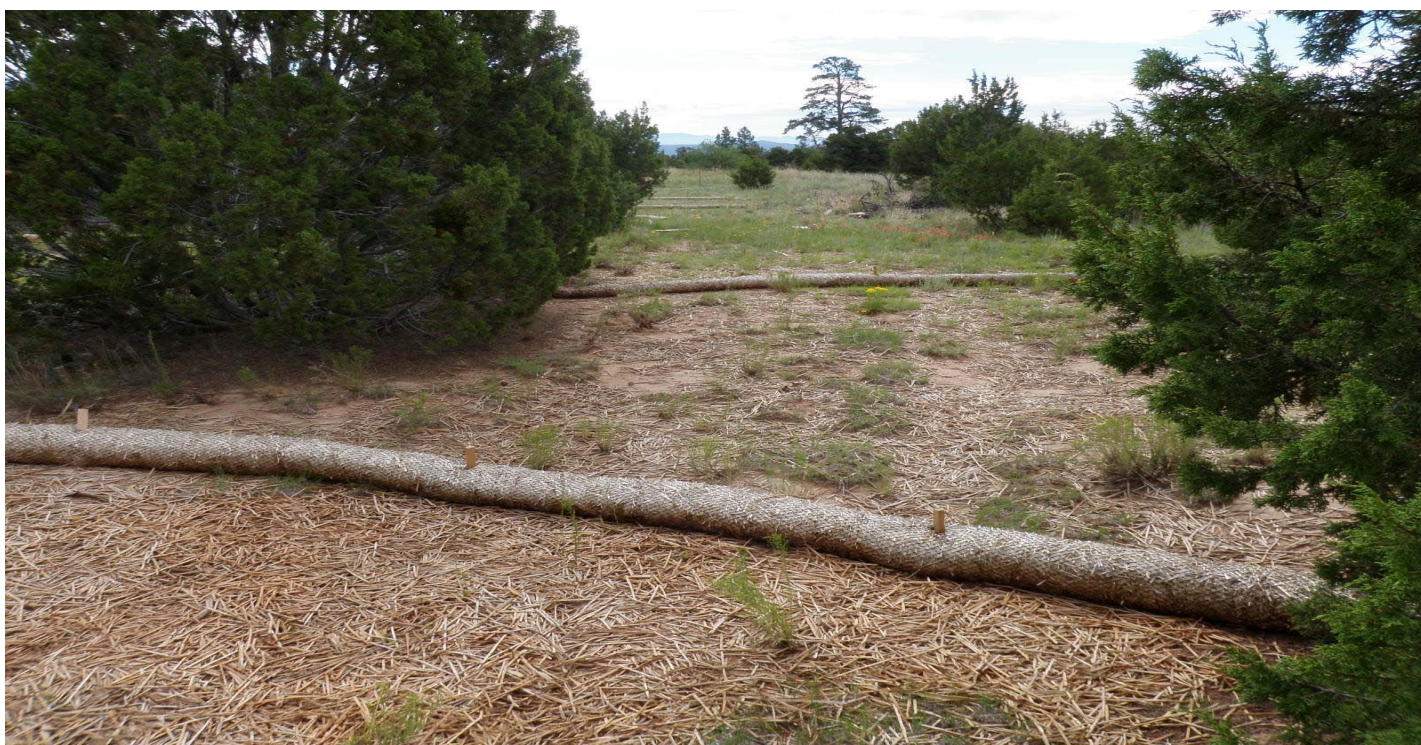
Photo 8519-3.JPG (taken 08/04/10) W01903060029 : Berms - Straw Wattles; W01903060031 : Berms - Straw Wattles; W01903060032 : Berms - Straw Wattles; W01903060035 : Berms - Straw Wattles.
