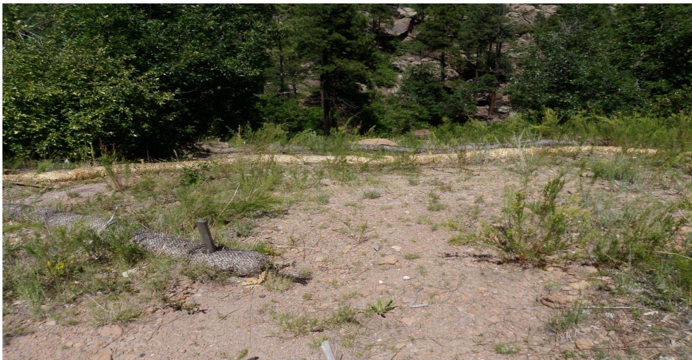
Photo 8527-9r.JPG (taken 08/18/10) V00703060011 : Berms - Straw Wattles.
