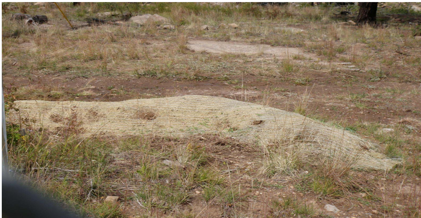
Photo 10881-2r.JPG (taken 10/04/10) E00702010001 : Established Vegetation - Permanent Vegetation Grasses and Shrubs; E00703010004 : Berms - Earthen Berm.
