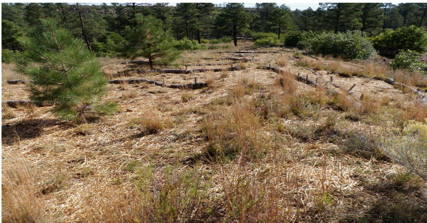
Photo 10878-4r.JPG (taken 10/07/10) W01801010015 : Seed and Mulch - Seed and Wood Mulch; W01803060014 : Berms - Straw Wattles.
