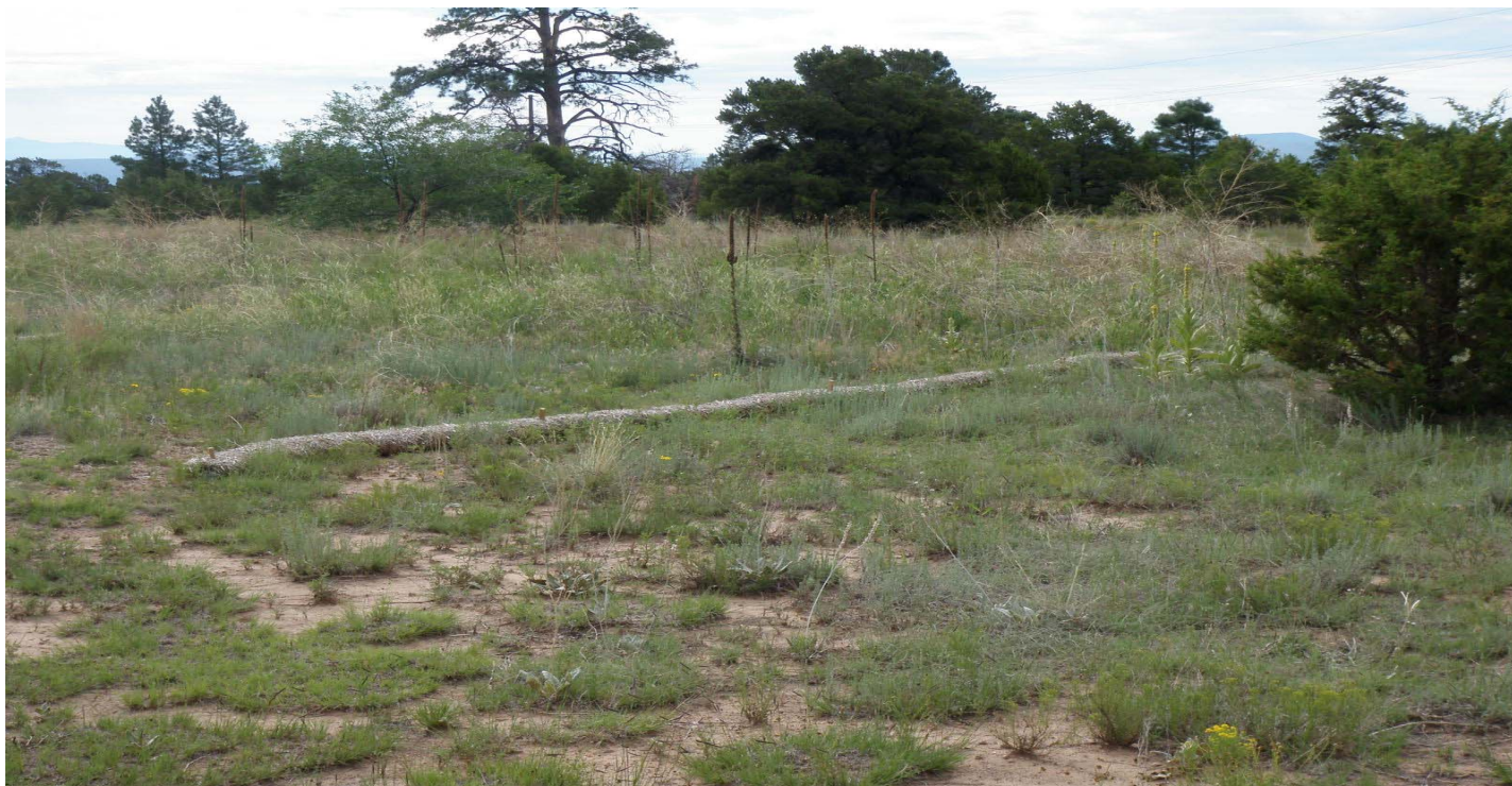
Photo 8519-8.JPG (taken 08/04/10) W01903060027 : Berms - Straw Wattles.
