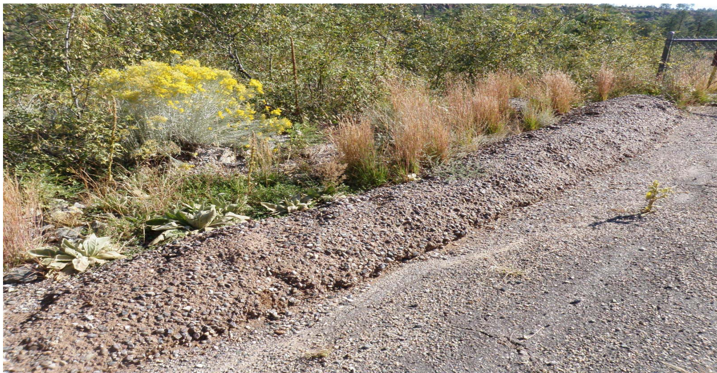
Photo 10876-2r.JPG (taken 10/07/10) W01603020007 : Berms - Base Course Berm.
