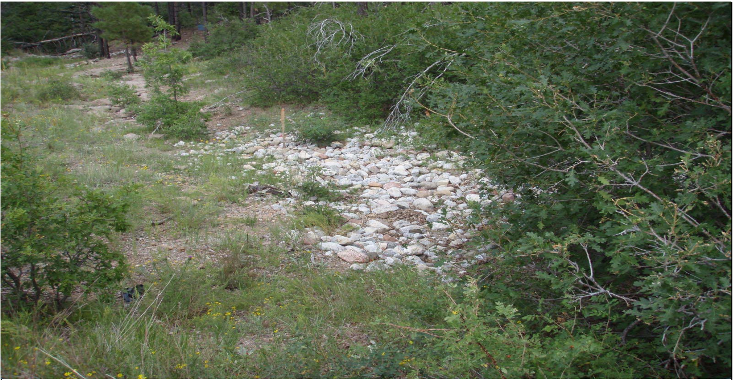
Photo 8531-05r.JPG (taken 08/23/10) W00604060006 : Channel/Swale - Rip Rap.
