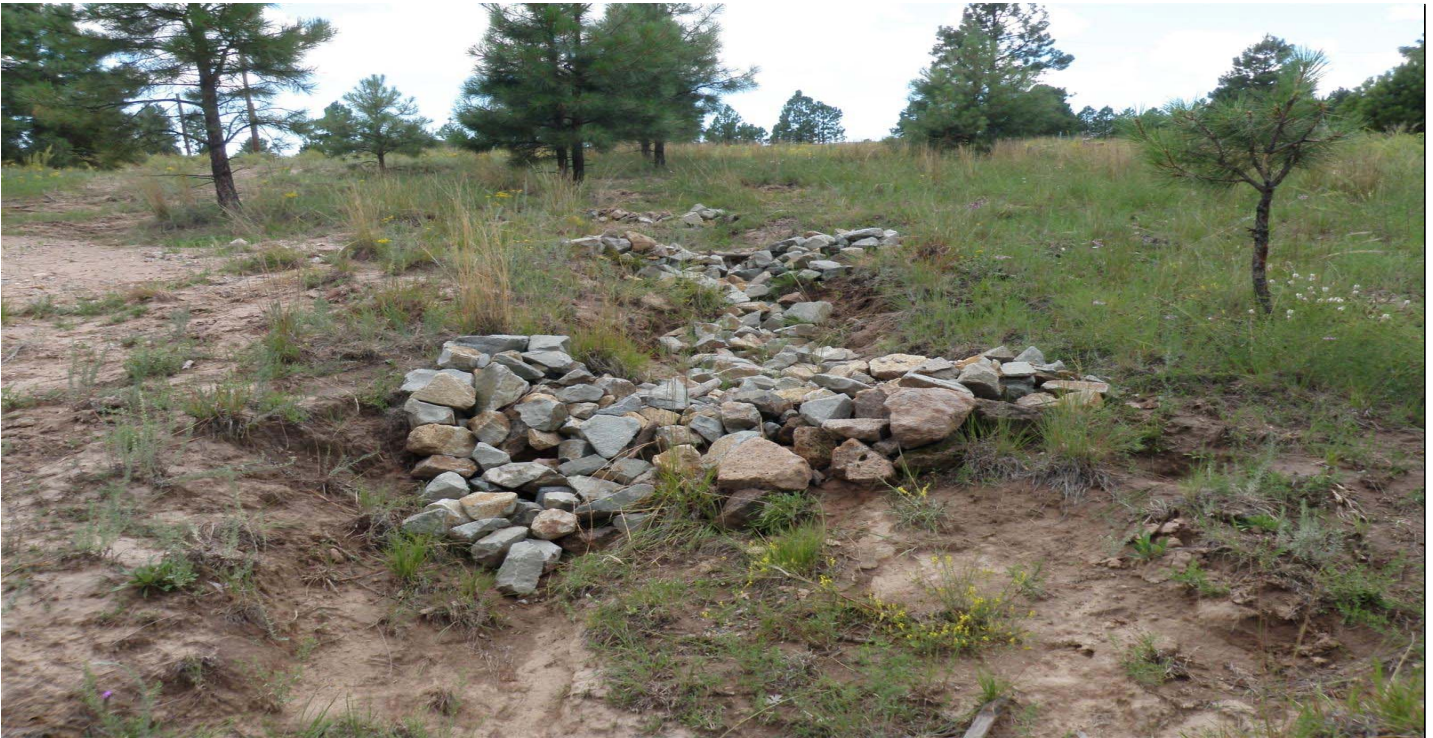
Photo 8518-3r.JPG (taken 08/13/10) E00206010006 : Check Dam - Rock Check Dam; E00206010007 : Check Dam - Rock Check Dam; E00206010008 : Check Dam - Rock Check Dam.
