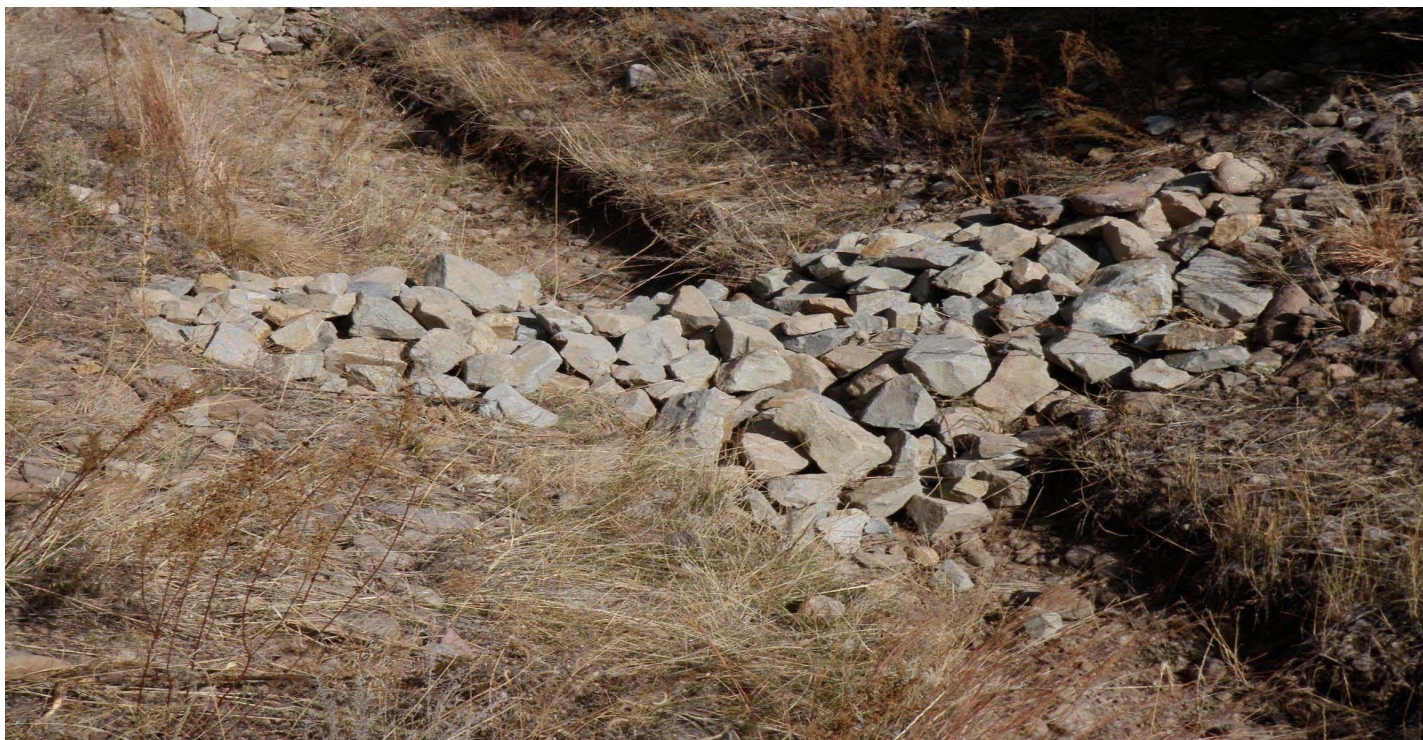
Photo 11699-4r.JPG (taken 11/15/10) V00506010013 : Check Dam - Rock Check Dam.
