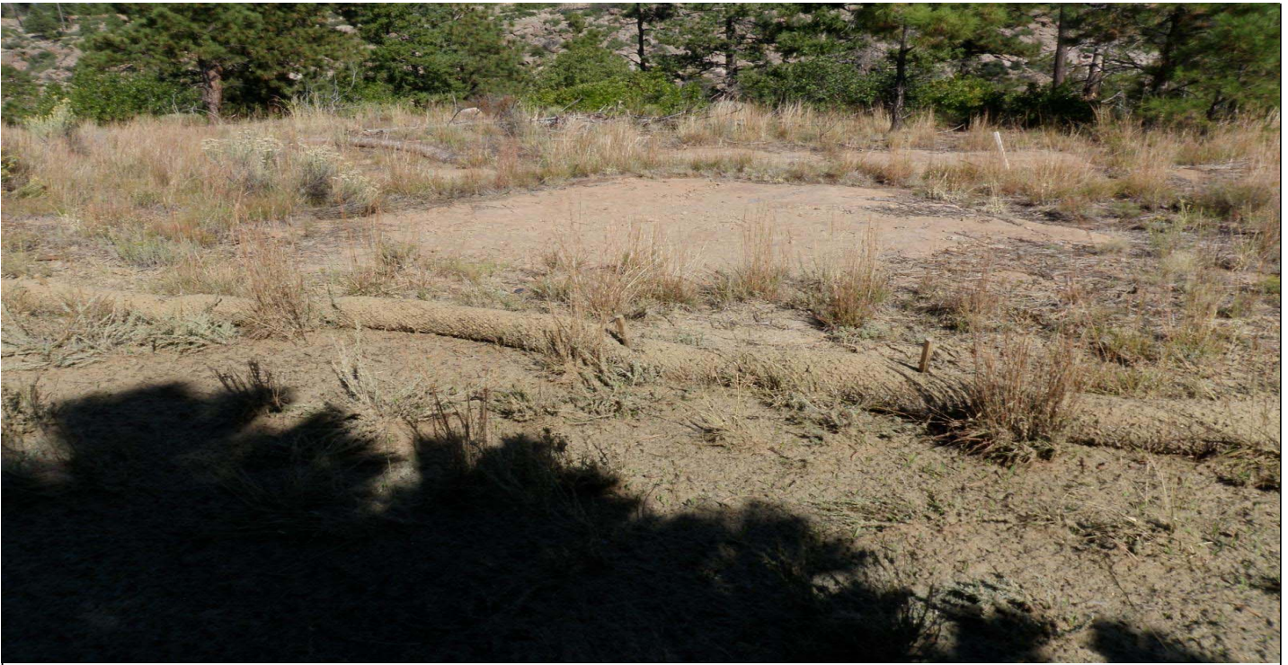
Photo 10872-11r.JPG (taken 10/07/10) H00403060010 : Berms - Straw Wattles.
