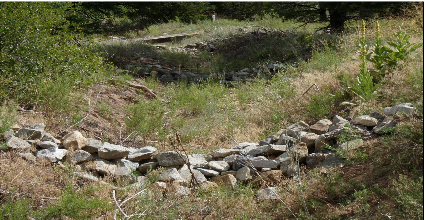
Photo 8519-15.JPG (taken 08/04/10) W01906010006 : Check Dam - Rock Check Dam; W01906010007 : Check Dam - Rock Check Dam; W01906010008 : Check Dam - Rock Check Dam.
