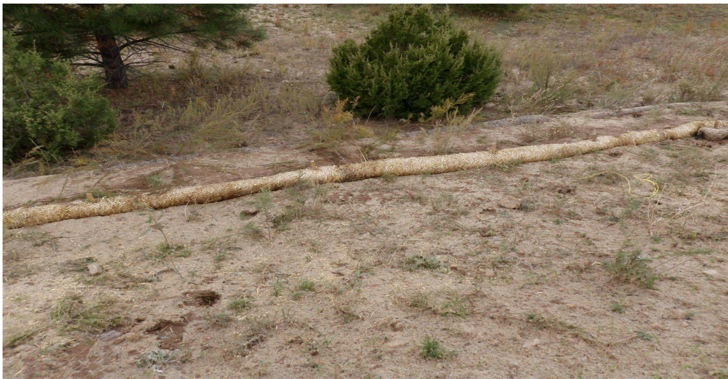
Photo 11461-1r.JPG (taken 10/22/10) E00503060012 : Berms - Straw Wattles.
