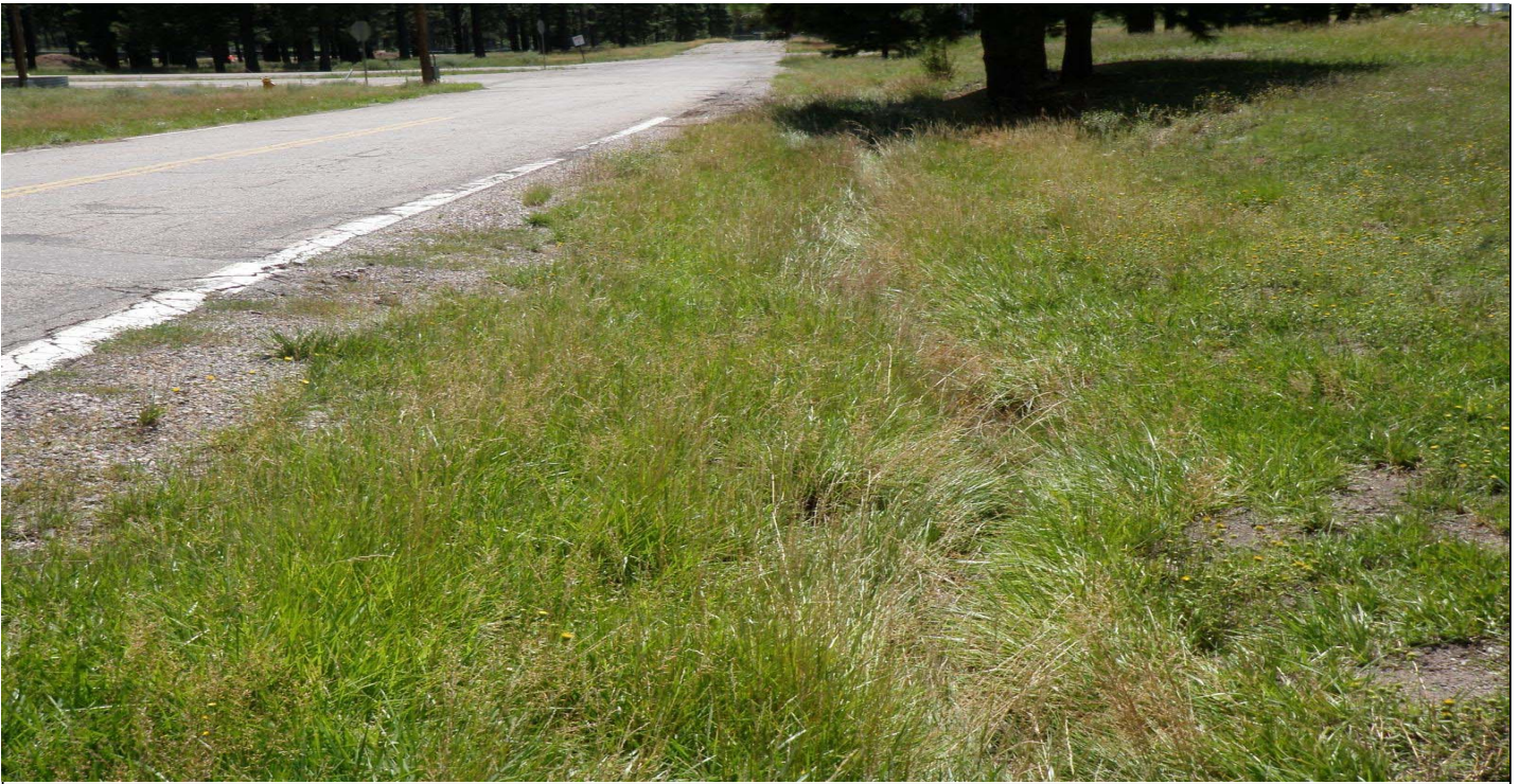
Photo 7800-2r.JPG (taken 08/17/10) W00202010001 : Established Vegetation - Permanent Vegetation Grasses and Shrubs; W00204070003 : Channel/Swale - Vegetated Swale.
