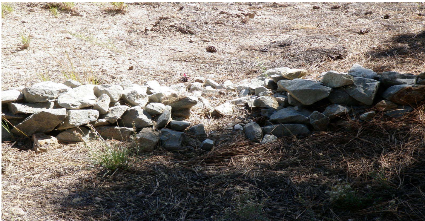
Photo 10865-3r.JPG (taken 10/07/10) J01406010011 : Check Dam - Rock Check Dam.
