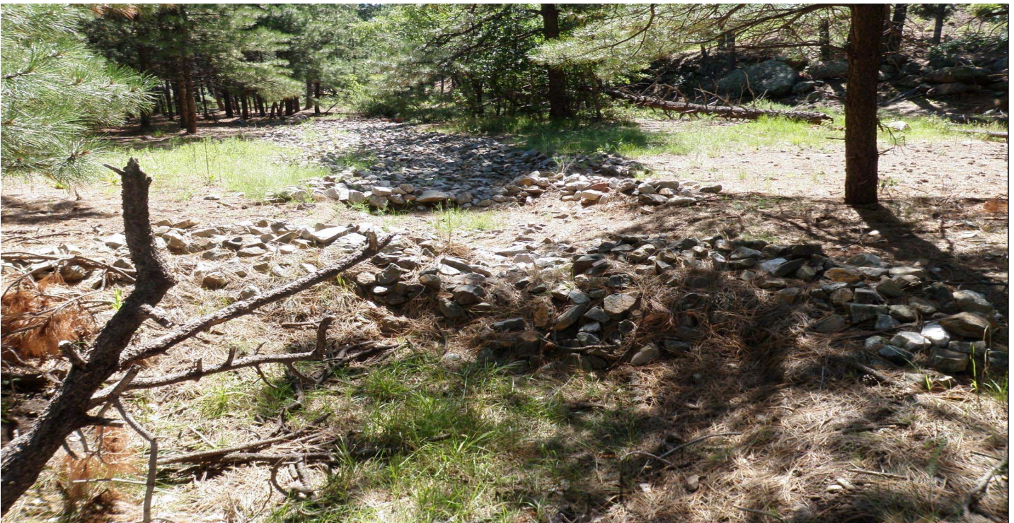
Photo 8522-09r.JPG (taken 08/18/10) V00304060001 : Channel/Swale - Rip Rap; V00306010006 : Check Dam - Rock Check Dam; V00306010012 : Check Dam - Rock Check Dam.
