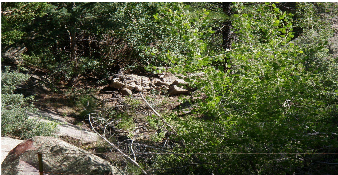
Photo 7806-4r.JPG (taken 08/17/10) W01102010003 : Established Vegetation - Permanent Vegetation Grasses and Shrubs; W01102020004 : Established Vegetation - Permanent Vegetation Forested/Needle Cast; W01106010002 : Check Dam - Rock Check Dam.
