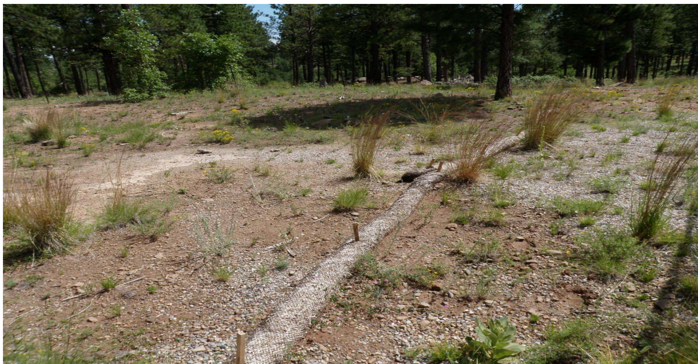
Photo 7807-1r.JPG (taken 08/17/10) W00302010001 : Established Vegetation - Permanent Vegetation Grasses and Shrubs; W00302020002 : Established Vegetation - Permanent Vegetation Forested/Needle Cast; W00303060003 : Berms - Straw Wattles.
