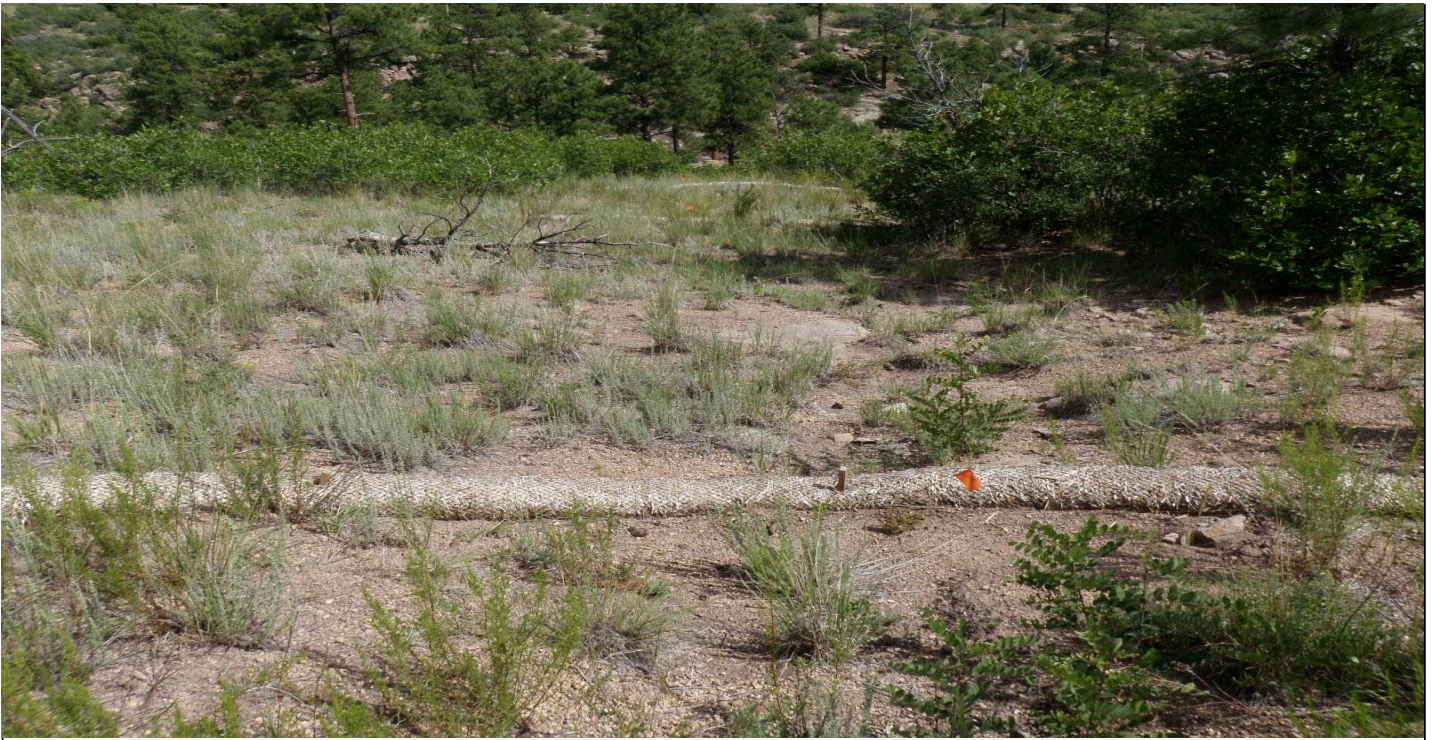
Photo 8516-4.JPG (taken 08/04/10) W02003060005 : Berms - Straw Wattles; W02003060006 : Berms - Straw Wattles; W02003060007 : Berms - Straw Wattles.
