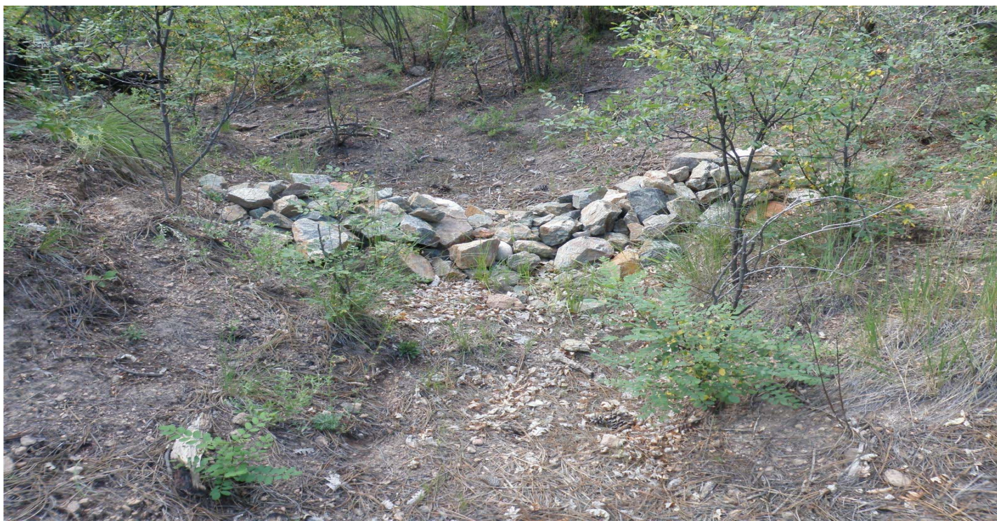
Photo 7802-4r.JPG (taken 08/17/10) W00806010004 : Check Dam - Rock Check Dam.
