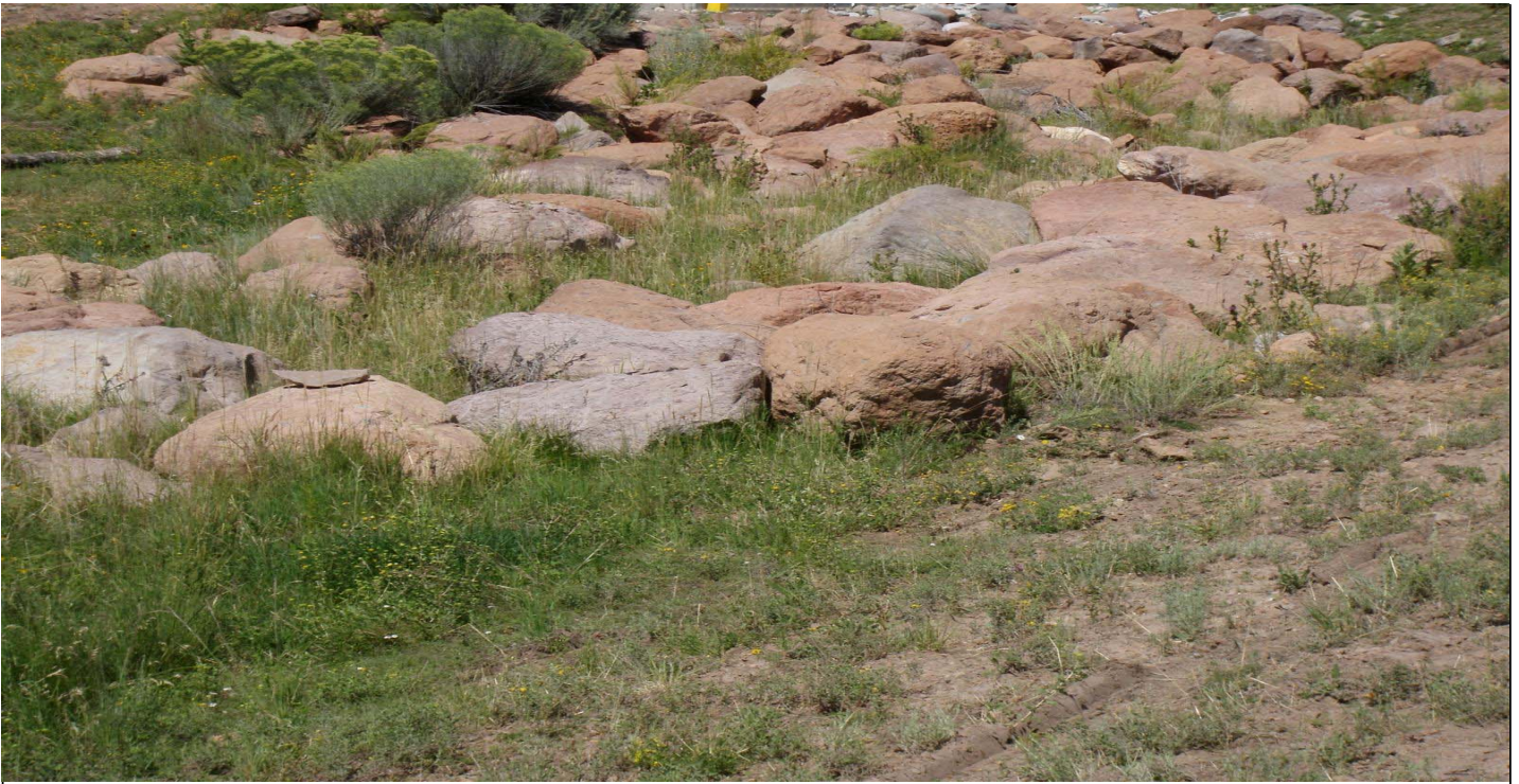
Photo 8524-01r.JPG (taken 08/18/10) V00904060006 : Channel/Swale - Rip Rap.
