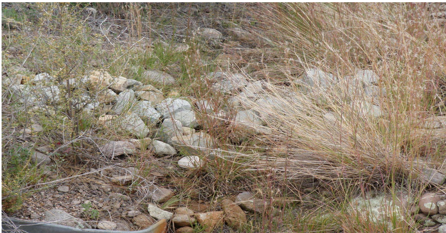
Photo 10885-3r.JPG (taken 10/01/10) V00506010008 : Check Dam - Rock Check Dam.
