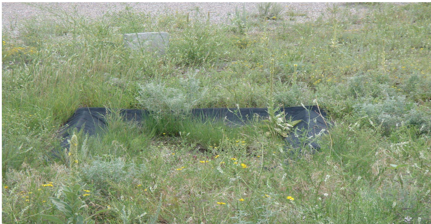
Photo 8517-2r.JPG (taken 08/13/10) H00203050002 : Berms - Silt Dike.
