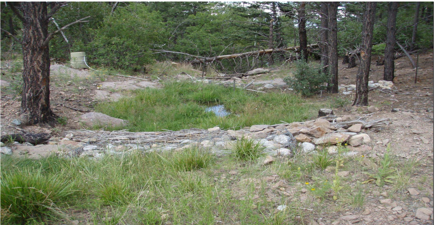
Photo 8531-06r.JPG (taken 08/23/10) W00606030005 : Check Dam - Juniper Bales; W00607010004 : Gabions - Gabions; W00607010010 : Gabions - Gabions.
