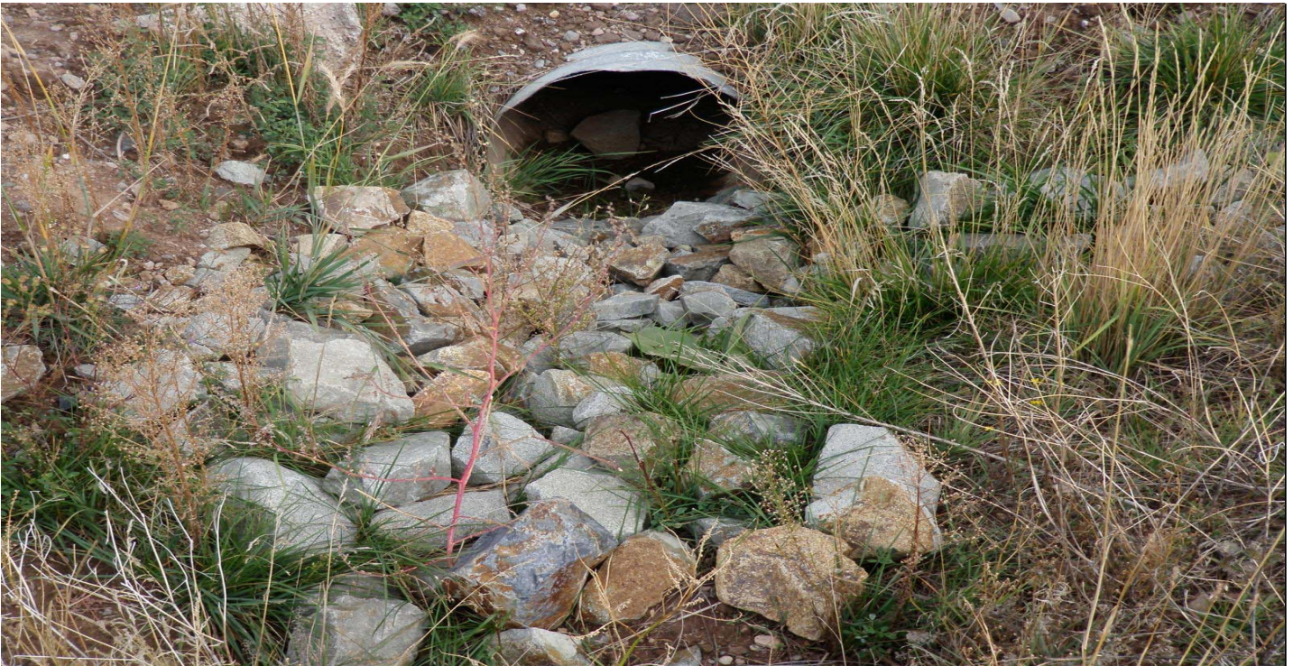
Photo 11025-2r.JPG (taken 10/21/10) C00404060008 : Channel/Swale - Rip Rap.
