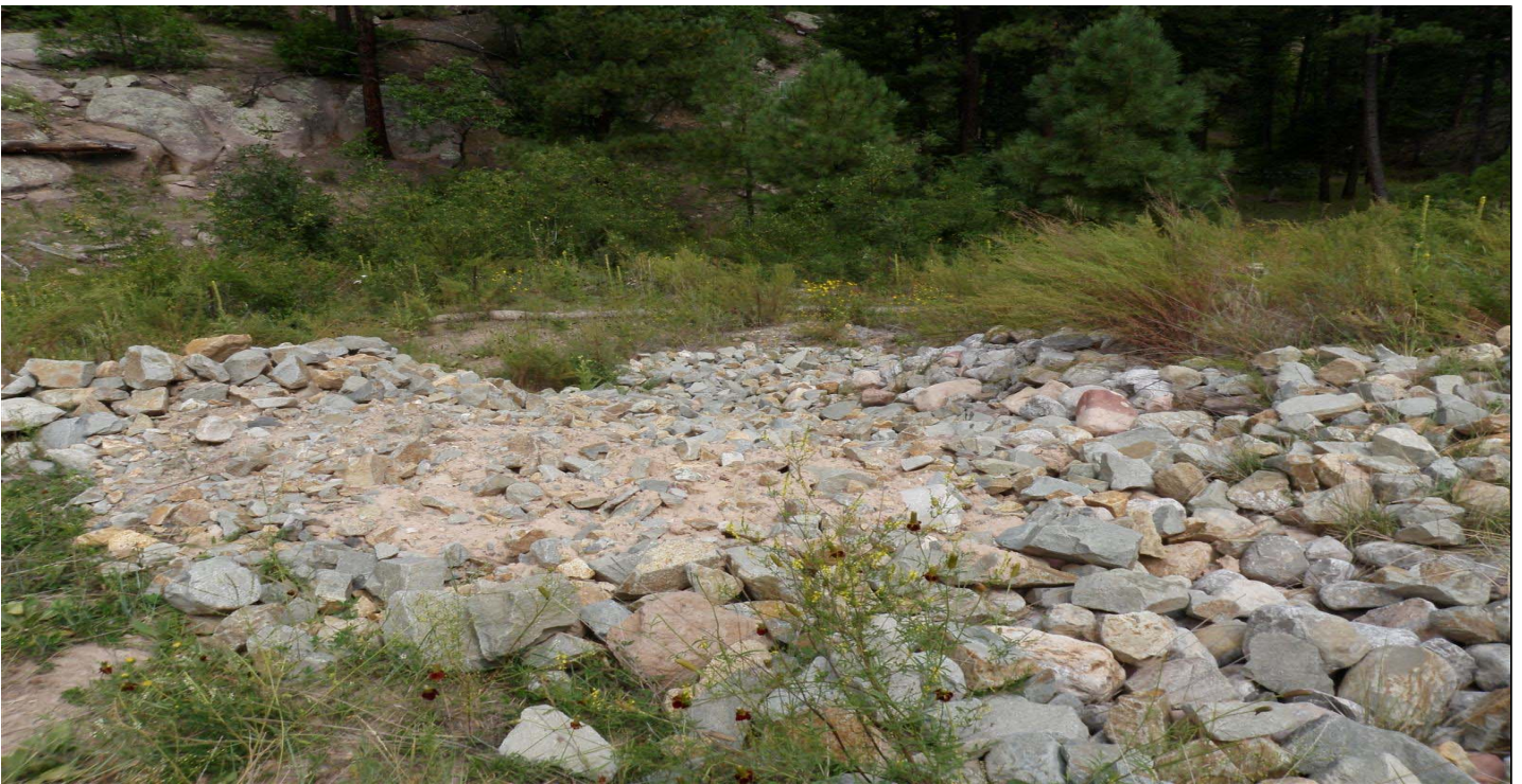
Photo 8793-4r.JPG (taken 09/07/10) V00802010005 : Established Vegetation - Permanent Vegetation Grasses and Shrubs; V00803060002 : Berms - Straw Wattles; V00804060010 : Channel/Swale - Rip Rap.
