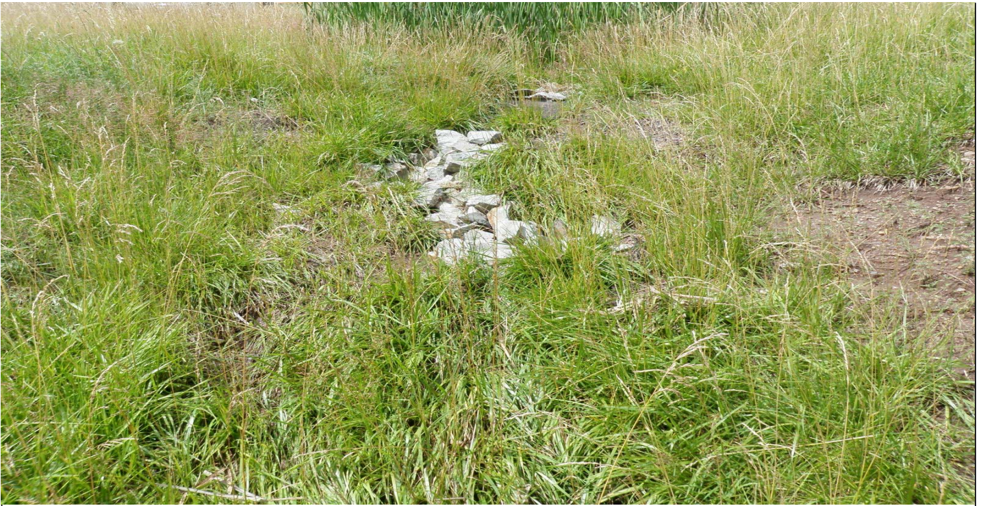
Photo 7800-6r.JPG (taken 08/17/10) W00204060007 : Channel/Swale - Rip Rap; W00204070002 : Channel/Swale - Vegetated Swale.
