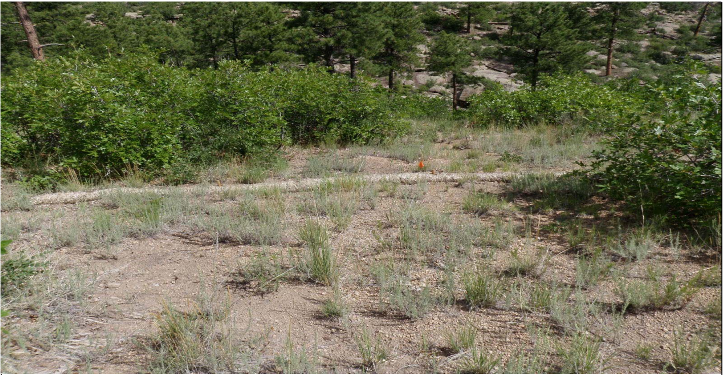
Photo 8516-5.JPG (taken 08/04/10) W02003060004 : Berms - Straw Wattles.
