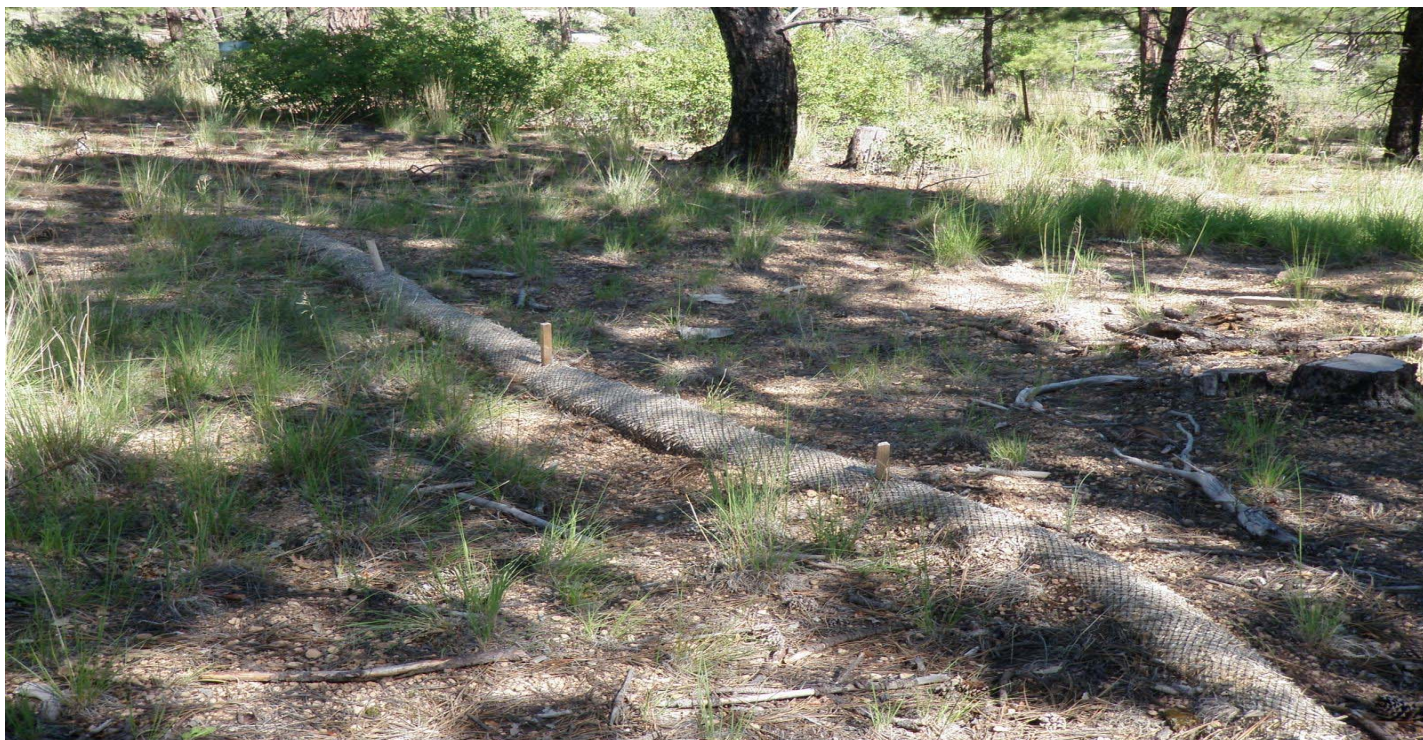
Photo 7805-6r.JPG (taken 08/17/10) W01303060005 : Berms - Straw Wattles.
