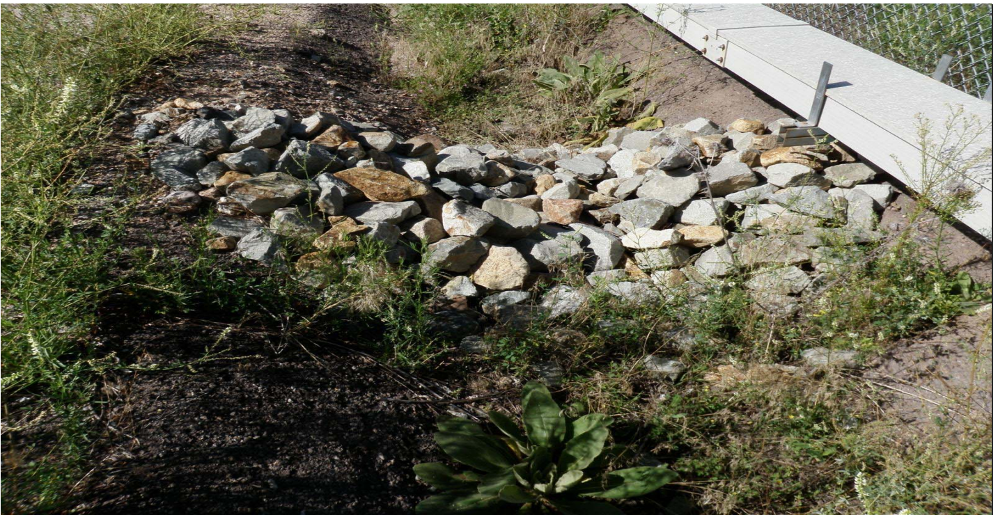
Photo 7523-6r.JPG (taken 08/12/10) J01606010005 : Check Dam - Rock Check Dam.
