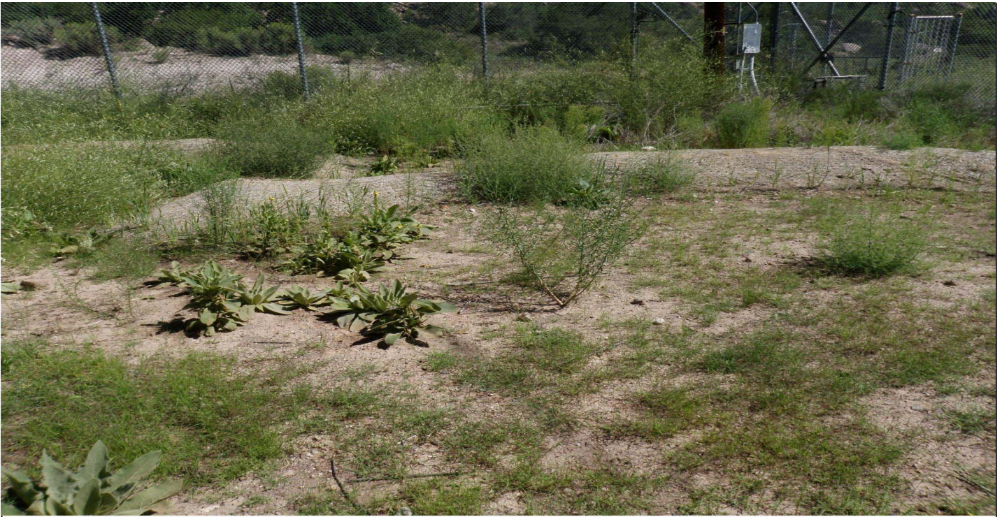
Photo 7593-4r.JPG (taken 08/13/10) H00603010008 : Berms - Earthen Berm.
