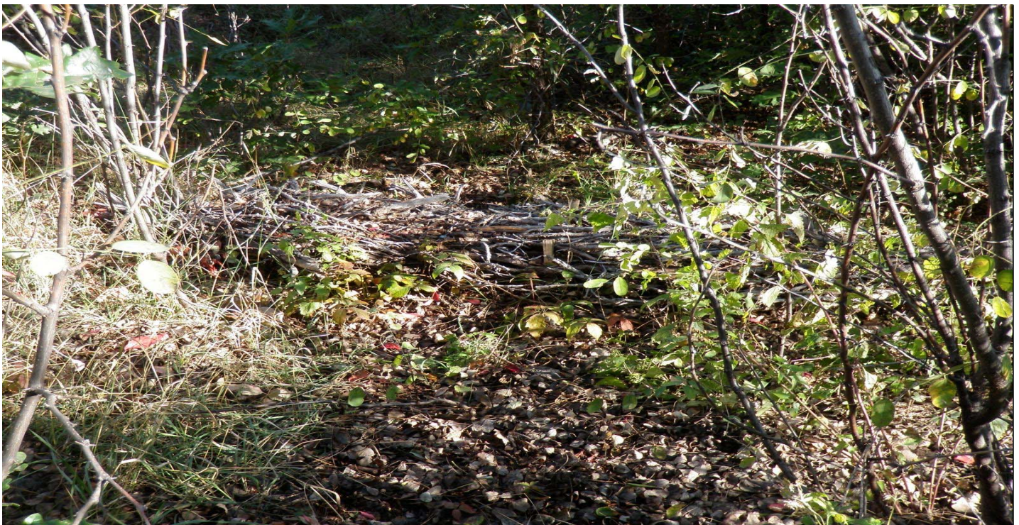
Photo 10875-1r.JPG (taken 10/07/10) W01506030005 : Check Dam - Juniper Bales.
