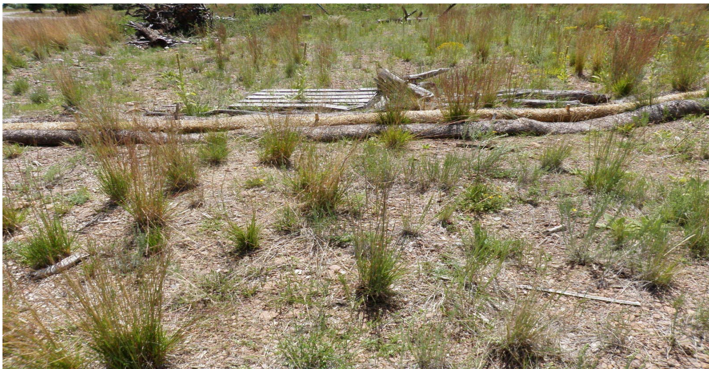
Photo 8527-7r.JPG (taken 08/18/10) V00703060009 : Berms - Straw Wattles.
