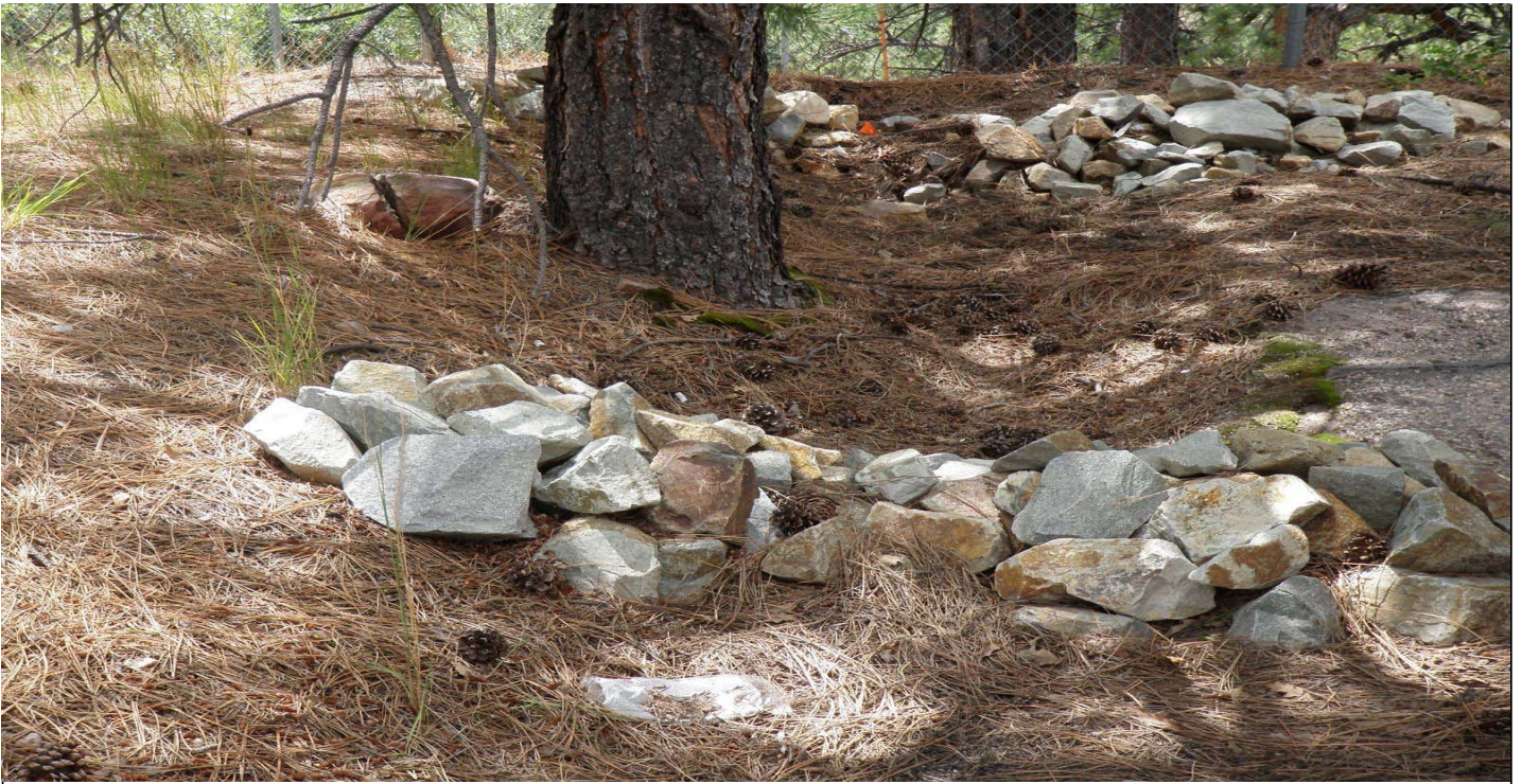
Photo 7520-2r.JPG (taken 08/12/10) E01002020002 : Established Vegetation - Permanent Vegetation Forested/Needle Cast; E01006010004 : Check Dam - Rock Check Dam; E01006010005 : Check Dam - Rock Check Dam.
