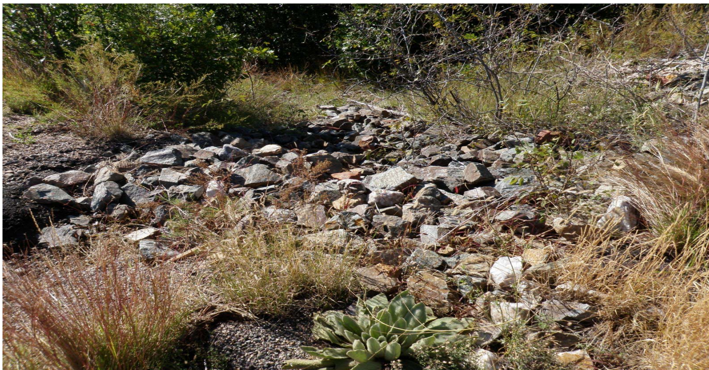
Photo 10878-9r.JPG (taken 10/07/10) W01804060004 : Channel/Swale - Rip Rap.
