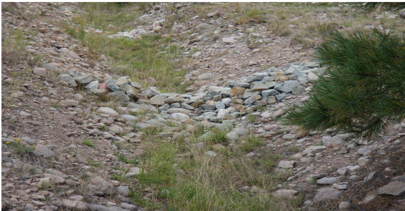
Photo 10885-4r.JPG (taken 10/01/10) V00506010006 : Check Dam - Rock Check Dam.
