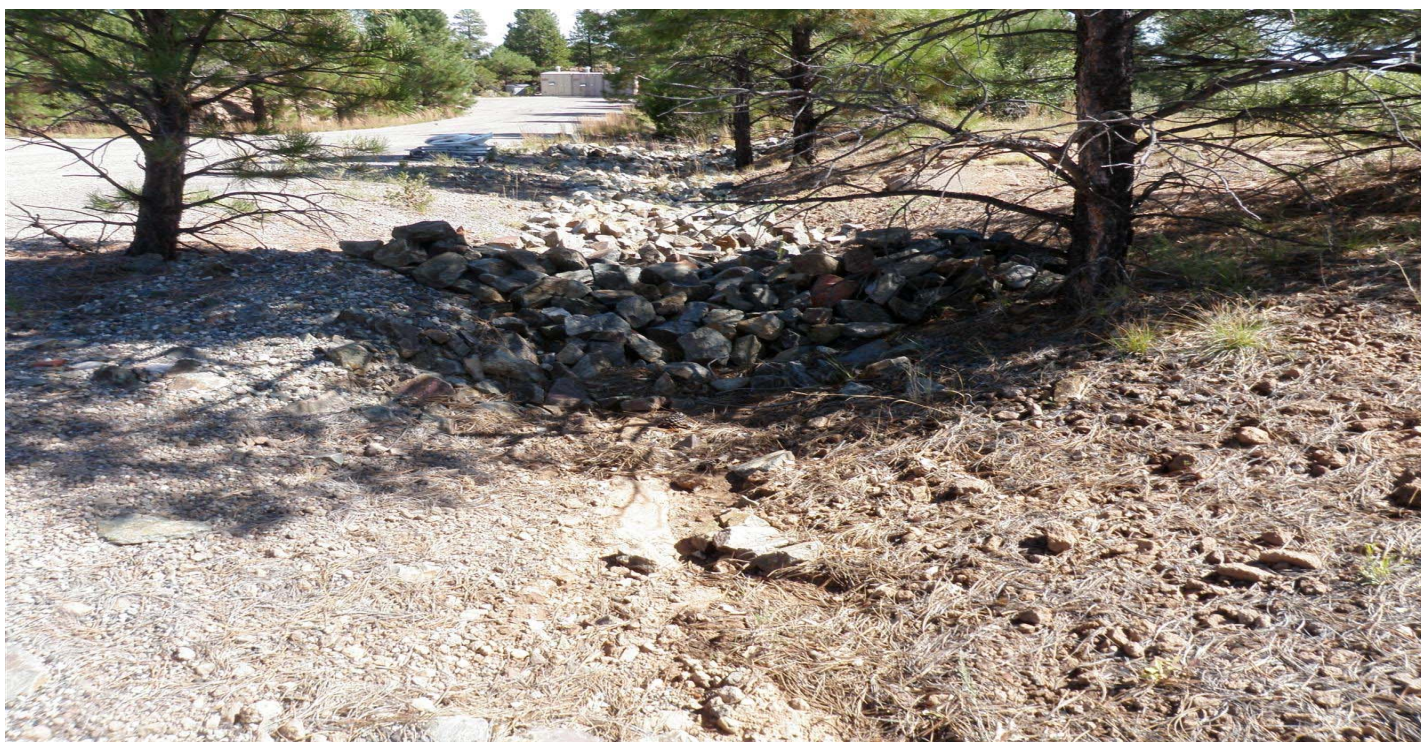
Photo 10873-08r.JPG (taken 10/07/10) H00304060001 : Channel/Swale - Rip Rap; H00306010006 : Check Dam - Rock Check Dam.
