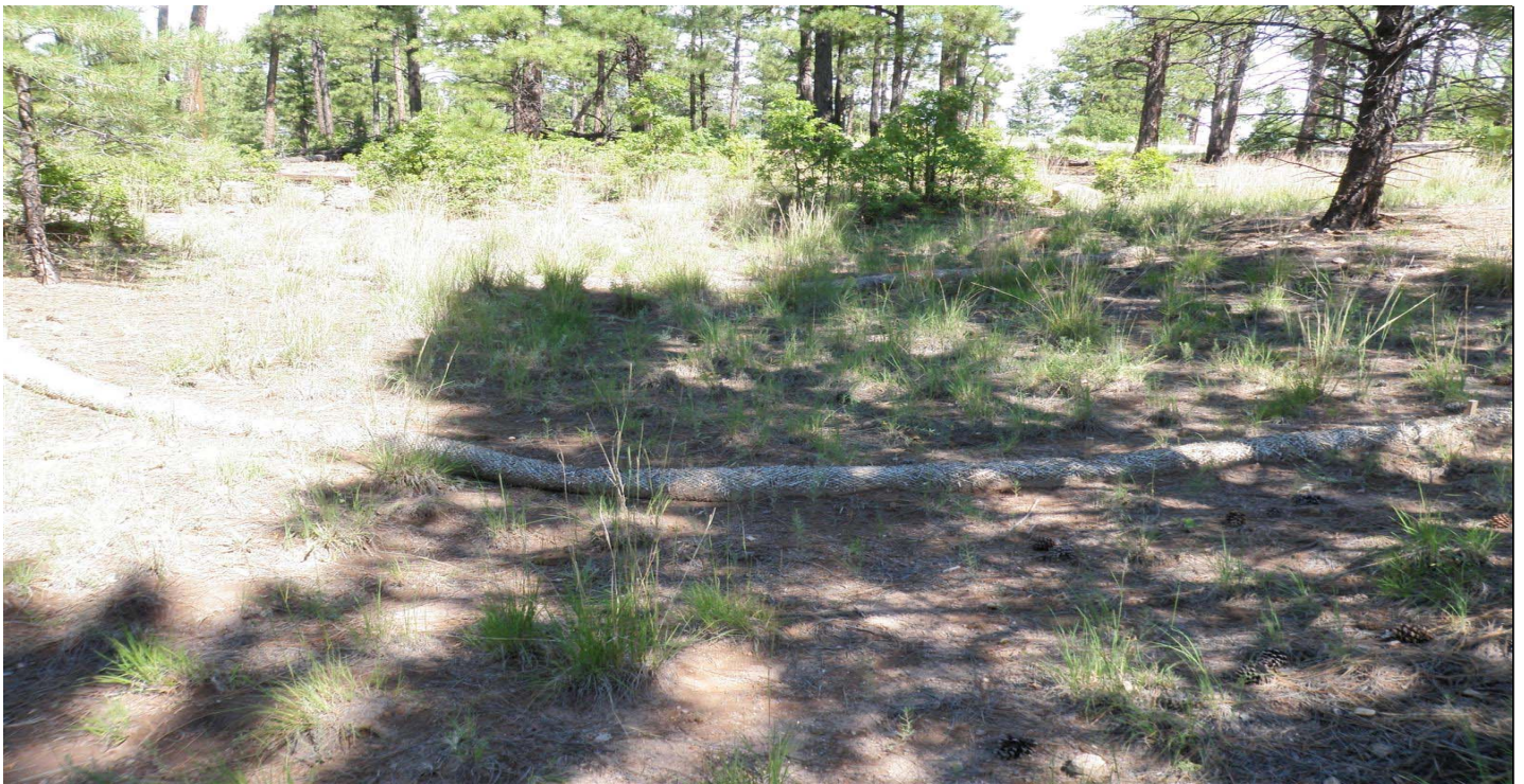
Photo 8525-02r.JPG (taken 08/18/10) V009A03060022 : Berms - Straw Wattles; V009A03060023 : Berms - Straw Wattles.
