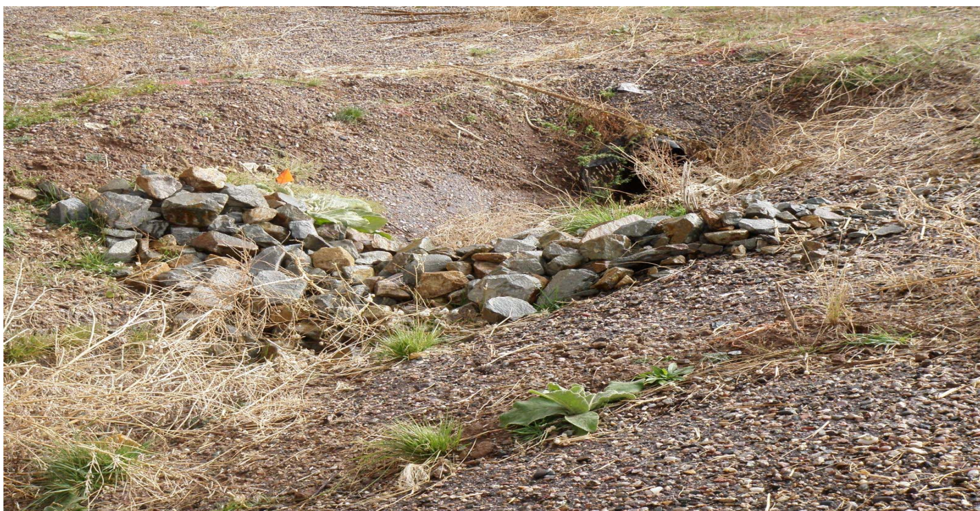
Photo 11025-8r.JPG (taken 10/21/10) C00406010010 : Check Dam - Rock Check Dam.
