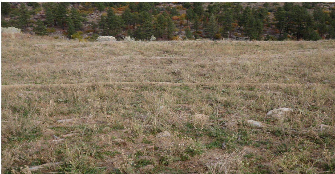
Photo 11465-3r.JPG (taken 10/22/10) V008A03060010 : Berms - Straw Wattles.
