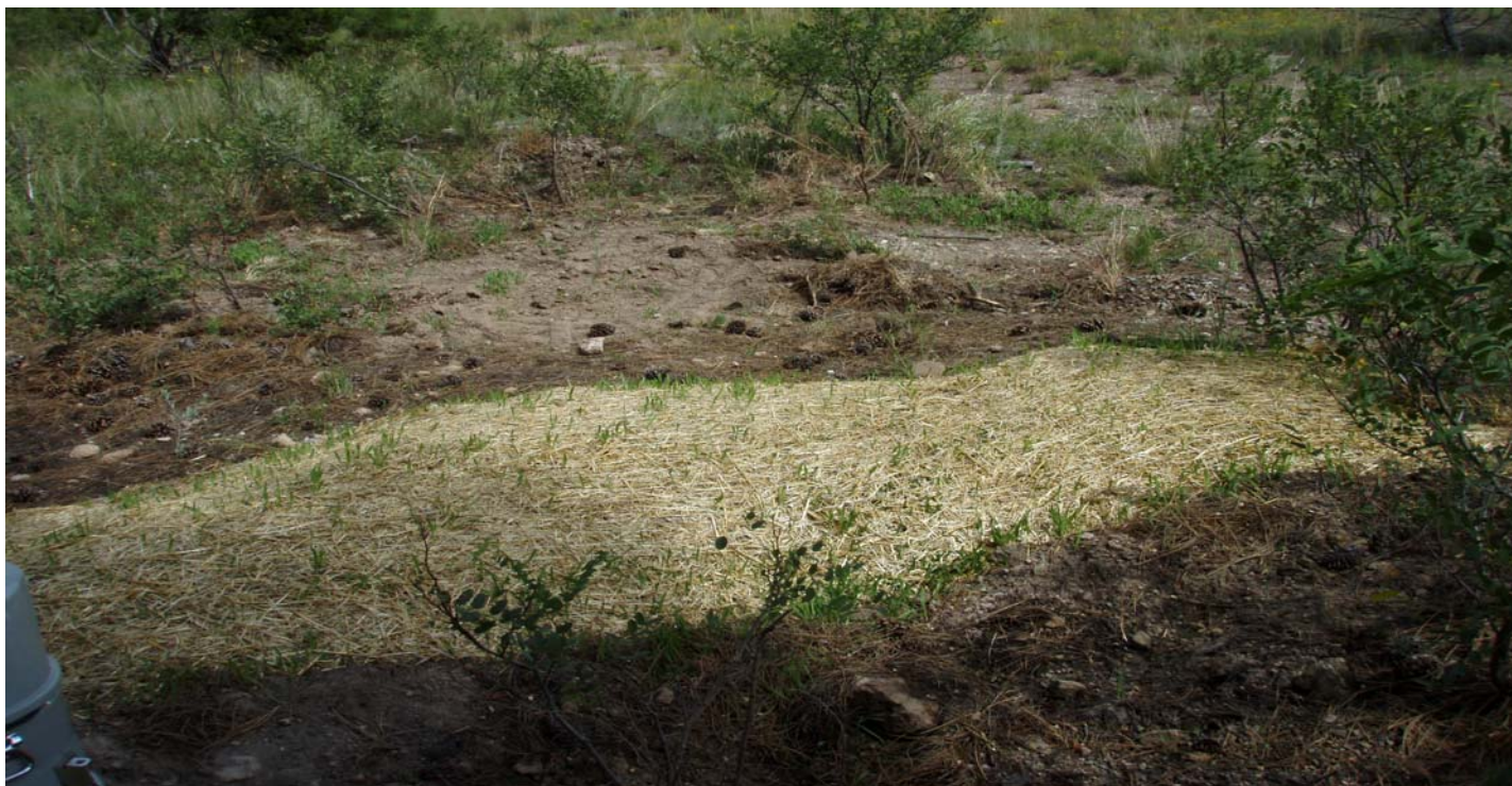
Photo 8534-2.JPG (taken 08/23/10) E01503010004 : Berms - Earthen Berm.
