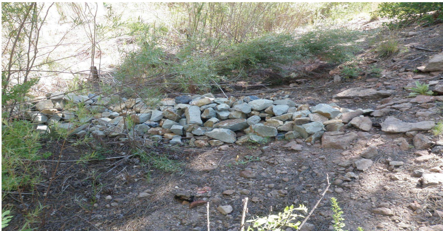
Photo 8529-2r.JPG (taken 08/18/10) V01406010004 : Check Dam - Rock Check Dam.
