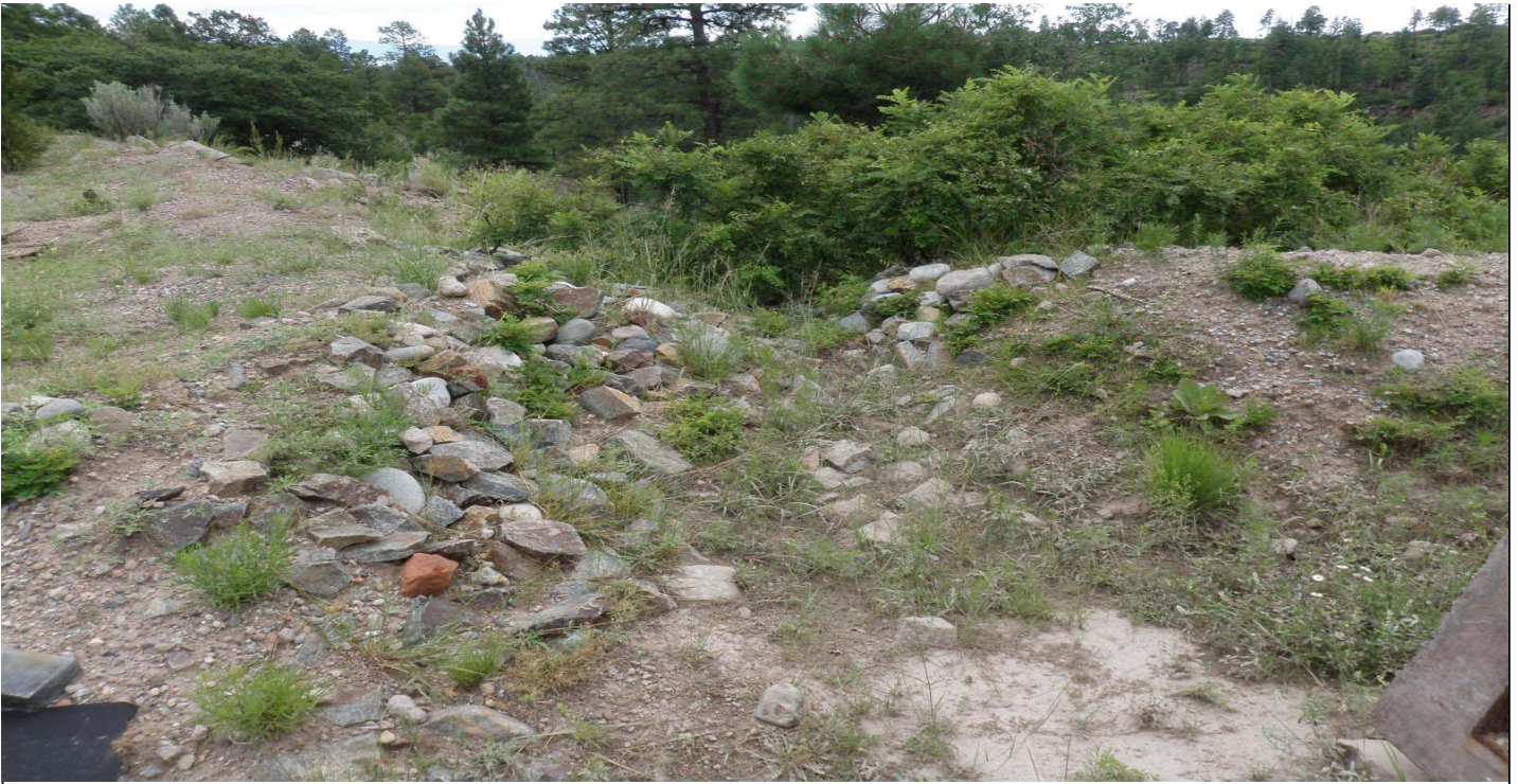
Photo 7512-2r.JPG (taken 08/12/10) J01206010006 : Check Dam - Rock Check Dam.
