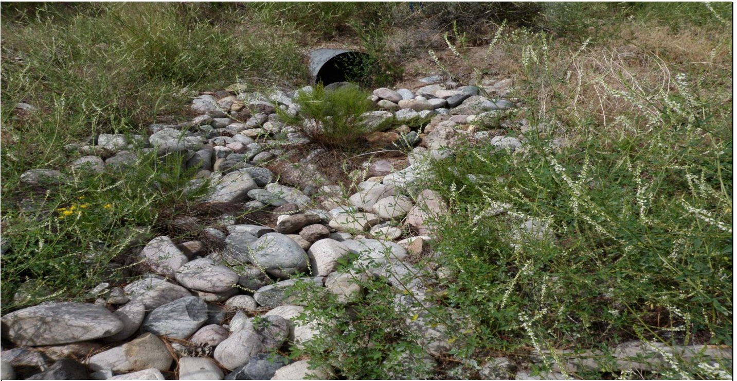
Photo 8516-1.JPG (taken 08/04/10) W02004060002 : Channel/Swale - Rip Rap.
