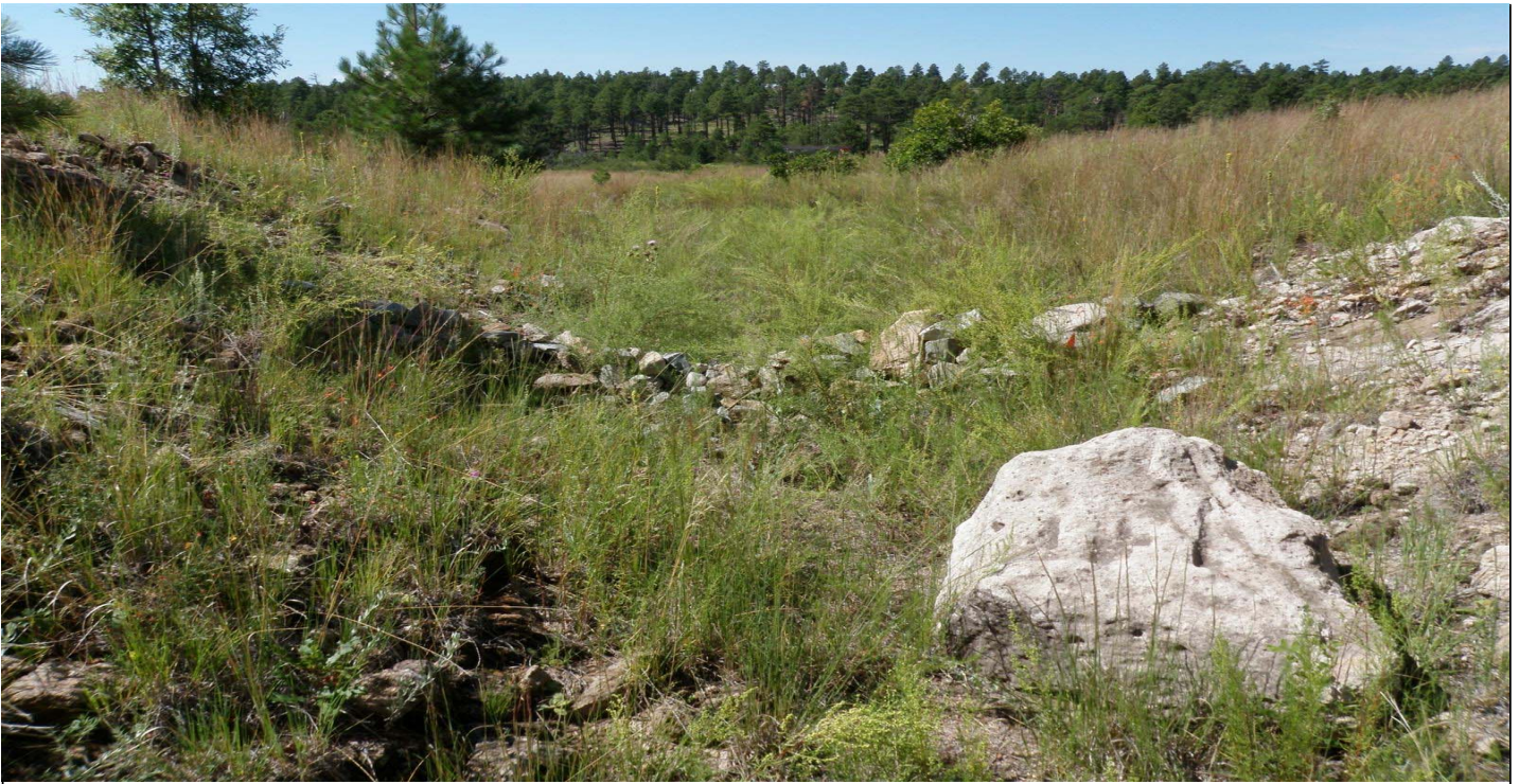
Photo 8525-05r.JPG (taken 08/18/10) V009A02010001 : Established Vegetation - Permanent Vegetation Grasses and Shrubs; V009A06010015 : Check Dam - Rock Check Dam.
