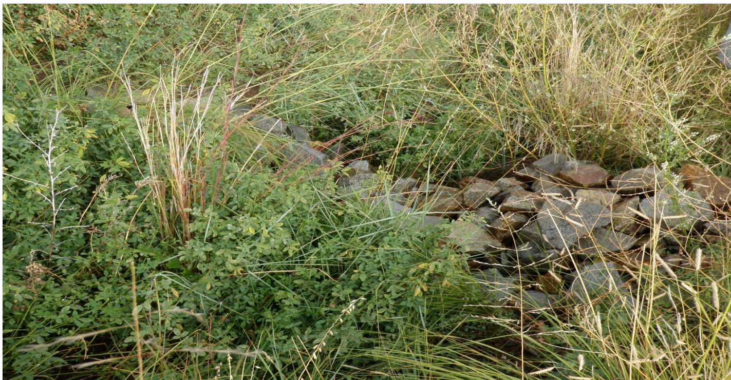
Photo 11025-6r.JPG (taken 10/21/10) C00406010011 : Check Dam - Rock Check Dam.
