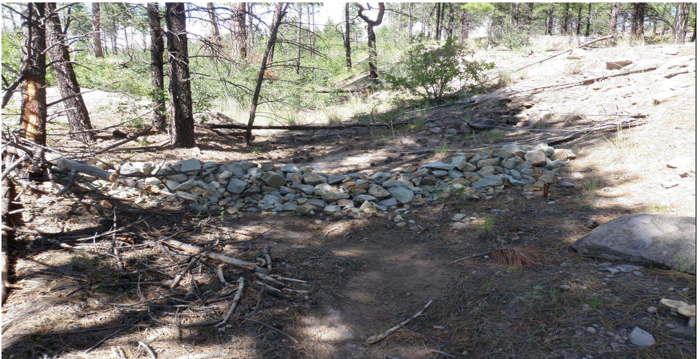
Photo 8529-1r.JPG (taken 08/18/10) V01402020001 : Established Vegetation - Permanent Vegetation Forested/Needle Cast; V01406010003 : Check Dam - Rock Check Dam.
