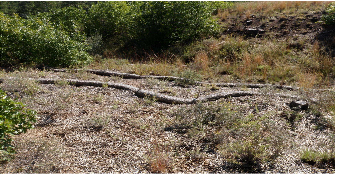
Photo 10877-3r.JPG (taken 10/07/10) W01703060007 : Berms - Straw Wattles; W01703060008 : Berms - Straw Wattles.
