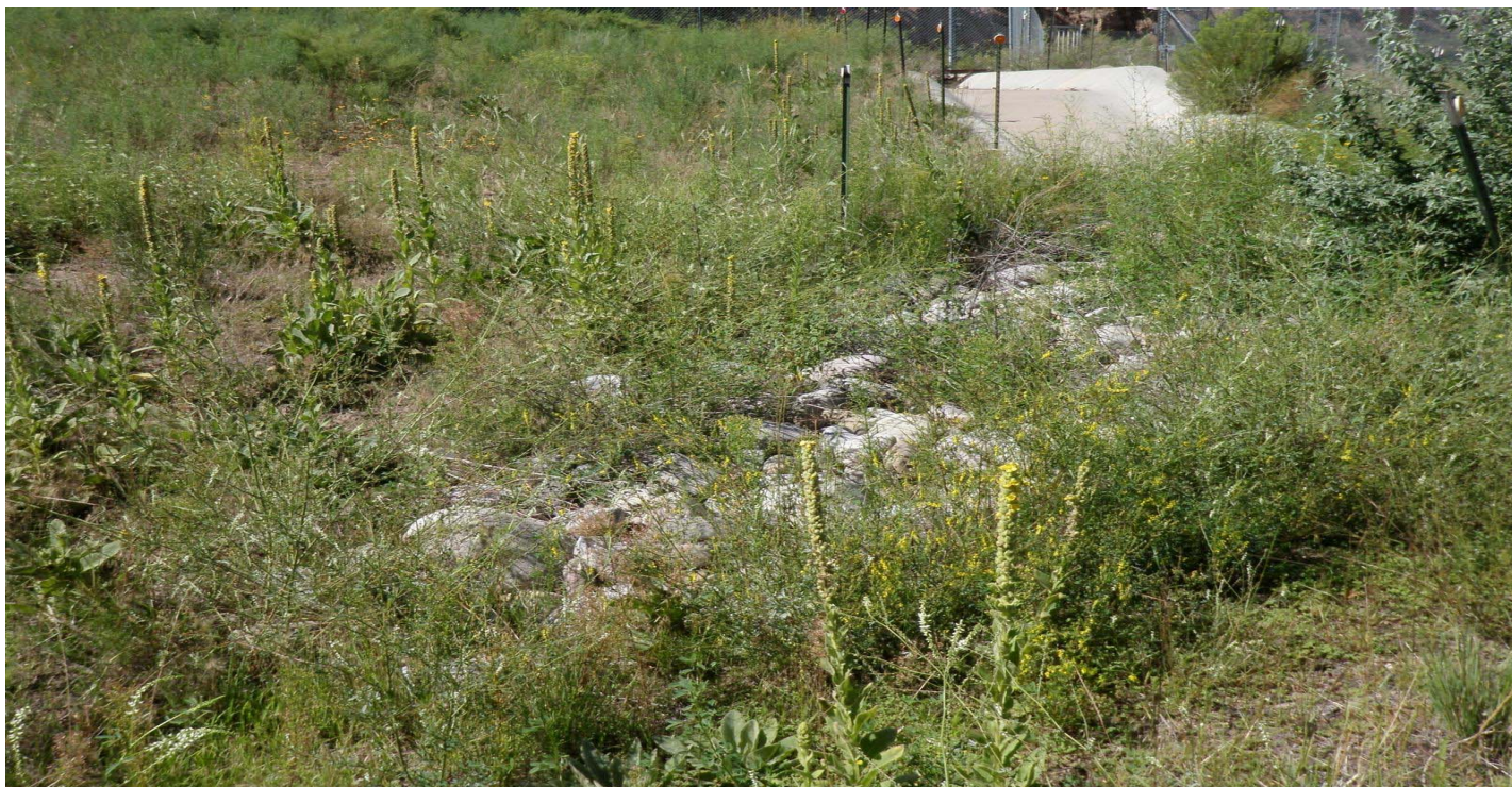
Photo 7593-1r.JPG (taken 08/13/10) H00604020009 : Channel/Swale - Concrete/Asphalt Channel/Swale; H00604060005 : Channel/Swale - Rip Rap.
