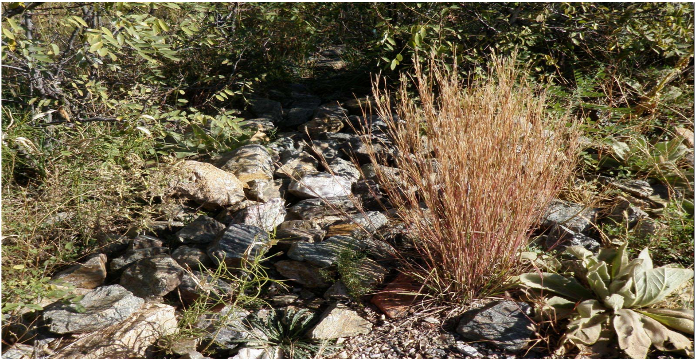
Photo 10876-1r.JPG (taken 10/07/10) W01604060003 : Channel/Swale - Rip Rap.
