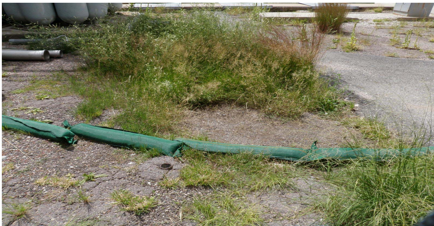
Photo 7521-1r.JPG (taken 08/12/10) E01103100002 : Berms - Gravel Bags.
