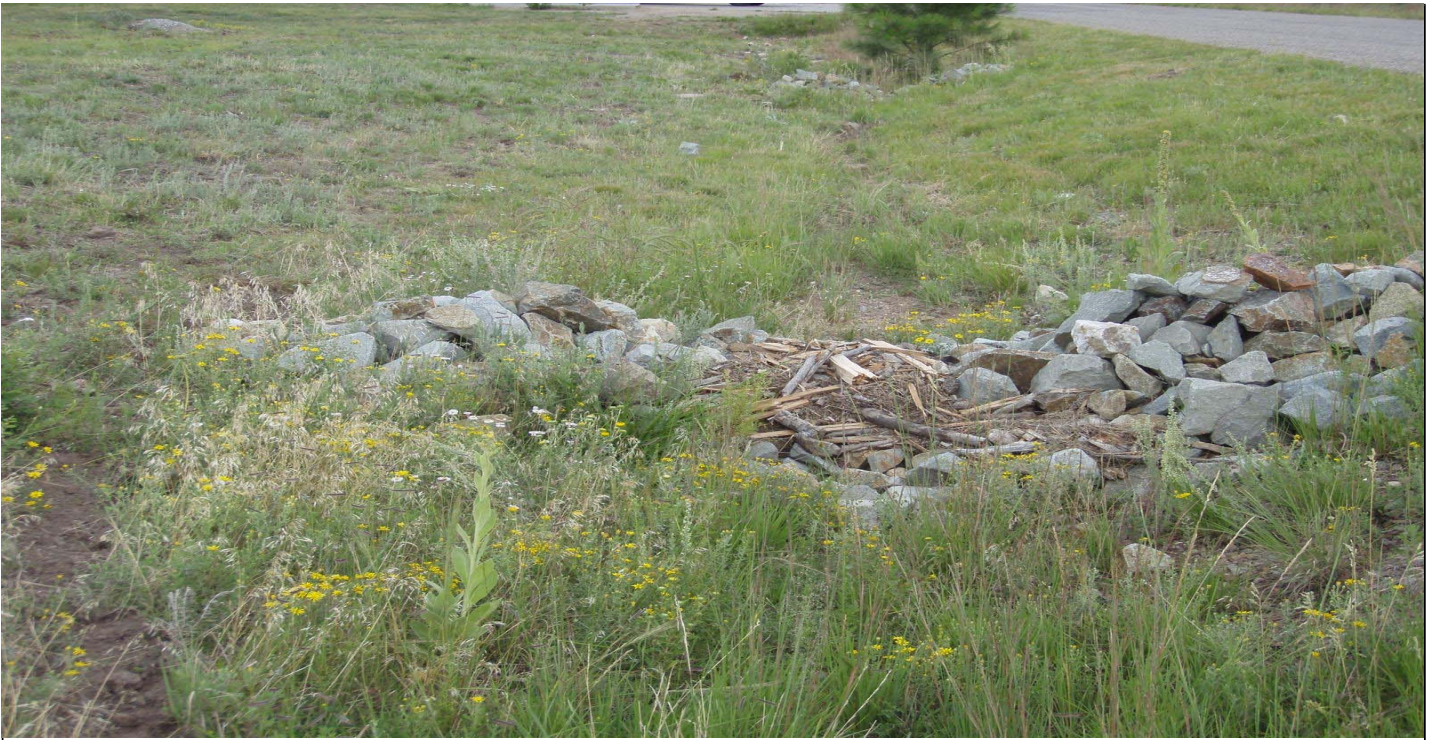
Photo 8531-01r.JPG (taken 08/23/10) W00602010009 : Established Vegetation - Permanent Vegetation Grasses and Shrubs; W00606010016 : Check Dam - Rock Check Dam; W00606010017 : Check Dam - Rock Check Dam.
