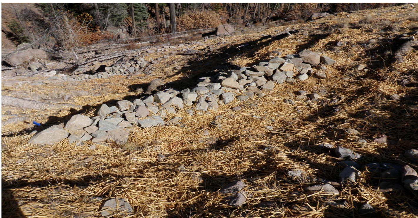
Photo 11699-1r.JPG (taken 11/15/10) V00506010012 : Check Dam - Rock Check Dam.
