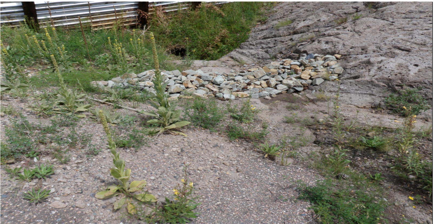
Photo 8503-4r.JPG (taken 08/19/10) C00306010006 : Check Dam - Rock Check Dam.
