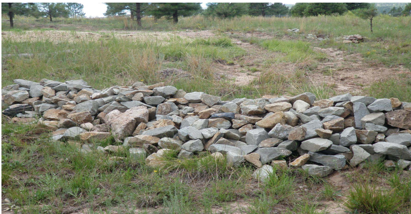
Photo 8518-2r.JPG (taken 08/13/10) E00203120003 : Berms - Rock Berm.
