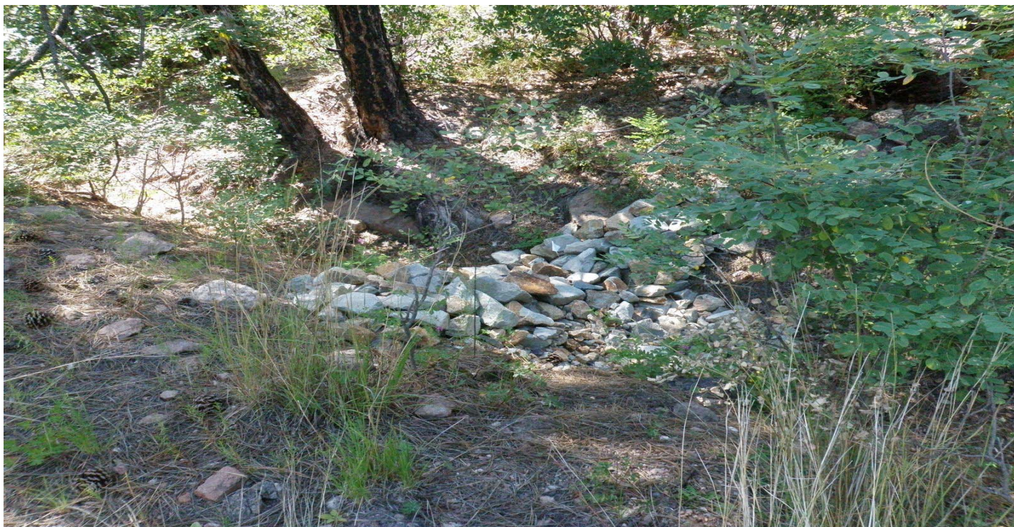
Photo 8529-4r.JPG (taken 08/18/10) V01406010005 : Check Dam - Rock Check Dam.
