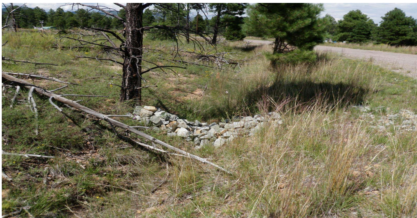
Photo 8530-3r.JPG (taken 08/18/10) W01206010007 : Check Dam - Rock Check Dam.
