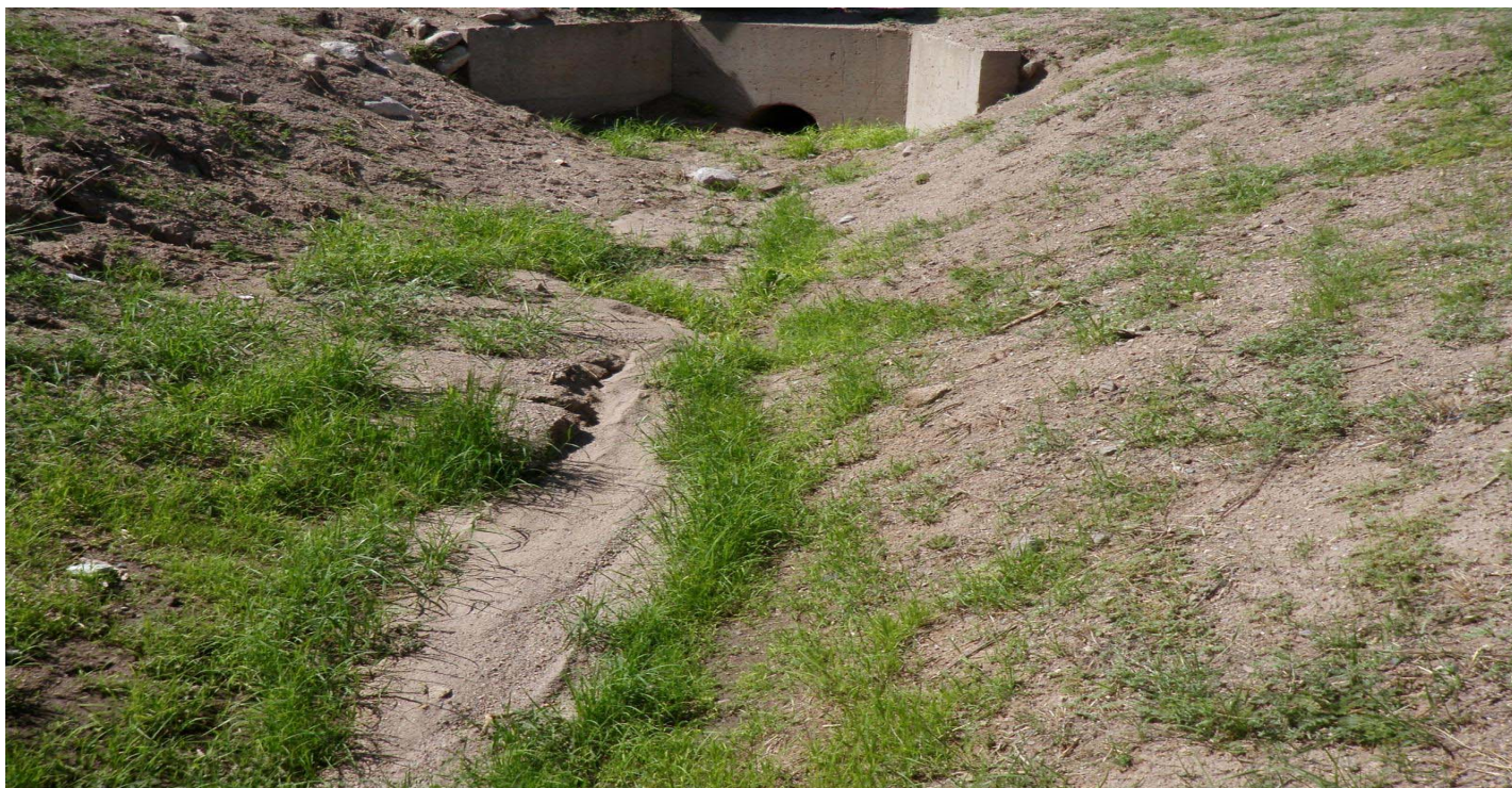
Photo 8526-1r.JPG (taken 08/18/10) F00104040003 : Channel/Swale - Culvert.
