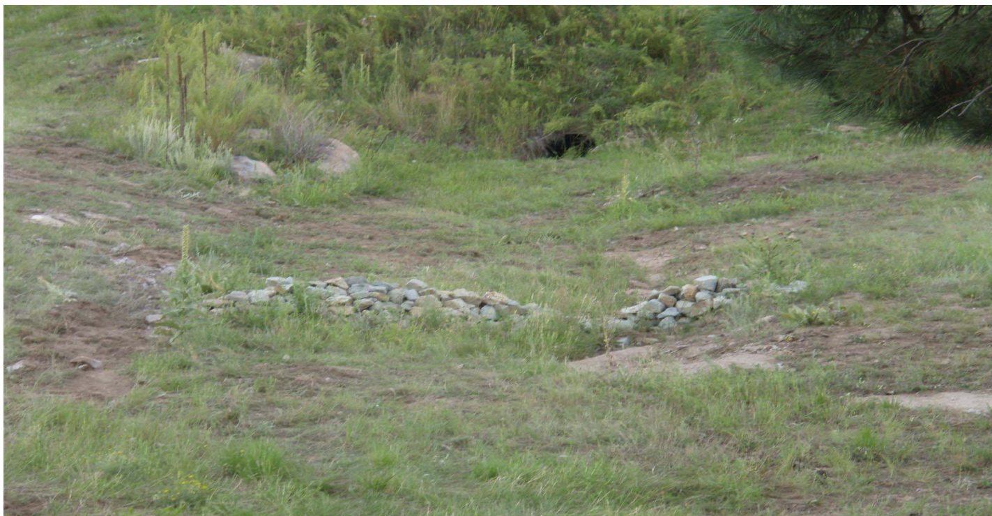
Photo 8531-03r.JPG (taken 08/23/10) W00606010013 : Check Dam - Rock Check Dam.
