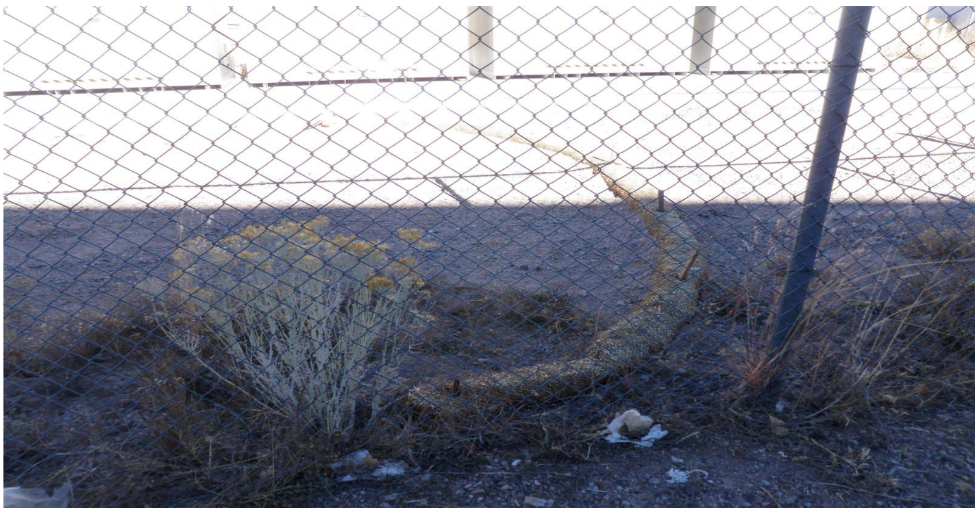
Photo 12126-4r.JPG (taken 12/02/10) E01203060009 : Berms - Straw Wattles.
