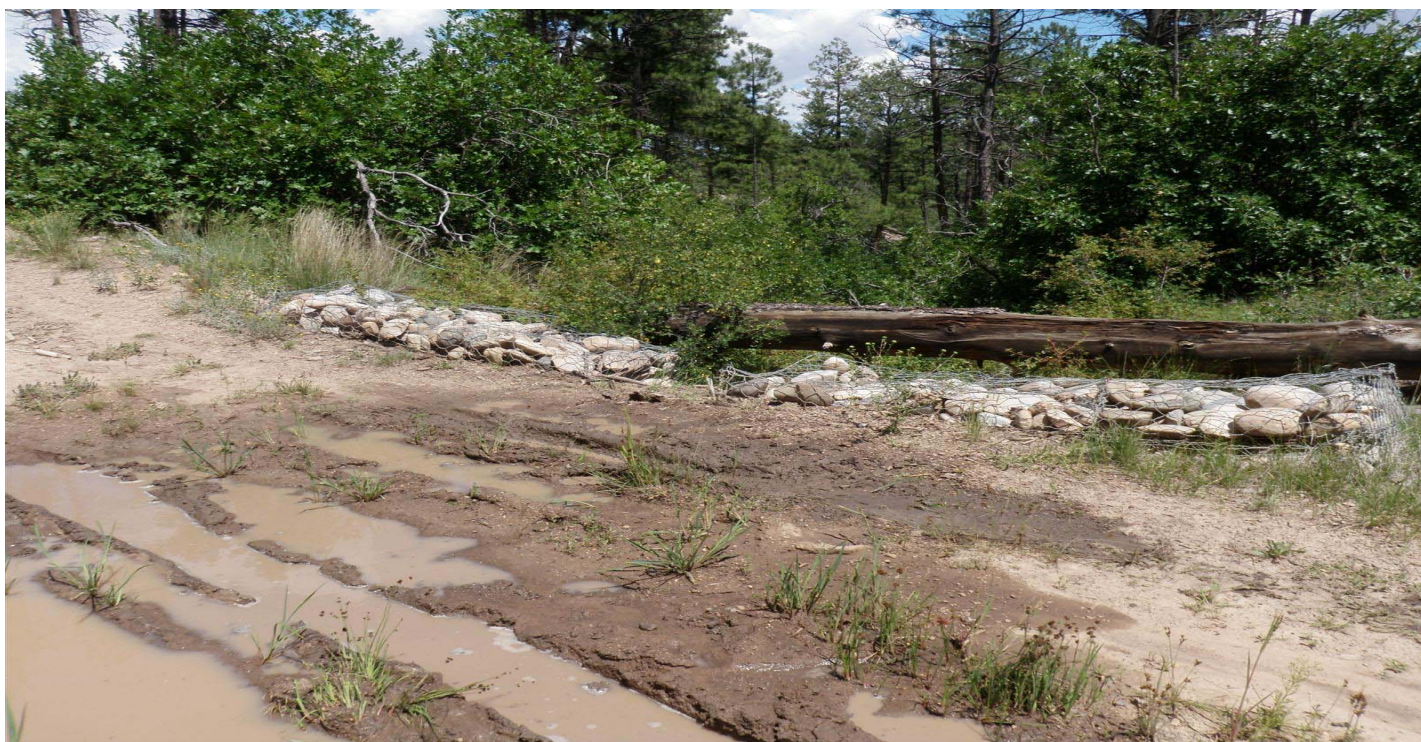
Photo 8527-4r.JPG (taken 08/18/10) V00707010002 : Gabions - Gabions.
