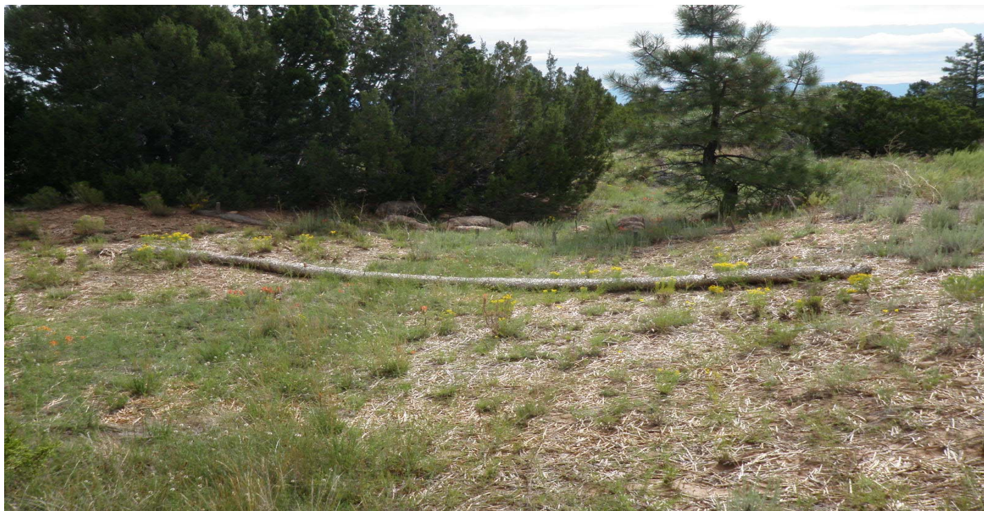
Photo 8519-10.JPG (taken 08/04/10) W01903060019 : Berms - Straw Wattles.
