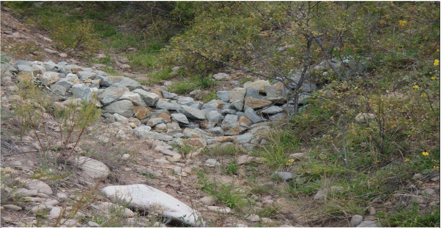
Photo 10885-5r.JPG (taken 10/01/10) V00506010007 : Check Dam - Rock Check Dam.
