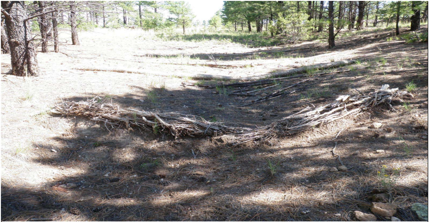
Photo 8525-01r.JPG (taken 08/18/10) V009A02020002 : Established Vegetation - Permanent Vegetation Forested/Needle Cast; V009A06030017 : Check Dam - Juniper Bales.
