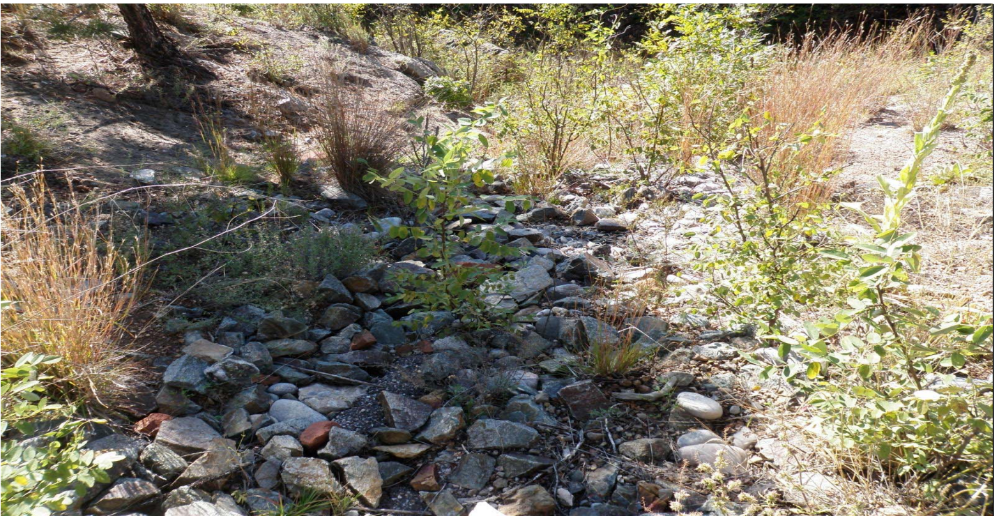
Photo 10878-6r.JPG (taken 10/07/10) W01804060013 : Channel/Swale - Rip Rap.
