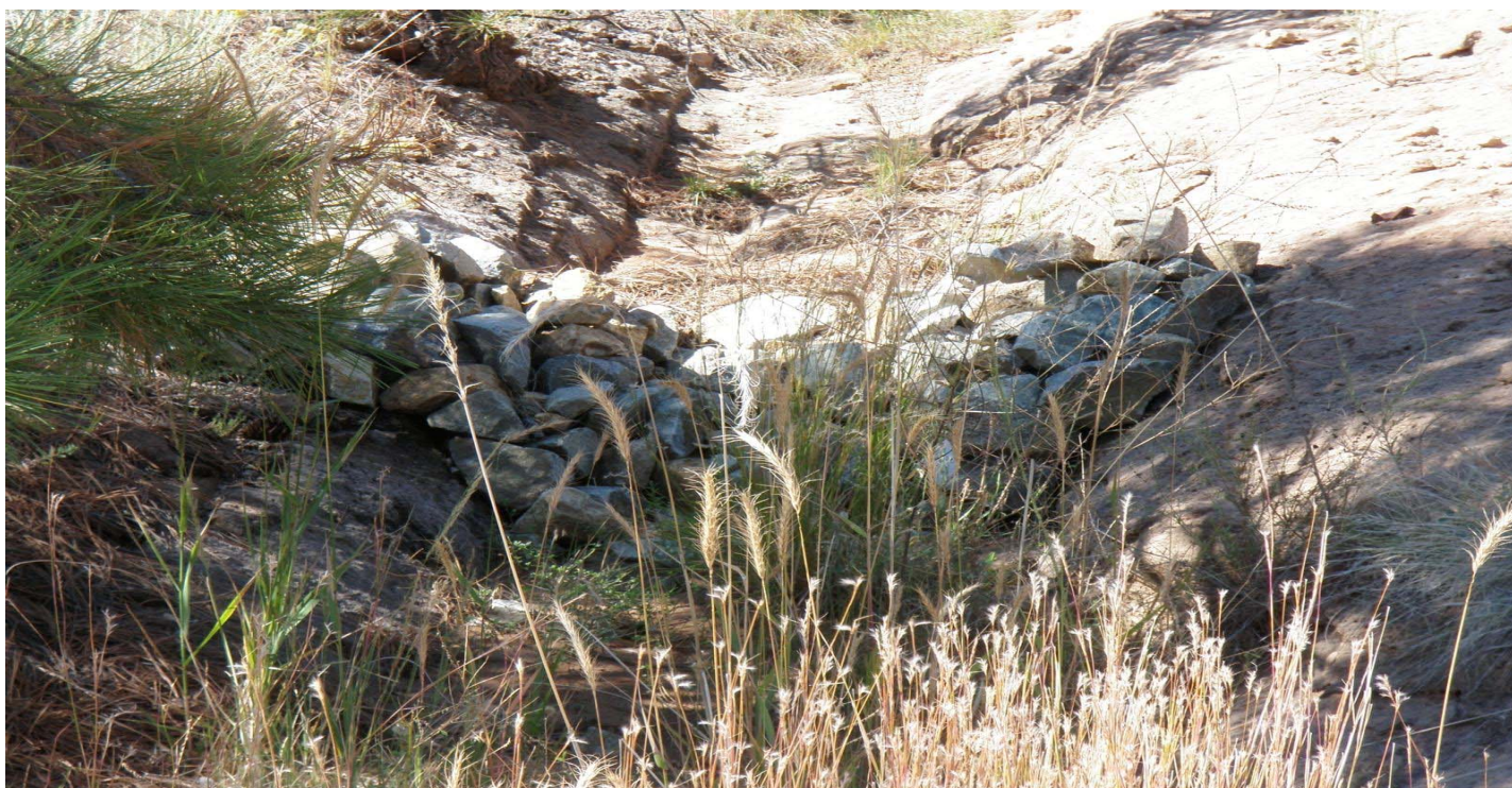
Photo 10873-04r.JPG (taken 10/07/10) H00306010010 : Check Dam - Rock Check Dam.
