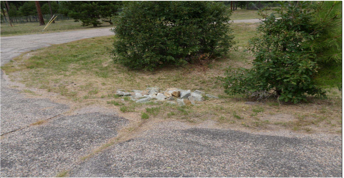
Photo 8794-1r.JPG (taken 09/07/10) W00402010002 : Established Vegetation - Permanent Vegetation Grasses and Shrubs; W00404060003 : Channel/Swale - Rip Rap.
