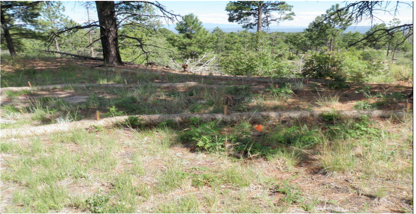
Photo 7802-1r.JPG (taken 08/17/10) W00802010002 : Established Vegetation - Permanent Vegetation Grasses and Shrubs; W00802020009 : Established Vegetation - Permanent Vegetation Forested/Needle Cast; W00803060010 : Berms - Straw Wattles; W00803060011 : Berms - Straw Wattles; W00803060012 : Berms - Straw Wattles.
