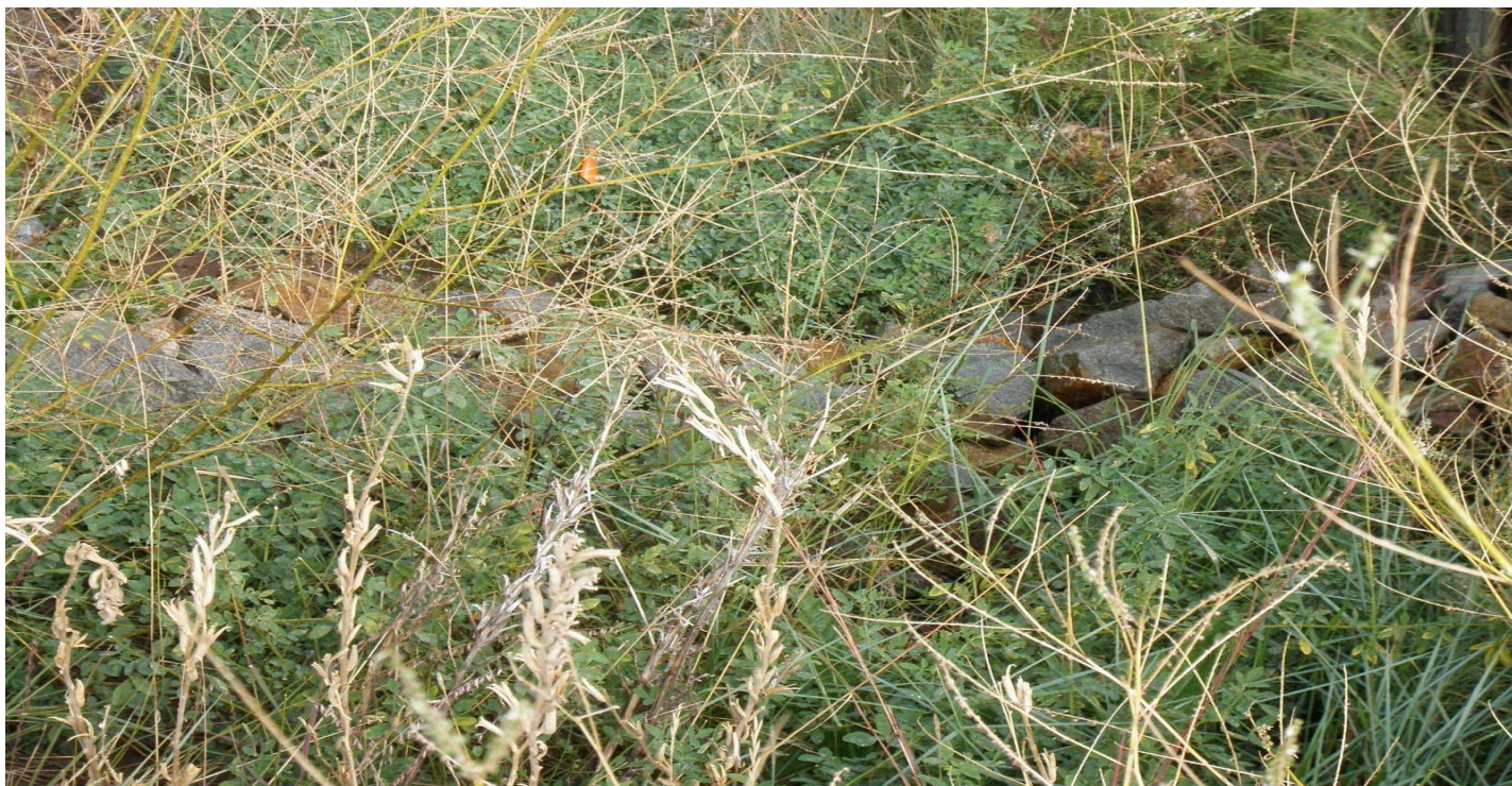
Photo 11025-7r.JPG (taken 10/21/10) C00406010012 : Check Dam - Rock Check Dam.
