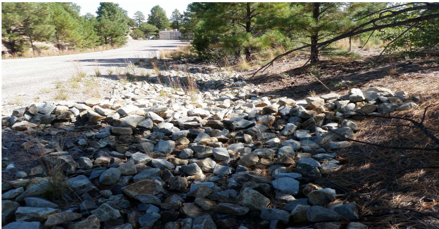
Photo 10873-09r.JPG (taken 10/07/10) H00306010005 : Check Dam - Rock Check Dam.
