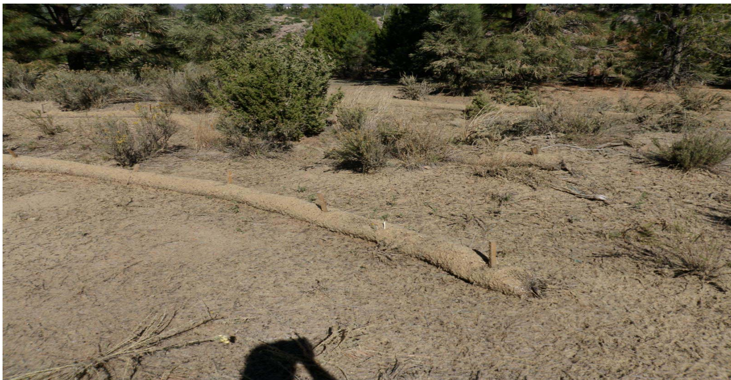
Photo 10872-05r.JPG (taken 10/07/10) H00403060014 : Berms - Straw Wattles; H00403060015 : Berms - Straw Wattles; H00403060027 : Berms - Straw Wattles.
