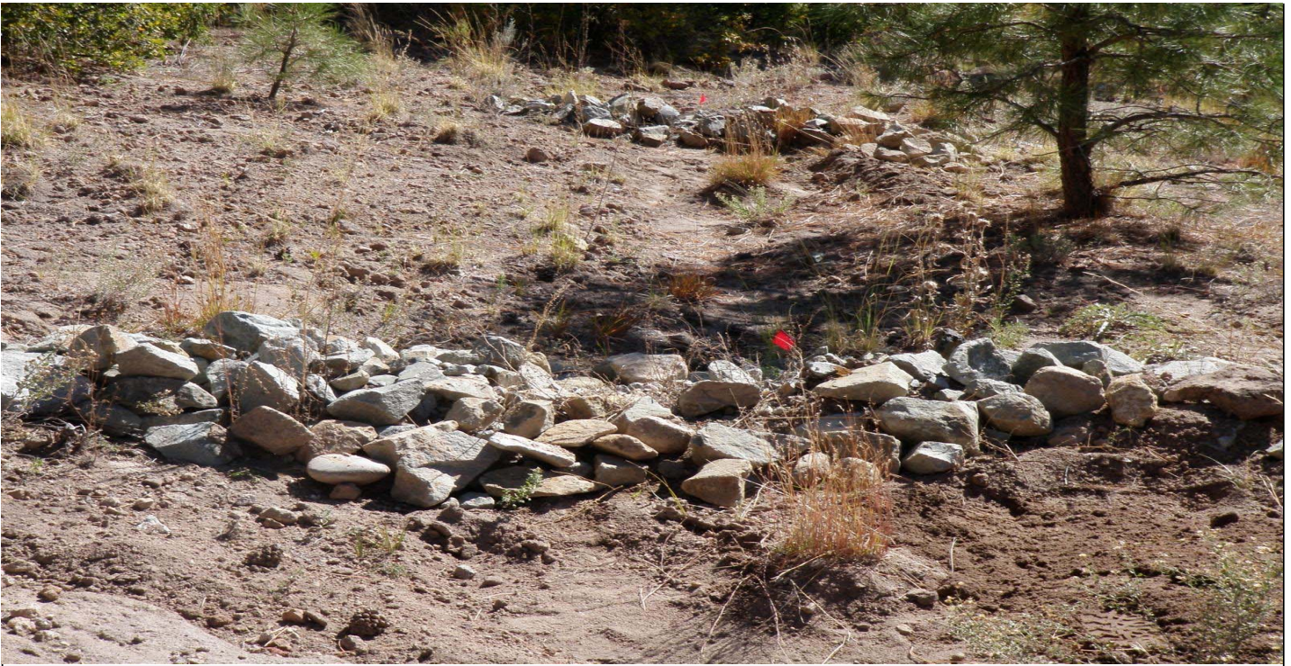
Photo 11459-3r.JPG (taken 10/26/10) J01406010004 : Check Dam - Rock Check Dam; J01406010005 : Check Dam - Rock Check Dam.
