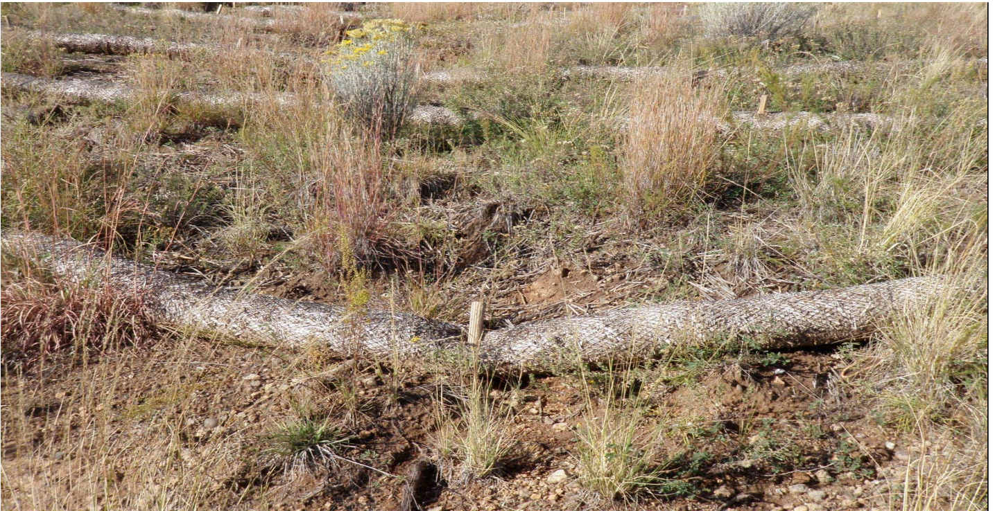
Photo 10877-2r.JPG (taken 10/07/10) W01703060013 : Berms - Straw Wattles; W01703060014 : Berms - Straw Wattles; W01703060016 : Berms - Straw Wattles.
