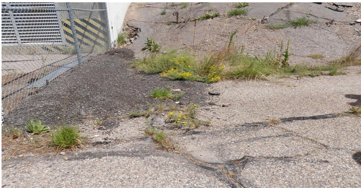
Photo 7520-1r.JPG (taken 08/12/10) E01003040003 : Berms - Asphalt Berm.
