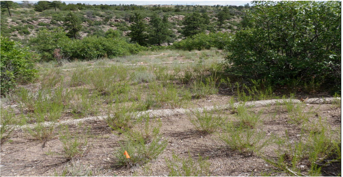
Photo 8516-3.JPG (taken 08/04/10) W02003060008 : Berms - Straw Wattles; W02003060009 : Berms - Straw Wattles; W02003060010 : Berms - Straw Wattles.
