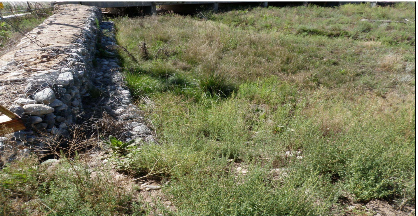
Photo 7523-4r.JPG (taken 08/12/10) J01602030003 : Established Vegetation - Permanent Vegetation Vegetative Buffer Strip; J01607010002 : Gabions - Gabions.
