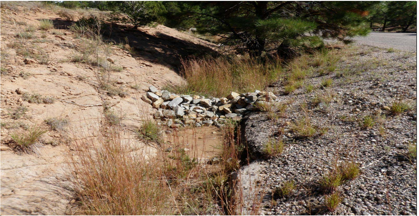
Photo 10873-05r.JPG (taken 10/07/10) H00306010009 : Check Dam - Rock Check Dam.
