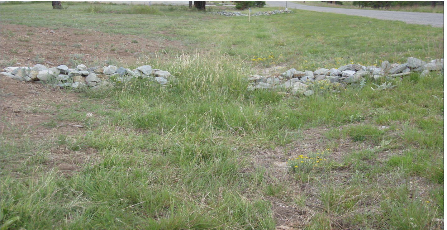
Photo 8531-02r.JPG (taken 08/23/10) W00606010014 : Check Dam - Rock Check Dam; W00606010015 : Check Dam - Rock Check Dam.
