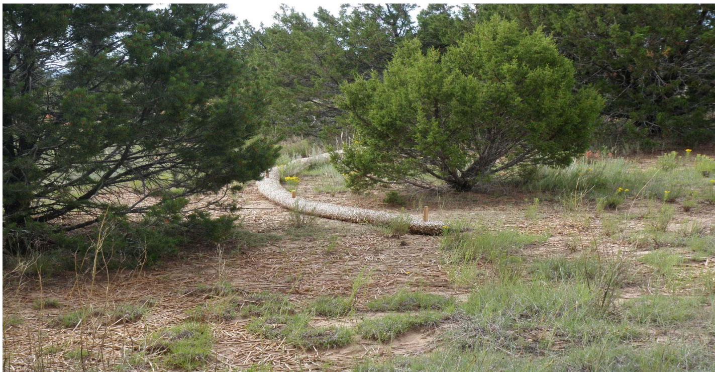
Photo 8519-4.JPG (taken 08/04/10) W01903060033 : Berms - Straw Wattles.
