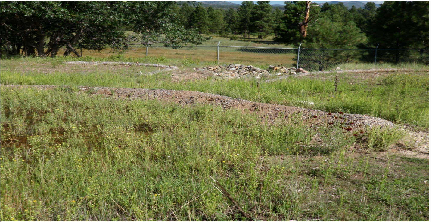
Photo 8520-1r.JPG (taken 08/18/10) V00101010003 : Seed and Mulch - Seed and Wood Mulch; V00101010004 : Seed and Mulch - Seed and Wood Mulch; V00102010002 : Established Vegetation - Permanent Vegetation Grasses and Shrubs; V00103020008 : Berms - Base Course Berm; V00103060005 : Berms - Straw Wattles; V00103060006 : Berms - Straw Wattles; V00106010007 : Check Dam - Rock Check Dam.
