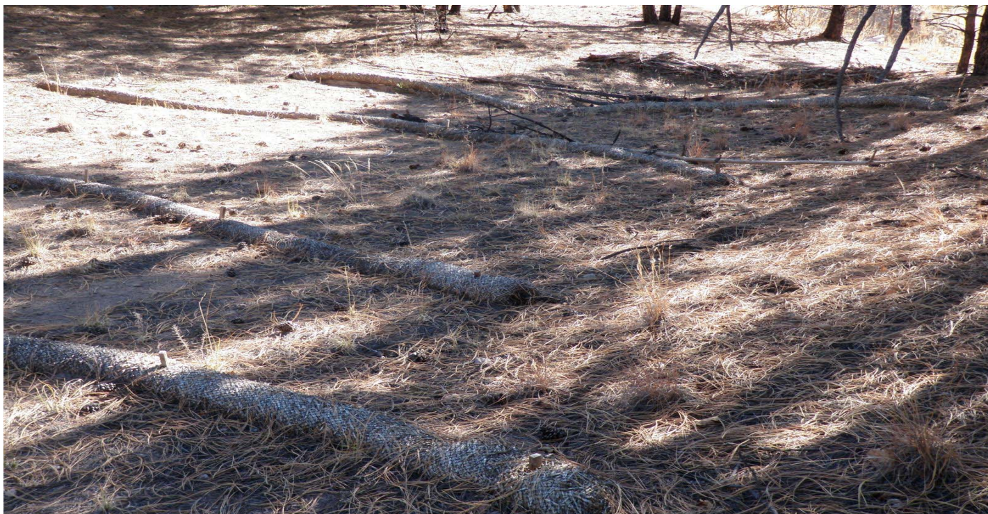
Photo 11807-1r.JPG (taken 08/18/10) V009A03060024 : Berms - Straw Wattles; V009A03060025 : Berms - Straw Wattles; V009A03060026 : Berms - Straw Wattles; V009A03060027 : Berms - Straw Wattles.
