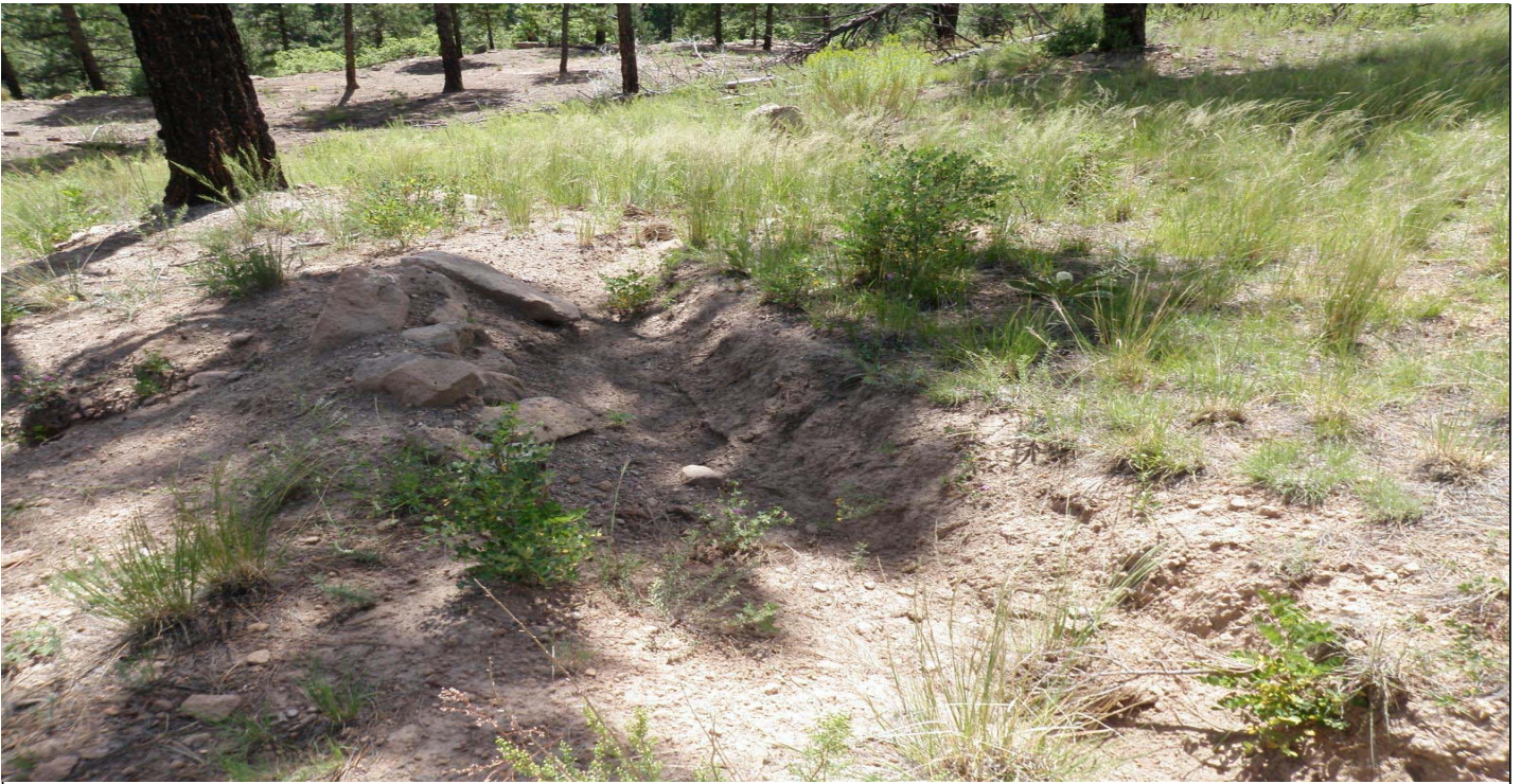
Photo 7507-2r.JPG (taken 08/11/10) J00604010004 : Channel/Swale - Earthen Channel/Swale.
