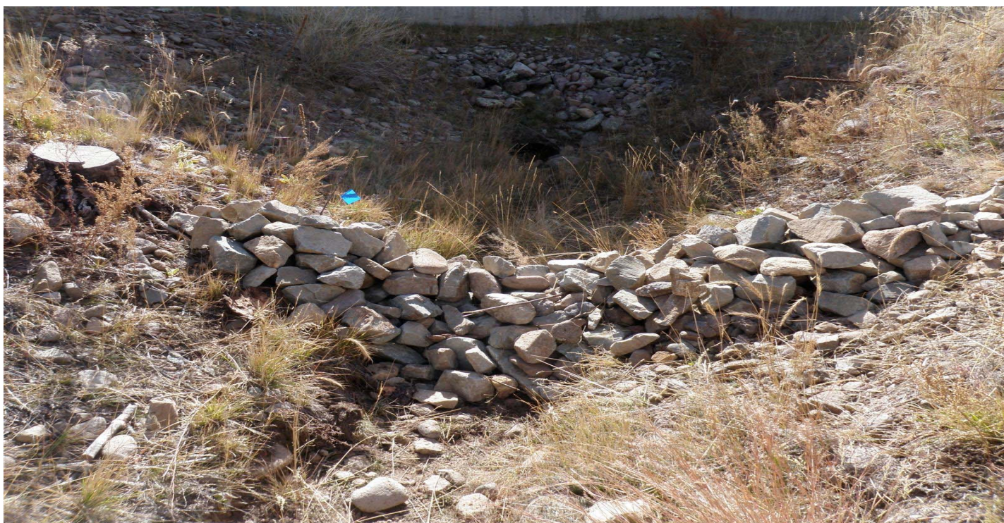
Photo 11699-3r.JPG (taken 11/15/10) V00506010014 : Check Dam - Rock Check Dam.
