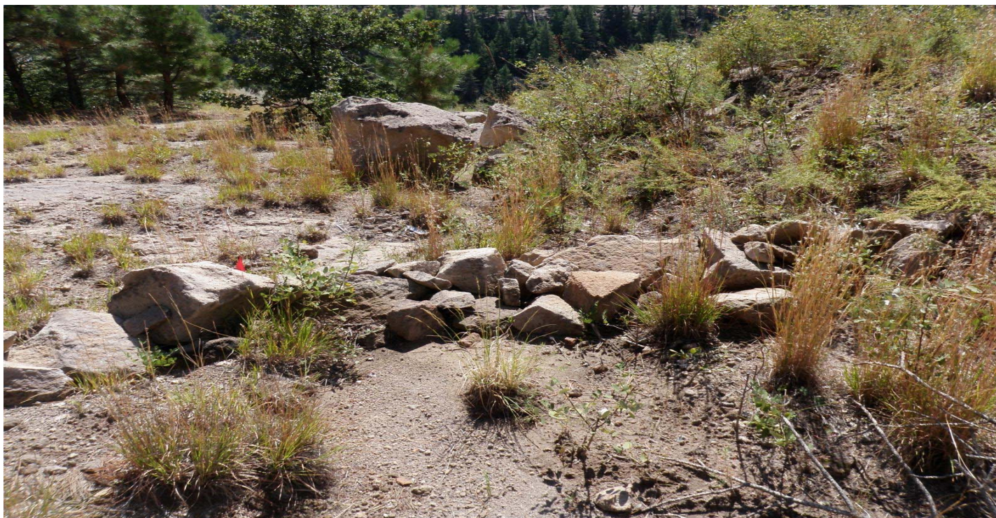
Photo 10865-6r.JPG (taken 10/07/10) J01406010007 : Check Dam - Rock Check Dam.
