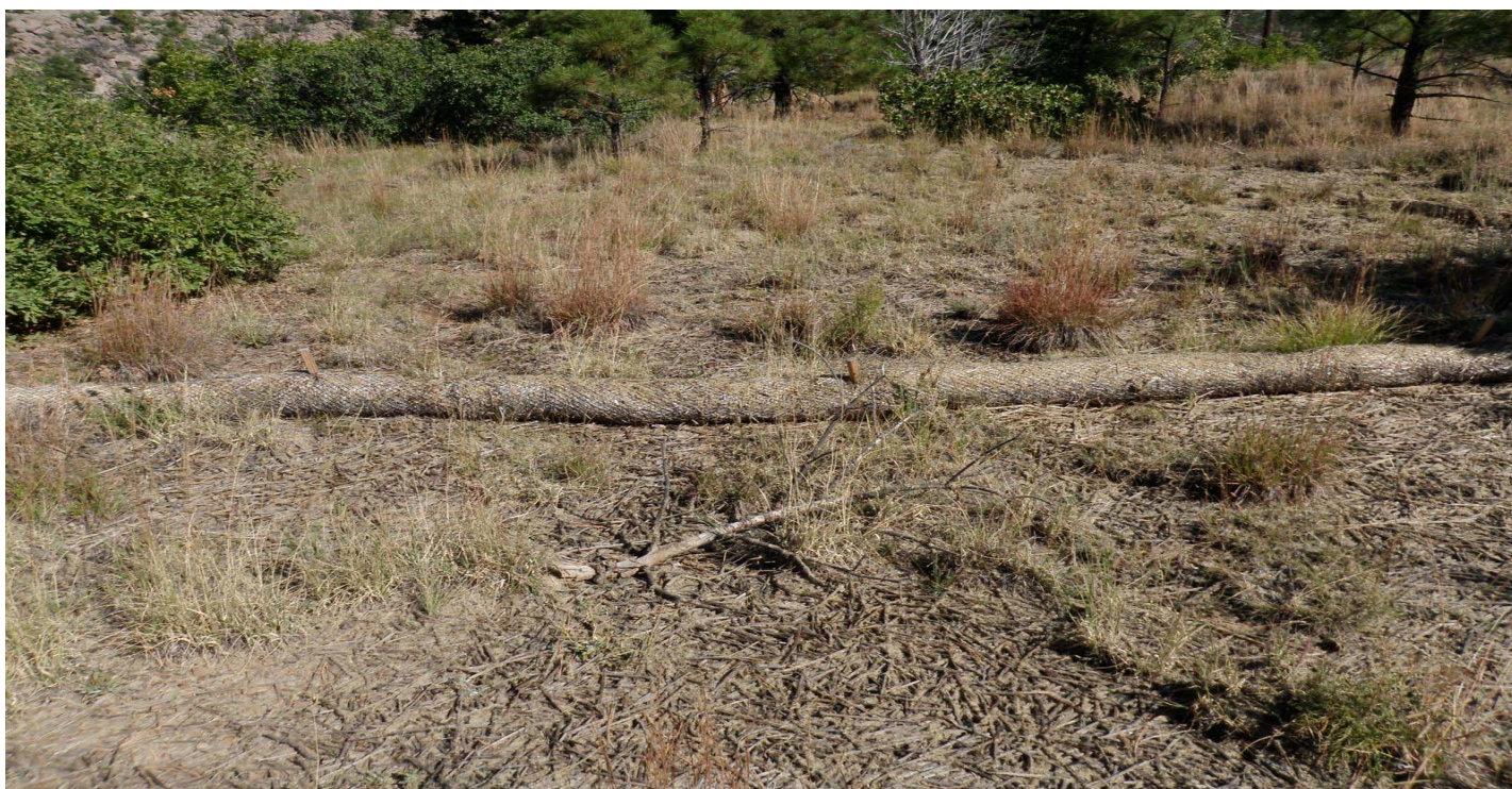
Photo 10872-09r.JPG (taken 10/07/10) H00403060003 : Berms - Straw Wattles.
