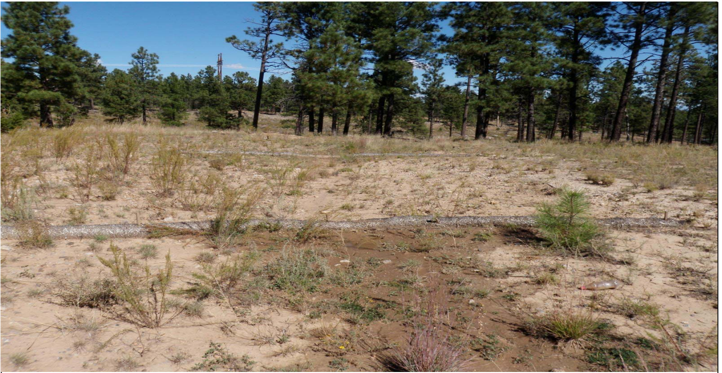
Photo 10867-5r.JPG (taken 10/08/10) E00503060005 : Berms - Straw Wattles; E00503060006 : Berms - Straw Wattles.
