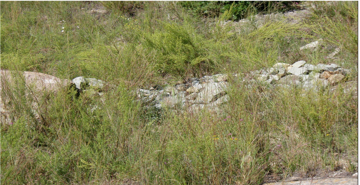
Photo 8525-08r.JPG (taken 08/18/10) V009A06010013 : Check Dam - Rock Check Dam.
