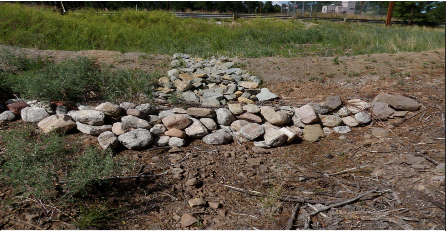
Photo 7801-3r.JPG (taken 08/17/10) W00906010001 : Check Dam - Rock Check Dam.
