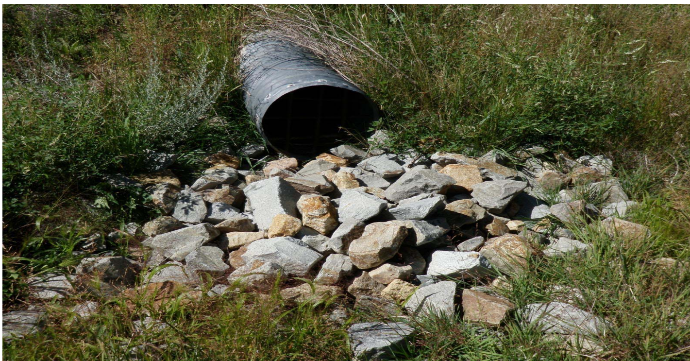
Photo 7593-2r.JPG (taken 08/13/10) H00604060006 : Channel/Swale - Rip Rap.
