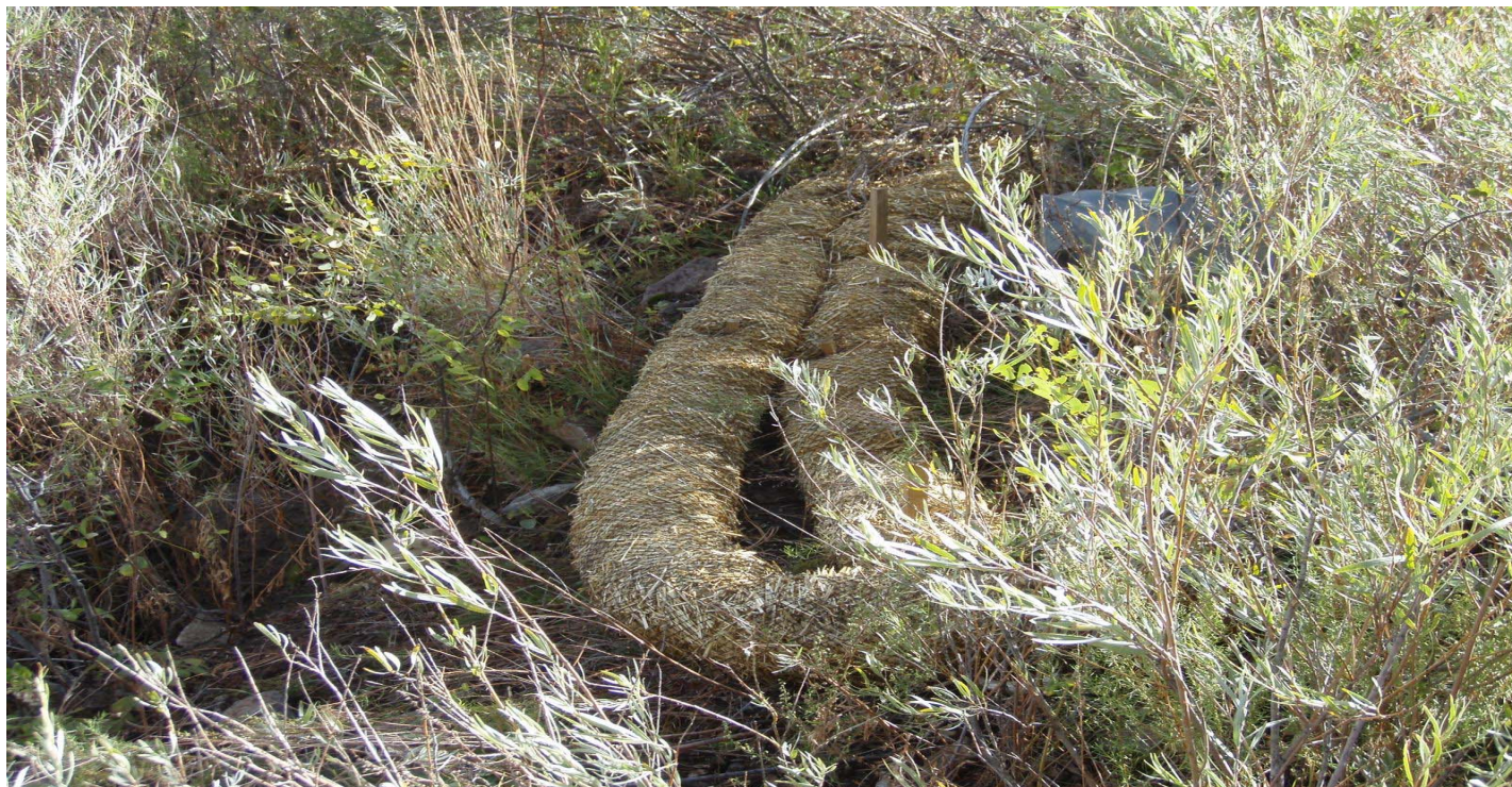
Photo 10879-1r.JPG (taken 10/04/10) W00503060002 : Berms - Straw Wattles.
