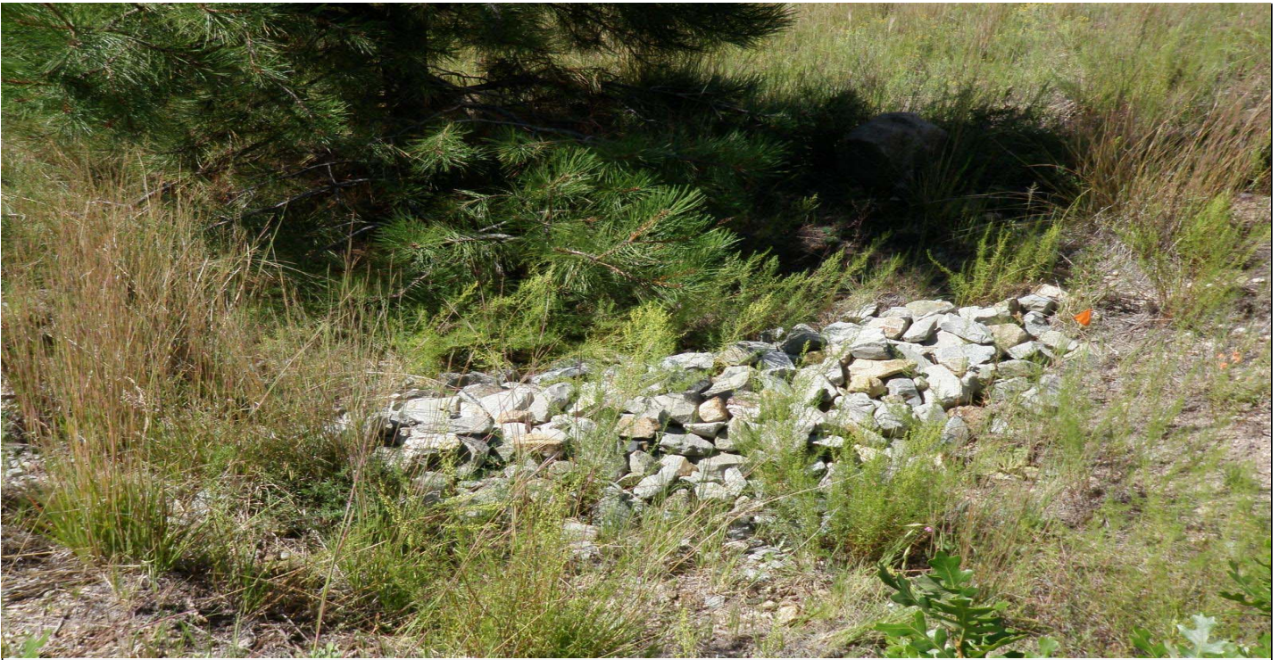
Photo 8525-06r.JPG (taken 08/18/10) V009A06010014 : Check Dam - Rock Check Dam.
