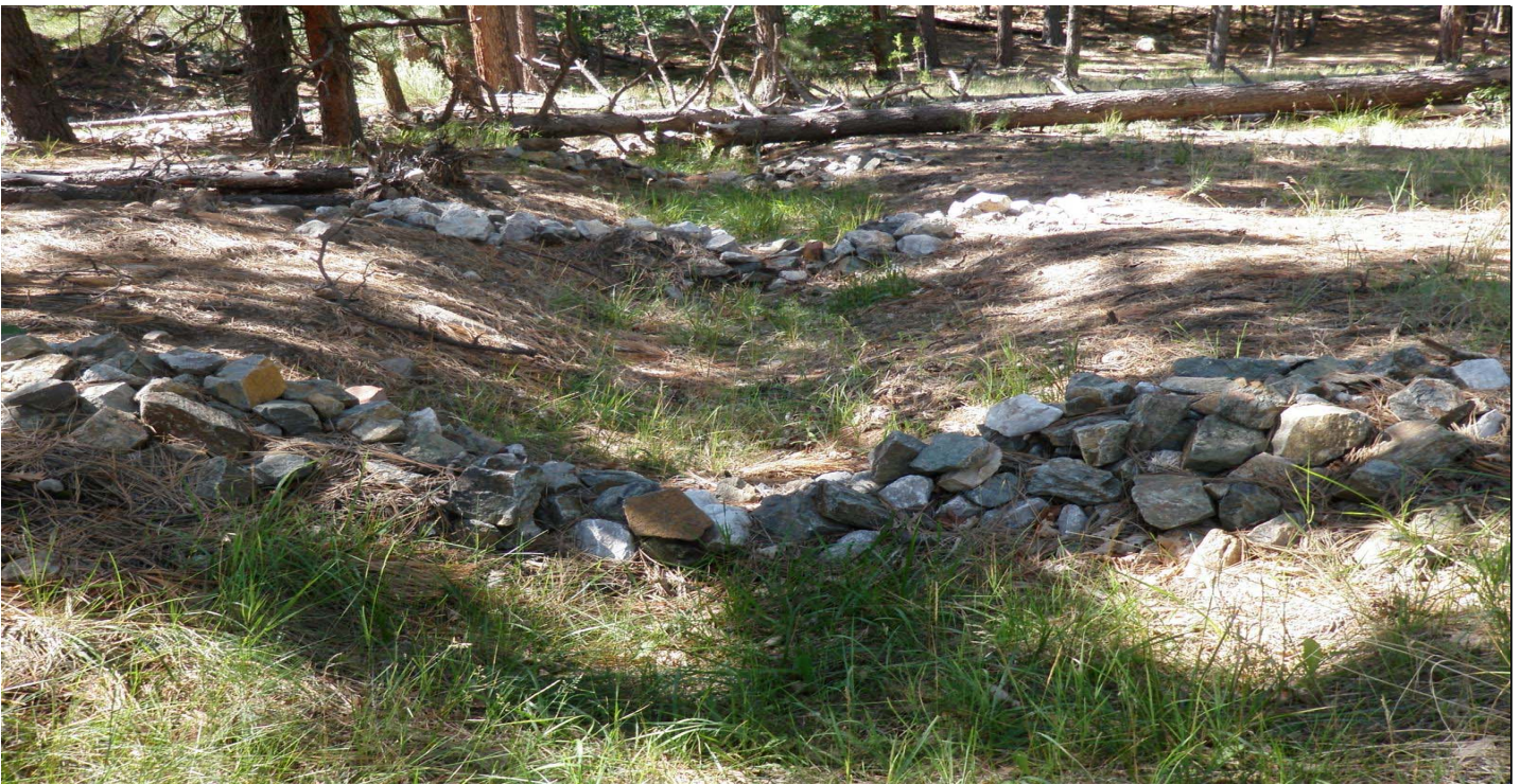
Photo 8522-07r.JPG (taken 08/18/10) V00306010008 : Check Dam - Rock Check Dam; V00306010009 : Check Dam - Rock Check Dam; V00306010010 : Check Dam - Rock Check Dam.
