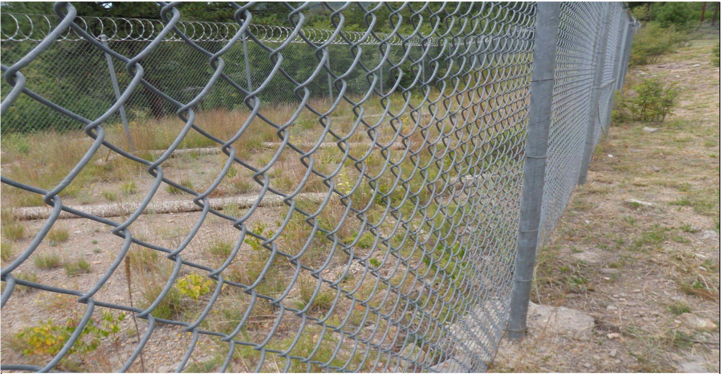
Photo 8794-2r.JPG (taken 09/07/10) W00403060004 : Berms - Straw Wattles; W00403060005 : Berms - Straw Wattles; W00403060006 : Berms - Straw Wattles.
