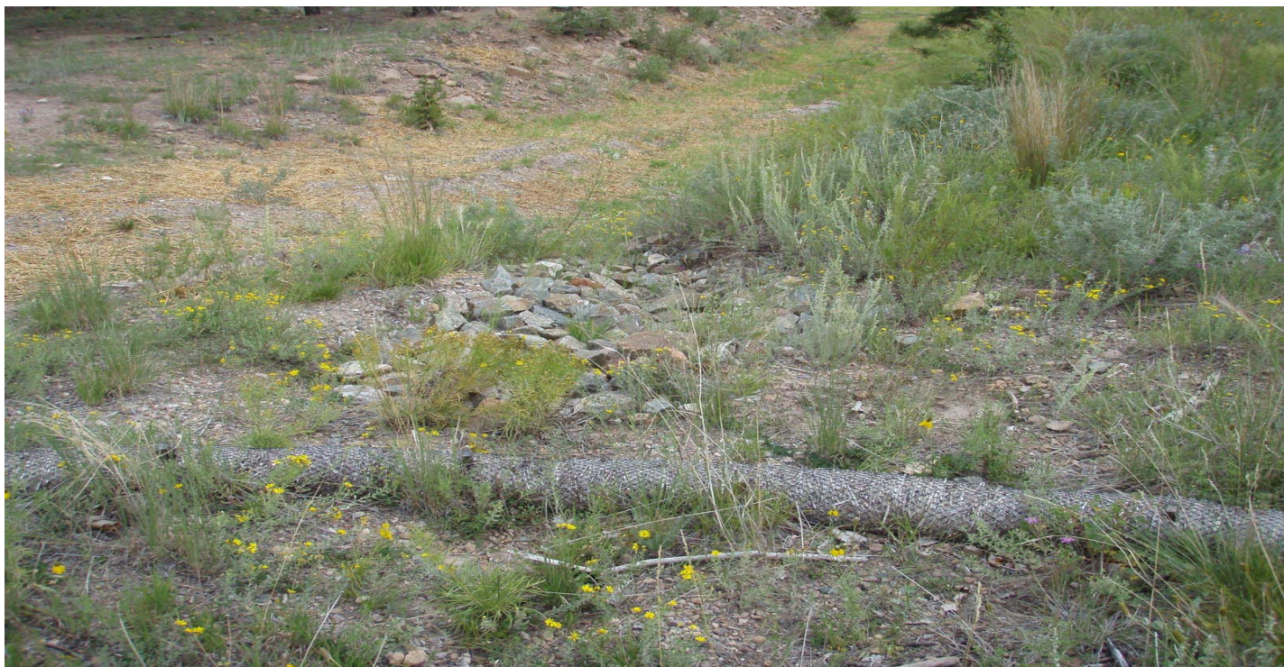
Photo 8531-09r.JPG (taken 08/23/10) W00603060001 : Berms - Straw Wattles; W00604060007 : Channel/Swale - Rip Rap.
