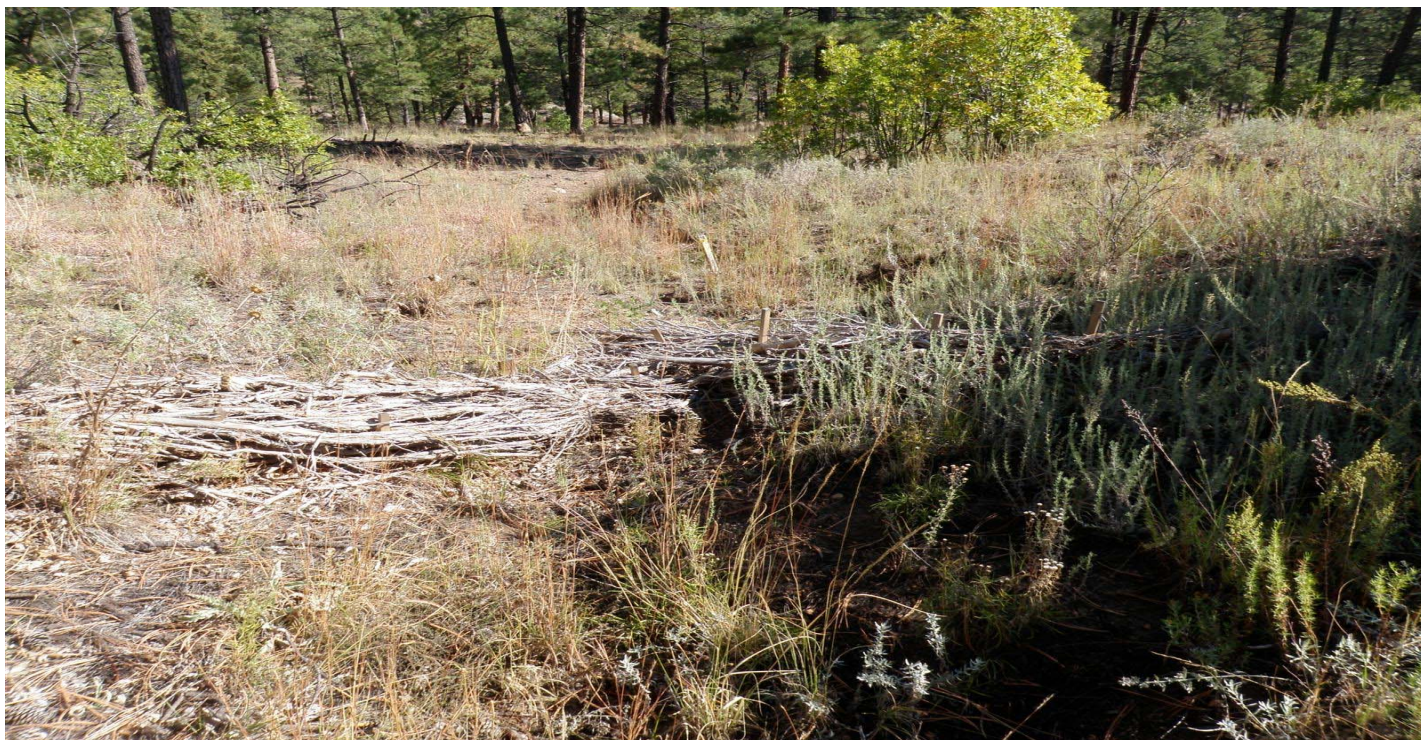
Photo 10877-5r.JPG (taken 10/07/10) W01706030004 : Check Dam - Juniper Bales.
