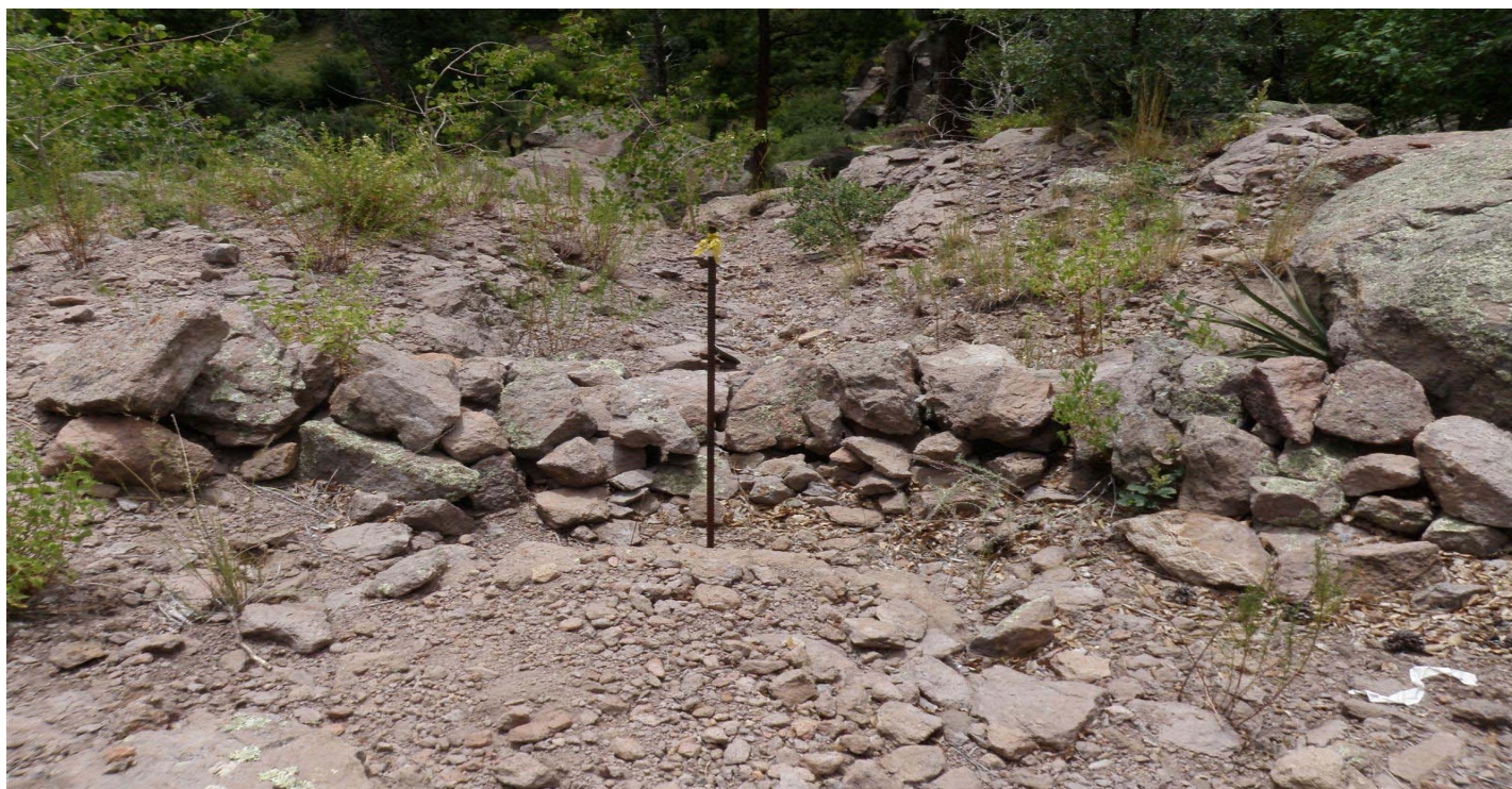
Photo 8796-1r.JPG (taken 09/07/10) W01006010003 : Check Dam - Rock Check Dam.
