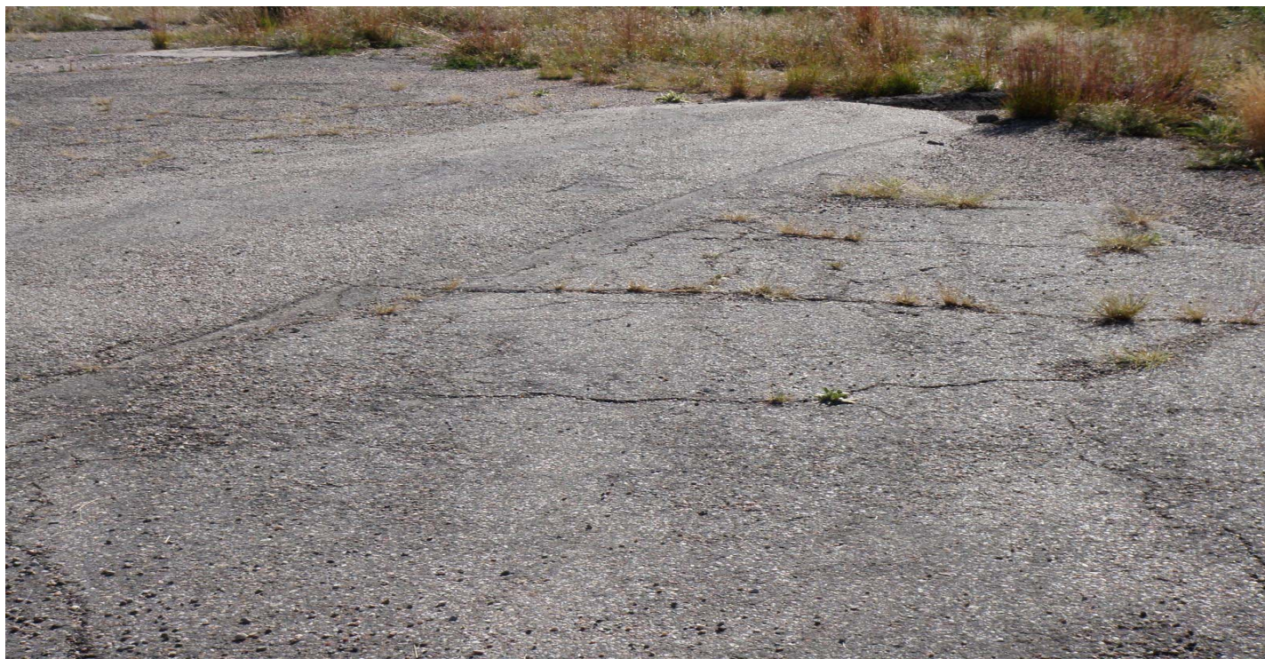
Photo 10878-7r.JPG (taken 10/07/10) W01803040016 : Berms - Asphalt Berm.
