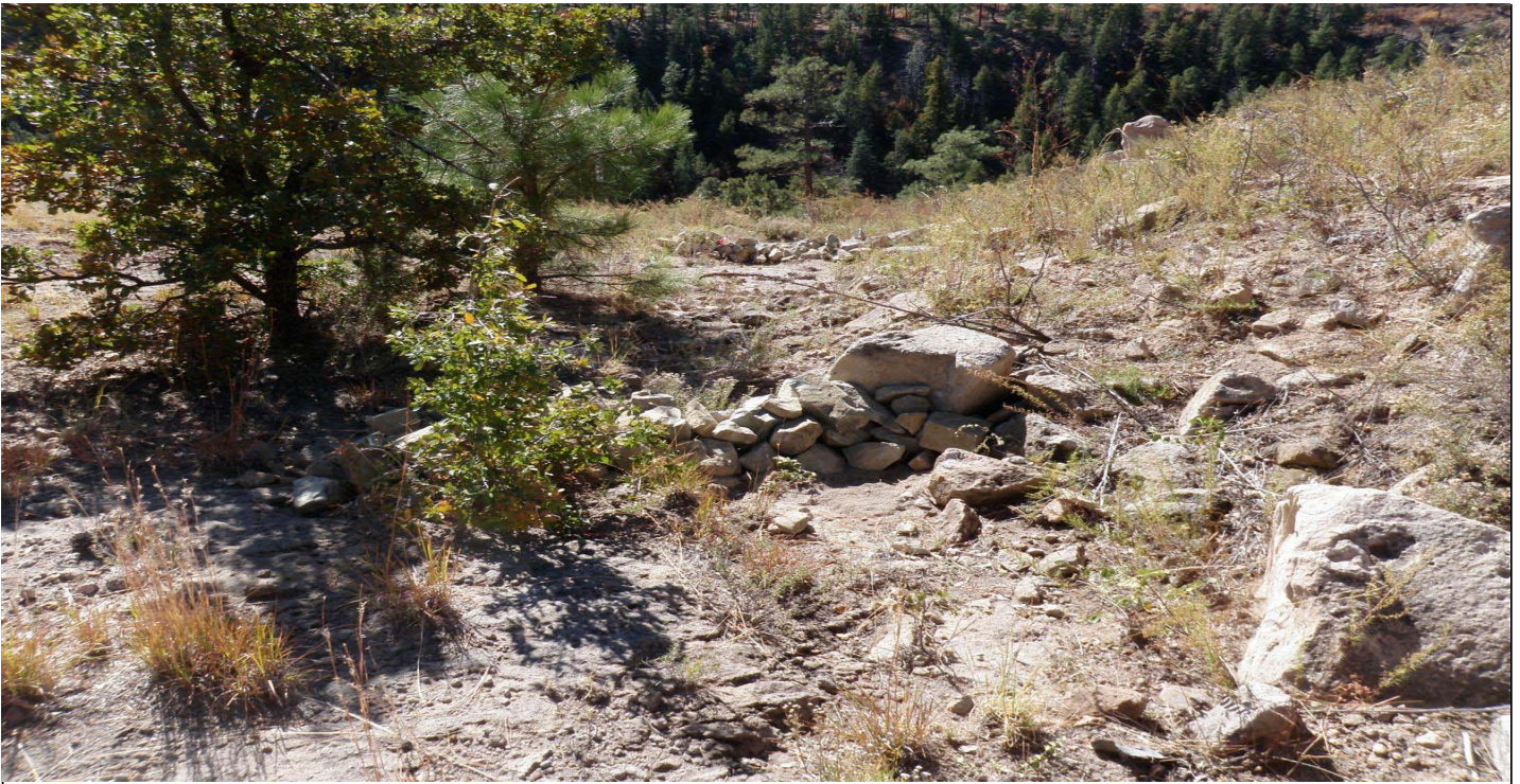
Photo 11459-2r.JPG (taken 10/26/10) J01406010008 : Check Dam - Rock Check Dam; J01406010009 : Check Dam - Rock Check Dam.
