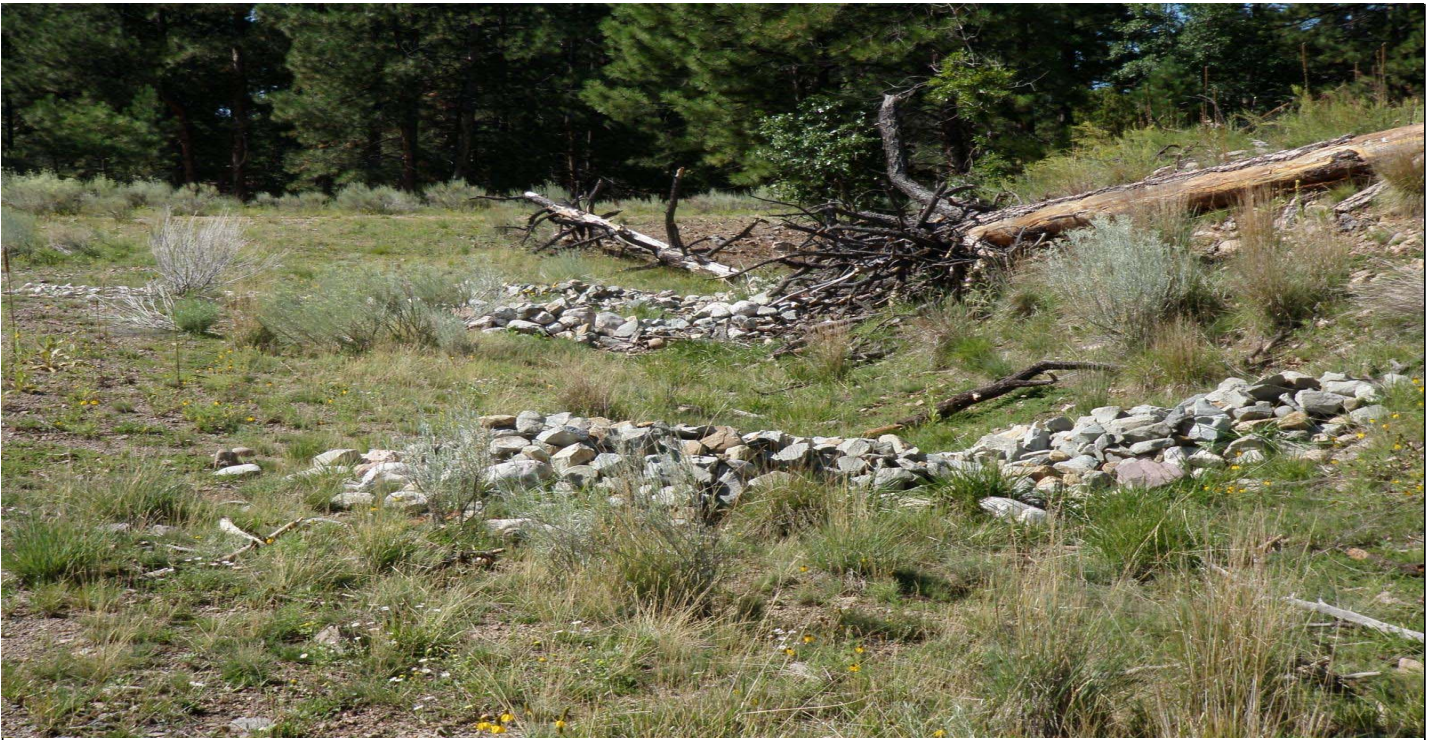
Photo 8522-02r.JPG (taken 08/18/10) V00306010004 : Check Dam - Rock Check Dam; V00306010016 : Check Dam - Rock Check Dam; V00306010026 : Check Dam - Rock Check Dam.
