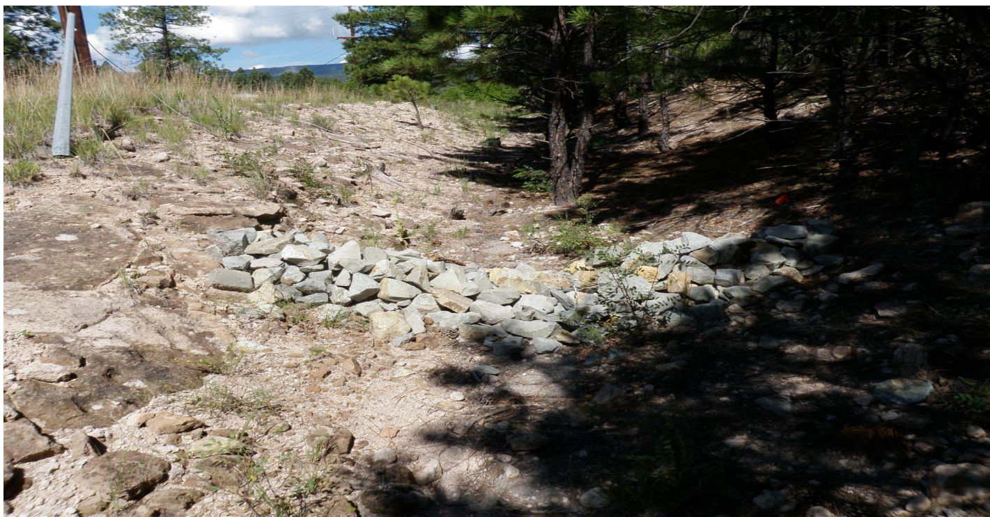
Photo 8525-04r.JPG (taken 08/18/10) V009A06010016 : Check Dam - Rock Check Dam.
