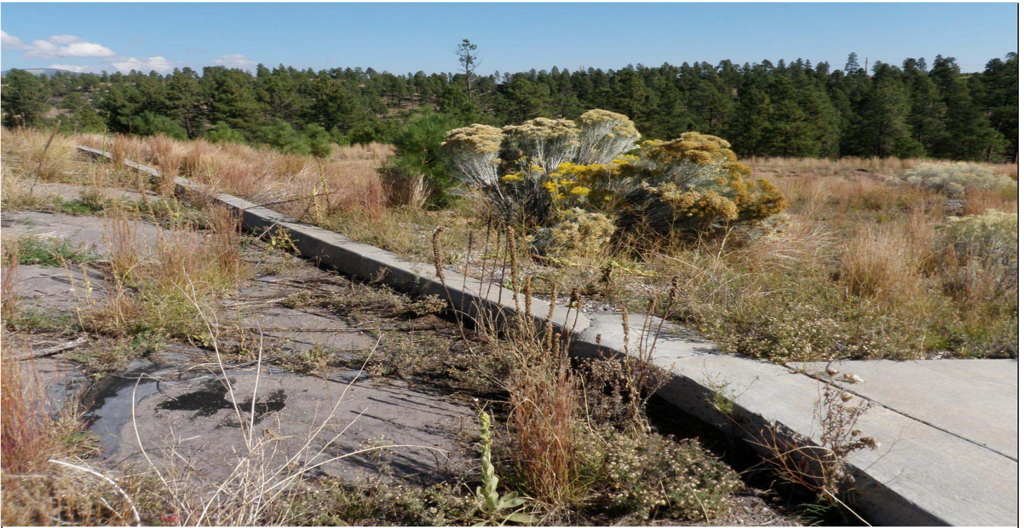
Photo 10878-5r.JPG (taken 10/07/10) W01802010009 : Established Vegetation - Permanent Vegetation Grasses and Shrubs; W01803090002 : Berms - Curbing.
