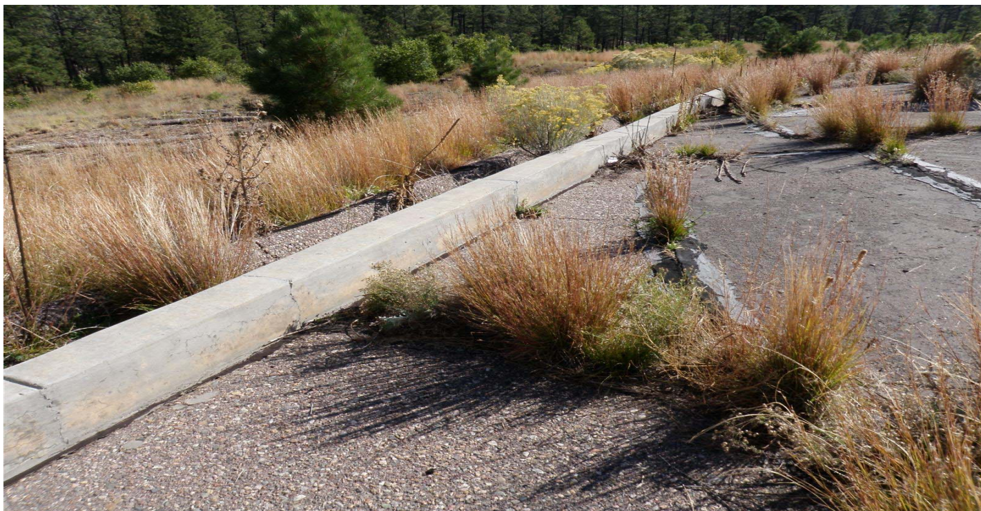
Photo 10877-6r.JPG (taken 10/07/10) W01703090001 : Berms - Curbing.
