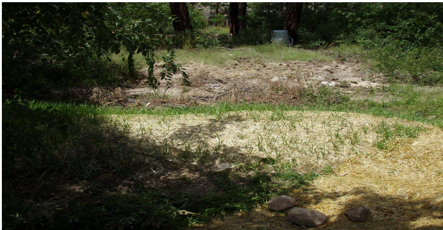
Photo 8536-2r.JPG (taken 08/23/10) V01503010004 : Berms - Earthen Berm.
