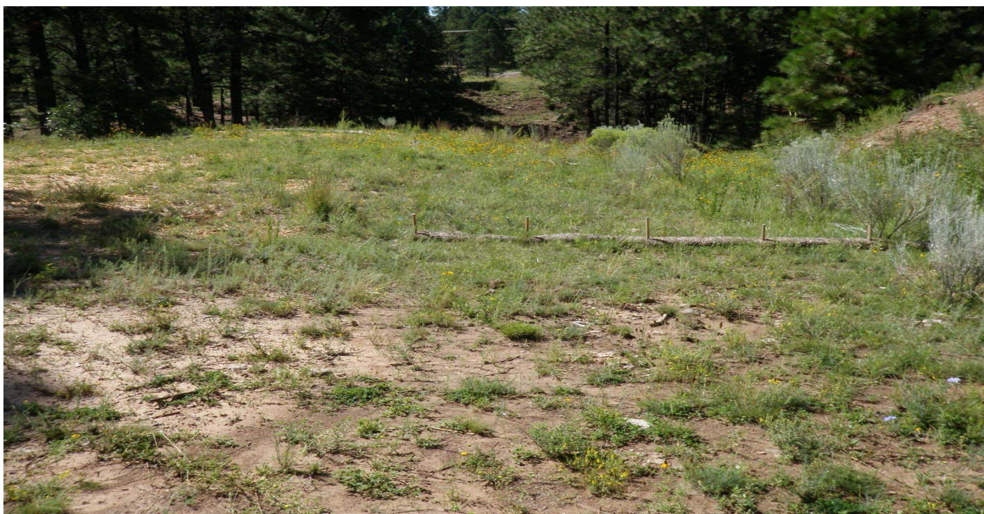
Photo 8522-15r.JPG (taken 08/18/10) V00303060018 : Berms - Straw Wattles.
