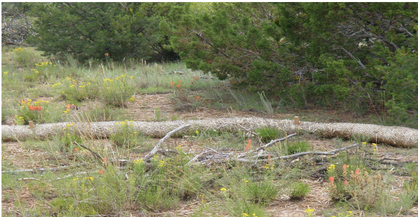
Photo 8519-5.JPG (taken 08/04/10) W01903060030 : Berms - Straw Wattles.
