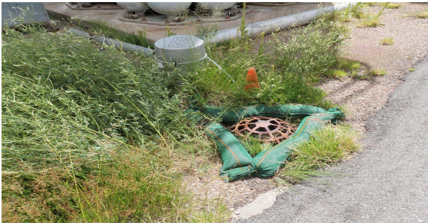
Photo 7521-2r.JPG (taken 08/12/10) E01103100003 : Berms - Gravel Bags.
