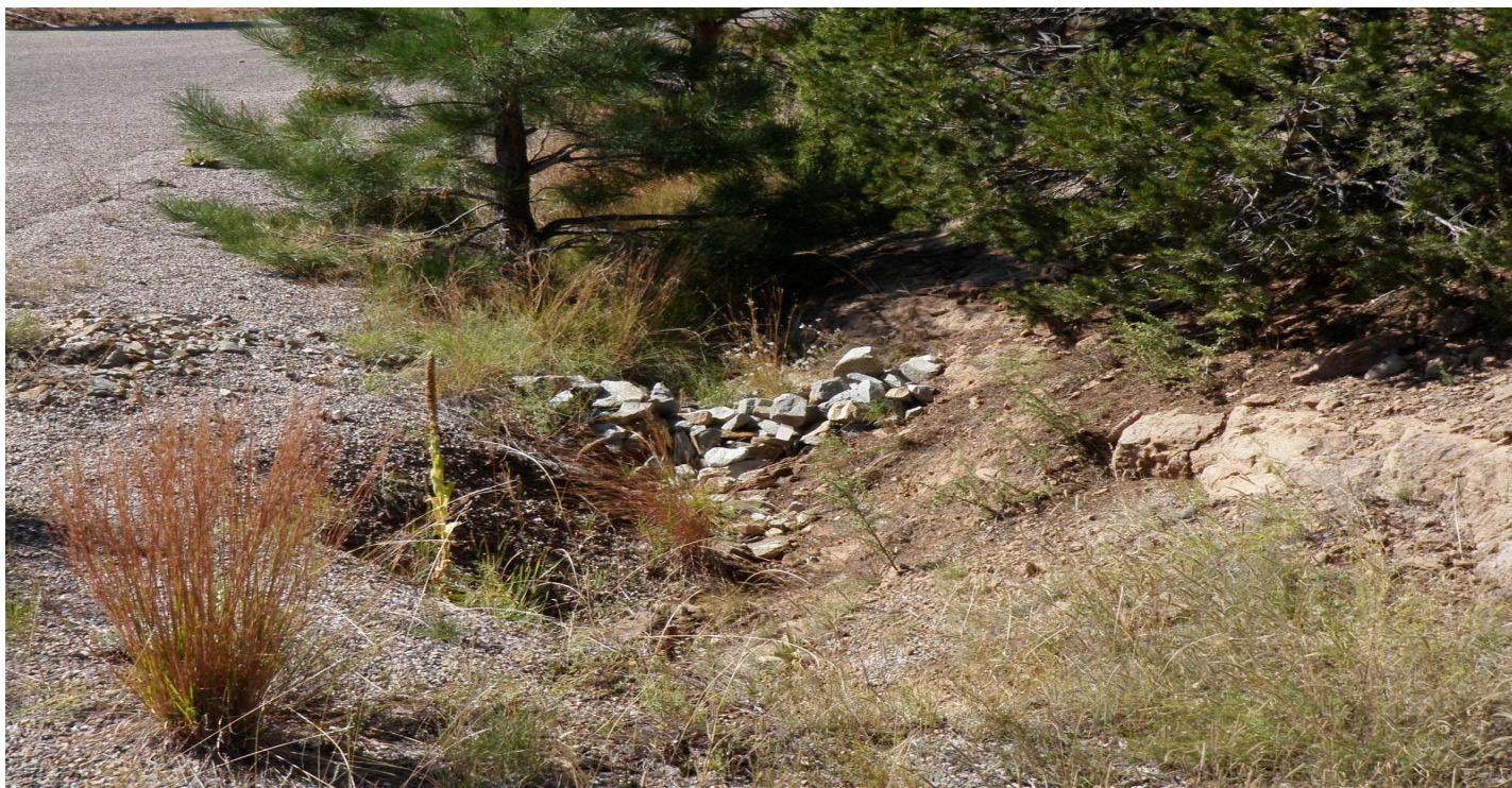
Photo 10873-03r.JPG (taken 10/07/10) H00306010011 : Check Dam - Rock Check Dam.
