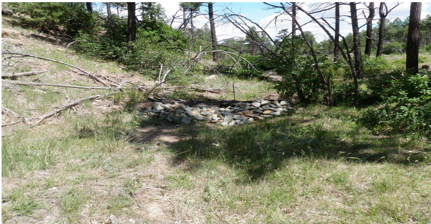
Photo 8527-3r.JPG (taken 08/18/10) V00706010005 : Check Dam - Rock Check Dam.
