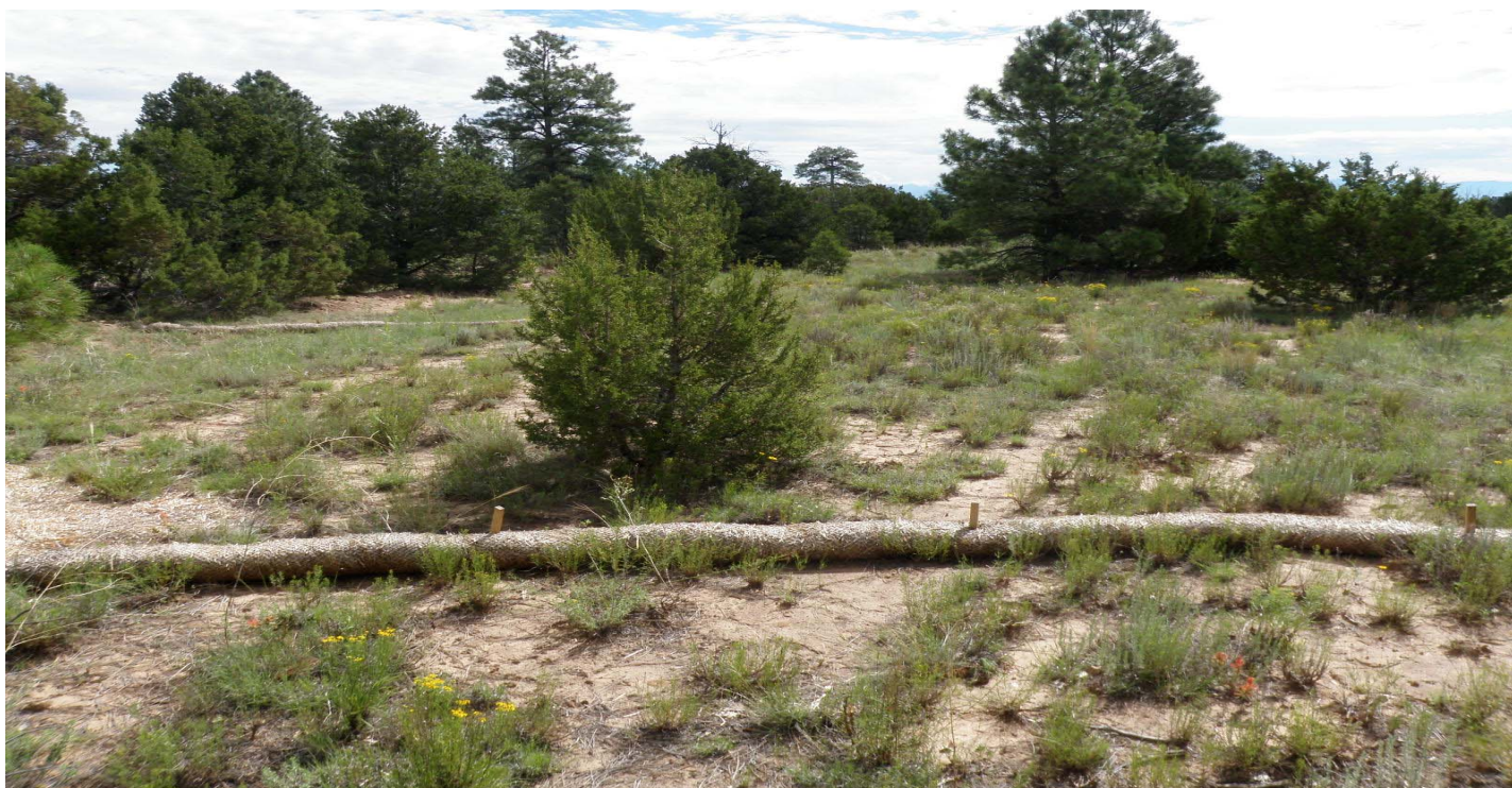
Photo 8519-13.JPG (taken 08/04/10) W01903060009 : Berms - Straw Wattles; W01903060011 : Berms - Straw Wattles.
