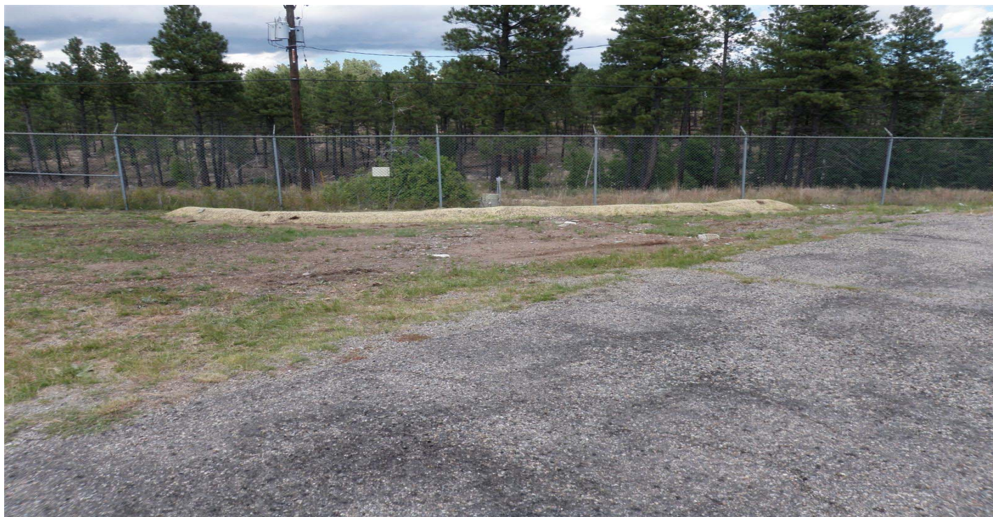
Photo 10881-1r.JPG (taken 10/04/10) E00703010005 : Berms - Earthen Berm.
