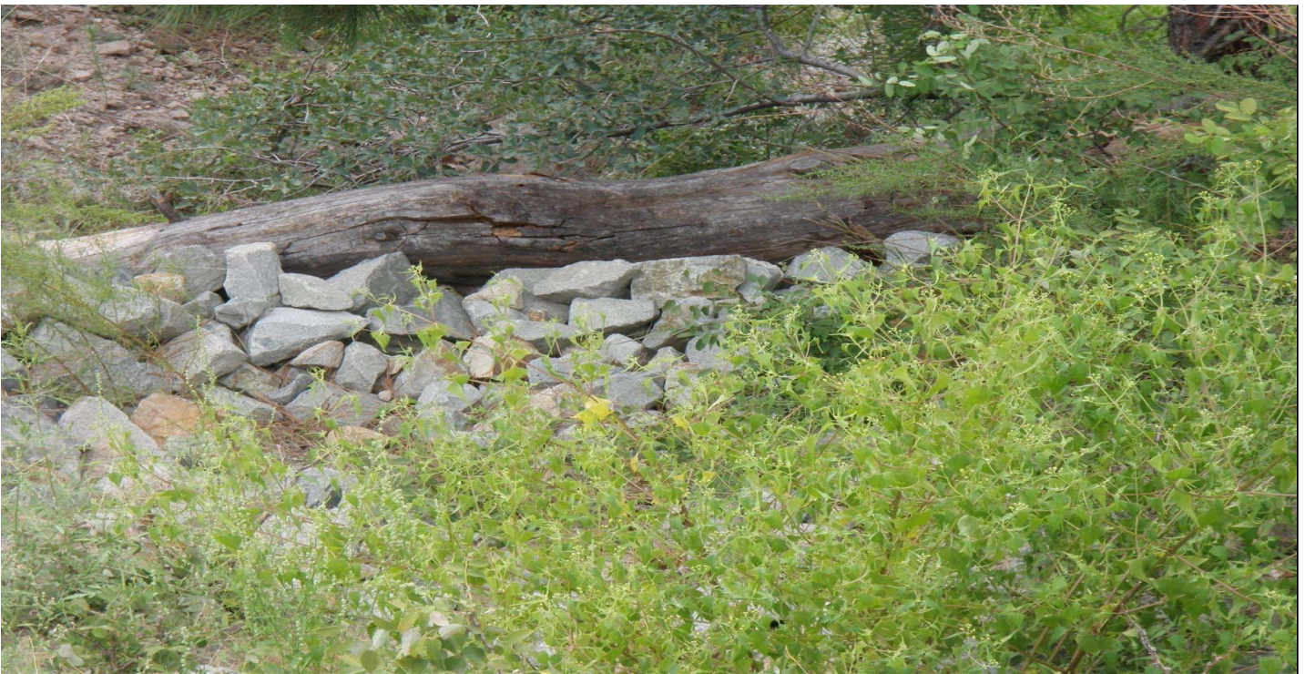
Photo 7512-3r.JPG (taken 08/12/10) J01202010005 : Established Vegetation - Permanent Vegetation Grasses and Shrubs; J01204060004 : Channel/Swale - Rip Rap.
