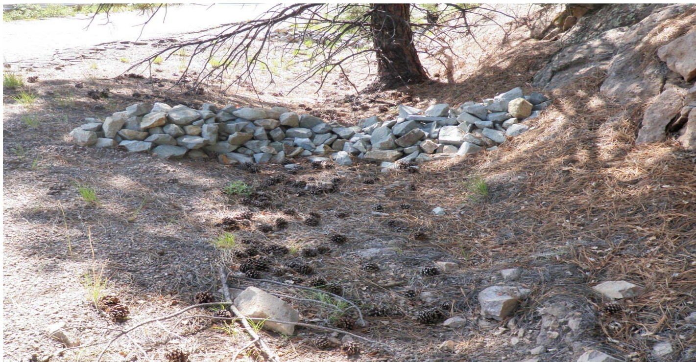
Photo 7806-1r.JPG (taken 08/17/10) W01106010006 : Check Dam - Rock Check Dam.
