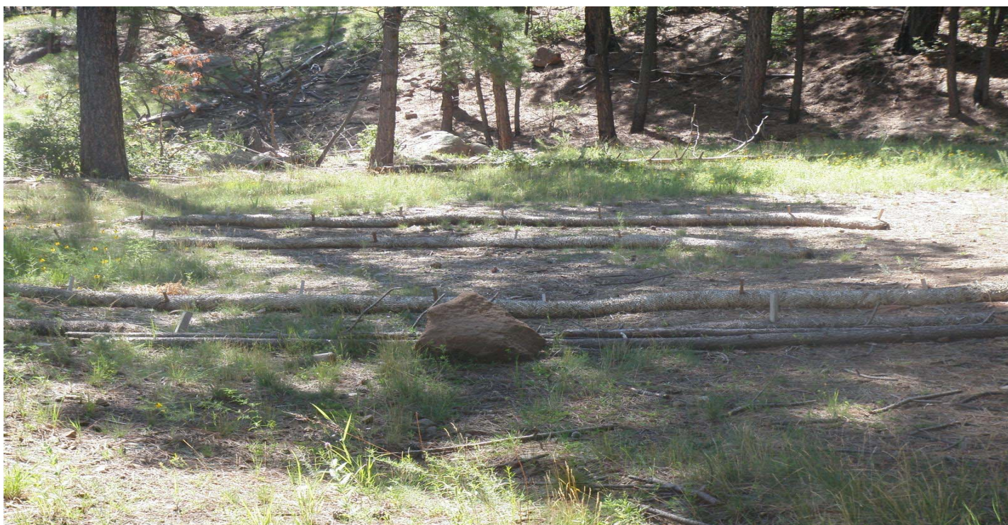
Photo 8522-11r.JPG (taken 08/18/10) V00303060022 : Berms - Straw Wattles; V00303060023 : Berms - Straw Wattles; V00303060024 : Berms - Straw Wattles.
