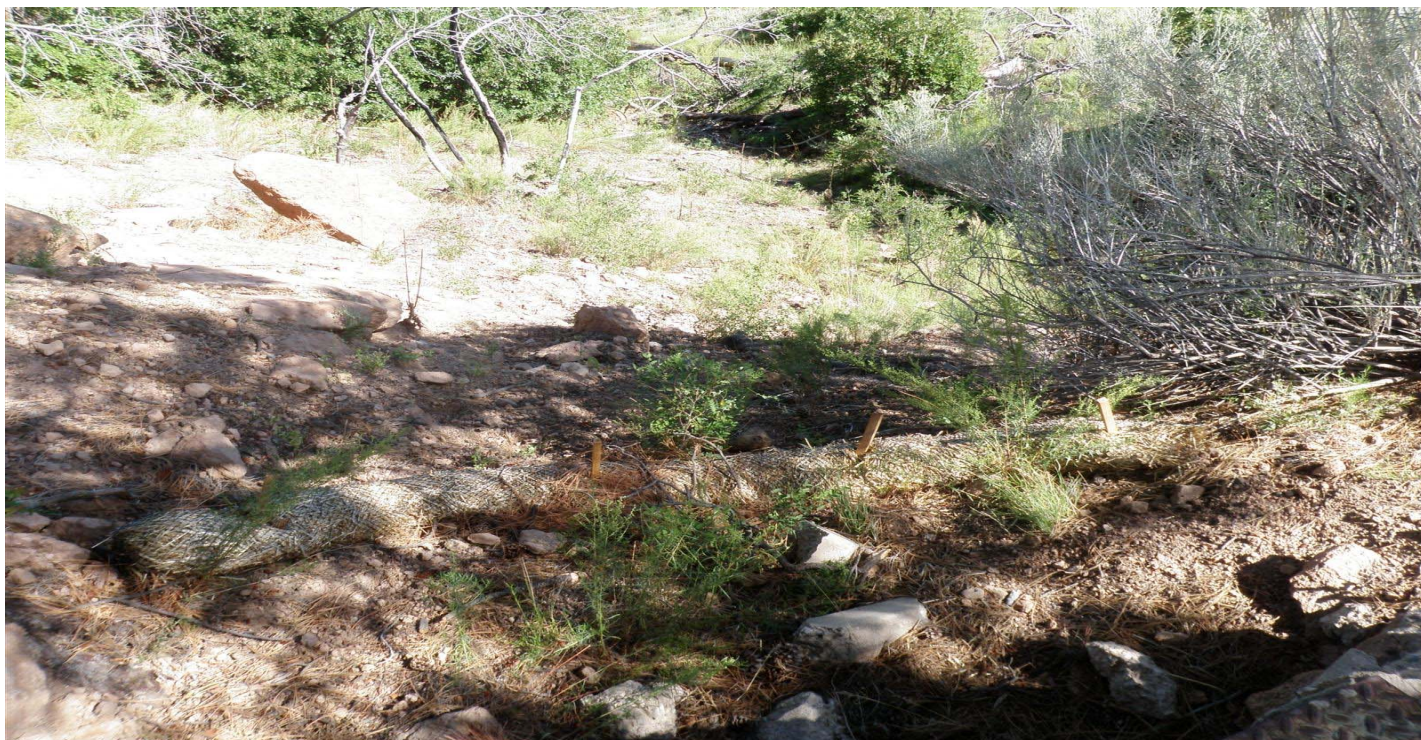
Photo 7804-2r.JPG (taken 08/17/10) W012A02010001 : Established Vegetation - Permanent Vegetation Grasses and Shrubs; W012A03060002 : Berms - Straw Wattles.
