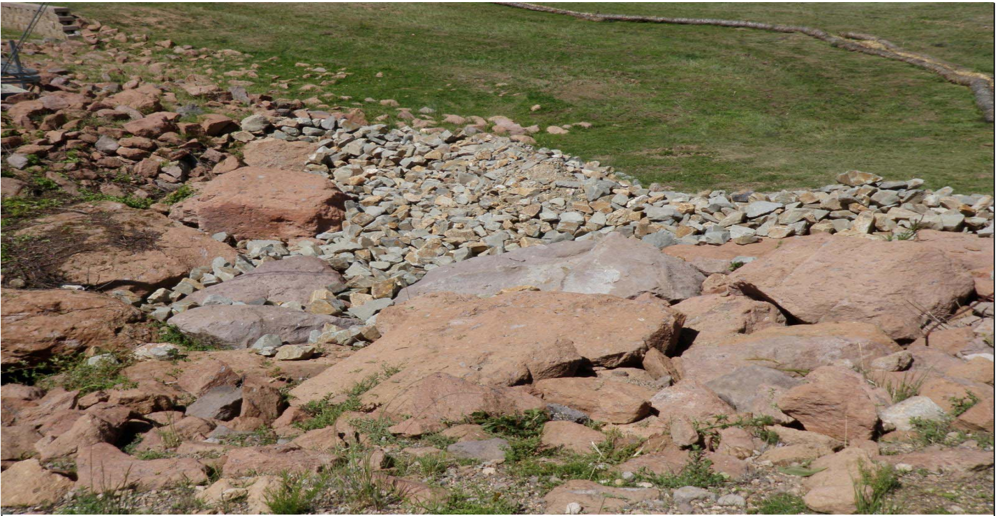
Photo 8524-03r.JPG (taken 08/18/10) V00904060005 : Channel/Swale - Rip Rap; V00906010022 : Check Dam - Rock Check Dam.
