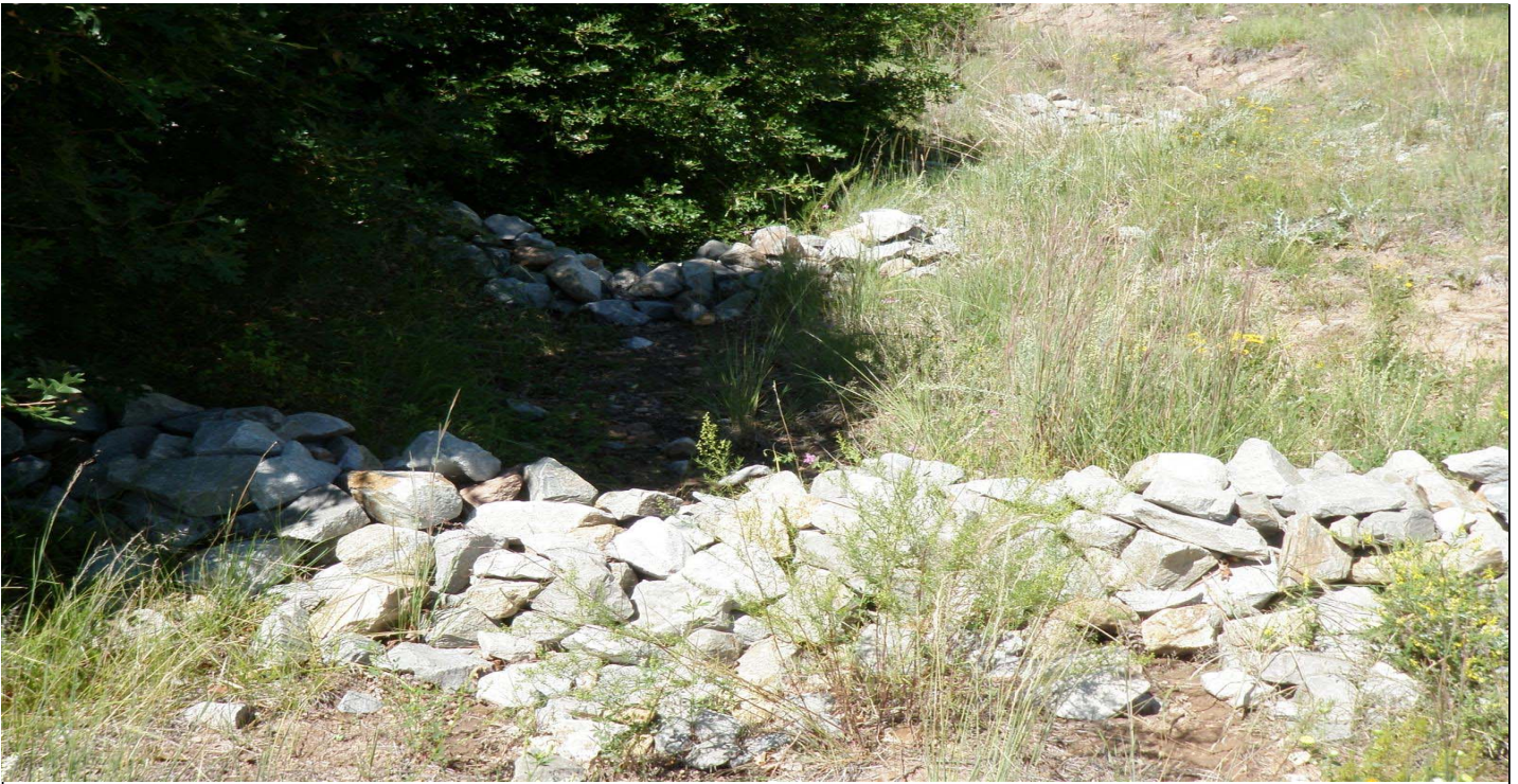
Photo 8524-05r.JPG (taken 08/18/10) V00906010017 : Check Dam - Rock Check Dam; V00906010018 : Check Dam - Rock Check Dam.
