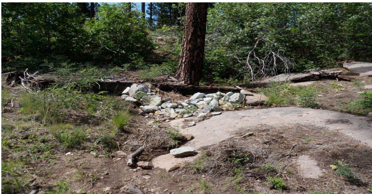
Photo 7807-3r.JPG (taken 08/17/10) W00306010004 : Check Dam - Rock Check Dam.
