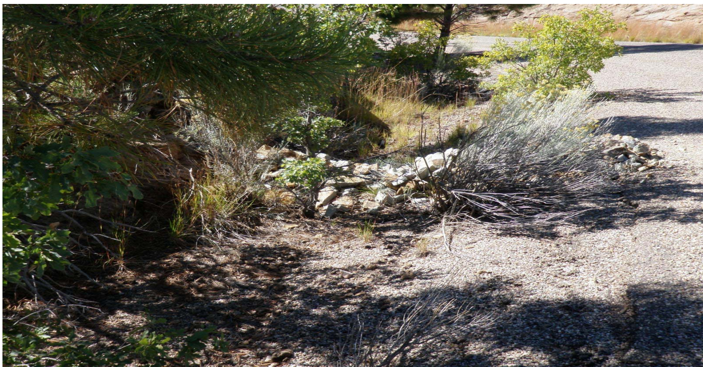
Photo 10873-02r.JPG (taken 10/07/10) H00306010013 : Check Dam - Rock Check Dam.
