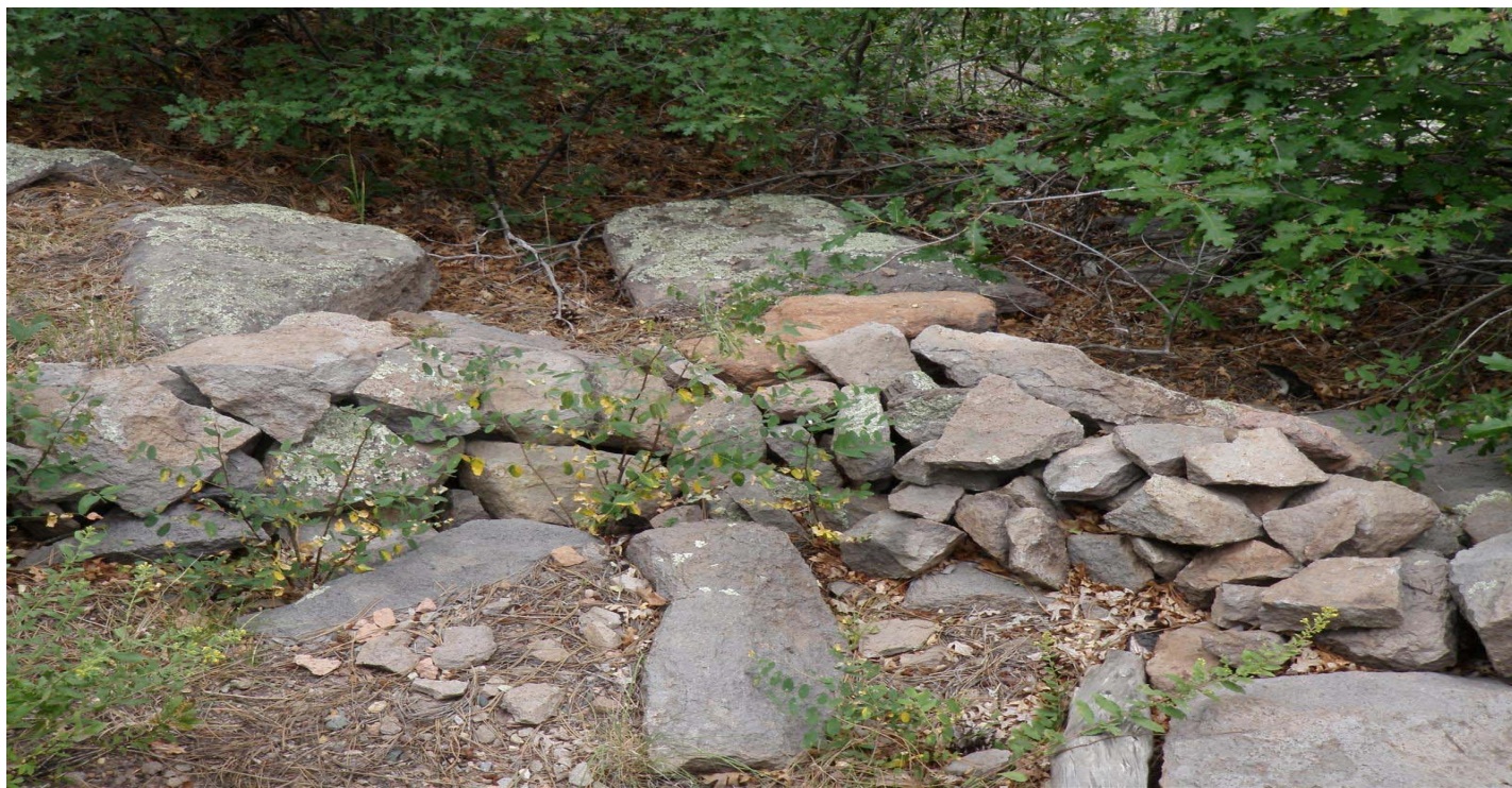
Photo 8794-3r.JPG (taken 09/07/10) W00406010007 : Check Dam - Rock Check Dam.
