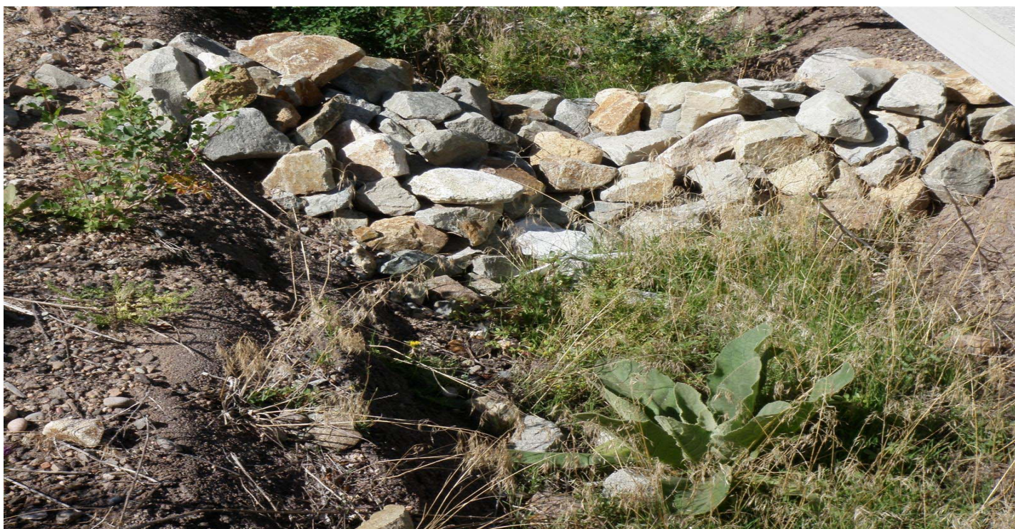
Photo 7523-2r.JPG (taken 08/12/10) J01606010006 : Check Dam - Rock Check Dam.
