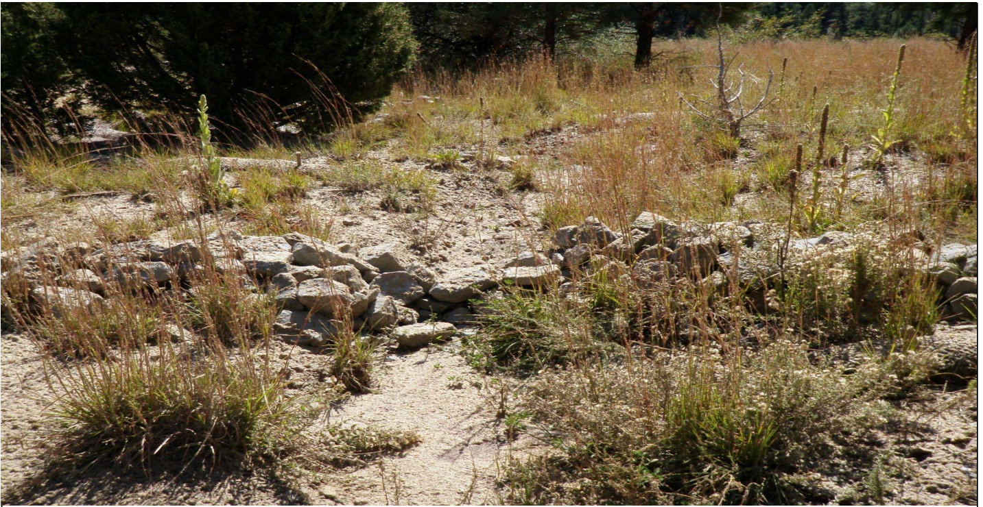
Photo 10864-3r.JPG (taken 10/07/10) J01306010005 : Check Dam - Rock Check Dam.
