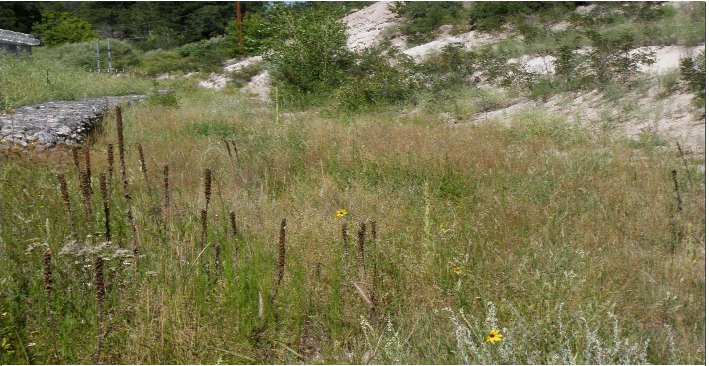
Photo 7593-3r.JPG (taken 08/13/10) H00602010004 : Established Vegetation - Permanent Vegetation Grasses and Shrubs; H00607010002 : Gabions - Gabions.
