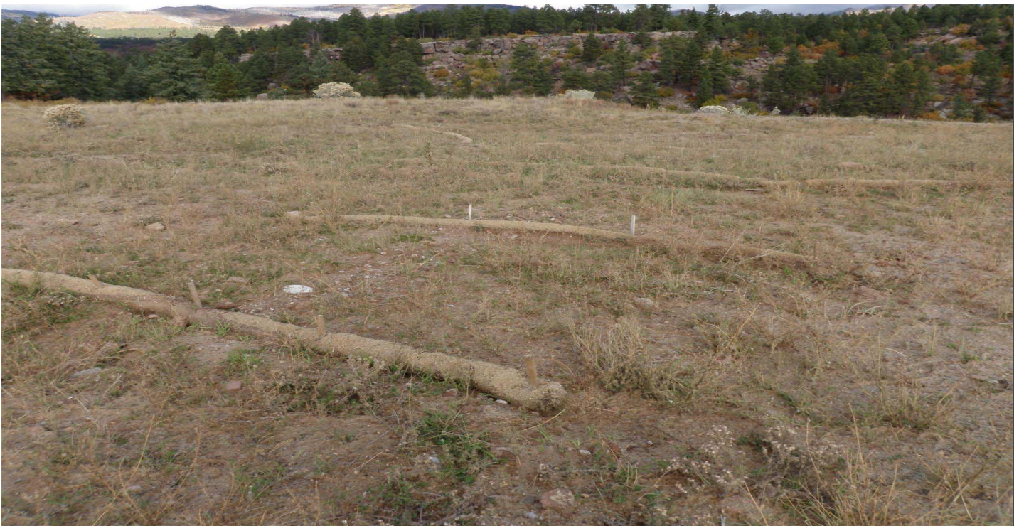
Photo 11465-2r.JPG (taken 10/22/10) V008A03060008 : Berms - Straw Wattles; V008A03060011 : Berms - Straw Wattles; V008A03060012 : Berms - Straw Wattles; V008A03060014 : Berms - Straw Wattles.
