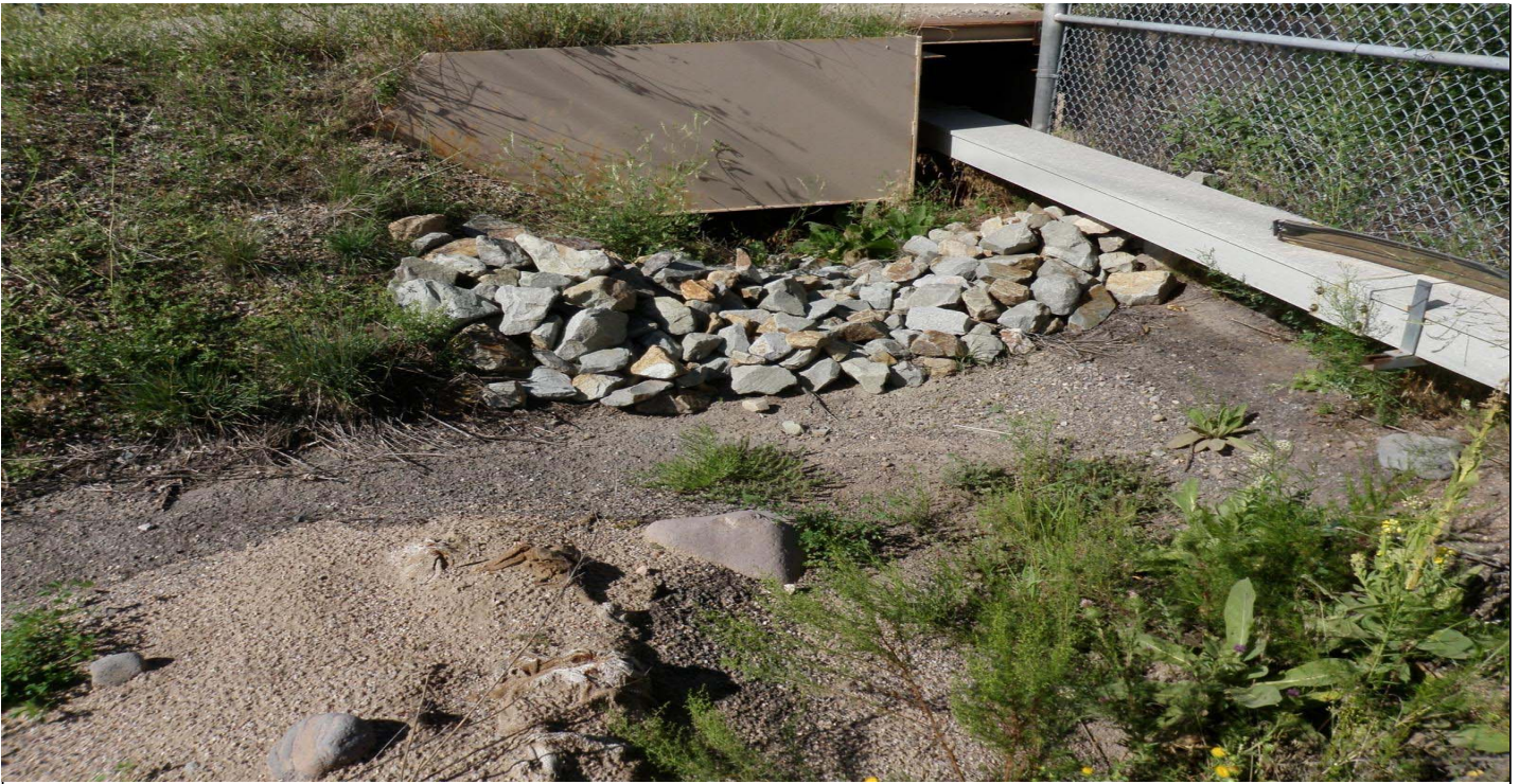
Photo 7523-3r.JPG (taken 08/12/10) J01606010004 : Check Dam - Rock Check Dam.
