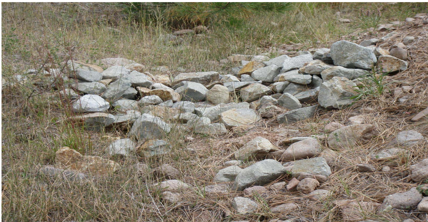
Photo 10885-1r.JPG (taken 10/01/10) V00506010010 : Check Dam - Rock Check Dam.
