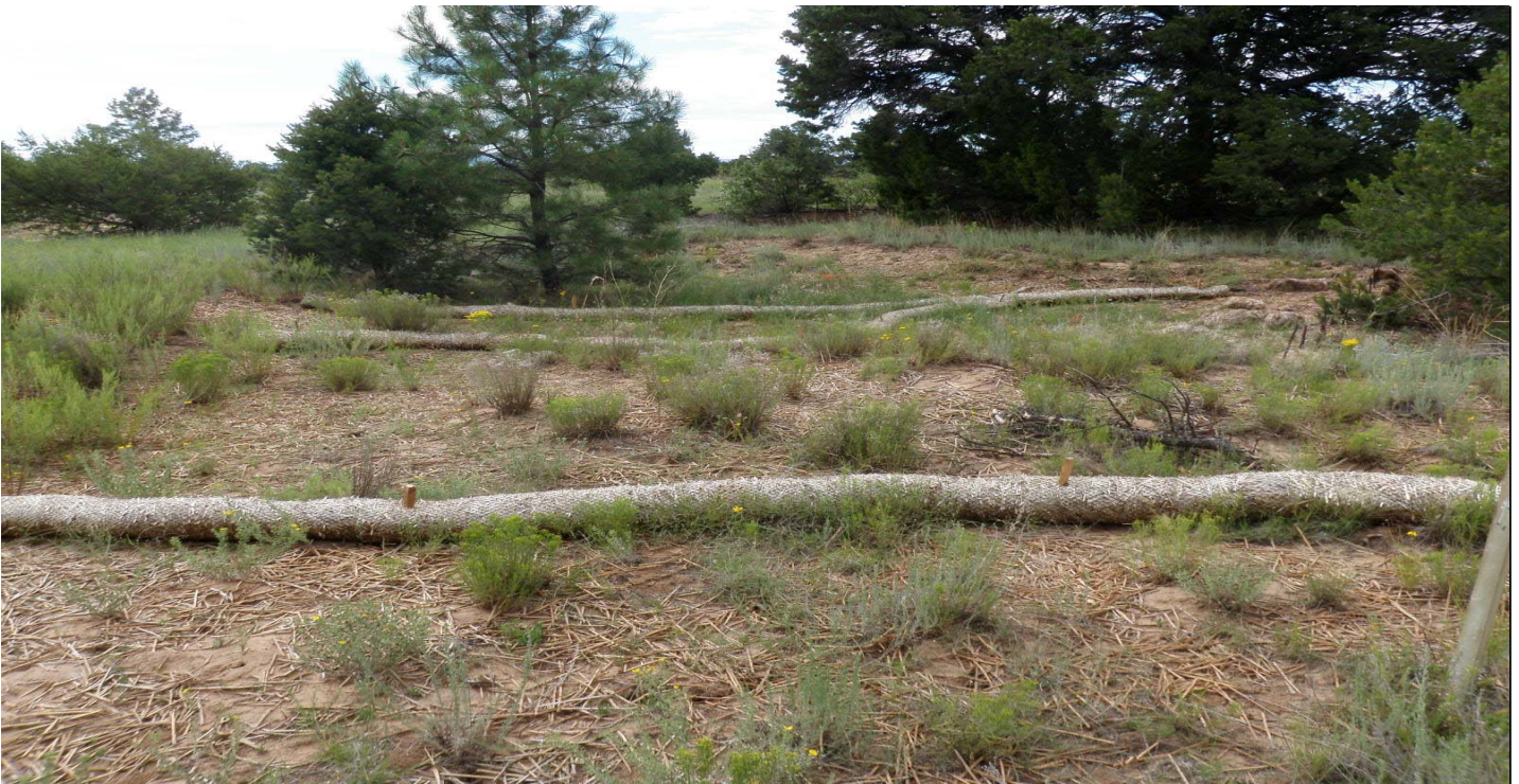
Photo 8519-7.JPG (taken 08/04/10) W01901010039 : Seed and Mulch - Seed and Wood Mulch; W01903060020 : Berms - Straw Wattles; W01903060021 : Berms - Straw Wattles; W01903060022 : Berms - Straw Wattles.
