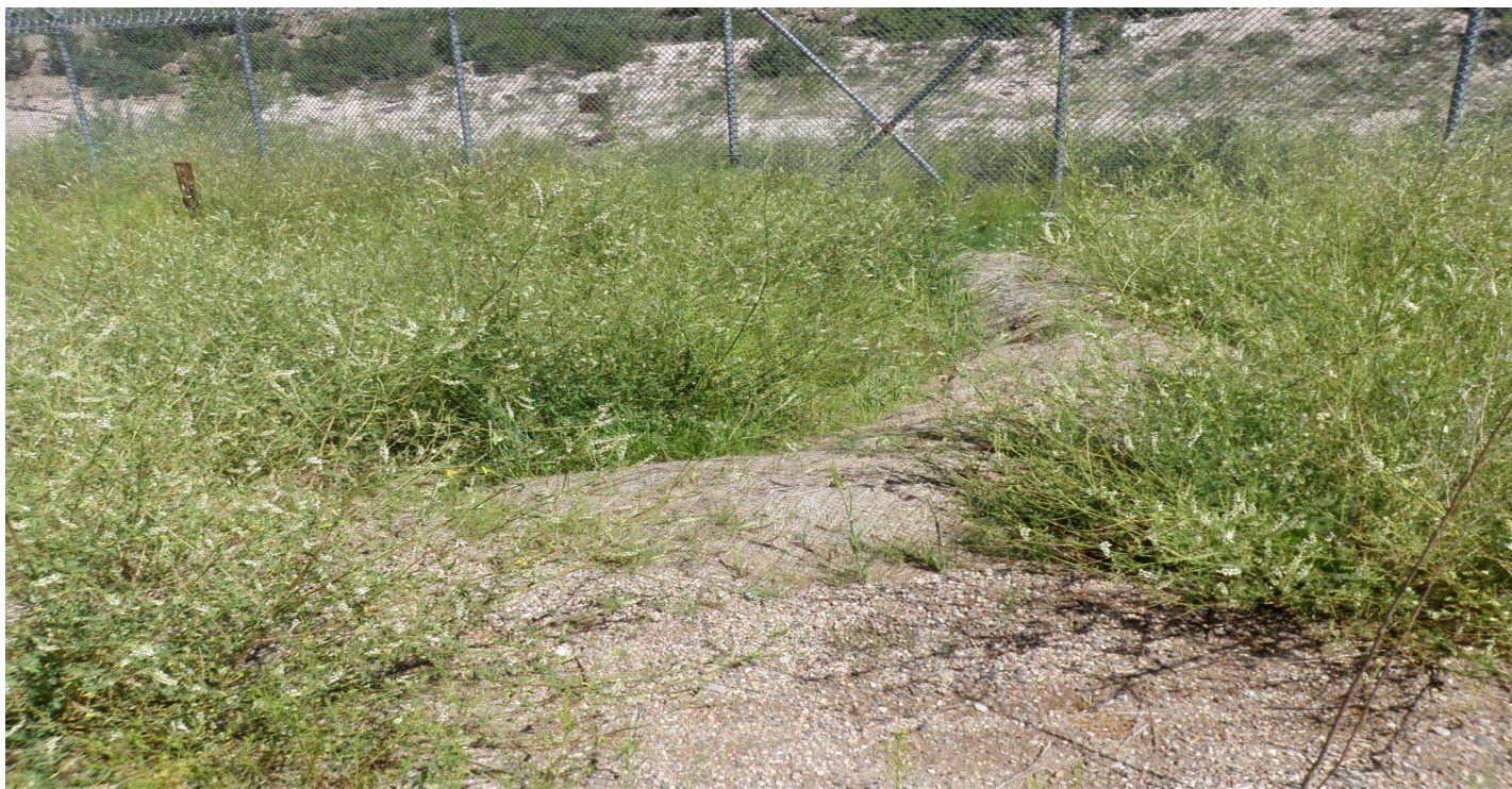
Photo 7593-5r.JPG (taken 08/13/10) H00603010007 : Berms - Earthen Berm.
