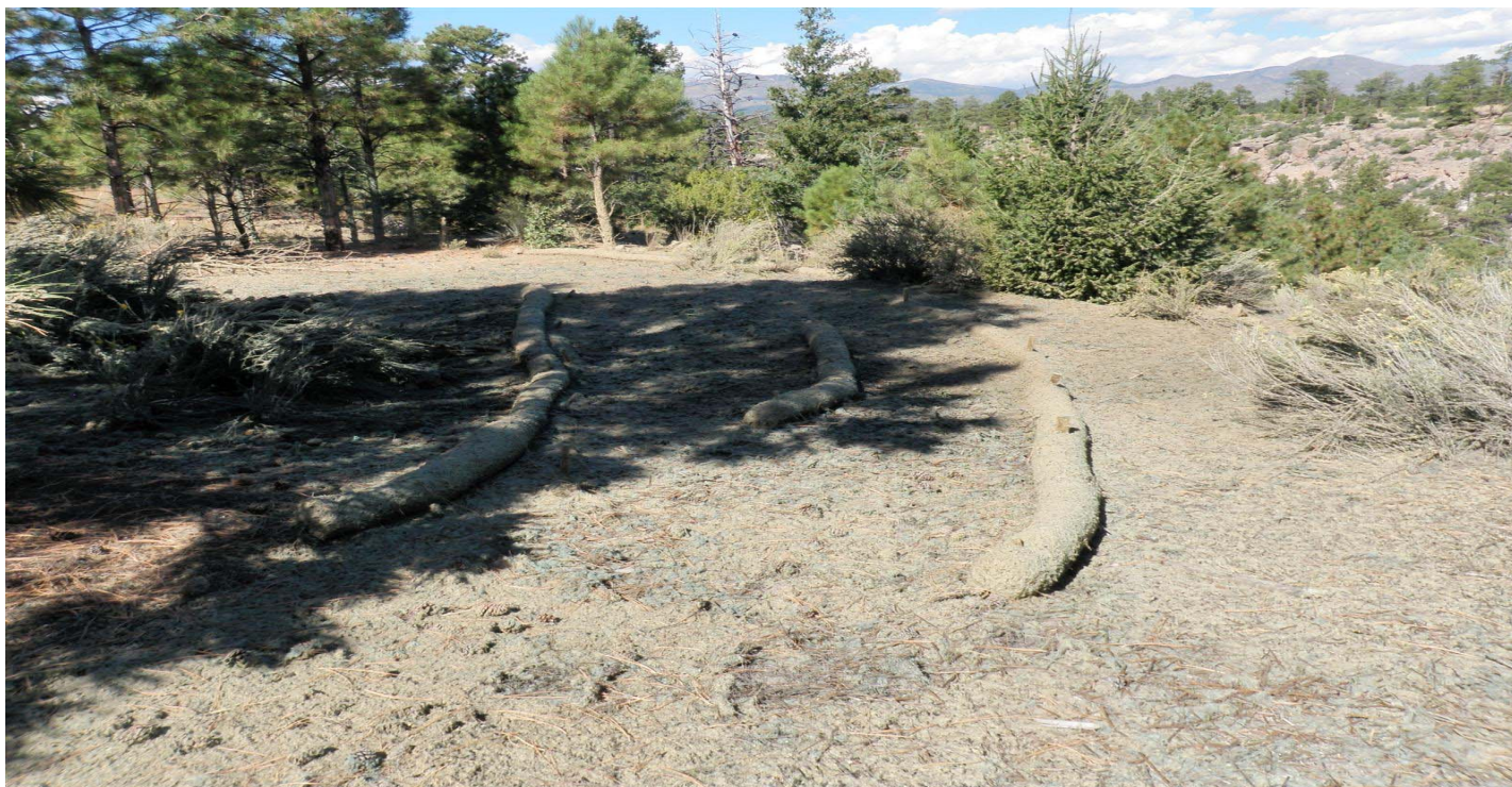
Photo 10872-06r.JPG (taken 10/07/10) H00403060011 : Berms - Straw Wattles; H00403060012 : Berms - Straw Wattles; H00403060013 : Berms - Straw Wattles; H00403060024 : Berms - Straw Wattles.
