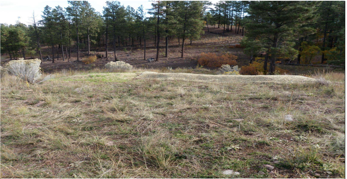
Photo 11465-5r.JPG (taken 10/22/10) V008A03010016 : Berms - Earthen Berm.
