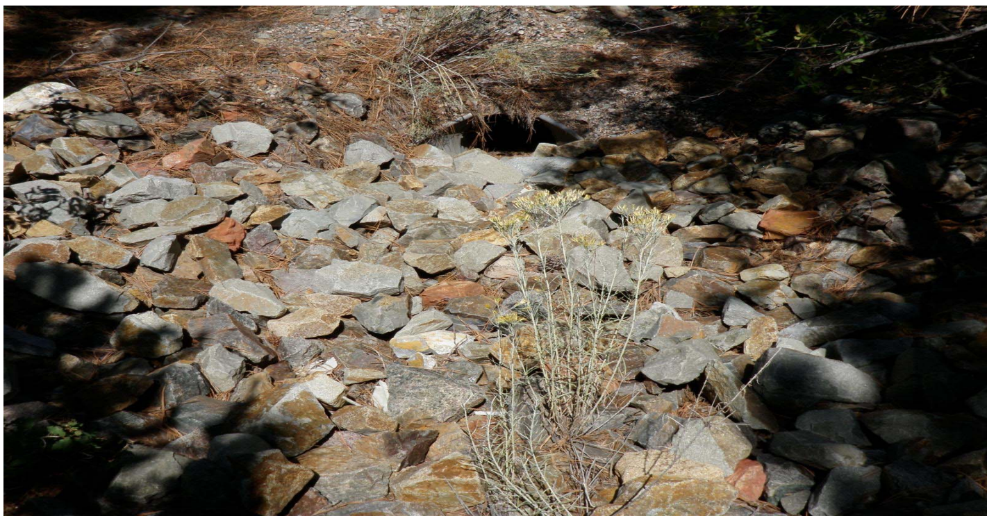
Photo 10873-12r.JPG (taken 10/07/10) H00304060004 : Channel/Swale - Rip Rap.
