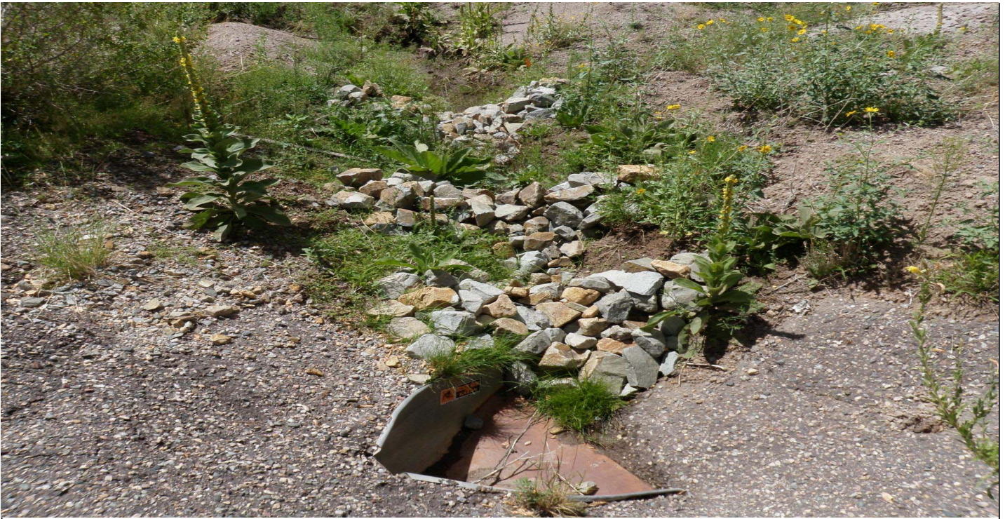
Photo 8503-3r.JPG (taken 08/19/10) C00306010013 : Check Dam - Rock Check Dam; C00306010015 : Check Dam - Rock Check Dam; C00306010016 : Check Dam - Rock Check Dam.
