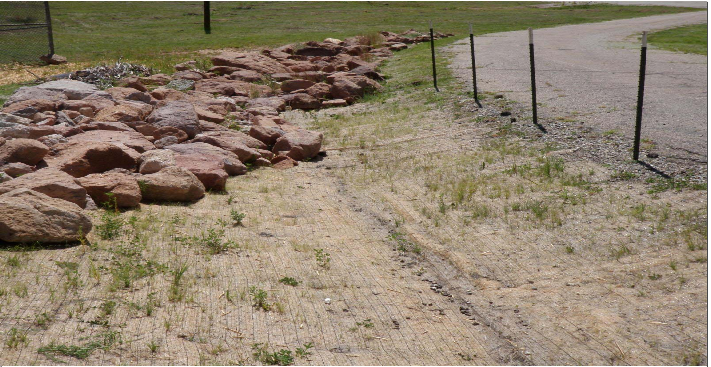
Photo 8524-09r.JPG (taken 08/18/10) V00904060007 : Channel/Swale - Rip Rap.
