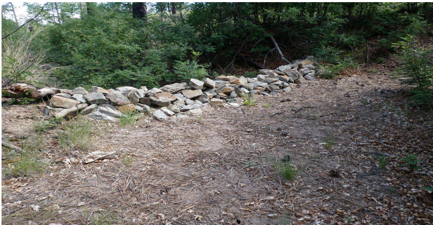
Photo 7802-3r.JPG (taken 08/17/10) W00801010005 : Seed and Mulch - Seed and Wood Mulch; W00806010001 : Check Dam - Rock Check Dam.
