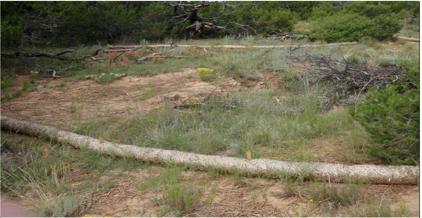
Photo 8519-6.JPG (taken 08/04/10) W01903060025 : Berms - Straw Wattles; W01903060026 : Berms - Straw Wattles.
