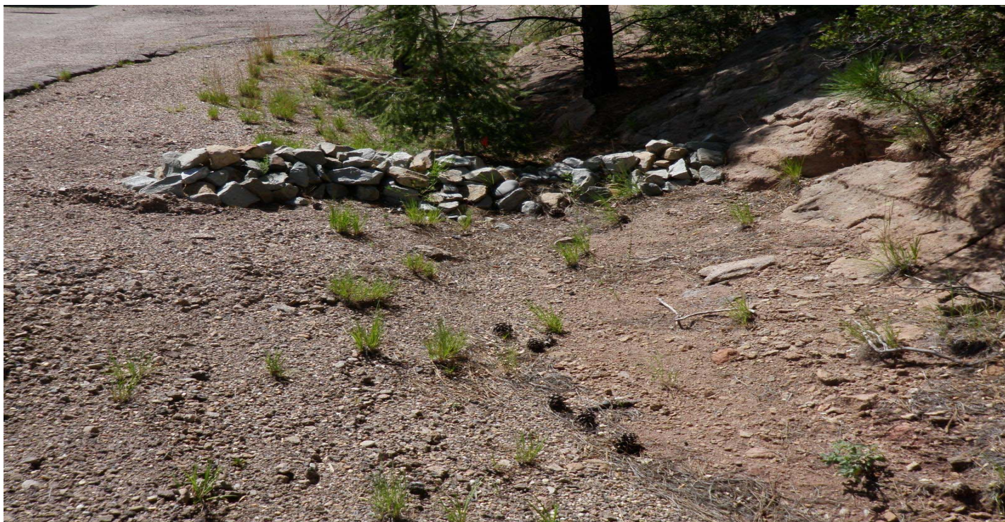
Photo 7806-2r.JPG (taken 08/17/10) W01106010005 : Check Dam - Rock Check Dam.
