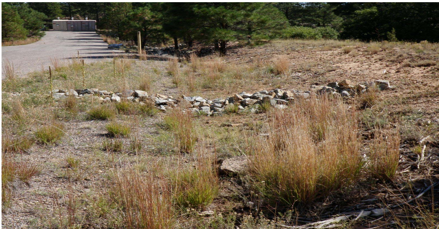
Photo 10873-07r.JPG (taken 10/07/10) H00306010012 : Check Dam - Rock Check Dam.
