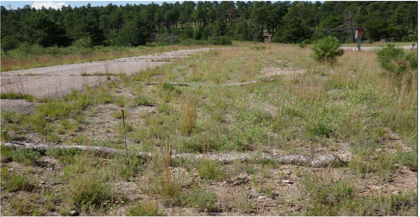
Photo 8525-07r.JPG (taken 08/18/10) V009A03060007 : Berms - Straw Wattles; V009A03060008 : Berms - Straw Wattles; V009A03060009 : Berms - Straw Wattles; V009A03060010 : Berms - Straw Wattles; V009A03060011 : Berms - Straw Wattles.
