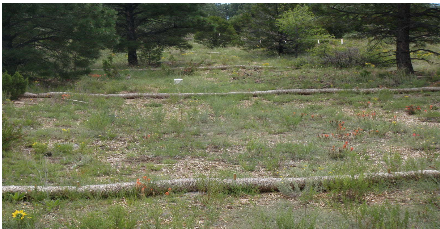
Photo 8519-11.JPG (taken 08/04/10) W01903060015 : Berms - Straw Wattles; W01903060016 : Berms - Straw Wattles; W01903060017 : Berms - Straw Wattles; W01903060018 : Berms - Straw Wattles.
