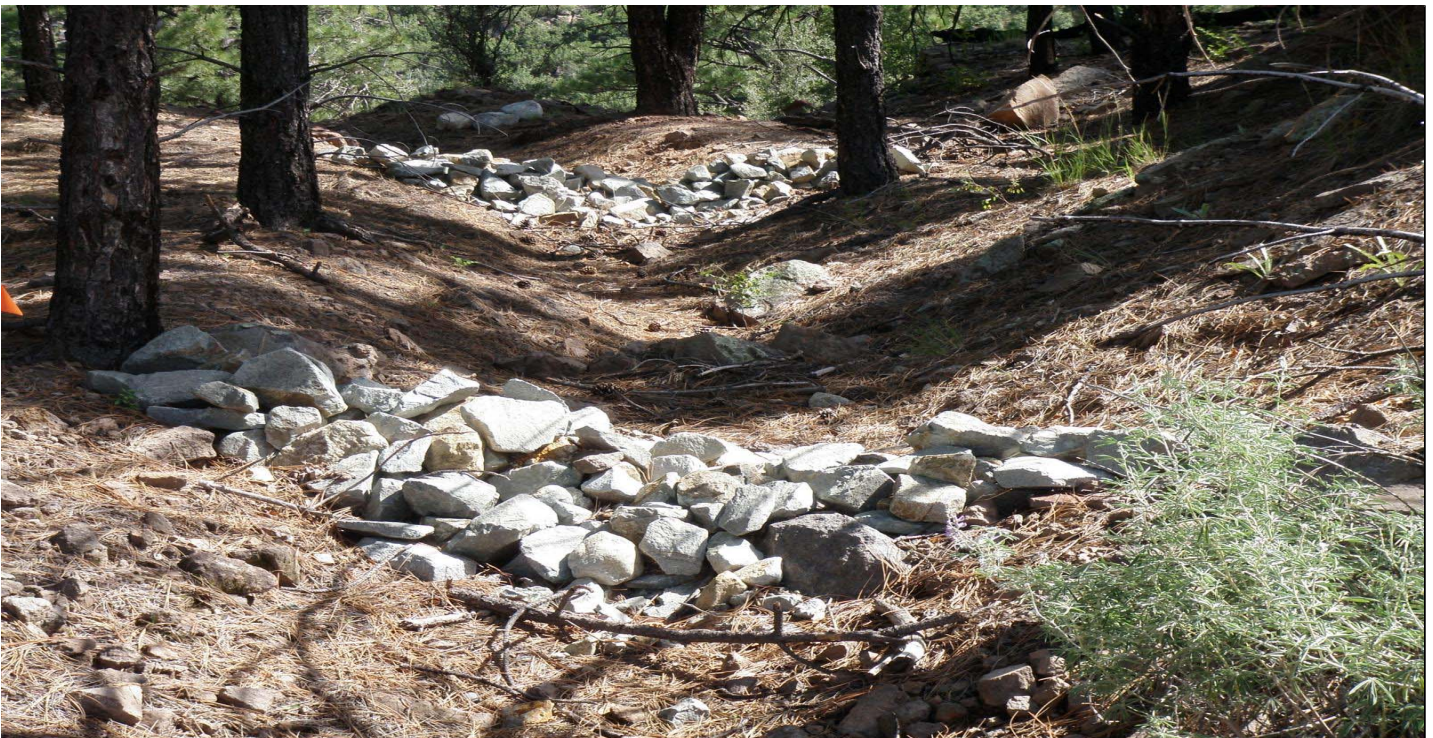
Photo 7801-4r.JPG (taken 08/17/10) W00906010005 : Check Dam - Rock Check Dam; W00906010006 : Check Dam - Rock Check Dam.
