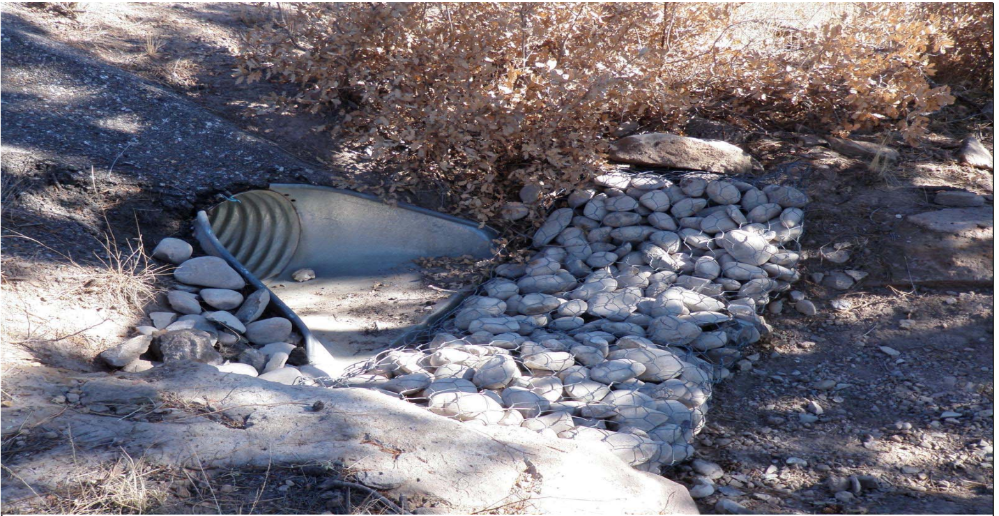
Photo 12126-1r.JPG (taken 12/02/10) E01207020010 : Gabions - Gabion Blanket.
