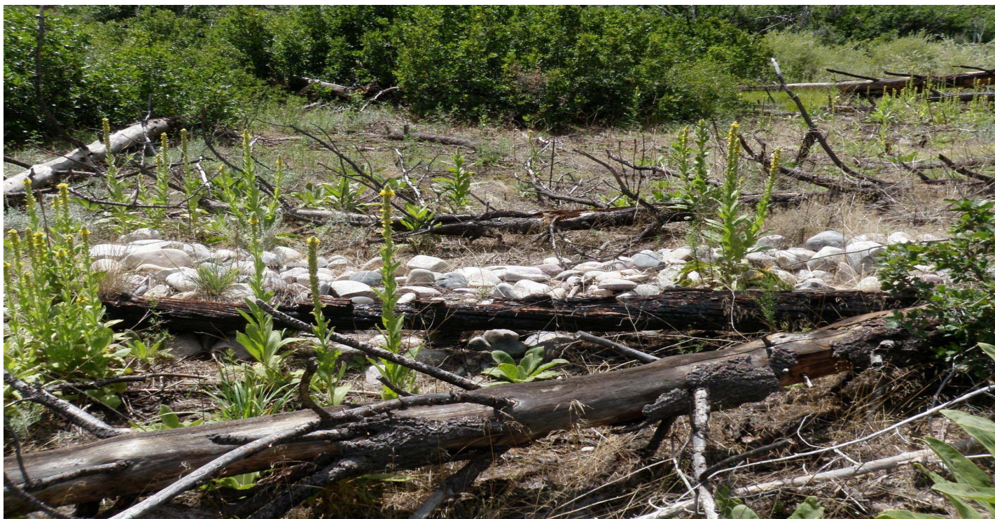
Photo 8503-7r.JPG (taken 08/19/10) C00306010009 : Check Dam - Rock Check Dam.
