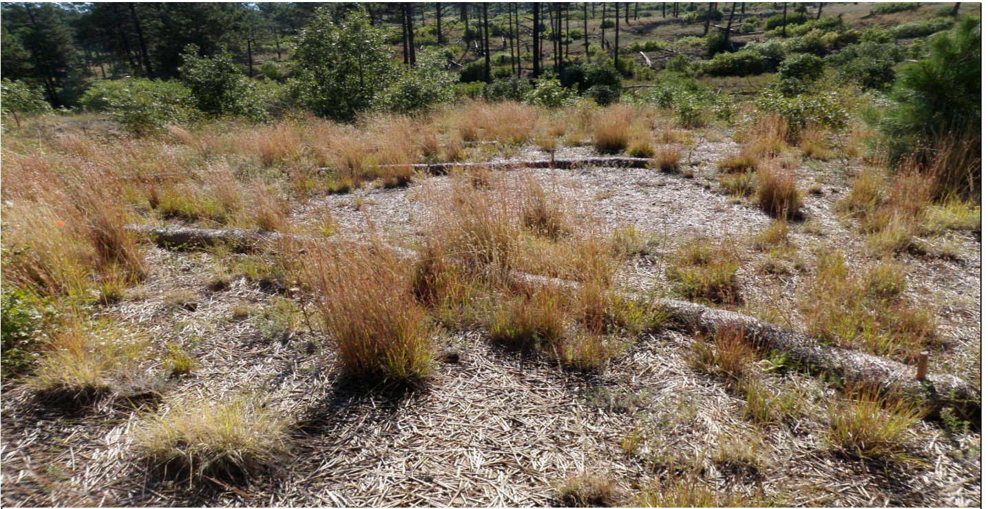
Photo 10878-1r.JPG (taken 10/07/10) W01801010017 : Seed and Mulch - Seed and Wood Mulch; W01803060020 : Berms - Straw Wattles; W01803060021 : Berms - Straw Wattles.
