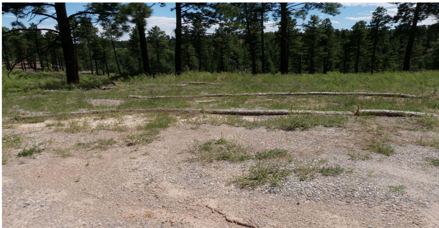
Photo 7507-1r.JPG (taken 08/11/10) J00603060005 : Berms - Straw Wattles; J00603060006 : Berms - Straw Wattles.
