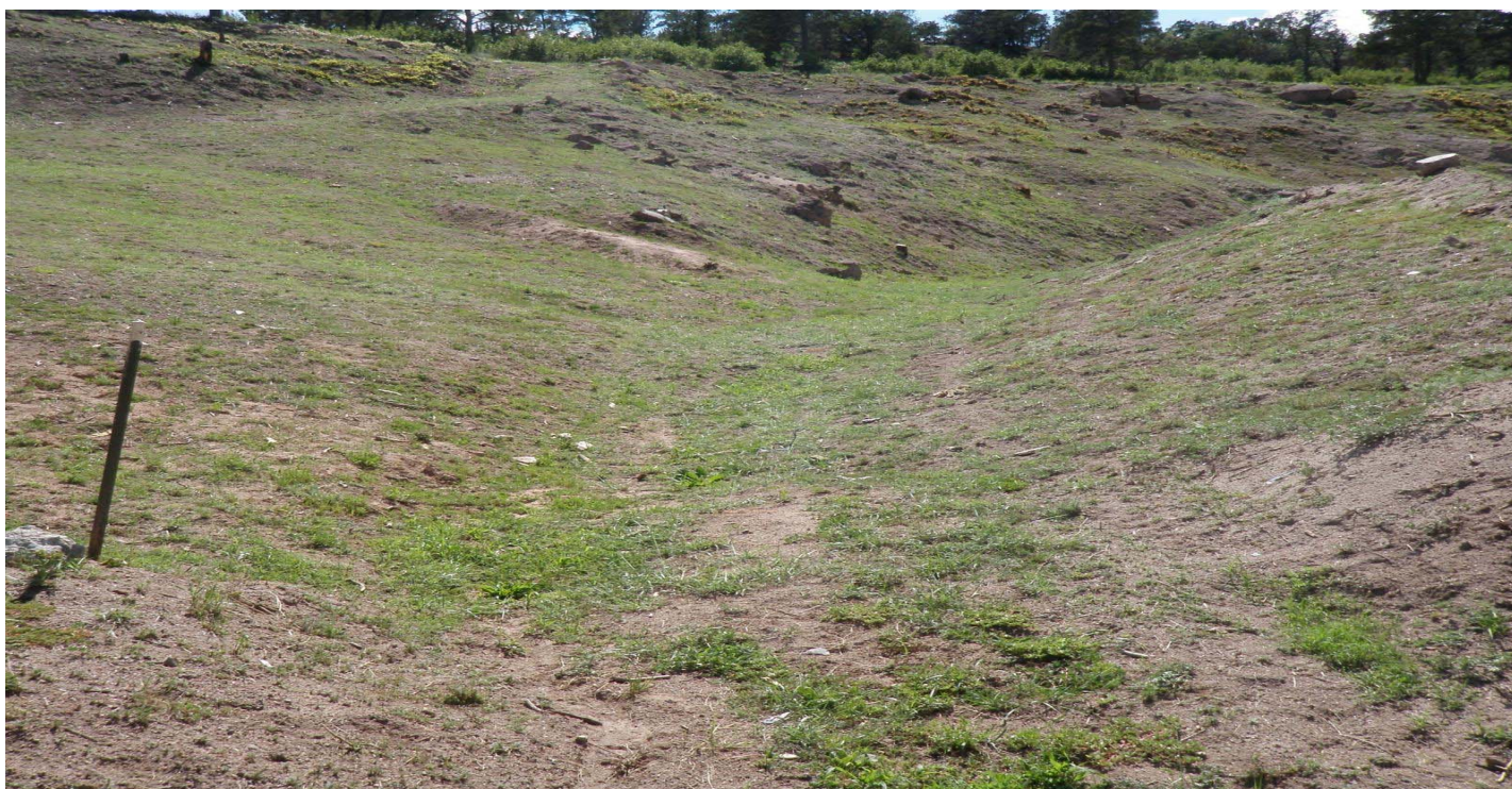
Photo 8526-2r.JPG (taken 08/18/10) F00104010001 : Channel/Swale - Earthen Channel/Swale.
