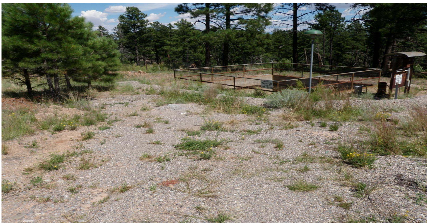
Photo 8530-5r.JPG (taken 08/18/10) W01203020009 : Berms - Base Course Berm.
