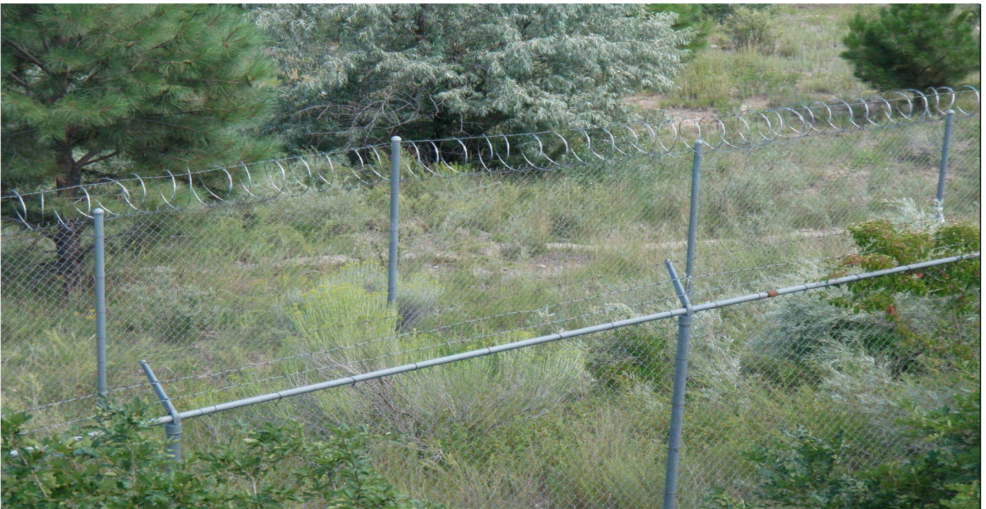
Photo 7803-2r.JPG (taken 08/17/10) W00503060005 : Berms - Straw Wattles.
