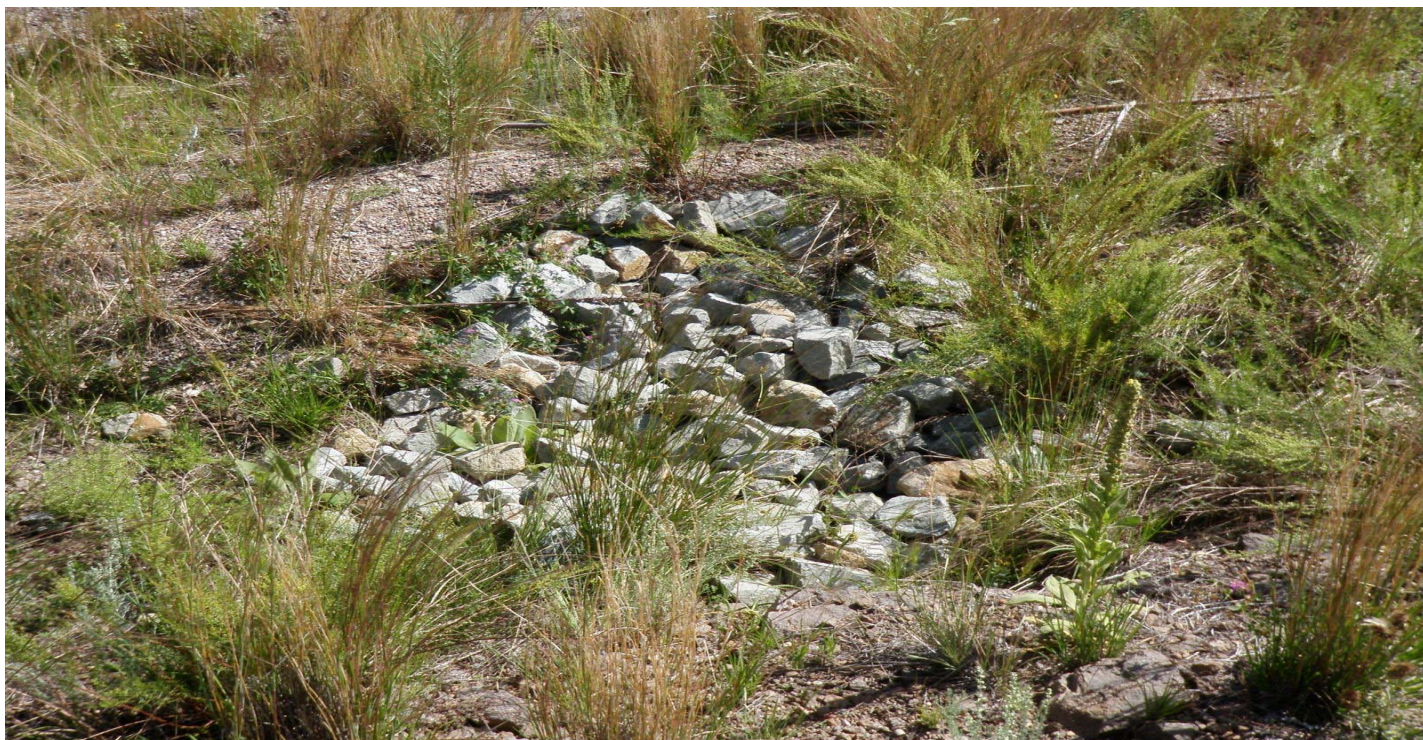
Photo 7801-1r.JPG (taken 08/17/10) W00904060003 : Channel/Swale - Rip Rap.
