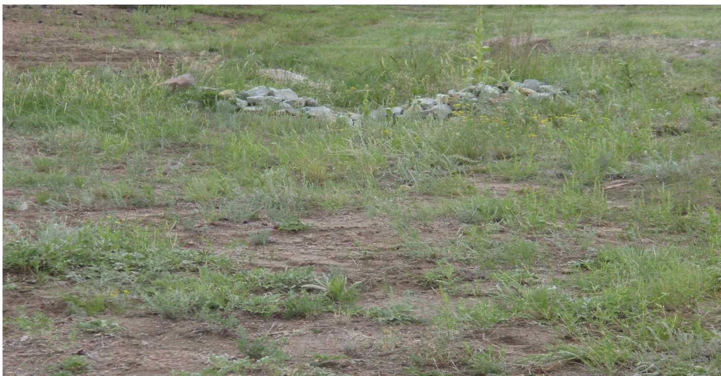
Photo 8531-04r.JPG (taken 08/23/10) W00606010012 : Check Dam - Rock Check Dam.
