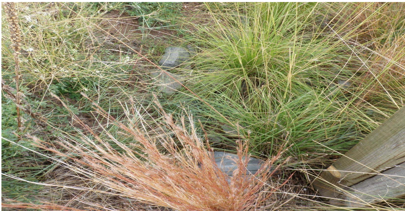
Photo 11025-5r.JPG (taken 10/21/10) C00404060006 : Channel/Swale - Rip Rap.
