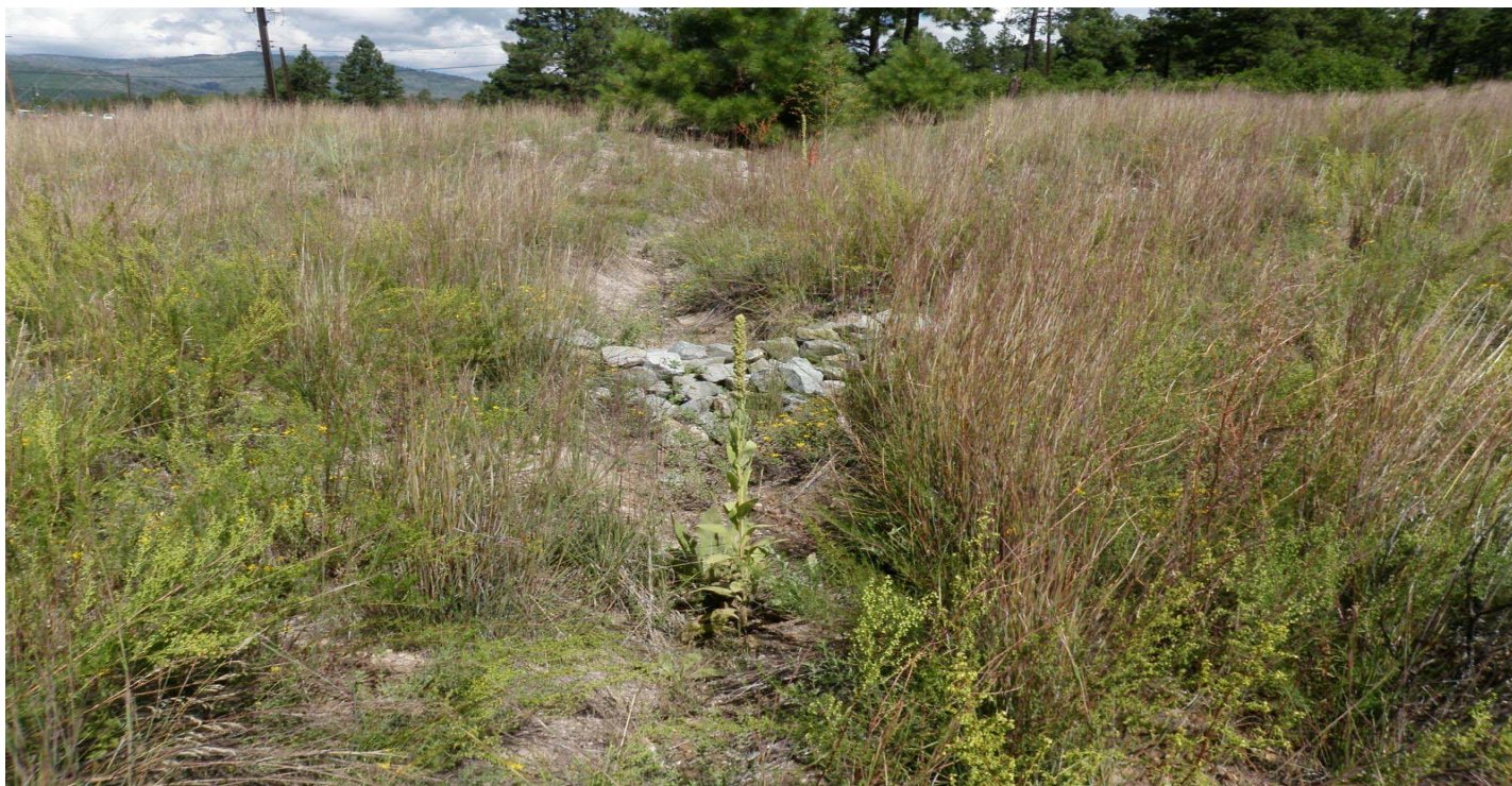
Photo 8525-11r.JPG (taken 08/18/10) V009A06010006 : Check Dam - Rock Check Dam.
