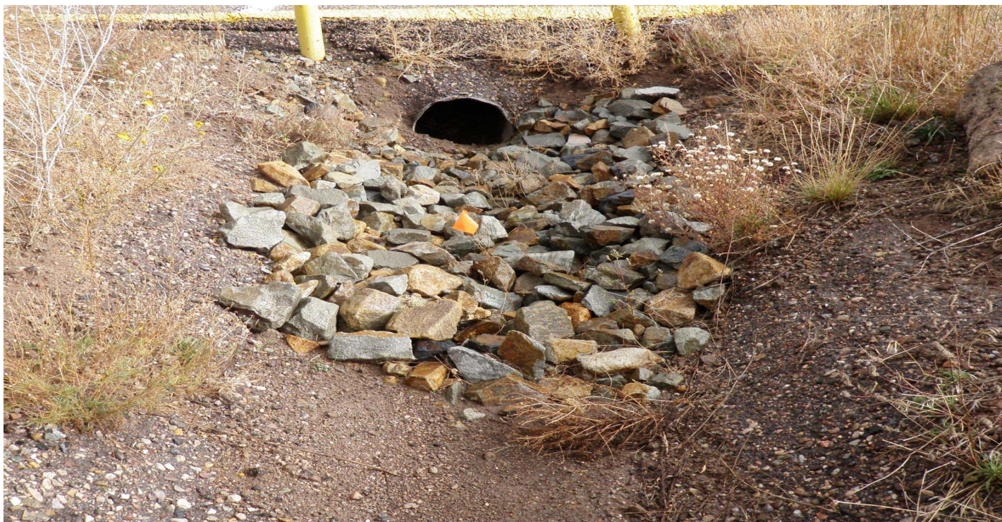
Photo 11025-9r.JPG (taken 10/21/10) C00404060009 : Channel/Swale - Rip Rap.
