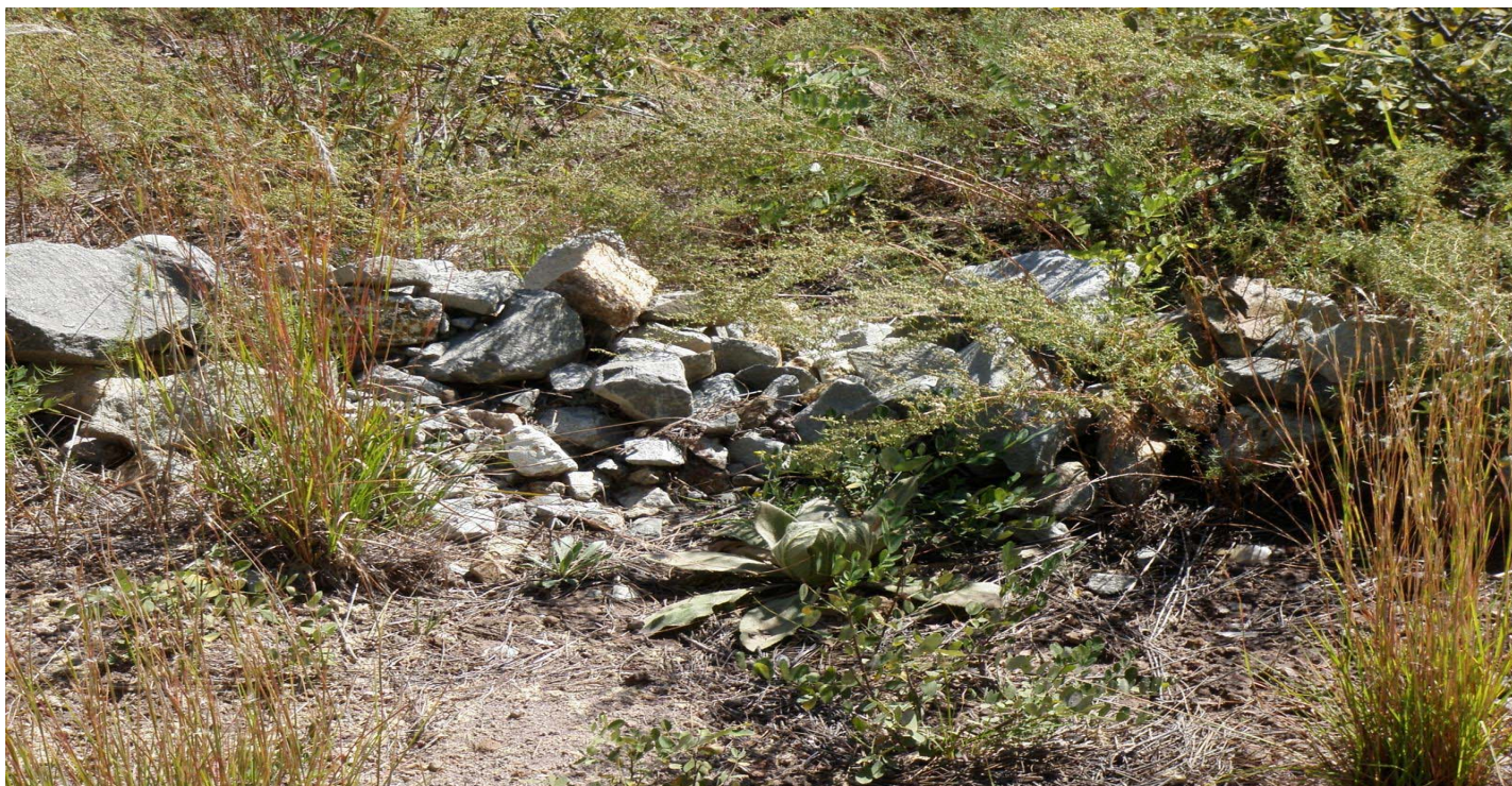
Photo 10865-2r.JPG (taken 10/07/10) J01406010010 : Check Dam - Rock Check Dam.
