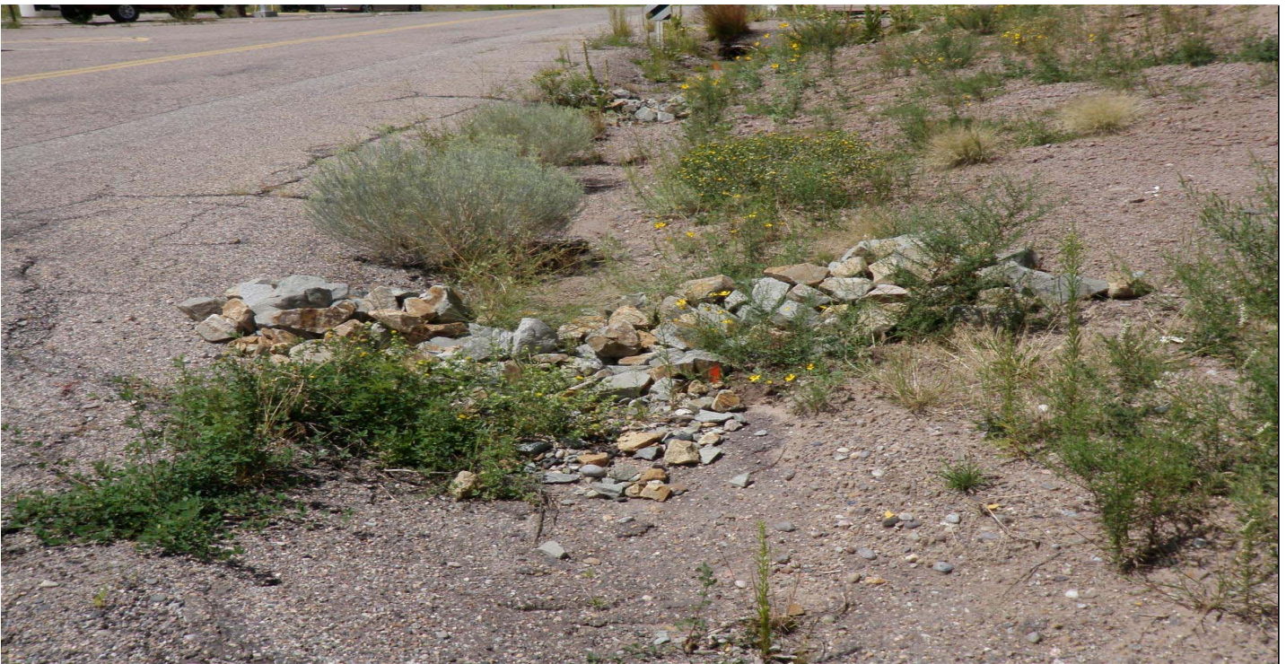
Photo 8503-2r.JPG (taken 08/19/10) C00306010017 : Check Dam - Rock Check Dam; C00306010018 : Check Dam - Rock Check Dam.
