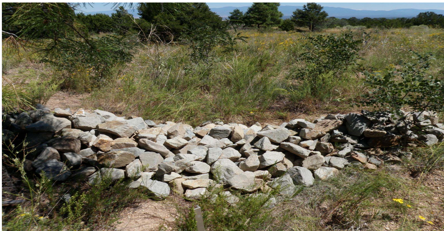
Photo 8514-1r.JPG (taken 08/20/10) W02202010002 : Established Vegetation - Permanent Vegetation Grasses and Shrubs; W02206010003 : Check Dam - Rock Check Dam.
