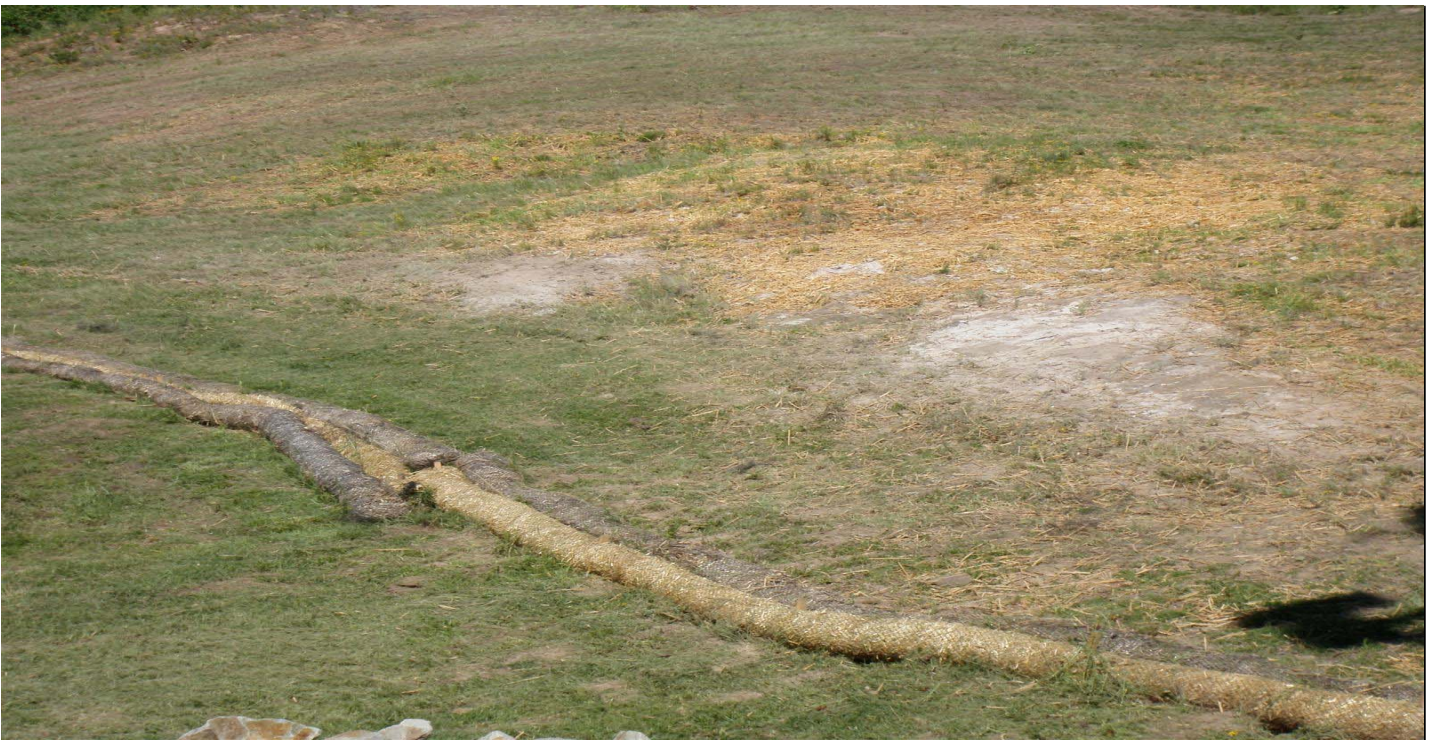
Photo 8524-04r.JPG (taken 08/18/10) V00901010004 : Seed and Mulch - Seed and Wood Mulch; V00903060019 : Berms - Straw Wattles.
