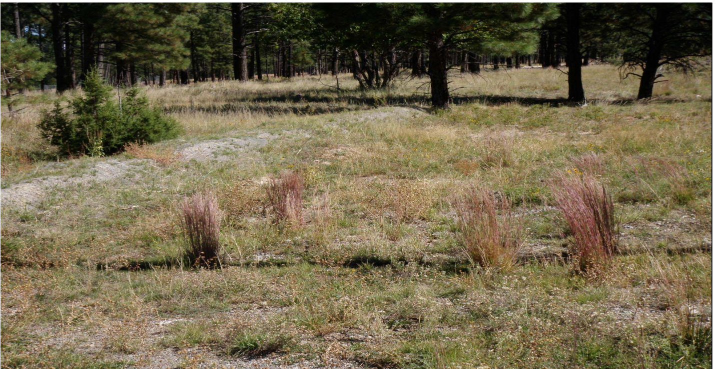
Photo 10867-2r.JPG (taken 10/08/10) E00501060009 : Seed and Mulch - Erosion Control Blanket; E00503010007 : Berms - Earthen Berm.
