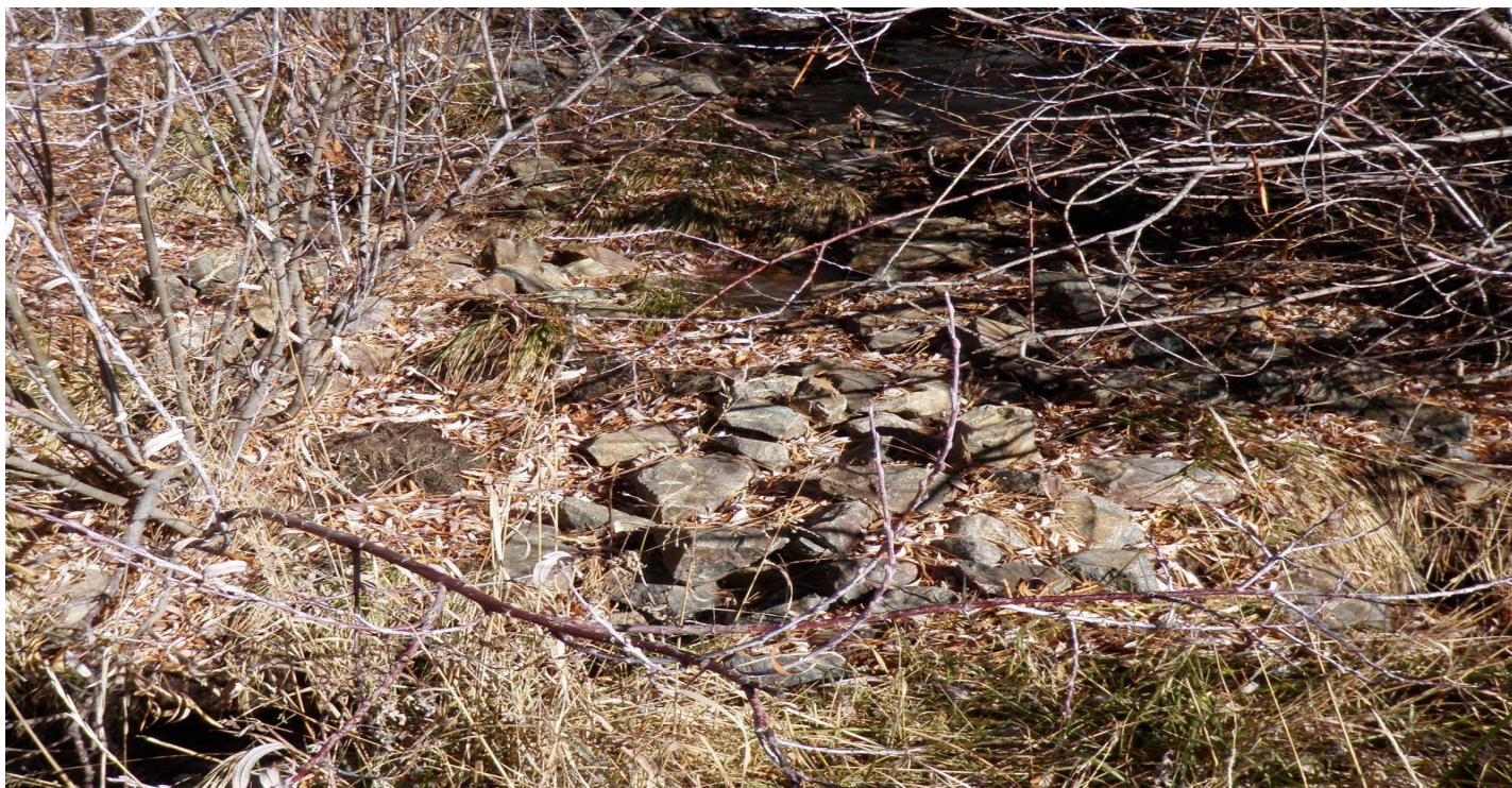
Photo 12126-3r.JPG (taken 12/02/10) E01204060001 : Channel/Swale - Rip Rap.
