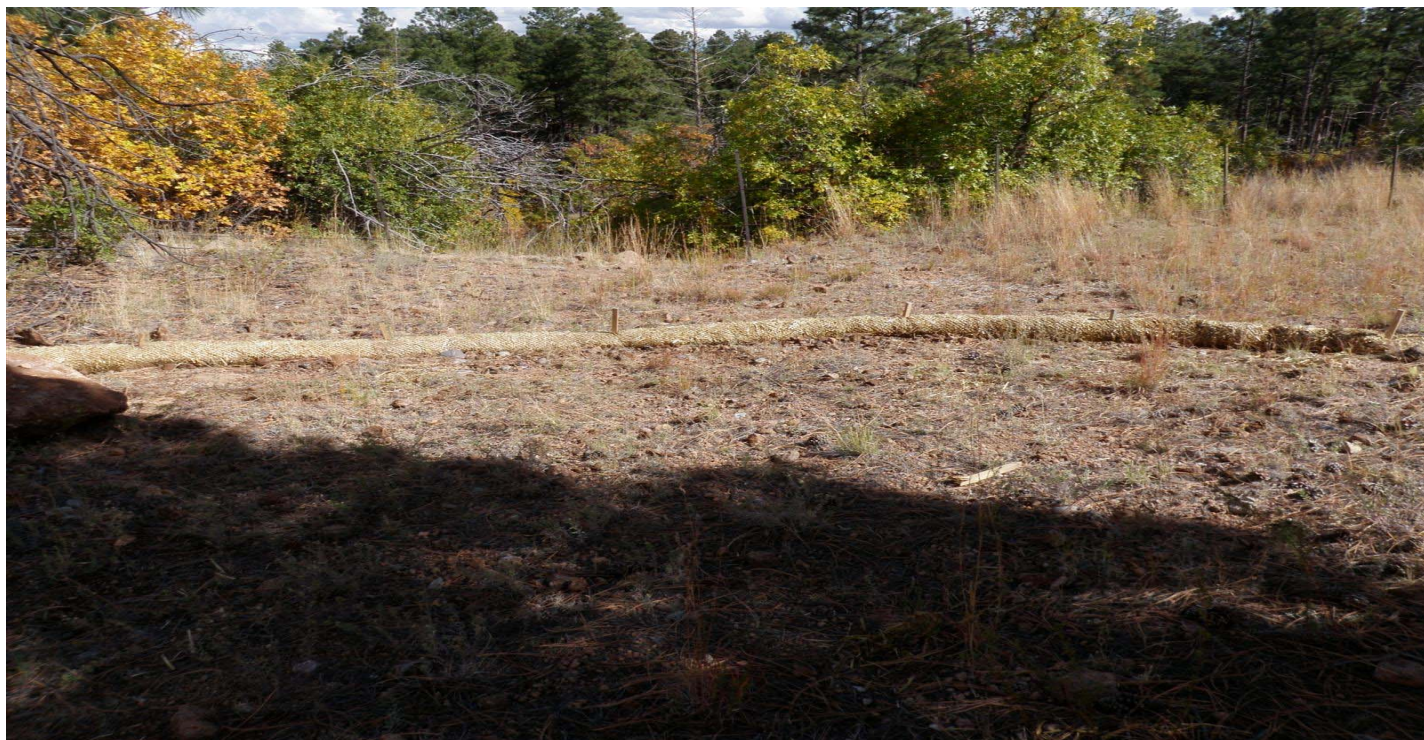
Photo 11024-1r.JPG (taken 10/21/10) W01203060010 : Berms - Straw Wattles.
