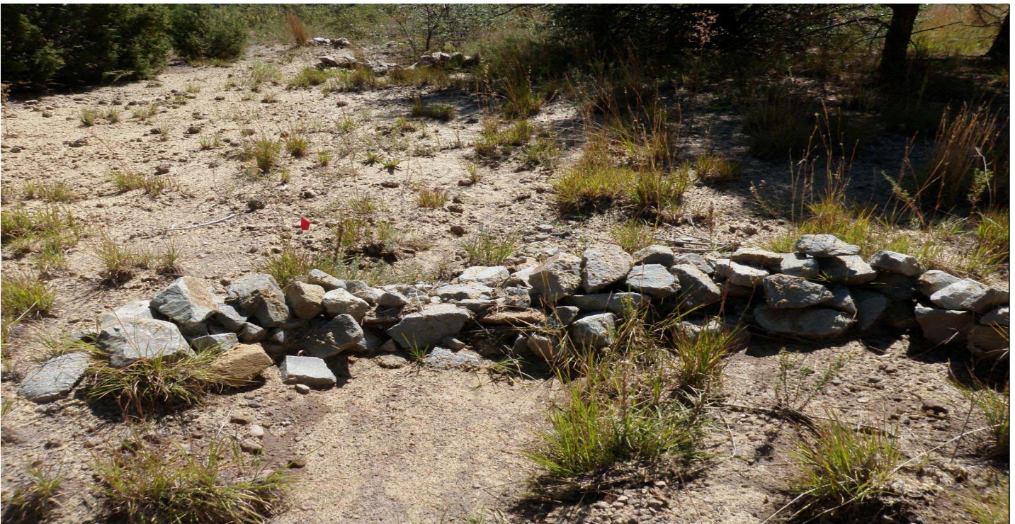
Photo 10864-6r.JPG (taken 10/07/10) J01306010006 : Check Dam - Rock Check Dam; J01306010007 : Check Dam - Rock Check Dam.
