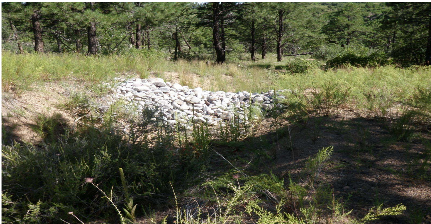
Photo 7805-3r.JPG (taken 08/17/10) W01306010001 : Check Dam - Rock Check Dam.
