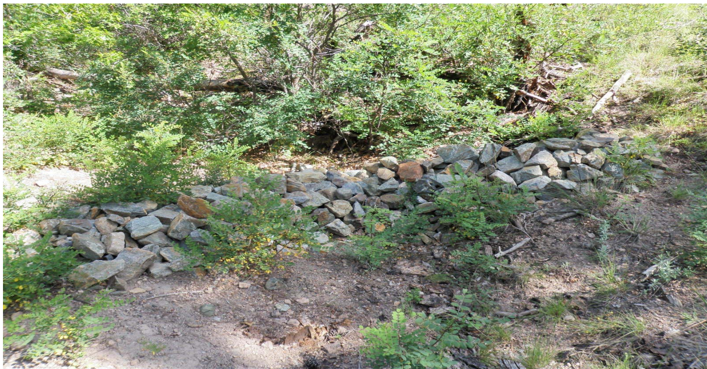
Photo 7802-5r.JPG (taken 08/17/10) W00806010003 : Check Dam - Rock Check Dam.
