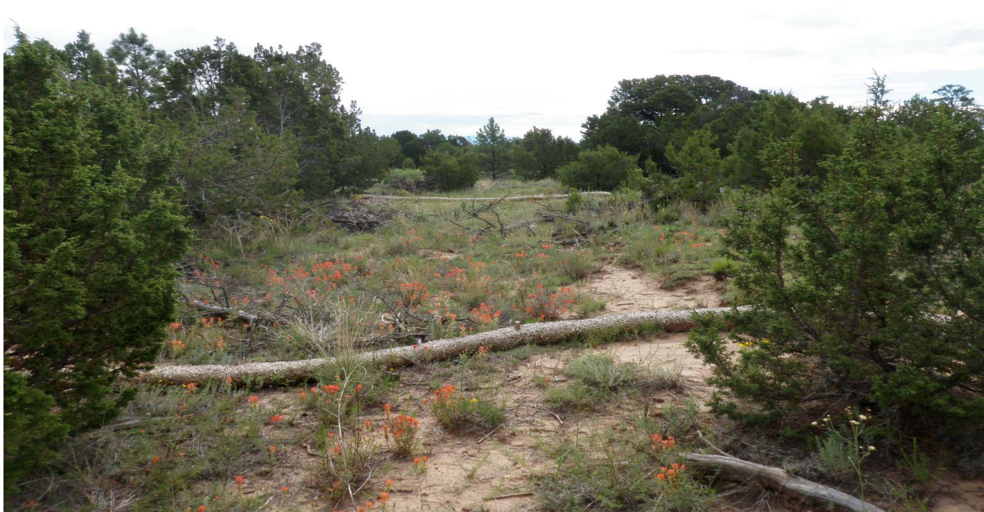
Photo 8519-2.JPG (taken 08/04/10) W01903060028 : Berms - Straw Wattles; W01903060036 : Berms - Straw Wattles.
