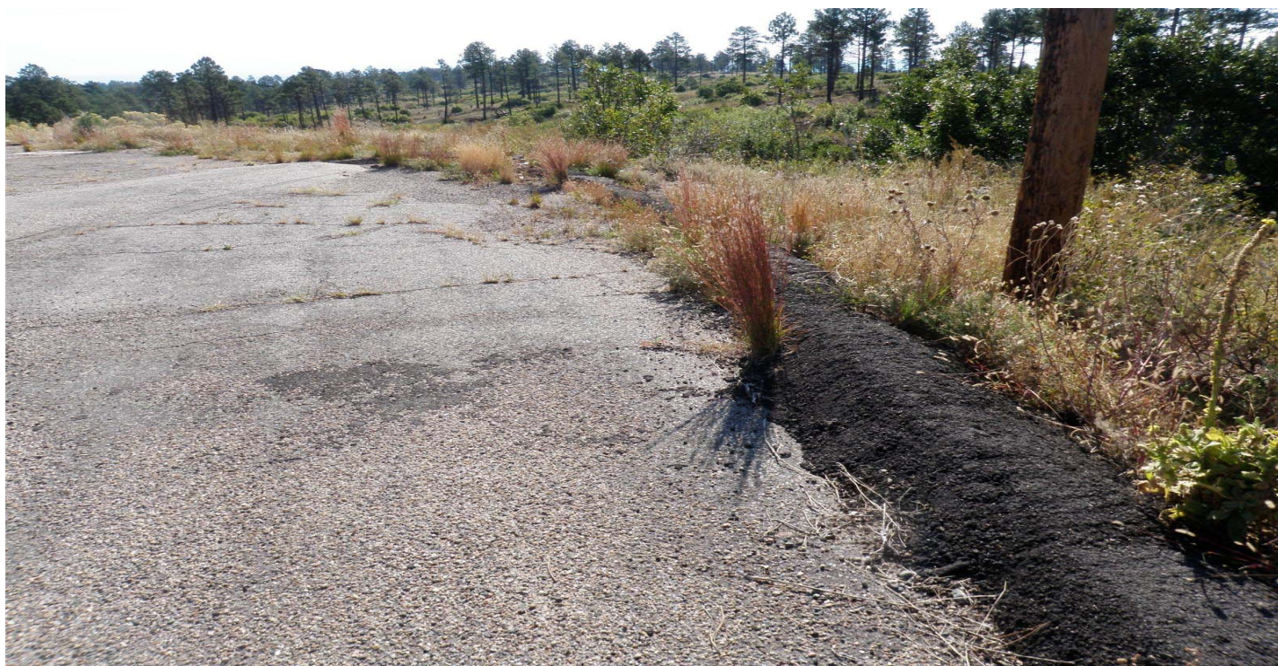
Photo 10878-8r.JPG (taken 10/07/10) W01803040010 : Berms - Asphalt Berm.
