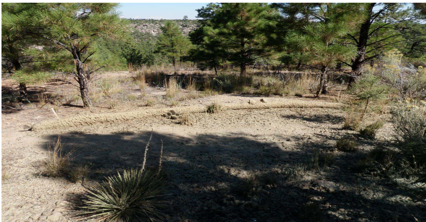
Photo 10872-03r.JPG (taken 10/07/10) H00403060018 : Berms - Straw Wattles.
