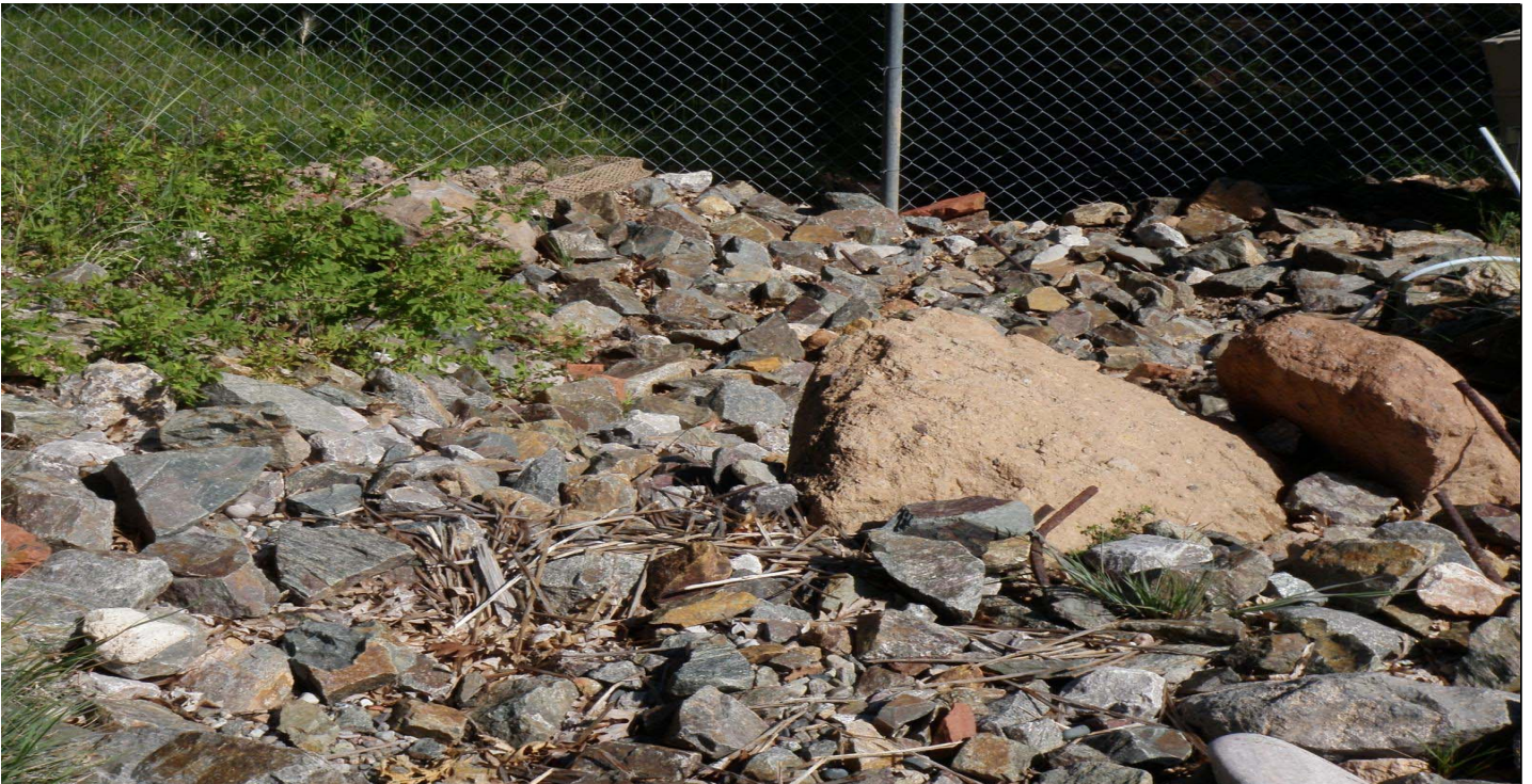
Photo 8520-2r.JPG (taken 08/18/10) V00104060001 : Channel/Swale - Rip Rap.
