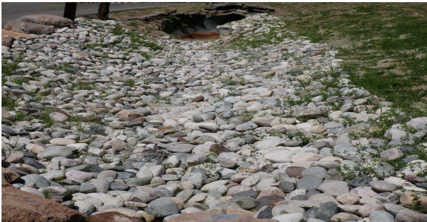
Photo 8524-07r.JPG (taken 08/18/10) V00904060009 : Channel/Swale - Rip Rap.
