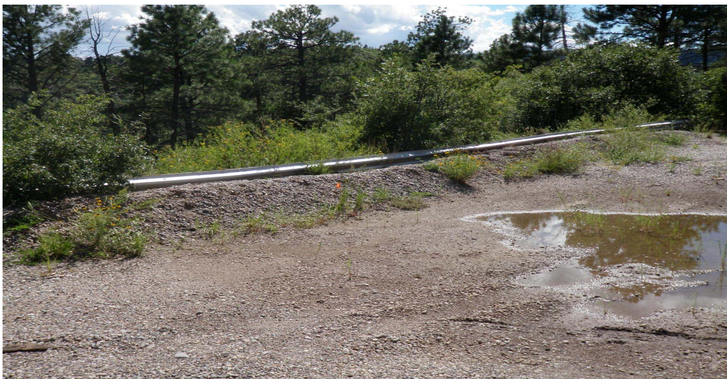
Photo 7806-3r.JPG (taken 08/17/10) W01103020001 : Berms - Base Course Berm.
