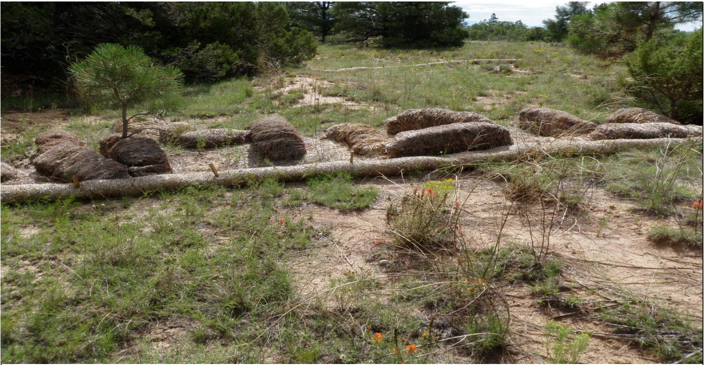
Photo 8519-14.JPG (taken 08/04/10) W01903060010 : Berms - Straw Wattles.
