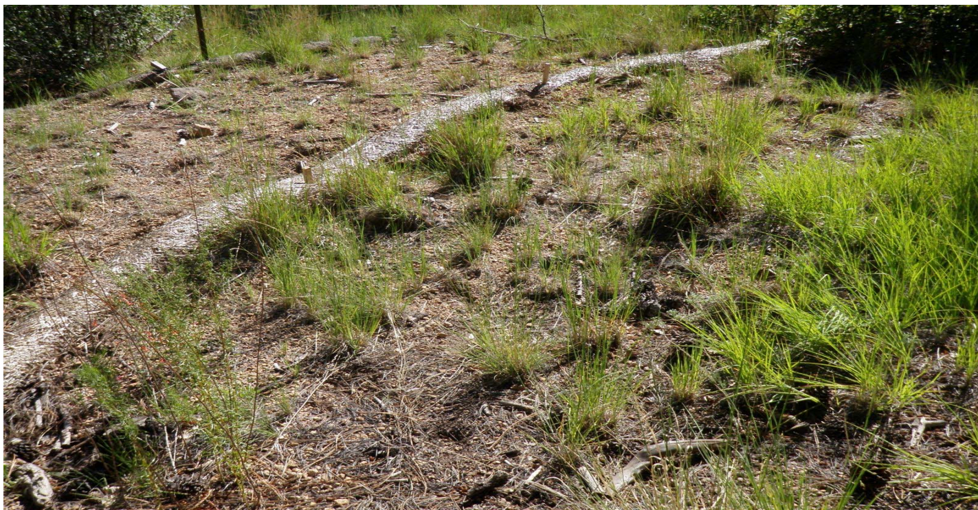
Photo 7805-5r.JPG (taken 08/17/10) W01303060006 : Berms - Straw Wattles.
