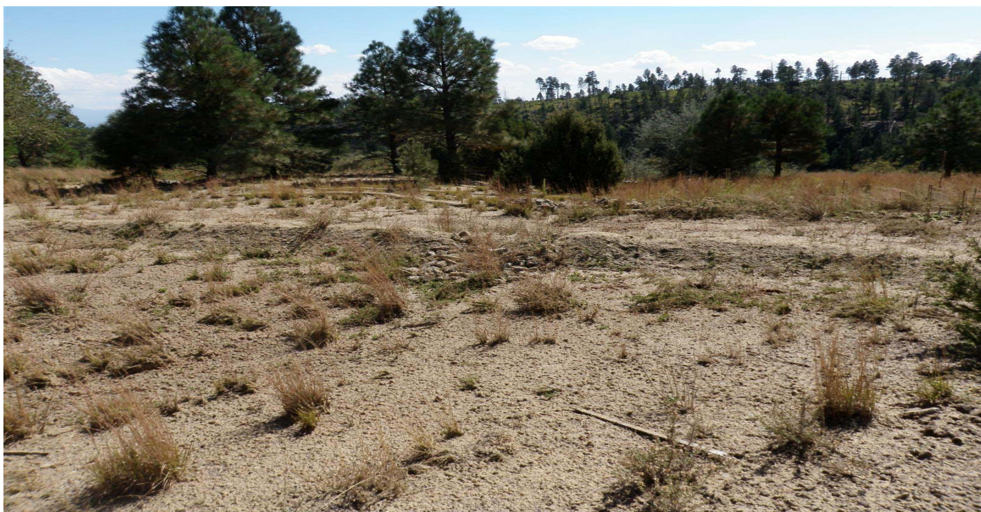
Photo 10864-2r.JPG (taken 10/07/10) J01303010003 : Berms - Earthen Berm.
