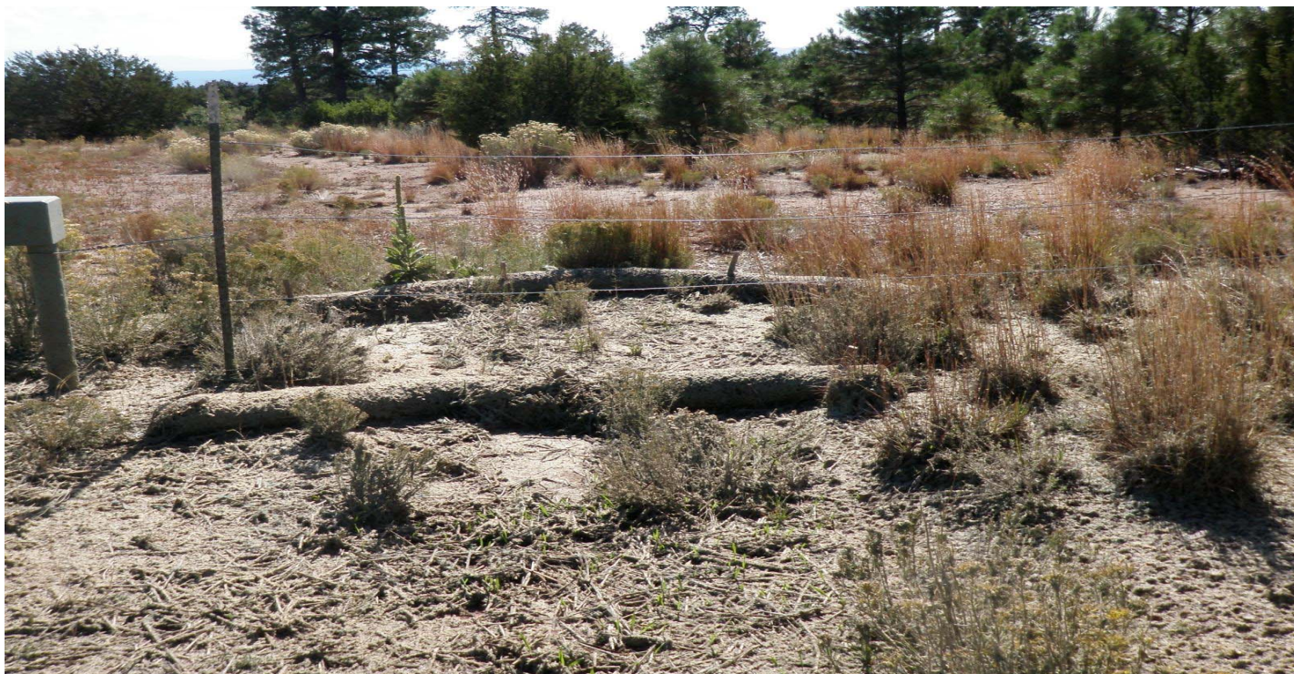
Photo 10872-01r.JPG (taken 10/07/10) H00403060020 : Berms - Straw Wattles; H00403060021 : Berms - Straw Wattles.
