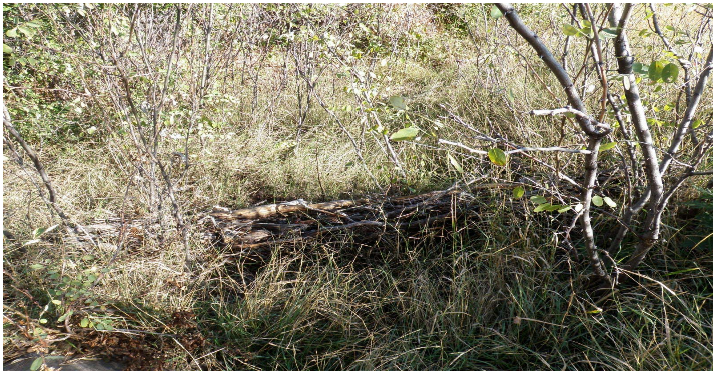
Photo 10875-4r.JPG (taken 10/07/10) W01506030004 : Check Dam - Juniper Bales.
