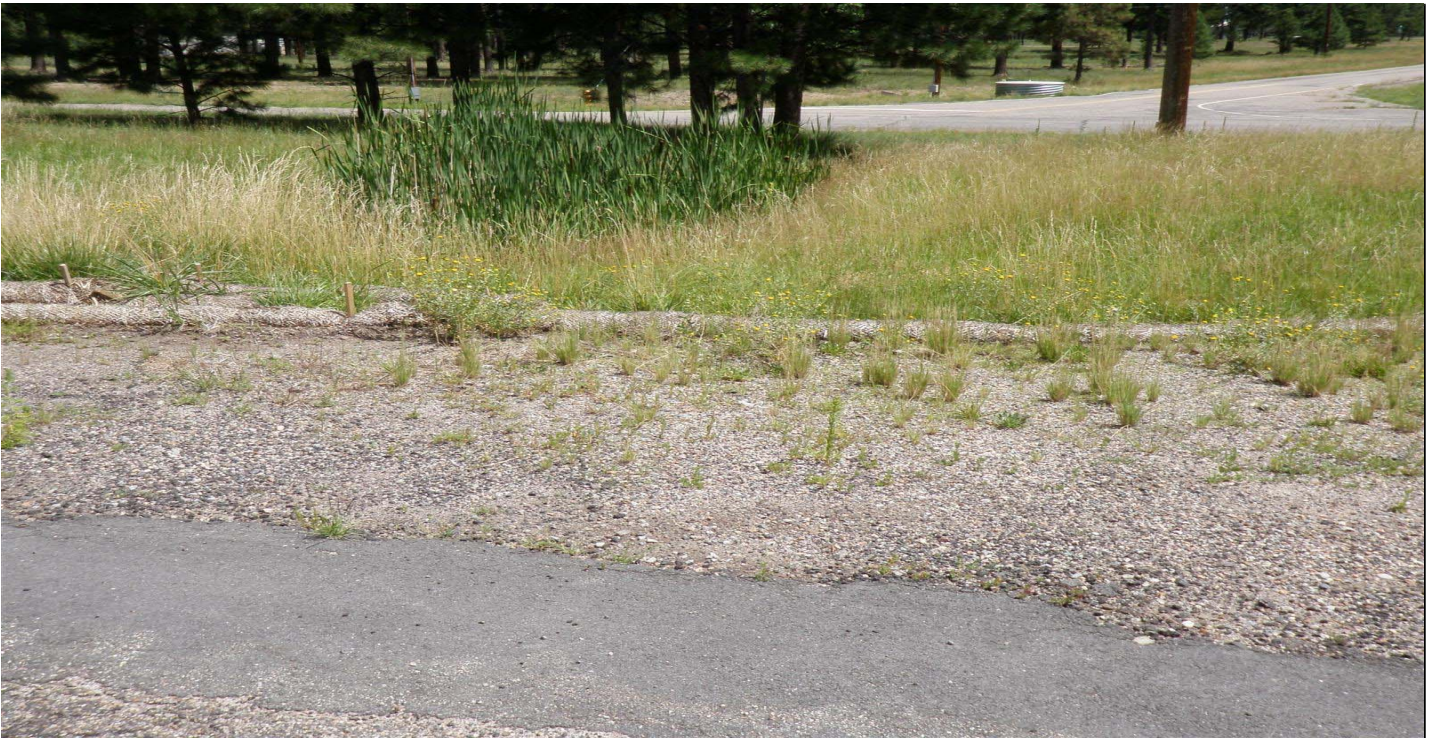
Photo 7800-7r.JPG (taken 08/17/10) W00203060004 : Berms - Straw Wattles; W00203060005 : Berms - Straw Wattles.
