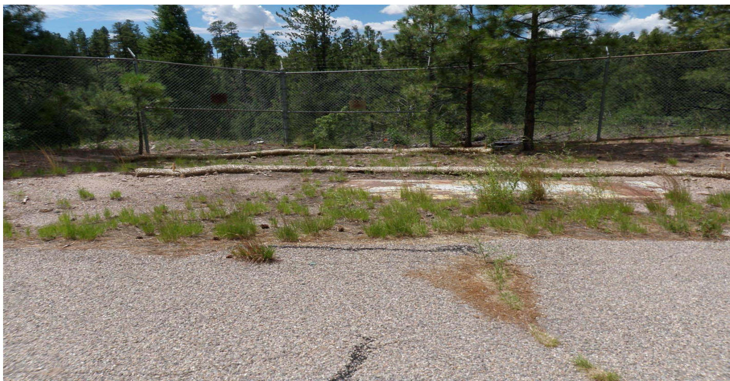
Photo 7517-1r.JPG (taken 08/12/10) E00903060006 : Berms - Straw Wattles; E00903060007 : Berms - Straw Wattles.
