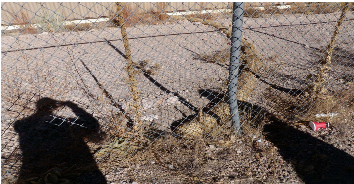
Photo 12126-6r.JPG (taken 12/02/10) E01203060007 : Berms - Straw Wattles.
