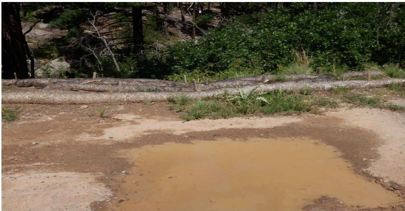
Photo 8527-6r.JPG (taken 08/18/10) V00703060008 : Berms - Straw Wattles.
