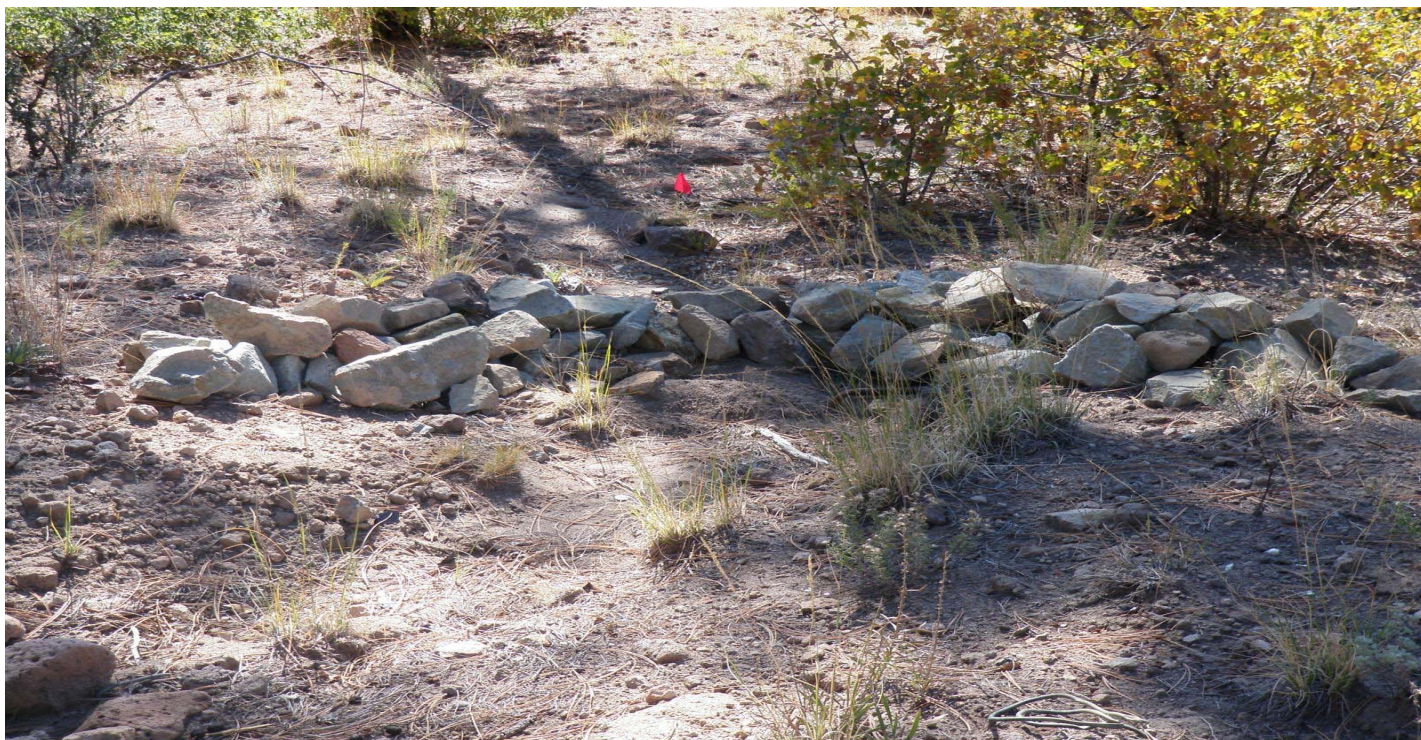
Photo 11459-4r.JPG (taken 10/26/10) J01406010006 : Check Dam - Rock Check Dam.
