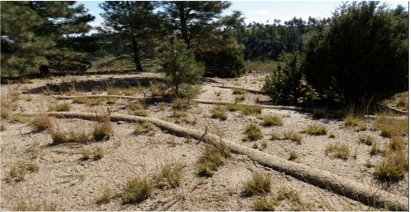
Photo 10864-5r.JPG (taken 10/07/10) J01303060012 : Berms - Straw Wattles; J01303060013 : Berms - Straw Wattles; J01303060014 : Berms - Straw Wattles.
