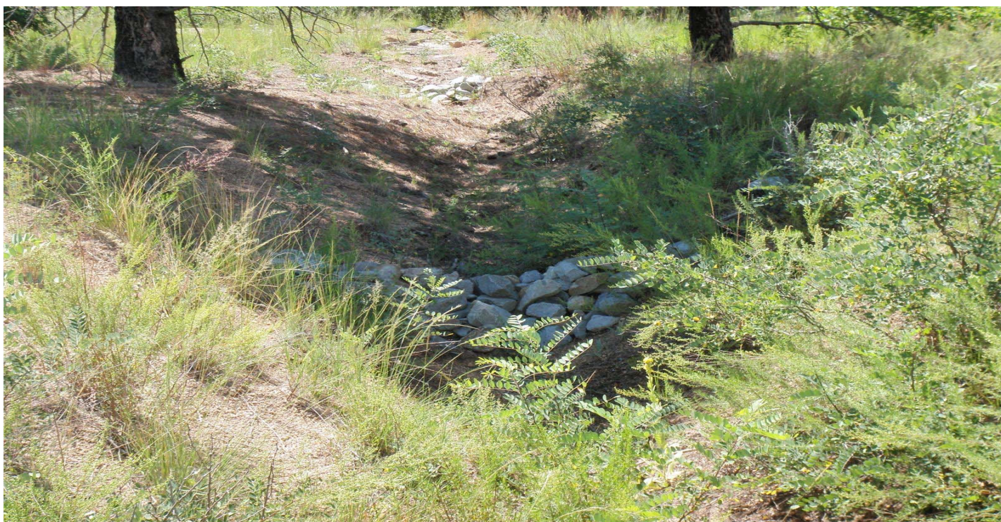
Photo 8525-10r.JPG (taken 08/18/10) V009A06010003 : Check Dam - Rock Check Dam; V009A06010004 : Check Dam - Rock Check Dam.
