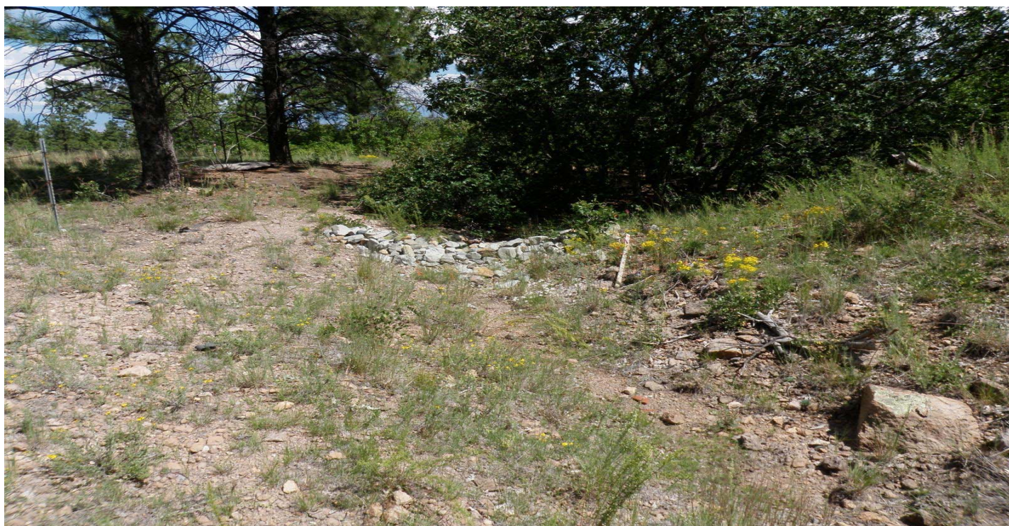
Photo 8530-1r.JPG (taken 08/18/10) W01202010004 : Established Vegetation - Permanent Vegetation Grasses and Shrubs; W01206010008 : Check Dam - Rock Check Dam.
