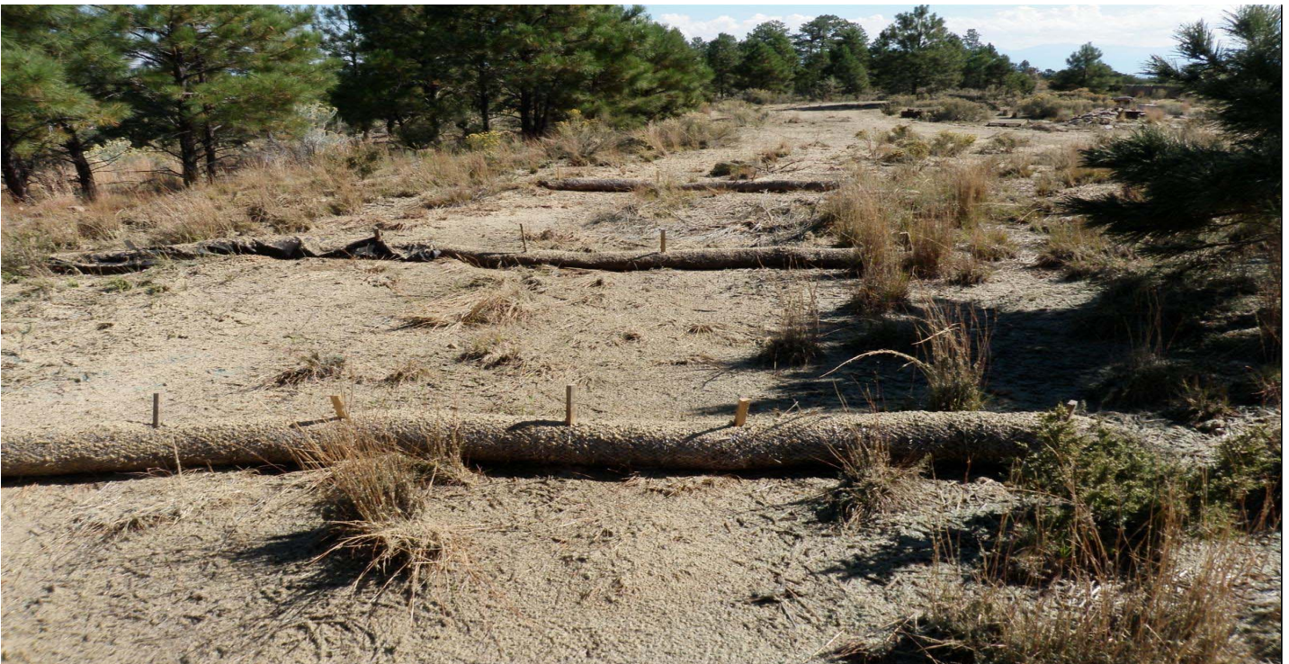
Photo 10872-13r.JPG (taken 10/07/10) H00403060007 : Berms - Straw Wattles; H00403060008 : Berms - Straw Wattles; H00403060009 : Berms - Straw Wattles.
