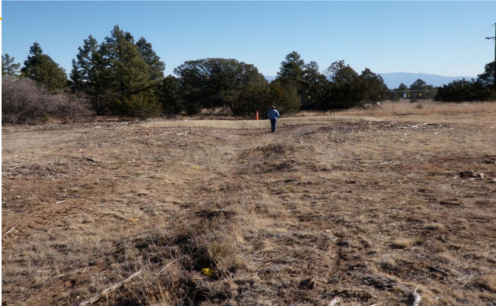
Swale and earthen berms installed in series to capture sheet flow.
