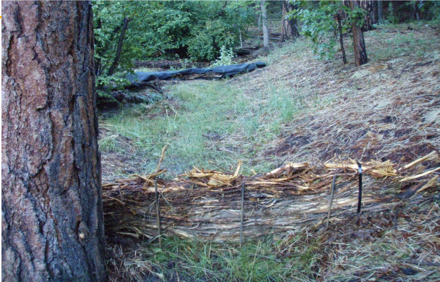
Juniper bales installed in drainage to assist with site stabilization.
