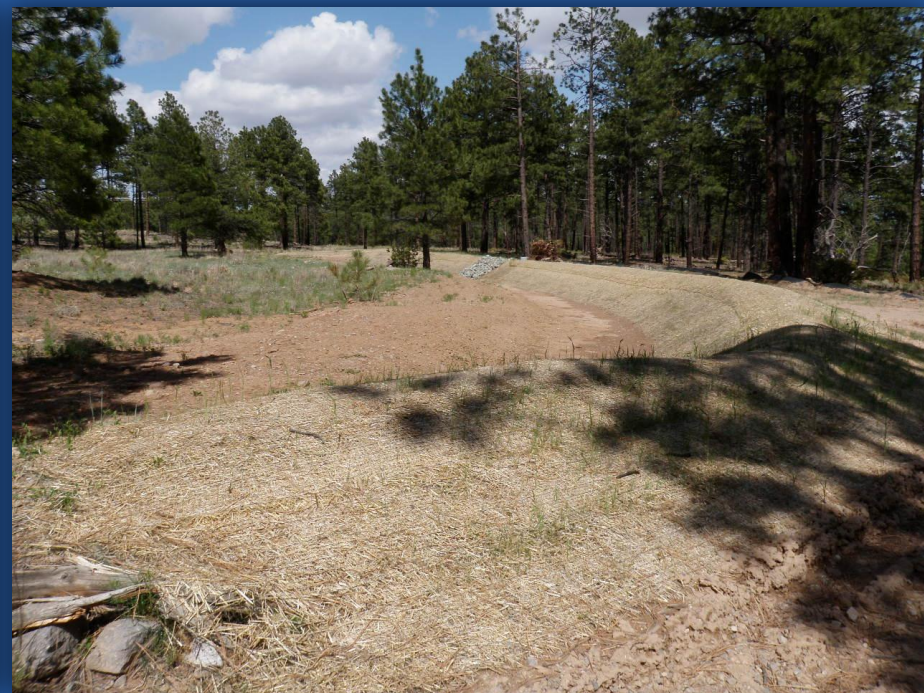
Run-off Control Berm
