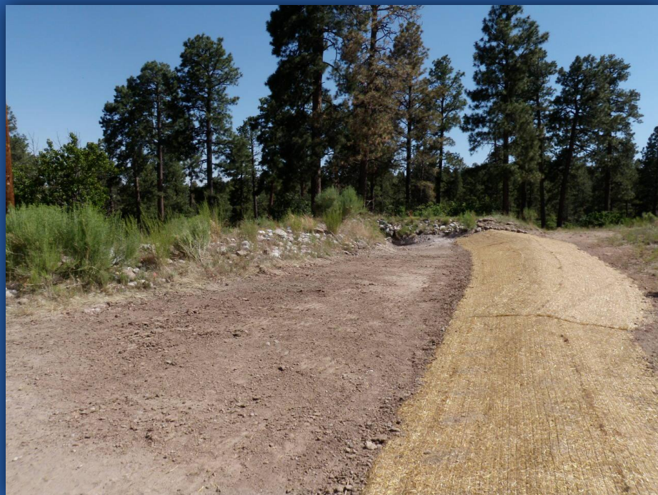
Run-on Control Berm
