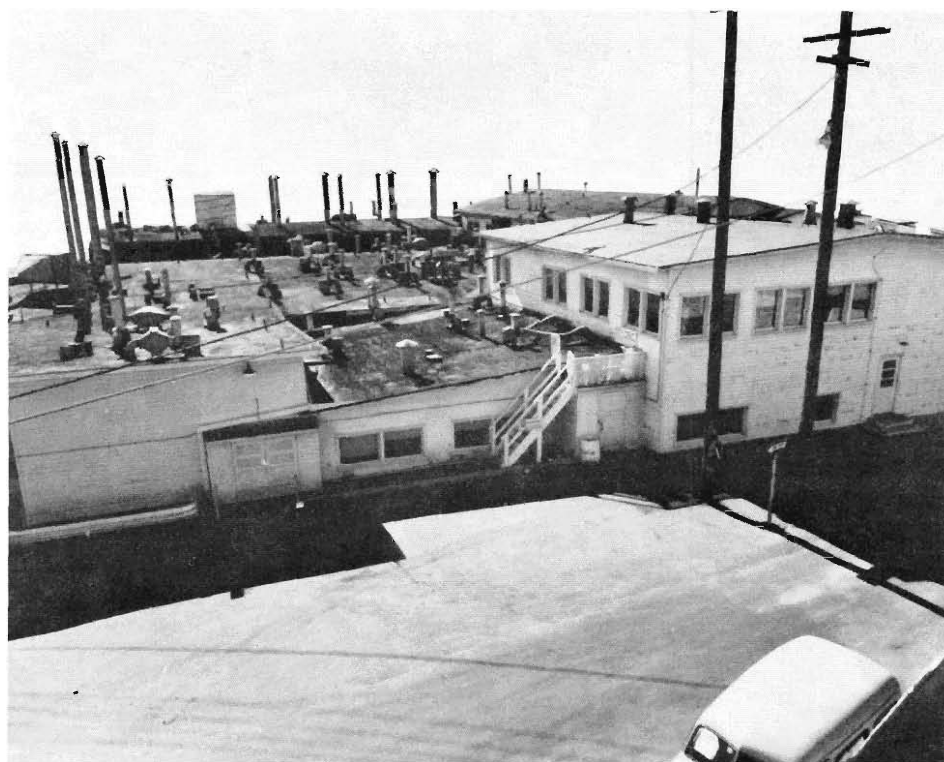
D Building, the air-conditioned wartime plutonium laboratory, bristling with separate external vents.
