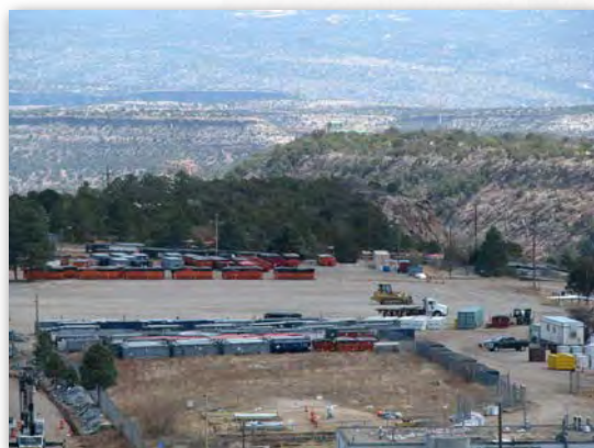
After TA-21 demolition was completed, only waste bins remained. The bins were sorted and shipped to repositories by waste type.
