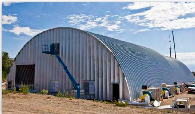
Enclosures were constructed at MDA B to protect the public from airborne radioactive dust and material.
