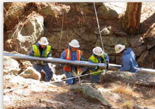
Installing piping to vacuum PCB-contaminated sediments from the drainage.
