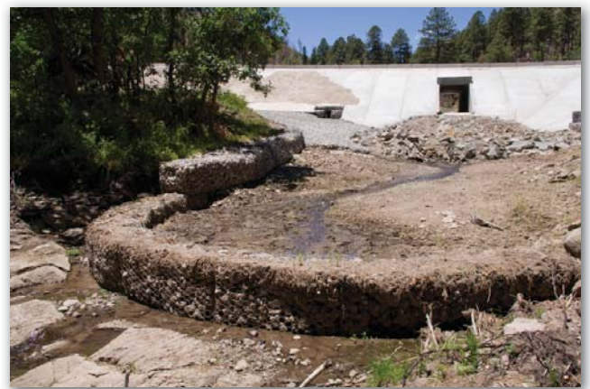
Sediment-control structures were built following the Las Conchas Fire to prevent the transport of ash and sediment.
