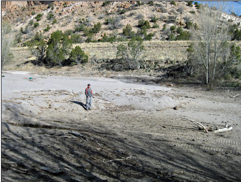
**Photo A1-23 April 2014 photograph of sediment accumulation and delta in the lower basin at the Los Alamos Canyon low-head weir**
