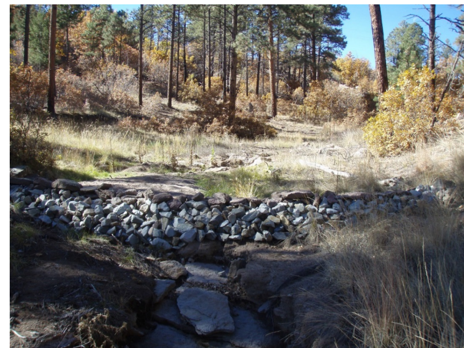
Figure 4 Rock check dam (V00706010024) in Fishladder Canyon (11/4/2015)
