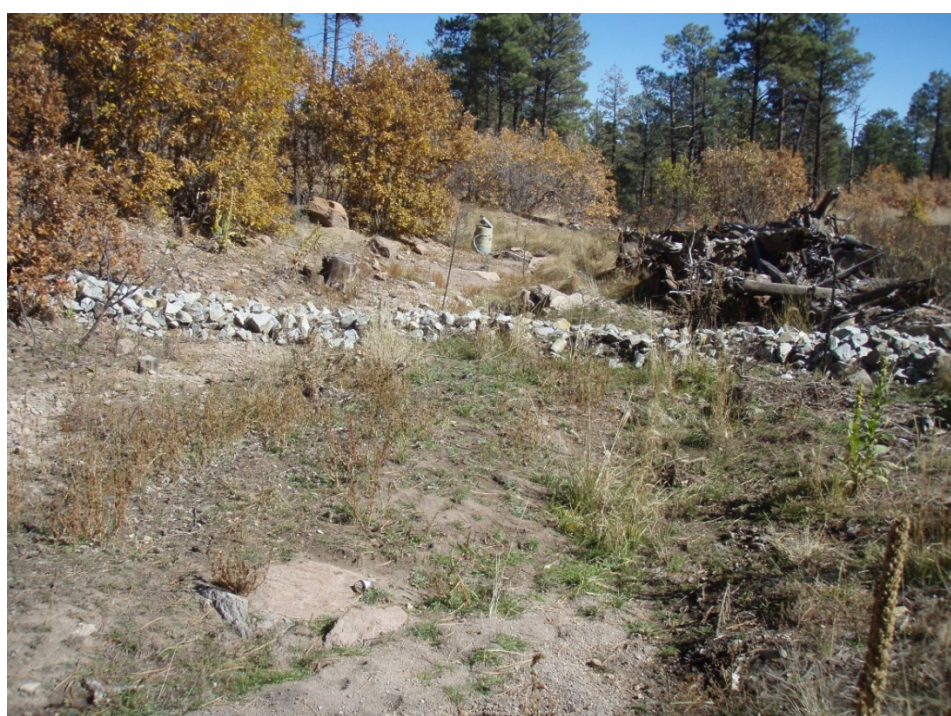
Figure 5 Rock check dam (V00706010025) in Fishladder Canyon (11/4/2015)
