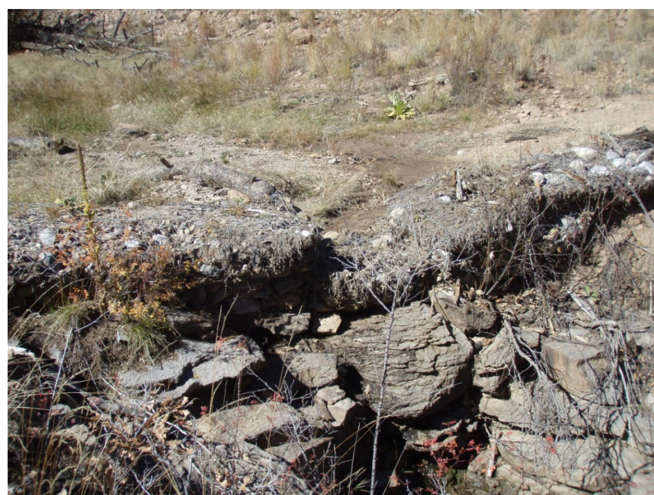
Figure 6 Gabion (V00707010002) at access road crossing in Fishladder Canyon (11/4/2015)
