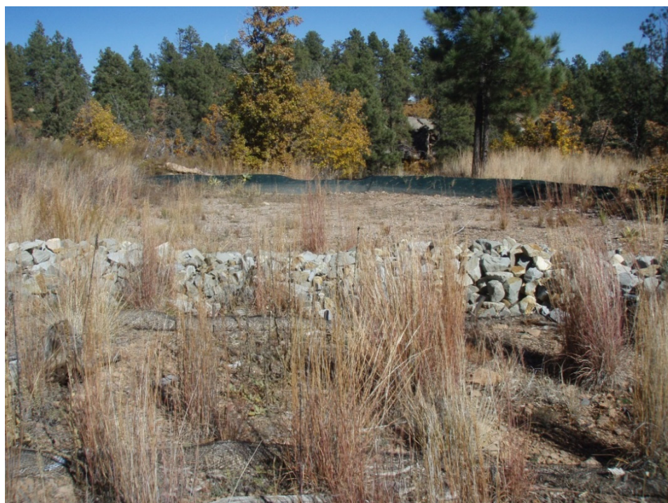
Figure 2 Rock berm (V00703120026) and earth berm (V00703010027) at the top of drainage into Fishladder Canyon (11/4/2015)
