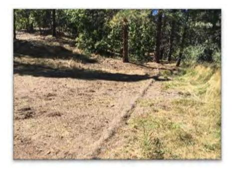
Figure E-2.1-6 September 2017: Logs were trenched end-to-end to create a flow spreader. This control will encourage sheet flow into the wetland, rather than allowing more erosive concentrated flows. Looking west.
