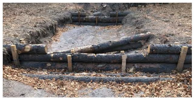
Figure E-2.1-3 December 2017: View of failed log check dams with displaced scour protection logs. Looking upstream.
