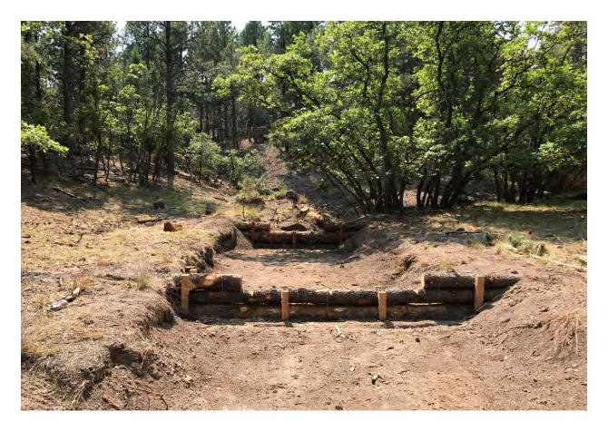
Figure E-2.1-2 September 2017: View of newly installed log check dams looking upstream
