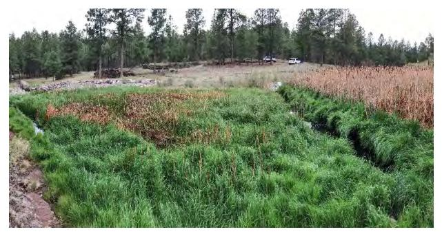
Figure E-3.5-1 May 2017: Wetland vegetation well established. Dispersing flow evenly throughout GCS. No evidence of channelization. No evidence of cracking on spalling on concrete wall.
