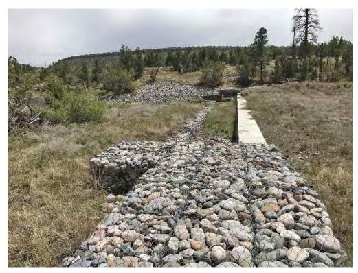
Photo C-5.4-1 May 2017—No cracks present in concrete. Structure and gabion baskets are in alignment and functioning as designed.
