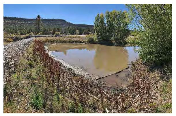
Photo C-4.2-2 October 2017—No change in condition from the last inspection (May 2017). Control at same sediment capacity and standing water at same level.
