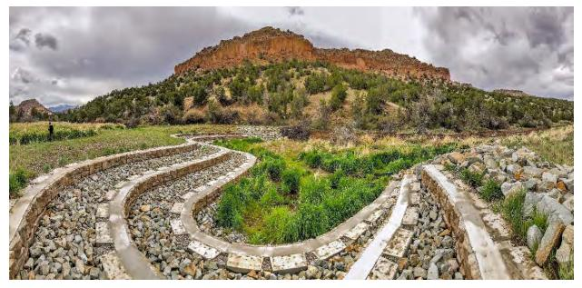
Photo C-6.1-1 May 2017—Redi-Rock structure shows no evidence of displacement or settling. Reed canary grace is well established both upstream and downstream of control.
