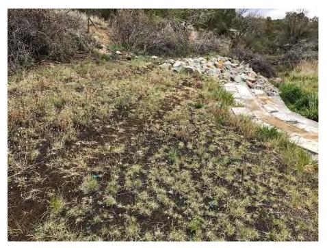
Photo C-6.2-1 May 2017—Minor growth of established vegetation occurring through matting. Slope is stable.
