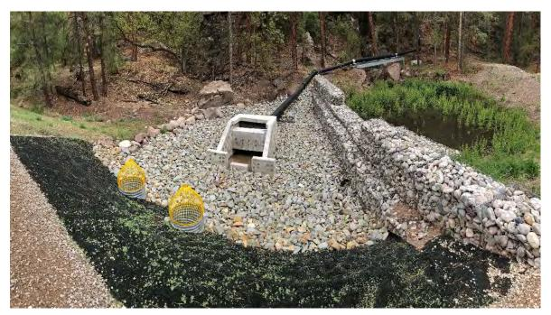
Photo C-3.7-1 May 2017—Pipeline outlet and energy dissipater is clear of debris with minor established vegetation occurring through turf reinforcement matting (TRM). Culvert outlet and inlets appear functional.
