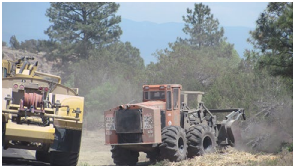
Figure 2-1: Masticators used to chip biomass in place
