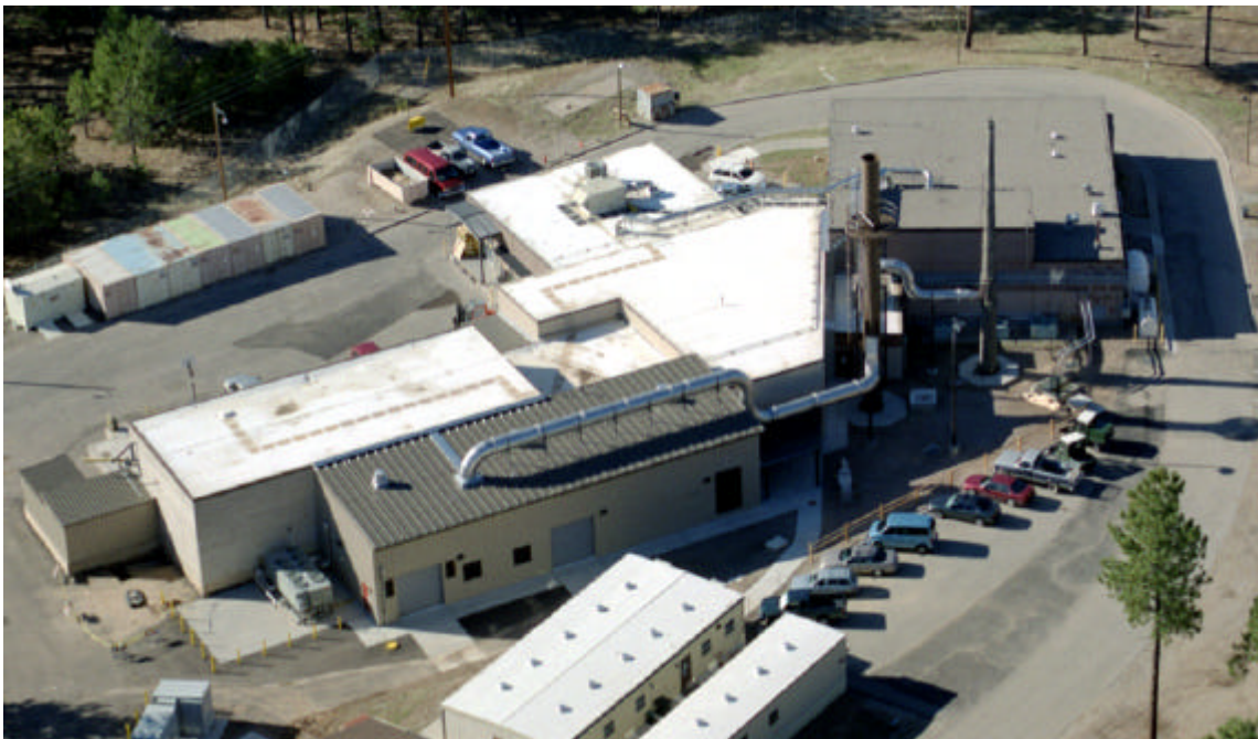
Figure 6. TA-16 Weapons Engineering Tritium Facility.
