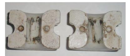
Fig. 4-4. Keyed Surfaces of a Split Knob. The two halves of a split knob fit together to form a doughnut-shaped insulator.
