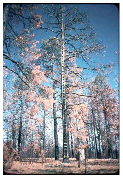
Fig. 2-12. Lookout Tree Ladder at the Wye Upper Crossing. In 1936–7 the Civilian Conservation Corps (CCC) built two ladder trees to help locate fires. One ladder tree was at Upper Crossing (above) and a similar ladder tree was at Corral Hill. Neither ladder tree remains. The CCC also extended the telephone lines to each of the Lookout trees. This photo was taken soon after the 1977 La Mesa Fire. (Photo: Chris Judson, National Park Service)
