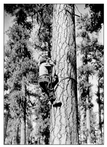
Fig. 1-3. Hanging the Telephone Line, 1933. Men used climbing spurs to attach telephone insulators twenty feet up in tall, straight ponderosas. (Photo: Forest History Society at Duke University)
