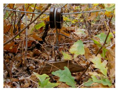
Fig. 5-28. Smooth Oval Knob on Line. This smooth type of oval split knob was found along the Duran Road where it climbs out of the south side of Los Alamos Canyon. The thimble and staple have pulled out of the tree, taking a wedge of wood with them. A long length of telephone line, edging the old road, is still strung through the split knob's center hole. (GPS waypoint D36)
