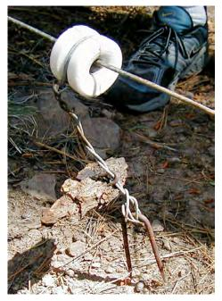
Fig. 4-17. Three-Inch Staple. The three-inch staple that once held this medium round split knob to the tree in Twomile Canyon has pulled off allowing the line to fall. (GPS waypoint TM4)
