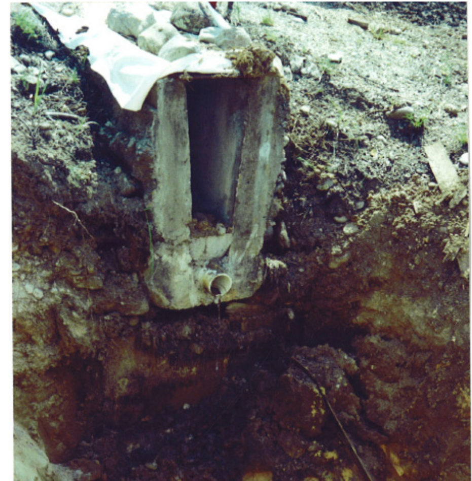
Figure 3.3-1 Photograph of concrete drainage trough
