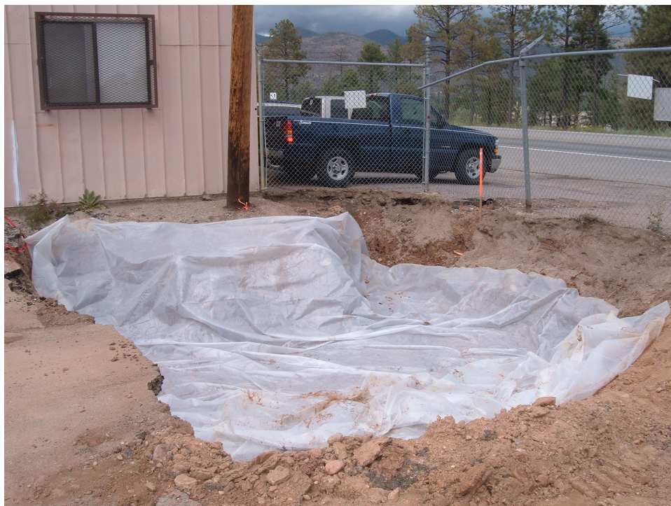
Figure B-12 Installation of plastic layer before backfilling with clean fill in northwestern corner of SWMU 61-002 where petroleum hydrocarbon contaminated soil was found (Building 61-23 in background)
