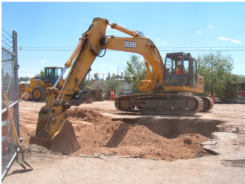
Figure B-10 Backfilling excavation with clean fill using trackhoe at SWMU 61-002 near access gate area
