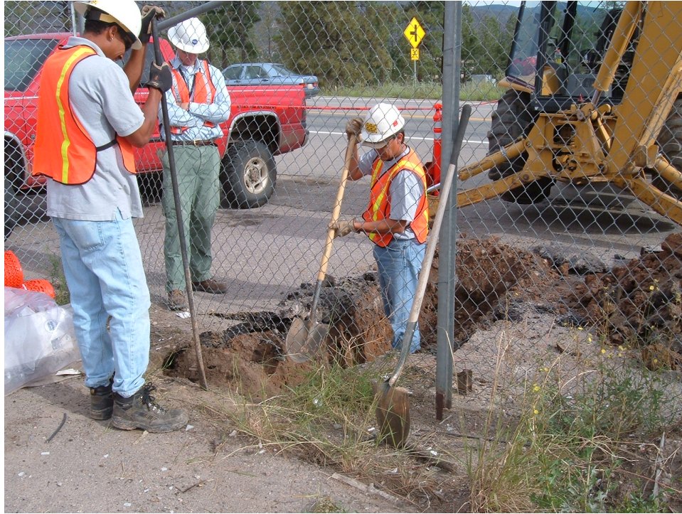
Figure B-5 Potholing before excavation at SWMU 61-002. Pothole dug for locating buried electrical cable near the northern fence line.
