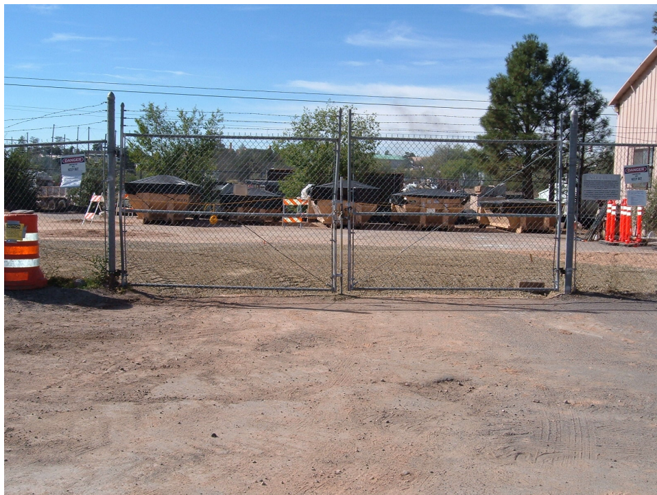
Figure B-15 Excavated area was restored with base course after backfilling was completed. Note five roll-off waste bins with covers that contain petroleum-contaminated soil removed from northwestern corner of SWMU 61-002.
