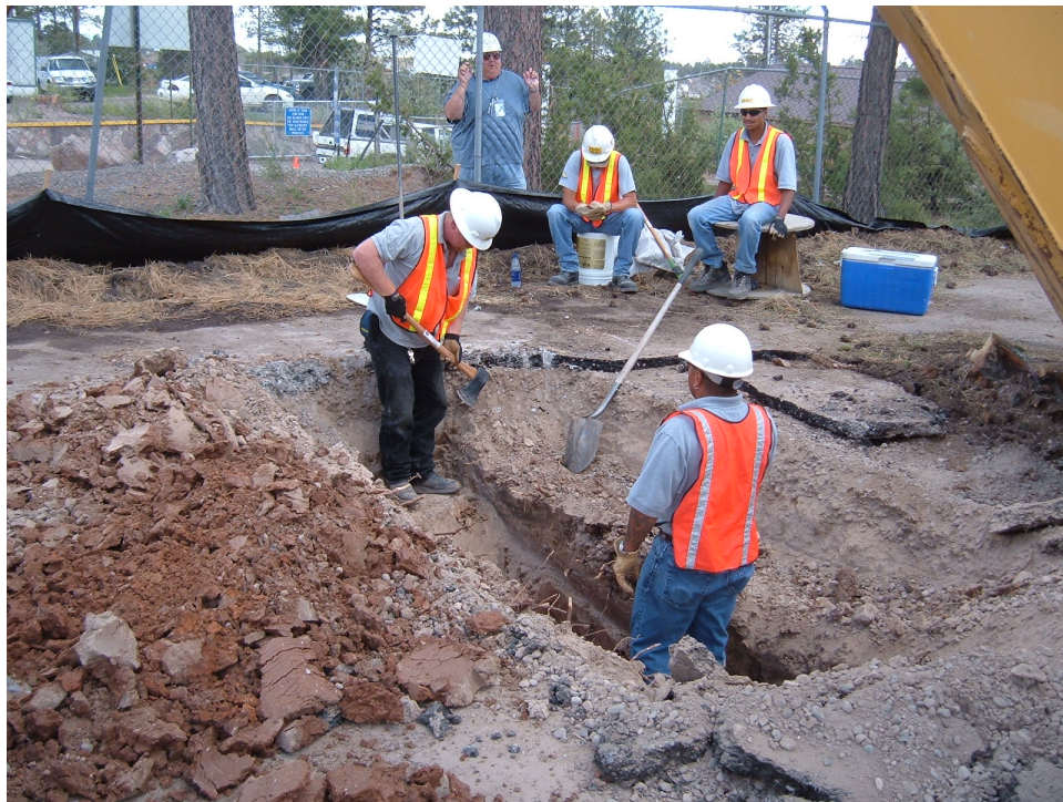
Figure B-6 Potholing before excavation at SWMU 61-002. Pothole dug to find water line shown on excavation permit map near northeast corner of property. No water line was found after hand digging to 6 ft bgs.
