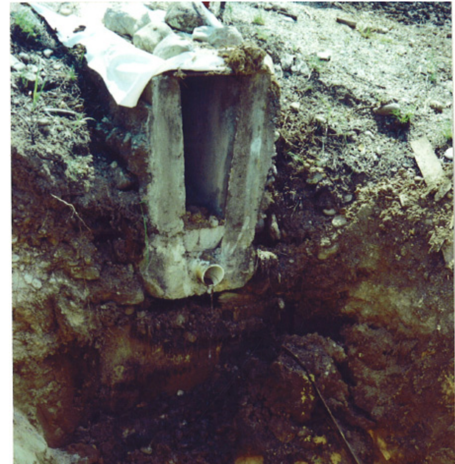
Figure 3.3-1 Photograph of concrete drainage trough
