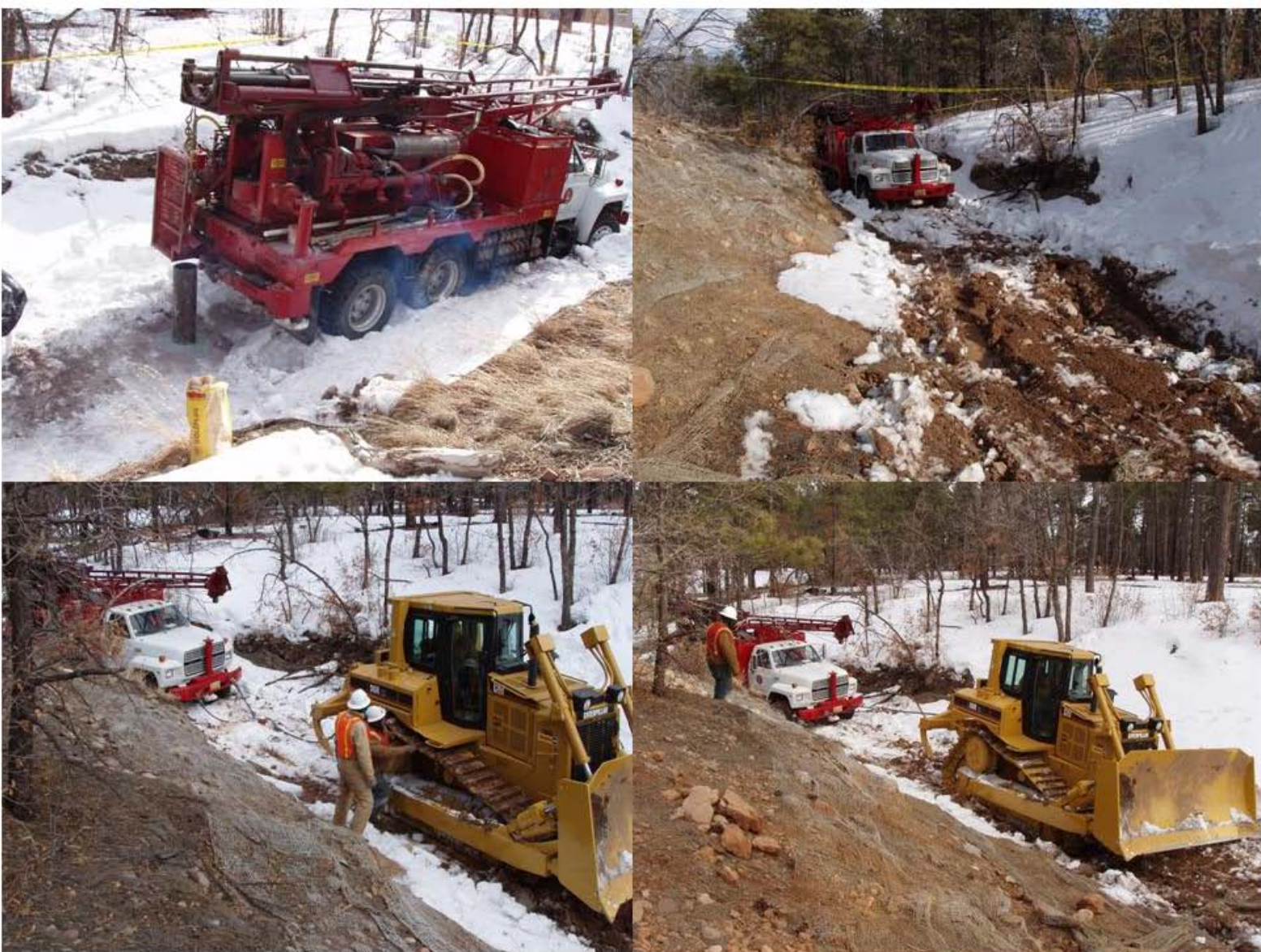
Figure C-5.1-1 Drilling and accessing borehole location 16-27667 in the 260 drainage, March 2, 2007
