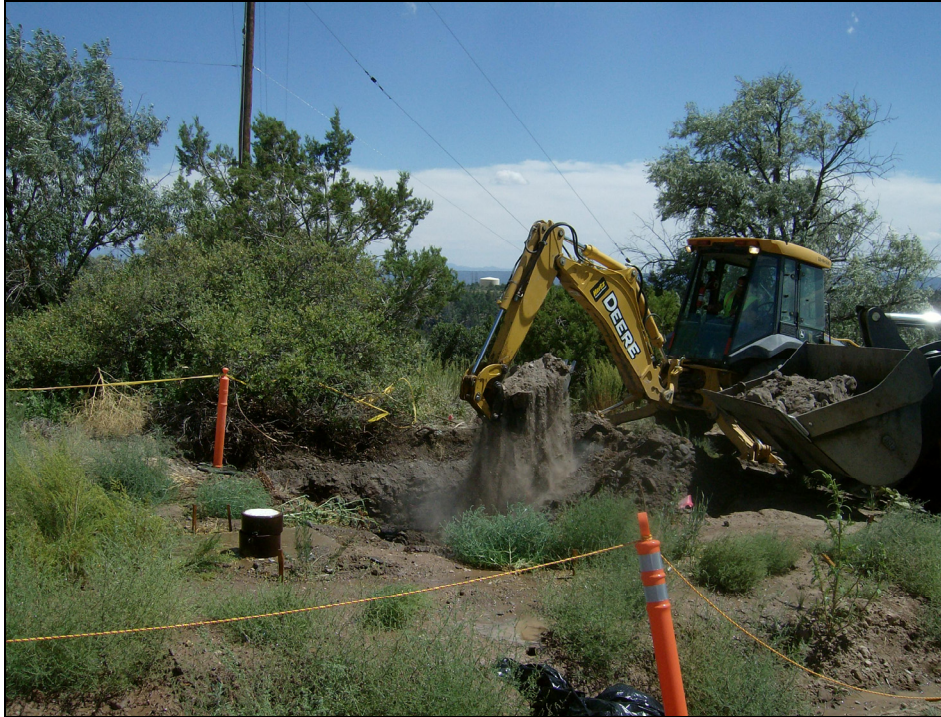
Photo 7 Excavation of elevated area of radioactivity, August-September 2007
