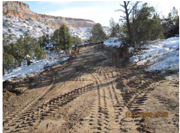
Photo 4 Grading of permanent access road
