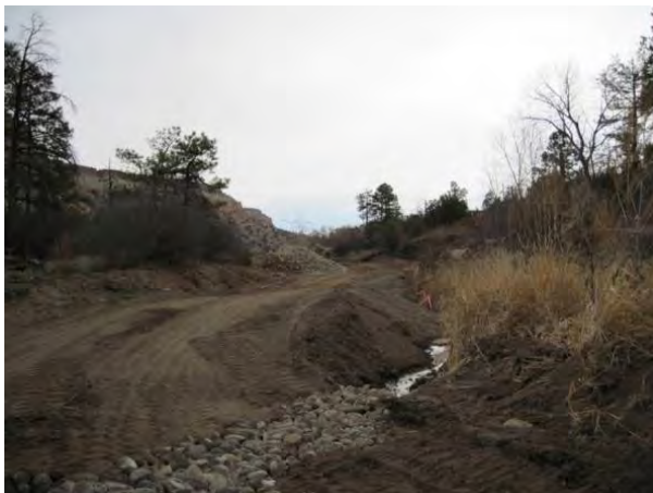
Photo 9 Stream through temporary access road, diversion channel-right side of photo
