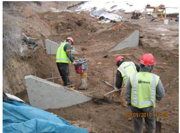
Photo 4 Flume subgrade compaction
