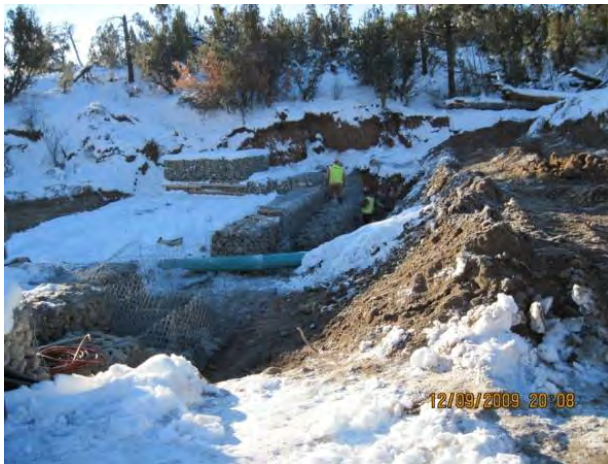
Photo 3 Gabion structure, looking south
