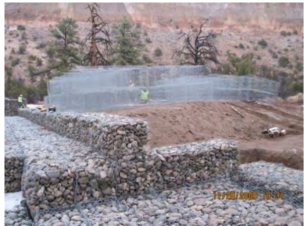
Photo 4 Structure looking northeast, gabion-basket production
