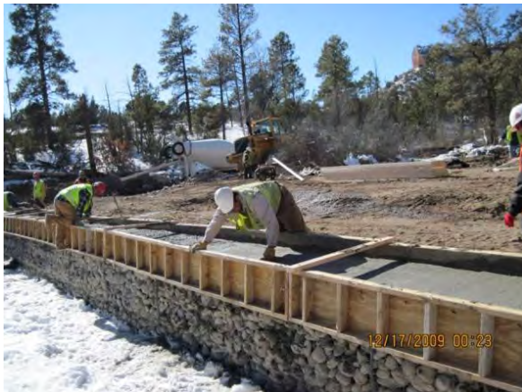
Photo 1 Concrete cap finishing
