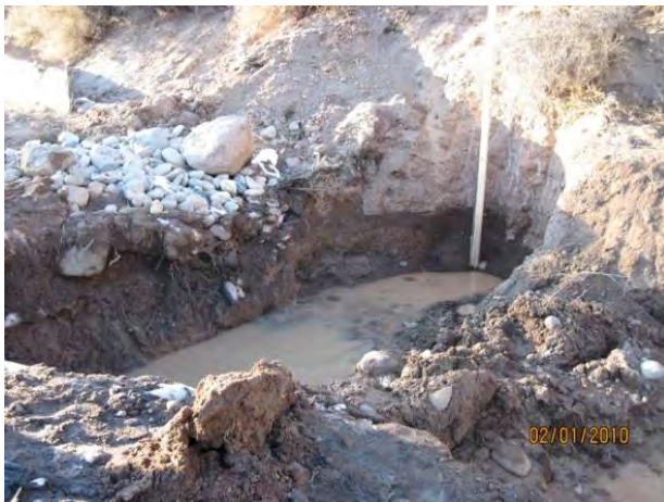
Photo 3 Groundwater intrusion in flume excavation
