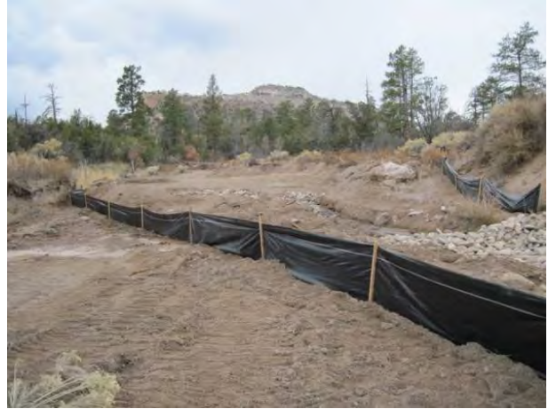
Photo 22 Silt fence, downstream of structure around borrow area
