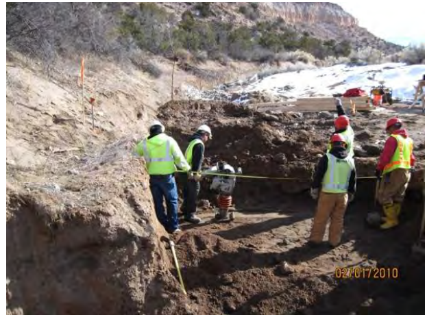
Photo 14 Headwall subgrade compaction
