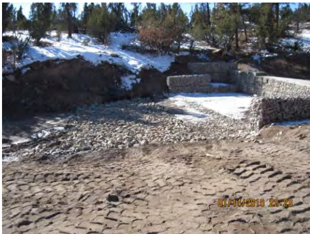
Photo 7 Stilling basin, downstream Class B rip rap armoring
