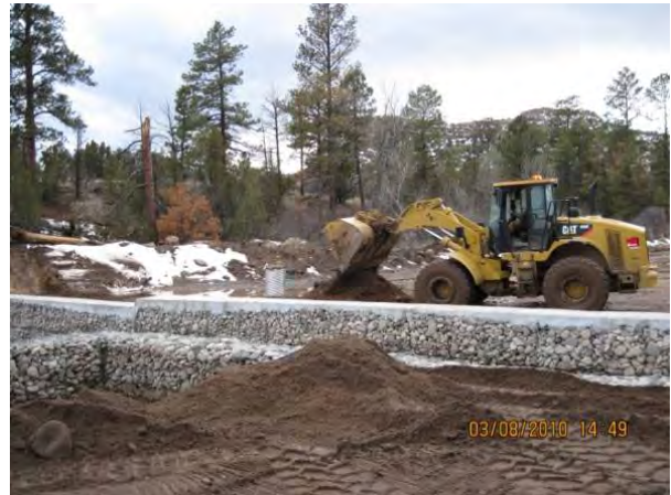
Photo 8 Final grading, upstream side of structure
