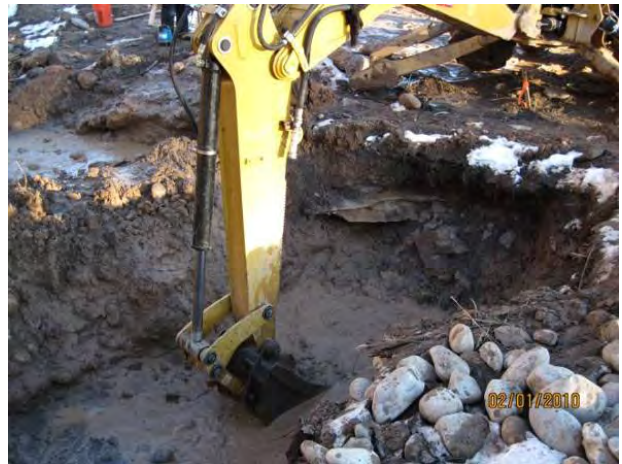
Photo 8 Excavation for flume
