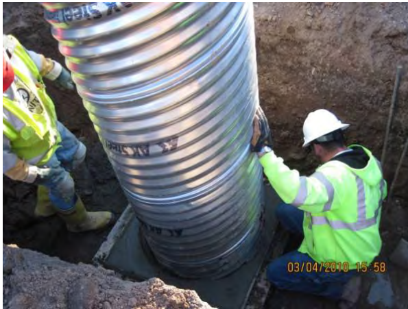
Photo 3 Placing stilling well for gage
