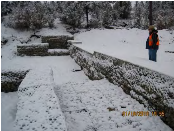
Photo 7 Overflow weir bench, overflow weir
