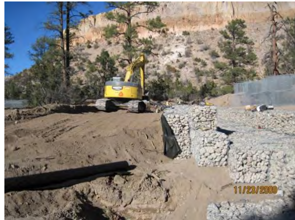
Photo 2 Subgrade overflow weir gabion baskets
