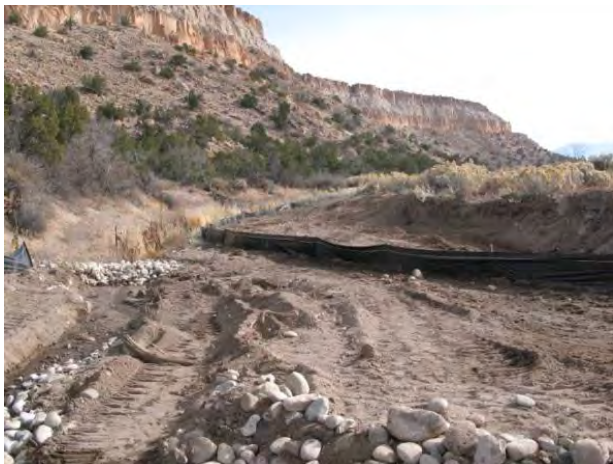
Photo 3 Silt fence and rock check dam, downgradient of structure
