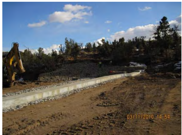
Photo 4 Upstream side of low-flow weir
