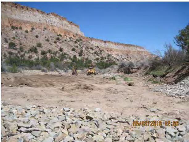
Photo 3 Flume Class B rip-rap installation looking downstream from structure
