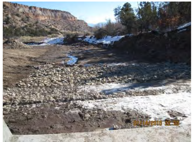
Photo 4 Class B rip rap, downstream side of stilling basin
