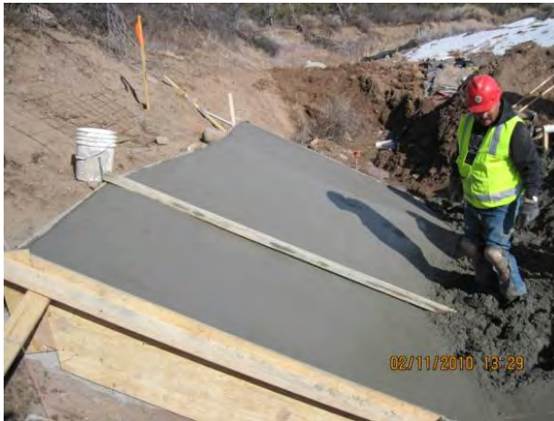
Photo 9 Concrete finishing of flume
