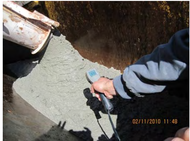
Photo 2 Monitoring temperature of concrete for flume concrete placement
