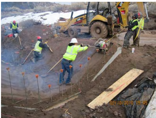
Photo 5 Flume subgrade compaction
