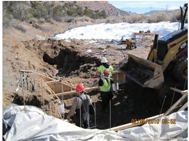
Photo 8 Flume headwall concrete placement
