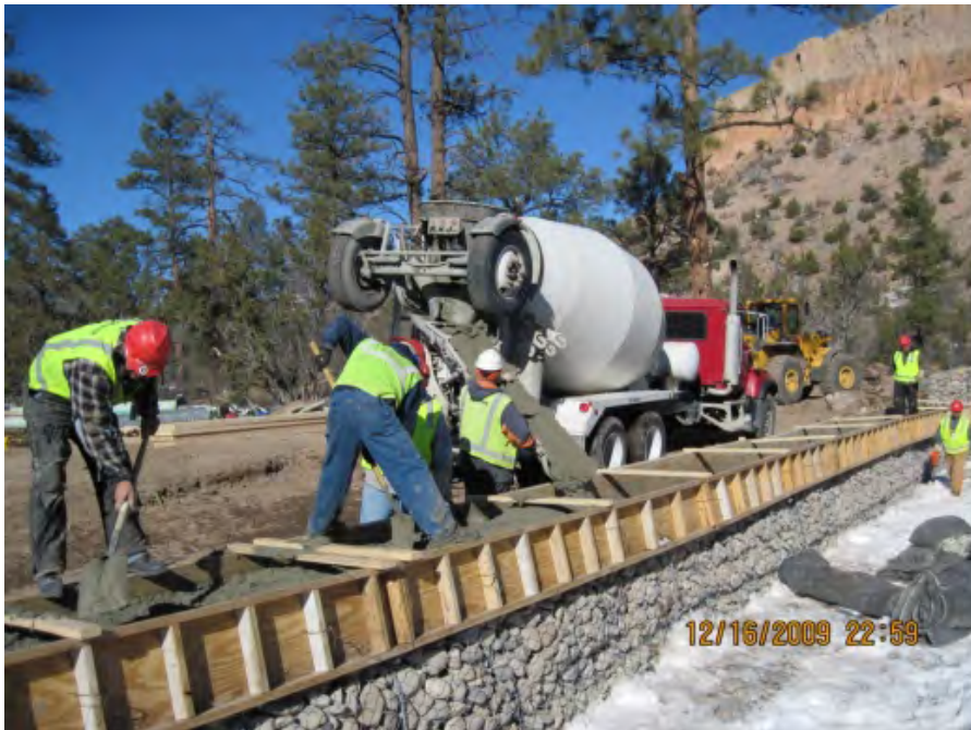
Figure 2.1-2 Placement of concrete cap
