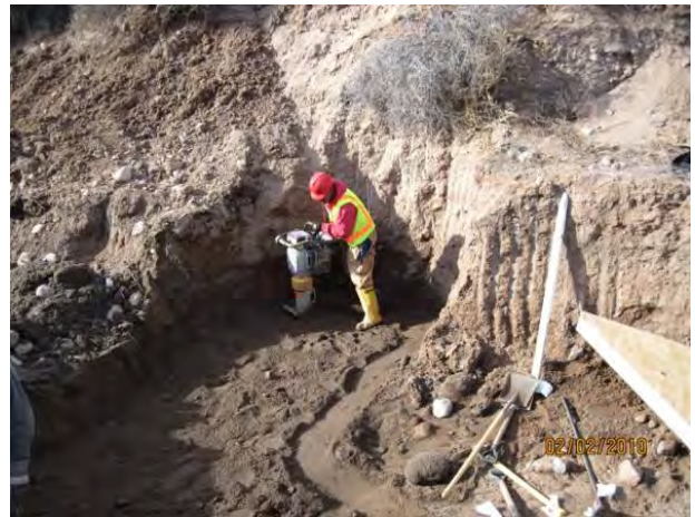
Photo 4 Headwall subgrade compaction
