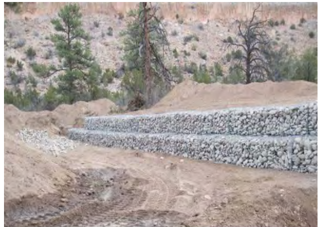
Photo 14 Gabion structure upstream, looking northeast at overflow weir subgrade and crest
