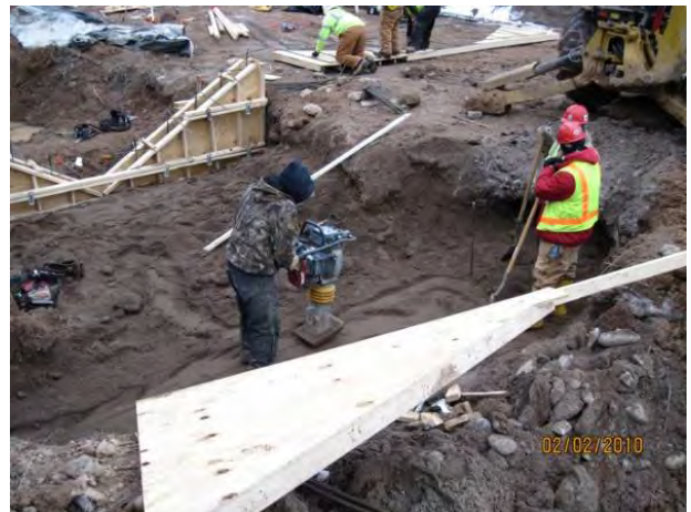
Photo 6 Headwall subgrade compaction
