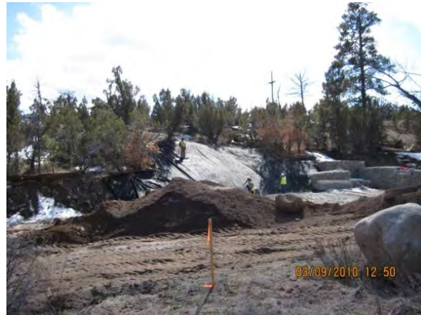
Photo 4 Preparing to place Class A rip-rap armoring on south slope downgradient of structure
