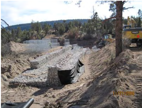
Photo 9 Geotextile fabric on upstream face of structure
