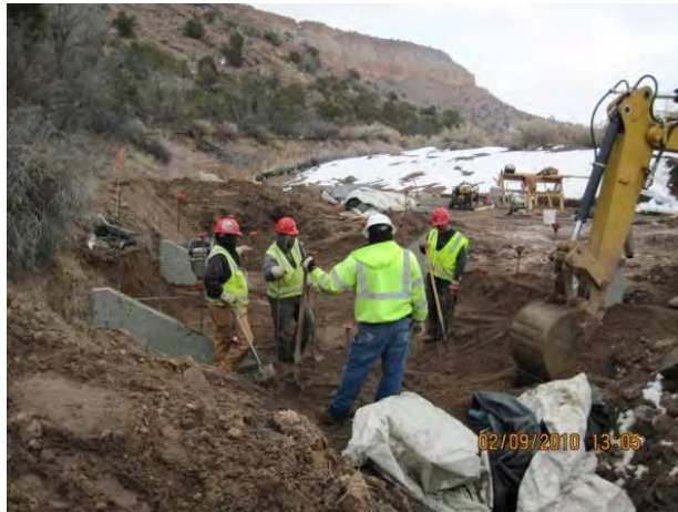
Photo 1 Excavation for flume subgrade
