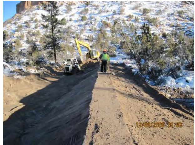
Photo 2 Earthen berm construction
