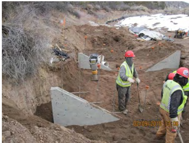
Photo 3 Flume headwalls
