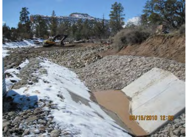
Photo 2 Concrete flume
