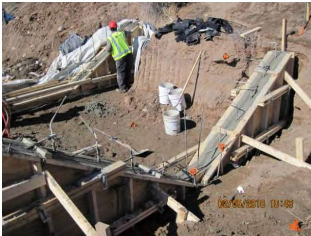
Photo 9 Flume headwall concrete placement
