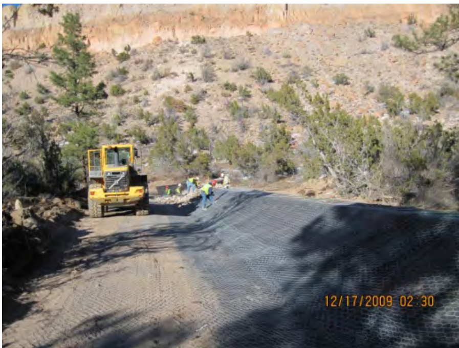
Figure 2.1-4 Construction of Class A rip-rap armored earthen berm (looking north)
