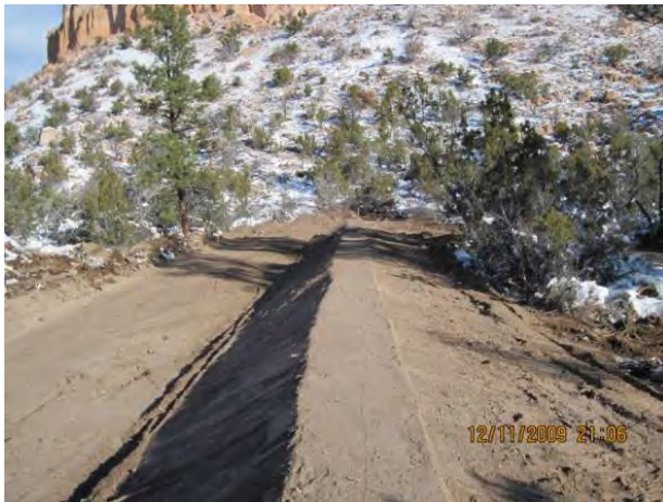
Photo 9 Compacted earthen berm
