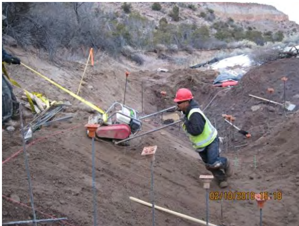
Photo 3 Flume subgrade compaction
