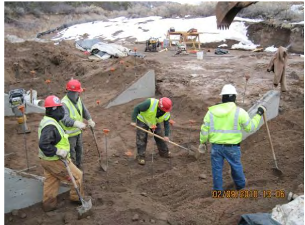
Photo 2 Excavation for flume subgrade
