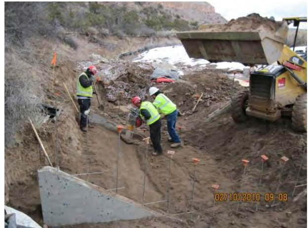
Photo 2 Flume subgrade compaction
