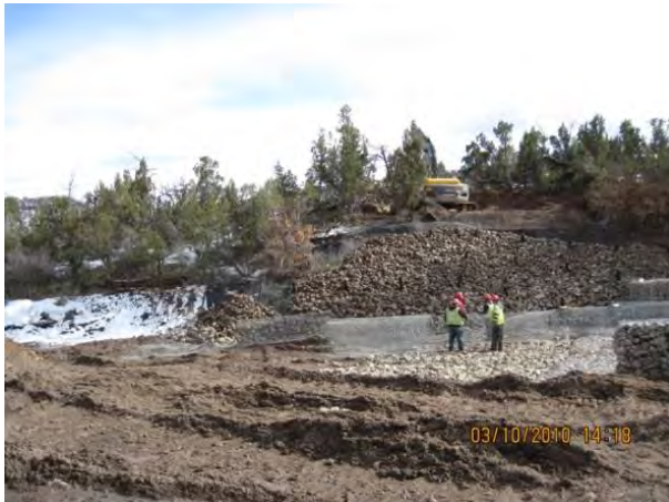
Photo 7 Working on installing Class A rip-rap armoring, south slope downgradient of structure
