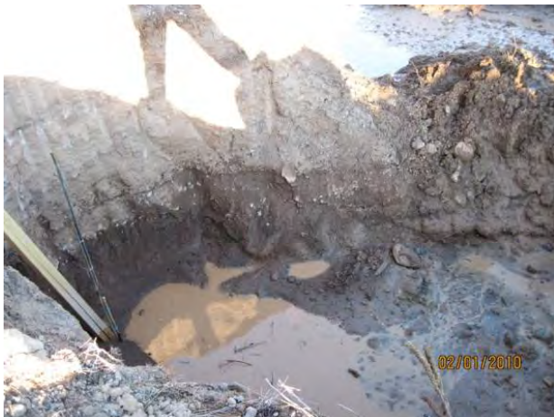
Photo 9 Excavation for flume, groundwater intrusion
