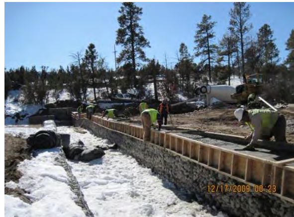
Photo 2 Looking south, concrete cap placement
