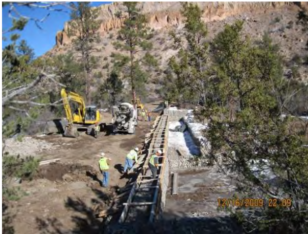
Photo 3 Form for concrete cap
