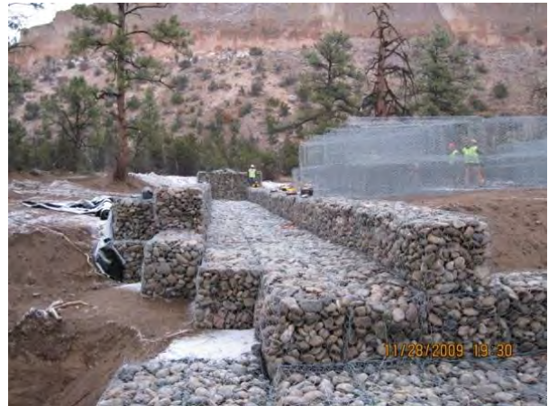
Photo 2 Structure looking north, gabion-basket production
