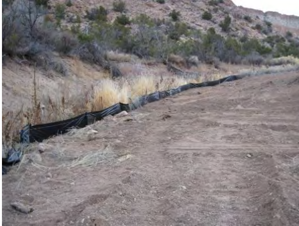
Photo 17 Silt fence along channel, looking downstream of borrow area
