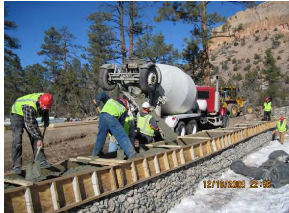
Photo 10 Concrete placement, low-flow and overflow weir
