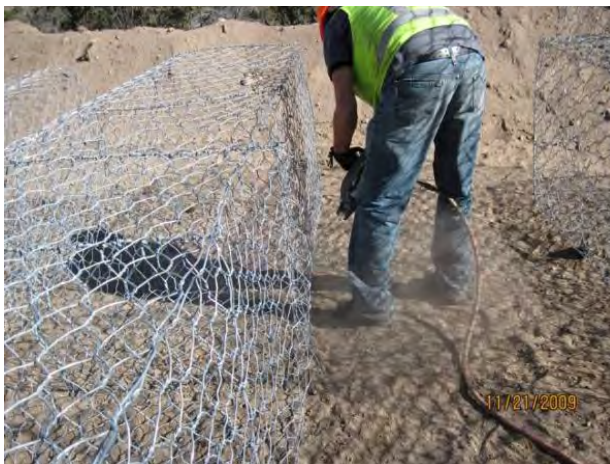
Photo 7 Gabion assembly
