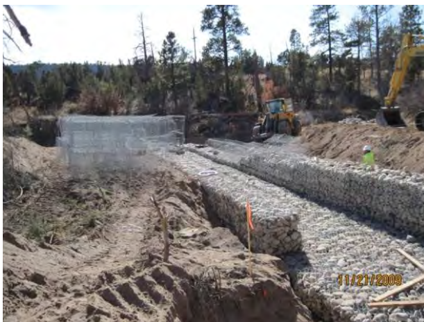
Photo 13 Overflow basin/gabion bench, looking southwest
