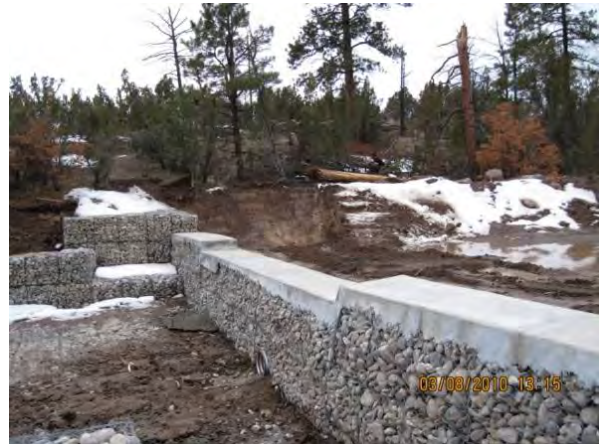
Photo 2 Structure, looking at south upgradient slope, being prepared for Class A rip-rap armoring installation
