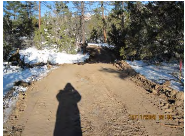
Photo 2 Grading of permanent access road
