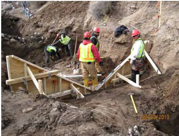
Photo 1 Flume headwall form work
