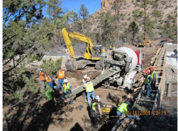
Photo 6 Concrete placement, low-flow and overflow weir
