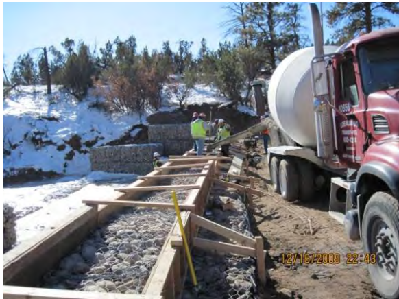
Photo 9 Concrete placement, low-flow and overflow weir
