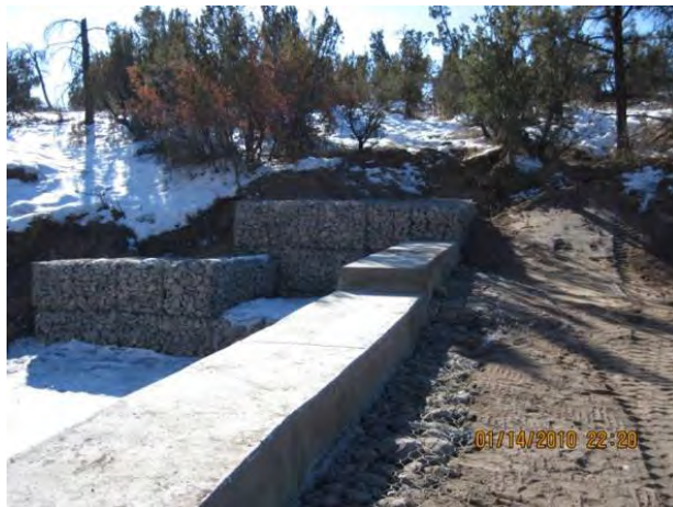
Photo 3 South portion of structure, low-flow weir (foreground), overflow weir, confinement wall and gabion bench
