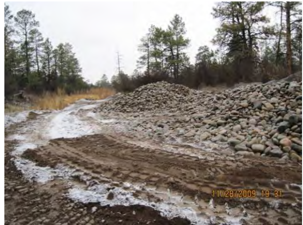
Photo 8 Class A rip-rap stone stockpiles
