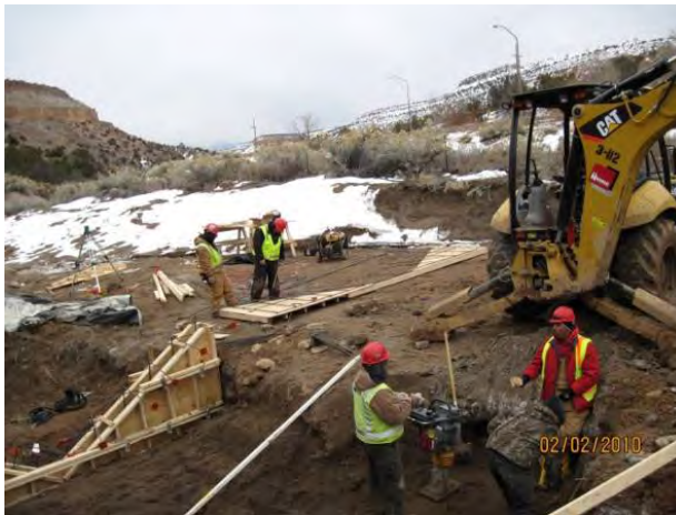
Photo 9 Headwall form work
