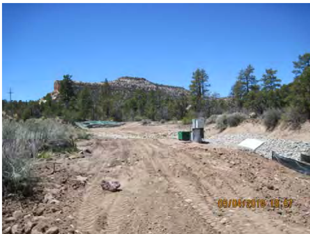
Photo 7 View looking upstream at flume and stilling well (foreground) and structure (background)
