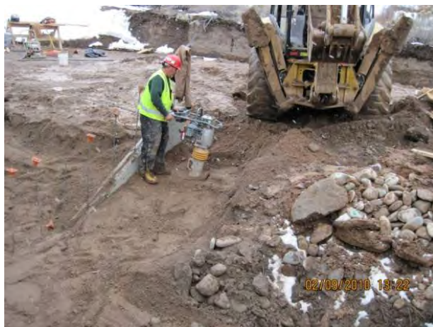
Photo 5 Flume subgrade compaction
