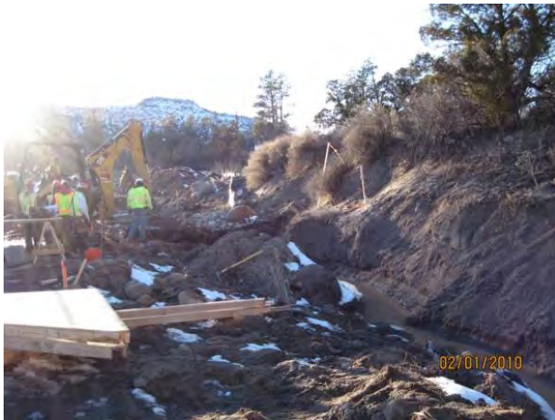
Photo 7 Form work for flume
