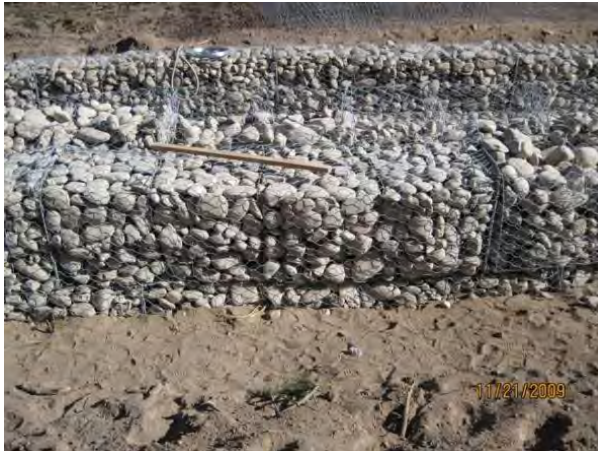
Photo 11 Close-up view of gabion baskets
