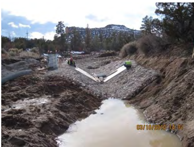
Photo 9 Working on Class A rip-rap entrance to flume
