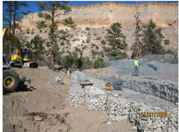
Photo 4 Gabion construction, looking north
