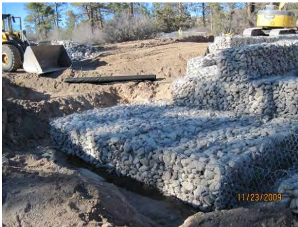
Photo 5 Stilling-basin gabion baskets, looking northwest
