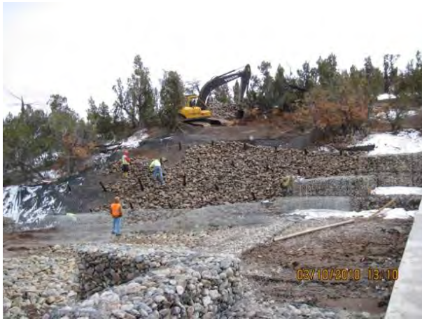
Photo 5 Looking south at south slope armoring
