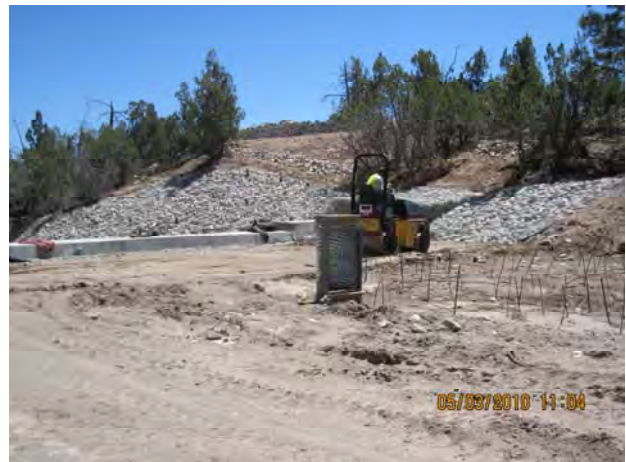
Photo 4 Final grading upstream of structure, riser pipe and willows in foreground
