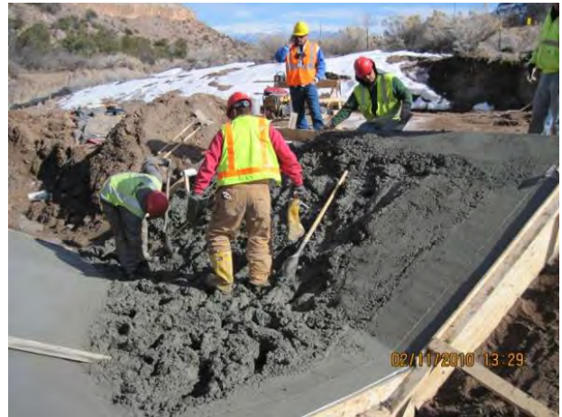
Photo 10 Concrete finishing of flume
