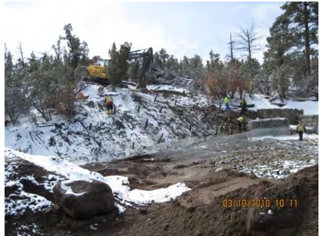
Photo 2 Looking upgradient at south downgradient slope Class A rip-rap armoring
