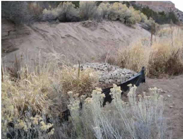
Photo 19 Check dam and silt fence
