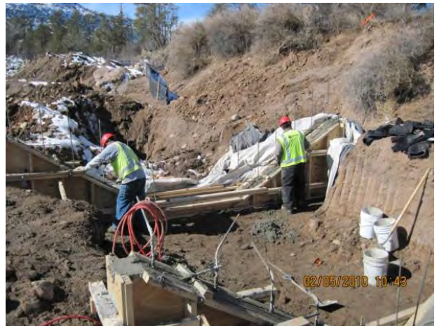
Photo 10 Flume headwall concrete placement
