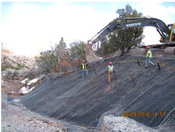
Photo 5 Preparing to place Class A rip-rap armoring on south slope downgradient of structure
