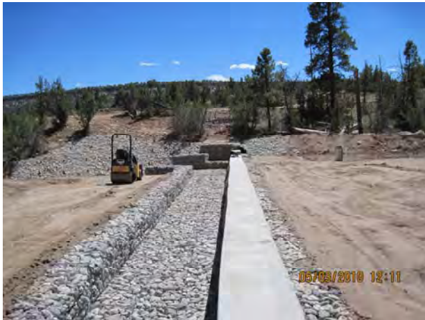
Photo 5 Final grading upstream and downstream of structure, south slope rip-rap armoring in background
