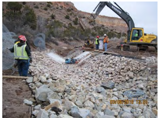
Photo 4 Installing Class A rip rap for flume
