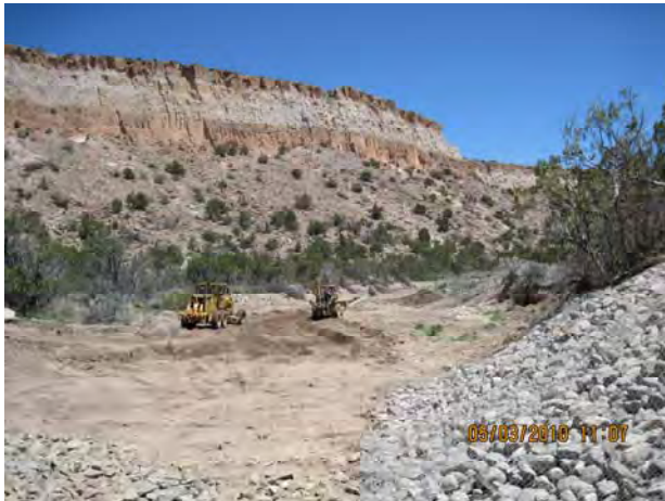
Photo 1 Flume Class B rip-rap installation looking downstream from structure
