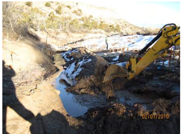
Photo 10 Excavation for flume, groundwater intrusion
