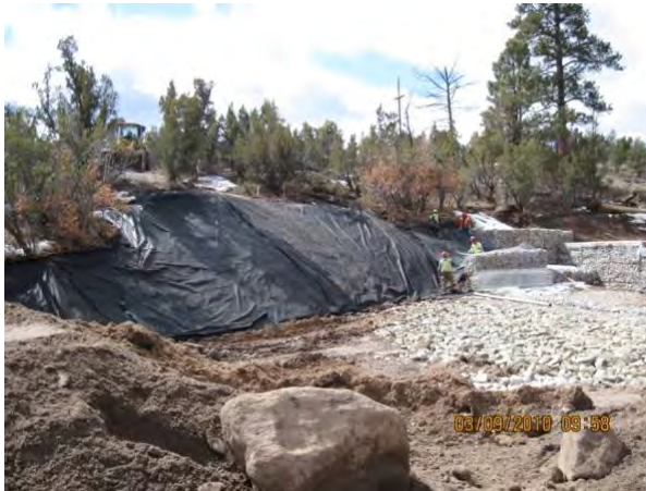
Photo 3 Placing geotextile for south slope rip rap, downstream of structure
