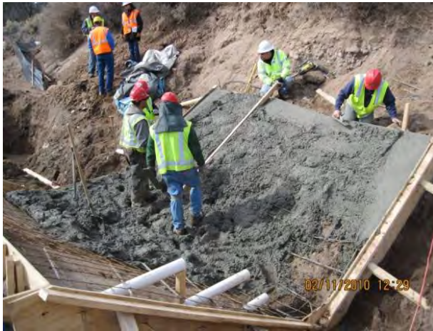
Photo 7 Concrete placement and finishing of flume
