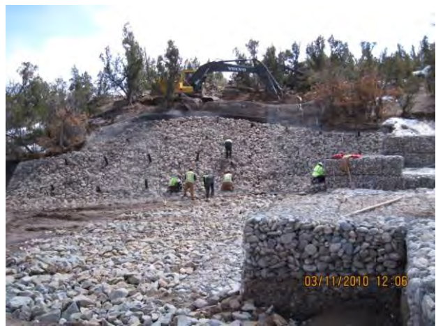
Photo 2 Placing rip-rap armor on south slope downgradient of structure
