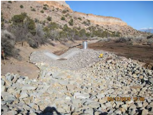
Photo 7 Class B (foreground) and Class A (background) rip-rap approach to flume
