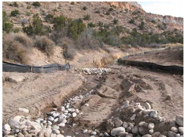
Photo 4 Silt fence and rock check dam
