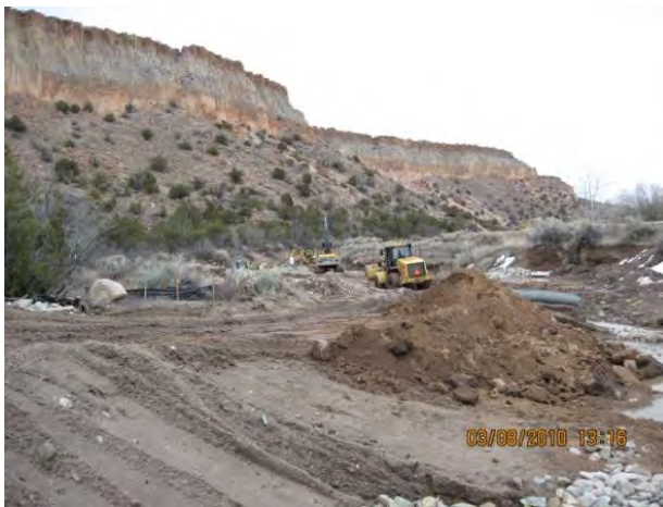
Photo 3 Working on Class B rip-rap installation upstream of flume
