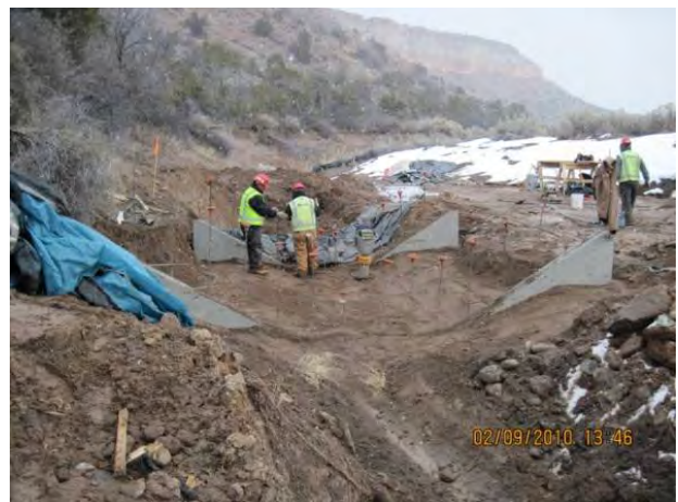
Photo 6 Flume subgrade compaction
