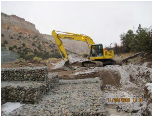
Photo 9 Excavation of south half of stilling basin
