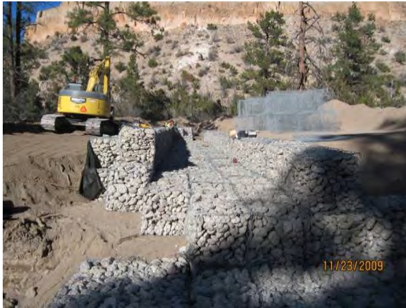
Photo 3 Overflow weir subgrade gabion baskets
