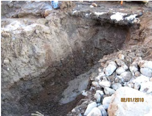
Photo 11 Excavation for flume, groundwater intrusion
