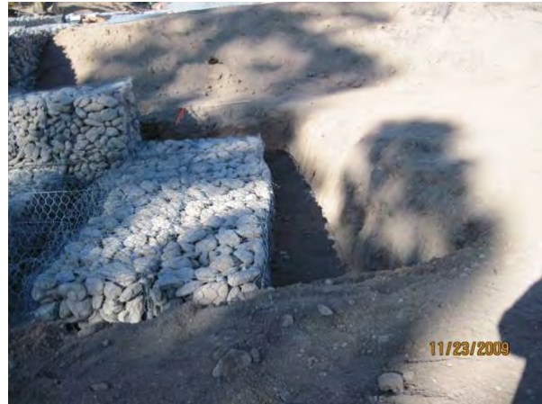
Photo 4 Excavated area for stilling-basin gabion baskets
