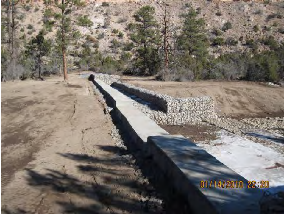
Figure 2.1-1 Pueblo grade-control structure (looking north) showing entire length of weir and 1-ft difference between overflow and low-flow weir crests
