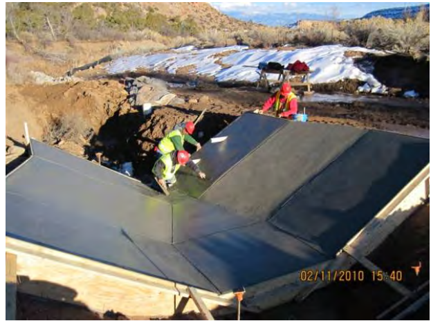
Photo 12 Concrete finishing of flume
