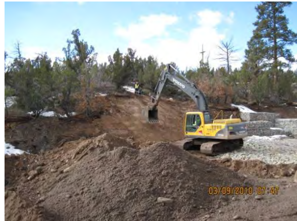
Photo 2 Preparing south slope, downstream of structure, for rip rap
