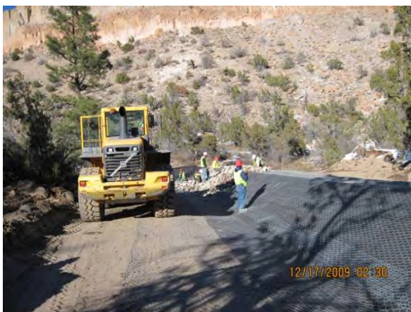
Photo 3 Placing Class A rip rap along upstream side of earthen berm
