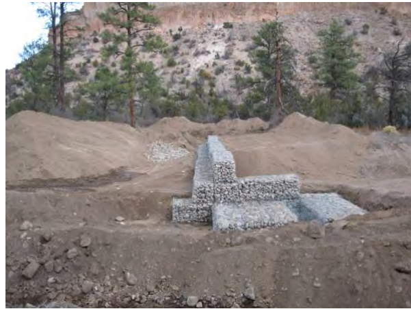
Photo 12 Gabion structure, looking north
