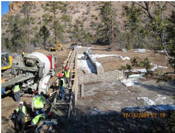
Photo 7 Concrete placement, low-flow and overflow weir
