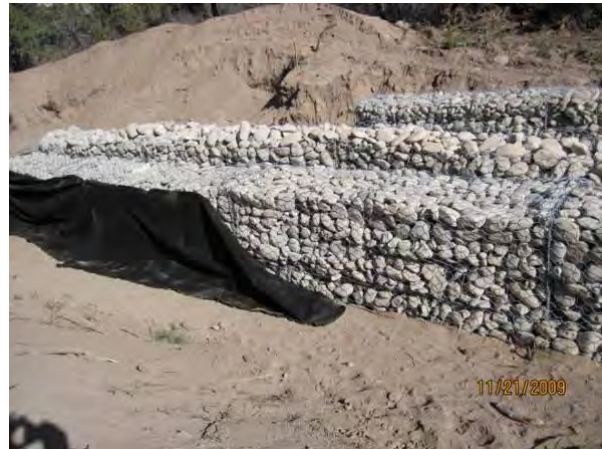
Photo 10 Geotextile fabric on upstream face of structure
