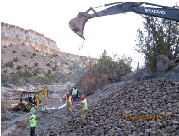
Photo 1 Placing Class A rip-rap armor on south slope downgradient of structure
