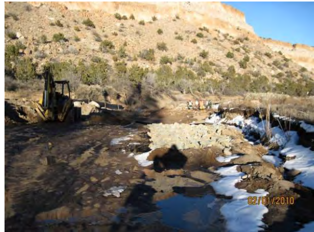
Photo 2 Downstream of structure, Class B rip rap for flume entrance
