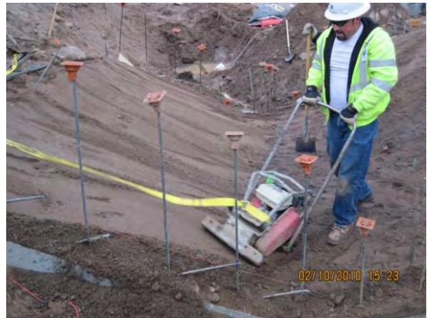
Photo 4 Flume subgrade compaction
