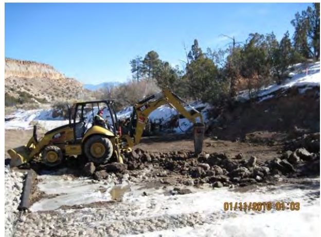
Photo 2 Excavation for installation of Class B rip-rap armoring, downstream side of structure stilling basin
