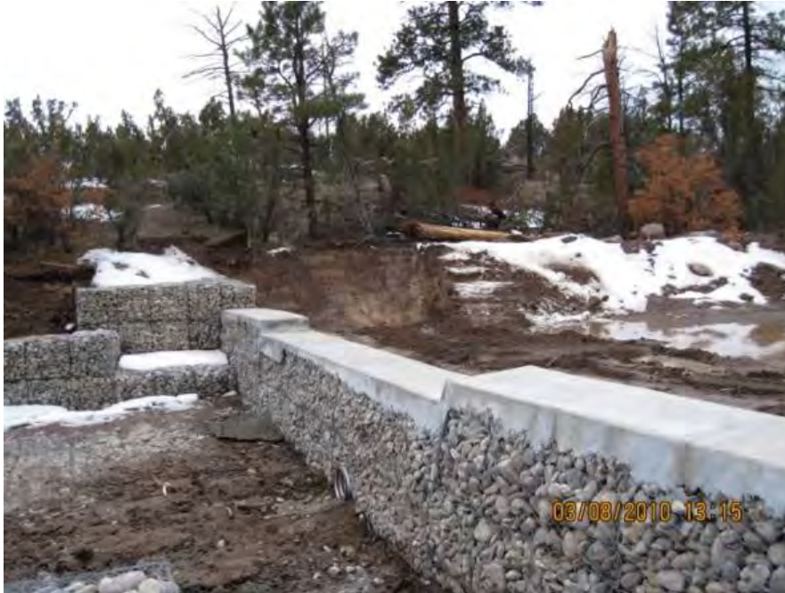
Figure 2.1-3 Pueblo grade-control structure (looking south). Concrete cap on weir
