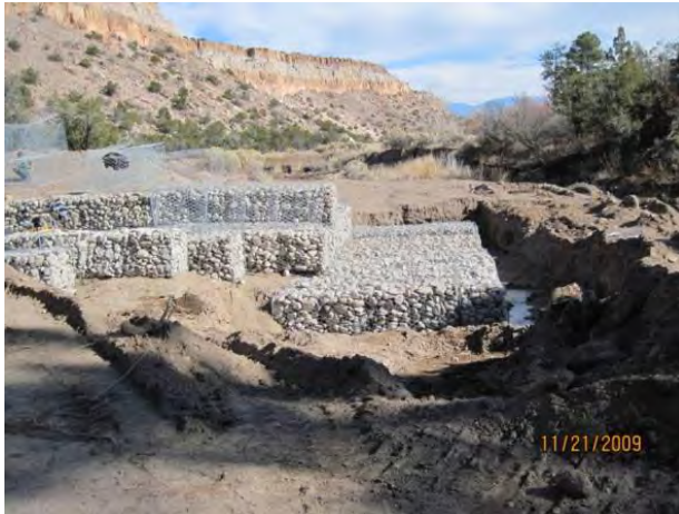
Photo 5 Gabion structure upstream, looking east at stilling basin and overflow weir
