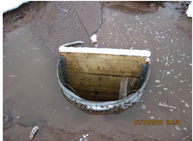
Photo 10 Riser pipe before extension
