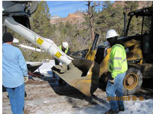
Photo 2 Mode of transporting concrete to flume
