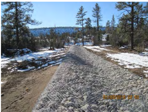
Photo 5 Earthen berm after rip-rap placement
