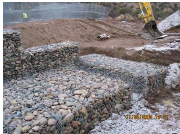
Photo 6 Subgrade gabion baskets for gabion bench and stilling basin
