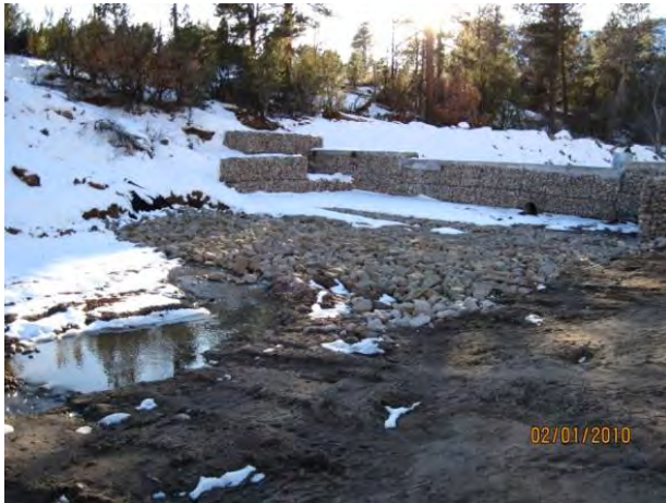
Photo 1 Structure, looking upstream at stilling basin and riser-pipe outlet pipe
