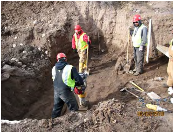
Photo 3 Headwall subgrade compaction
