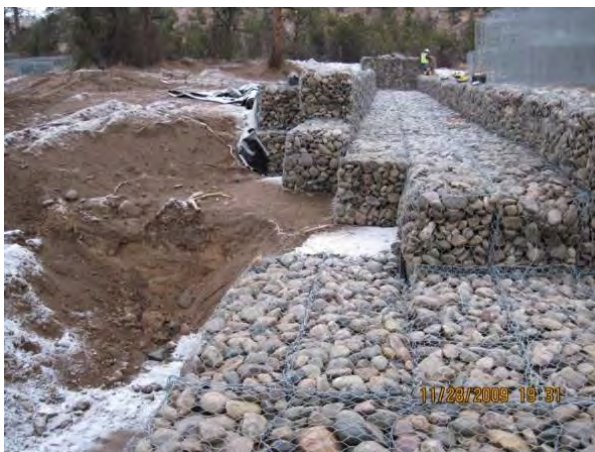
Photo 5 Subgrade gabion baskets for gabion bench and stilling basin
