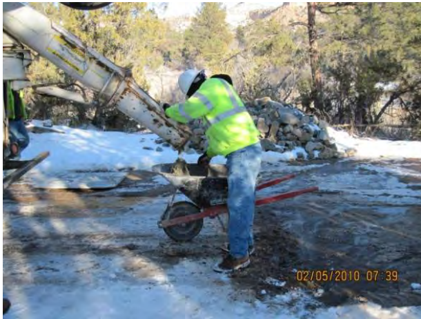
Photo 1 Concrete testing for flume headwall concrete placement
