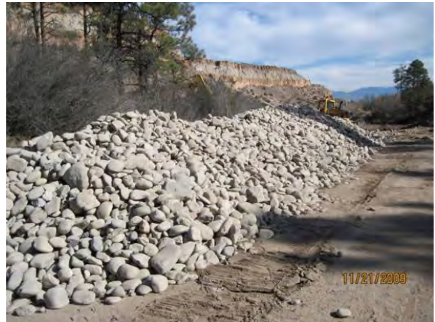
Photo 2 Gabion stone stockpile
