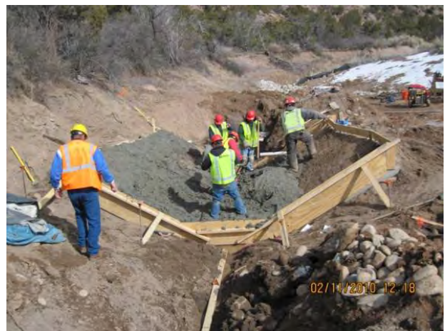
Photo 6 Placing concrete flume
