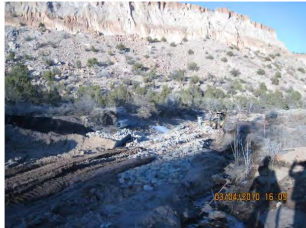
Photo 4 Working on flume rip-rap installation
