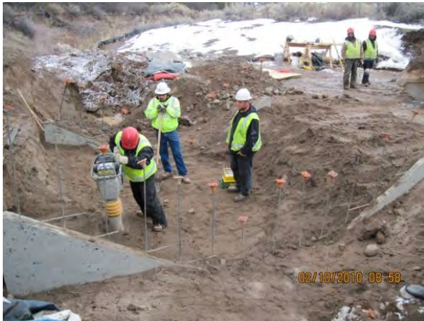
Photo 1 Flume subgrade compaction
