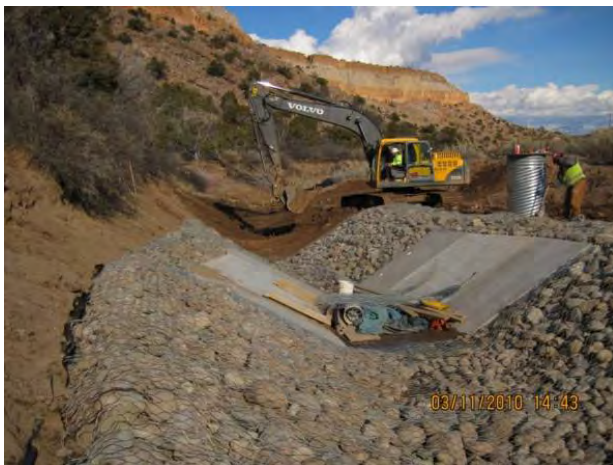
Photo 3 Finalizing grade downstream of flume
