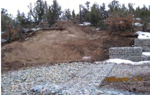
Photo 1 View of south downgradient slope being prepared for Class A rip-rap armoring installation
