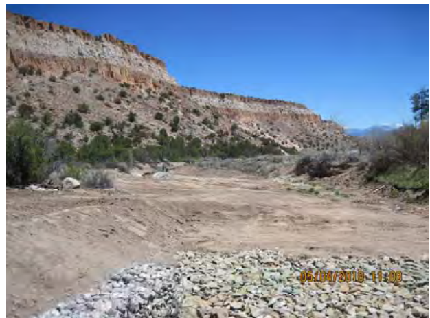
Photo 8 View looking downstream at flume from structure, Class B armoring on downstream side of structure in foreground
