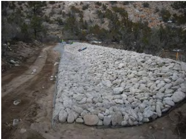
Photo 3 Class A rip-rap armoring of earthen berm, upstream face of berm
