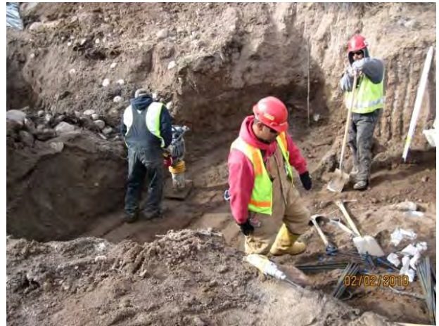
Photo 2 Headwall subgrade compaction
