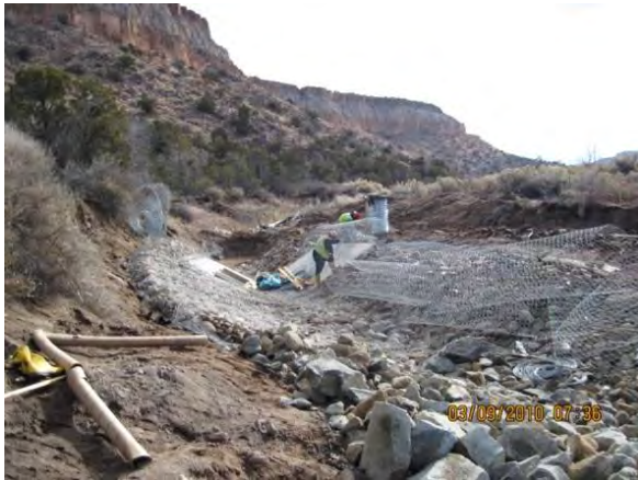
Photo 1 Gage station/flume rip-rap installation
