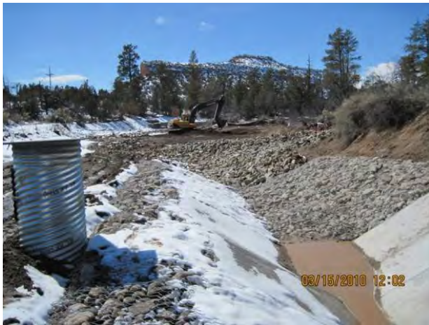
Photo 3 Flume and stilling well
