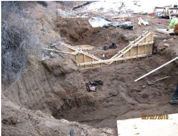
Photo 7 Headwall subgrade compaction
