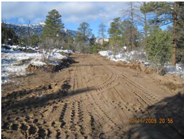
Photo 5 Grading of permanent access road
