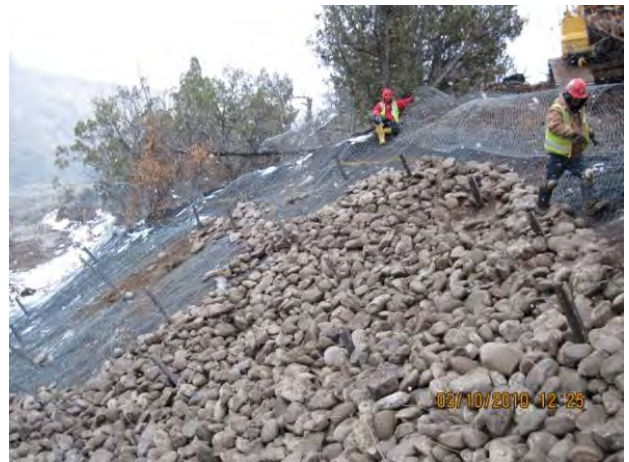
Photo 4 Class A rip-rap placement, south slope downgradient of structure
