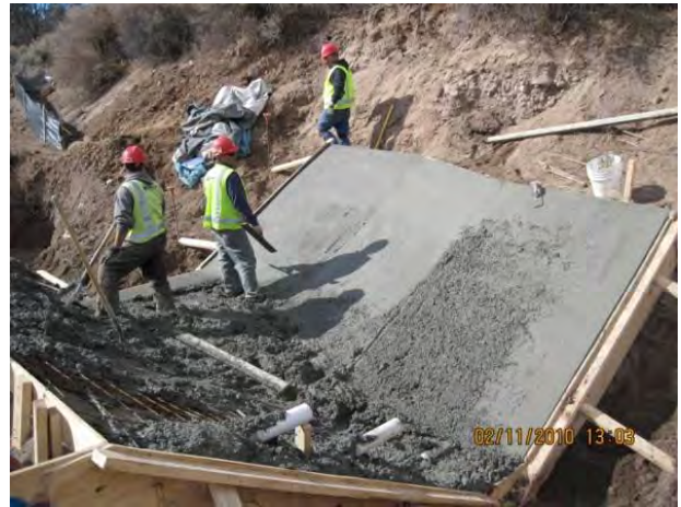
Photo 8 Concrete finishing of flume
