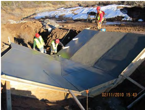
Photo 13 Concrete finishing of flume
