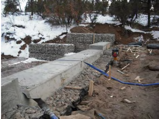
Photo 1 Concrete weir cap (low-flow and overflow weir)
