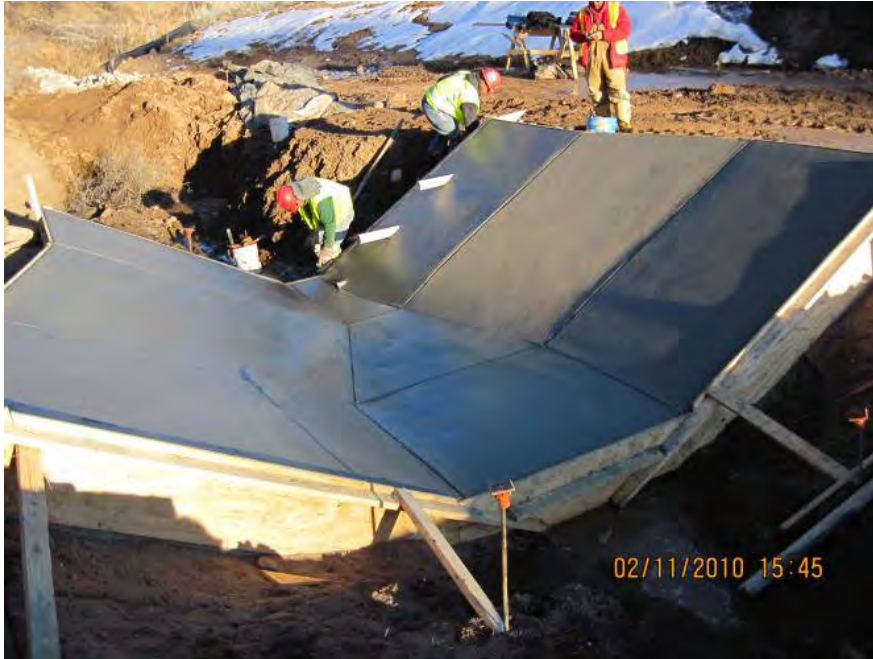
Figure 2.1-7 E060.1 stream-gage flume during construction
