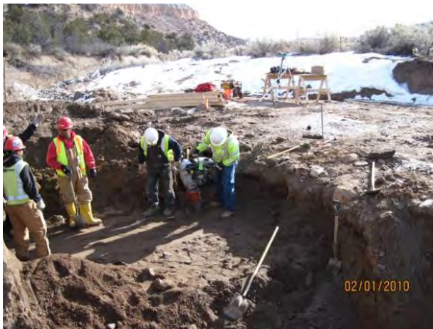
Photo 15 Headwall subgrade compaction
