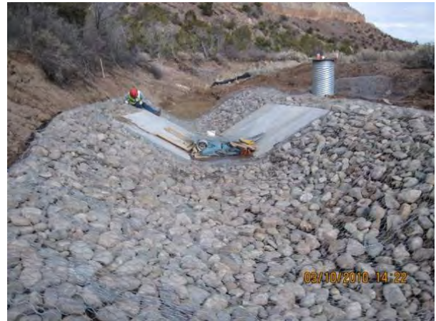
Photo 8 Working on Class A rip-rap exit from flume
