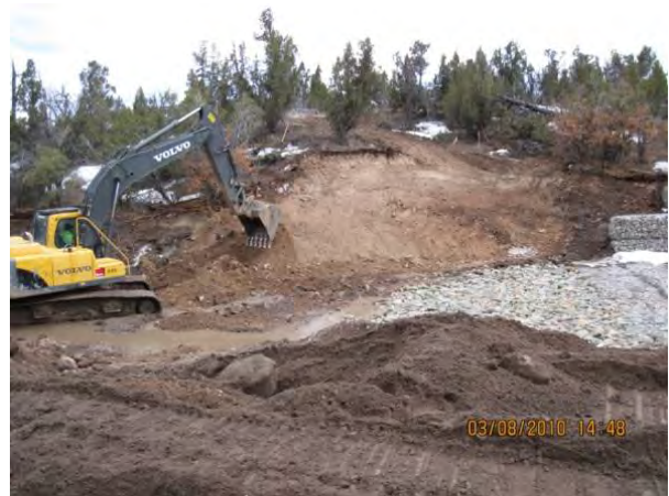
Photo 6 Preparing south downgradient slope for Class A rip-rap armoring
