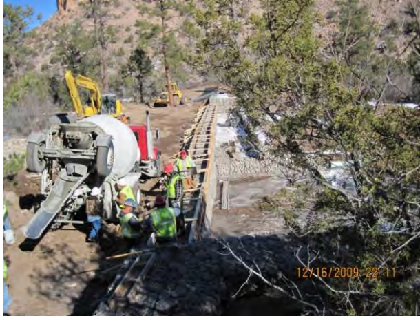
Photo 5 Concrete placement, low-flow and overflow weir
