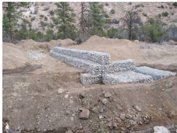
Photo 16 Gabion structure upstream, looking northeast at stilling basin and overflow weir
