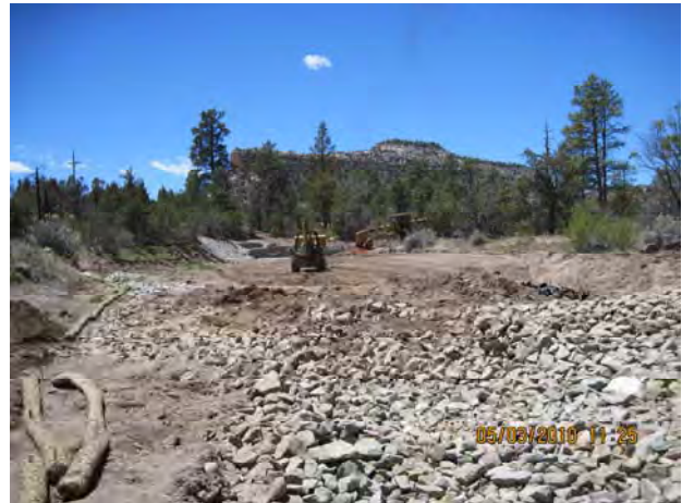
Photo 2 Flume Class B rip-rap installation looking upstream from flume
