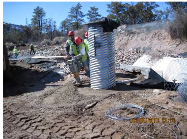
Photo 2 Stream gage stilling-well installation, compaction around well
