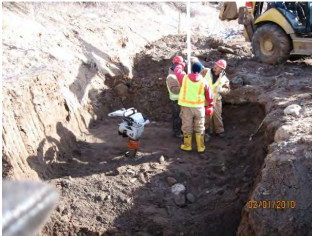
Photo 13 Headwall subgrade compaction
