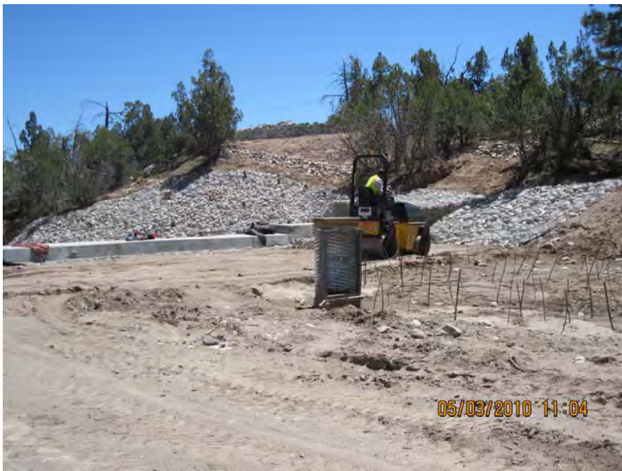
Figure 2.1-6 Riser pipe after extension
