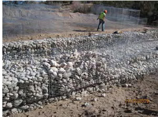
Photo 12 Close-up view of gabion baskets
