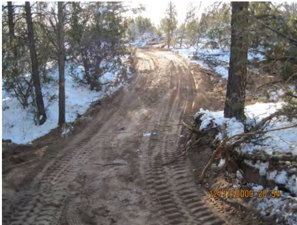
Photo 1 Grading of permanent access road
