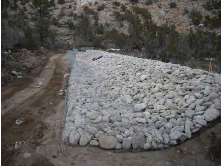
Figure 2.1-5 Class A armored earthen berm upon completion (looking north)
