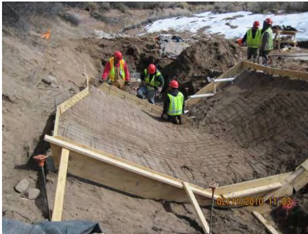
Photo 1 Wire mesh reinforcement for flume
