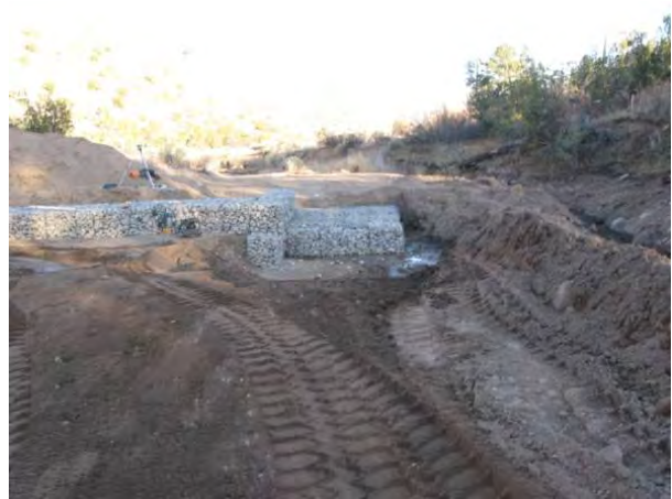
Photo 8 Gabion structure, looking downgradient at stilling-basin subgrade
