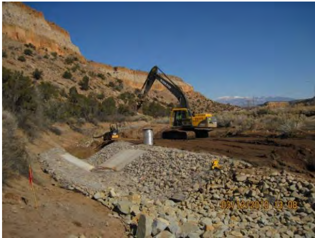
Photo 5 Grading and compacting area south of flume
