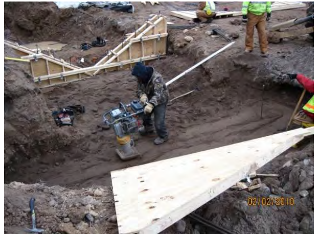
Photo 8 Headwall subgrade compaction
