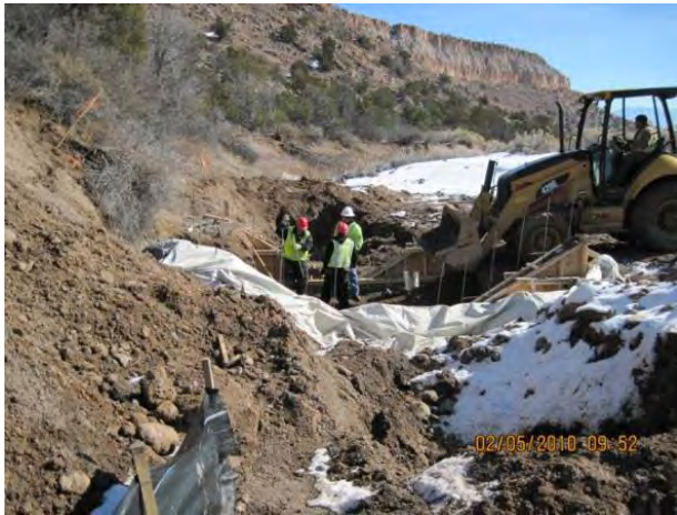
Photo 7 Flume headwall concrete placement
