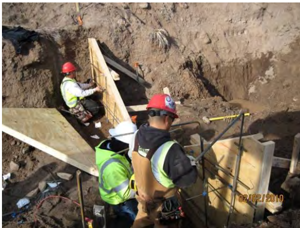
Photo 5 Headwall form work
