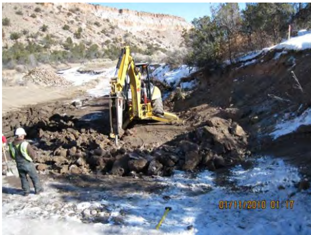
Photo 1 Excavation for installation of Class B rip-rap armoring, downstream side of structure stilling basin
