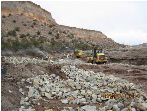
Photo 7 Downstream of structure, looking at gage station rip-rap installation
