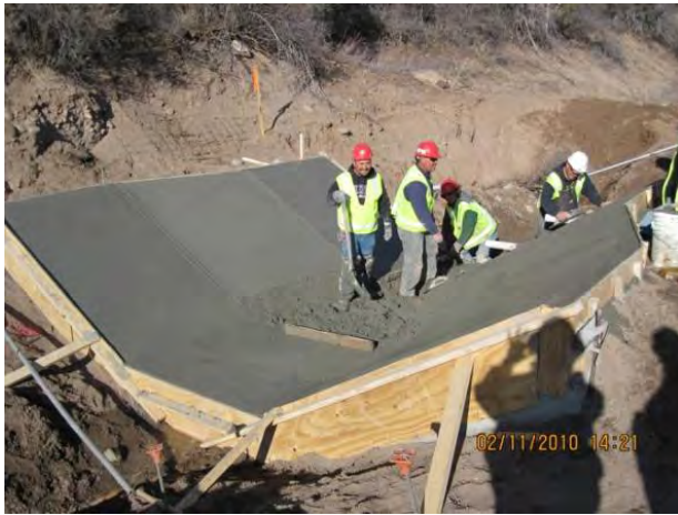
Photo 11 Concrete finishing of flume
