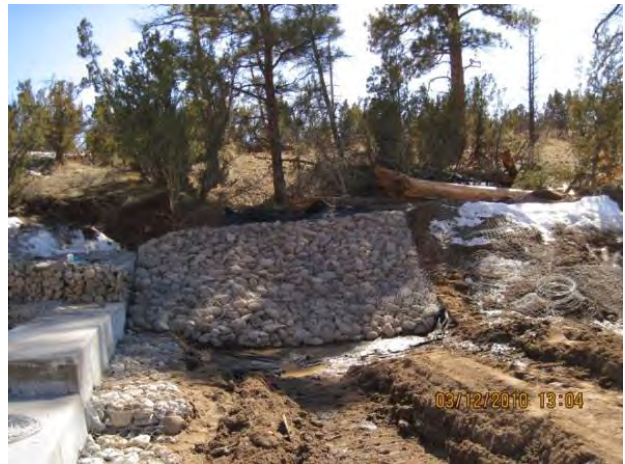
Photo 4 Class A rip-rap armoring of south slope on upstream side of structure
