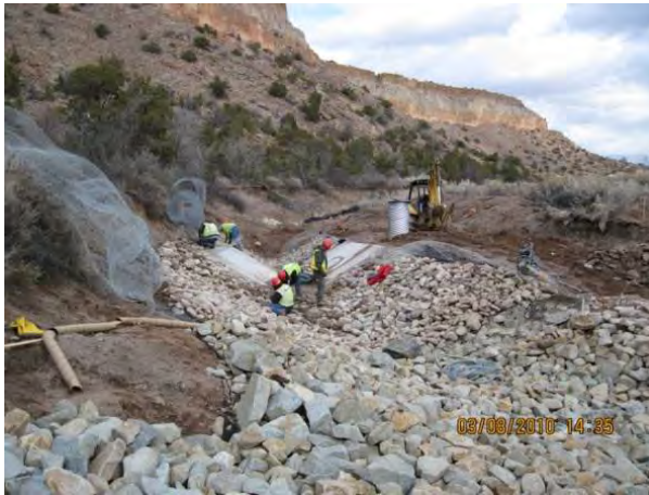
Photo 5 Installing Class A rip rap
