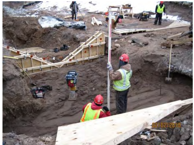
Photo 10 Headwall form work
