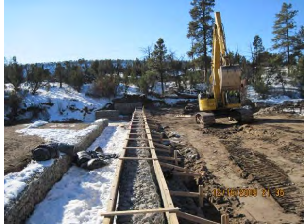
Photo 2 Forms for concrete cap
