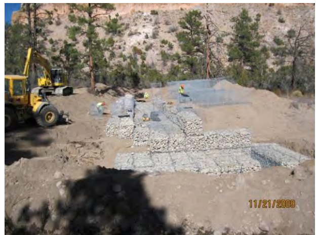
Photo 8 Structure looking north, gabion assembly
